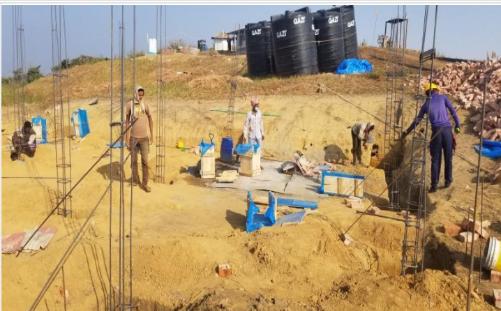
Shuttering fitting work for short column on 17-01-21
