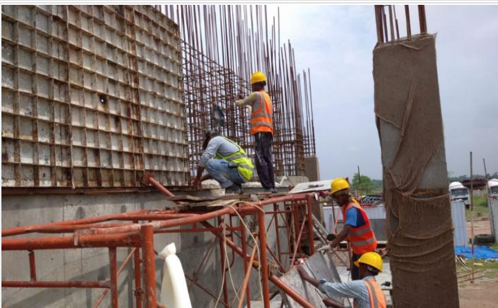
Ground Floor Lift Core Shuttering on 15-06-21
