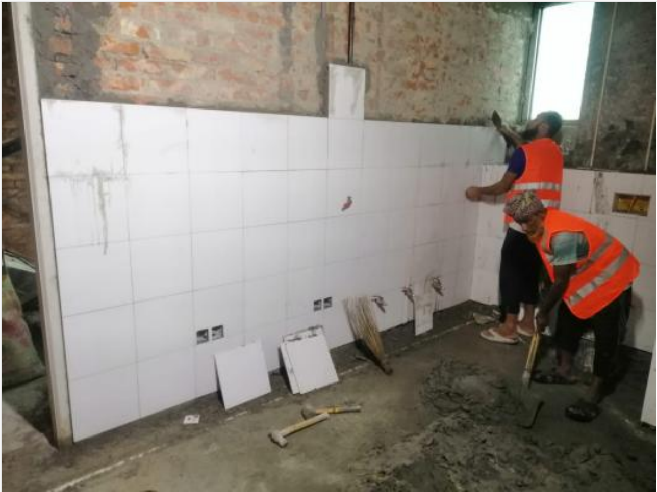
14th Floor-Kitchen Tile Fixing on 30-06-24
