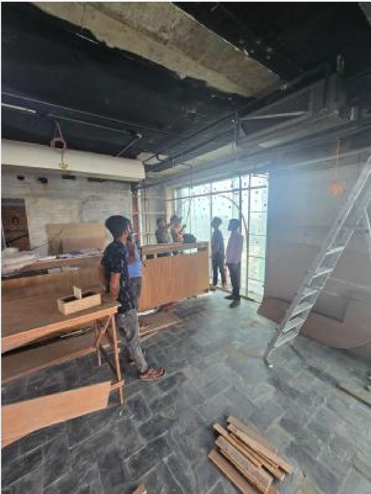
14th Floor Interior Works on 09-07-24
