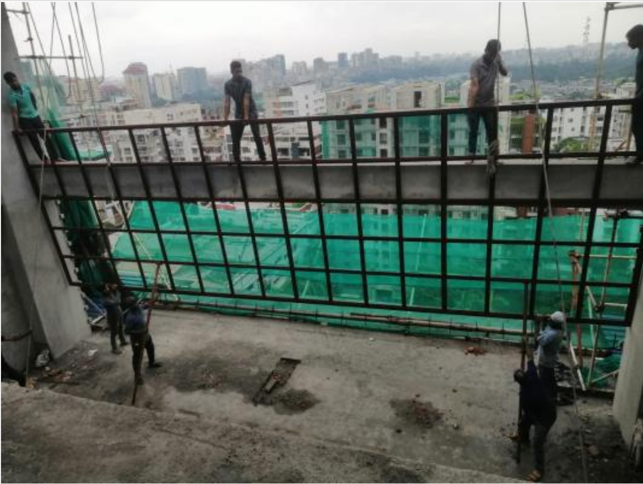
15th Floor-Double Height Grill Fixing on 30-06-24
