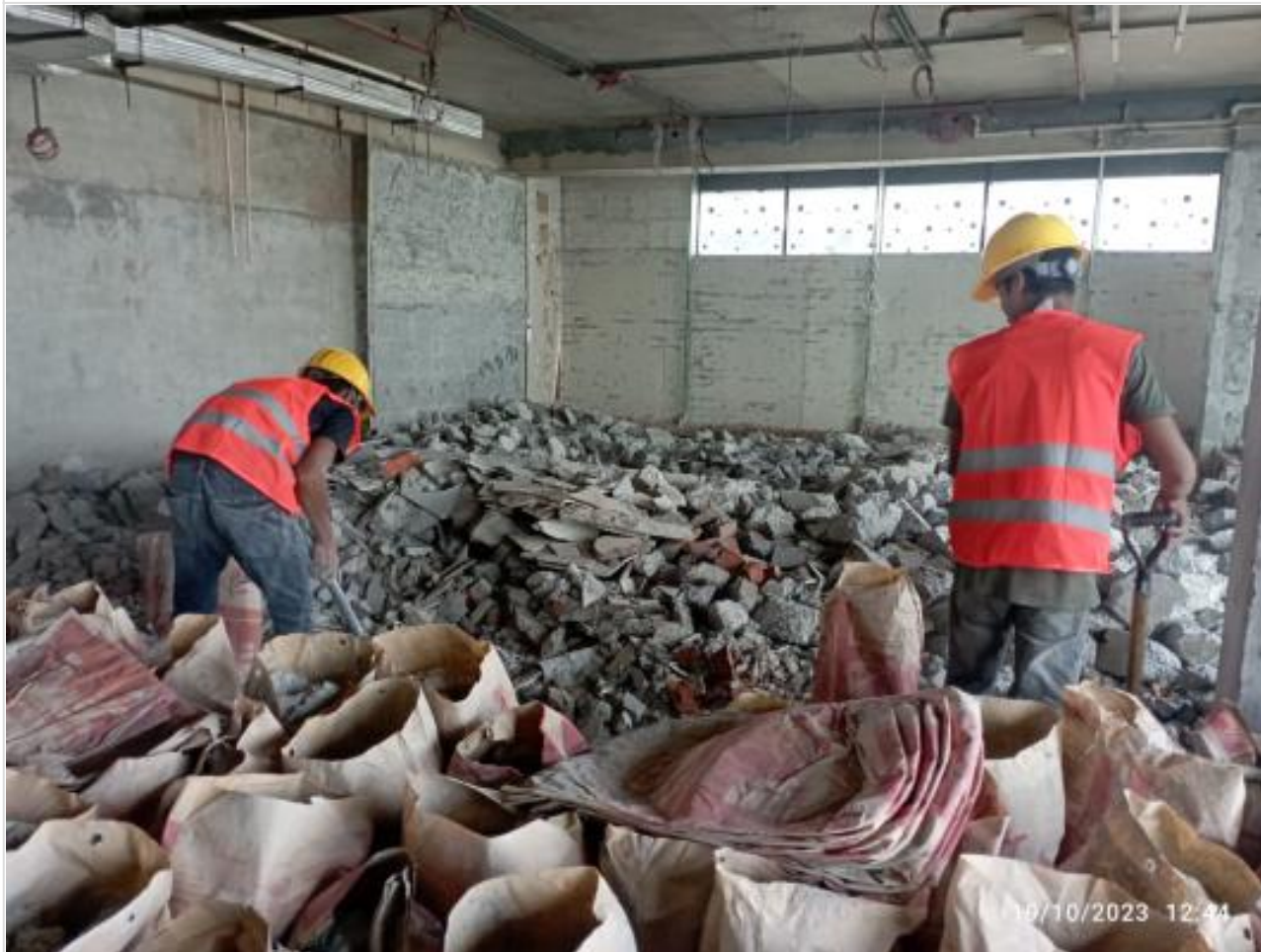
L-14-Kitcjen-Floor Dismantling on 19-10-23
