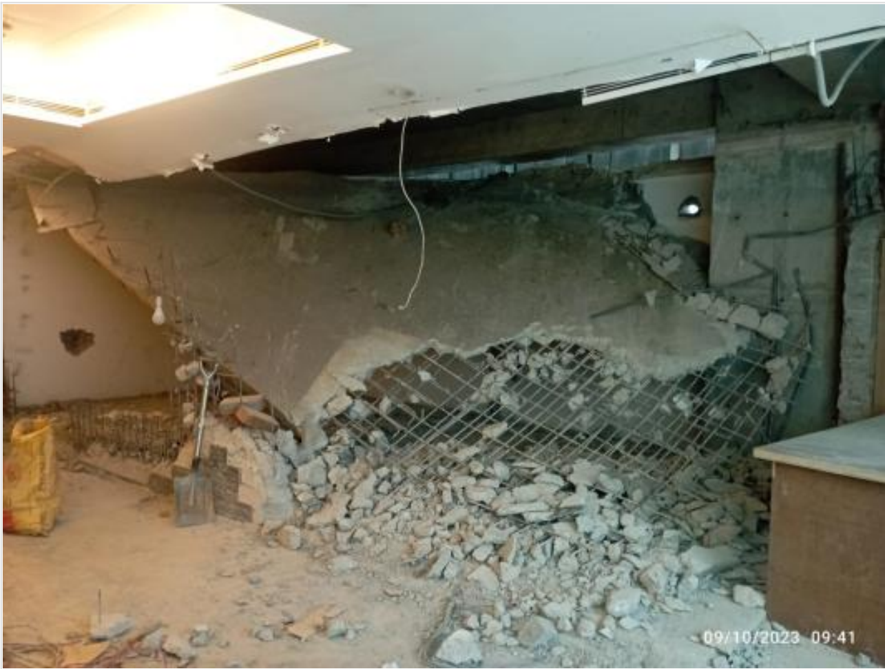
L-4-North-East Vault dismantling on 08-10-23
