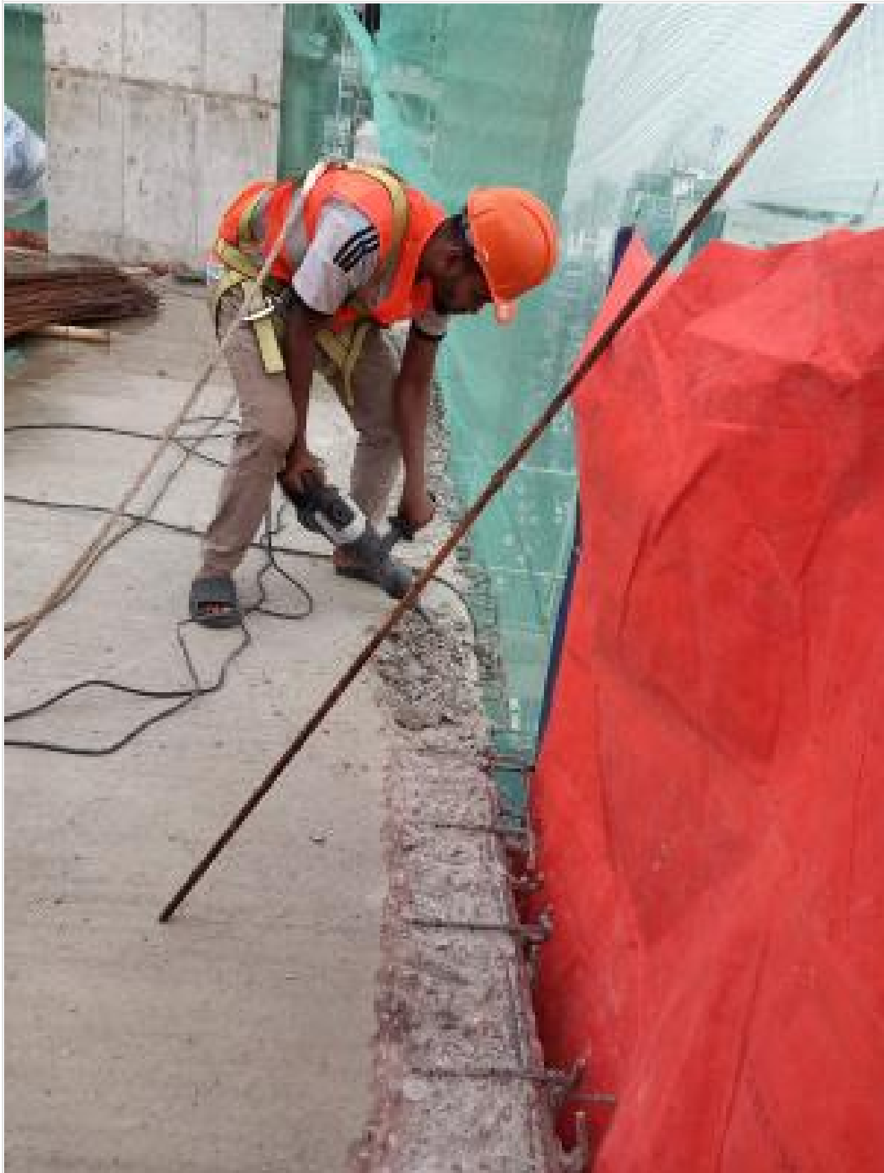
L-16-Dropwall old concrete dismantling on 29-03-23
