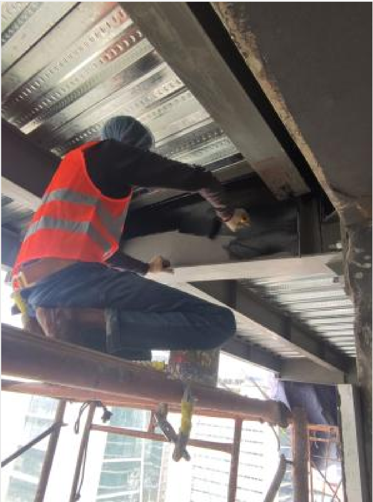
L-14-Ext Decking and Beam Painting on 27-02-23
