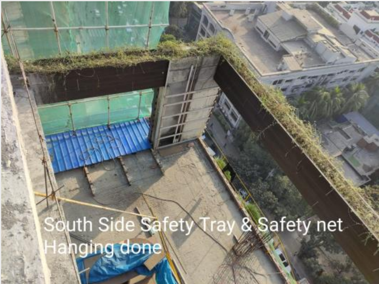
South-side safety tray & net complete on 02-02-23
