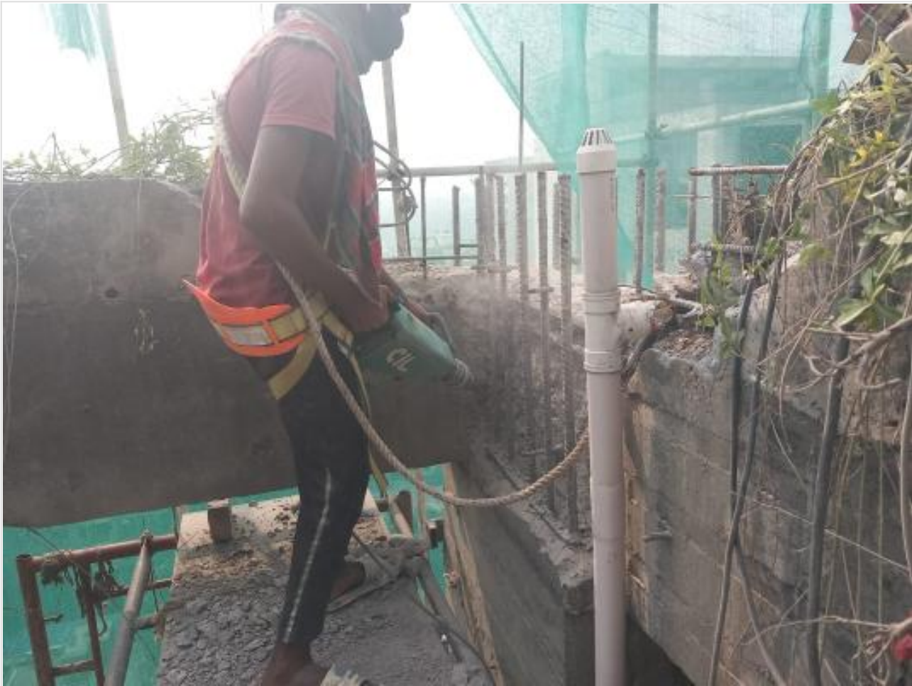
L-16-Old concrete removing on 22-03-23
