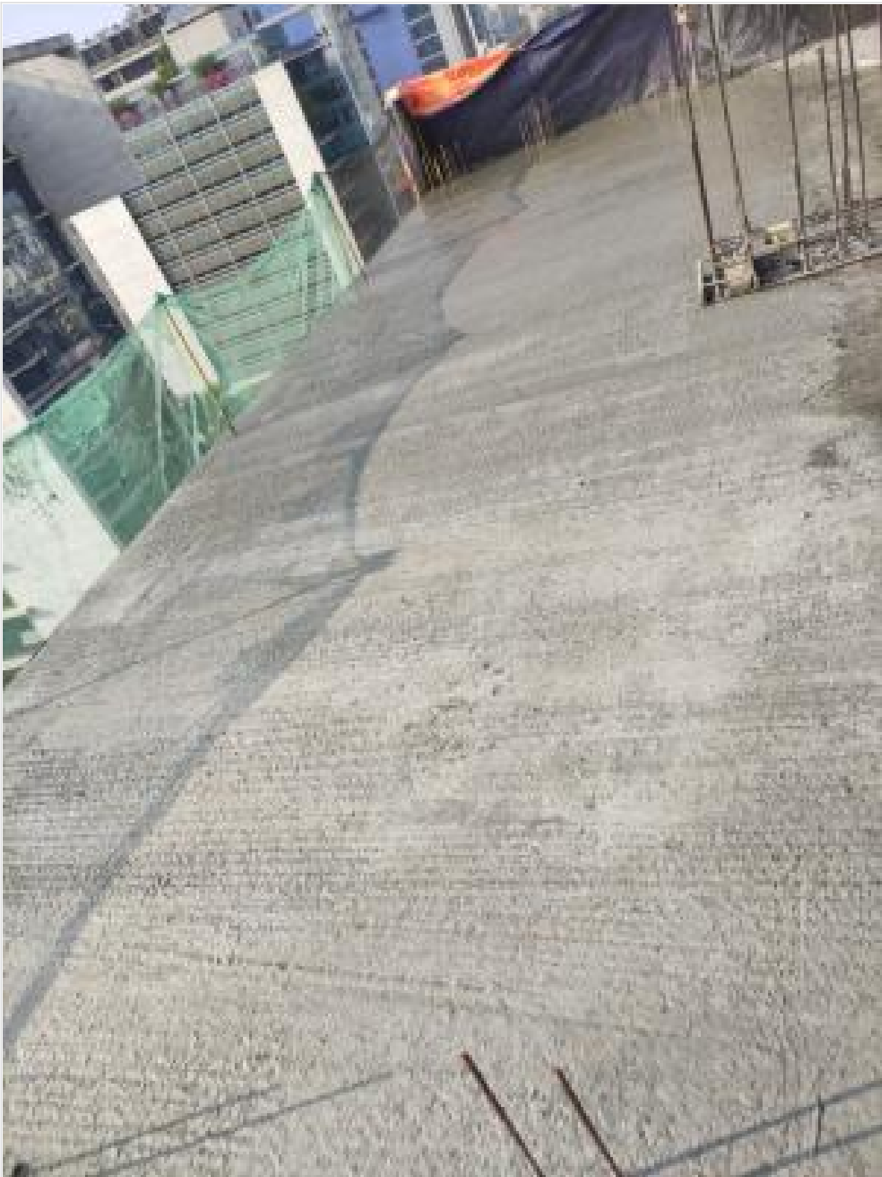
Level-15-Ext Slab Concreting on 25-02-23
