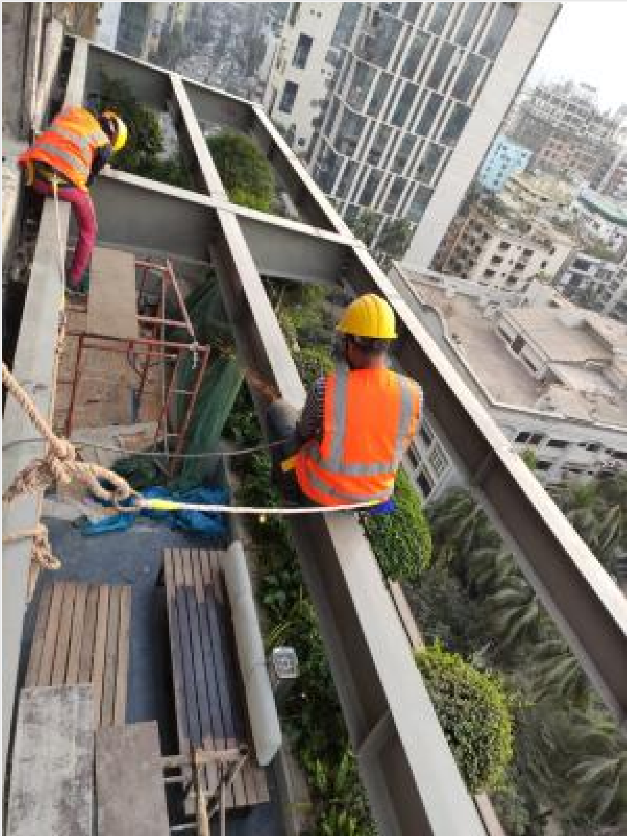
Level-14-Steel Work on 08-02-23
