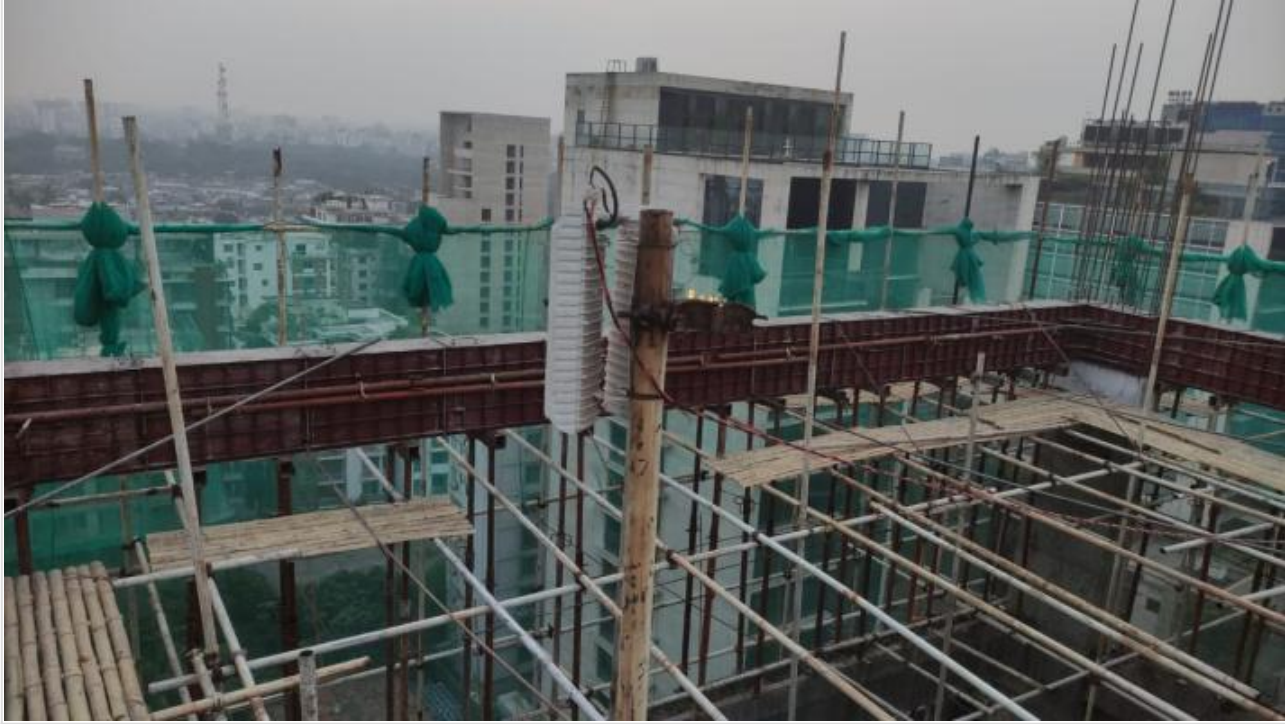
L-16-Beam concreting complete on 19-04-23
