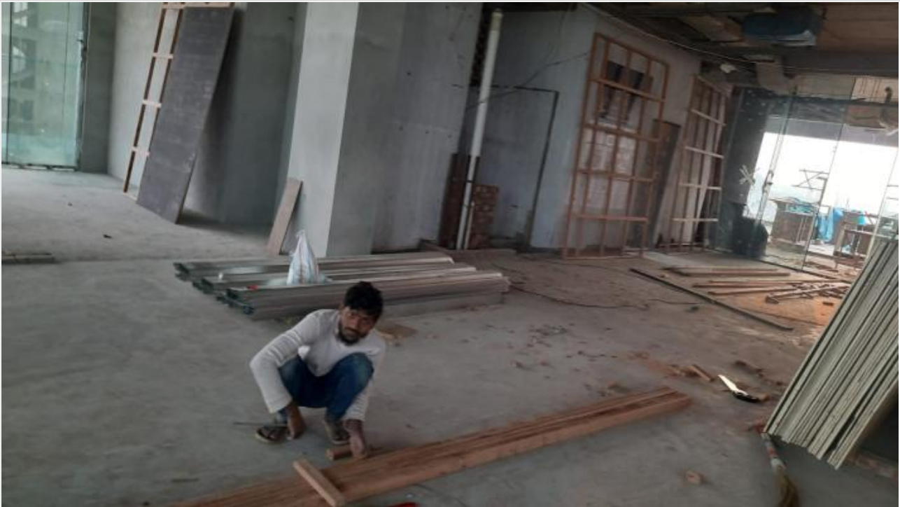
Wall Paneling on 08-02-23
