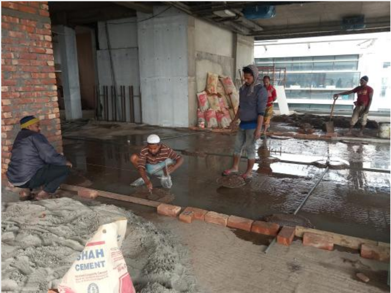
Floor Finishing-NCF on 03-01-23
