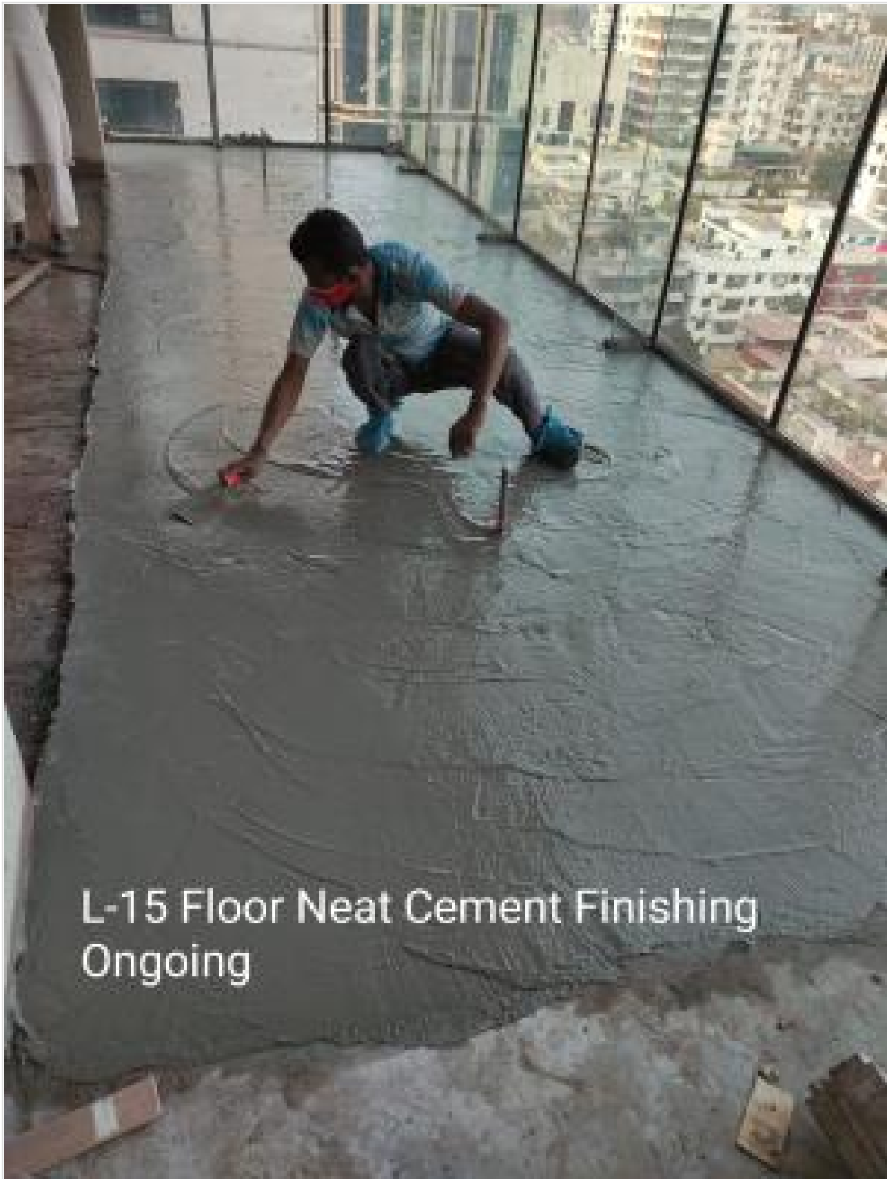
L-15-Floor Neat Cement Finishing on 12-02-23
