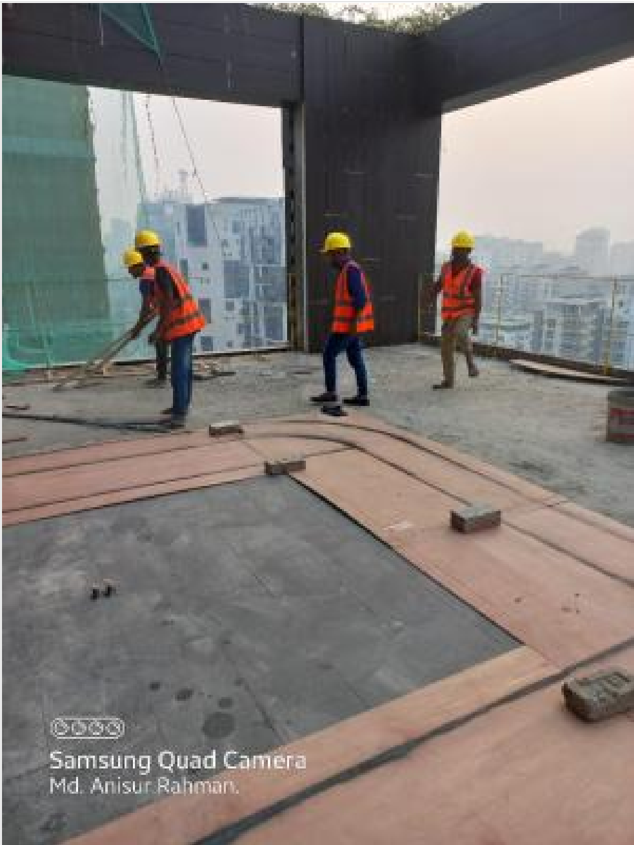
Carpentry Mock-up on 22-12-22
