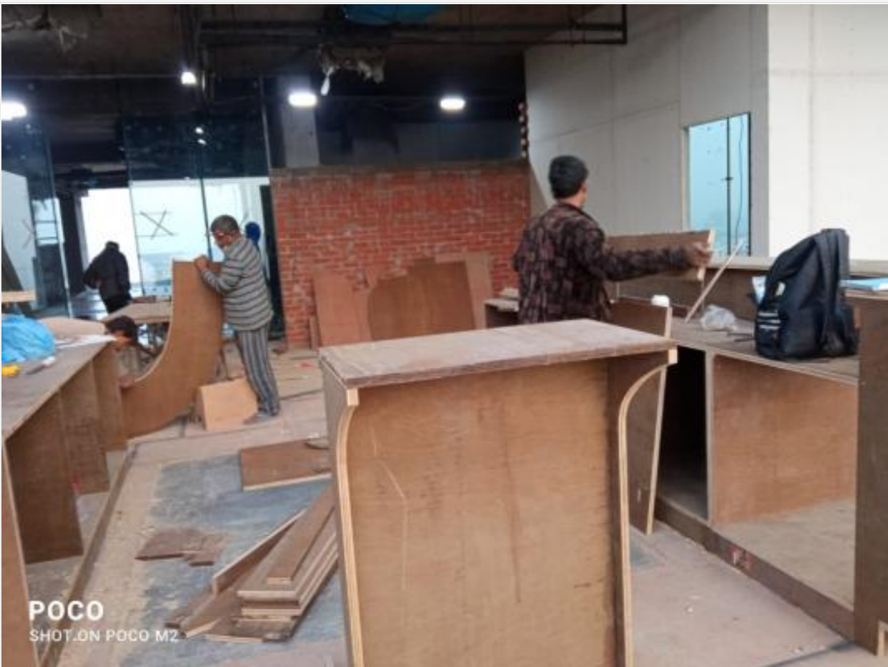
Interior works on 03-01-23
