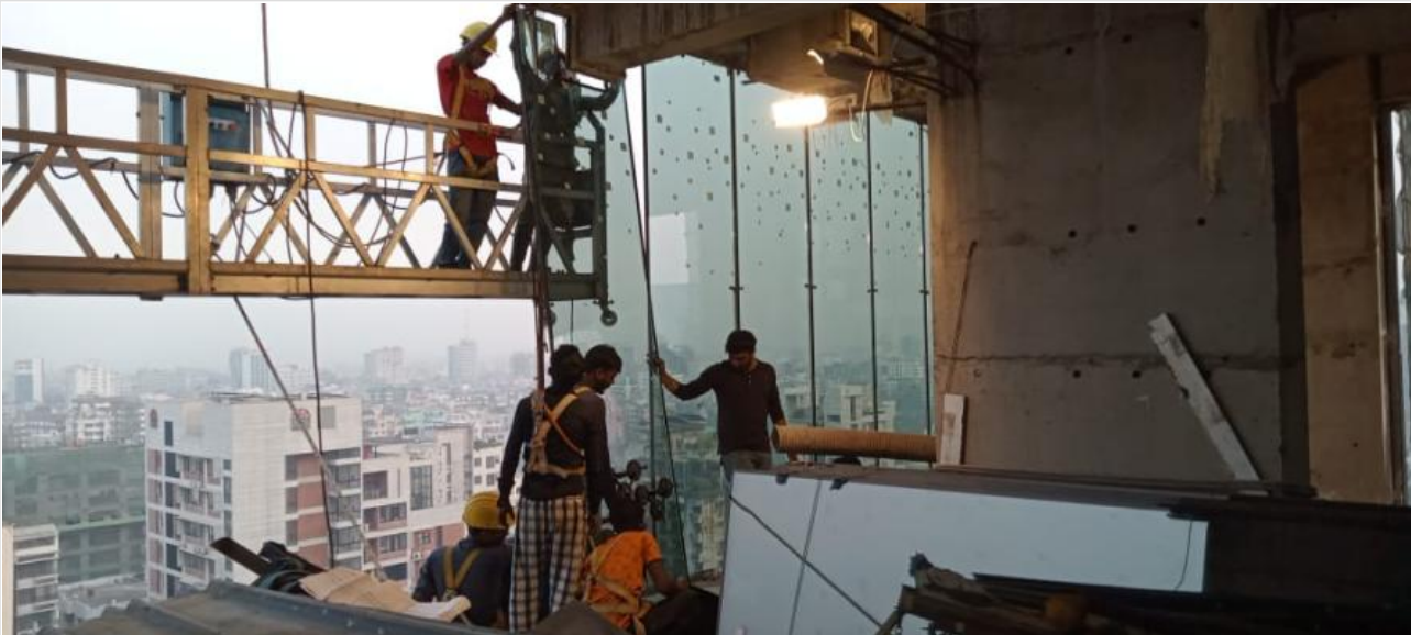
Fixing Glass on 09-01-23
