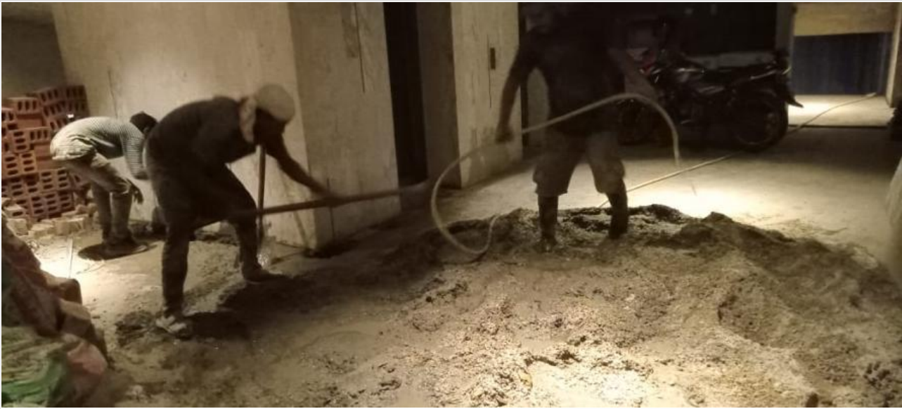
Basement-3 Lift-wall Concreting on 09-01-23
