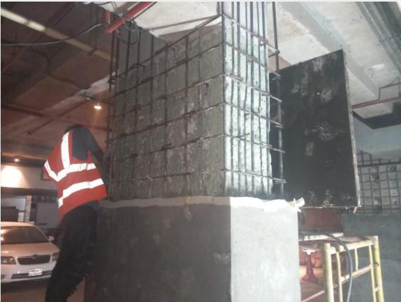
B-1-Column retrofit re-bar work on 09-03-23
