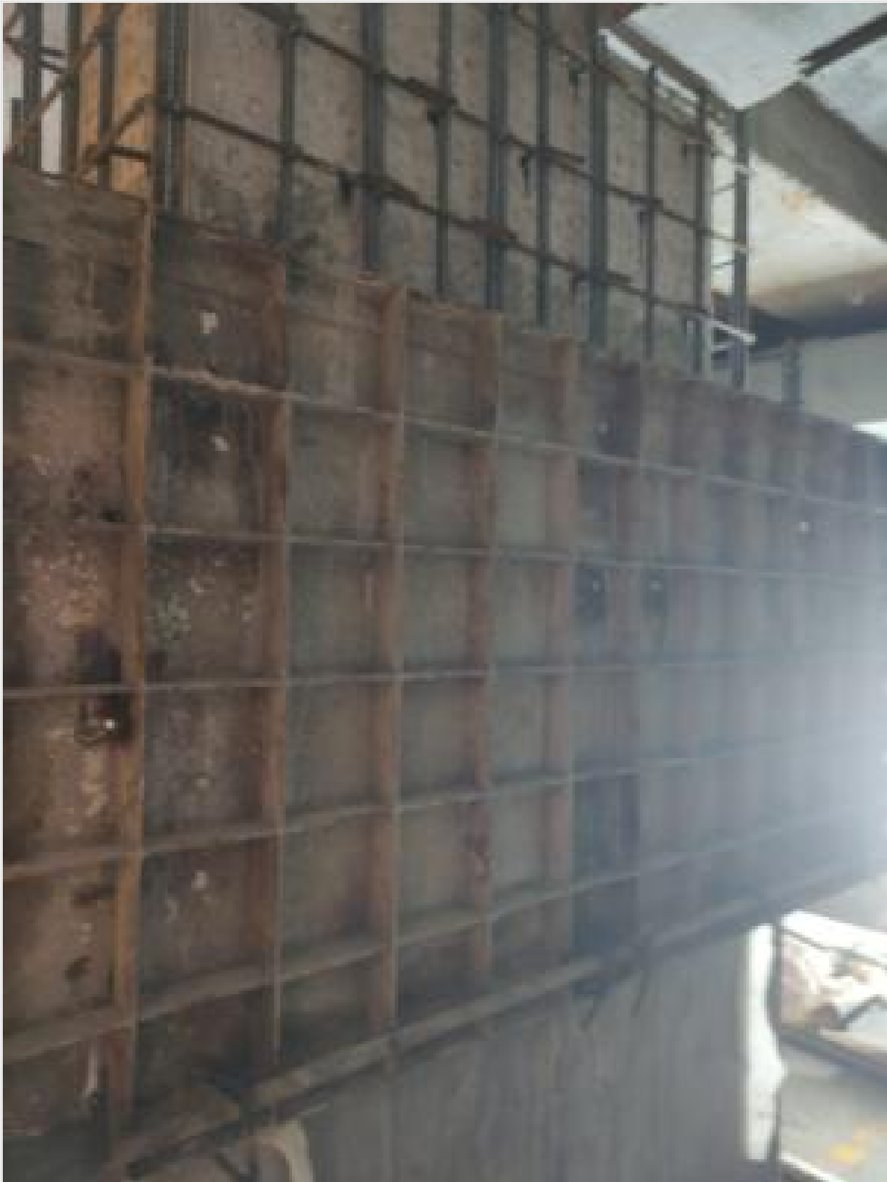
Retrofit-B-2 Column Shuttering on 27-02-23
