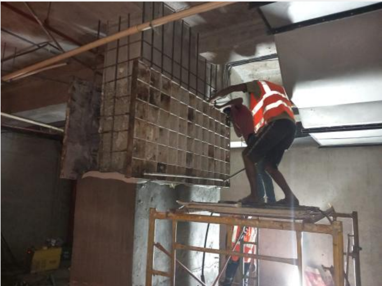
B-1-Column retrofit re-bar work on 09-03-23
