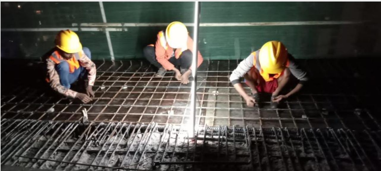
L-17 Slab Extension Re-bar Work on 22-12-22
