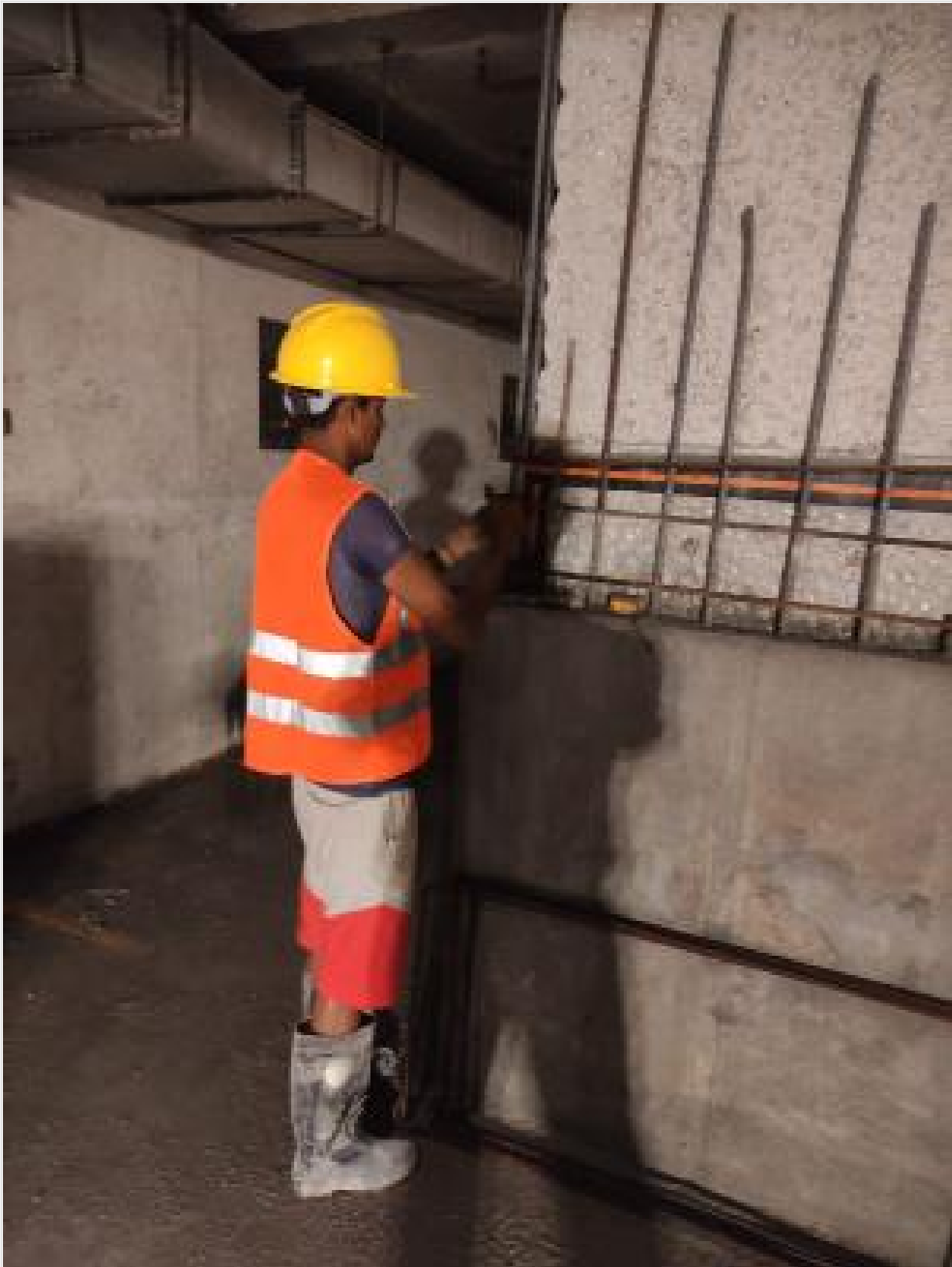
B2-Col Retrofit re-bar work on 20-02-23
