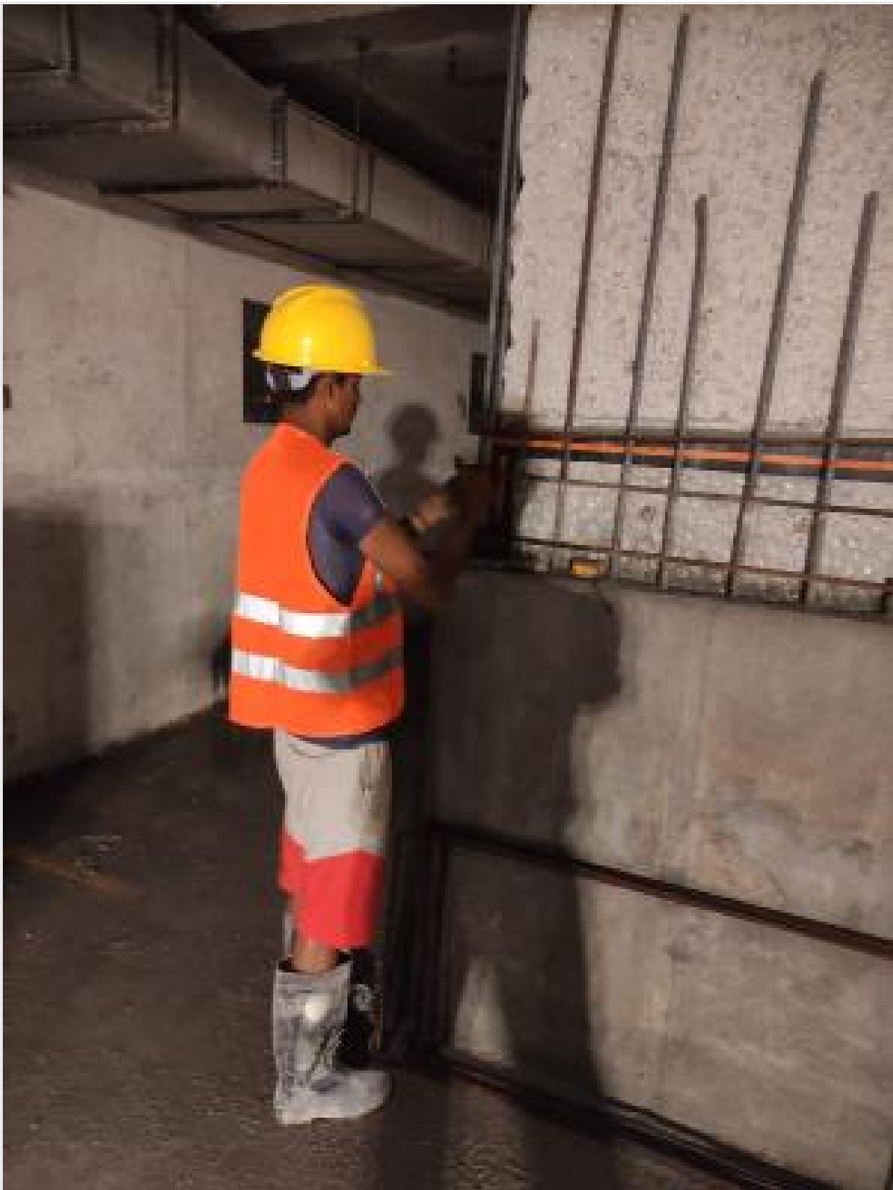
B-2 Col retrofit re-bar work on 20-02-23
