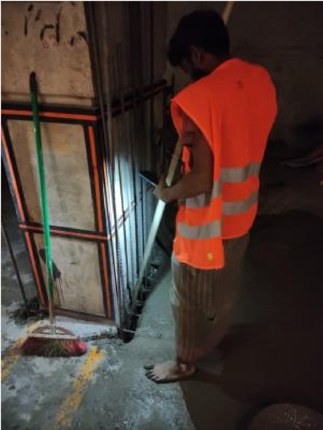
B-2-Column Retrofitting on 01-03-23
