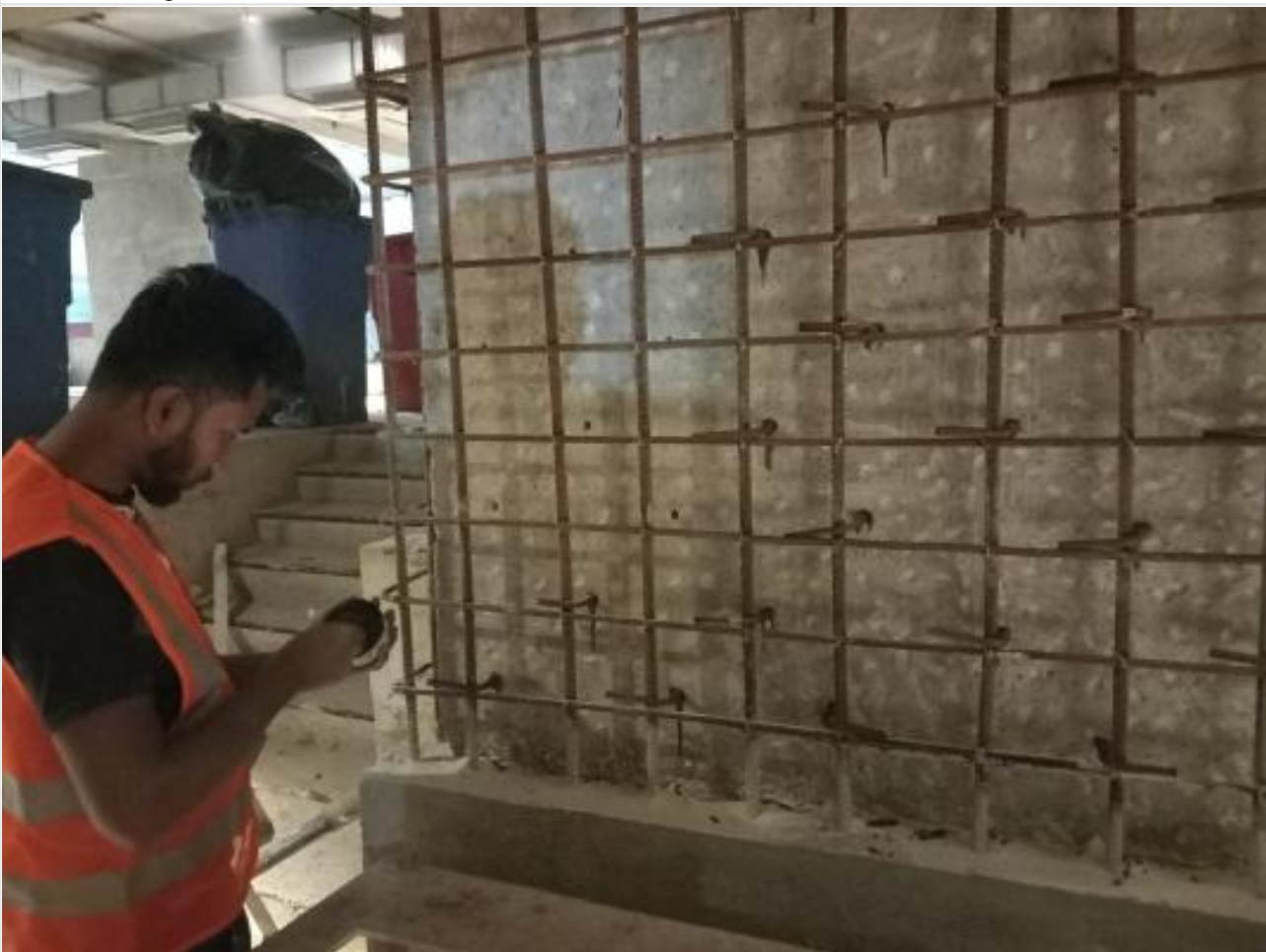
Shear Wall Retro. on 05-02-23
