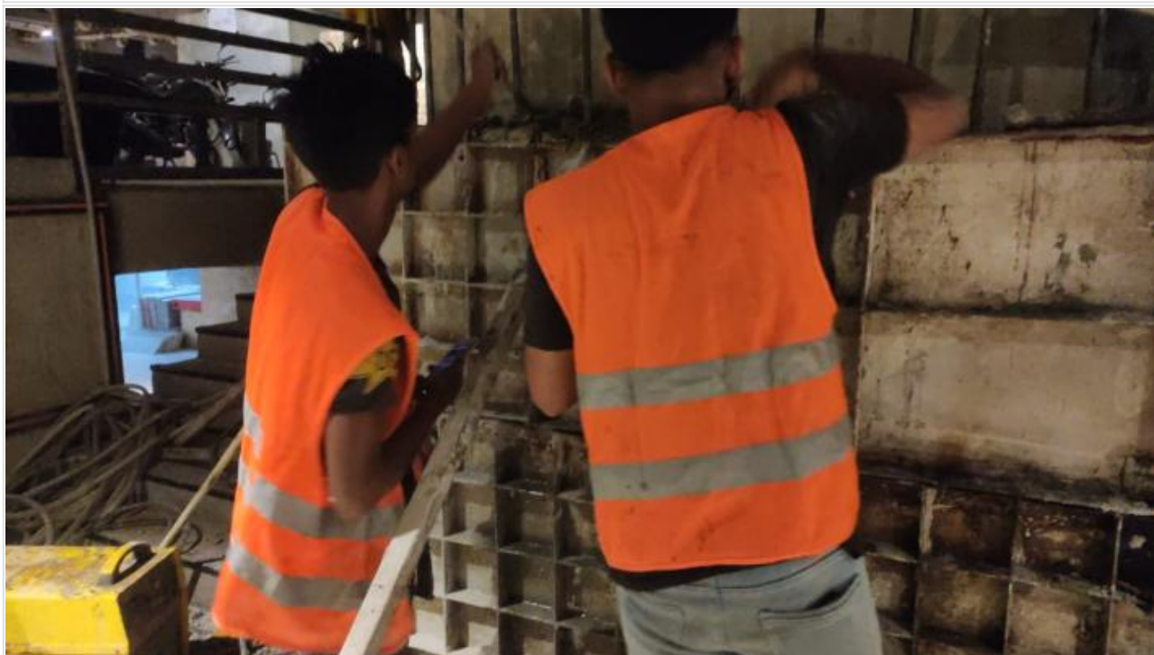
B-2-Column Retrofit shutter removing on 27-03-23
