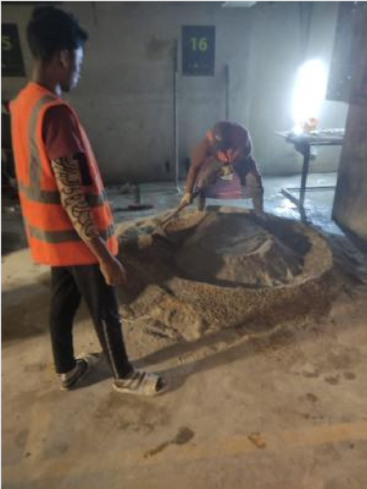
Retrofit-B2-Column Concrete on 27-02-23
