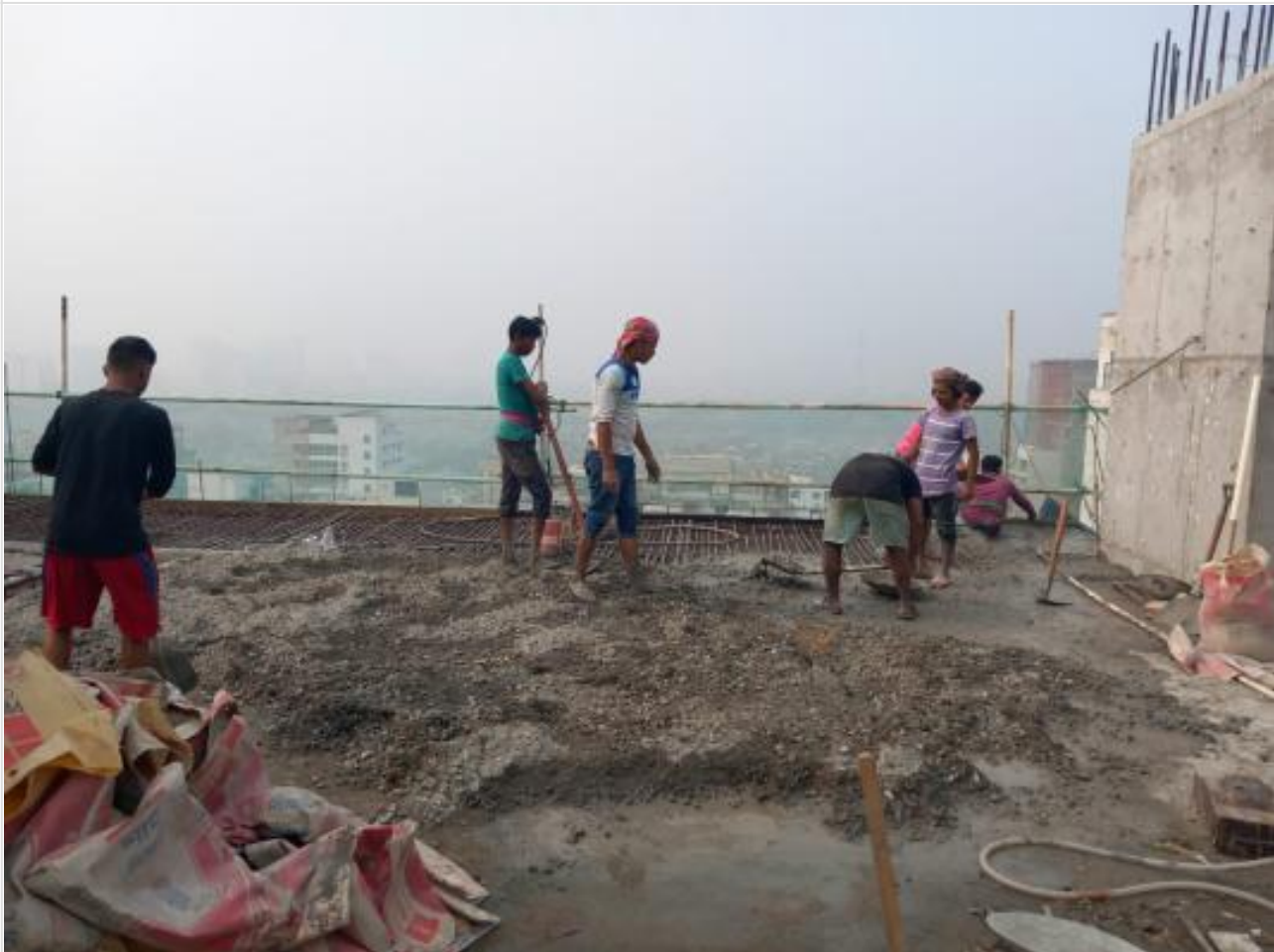
Level-17-Slab Extn Concreting on 28-12-22
