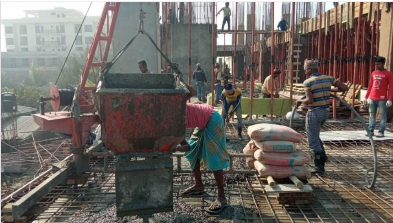
Tower-1-GF Roof Slab-4250sft Concreting on 27-01-21
