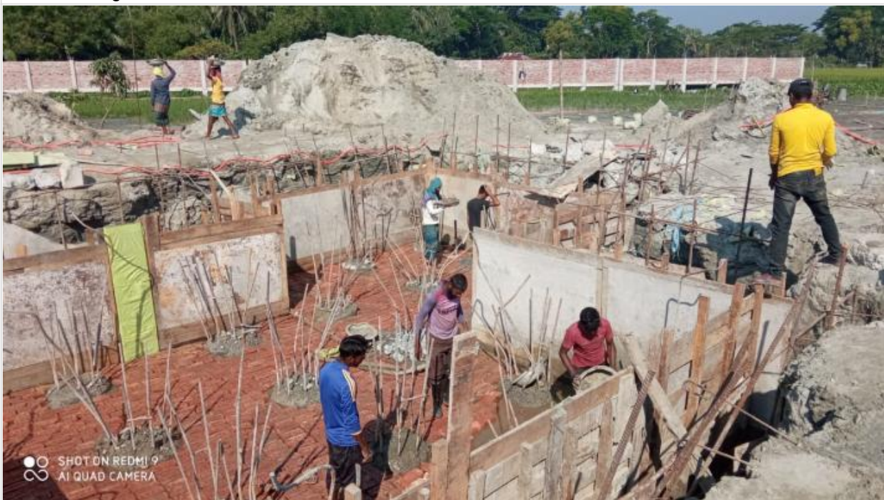
Tower-1-Pile Cap Work on 28-11-20
