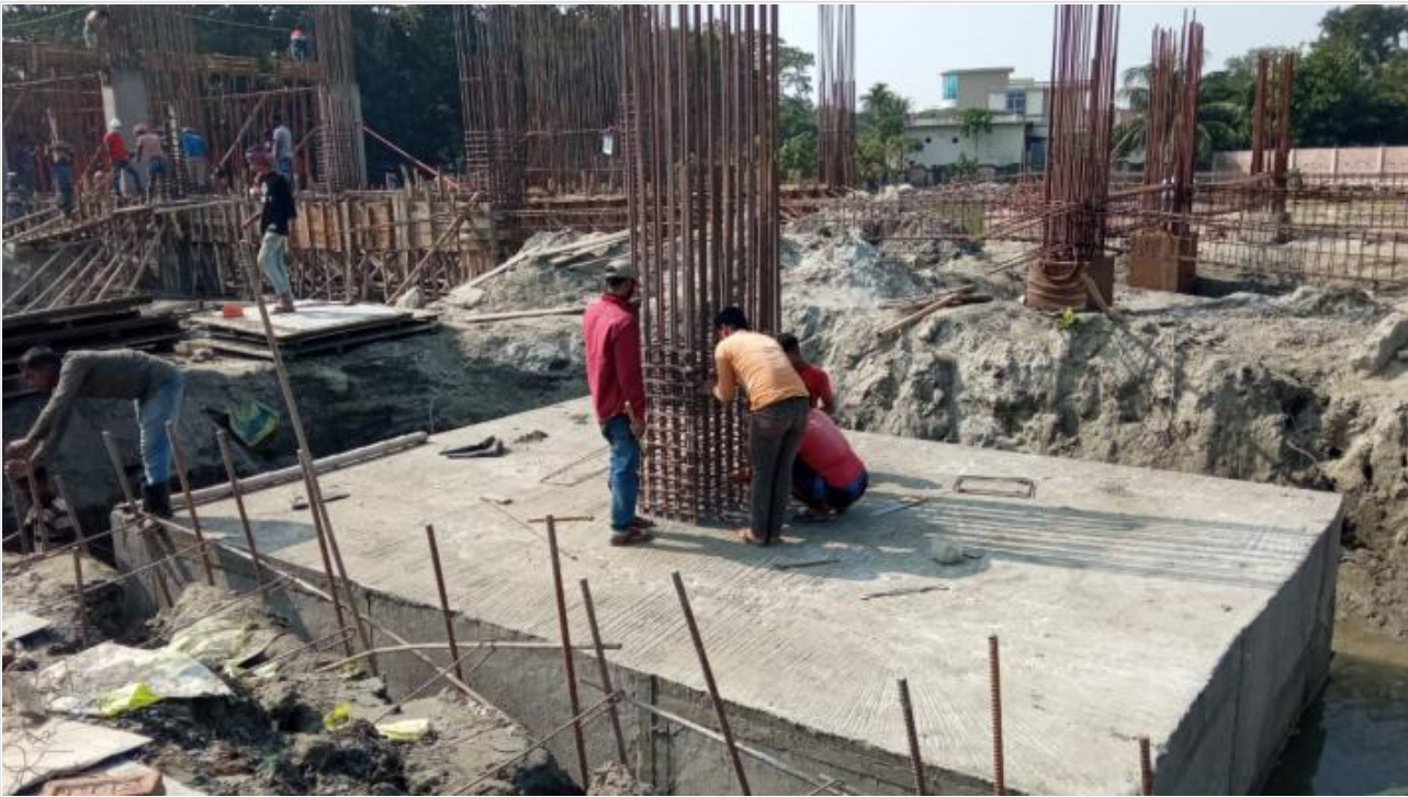
Tower-1-Coliumn Re-bar work on 15-12-20
