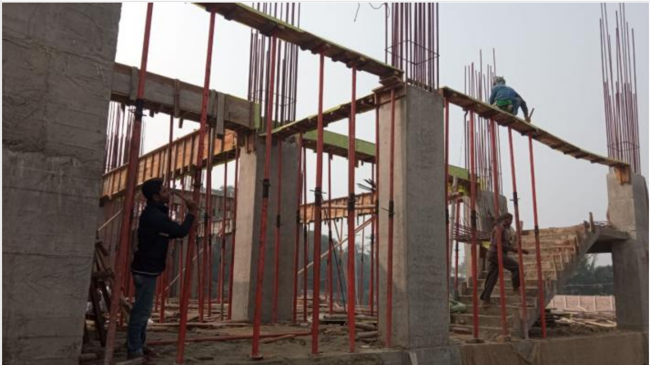
Tower-1-1st Floor Roof Beam Shuttering on 18-01-21
