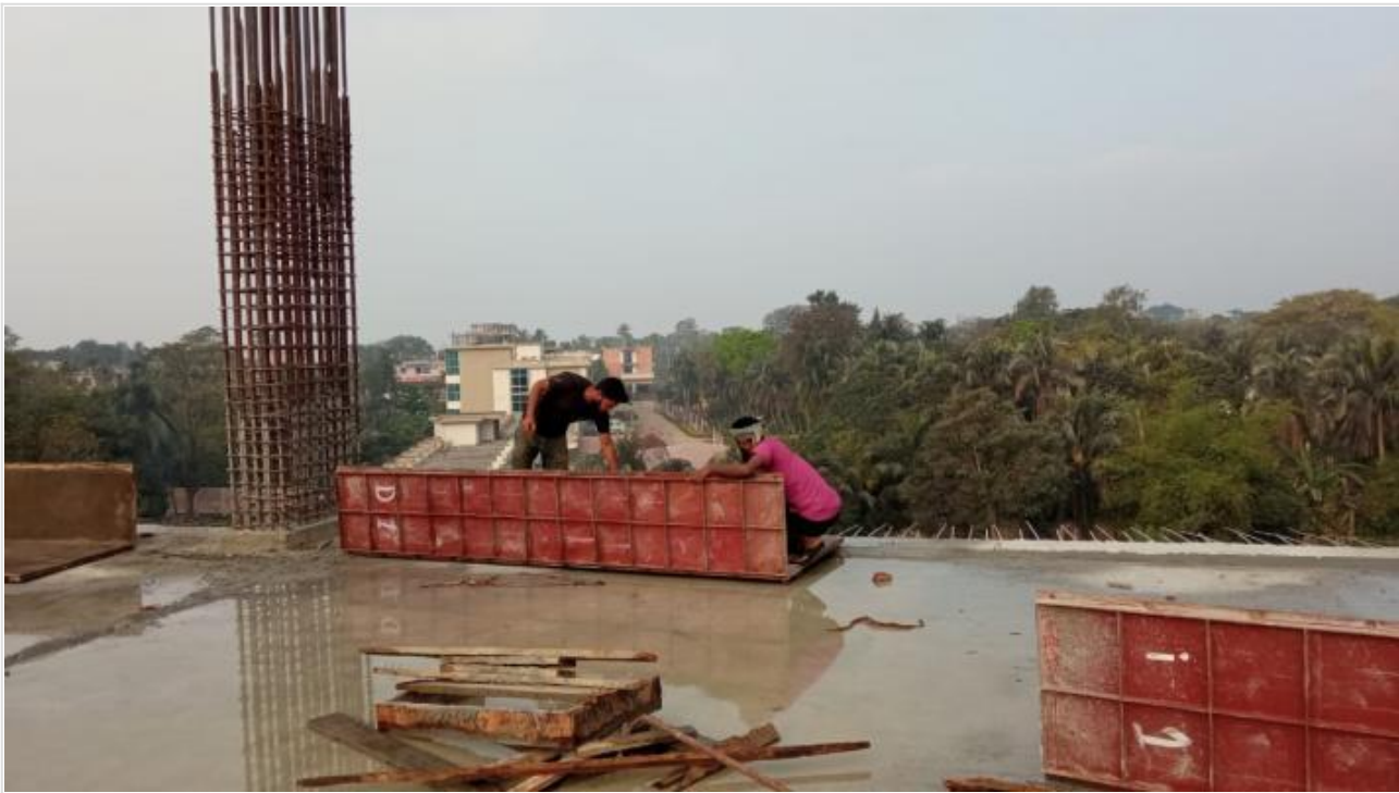
Tower-1-3rd Floor Column Shuttering on 28-02-21
