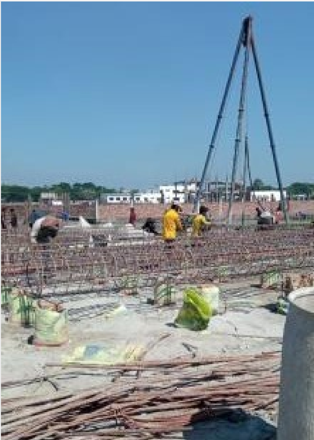
Tower-2-Pile Work on 12-11-20
