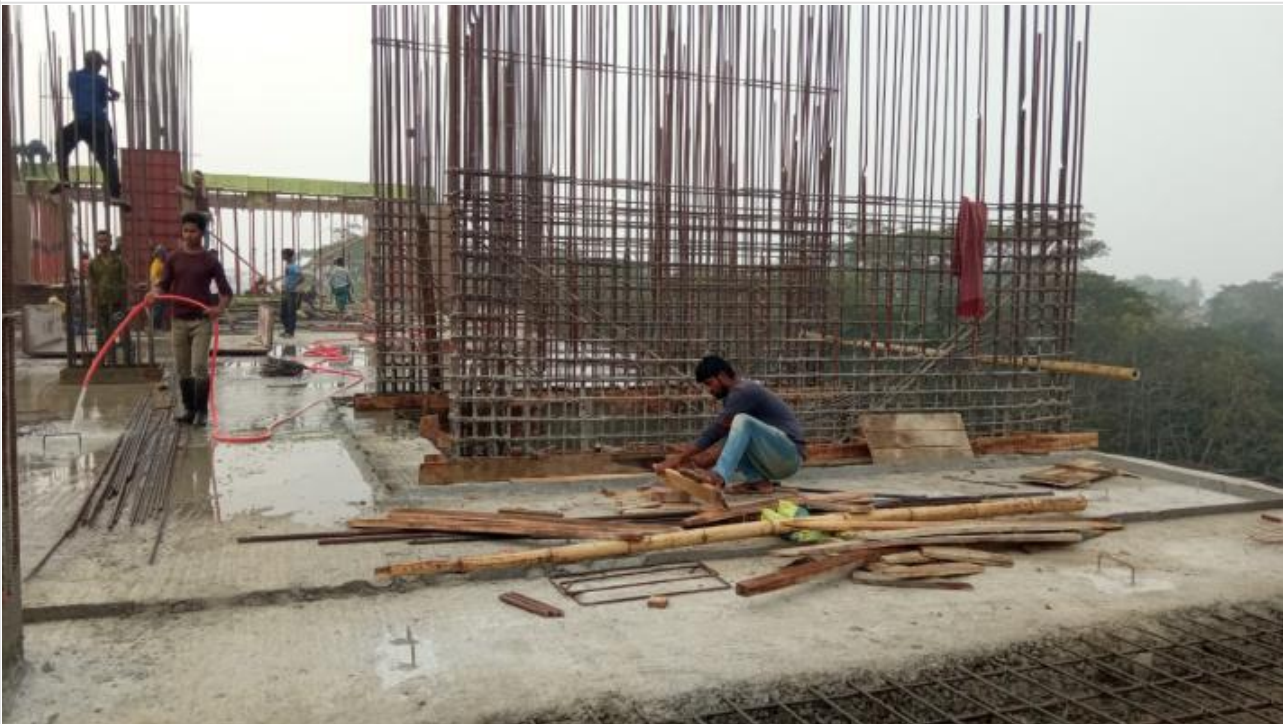
Tower-1-2nd Floor Roof Curing on 25-02-21
