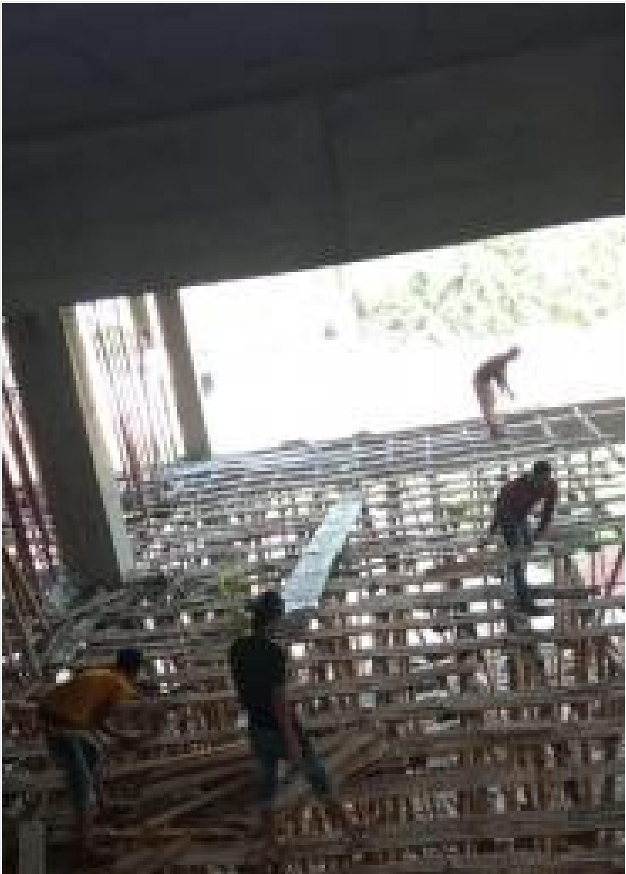
Roof Slab Shuttering on 02-05-21
