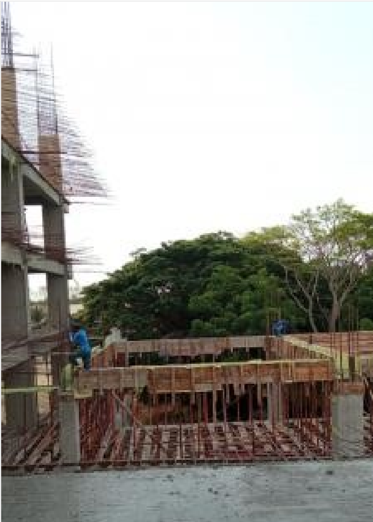
Tower-2-Gr.Flr Roof Slab(5a-6/H-J) Concr on 12-04-21
