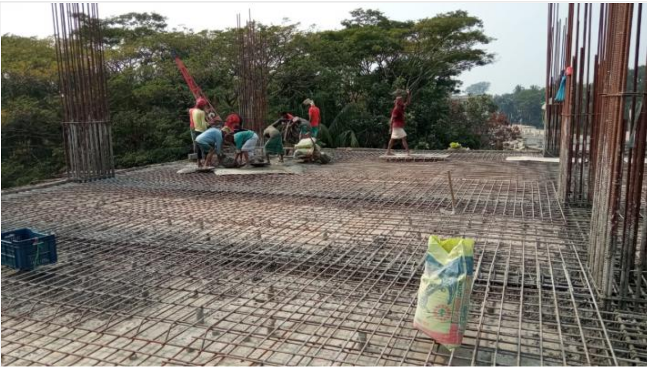
Tower-1-1st Floor Roof Slab 3600 sft Co on 11-01-21
