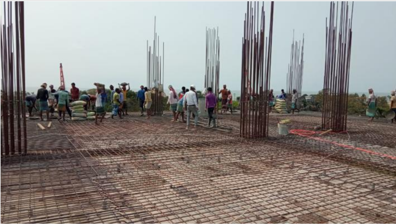
Tower-1-3rd Floor Roof Slab Concreting on 11-03-21
