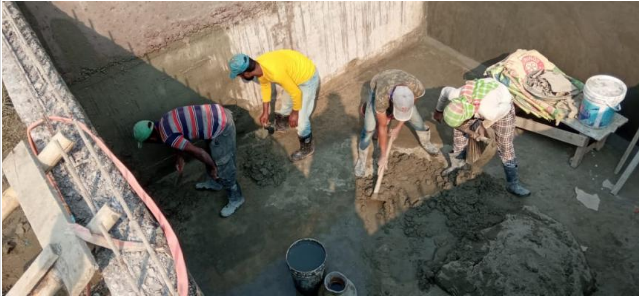
East Septic Tank Plastering on 01-02-22
