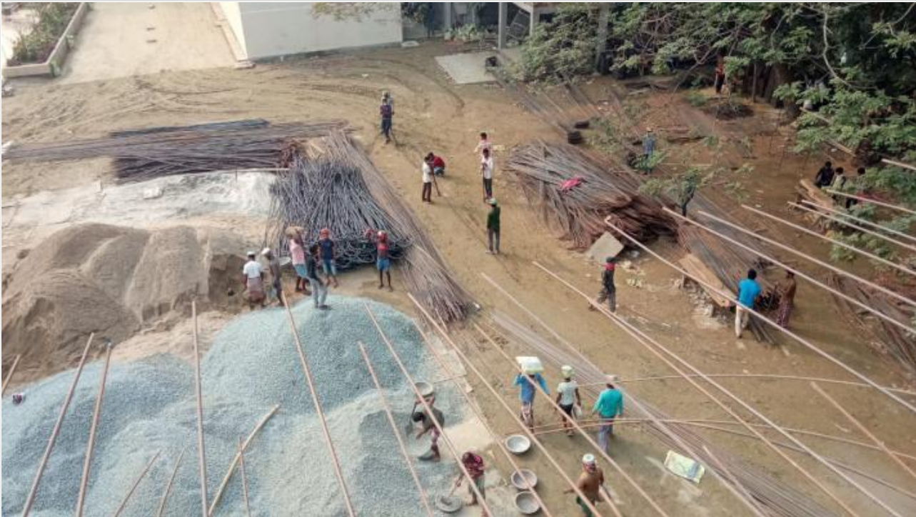
Tower-1-1st Floor Roof Slab Concreting on 11-01-21
