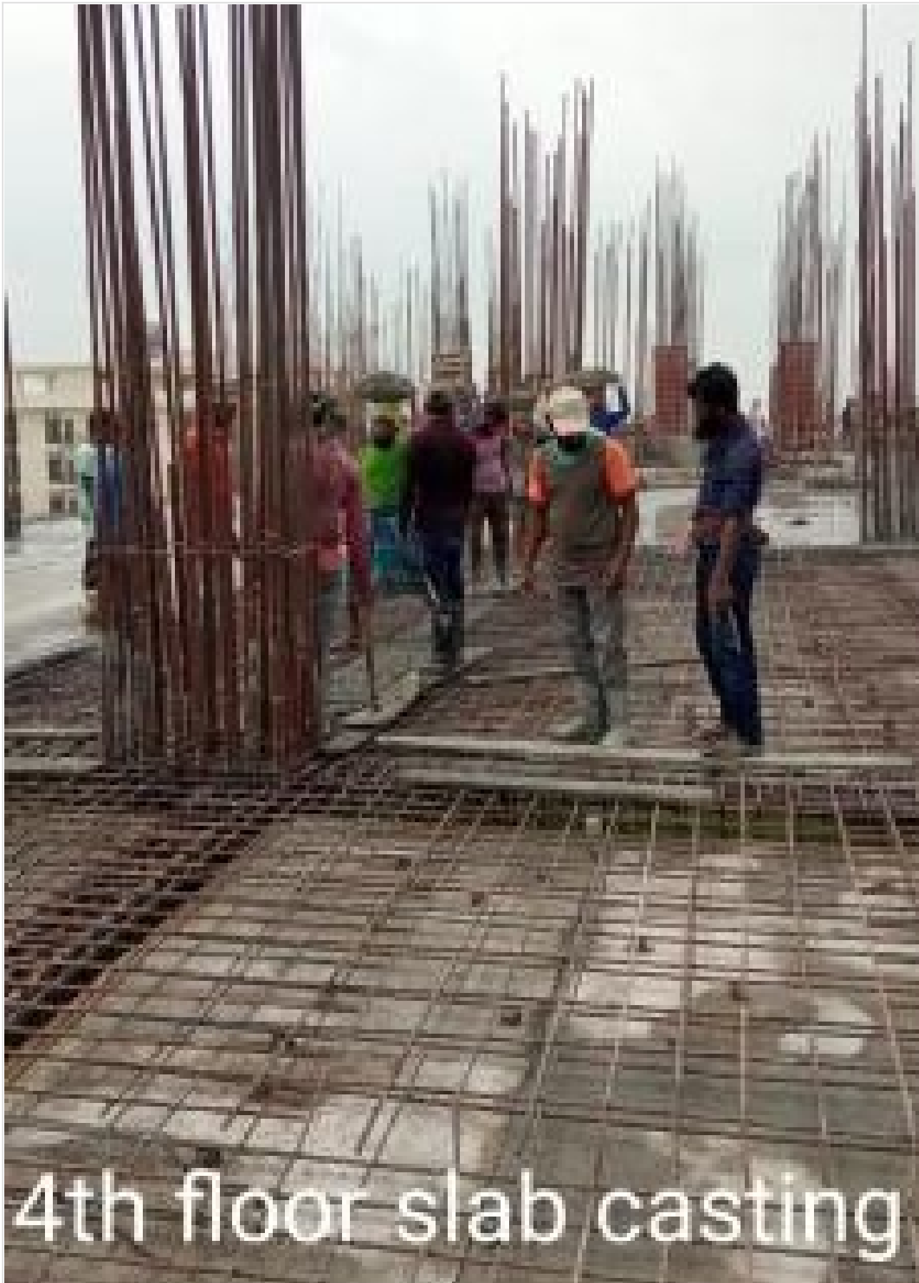
Tower-1-3rd Floor Roof Slab(B-E/6-7)Conc on 31-03-21
