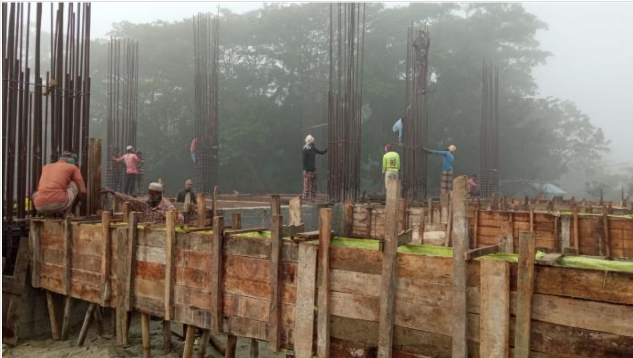
Tower-1 Grade Beam on 07-12-20
