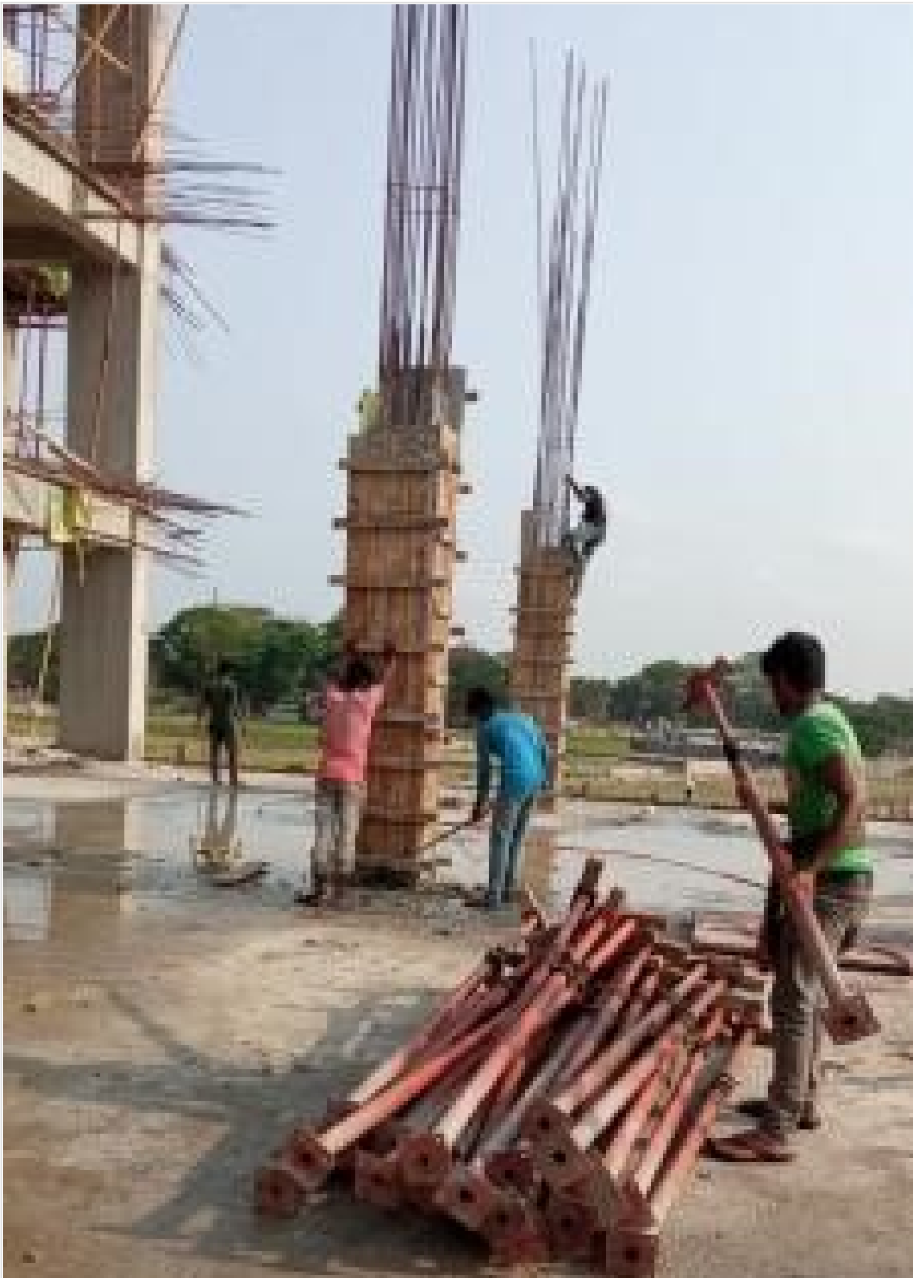
Column Concreting on 29-04-21
