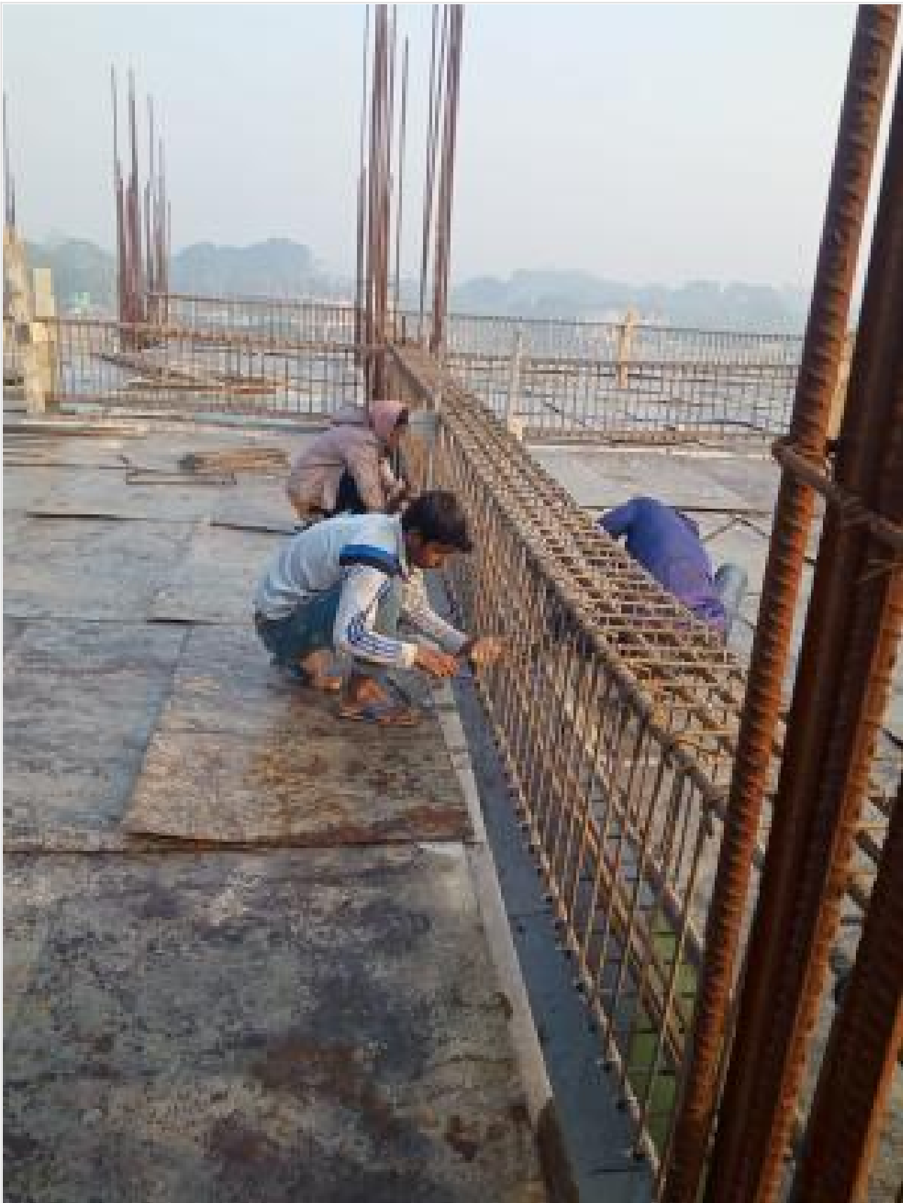
Tower-2-3rd Floor-Re-bar Work on 08-01-22
