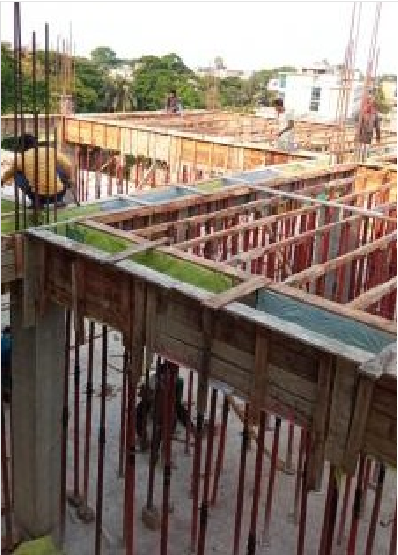
Beam Shuttering on 29-04-21
