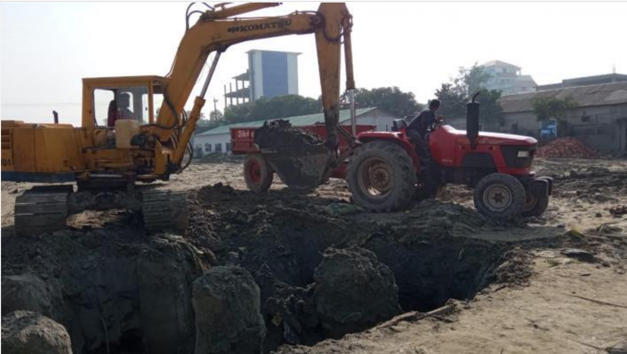
Tower-2-Excavation for Pile Head Breakin on 24-12-20
