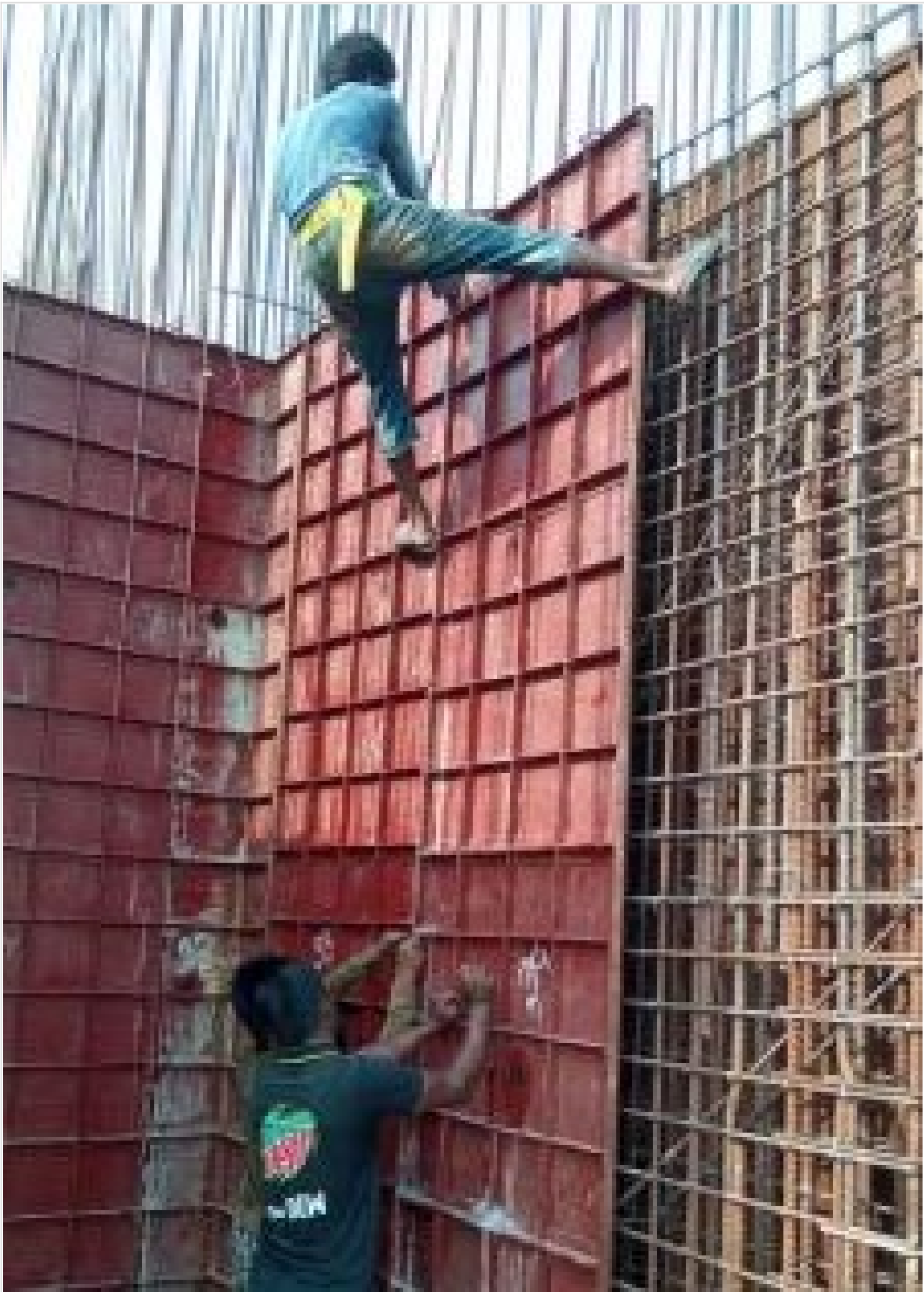
Lift Core Wall Shuttering on 26-04-21
