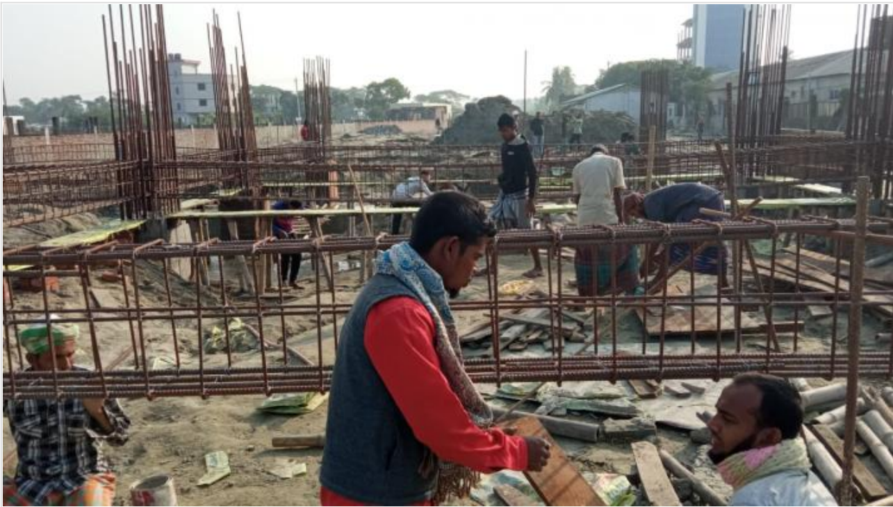
Tower-1-Grade Beam Re-bar Fabrication on 18-12-20
