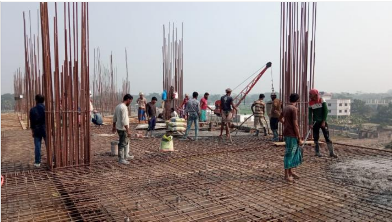
Tower-1-2nd Floor Roof Slab-3600sft Conc on 16-02-21
