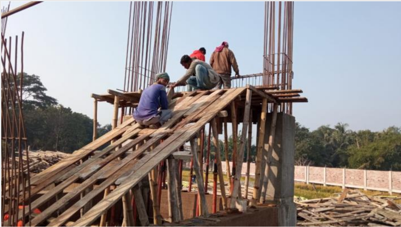
Tower-1-GF Stair Shuttering on 27-12-20
