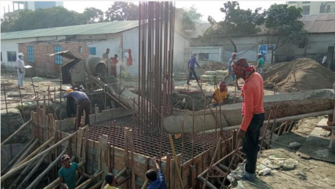
Tower-2-Pile Cap Concreting on 08-01-21
