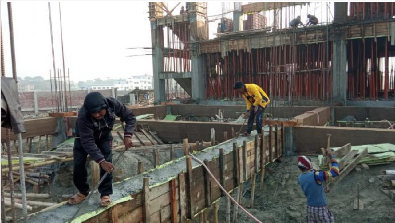
Tower-2-GB Shutter Removing on 05-02-21
