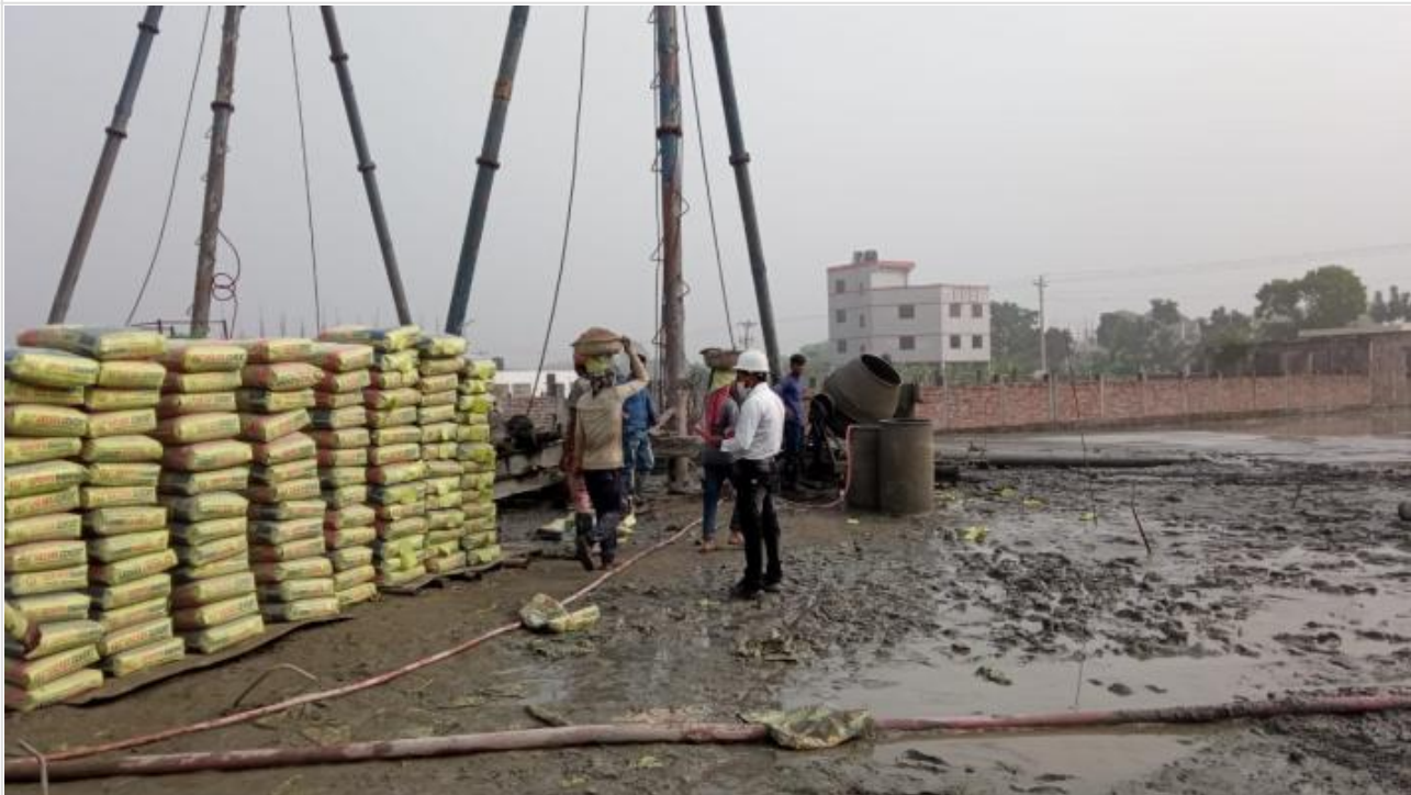
Tower-2-Pile Work on 09-12-20
