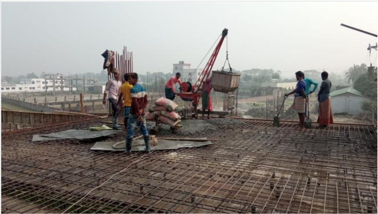
Tower-1-GF Roof Slab 1800 sft Concreting on 18-01-21
