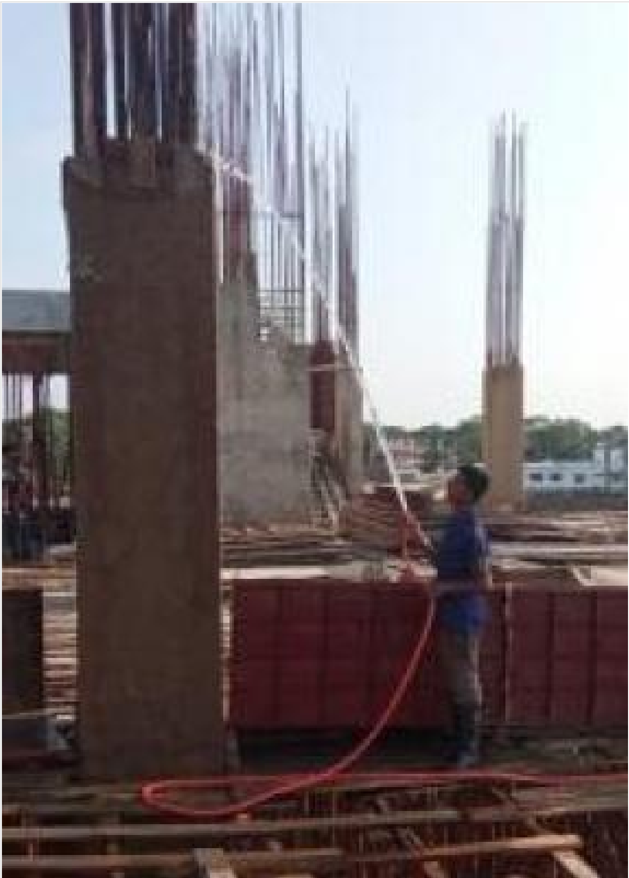
Curing Work on 09-05-21
