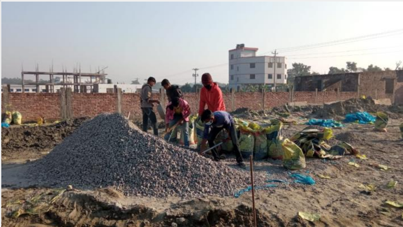
Tower-1-1st floor Roof Slab 2450sft Conc on 10-02-21
