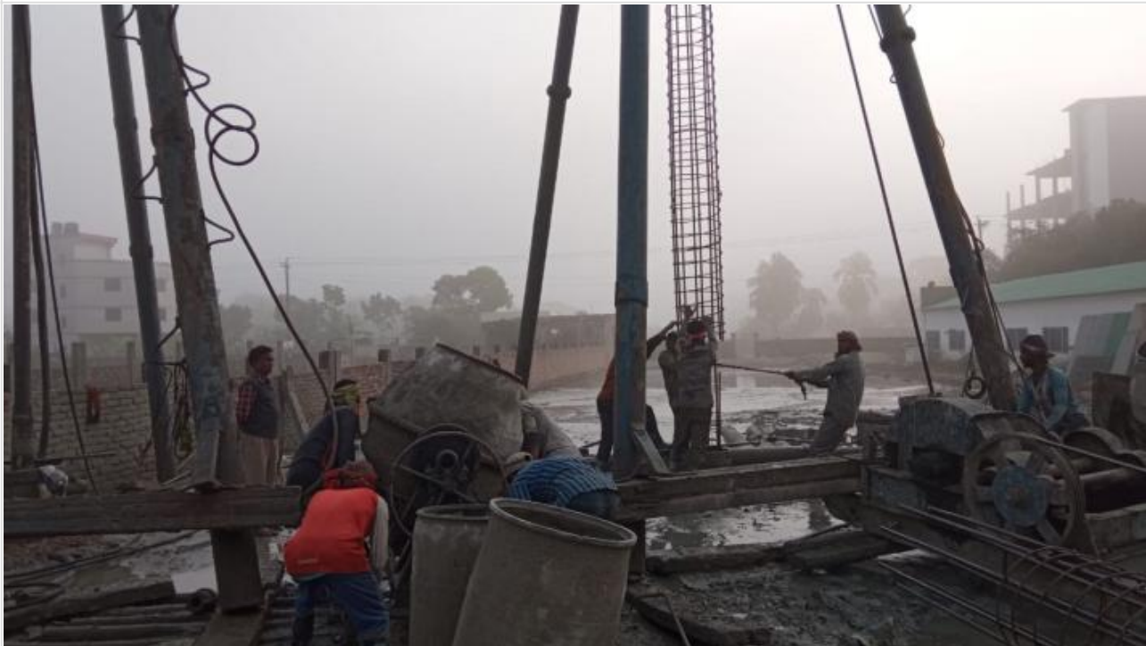
Tower-2-Pile Work on 04-12-20
