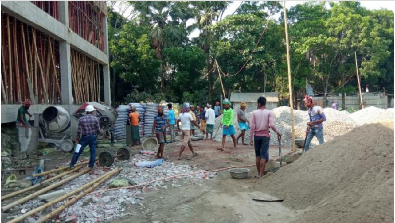
Restaurant GF Doubl Ht Slab-1-4/A-B-Conc on 24-04-21
