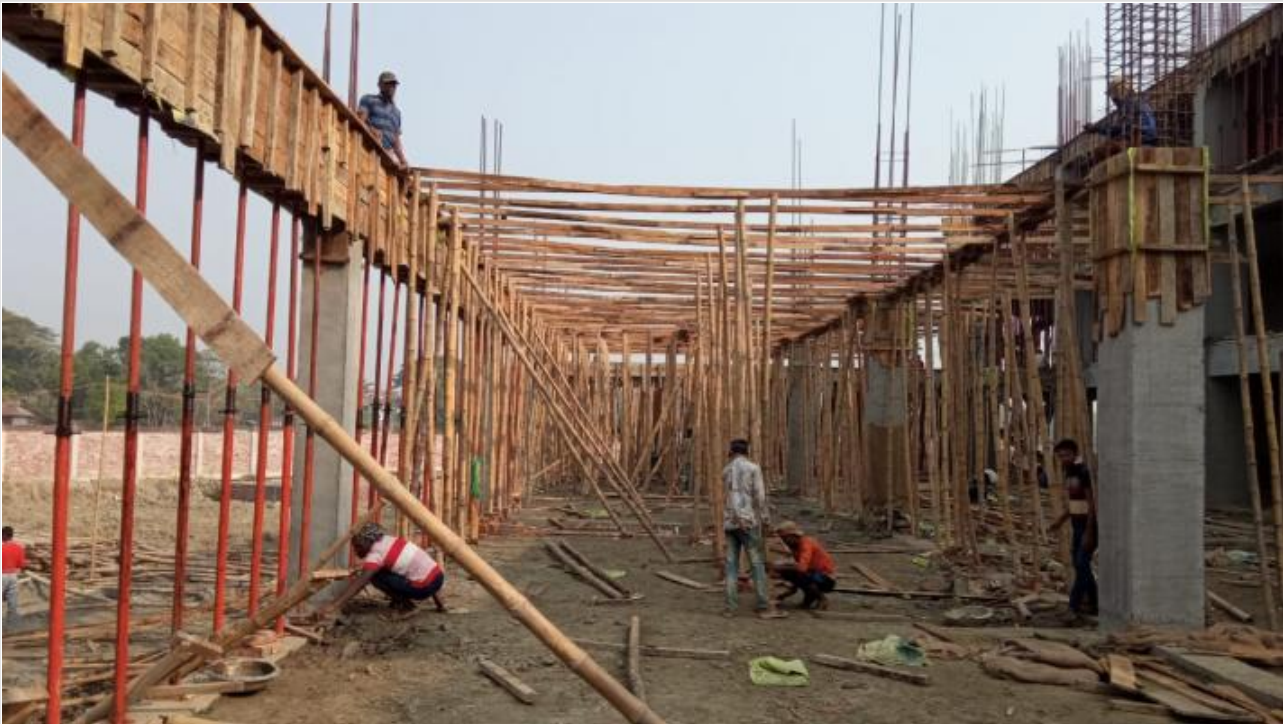
Restaurant Area Slab Shuttering on 23-02-21
