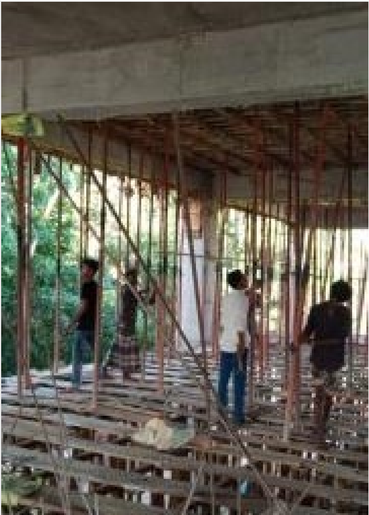
Restaurant GF Double Height Roof Slab on 24-05-21
