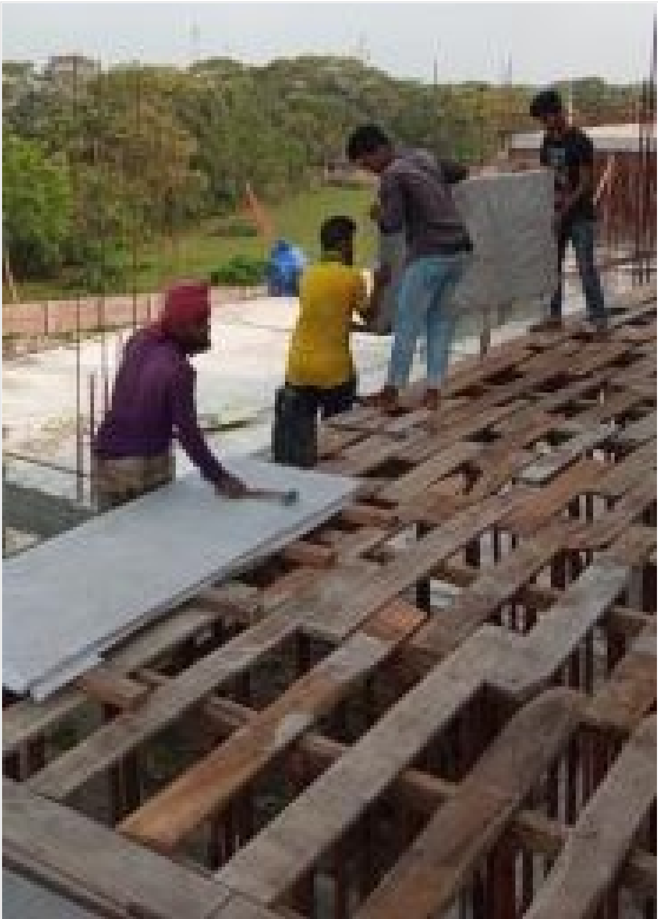
Slab Shuttering on 31-05-21
