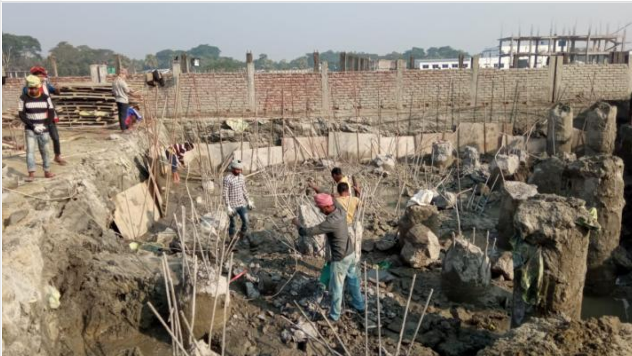
Tower-2-Pile Head Breaking on 27-12-20
