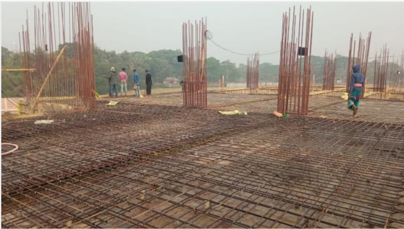
Tower-1-GF Roof Slab-3600sft Concreting on 16-01-21
