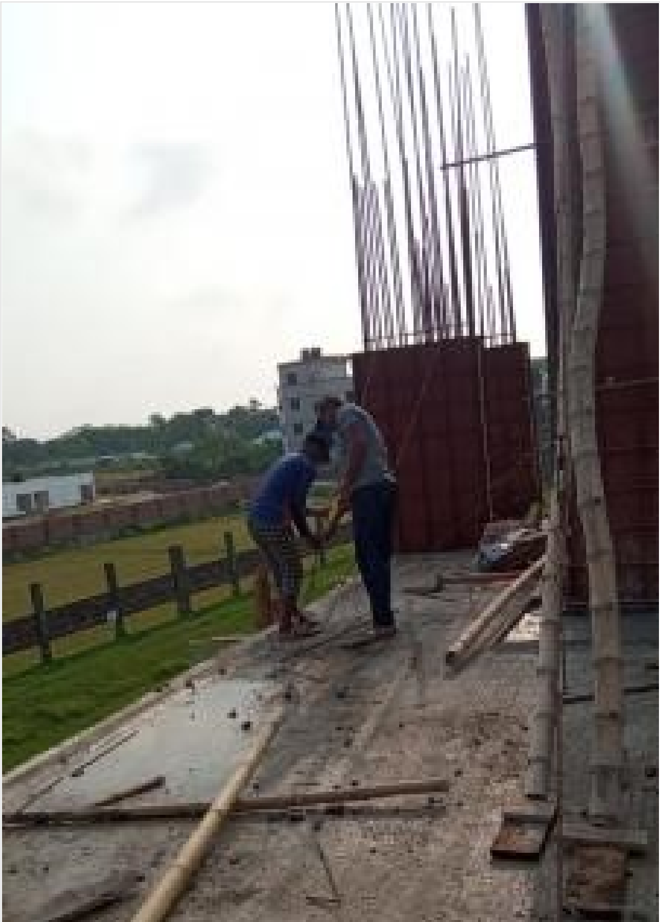
Column Shuttering Work on 30-04-21
