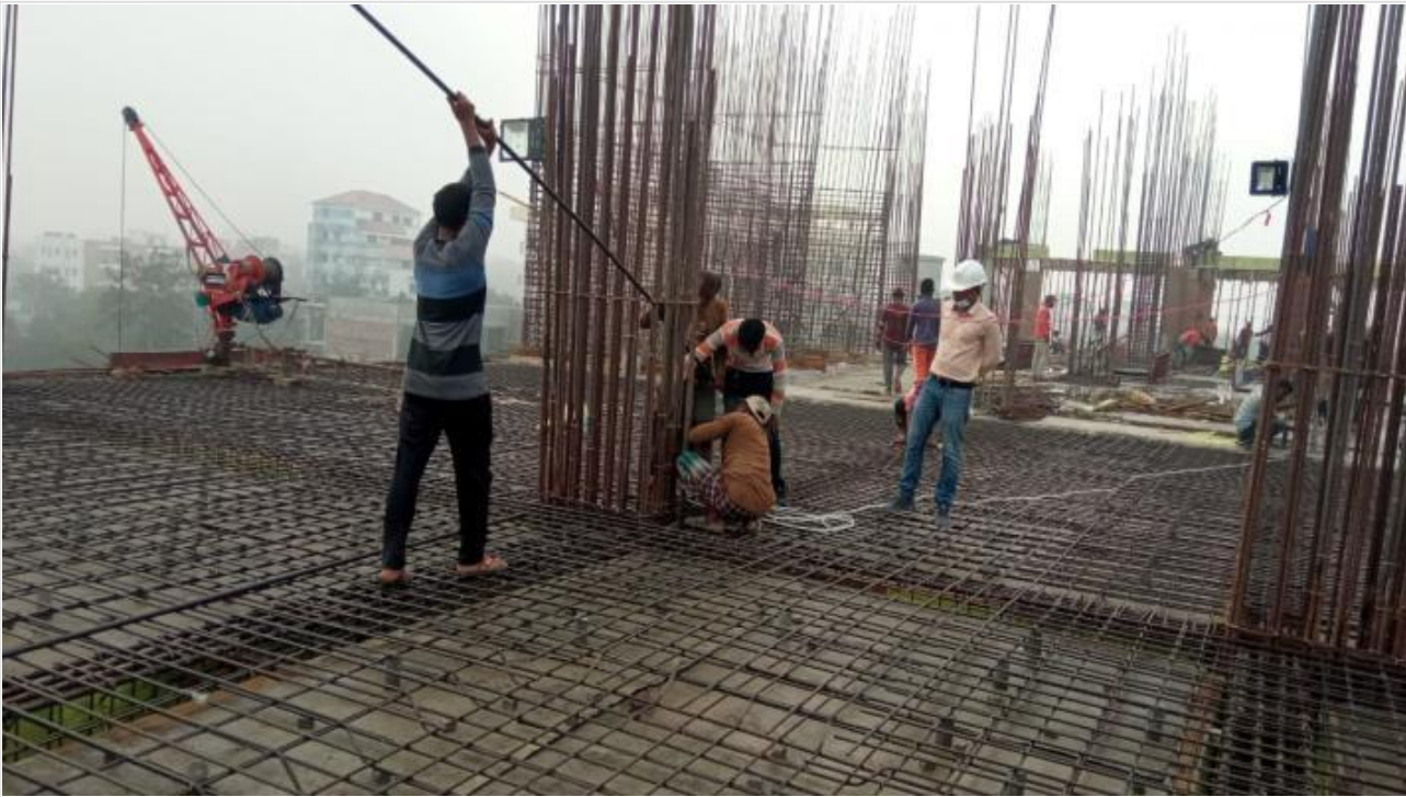
Tower-1-2nd Floor Roof Inspection on 25-02-21
