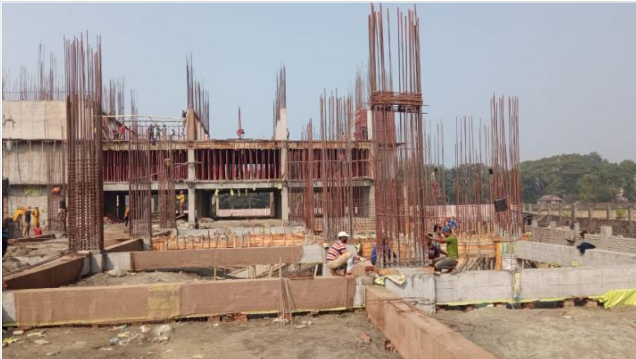
Tower-2-Column Re-bar Work on 16-02-21
