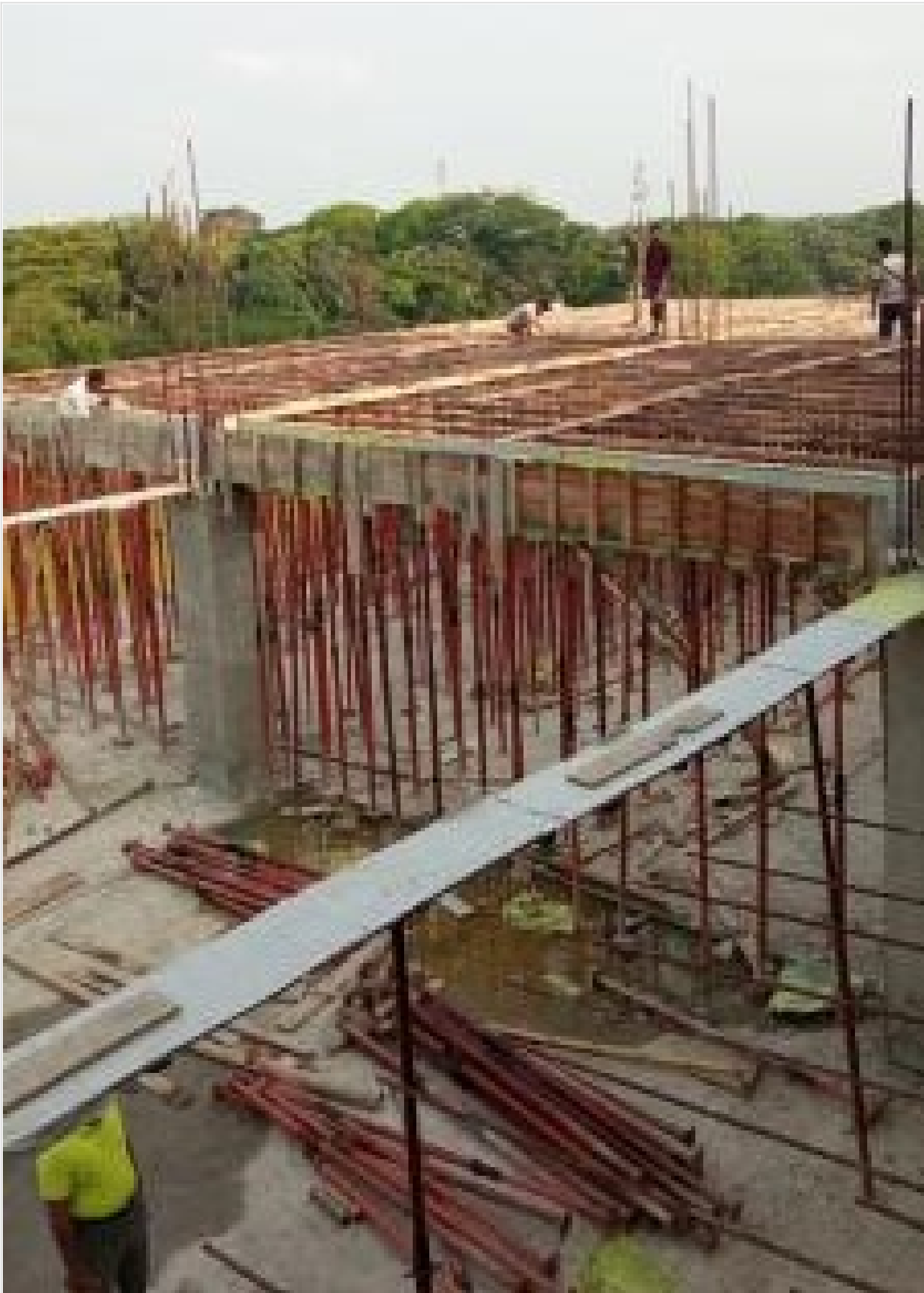
Beam Shuttering Work on 30-04-21
