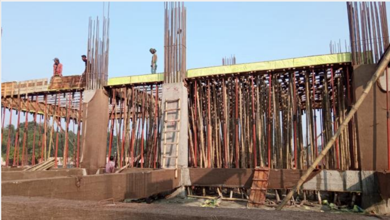
Tower-1-GF Beam Shuttering on 18-12-20
