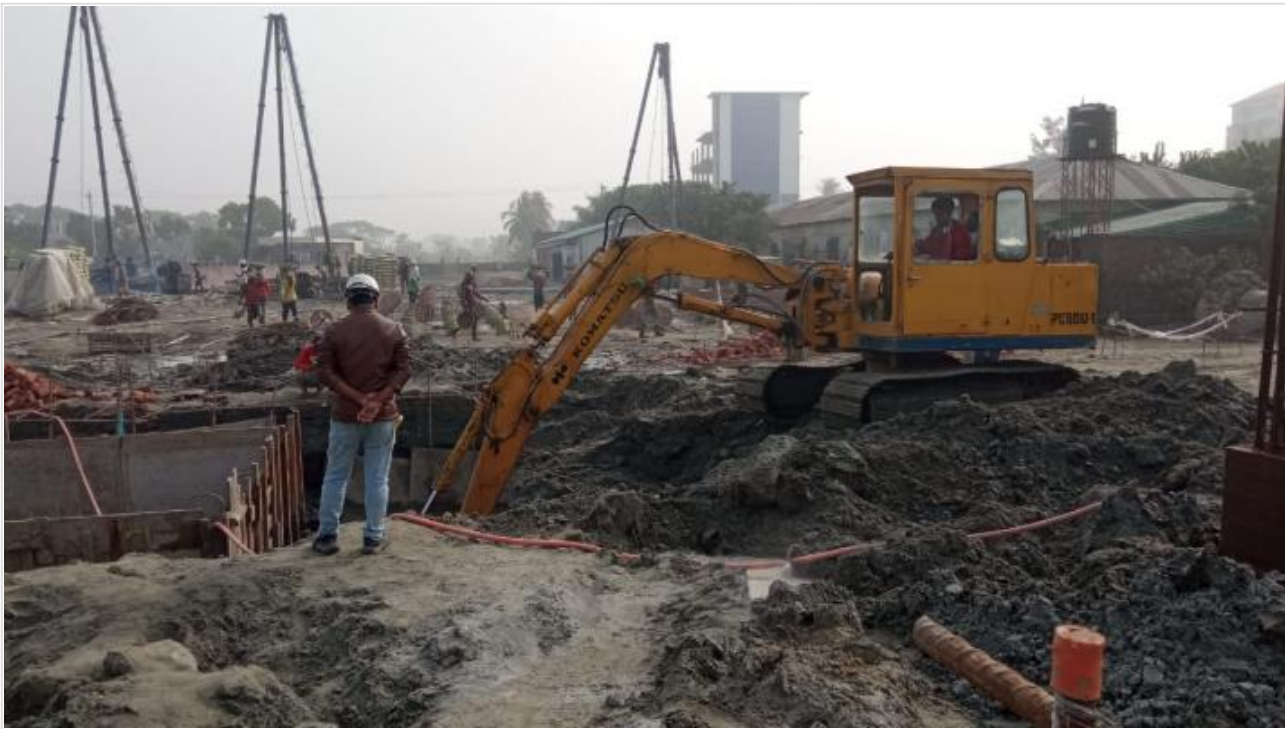
Tower-1-Excavation for Pile Cap on 09-12-20
