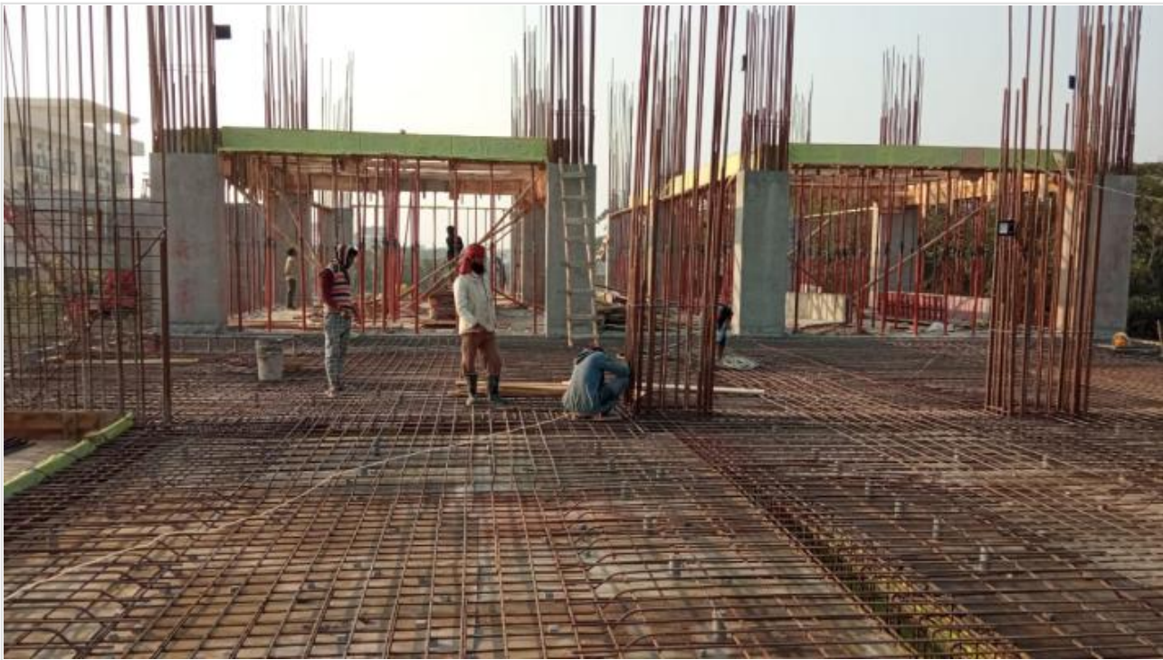
Tower-1-1st Floor Roof Slab 3600 sft Con on 05-02-21
