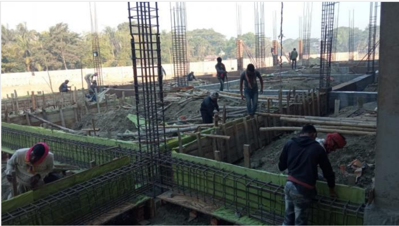
Tower-2-Grade Beam Shuttering on 10-02-21
