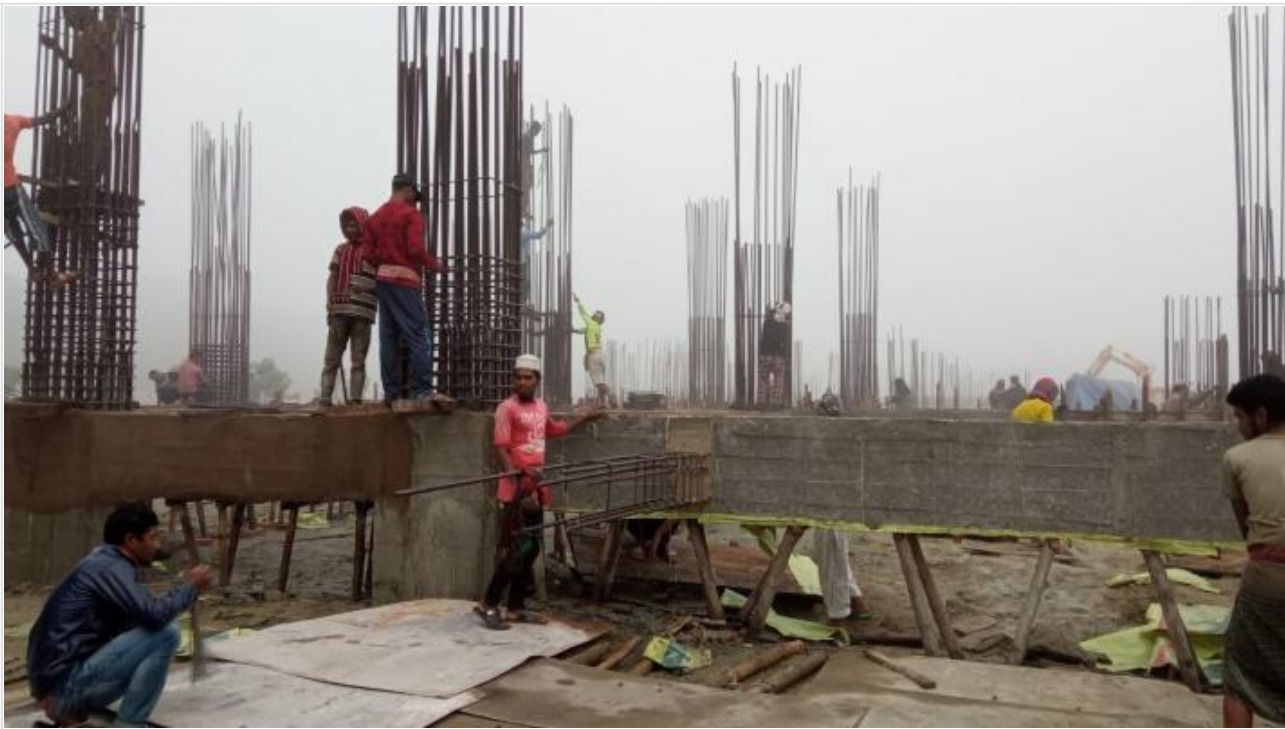
Column Work on 07-12-20
