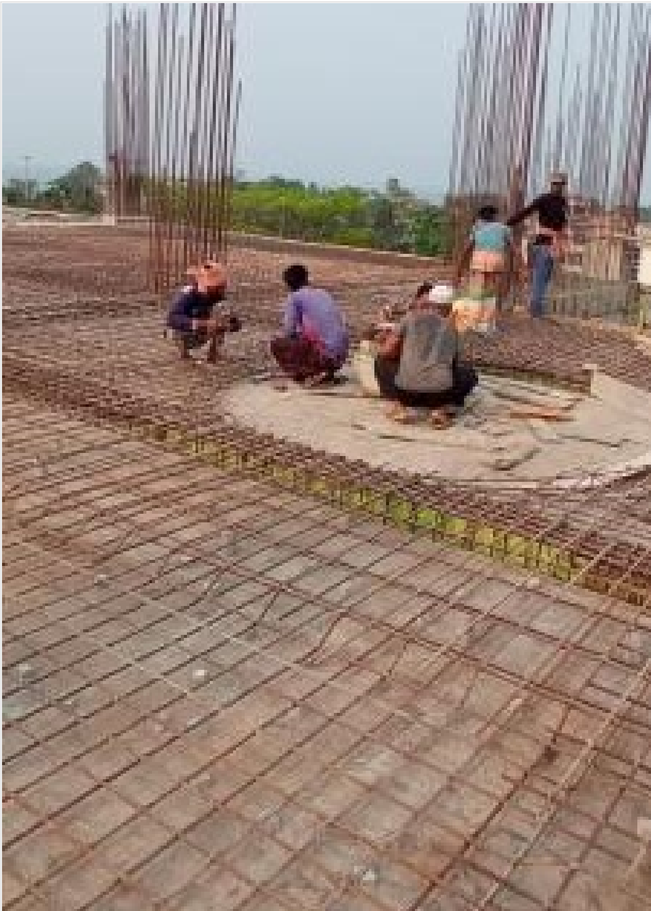
4th Floor Slab(3-5/B-E) Concreting-3600s on 24-03-21
