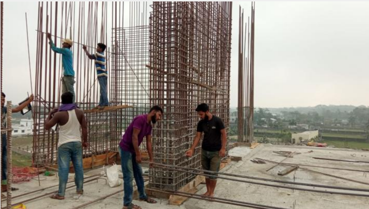
Tower-1-3rd Floor Lift Core Re-bar Work on 02-03-21
