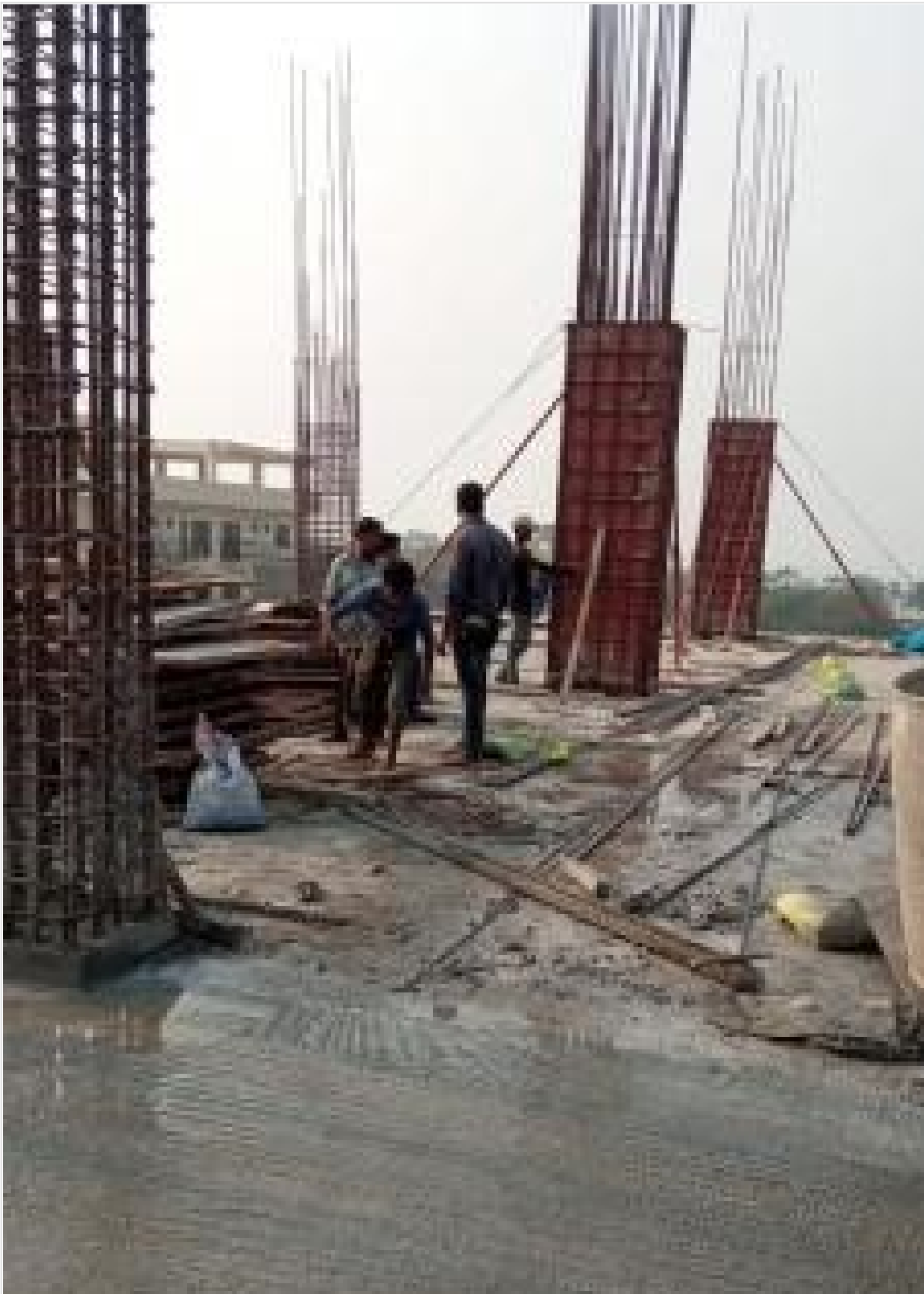
Column Shuttering Work on 25-03-21
