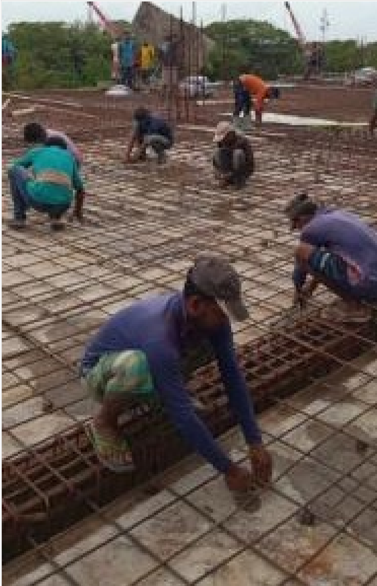
Restaurant-3rd Floor Slab Concreting on 12-06-21
