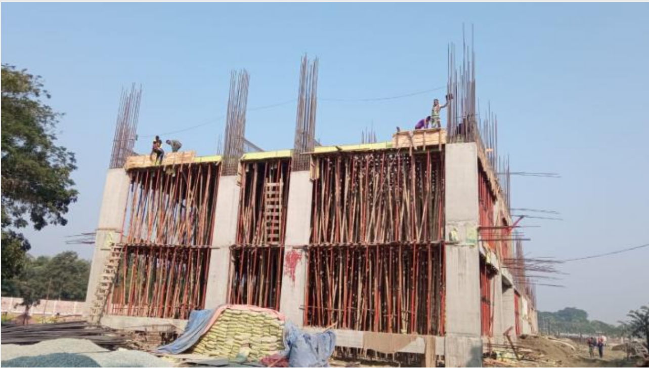
Tower-1-1st Floor Roof Slab Shuttering on 08-01-21
