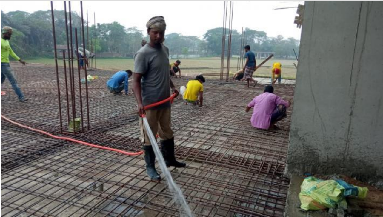
Restaurant-Double Height Slab Concreting on 02-03-21
