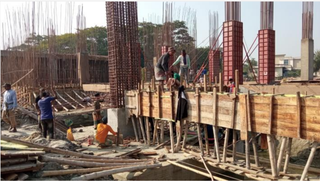
Tower-1-Grade Beam Shuttering on 24-12-20
