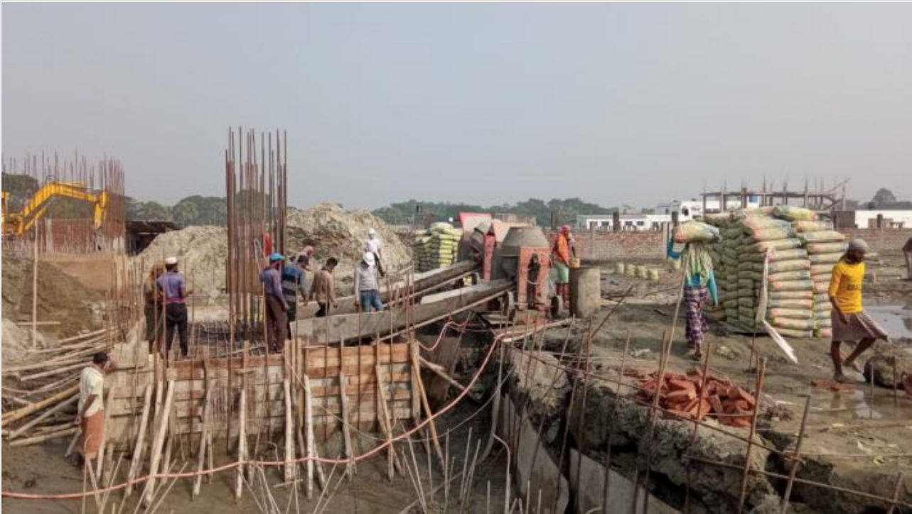
Tower-1-Pilecap Concreting on 12-12-20
