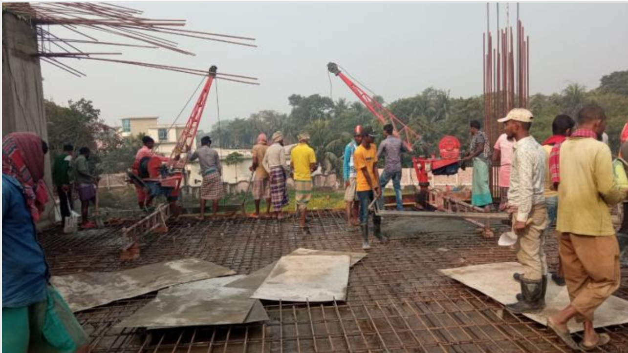
Tower-1-GF Roof Slab Concreting on 16-01-21
