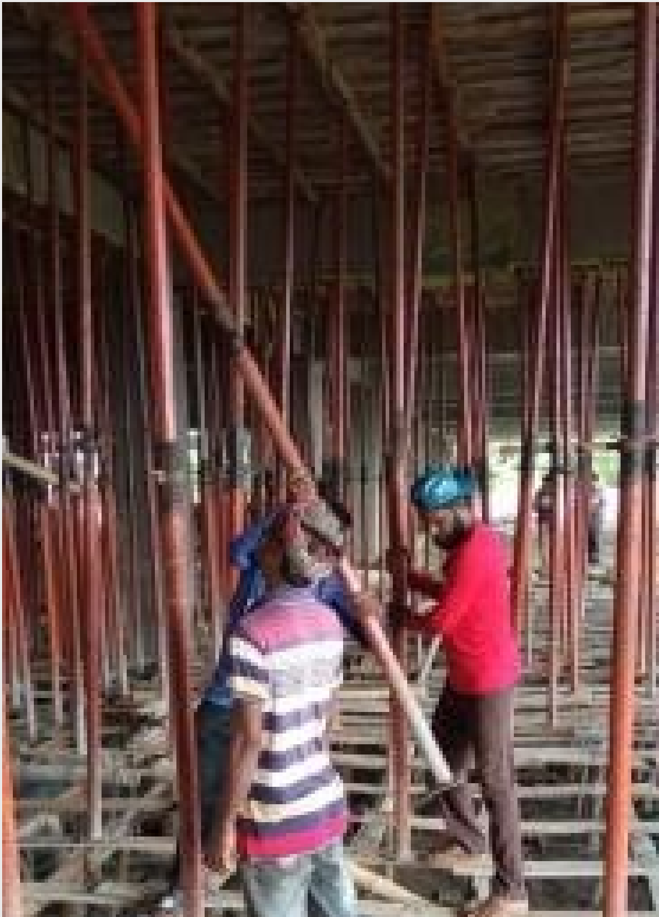
Roof Slab De-shuttering on 24-05-21
