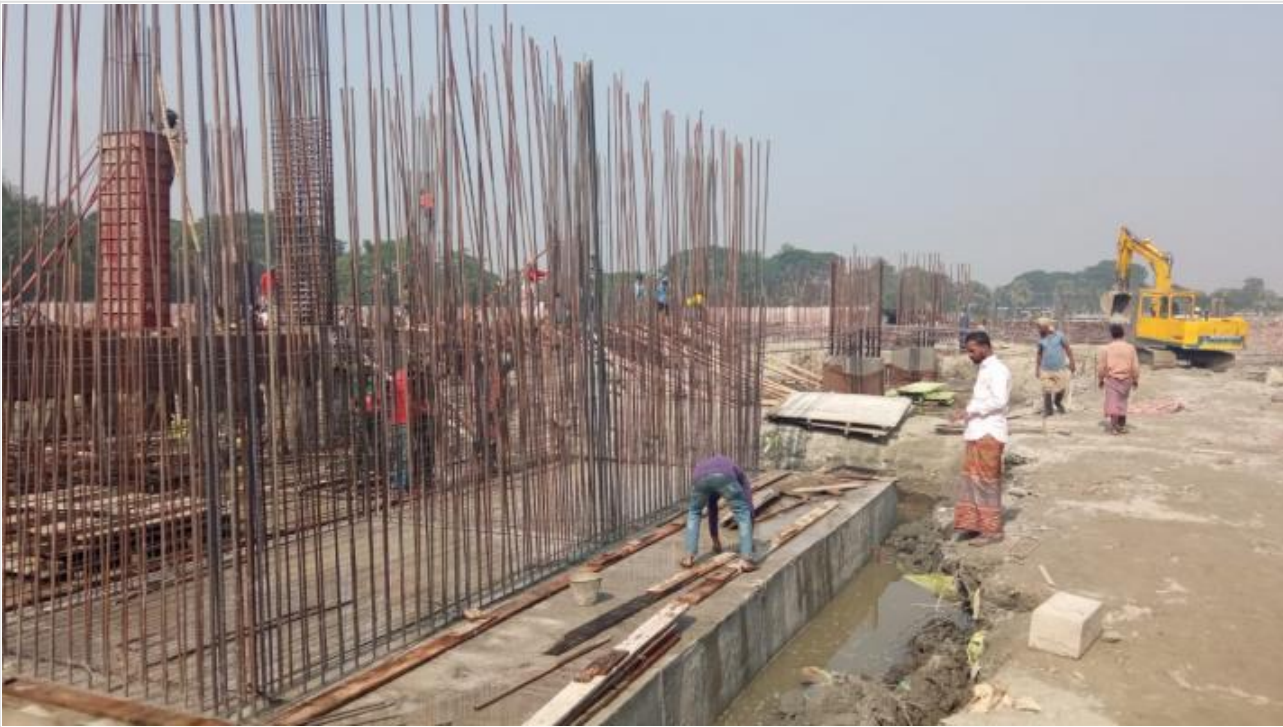
Tower-1-Lift Core Re-bar Work on 20-12-20
