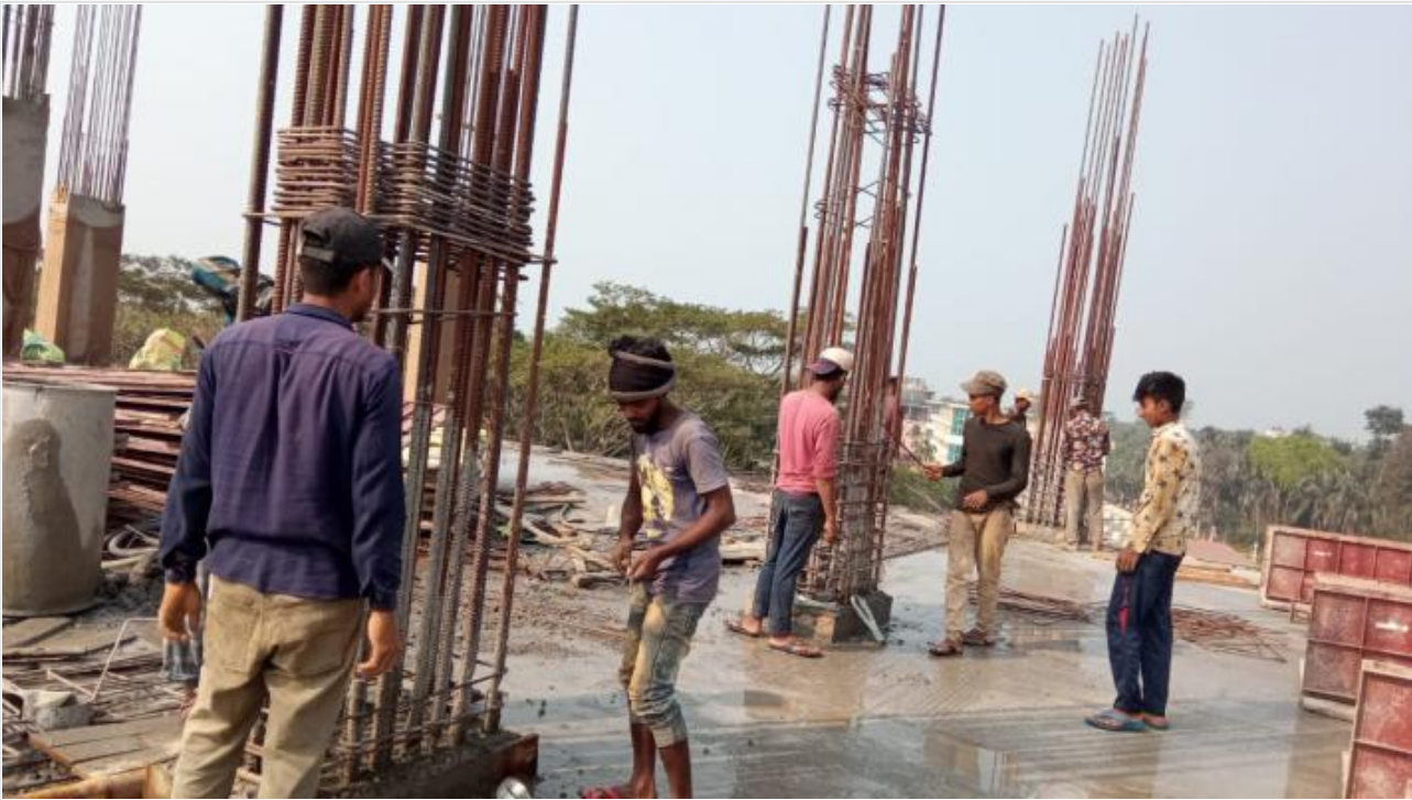
Tower-1-3rd Floor Column Re-bar Work on 23-02-21
