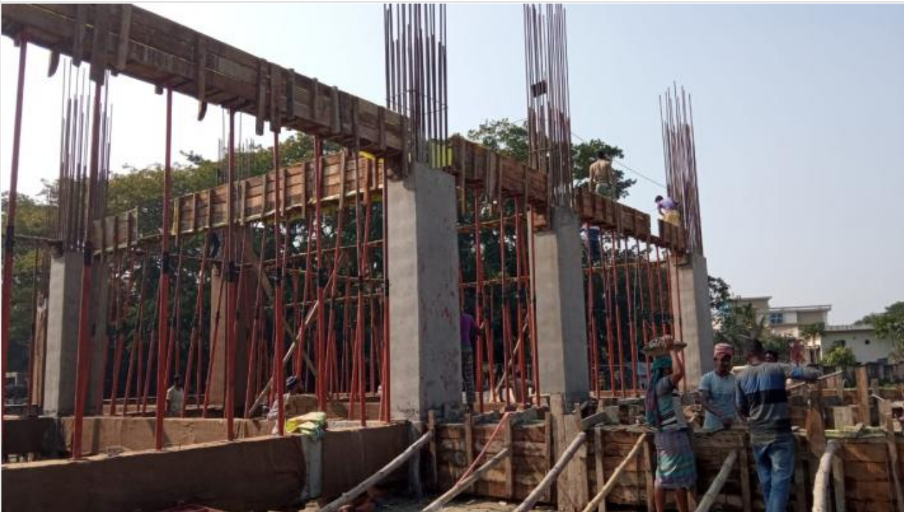
Tower-1-GF Beam Shuttering on 15-12-20
