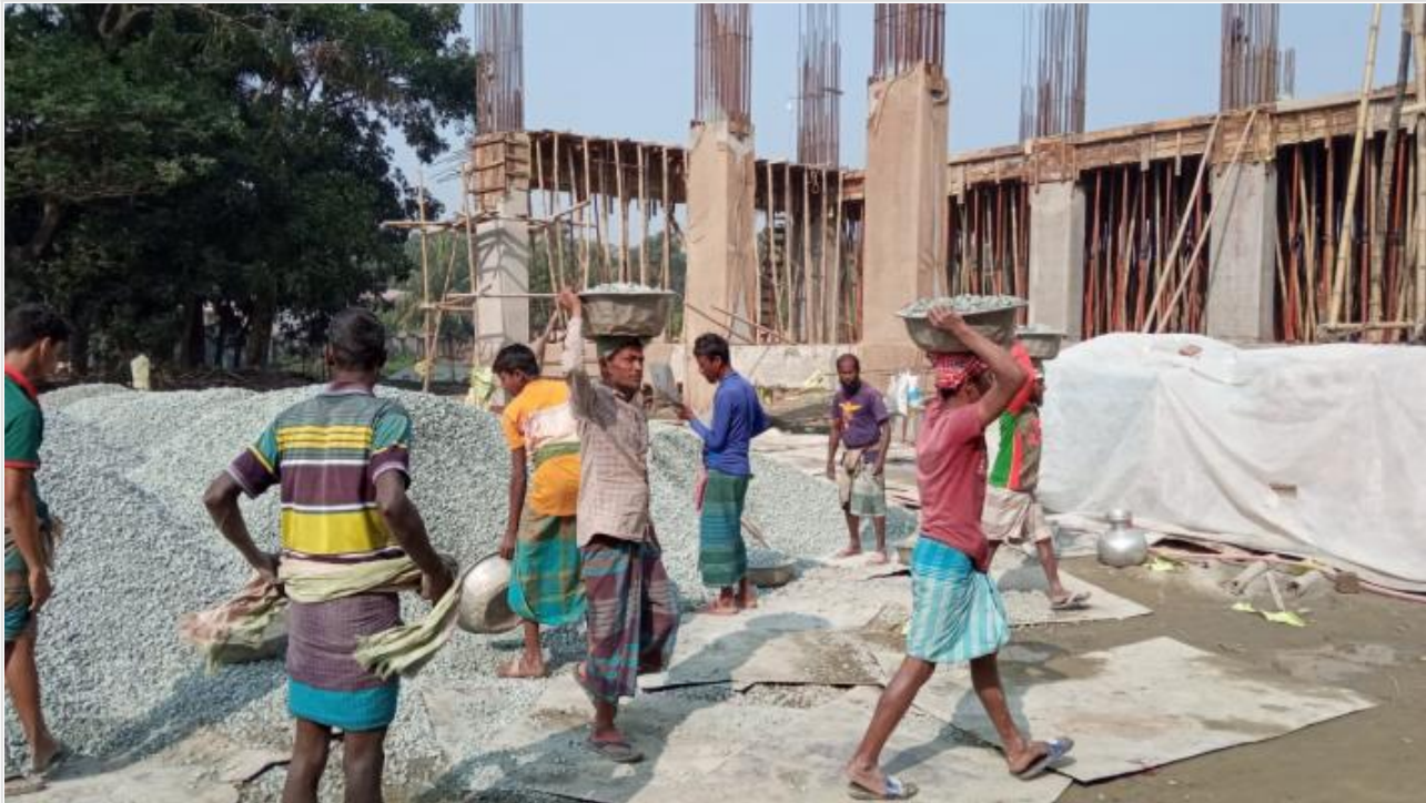
Tower-1-GF Roof Slab Concreting on 21-12-20
