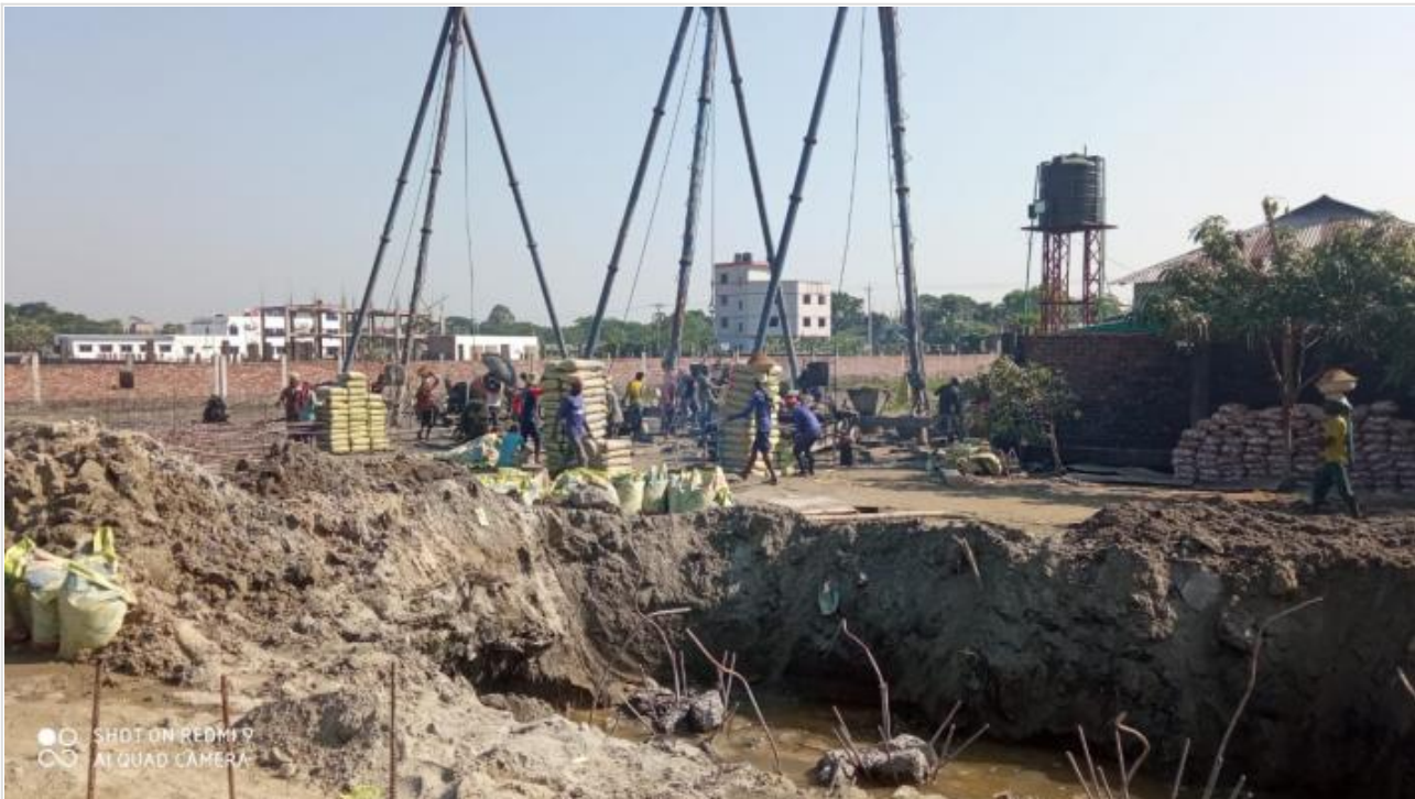
Tower-2-Piling Work on 28-11-20
