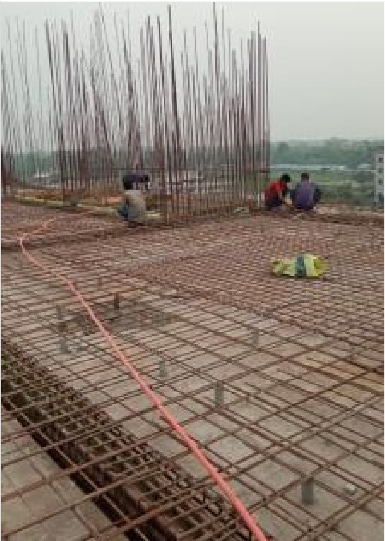
Restaurant GF Double Height Slab-6-9/A-B on 23-03-21
