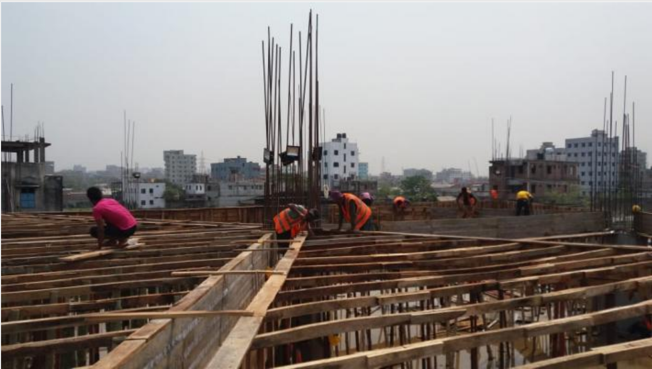
Mosque 1st Floor Slab Shuttering on 28-03-21
