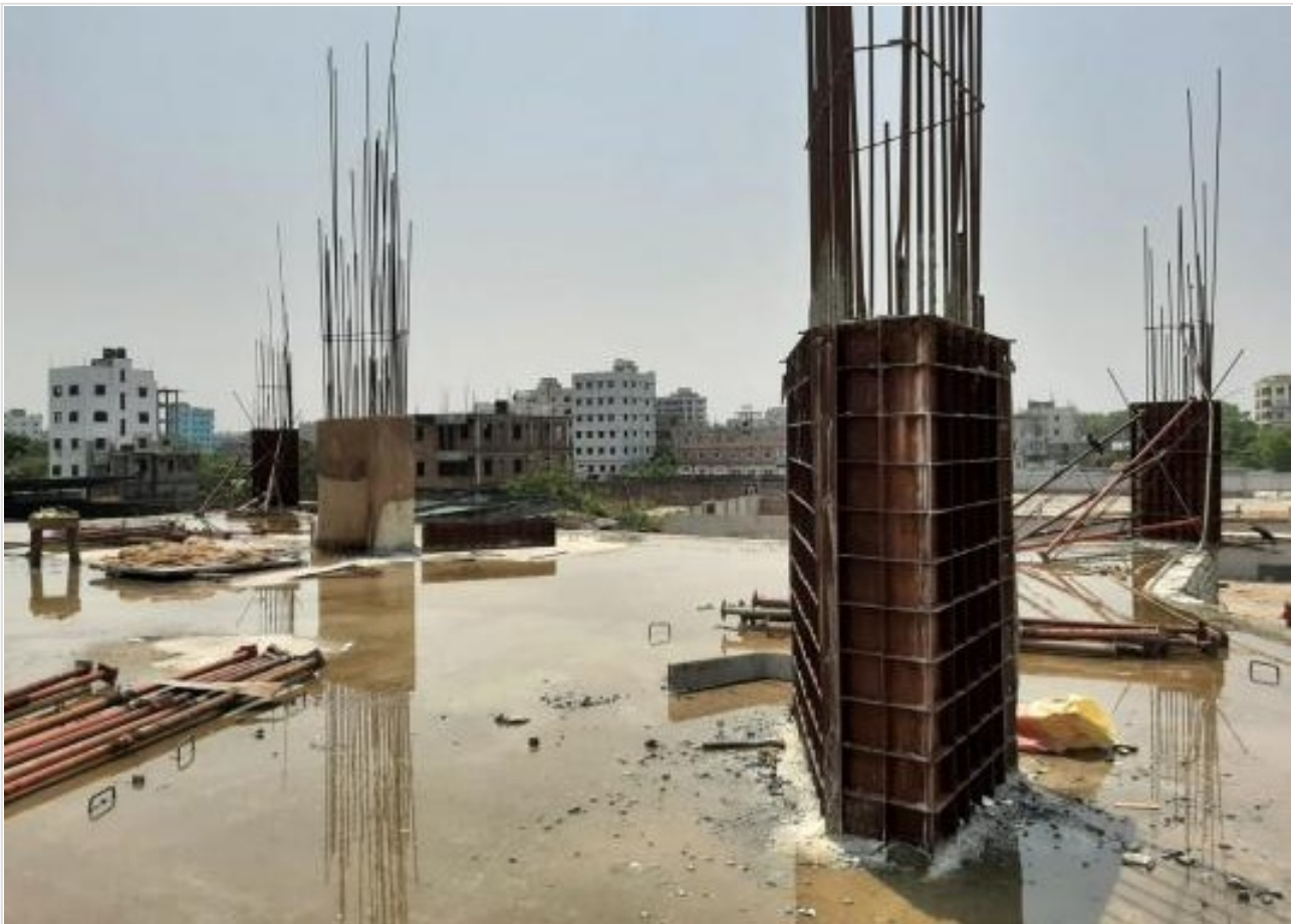
Mosque-1st Floor-Column Shuttering on 26-04-21
