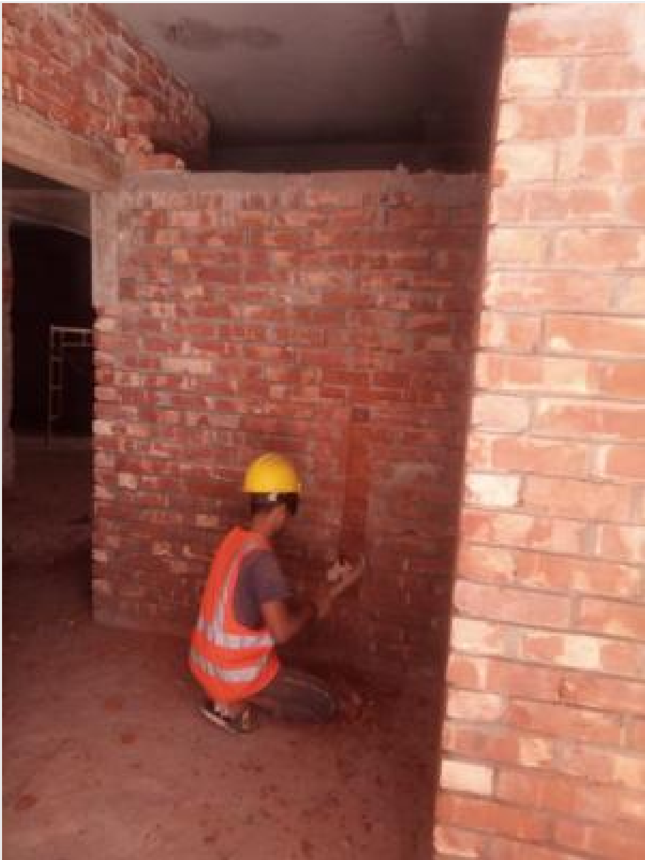
Electrical Conduit Conesealing on 25-02-21
