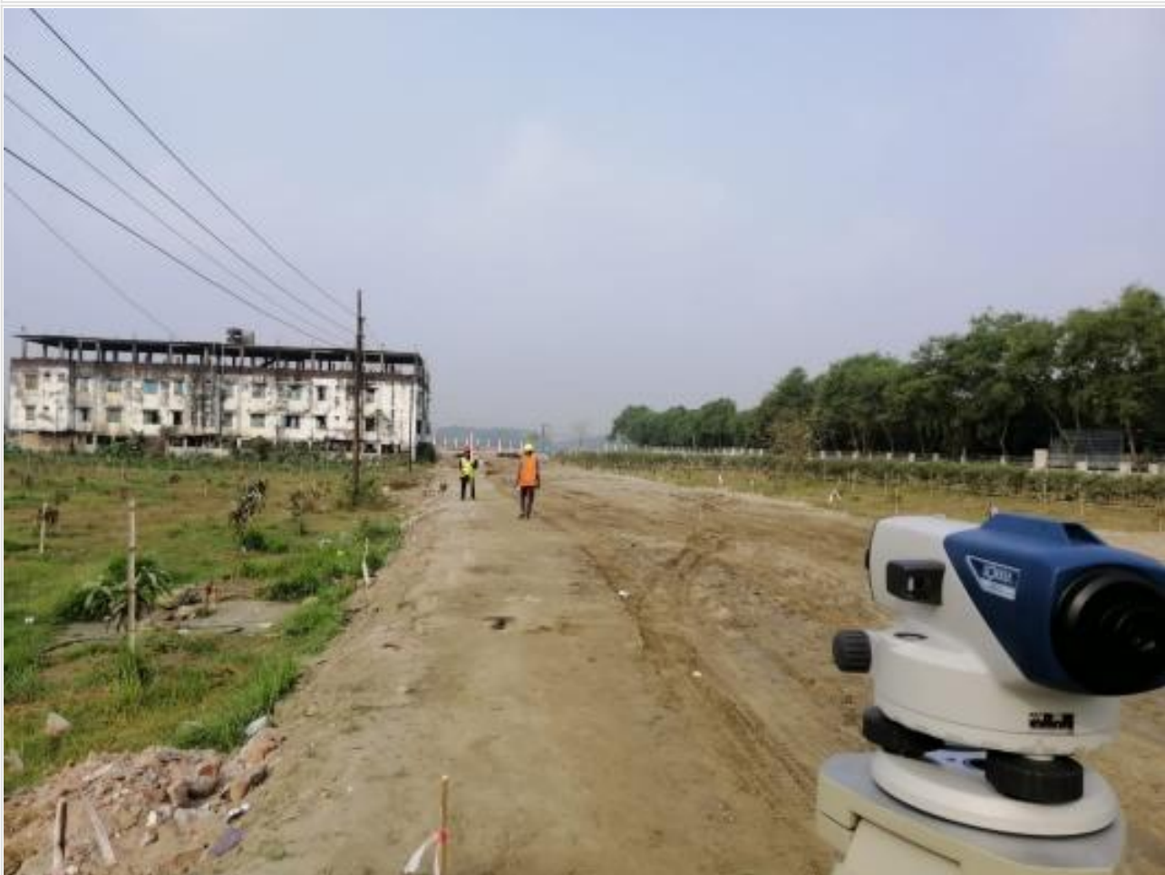
40 ft Road Dressing and Levelling on 01-03-21
