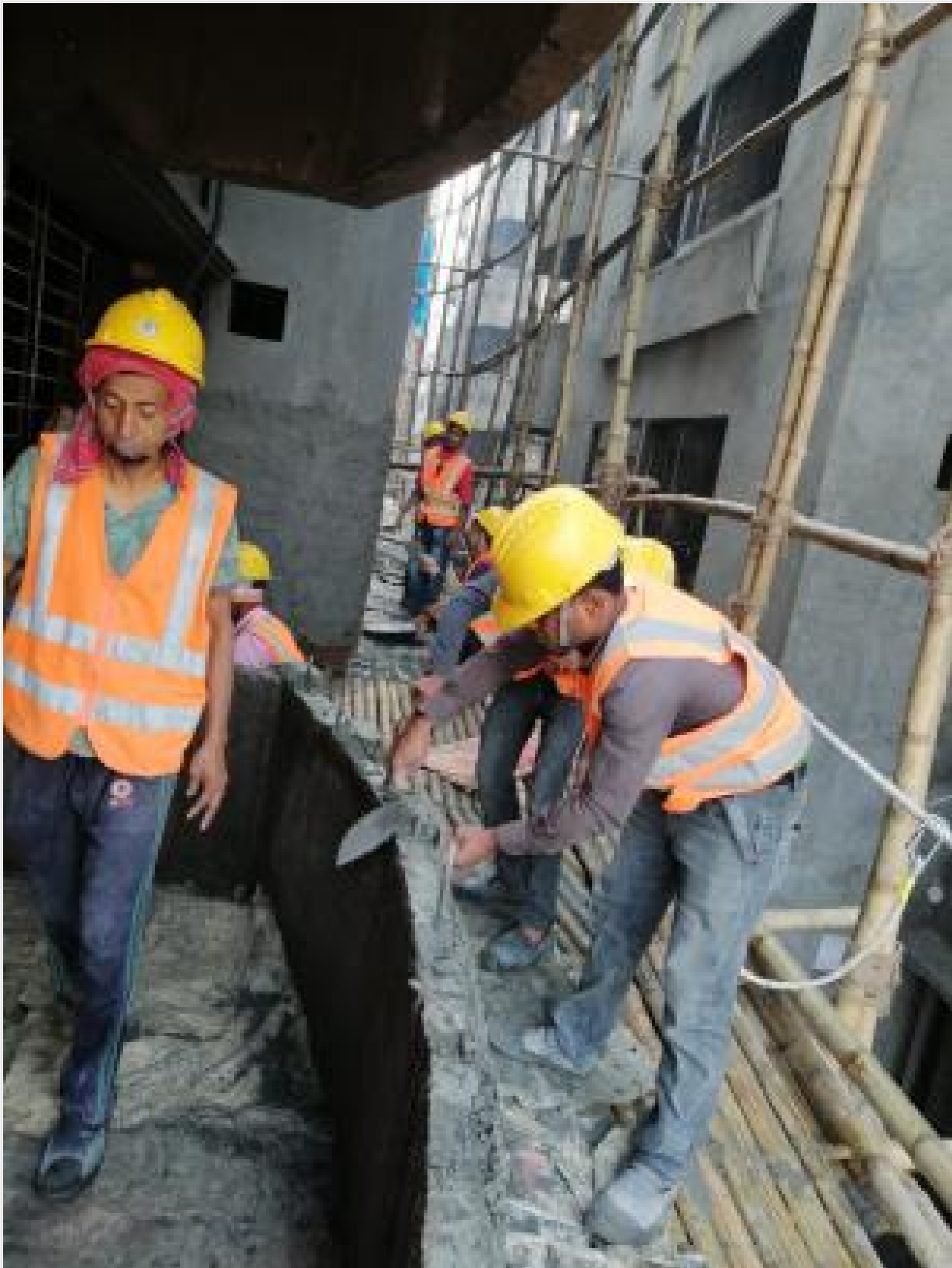
Out-side Plaster Work on 05-02-21
