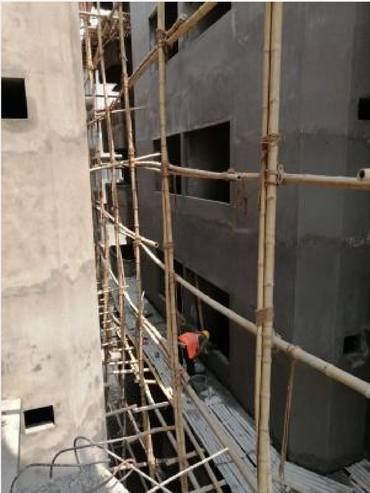
Out-side Plastering on 02-05-21
