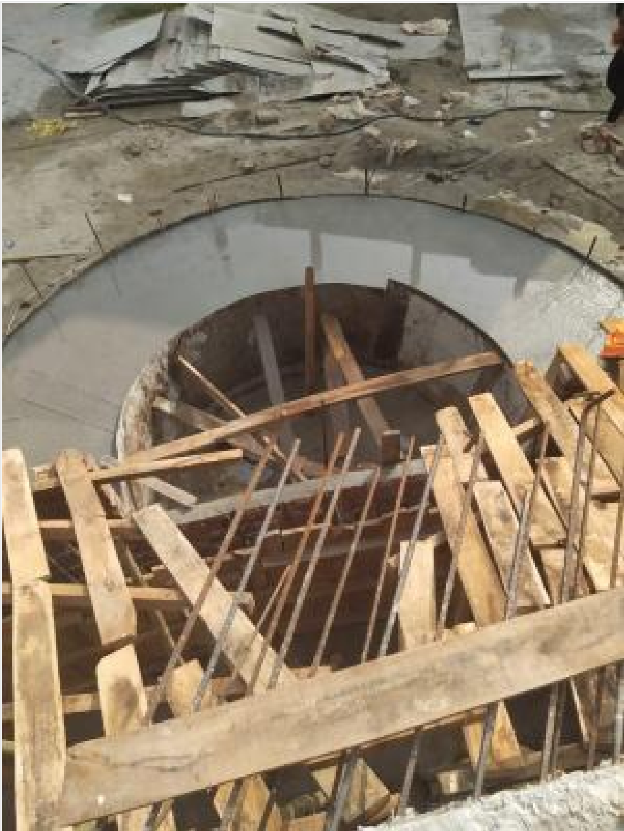
Mosque Ground Floor Stair Concreting on 27-03-21
