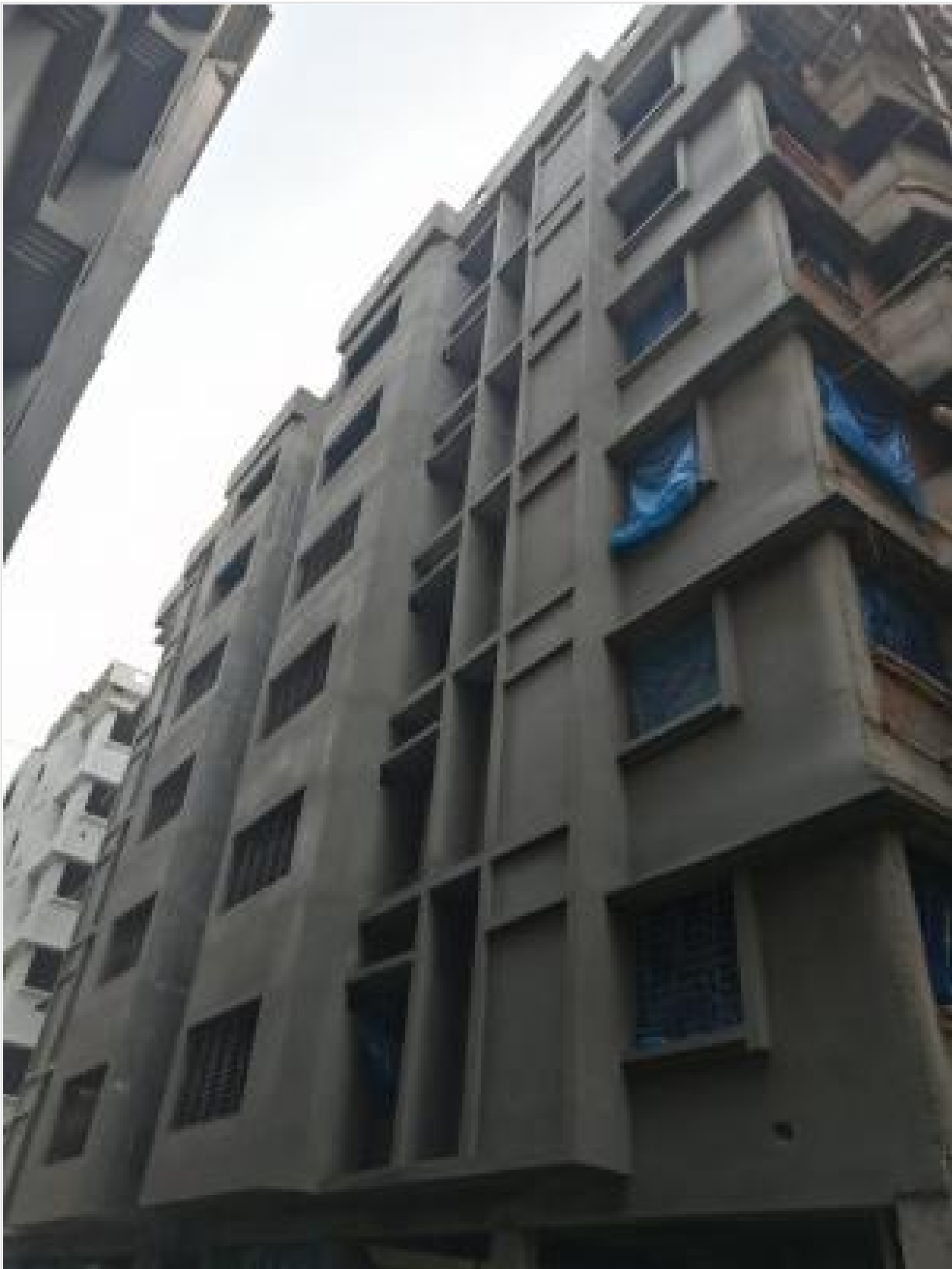
Building-J outside plastering on 28-01-21
