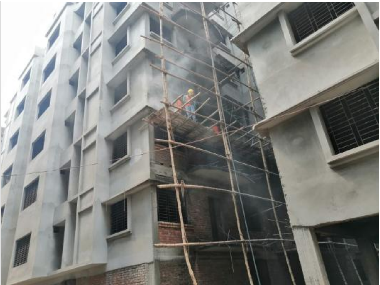
Building Outside Plastering on 08-03-21
