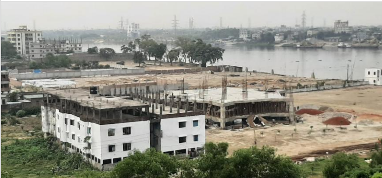
Mosque in Construction on 15-04-21
