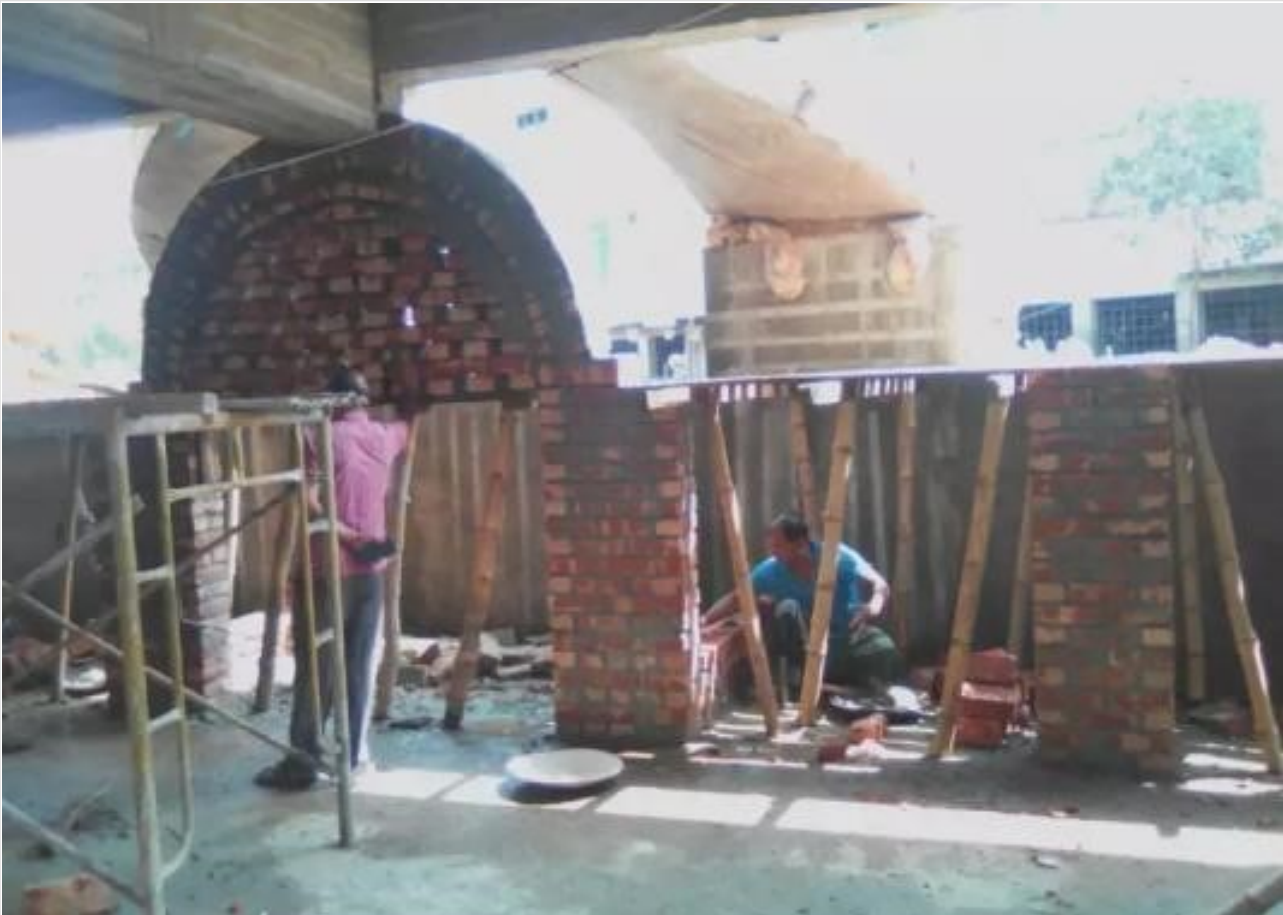
Mosque-Ground Floor Ancillary Works on 14-04-21
