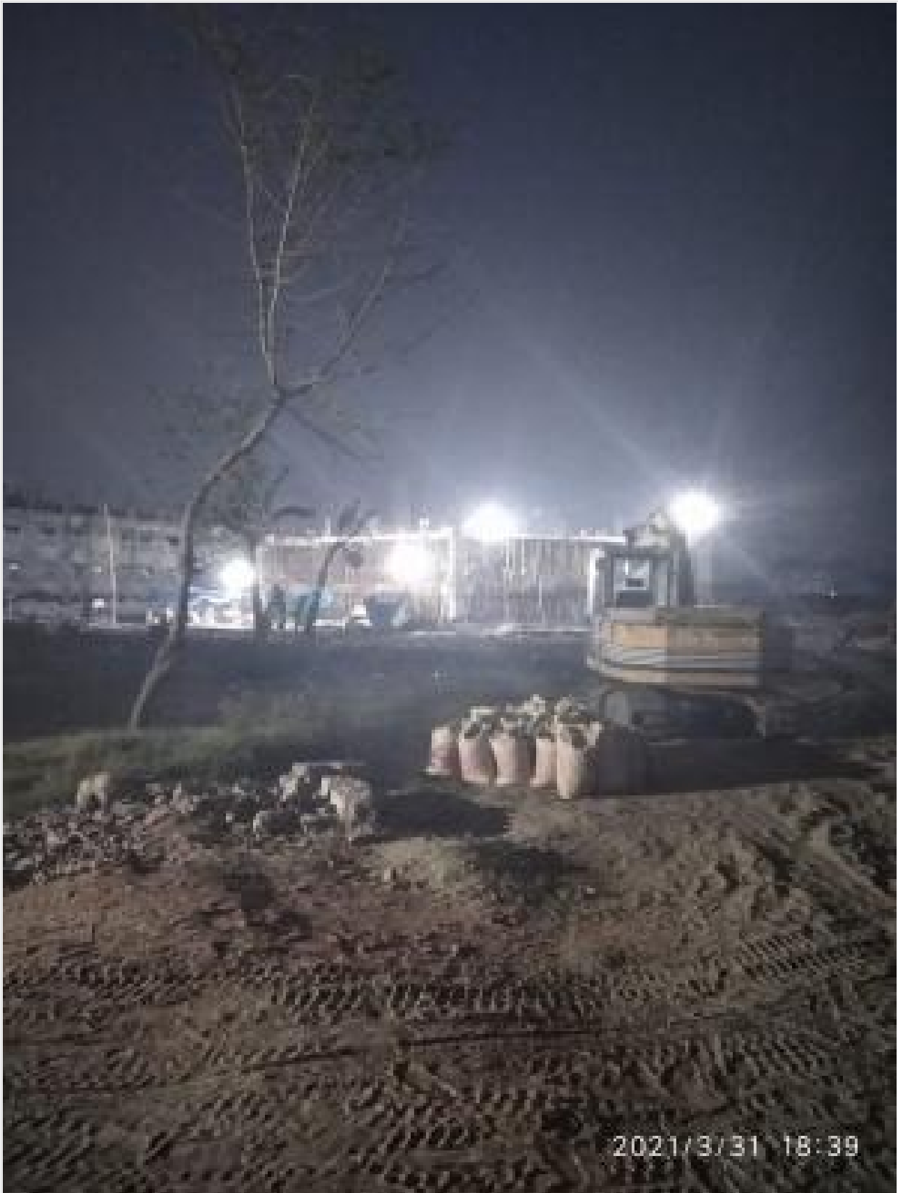
Mosque-Night Shift Work on 31-03-21
