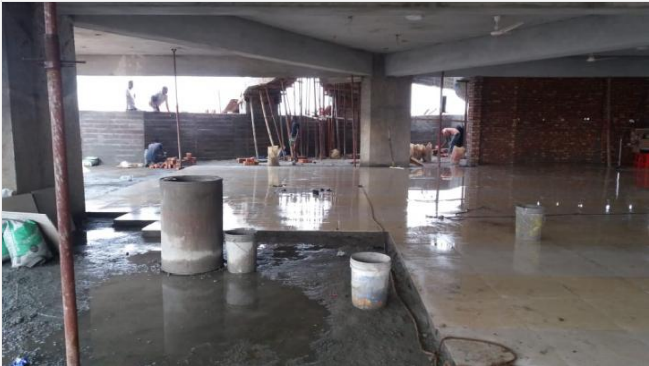
Mosque-Basement-Tile Work on 13-04-21
