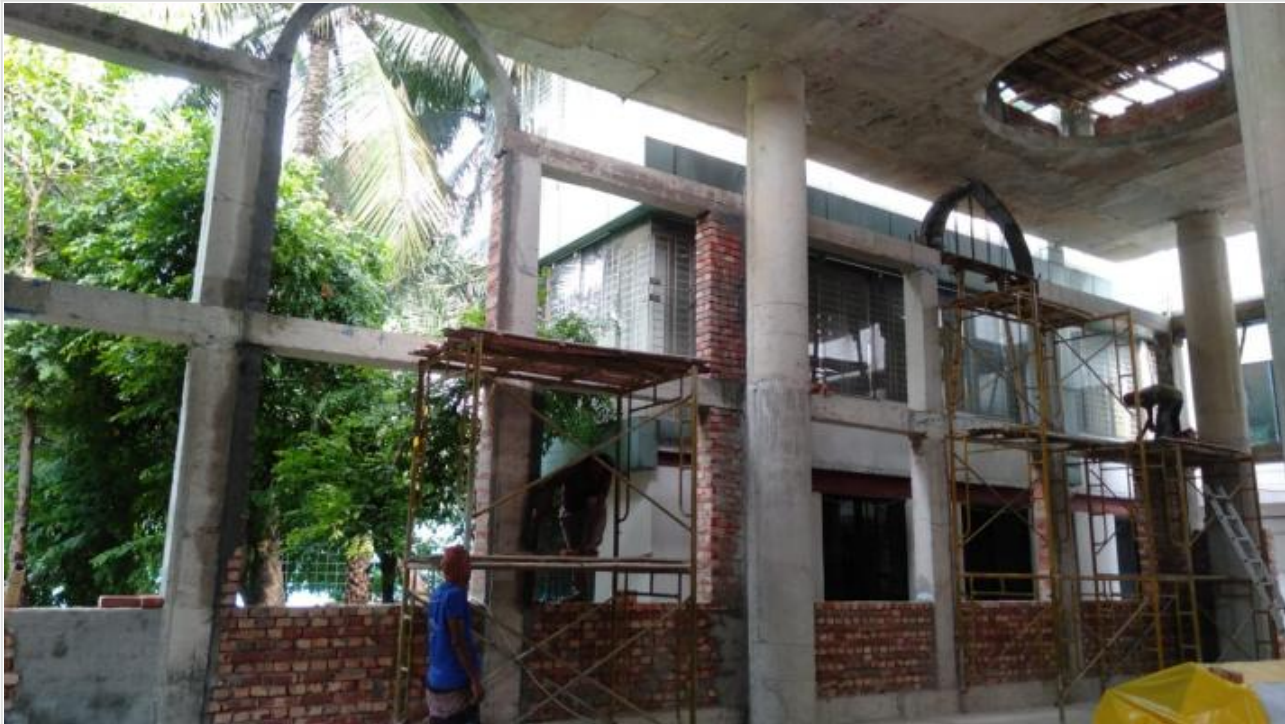
Mosque-Ground Floor-Ancillary Works on 31-05-21
