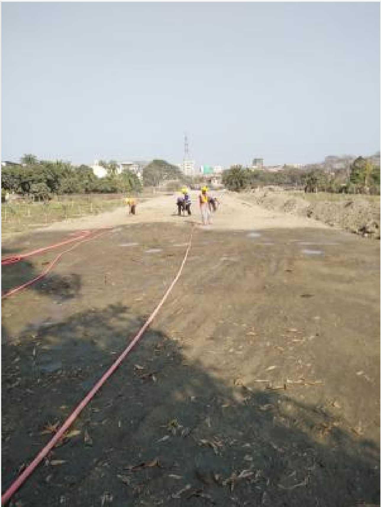
40 ft Road Dressing and Levelling on 28-02-21
