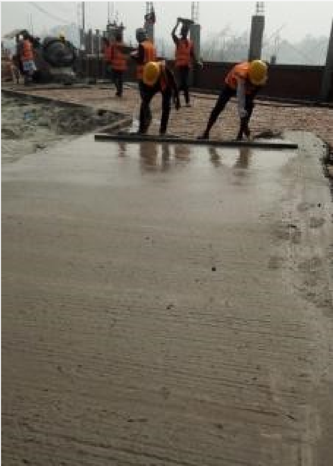
Riverside walkway CC work on 28-01-21
