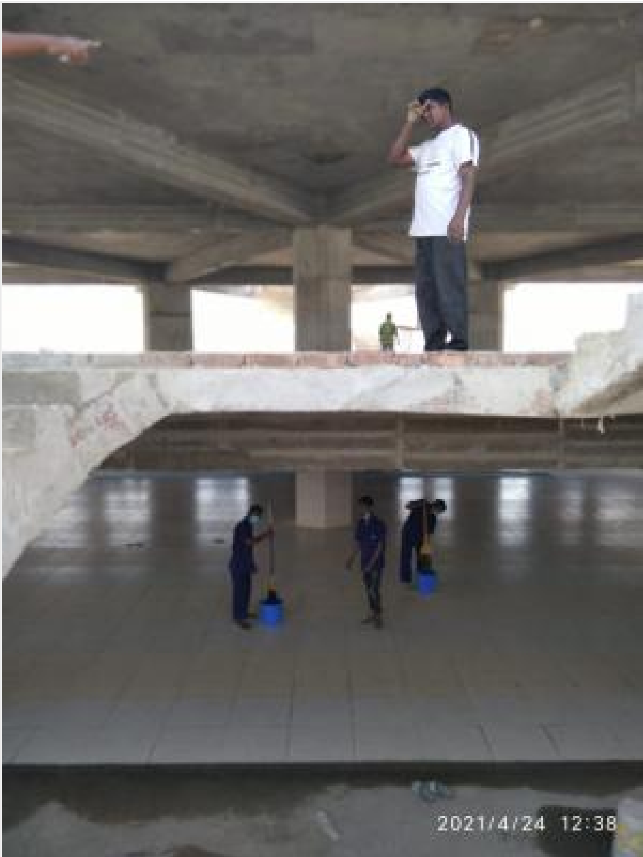
Mosque-Gr.Floor Roof De-shuttering on 24-04-21
