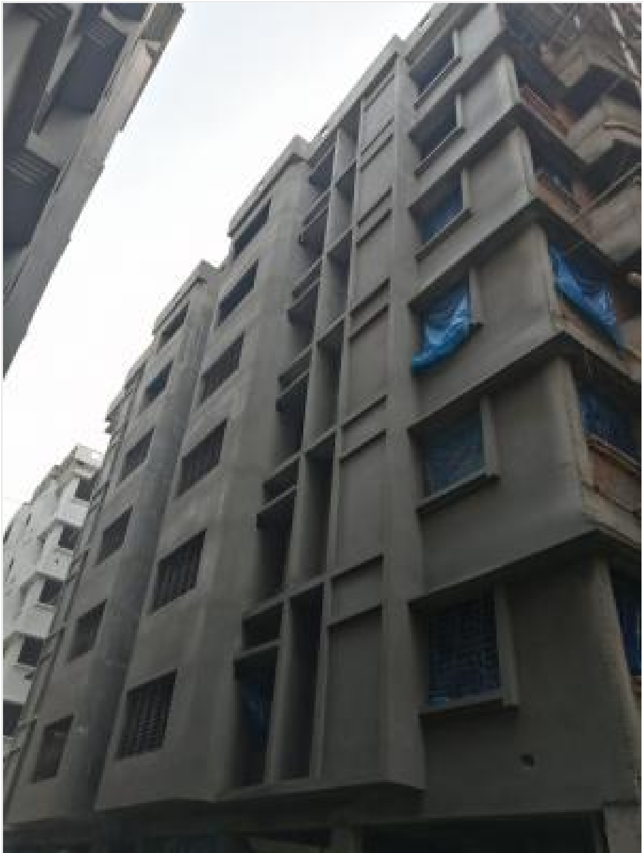
Building-J outside plastering on 28-01-21
