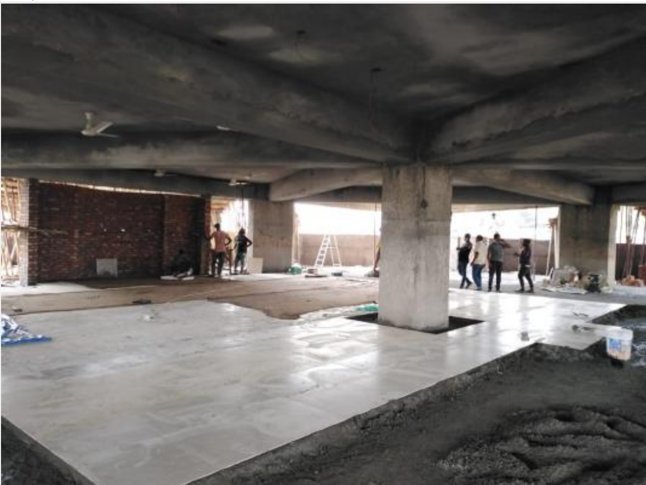
Mosque-Basement Tiles Work on 11-04-21
