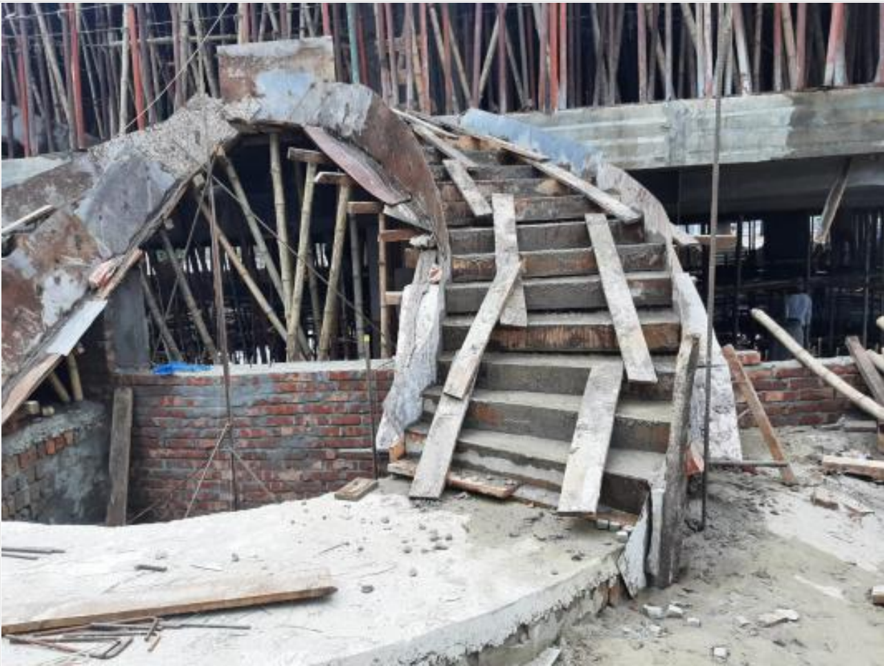
Mosque-Esatside Stair Case on 11-04-21
