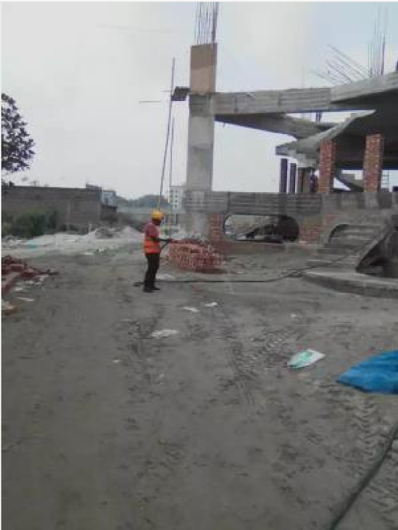
Mosque-Gr/1st Floor-Anciliary works on 04-05-21
