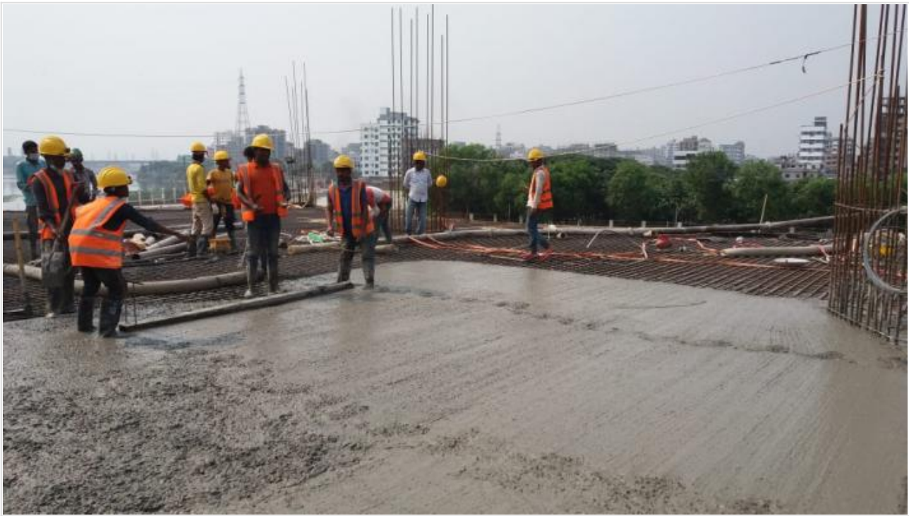
Mosque 1st Floor Slab Concreting on 06-04-21
