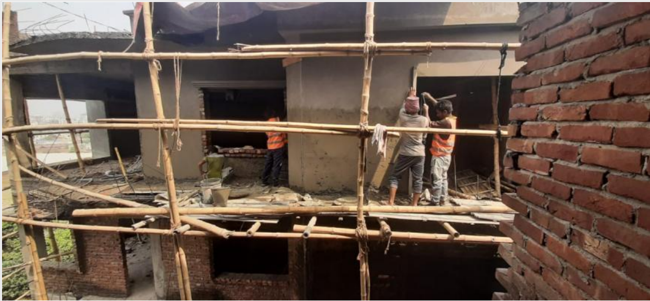
Out-side Plastering on 15-04-21
