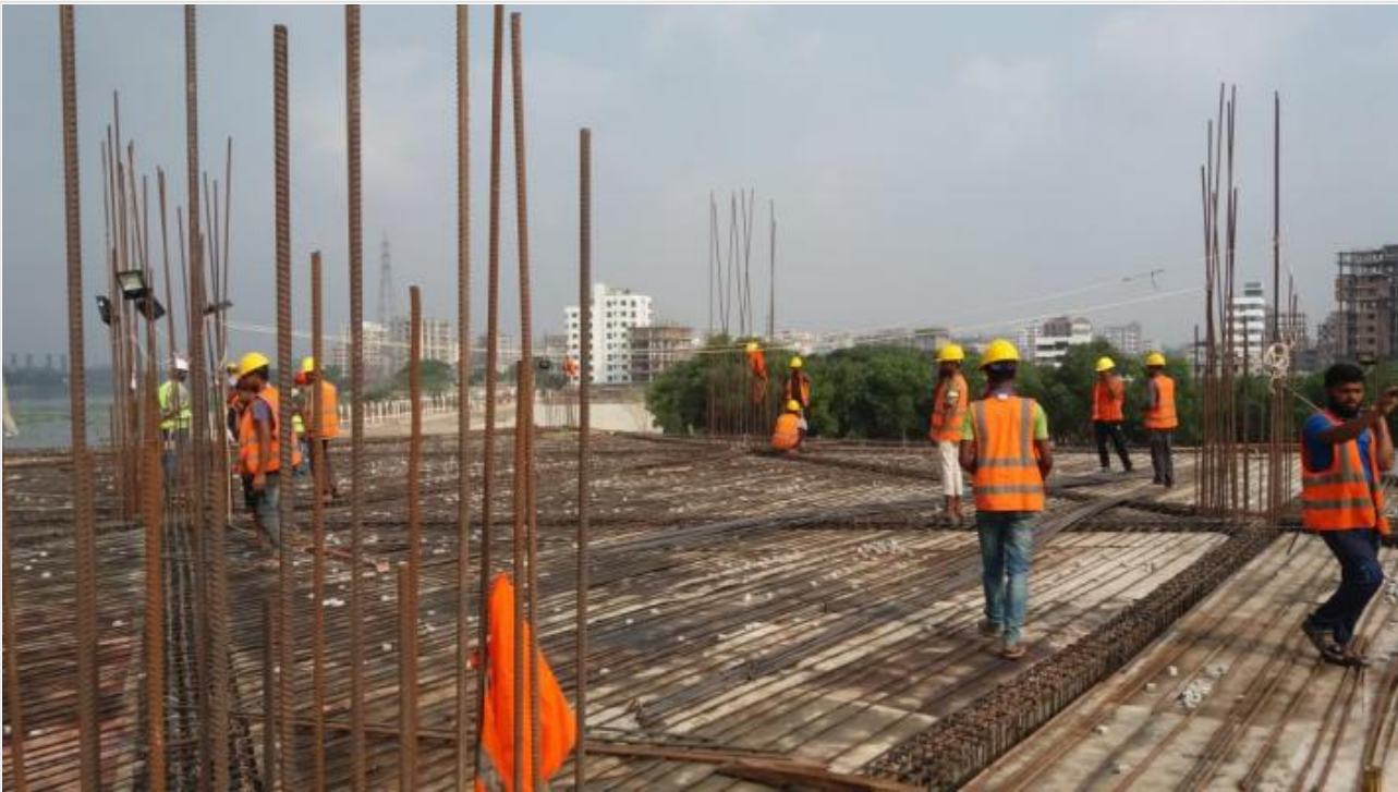
Mosque 1st Floor Slab Re-bar Work on 03-04-21
