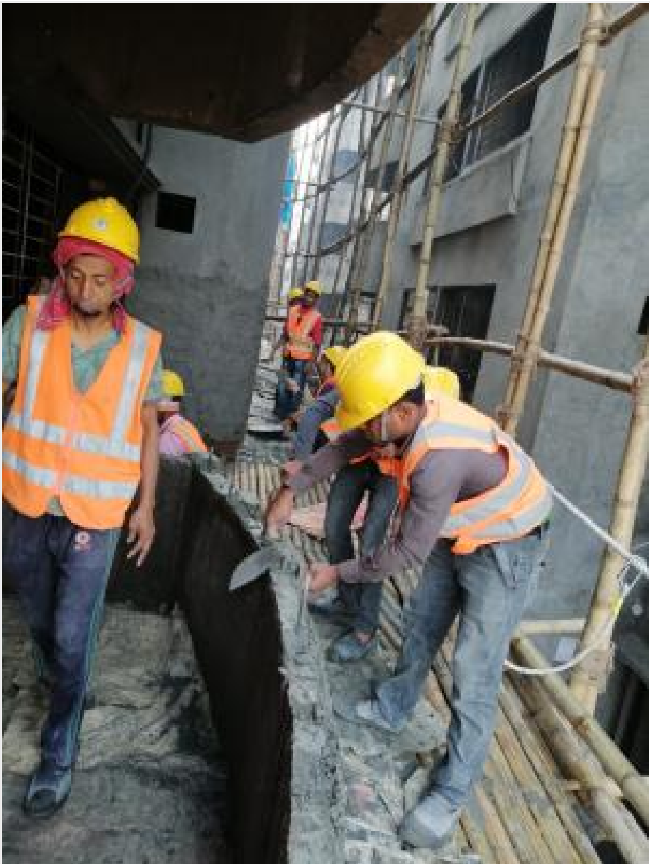
Out-side Plaster Work on 05-02-21
