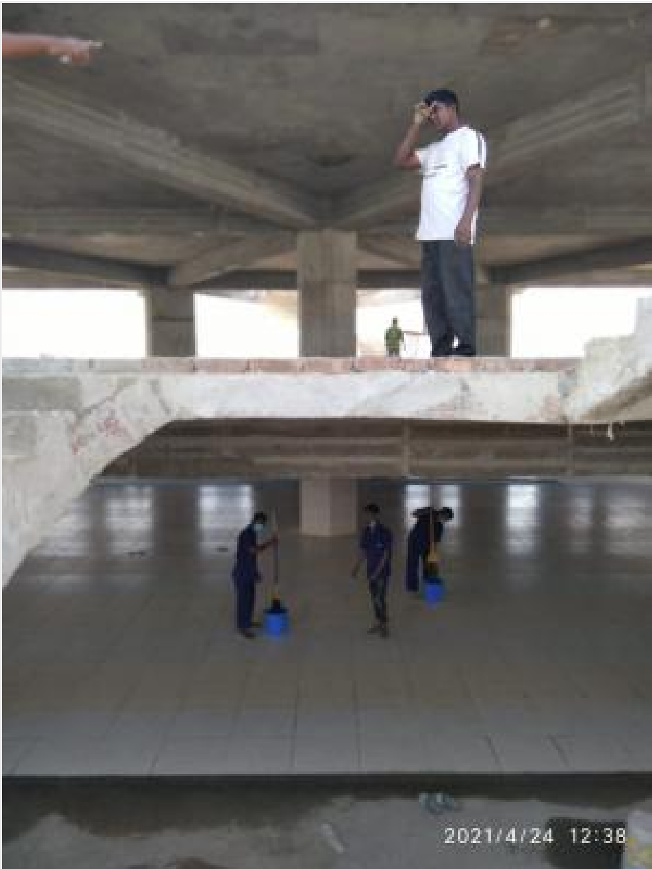
Mosque-Gr.Floor Roof De-shuttering on 24-04-21
