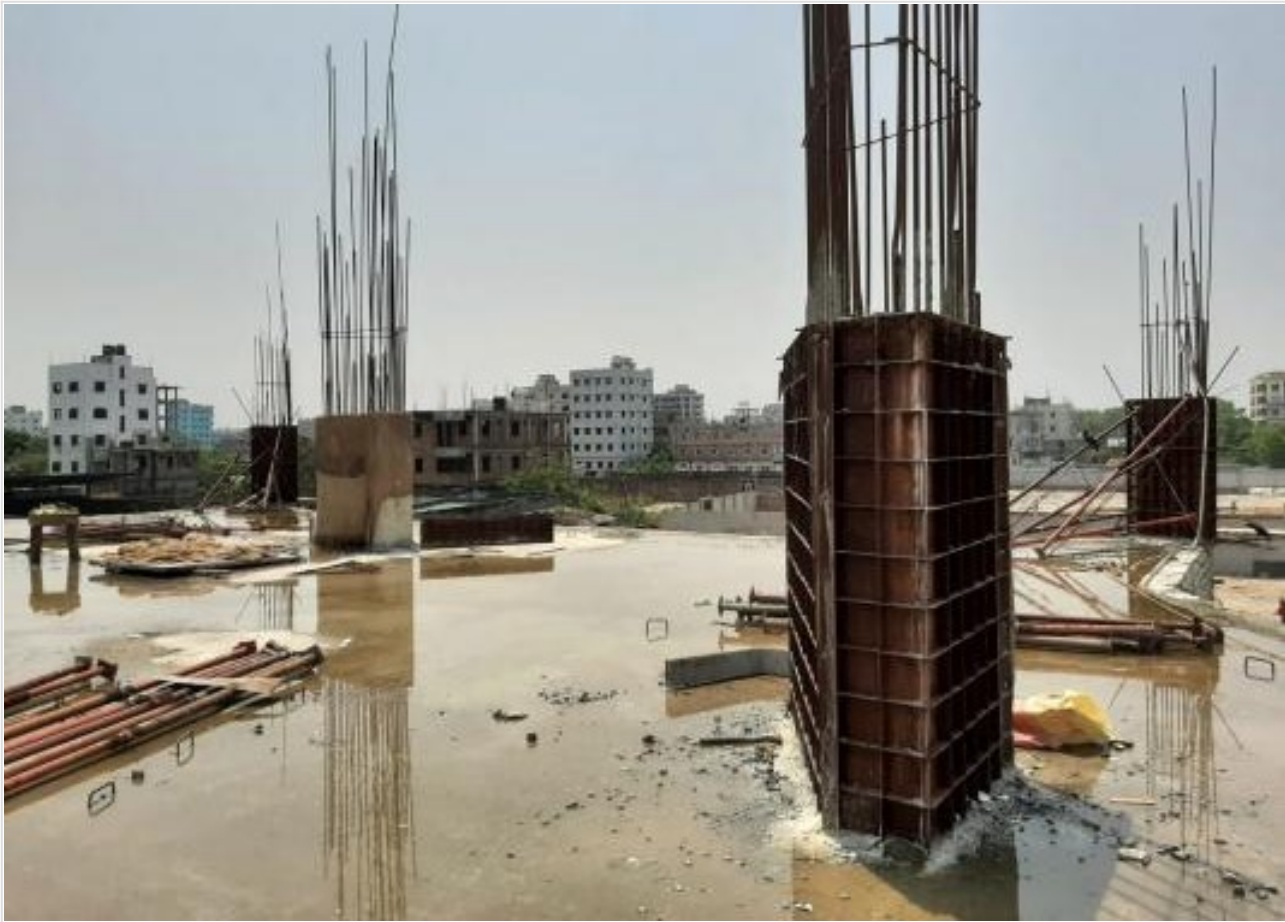
Mosque-1st Floor-Column Shuttering on 26-04-21
