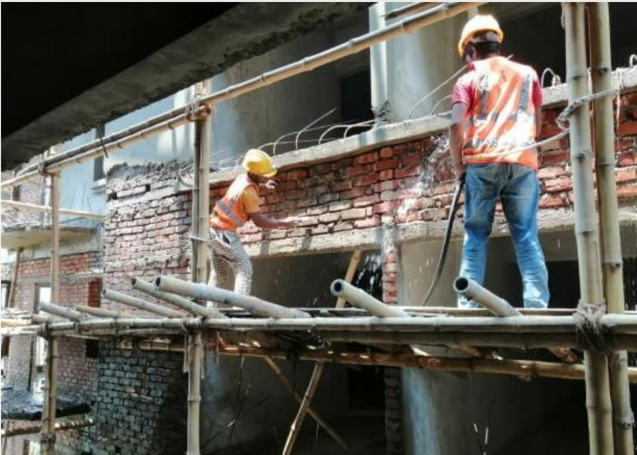
Out-side Plastering on 17-04-21
