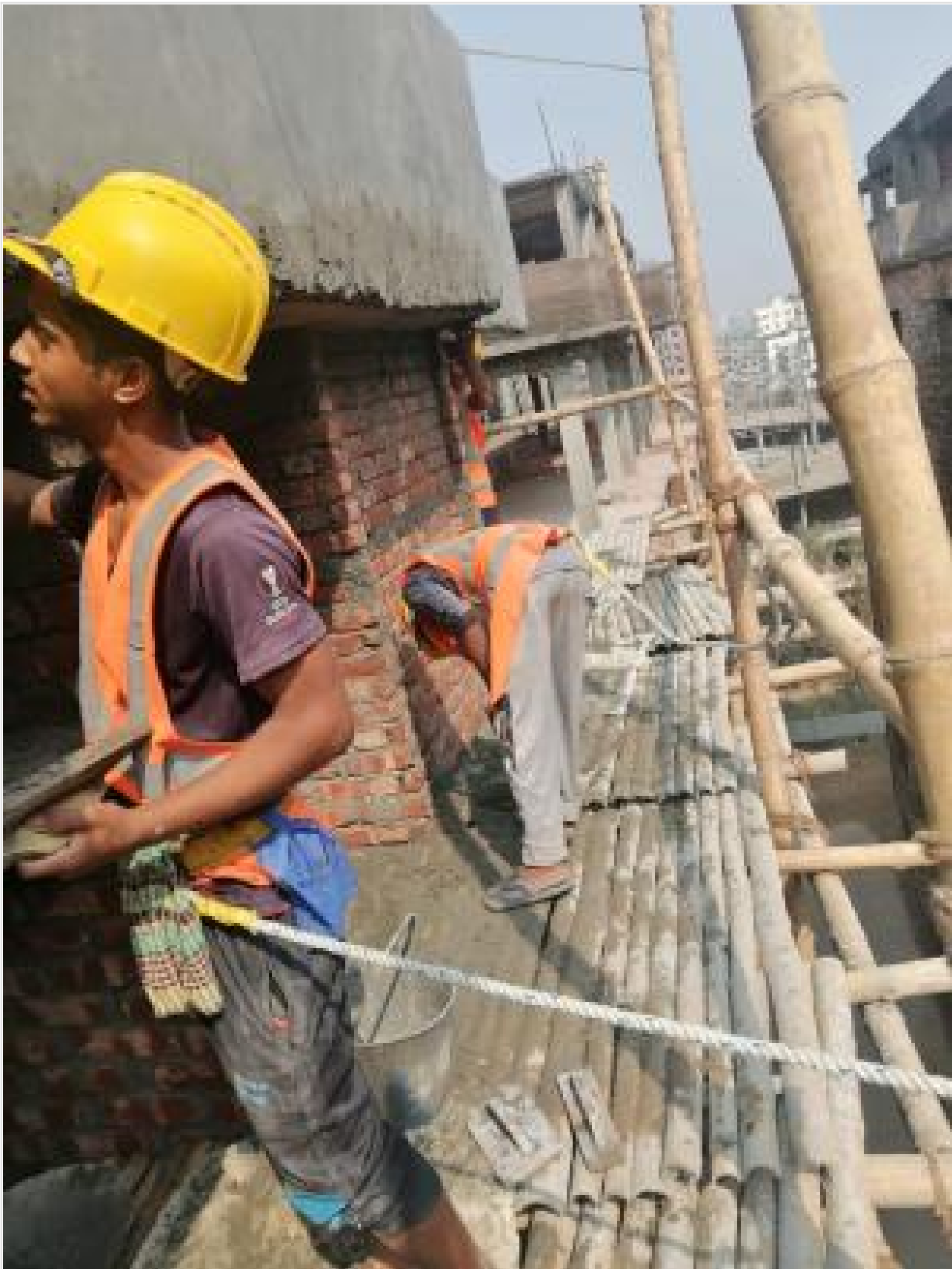
Building Outside Plastering on 01-03-21
