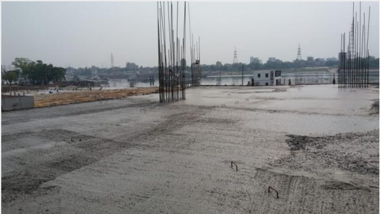
Mosque 1st Floor Slab Concreting on 06-04-21
