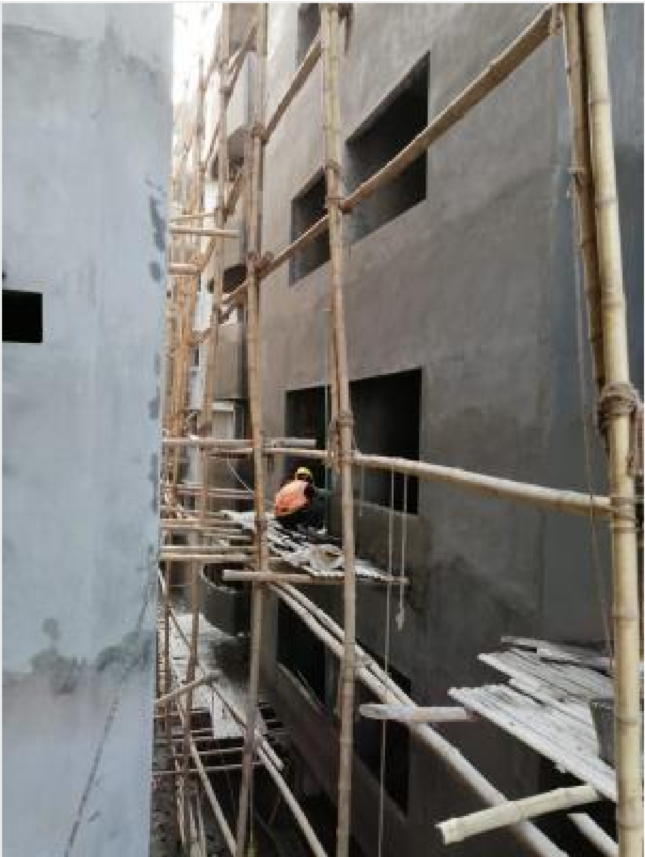
Bulding-Q-Out-side Plastering on 09-05-21
