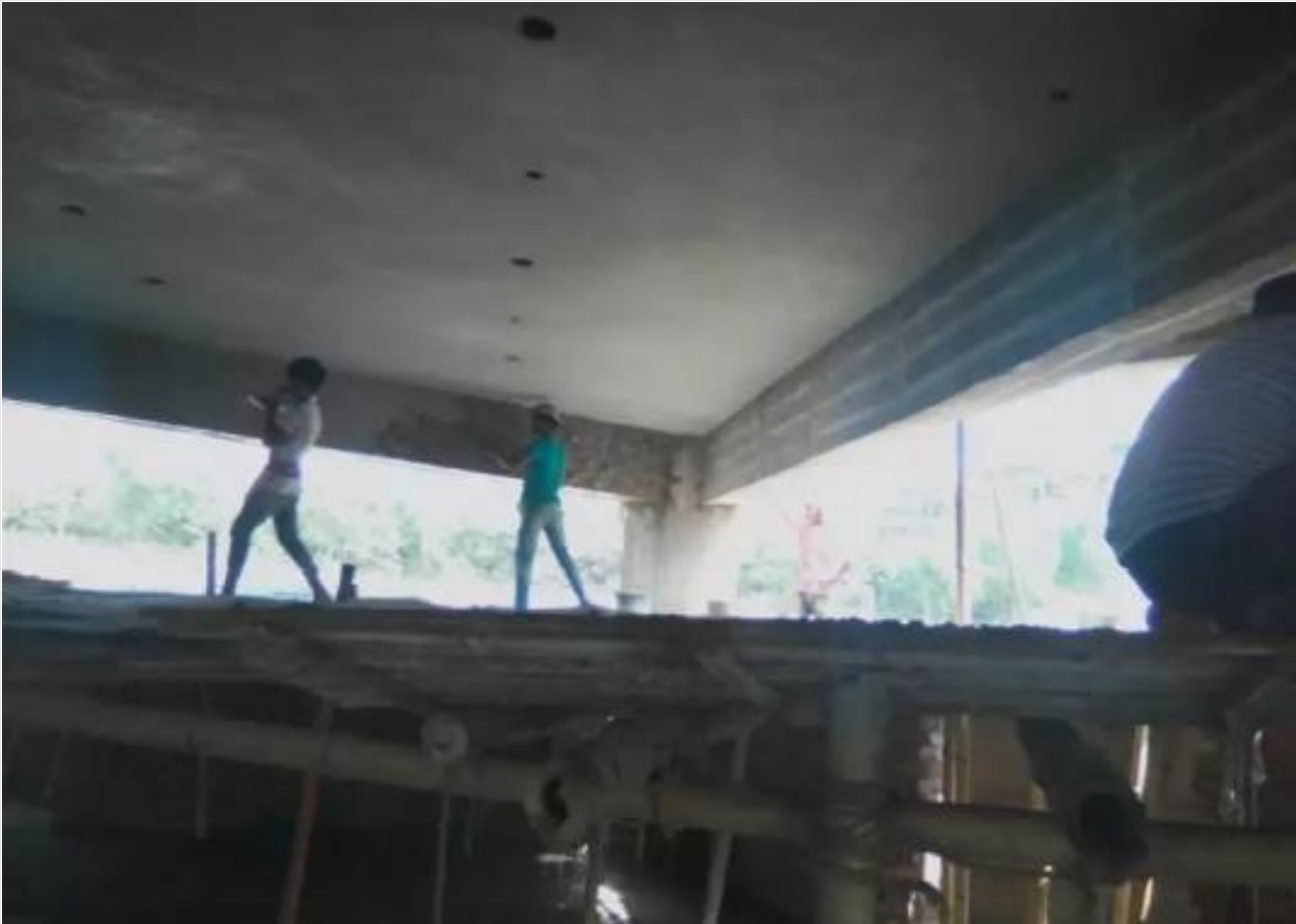
Mosque-Basment Plaster Work on 14-04-21
