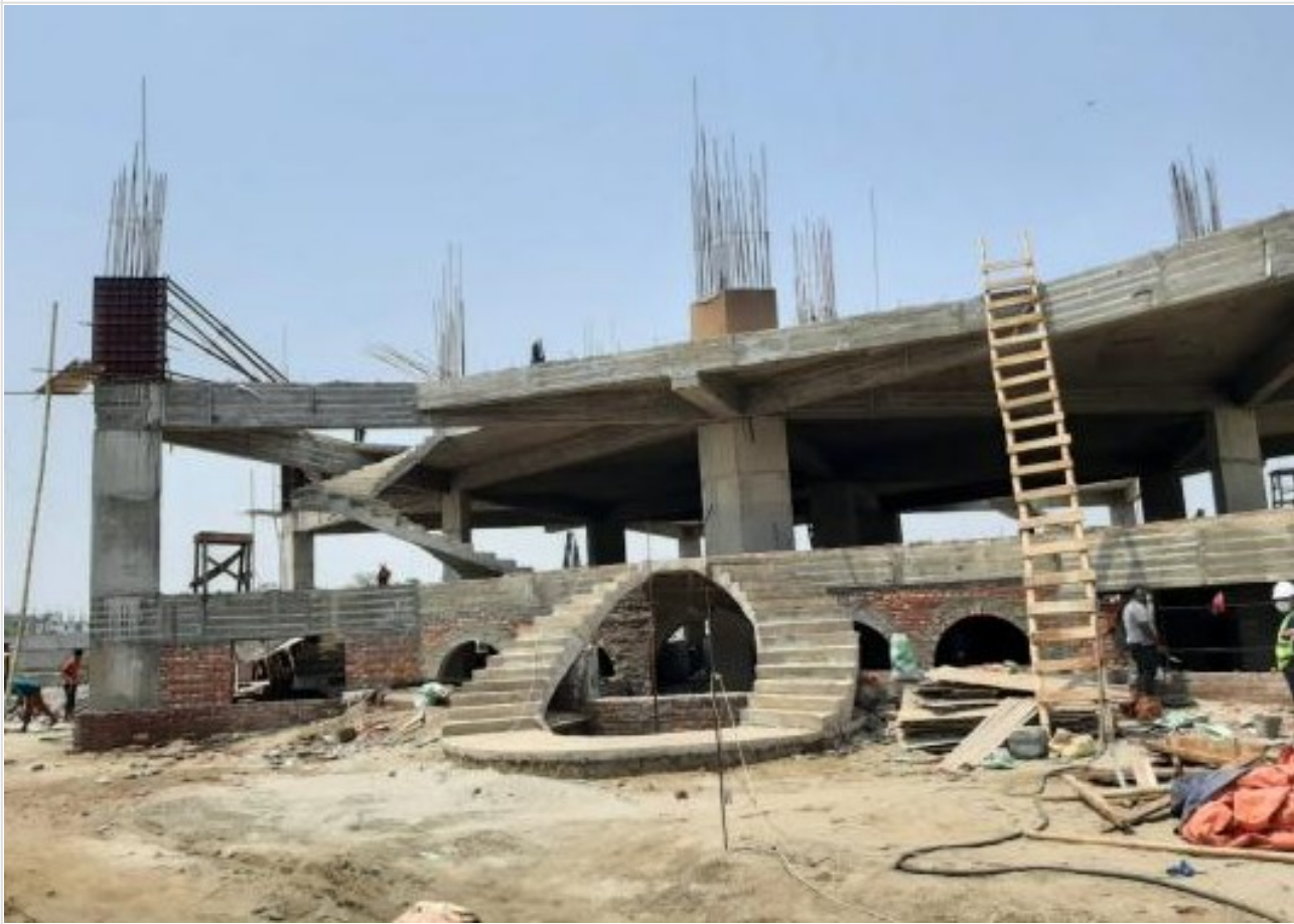
Mosque-Basement-Ancillary Work on 26-04-21
