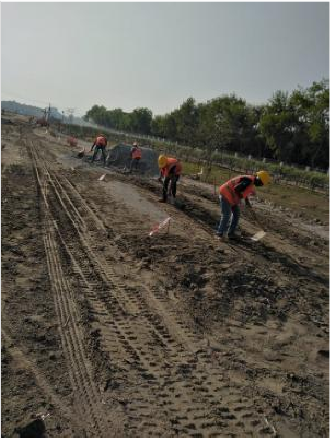
40 ft Road Levelling and dressing on 10-02-21
