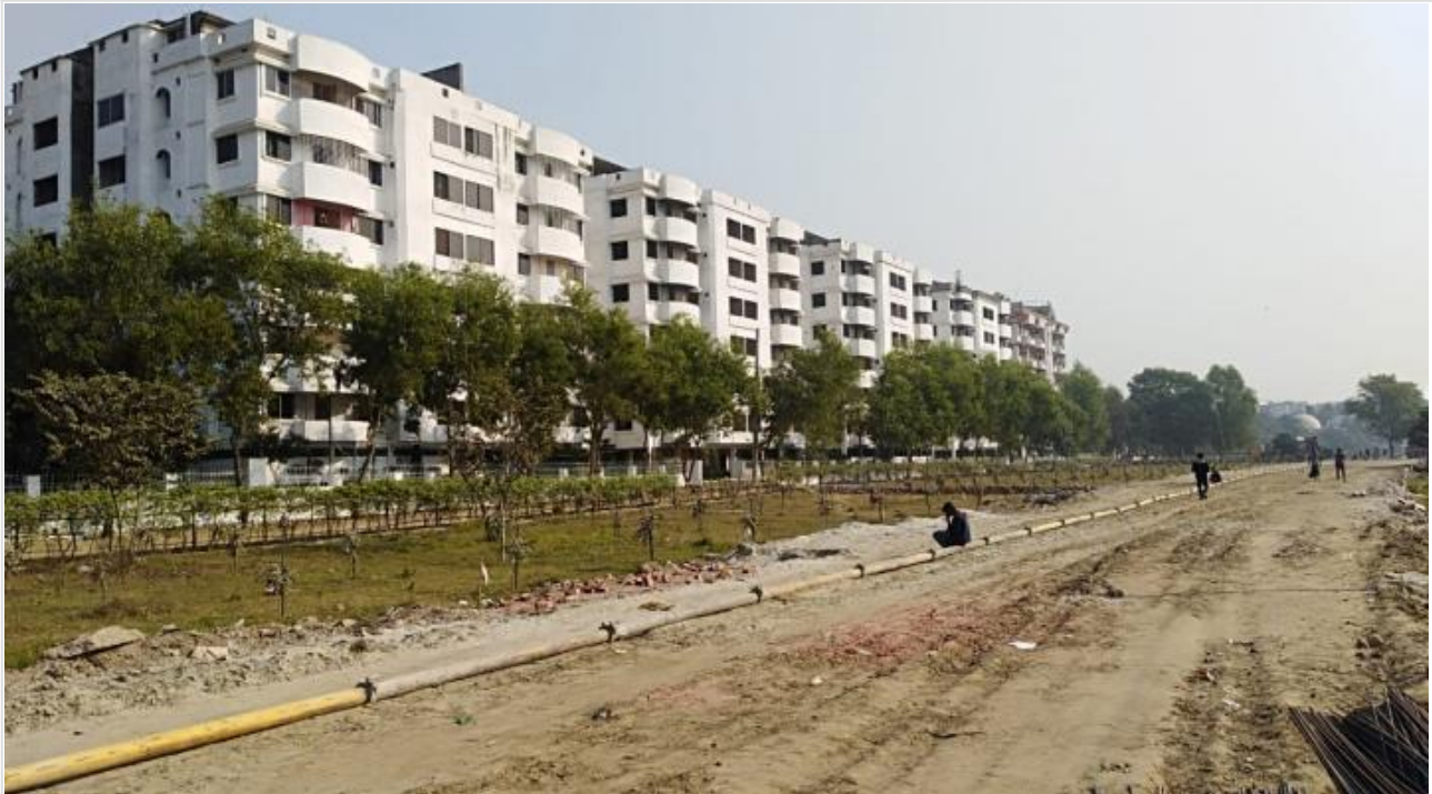
Building Outside Painting on 08-02-21
