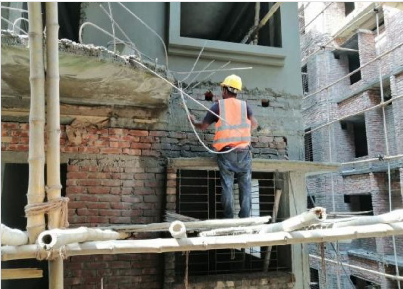
Out-side Plastering on 20-04-21
