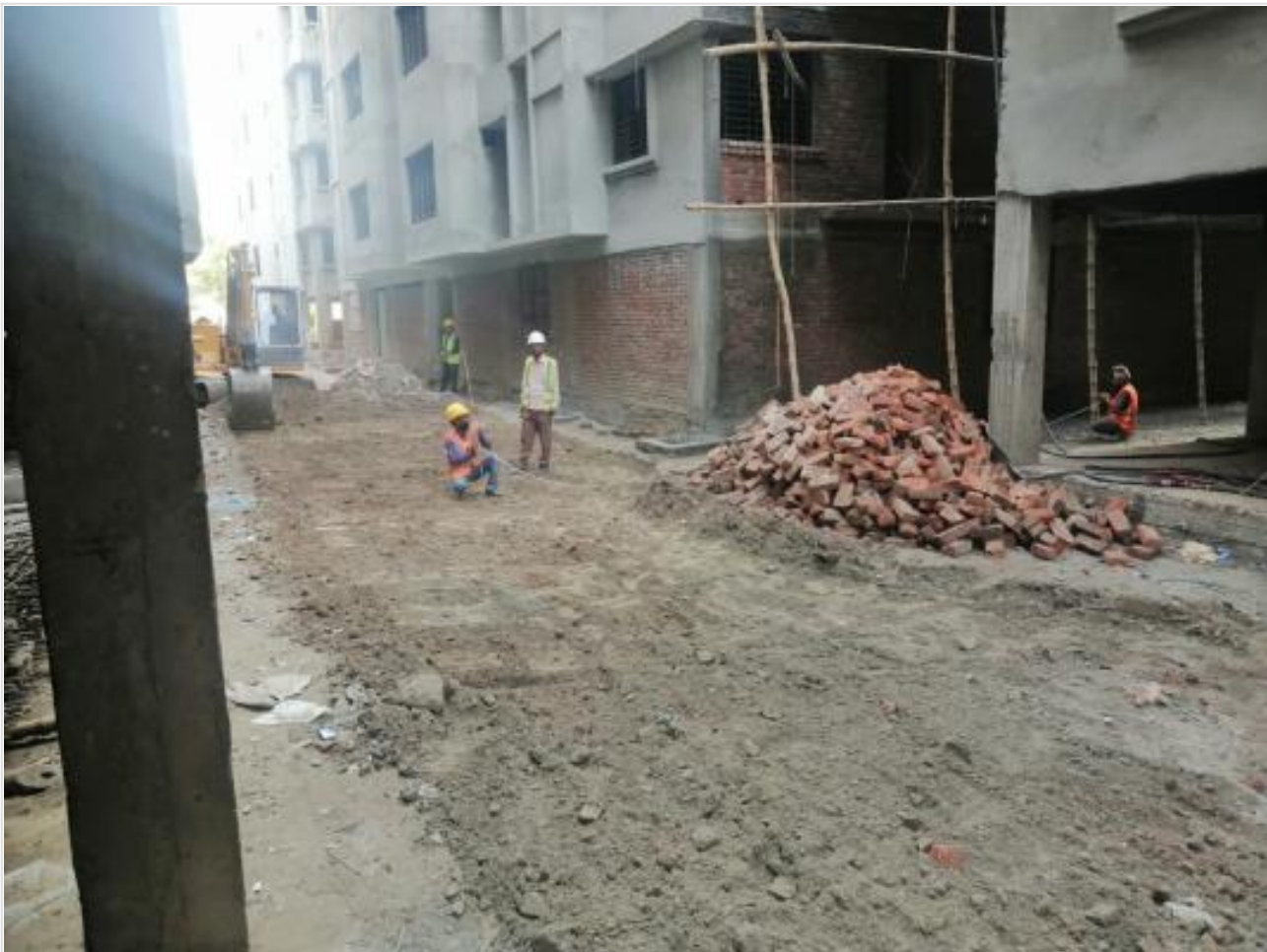
12 ft Road Filling on 28-02-21
