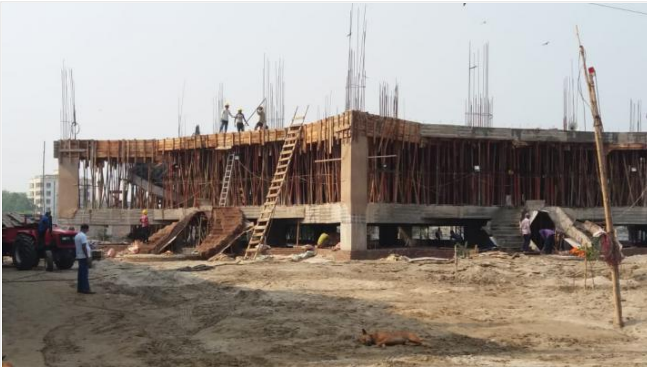
Mosque under Construction on 13-04-21
