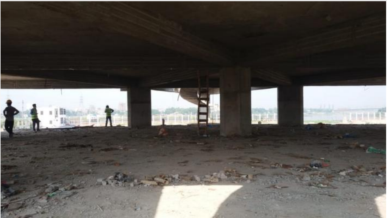
1st Floor Roof-De-shuttering on 25-04-21
