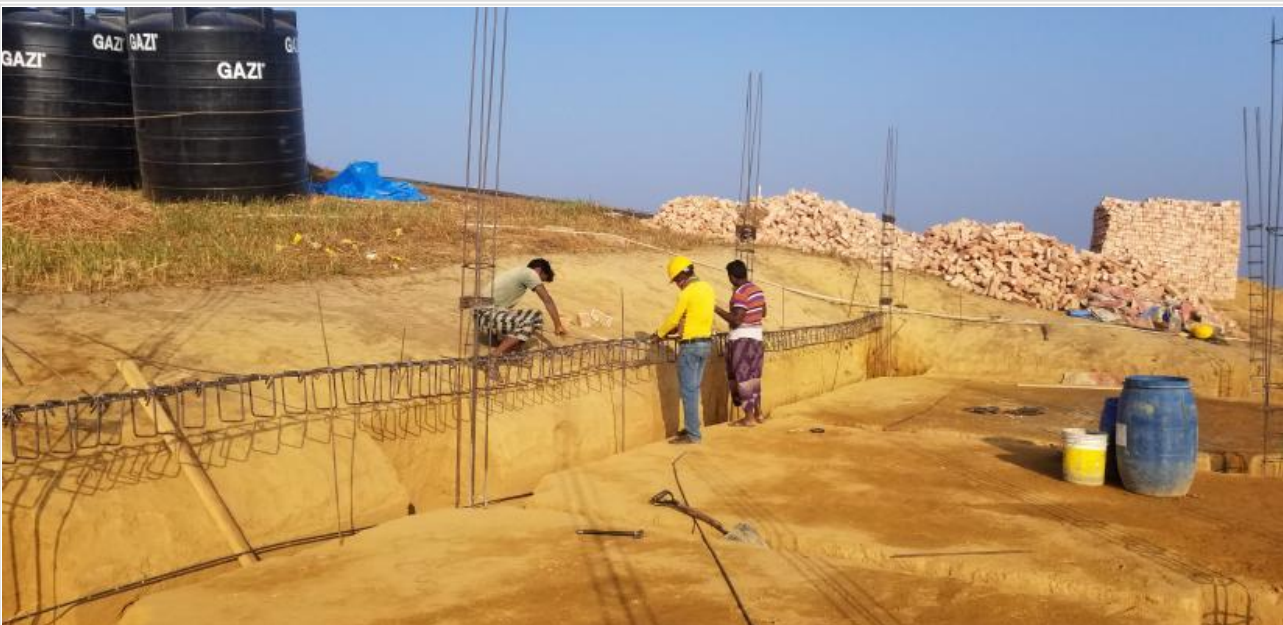
MS rod cutting & binding work for grade on 19-01-21
