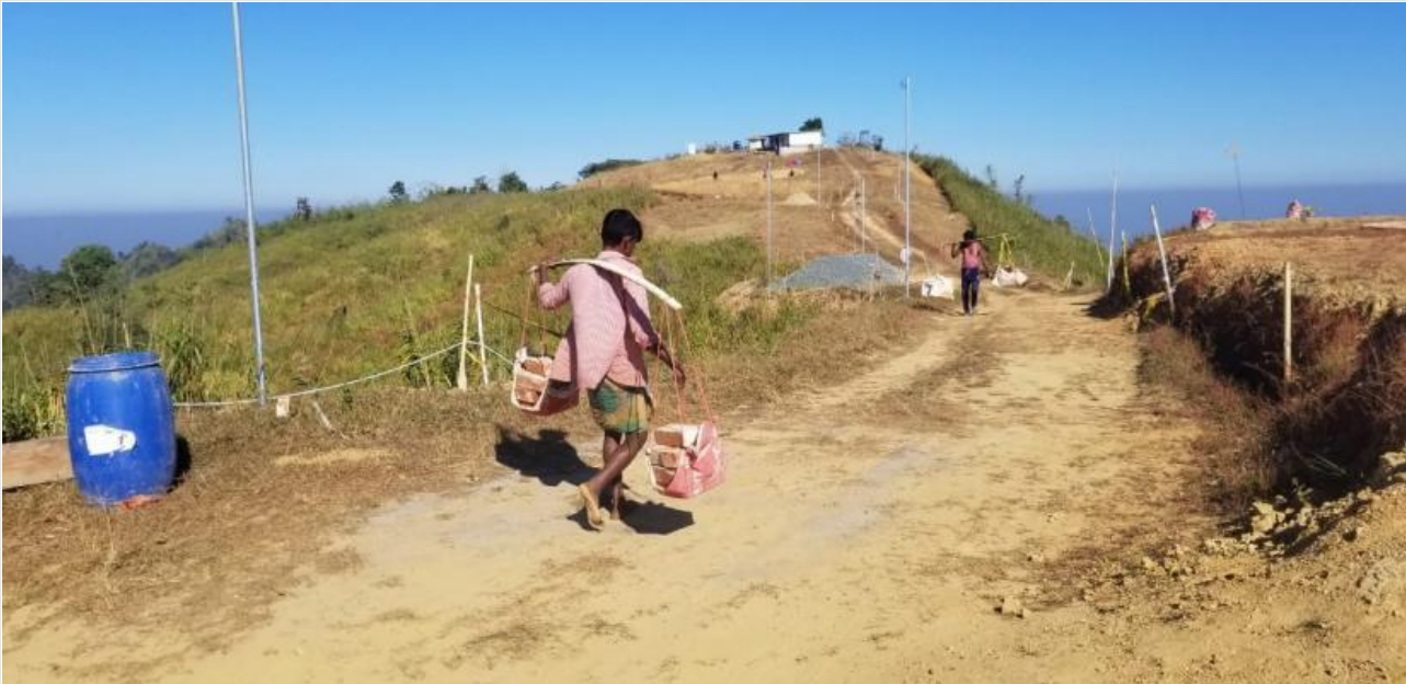
Brick Carrying on 09-01-21
