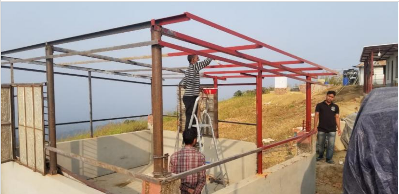
Mechanics Shed Frame Work on 20-01-21
