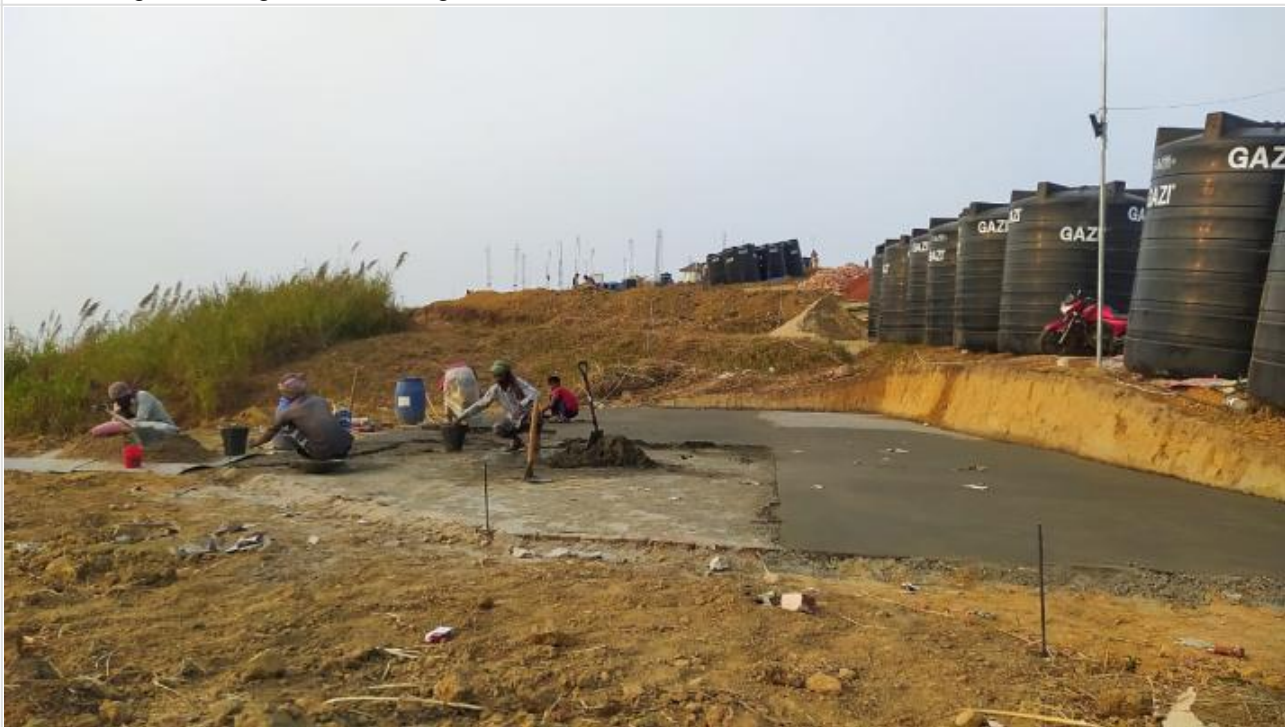
Solling joint fillup & plaster work at w on 21-01-21
