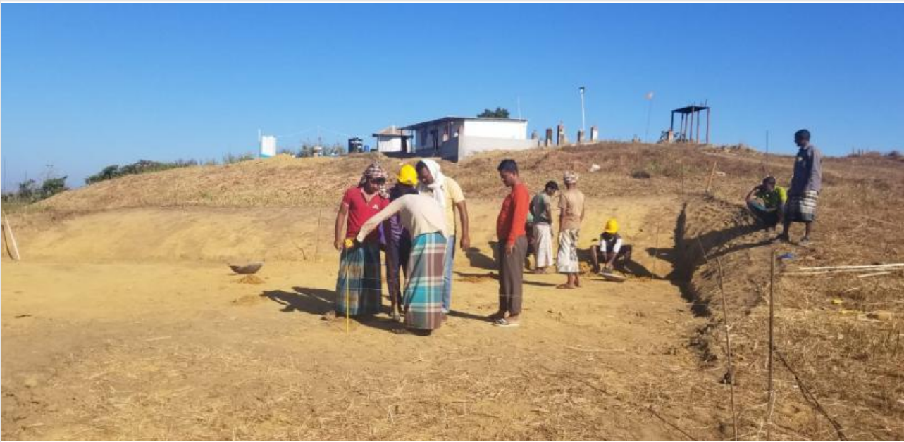
Guest House-Preparation for Layout on 05-01-21
