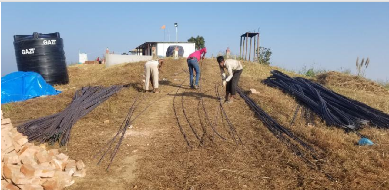
MS rod cutting & binding on 12-01-21
