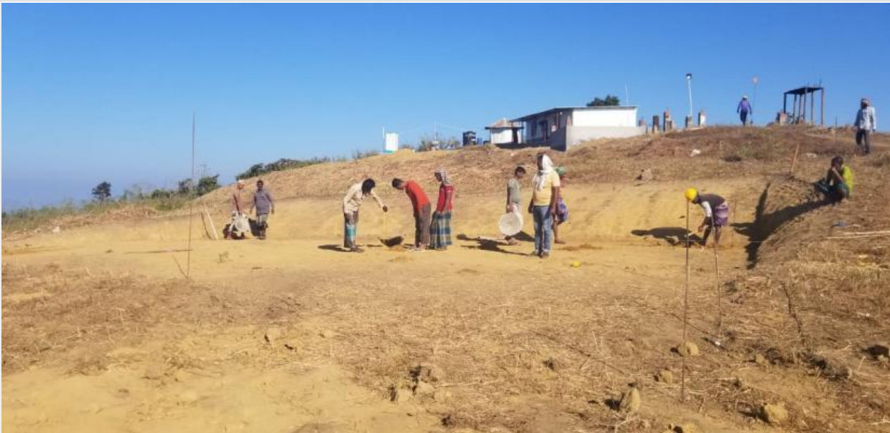
Guest House-Preparation for Layout on 05-01-21
