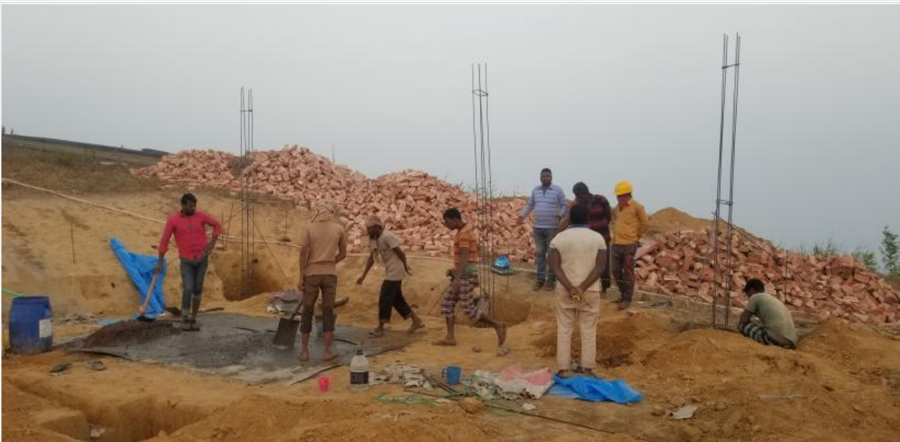
Footing & column casting work on going on 13-01-21
