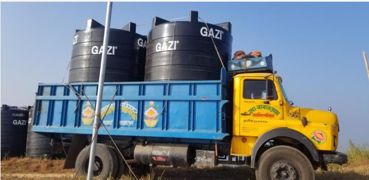
Reached water tank at project on 13-01-21
