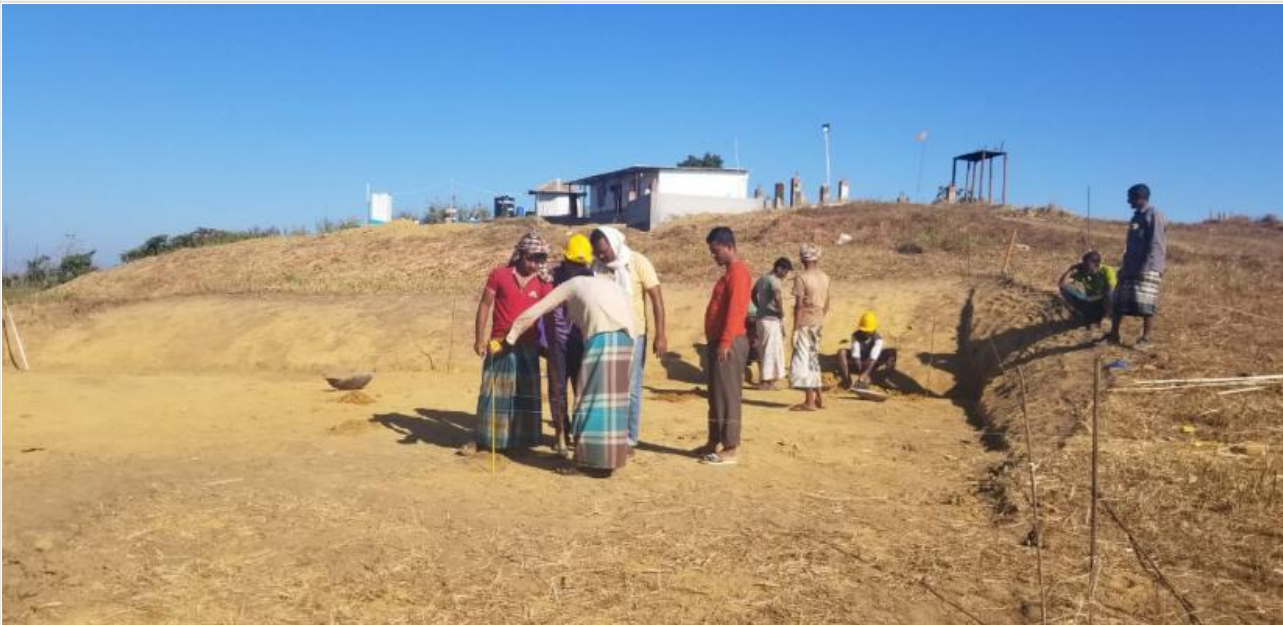
Guest House-Preparation for Layout on 06-01-21
