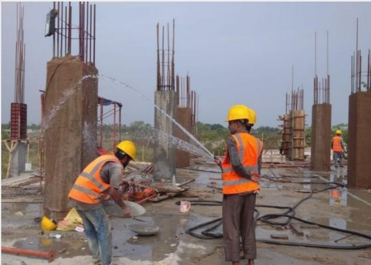
Column Curing on 09-05-21
