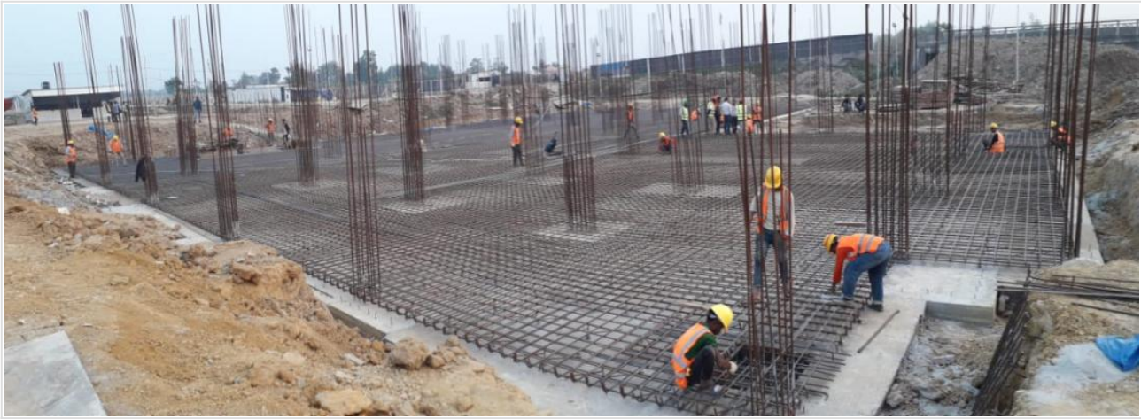
Mat Re-bar Work on 29-12-20
