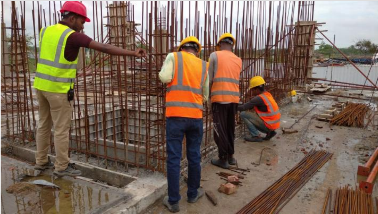
Ground Floor-Lift Core-Re-bar Work on 25-05-21
