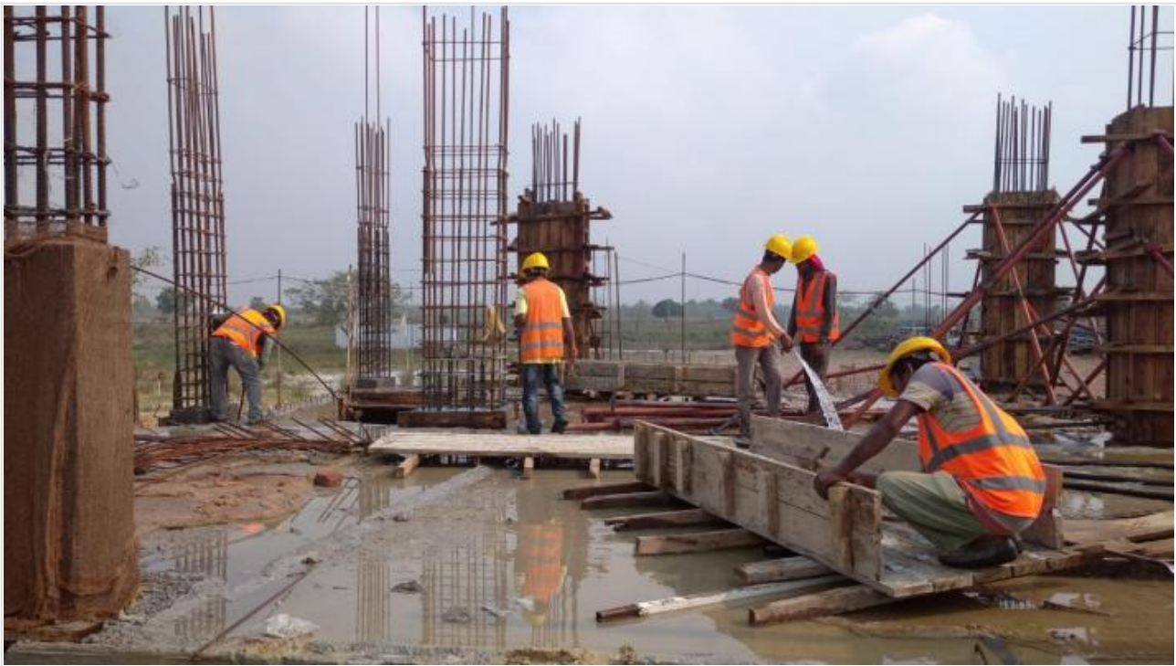
Column Shuttering Work on 04-05-21
