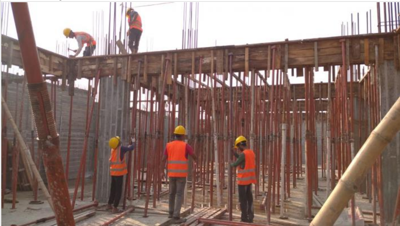
Ground Floor Slab Shuttering on 25-02-21
