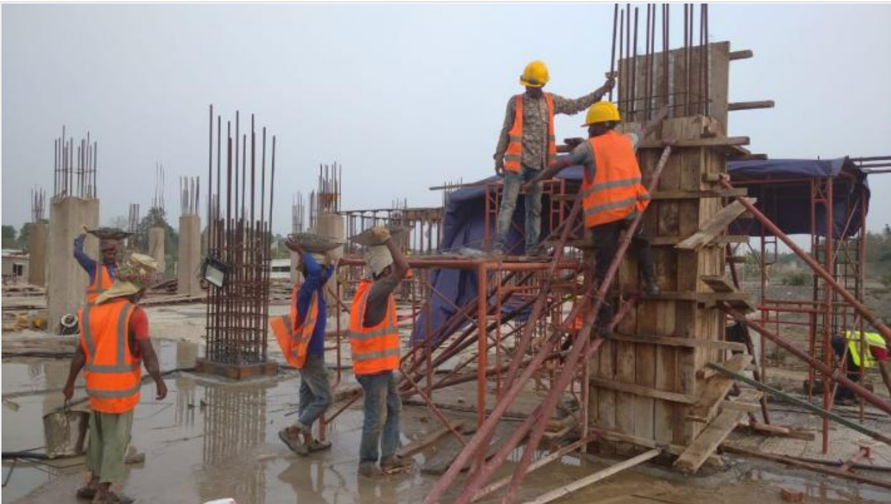
Column Re-bar Work on 04-05-21
