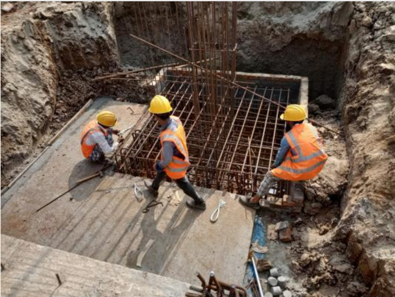
Footing Re-bar Placing on 19-12-20
