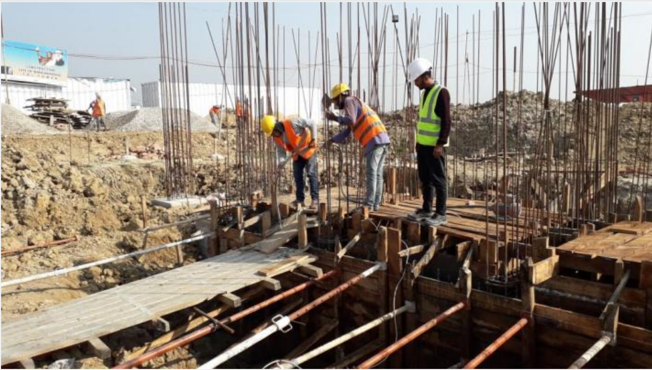
Lift Core Concreting on 19-12-20
