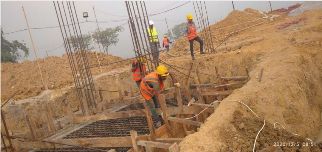
Pile Cap Re-bar Shuttering Work on 05-12-20
