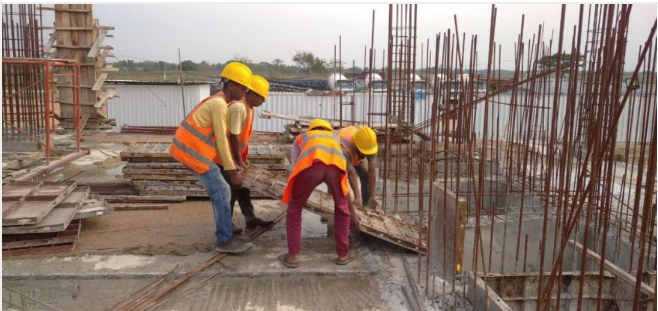
Column Re-bar Work on 08-05-21
