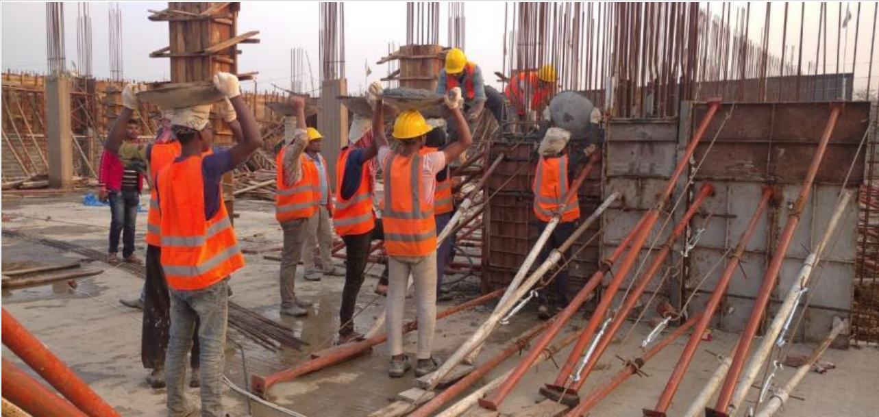
Retaining wall and Column Concreting on 28-01-21
