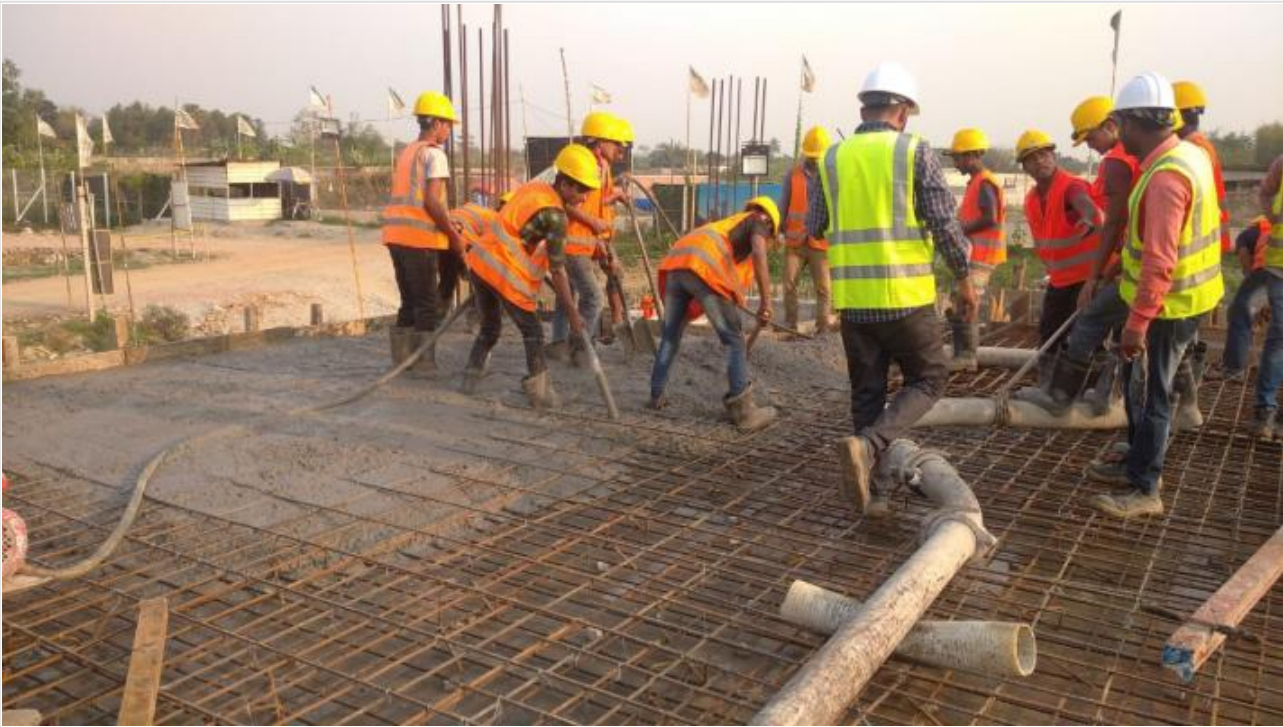
GF North-Slab 8000 sft Concreting on 15-03-21
