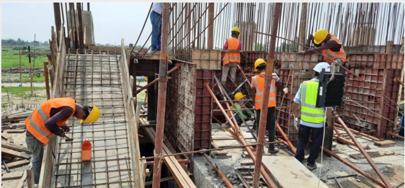
Ground Floor Stair Re-bar work on 09-06-21
