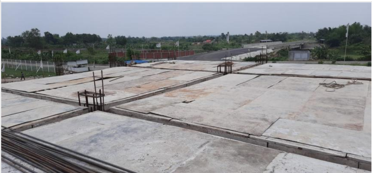
1st floor Slab Shuttering on 09-06-21
