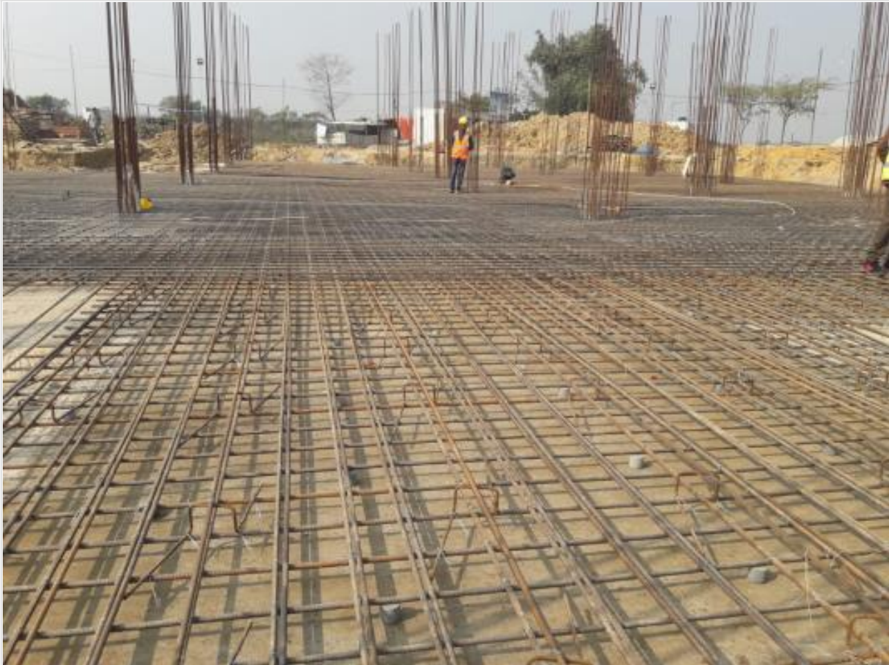
Mat Re-bar Work on 29-12-20
