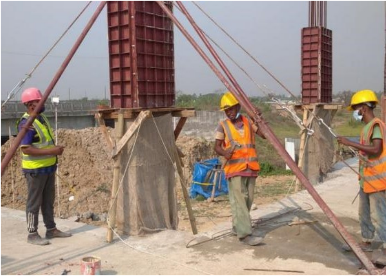
Column Shuttering on 09-05-21
