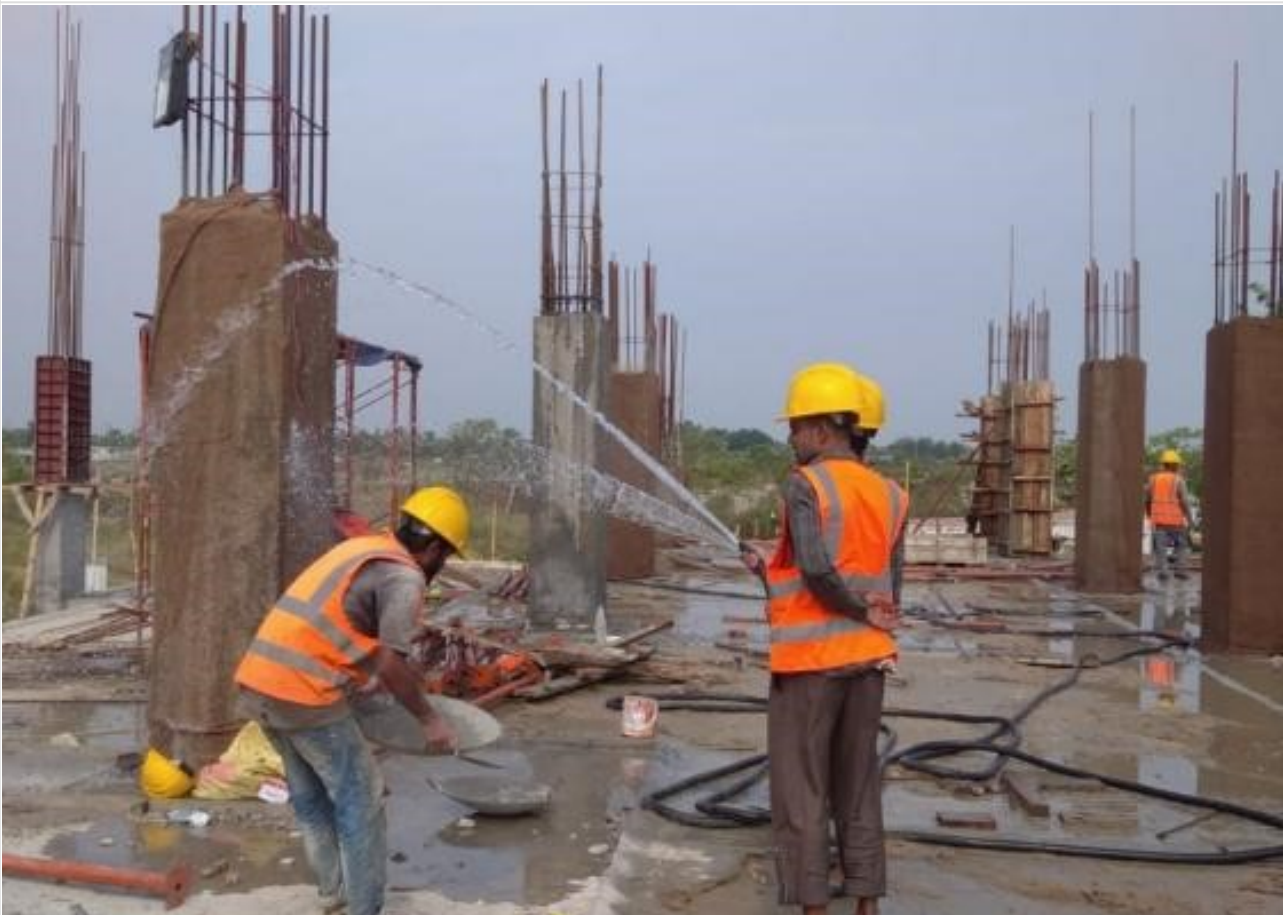
Column Curing on 09-05-21
