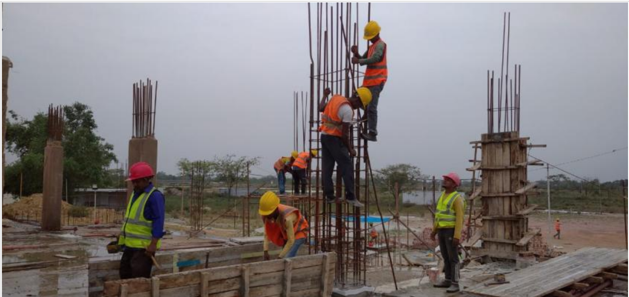
Column Re-bar Work on 08-05-21
