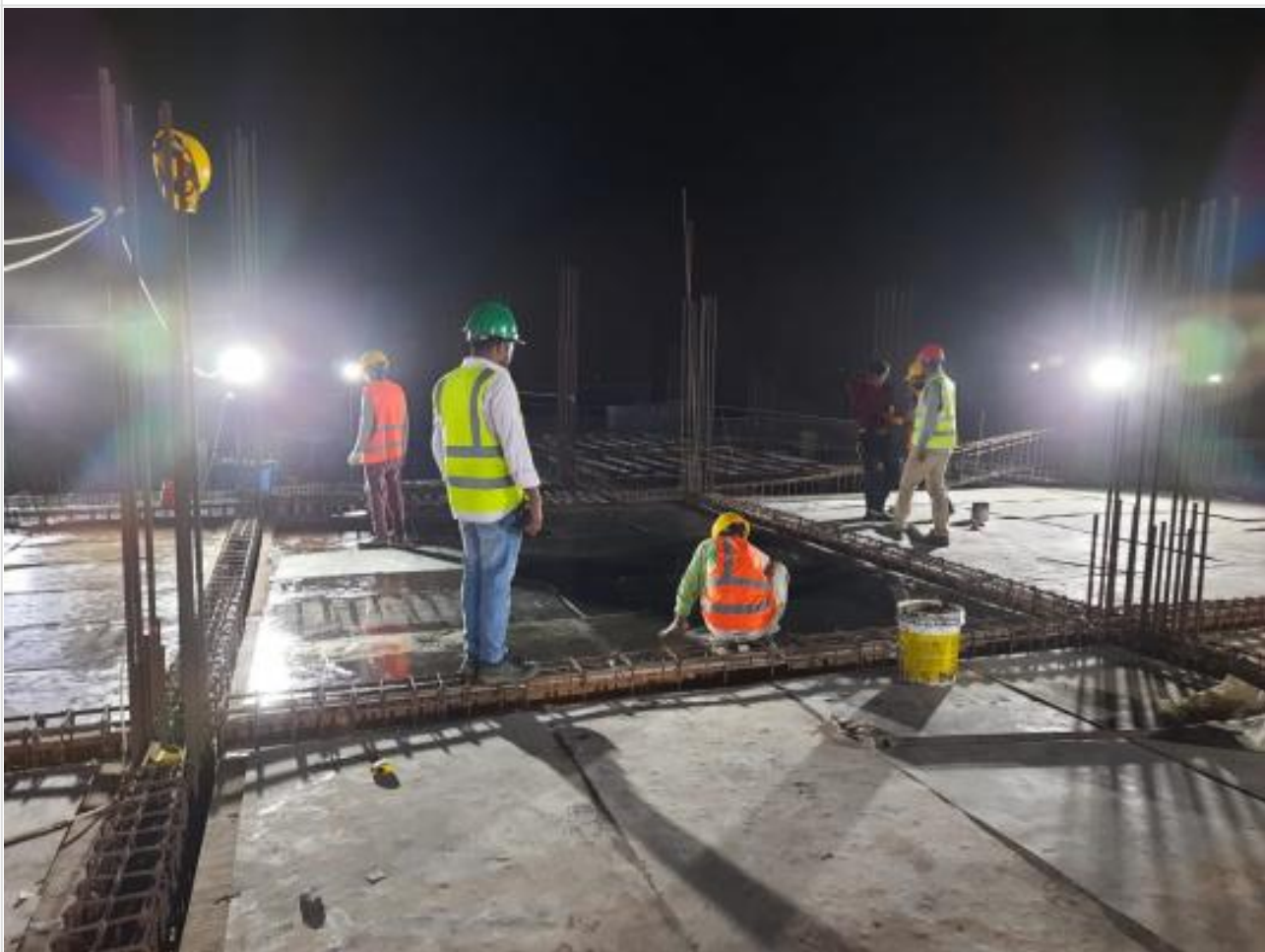
GF Slab Shuttering at Night Shift on 10-03-21
