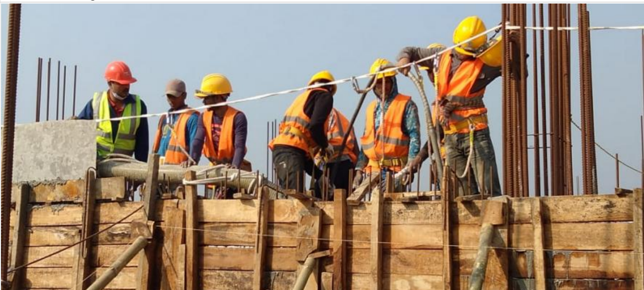
South Retaining wall 2nd Lift Concretin on 09-02-21
