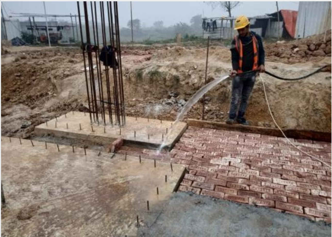
Footing Curing on 15-12-20
