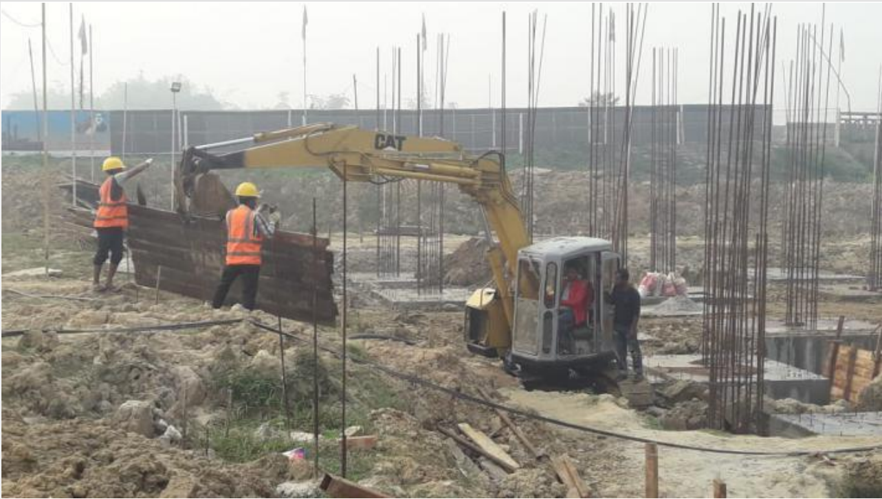
Pile Cap Re-bar Shuttering Work on 05-12-20
