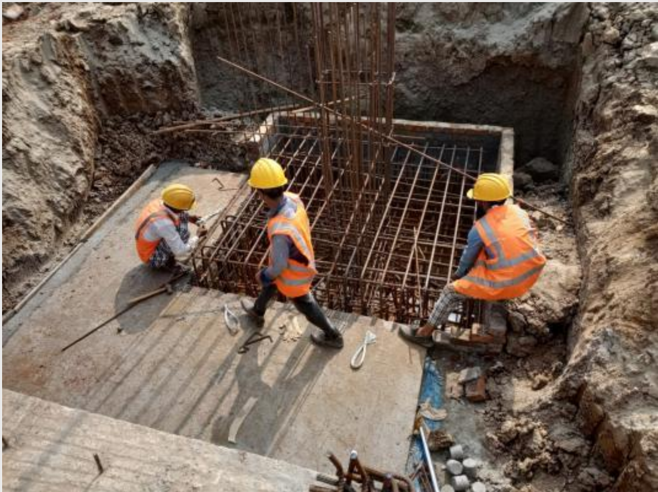
Footing Re-bar Placing on 19-12-20
