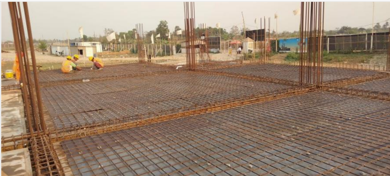
Ground Floor Slab Re-bar Work on 10-03-21
