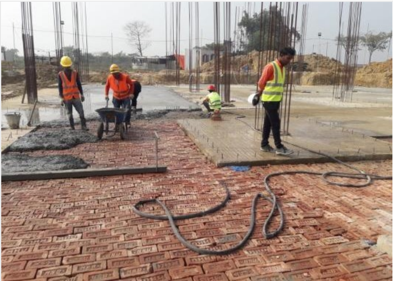
Mat CC Concreting on 15-12-20
