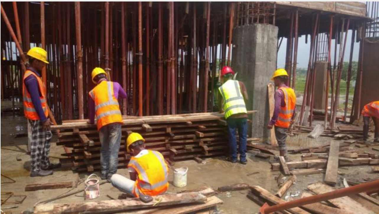
1st floor Slab Shuttering on 15-06-21
