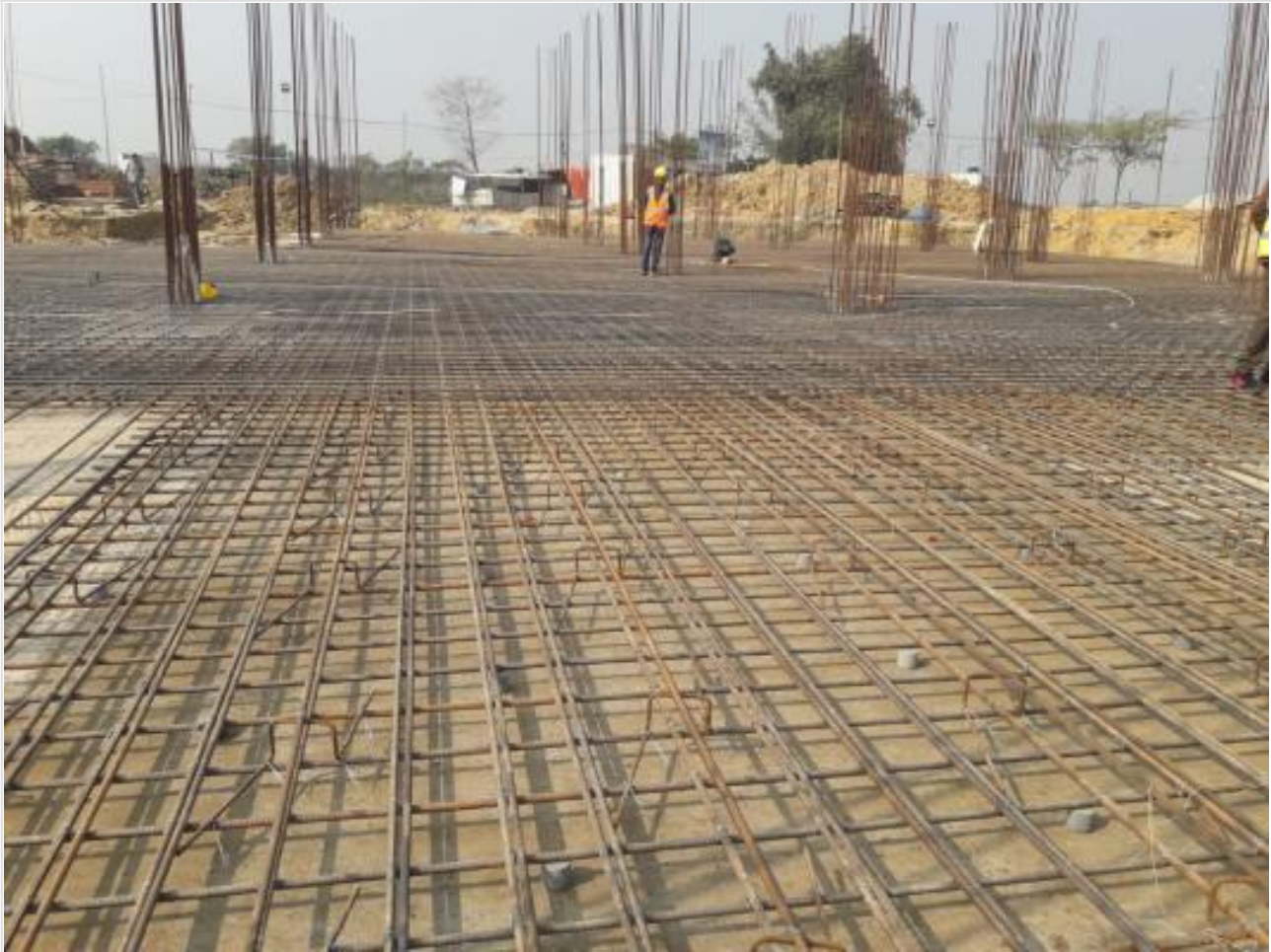
Mat Re-bar Work on 29-12-20
