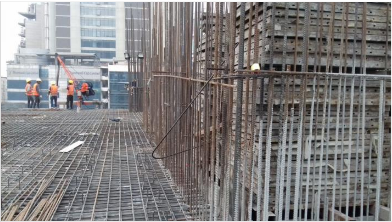
Roof Slab on 01-02-21
