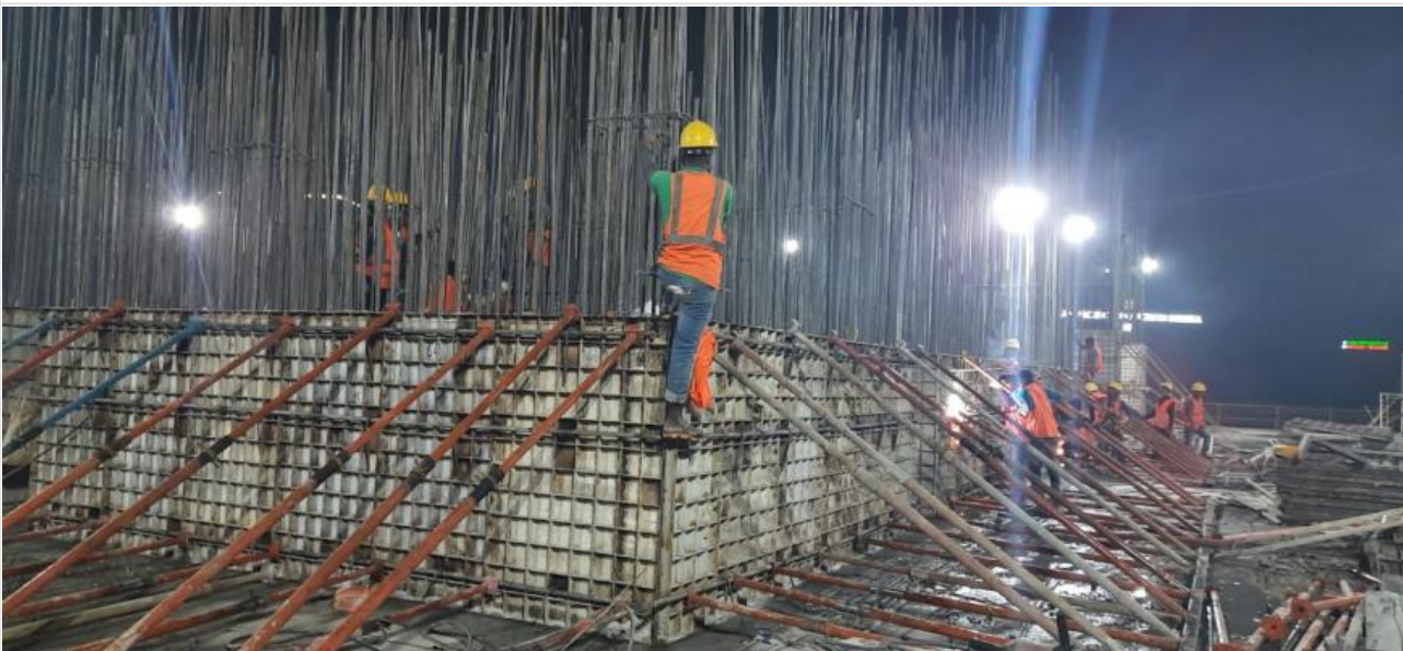
Lift Core Wall Shuttering on 16-01-21
