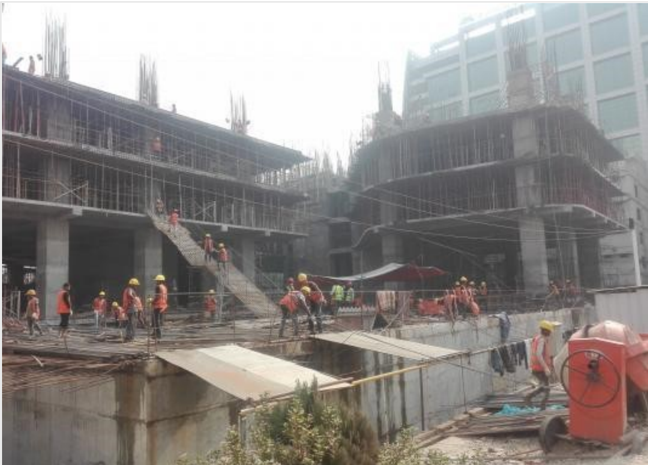
Project View from West Side on 06-02-21
