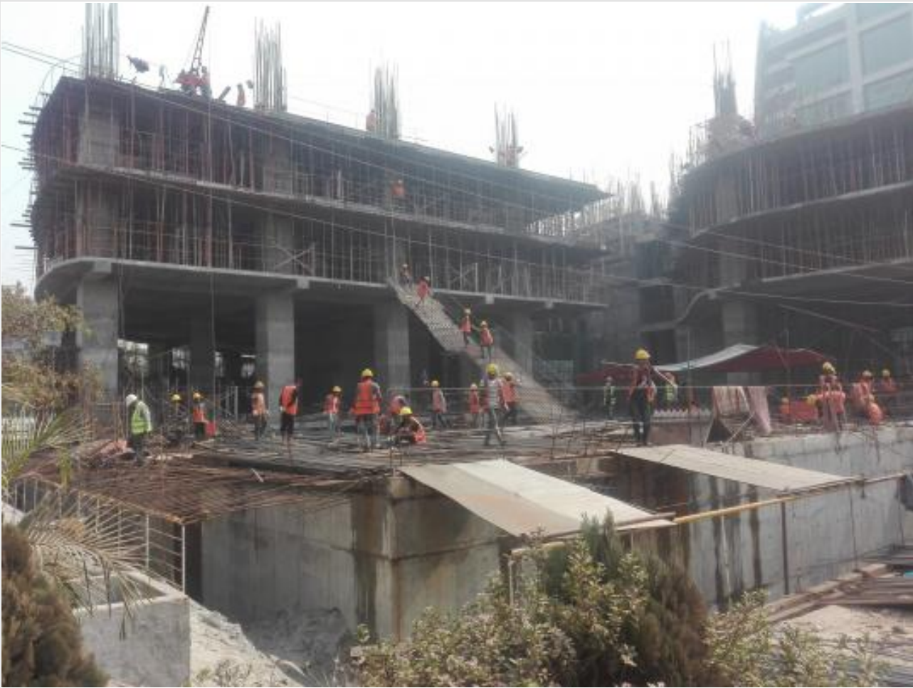
3rd Floor South Tower-Column Complete on 06-01-21
