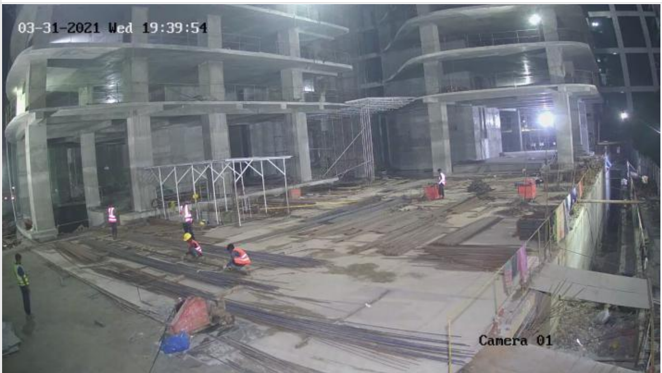
Night Shift Working on 31-03-21
