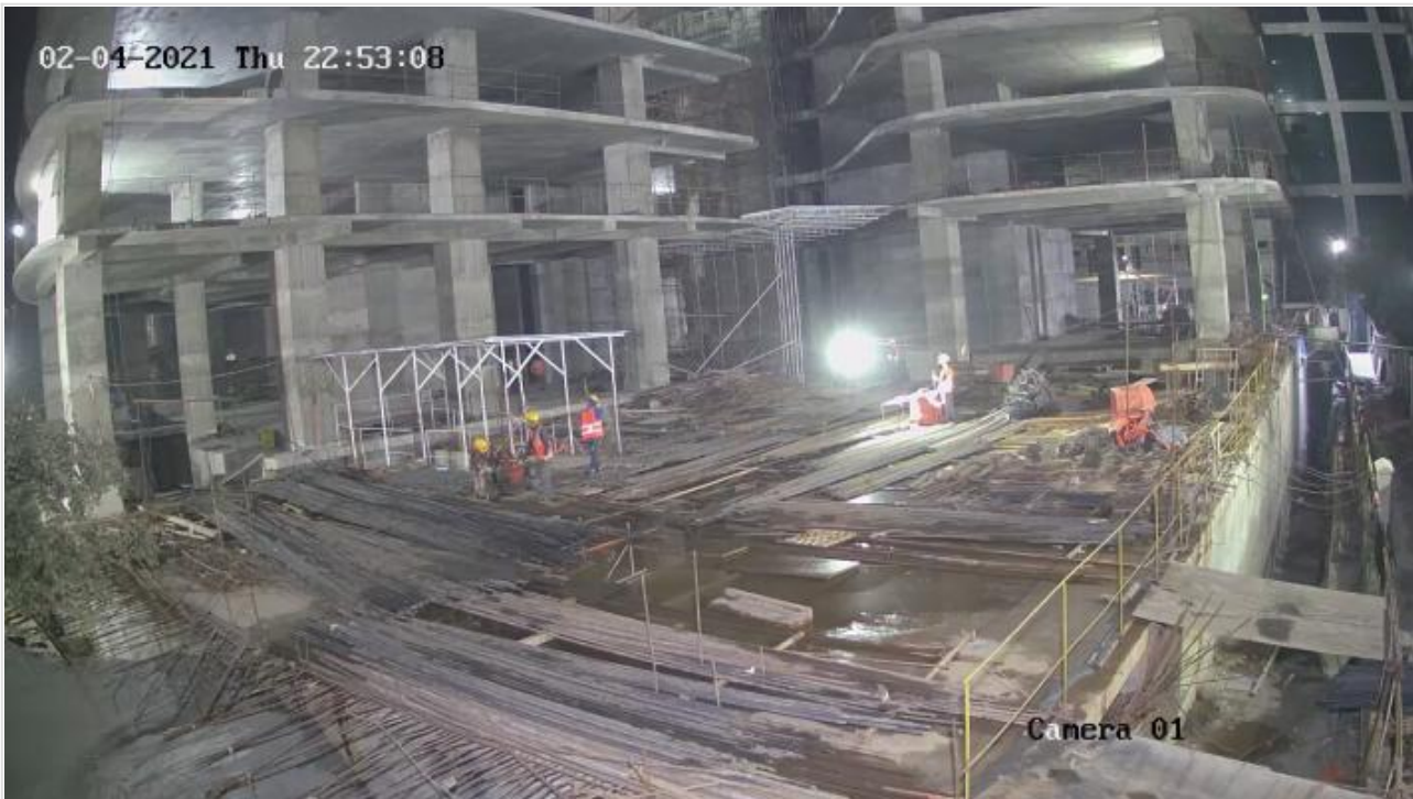
Night Shift Working on 04-02-21
