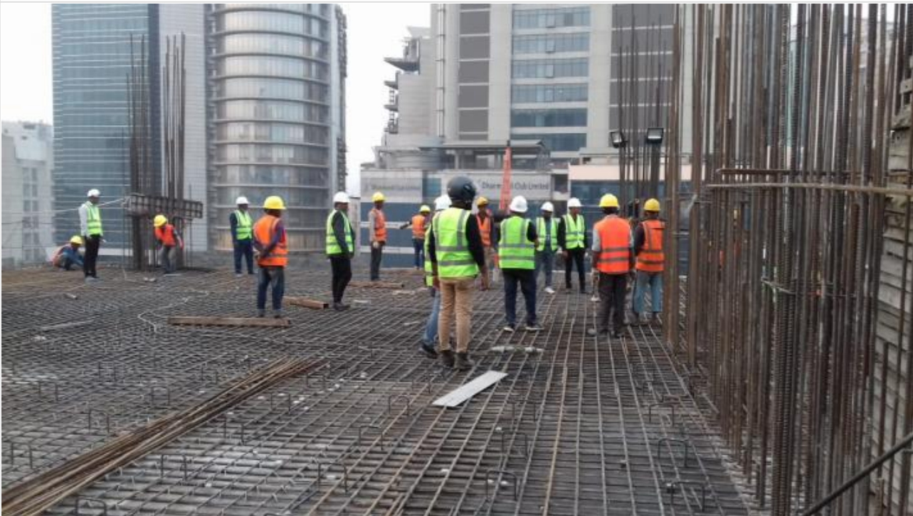
Work Inspection on 30-01-21
