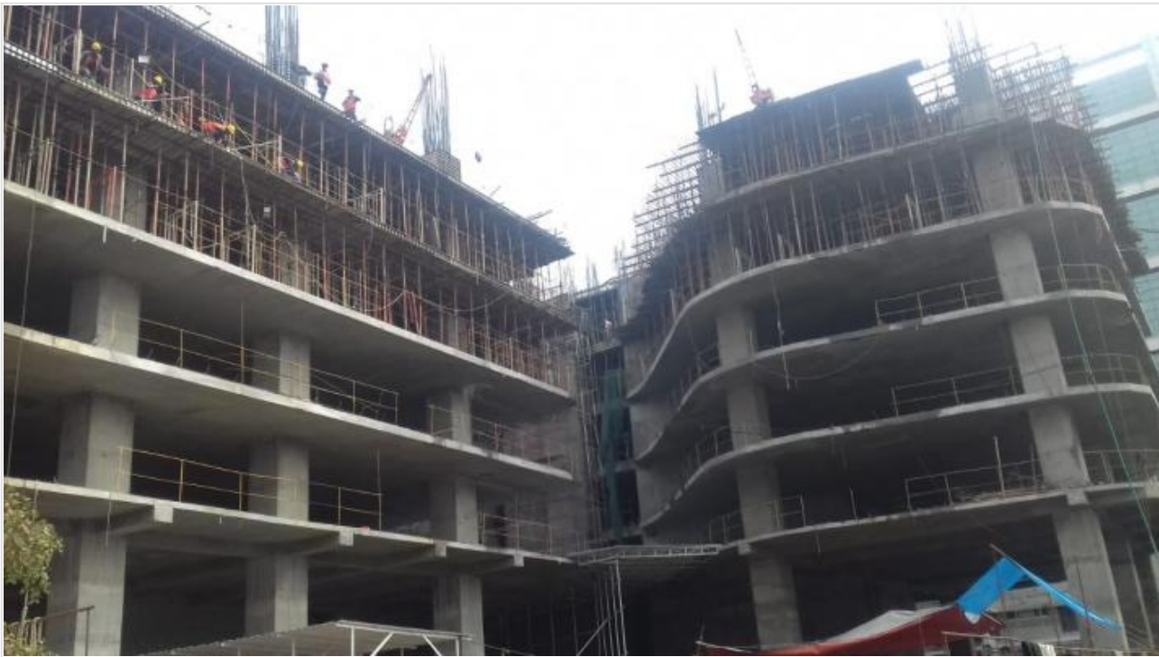
Project Picture on 29-01-21
