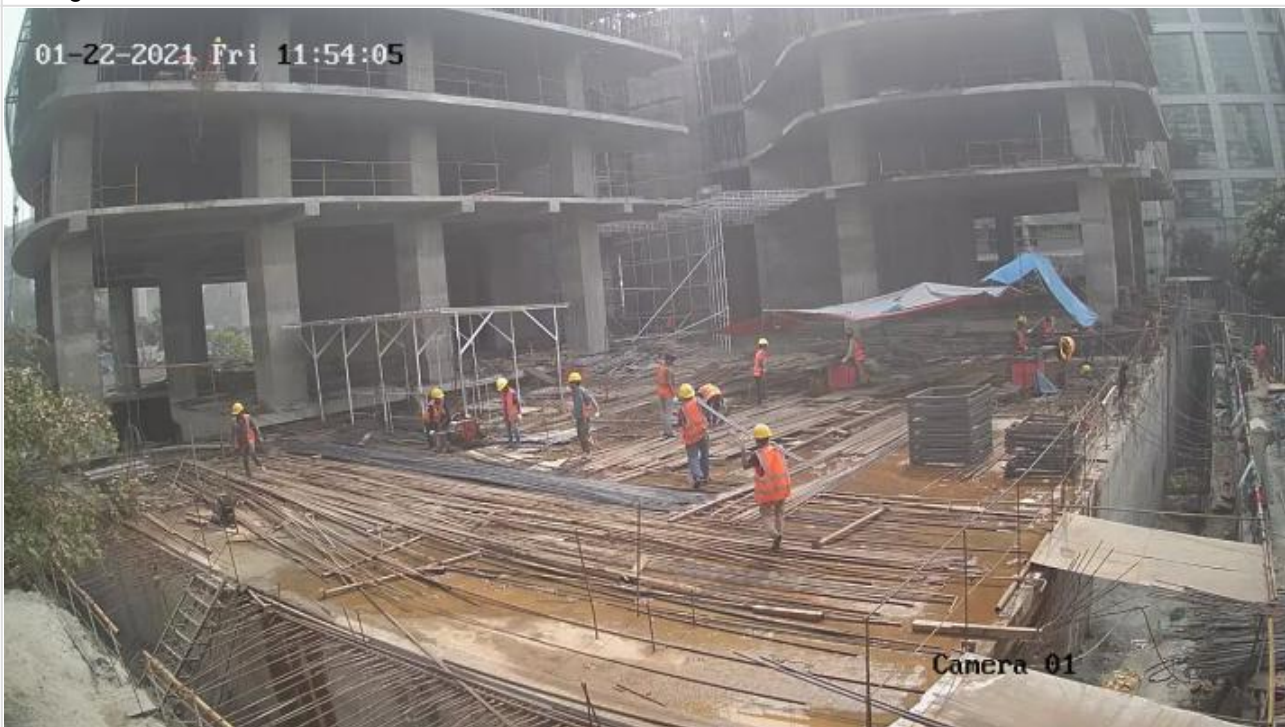
Re-bar Work on 22-01-21
