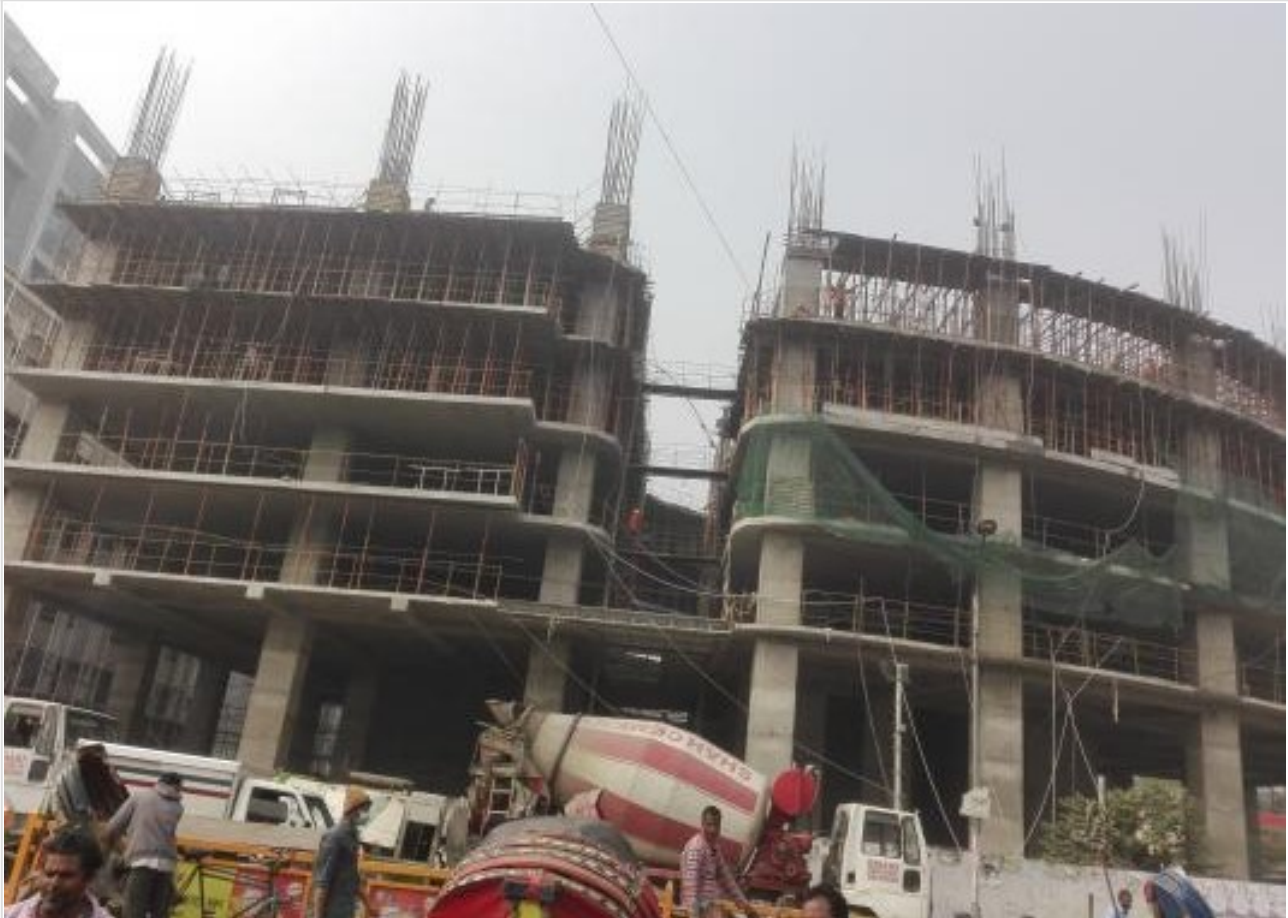
Project Picture on 24-01-21
