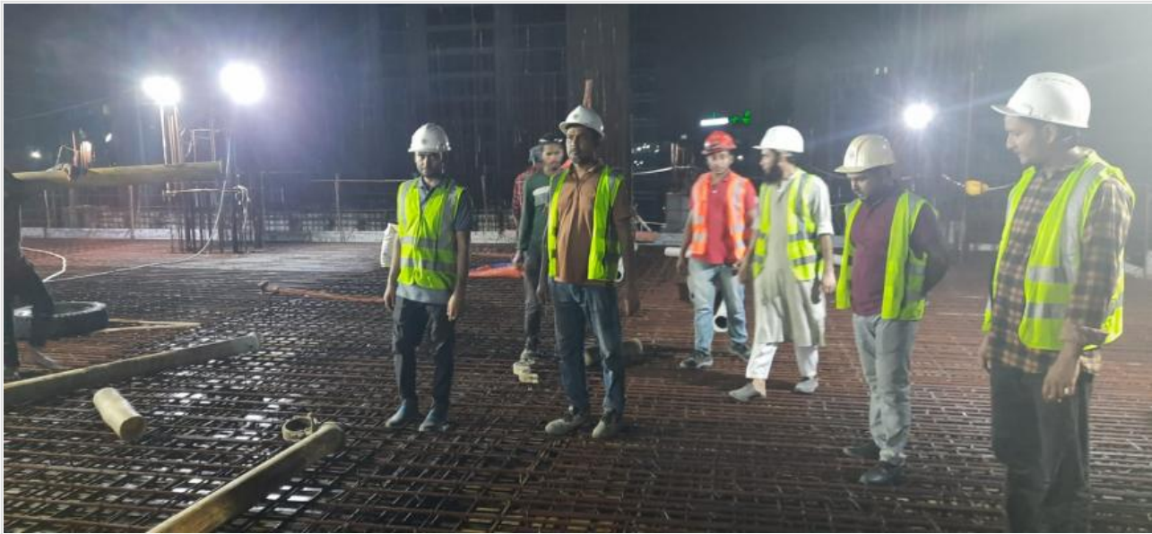
South Tower 11th Floor Slab Concreting on 02-09-21
