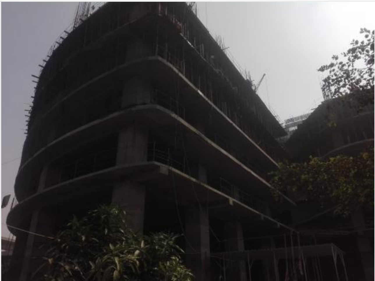
Project Picture on 03-02-21
