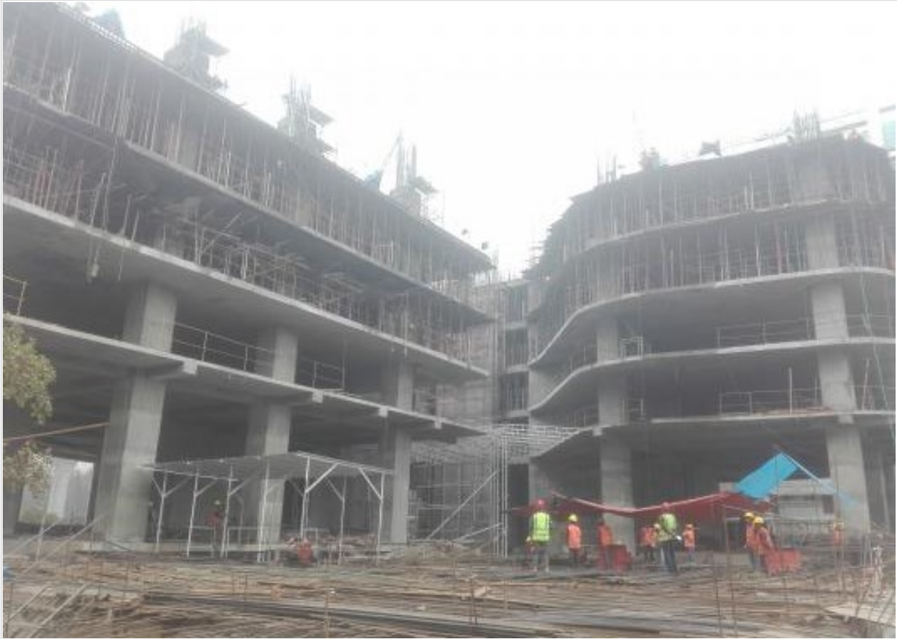
North Tower 4th Floor Lift Core Running on 20-01-21
