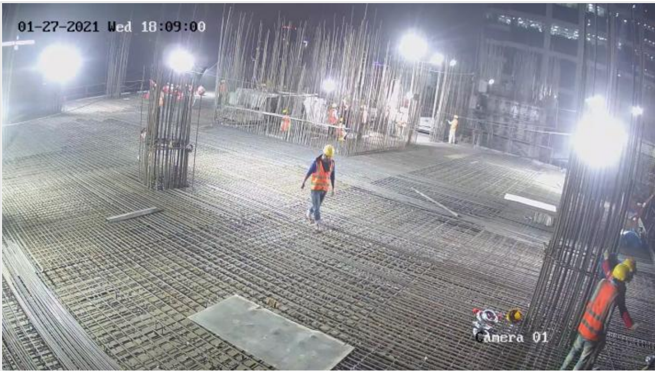
Slab Re-bar Work on 27-01-21
