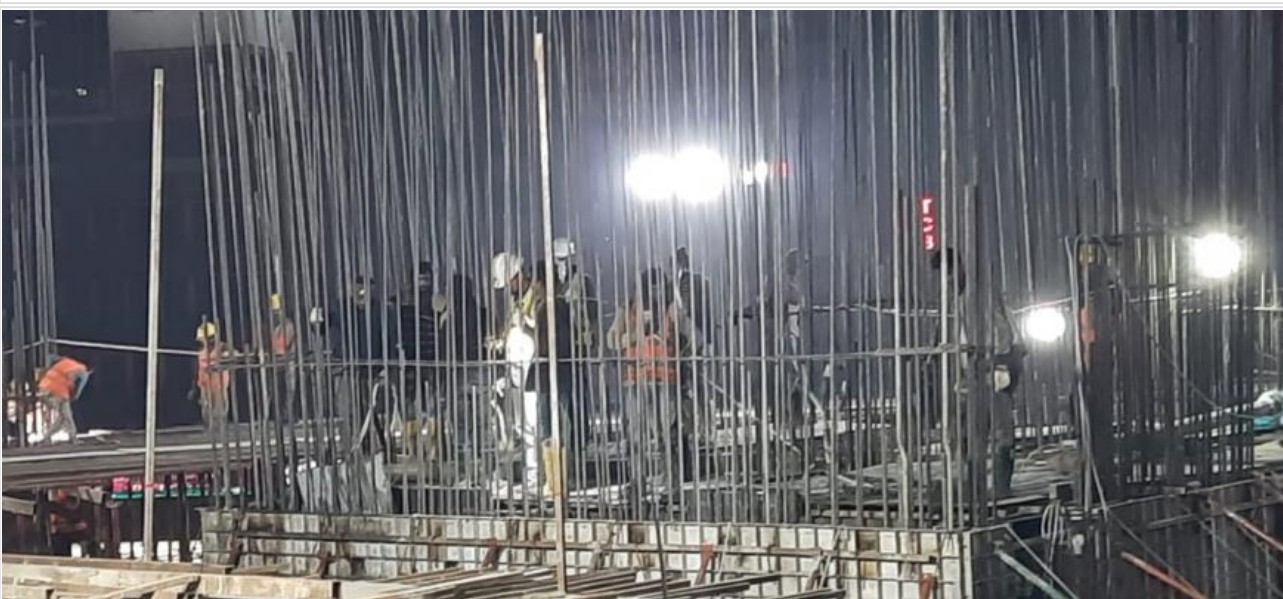
Re-bar Work on 18-01-21
