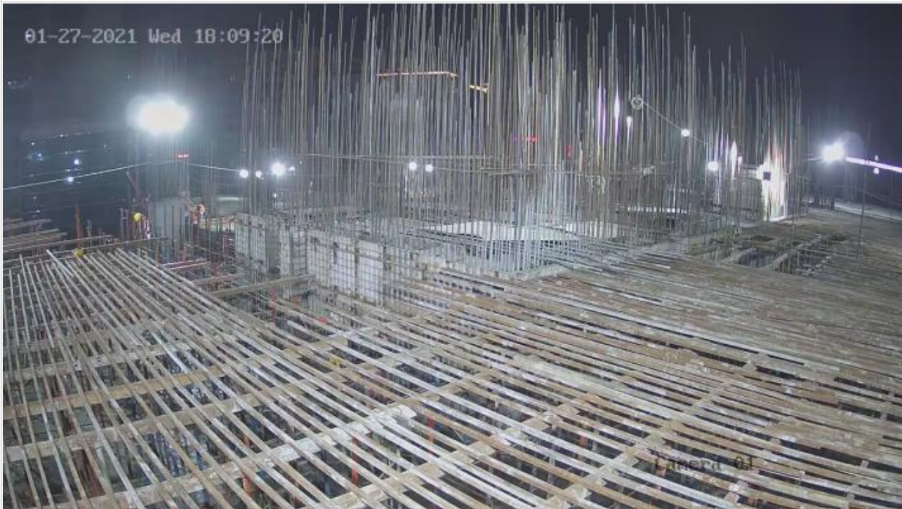
Slab Shuttering on 27-01-21
