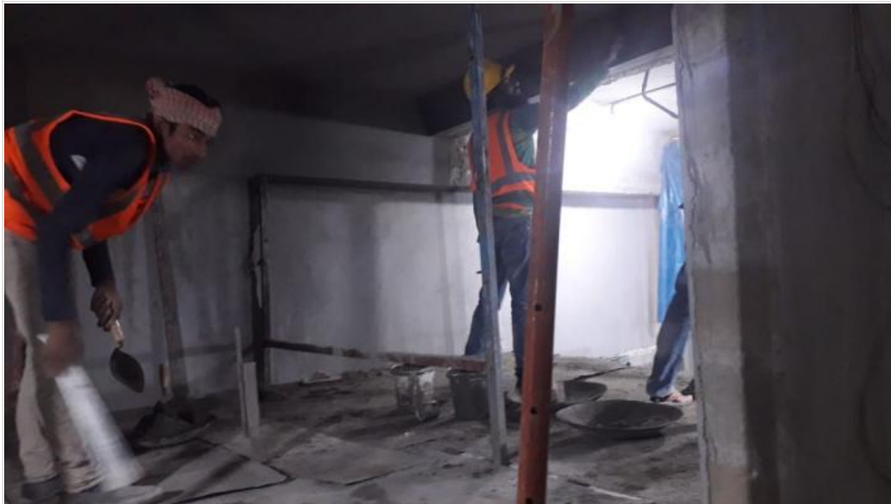
6F-Drive-way Beam Plaster on 23-01-21
