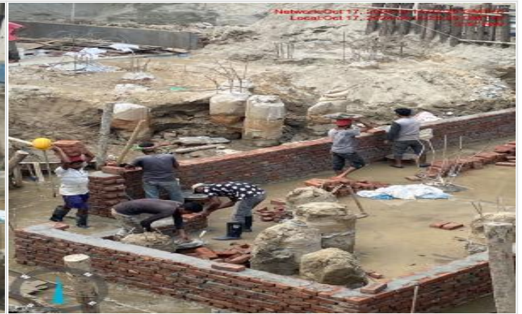
Water tank base brick wall shuttering on 17-10-24
