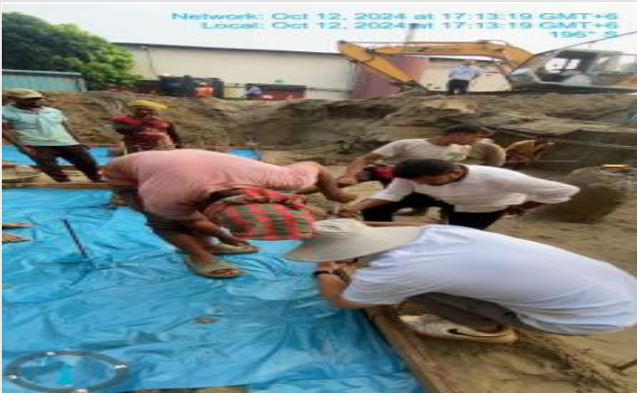
Checking before pile cap lean concreting on 12-10-24
