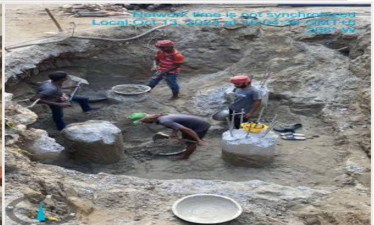
Earth excavation manually on 13-10-24
