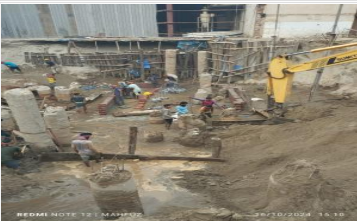
Excavation, brick-shuttering, steel shut on 16-10-24
