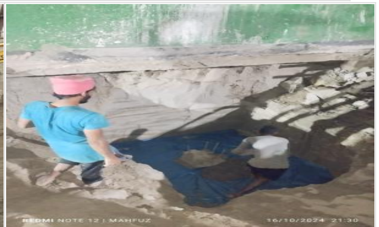
Pile Cap Lean concreting on 16-10-24
