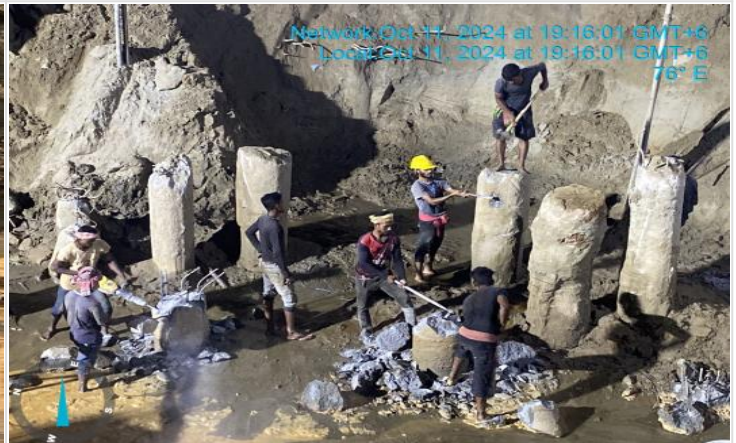
Pile head breaking on 11-10-24
