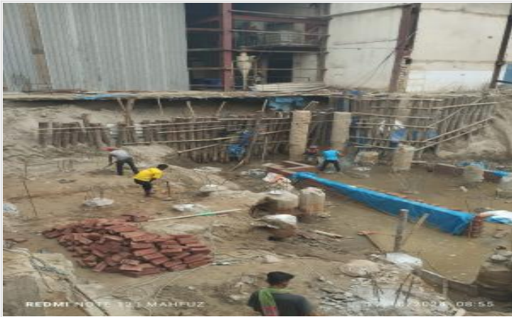
Pile head breaking on 17-10-24
