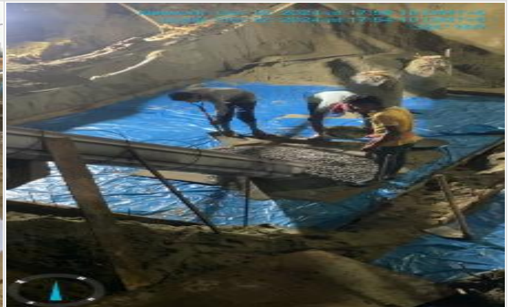
Pile cap lean concreting on 12-10-24
