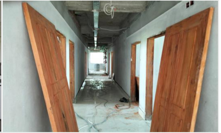
Dormitor-2nd Floor-Corridor on 23-04-24
