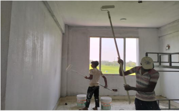
Dormitory-2nd Floor Painting on 23-04-24
