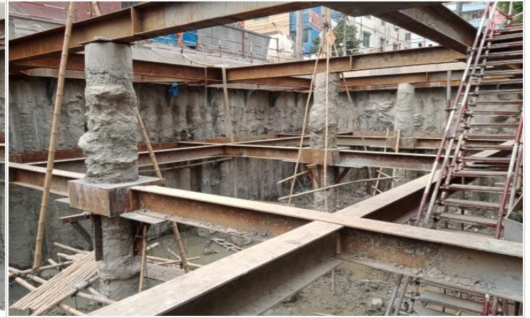
Pile gap water proofing on 30-04-22
