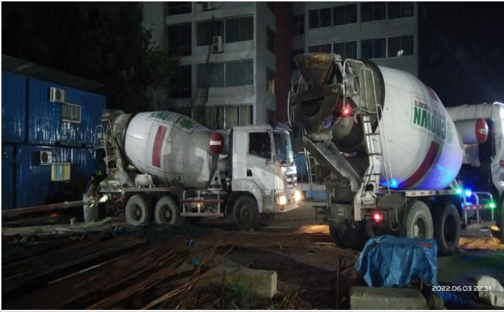
Ready mix car on 03-06-22
