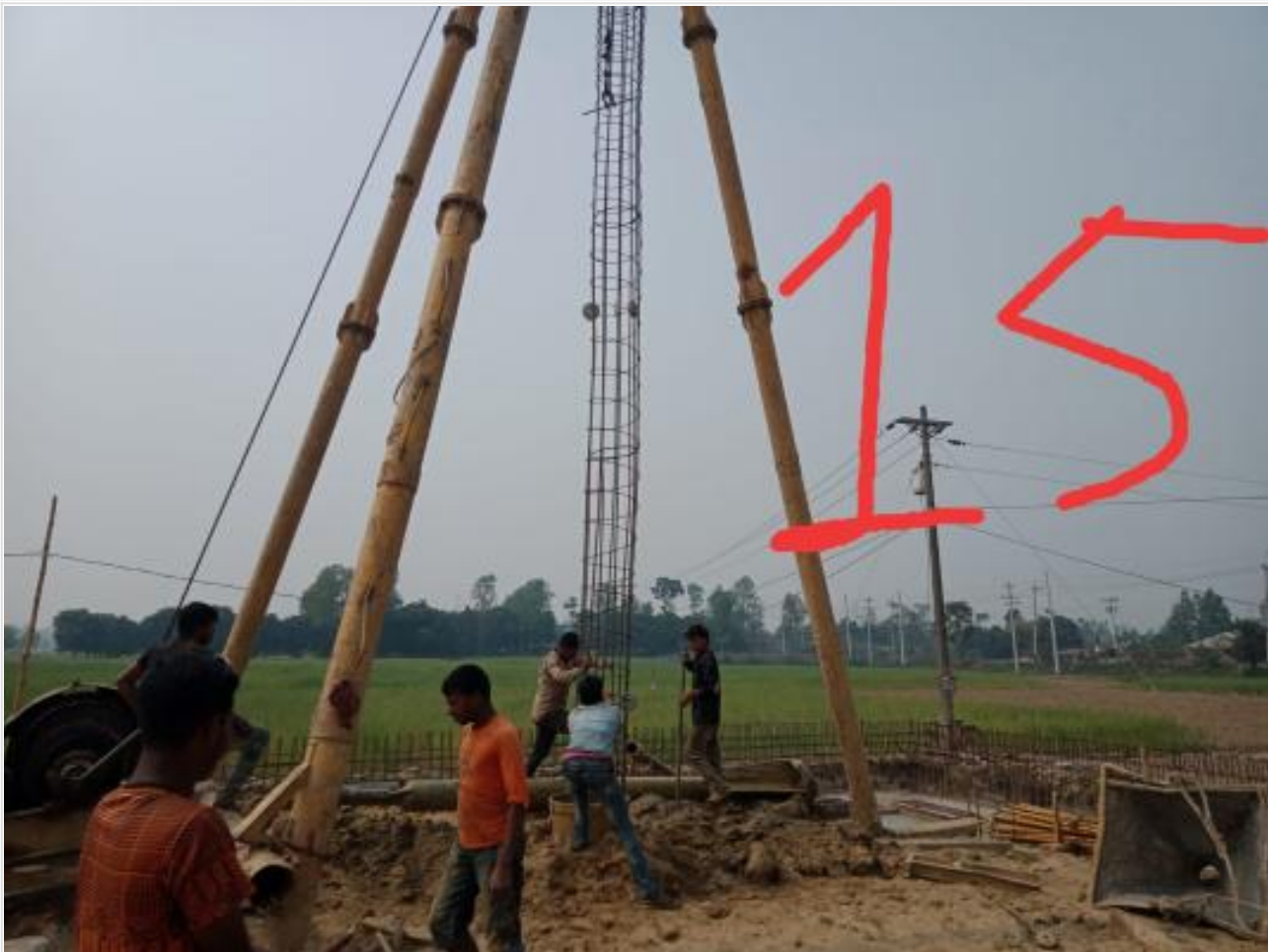
Com. Bldg. 15th pile boring on 19-02-23
