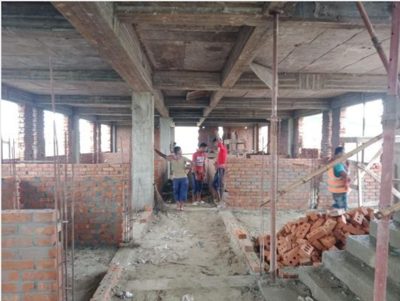
Dorm. Bldg Brick work on 25-09-23
