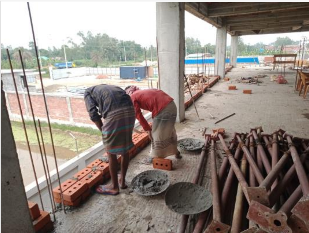
Comp-1st Floor-Brickwork on 22-08-23
