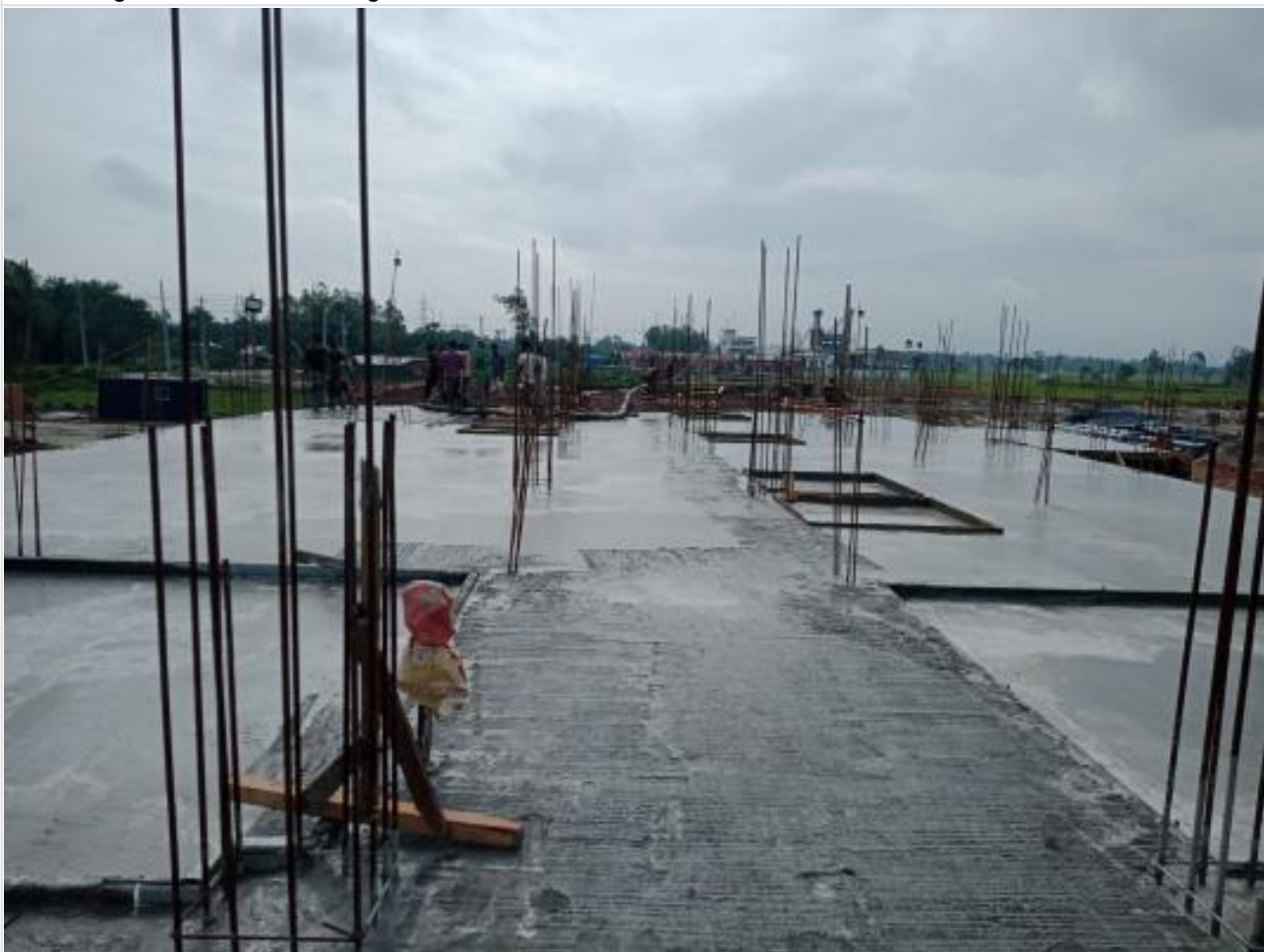
Comp. Bldg. Slab casting complete on 27-06-23
