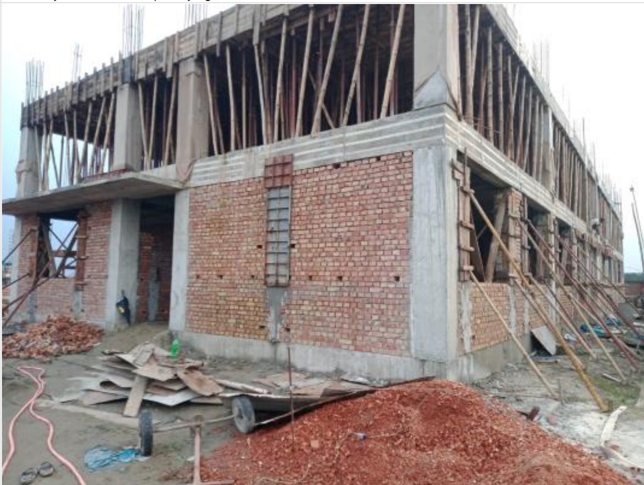
Comp.Bldg.GF Brick work on 09-08-23
