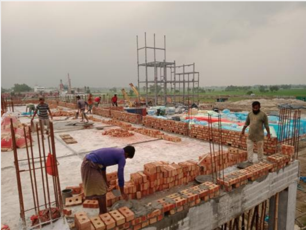
Comp-Parapet Brick-work on 14-08-23
