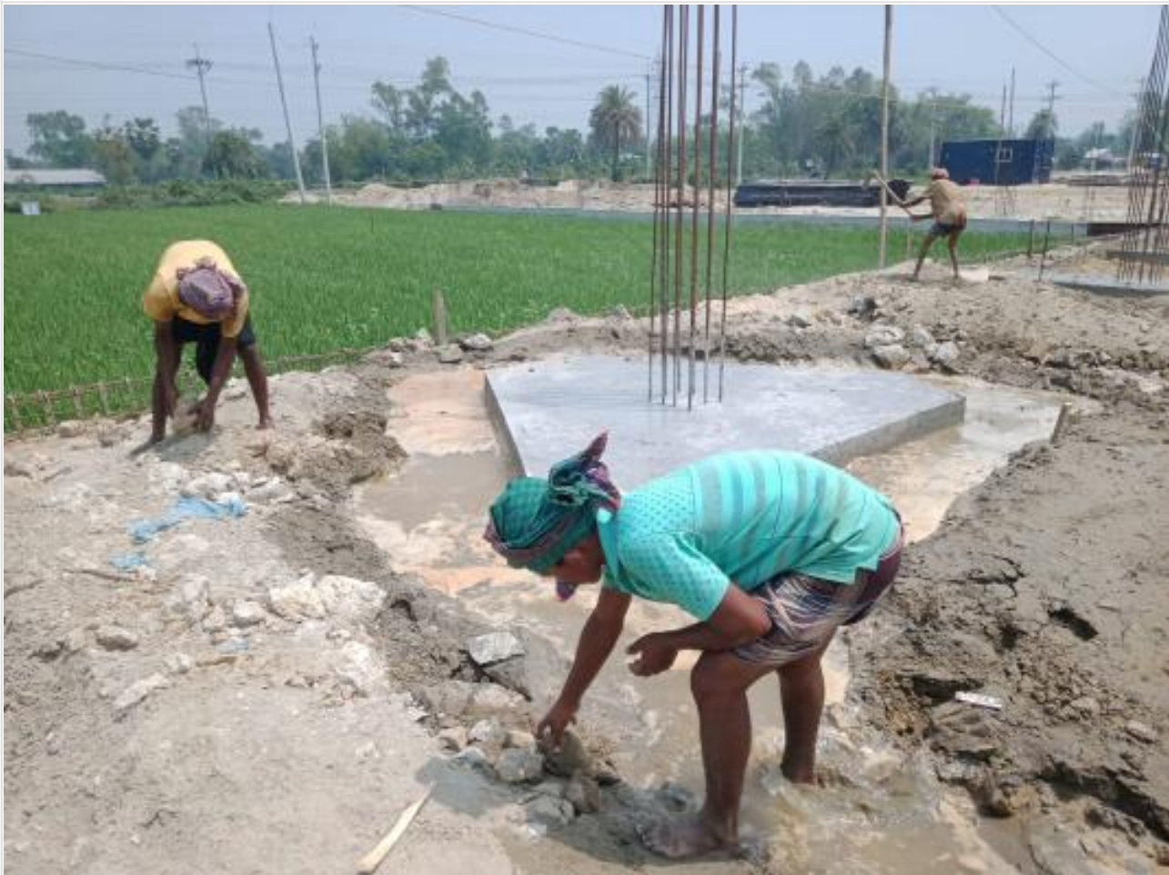
Back filling and levelling dressing. on 19-04-23
