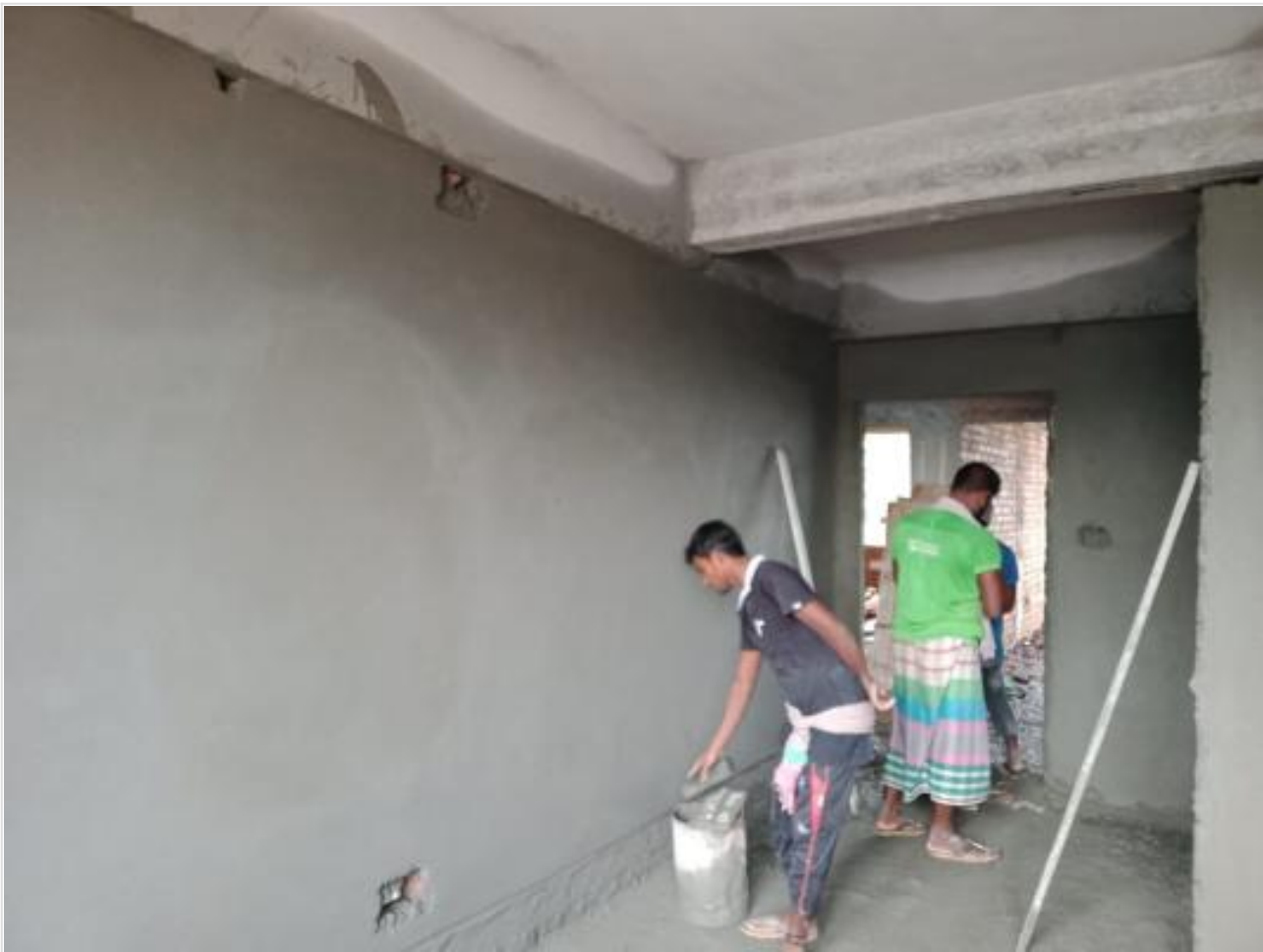
Comp. Bldg 1st fplaster work on 21-09-23
