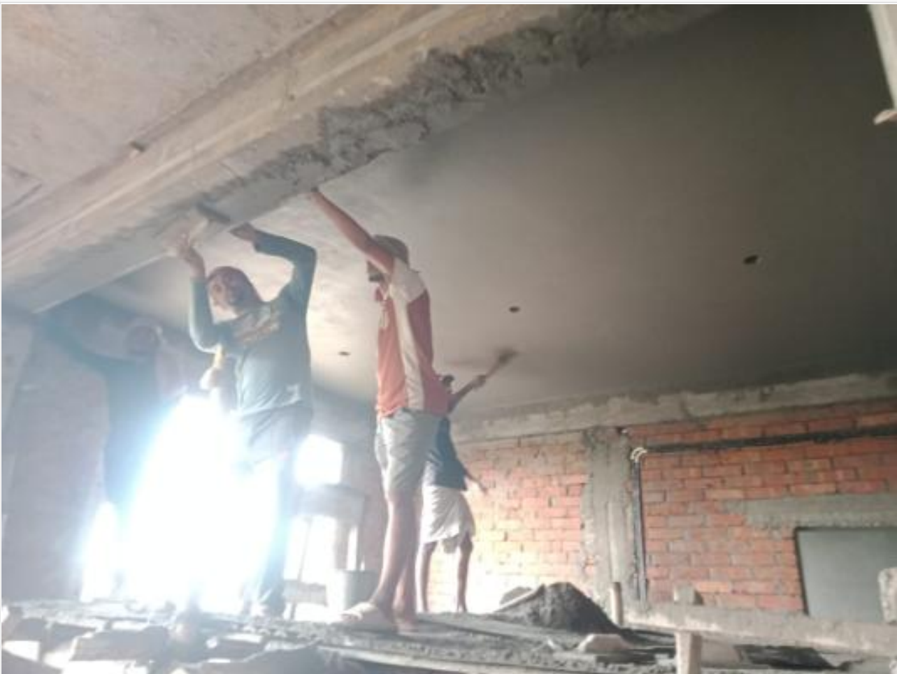
Dormitory-GF-Ceiling Plastering on 27-10-23
