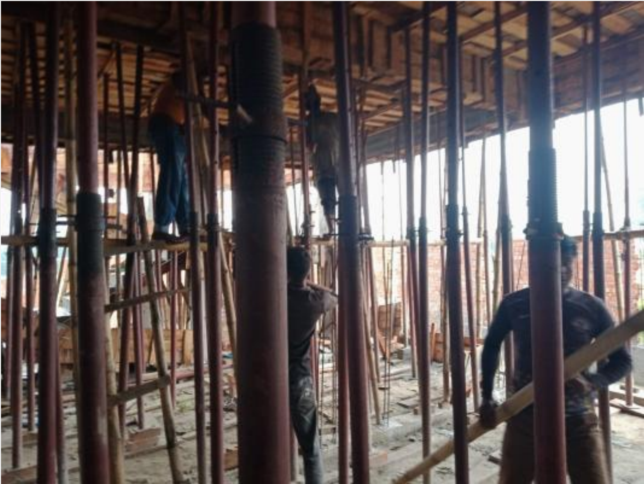
Shuttering work on 09-07-23
