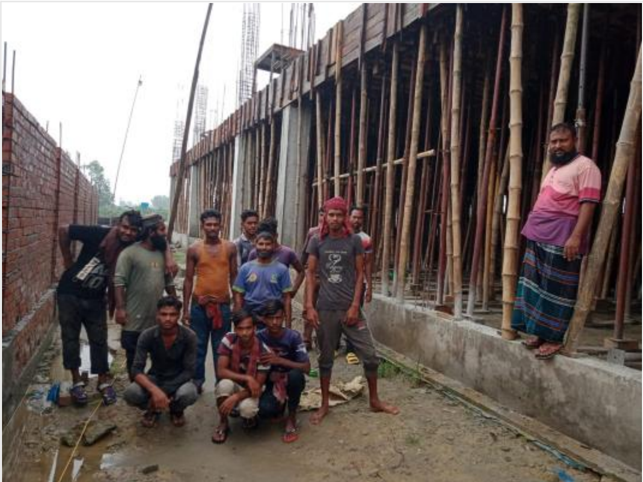
Civil worker on 09-07-23
