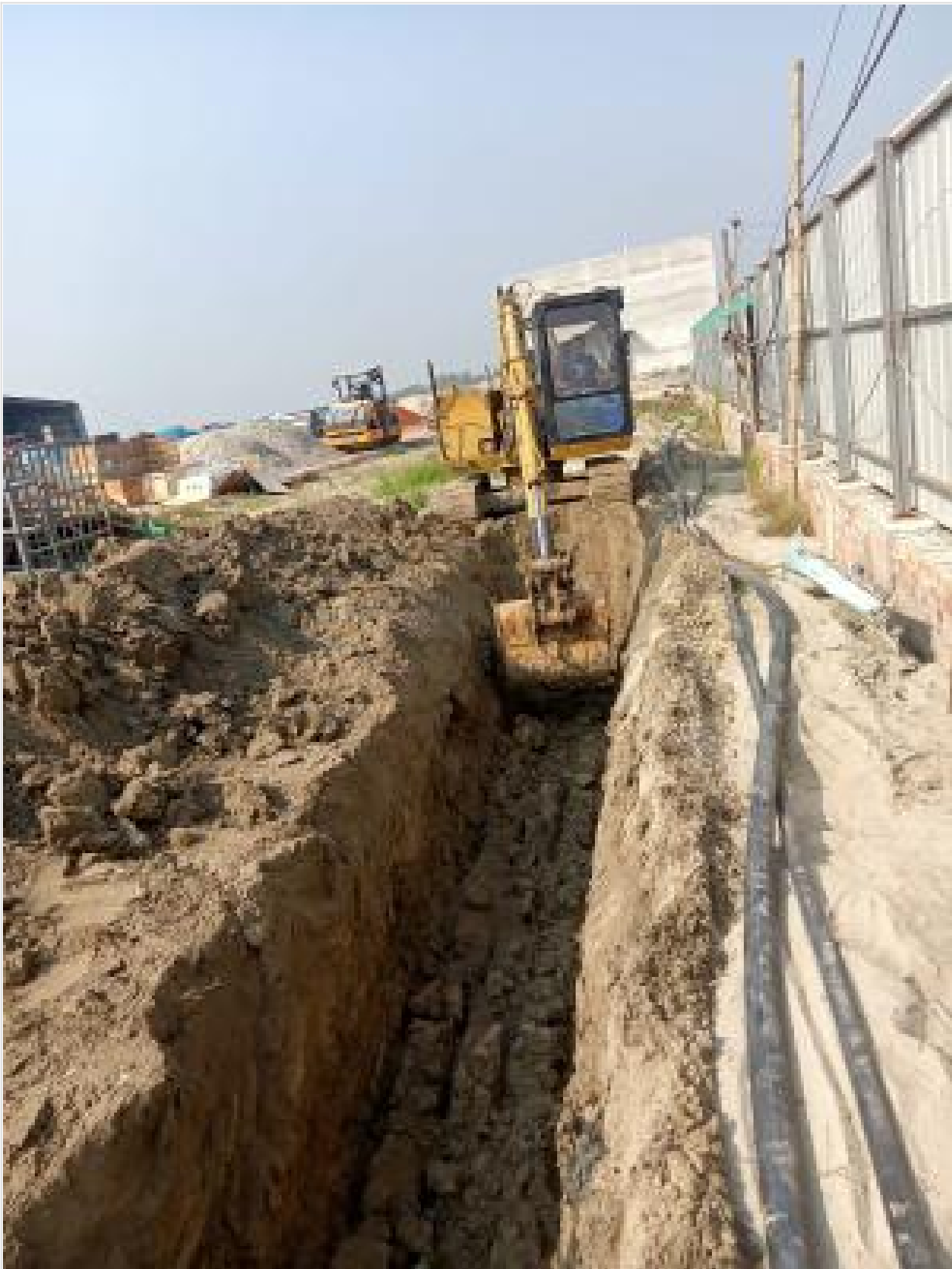
Power cable laying work on 03-11-23
