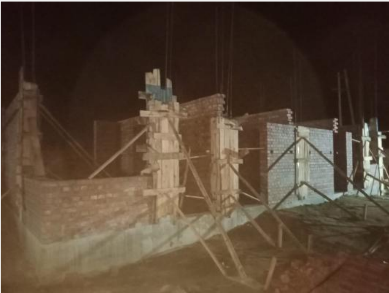
Gate House column casting on 18-06-23
