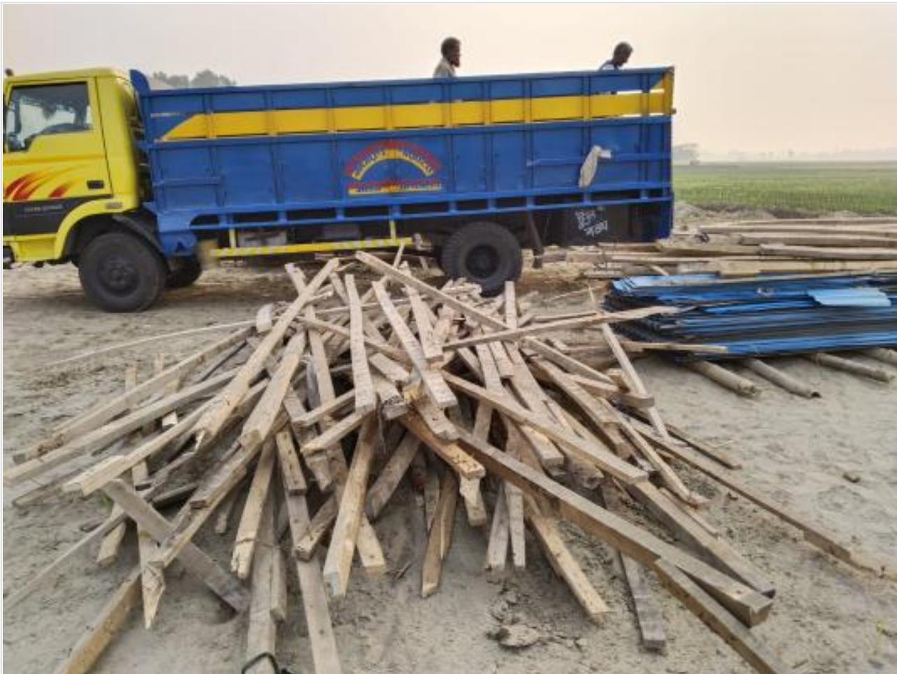
Materials for Shed on 14-01-23
