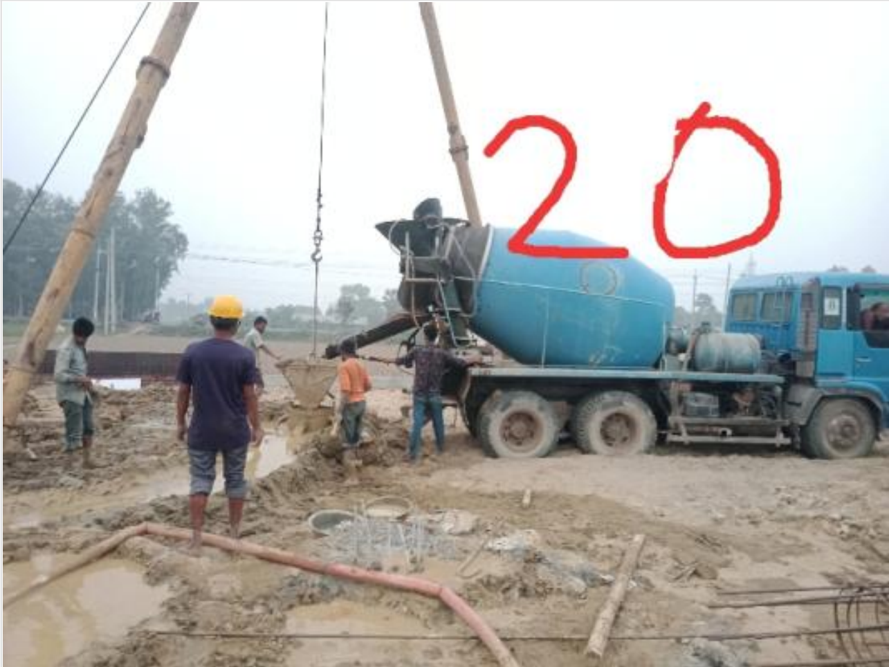
Ready mix concreting of pilewort on 22-02-23
