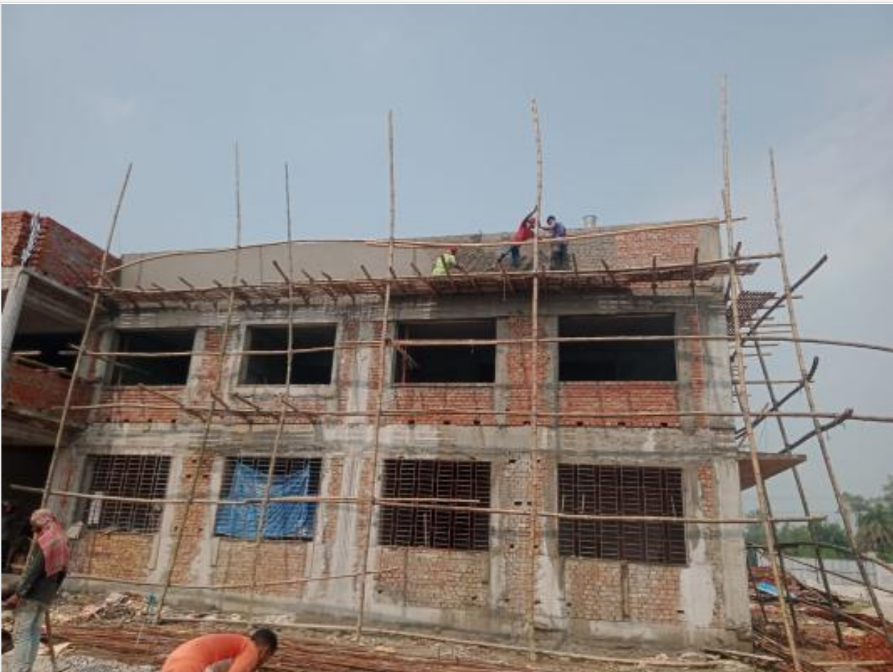
Comp. Bldg. Outside plaster work on 09-10-23
