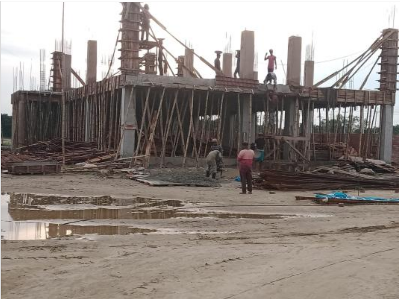
Comp. Bldg. 1st floor column work on 13-07-23
