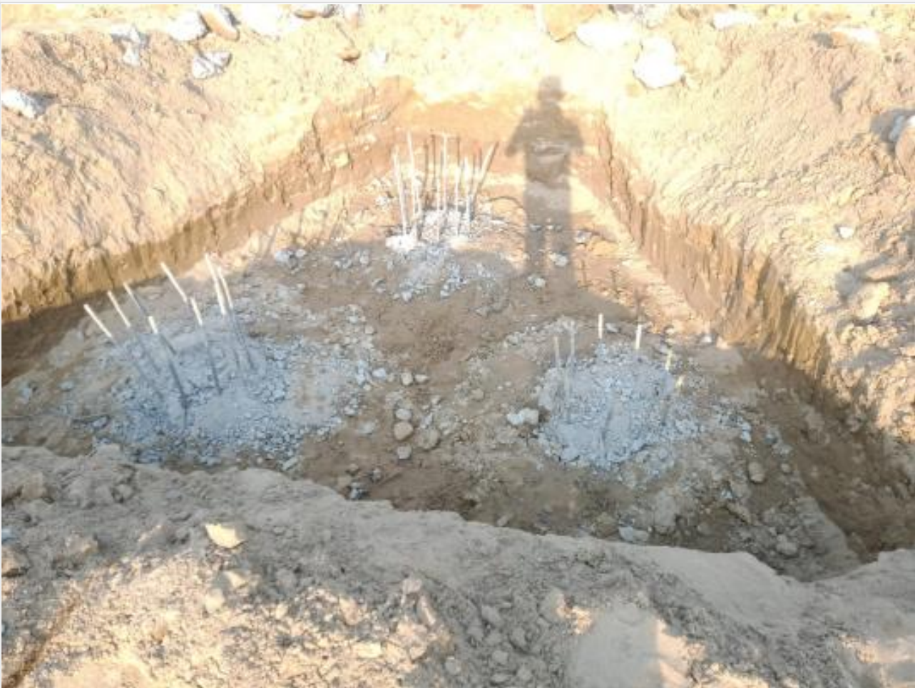
Dorm. Bldg. Pile head breaking on 07-05-23
