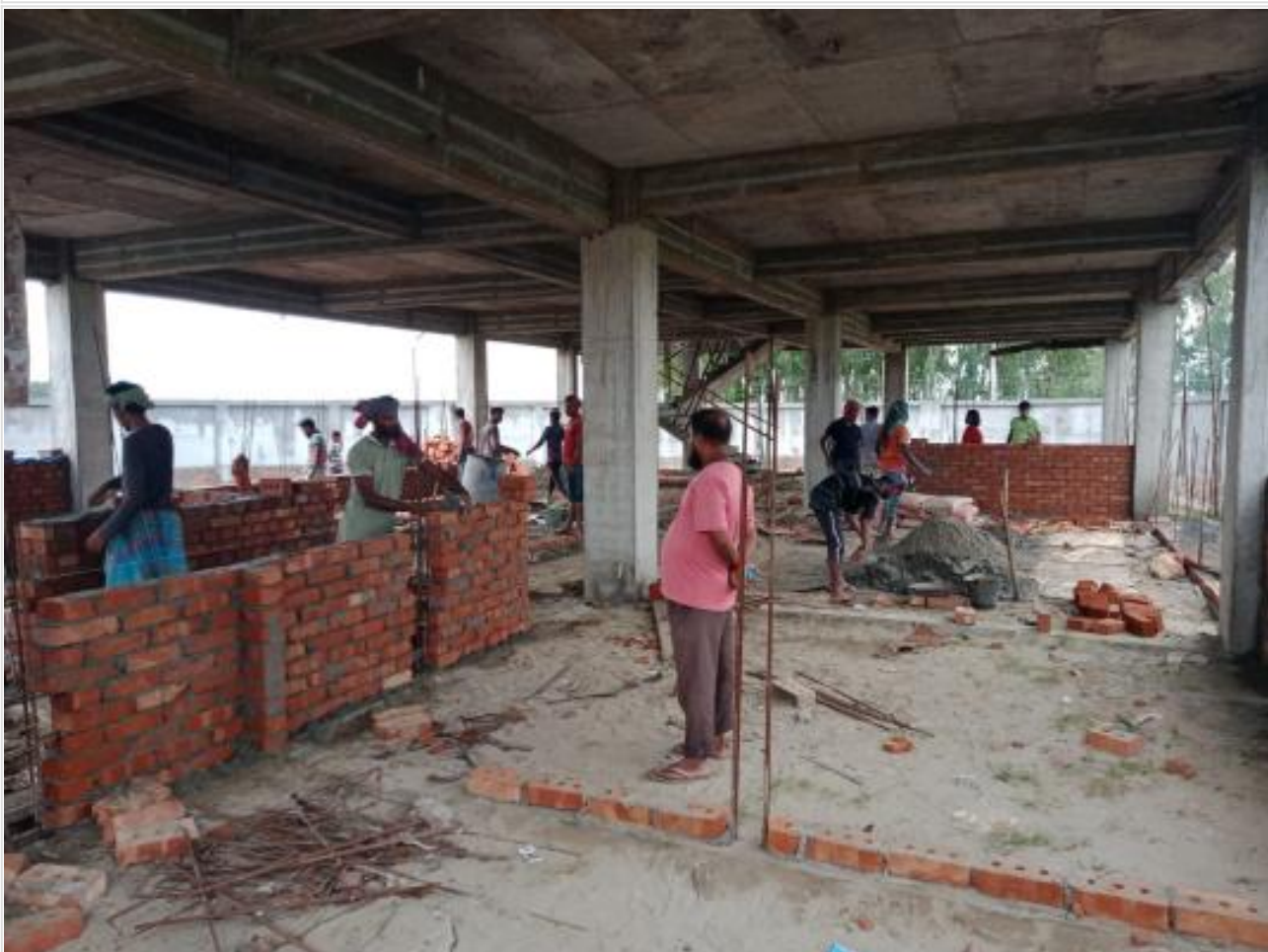
Dorm. Bldg GF Brick work on 22-09-23
