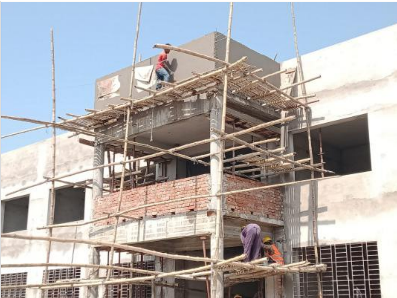
Comp. Building-Outside Plastering on 20-10-23
