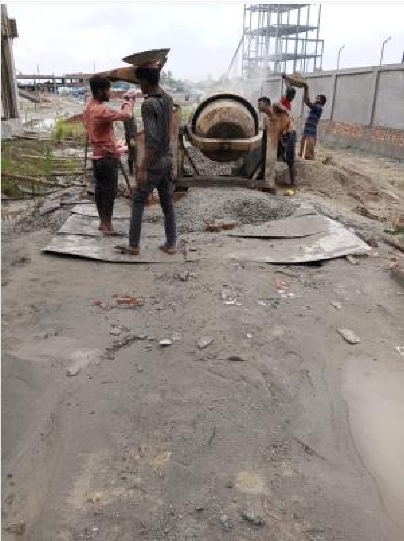
Dormitory column casting on 25-08-23
