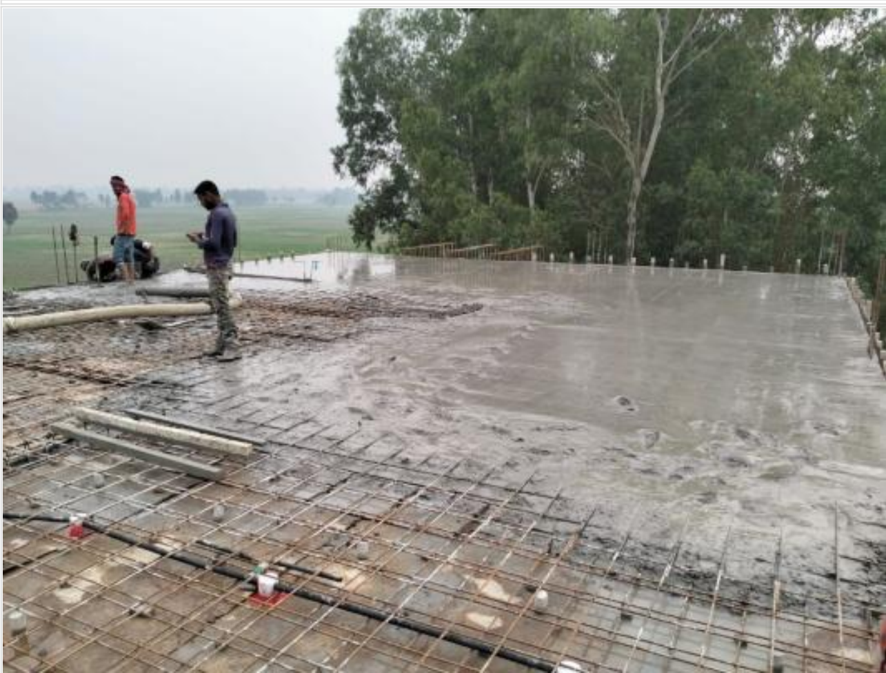
Dormitory-3rd Floor Slab Concreting on 23-12-23
