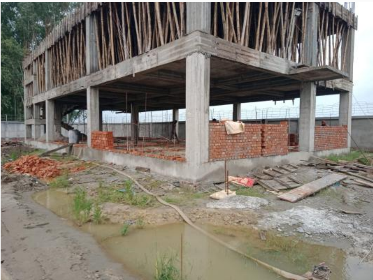
Dorm. Bldg GF Brick work on 21-09-23
