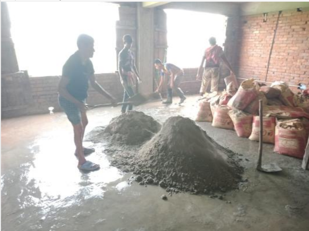
Comp. Bldg. GF casting on 29-09-23
