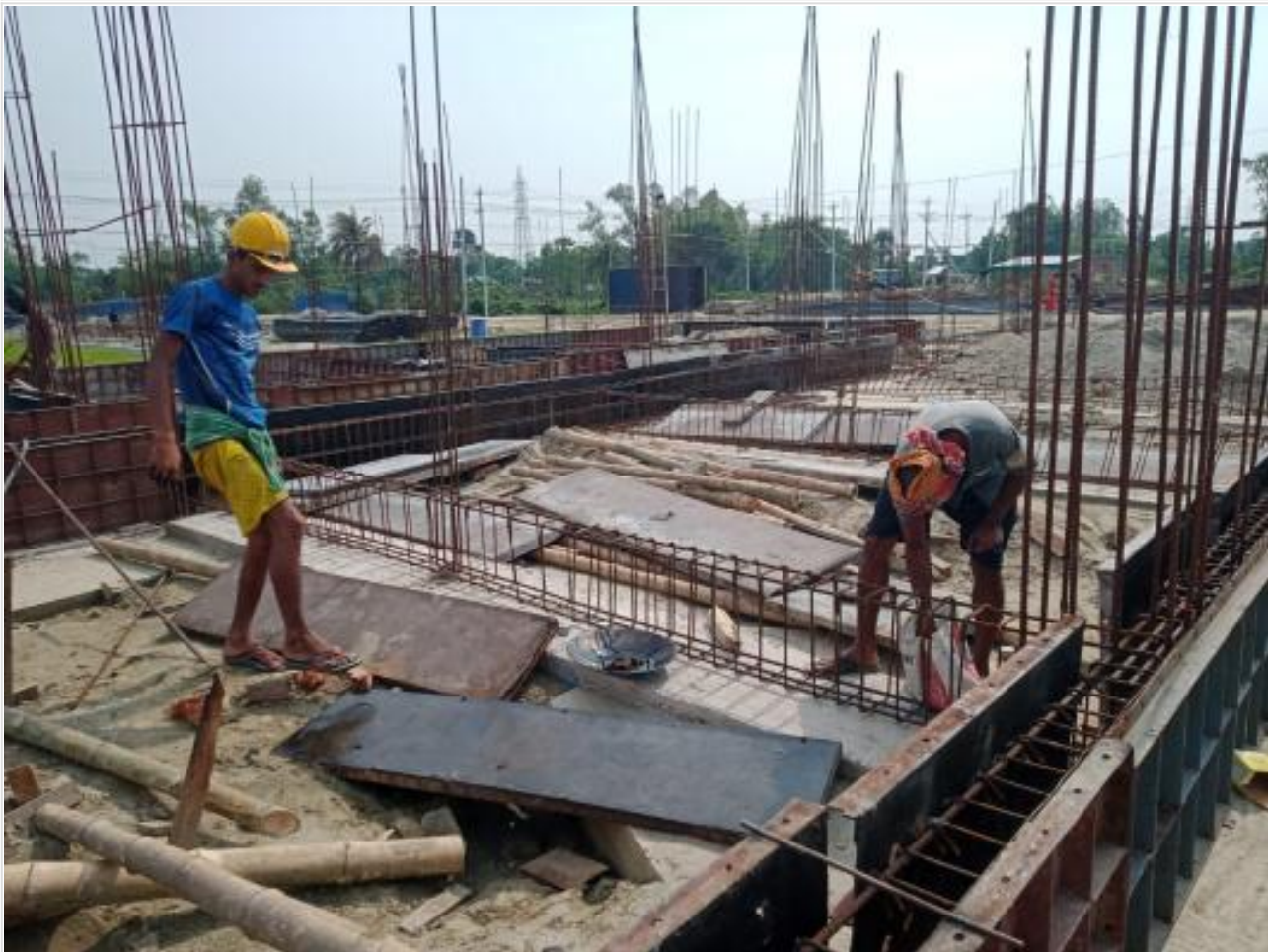
Comp. Bldg. GB Shuttering work on 14-05-23
