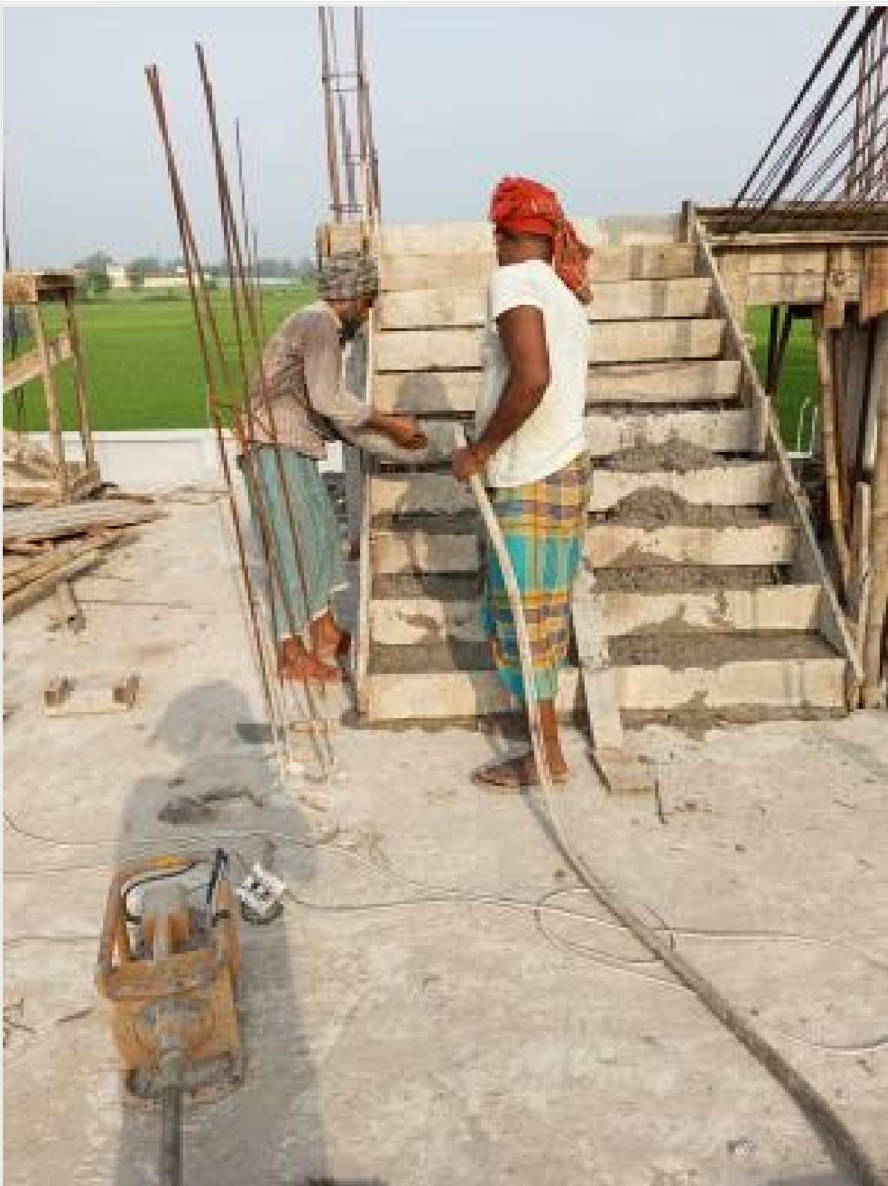
Dorm. Bldg. 1st flight stair casting on 30-08-23
