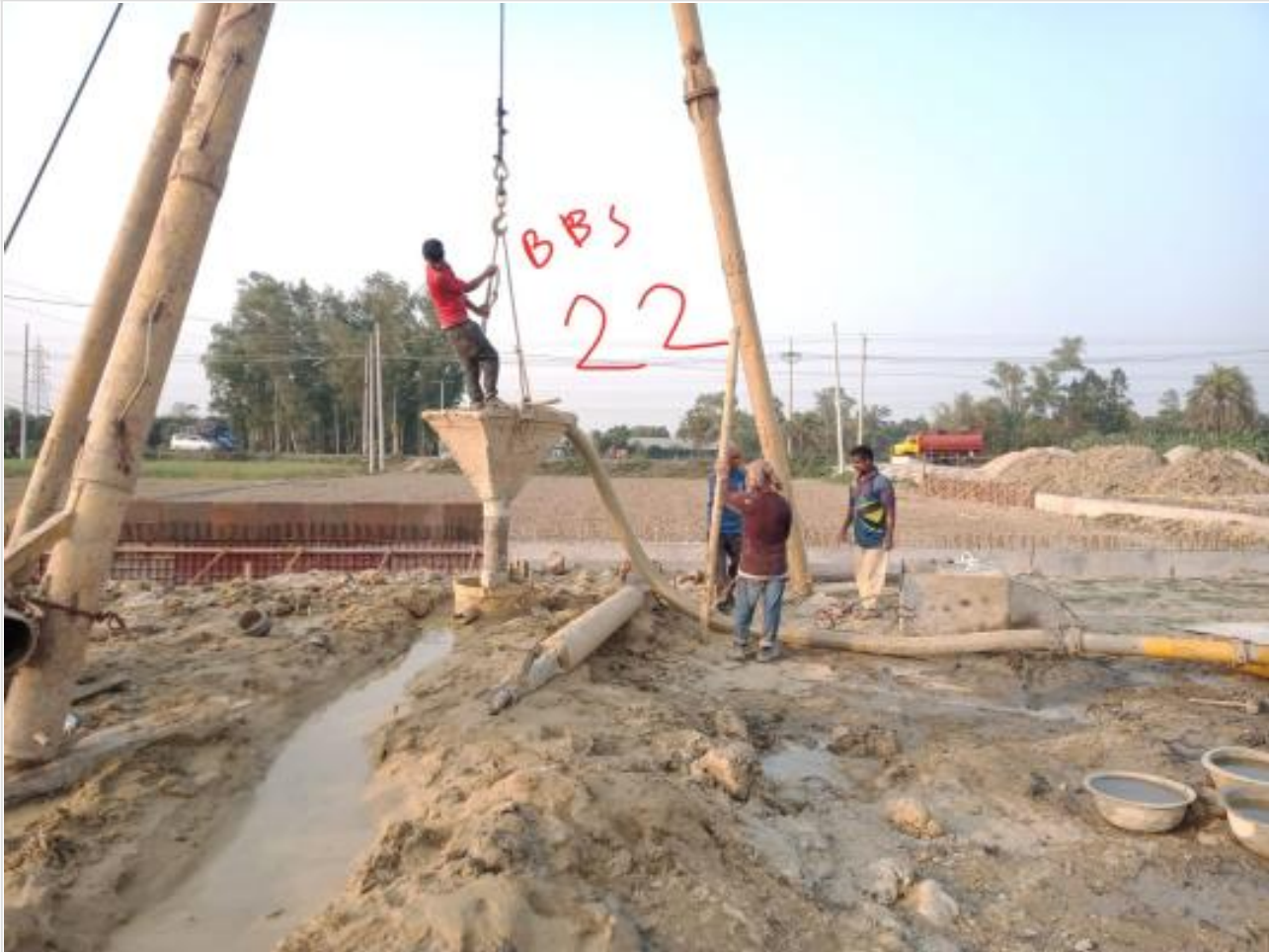
Ready mix concreting of pile on 23-02-23
