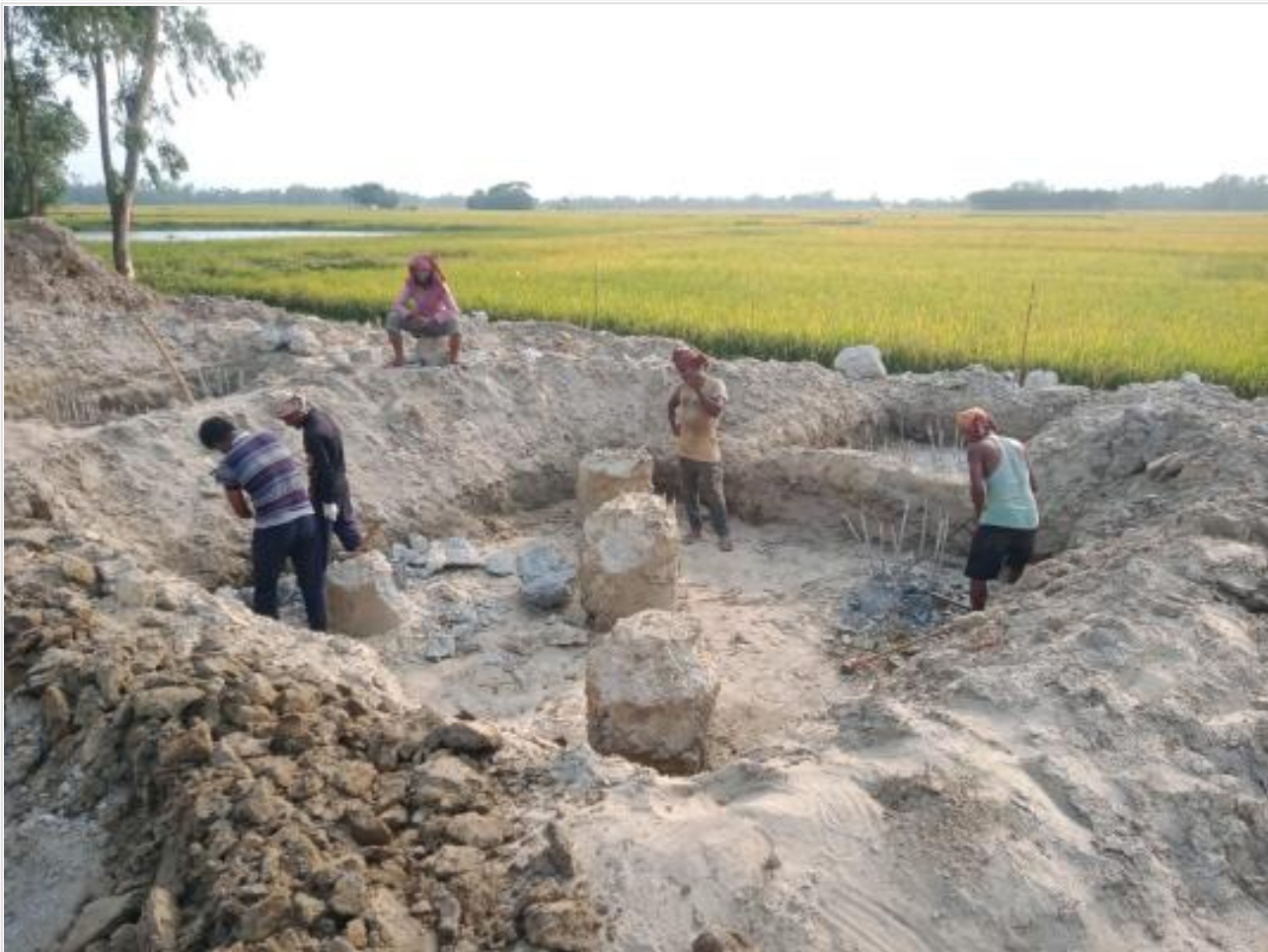
Dorm Bldg pile head breaking on 15-05-23
