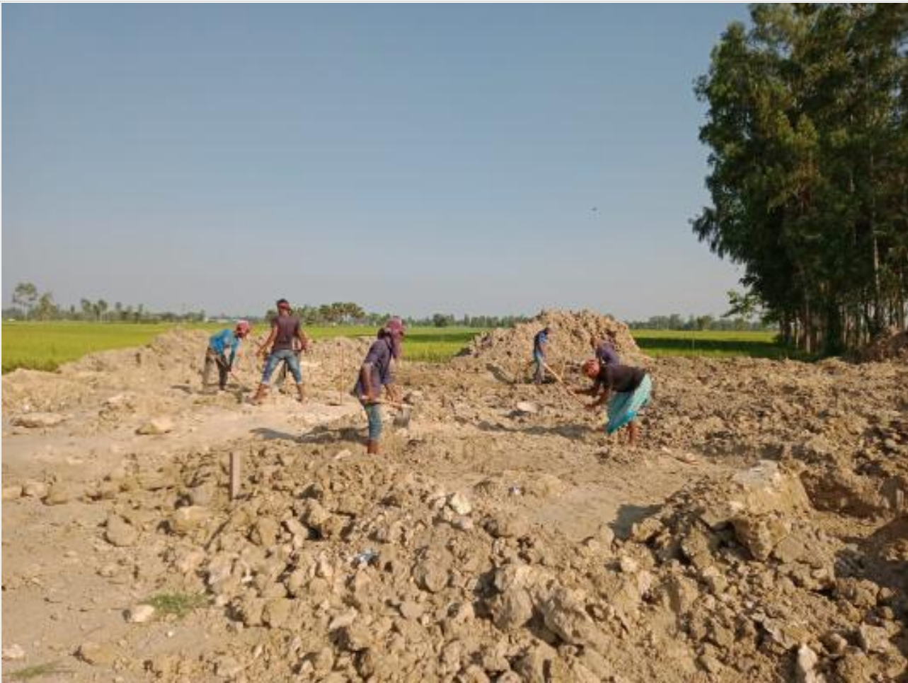
Earth cutting for dorm. Bldg. on 06-05-23
