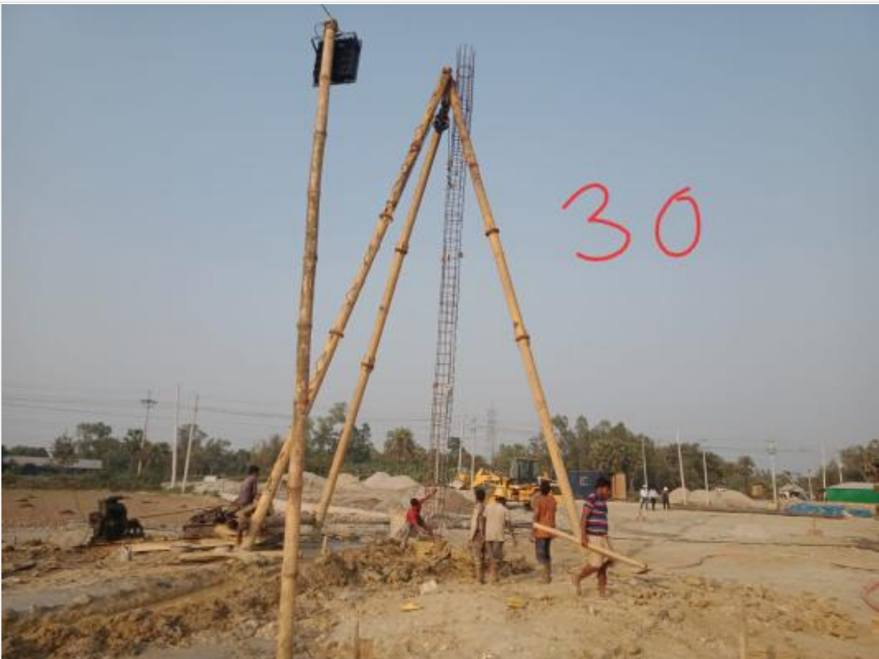
Com. Bldg. 30th pile boring on 26-02-23
