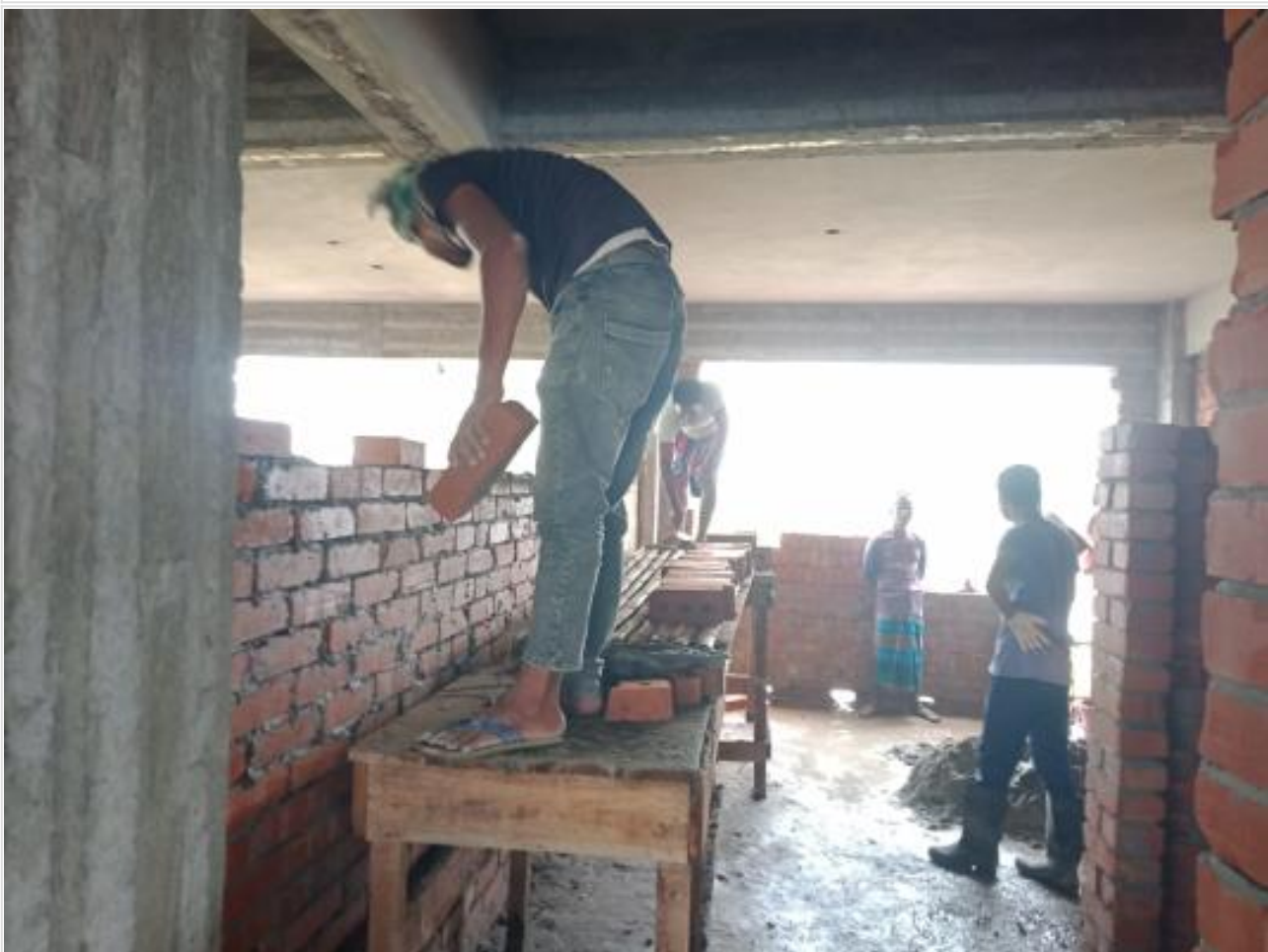
Comp. Bldg. 1st floor brick wall on 04-09-23
