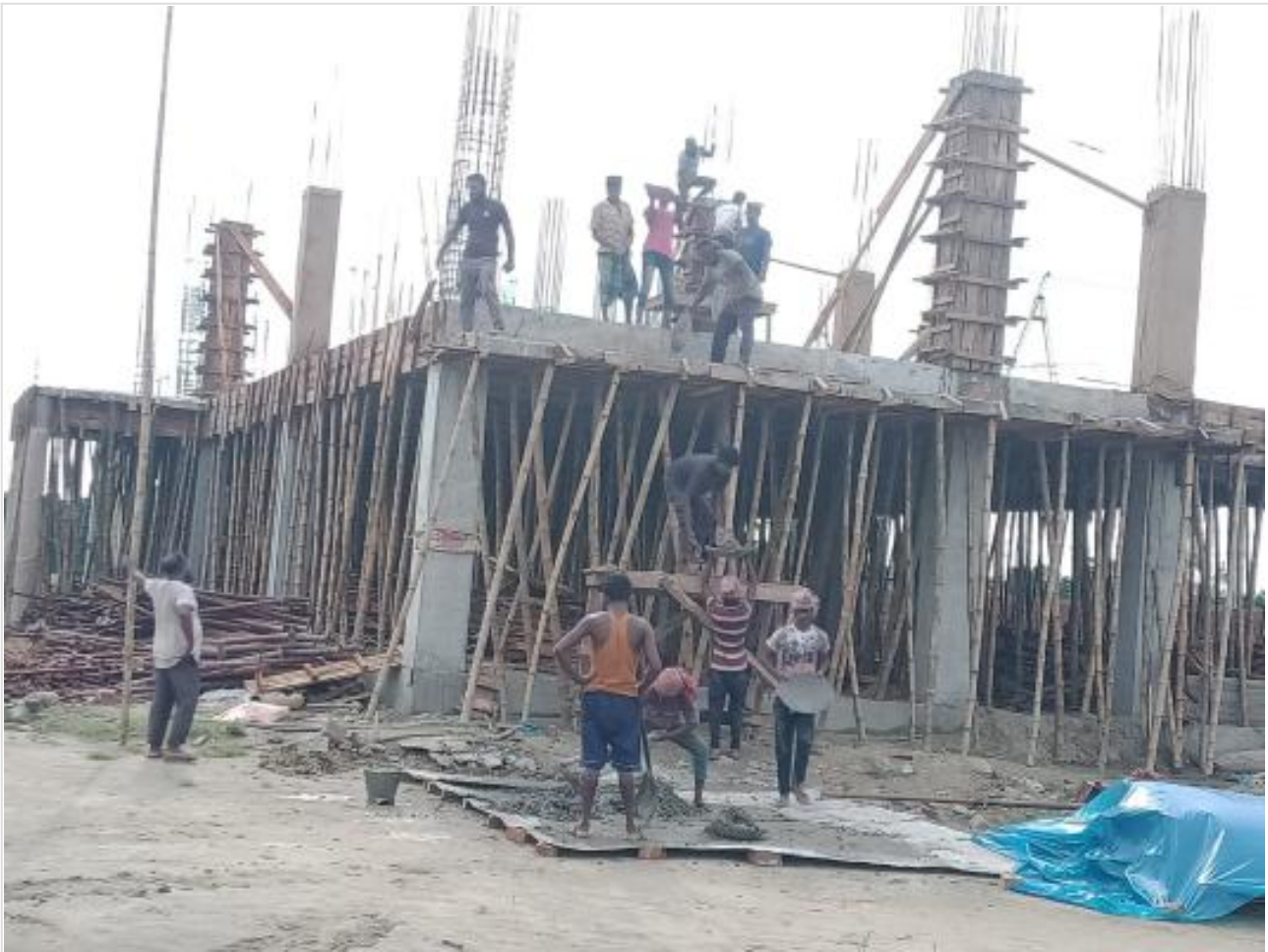
Comp. Bldg. 1st floor column casting on 12-07-23
