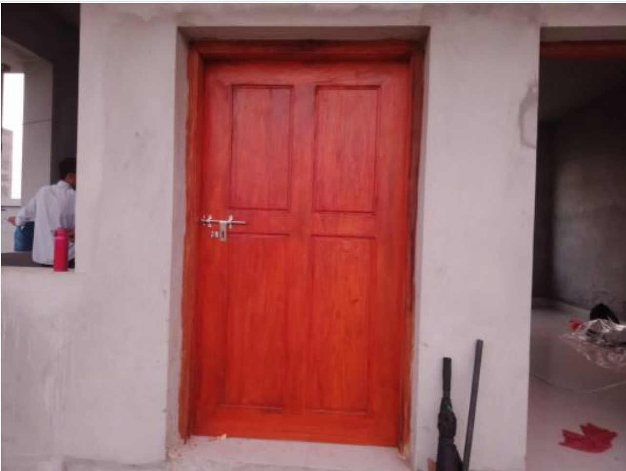
Gate House door fixed on 31-10-23
