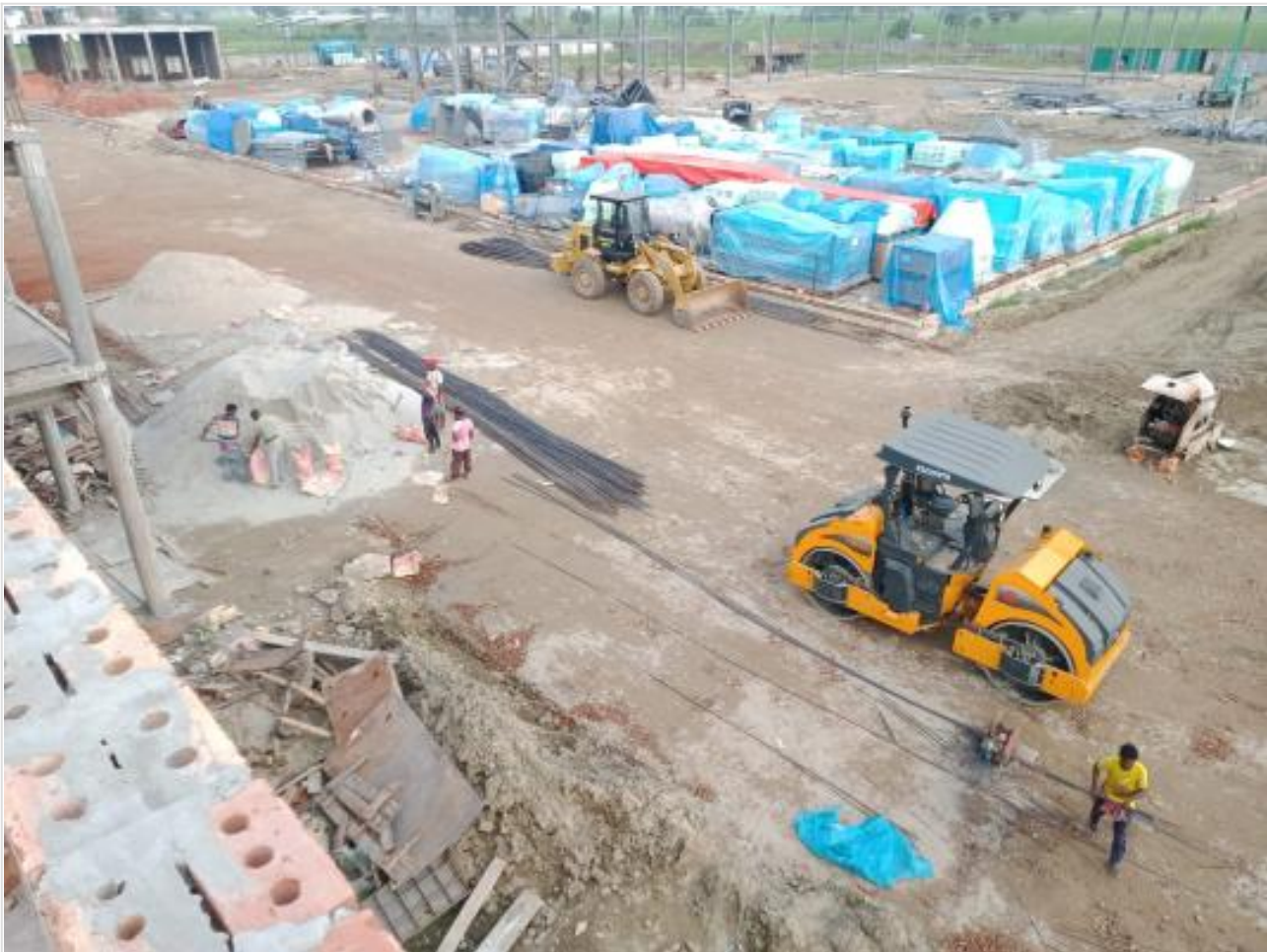
Road work on 03-09-23
