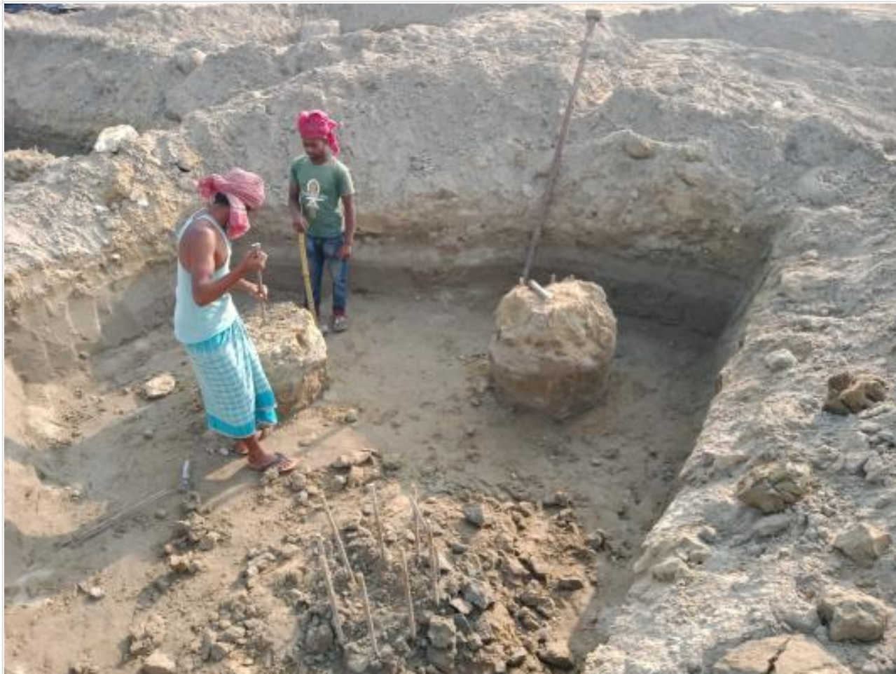
Pile cap earth cutting on 27-03-23
