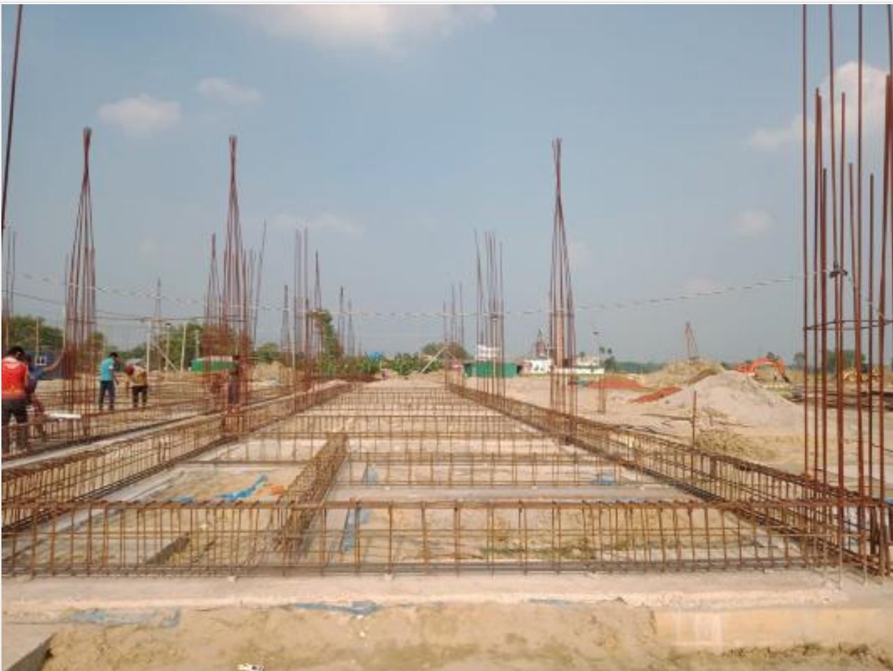
Comp. Bldg. GB Re-bar work on 05-05-23
