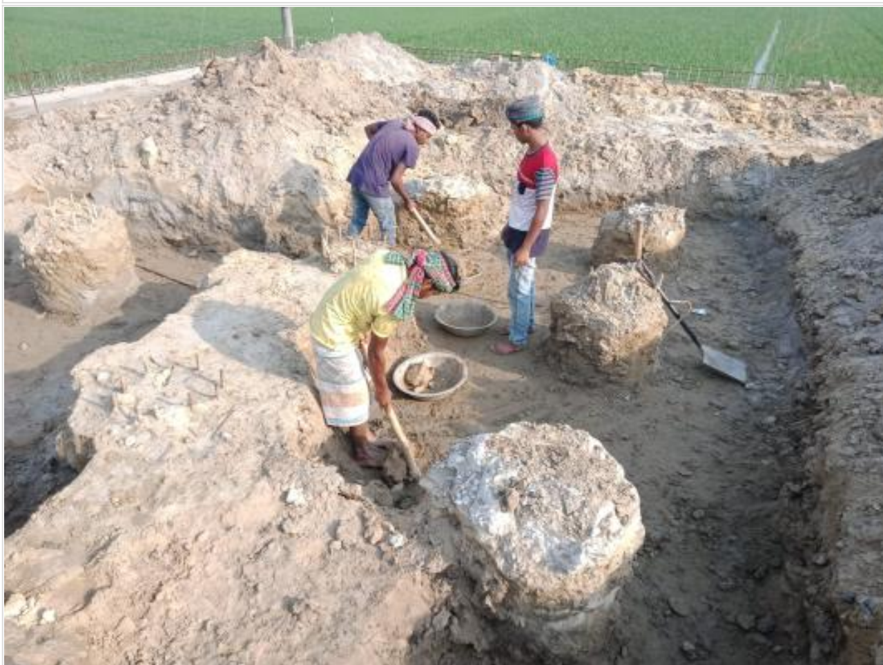
Pile cap earth cutting on 27-03-23
