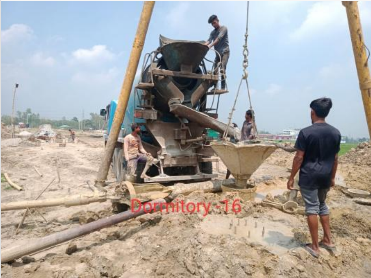
Ready mix concreting of pile on 02-04-23
