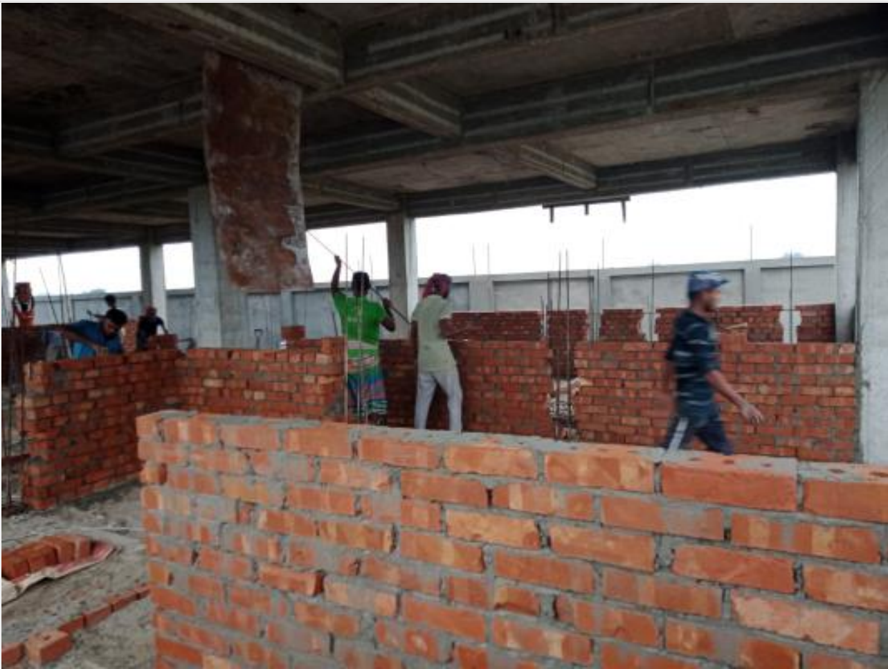
Dorm. Brick work on 22-09-23
