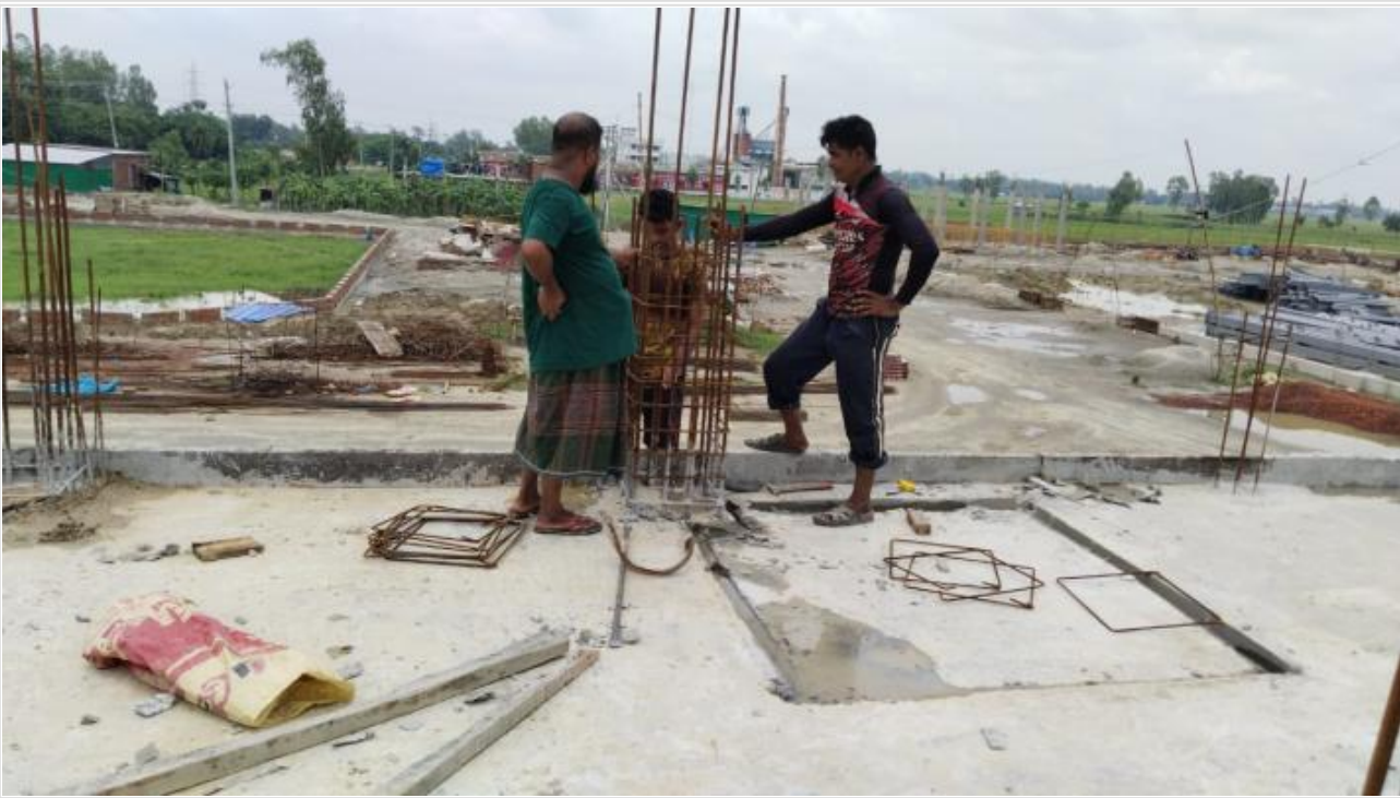
Comp. Bldg. 1st floor column Rebar work on 04-07-23
