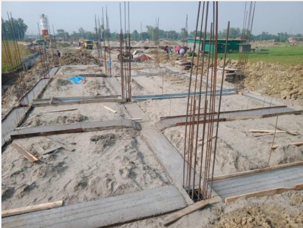
Dorm. Bldg. GB Bottom CC work on 03-06-23
