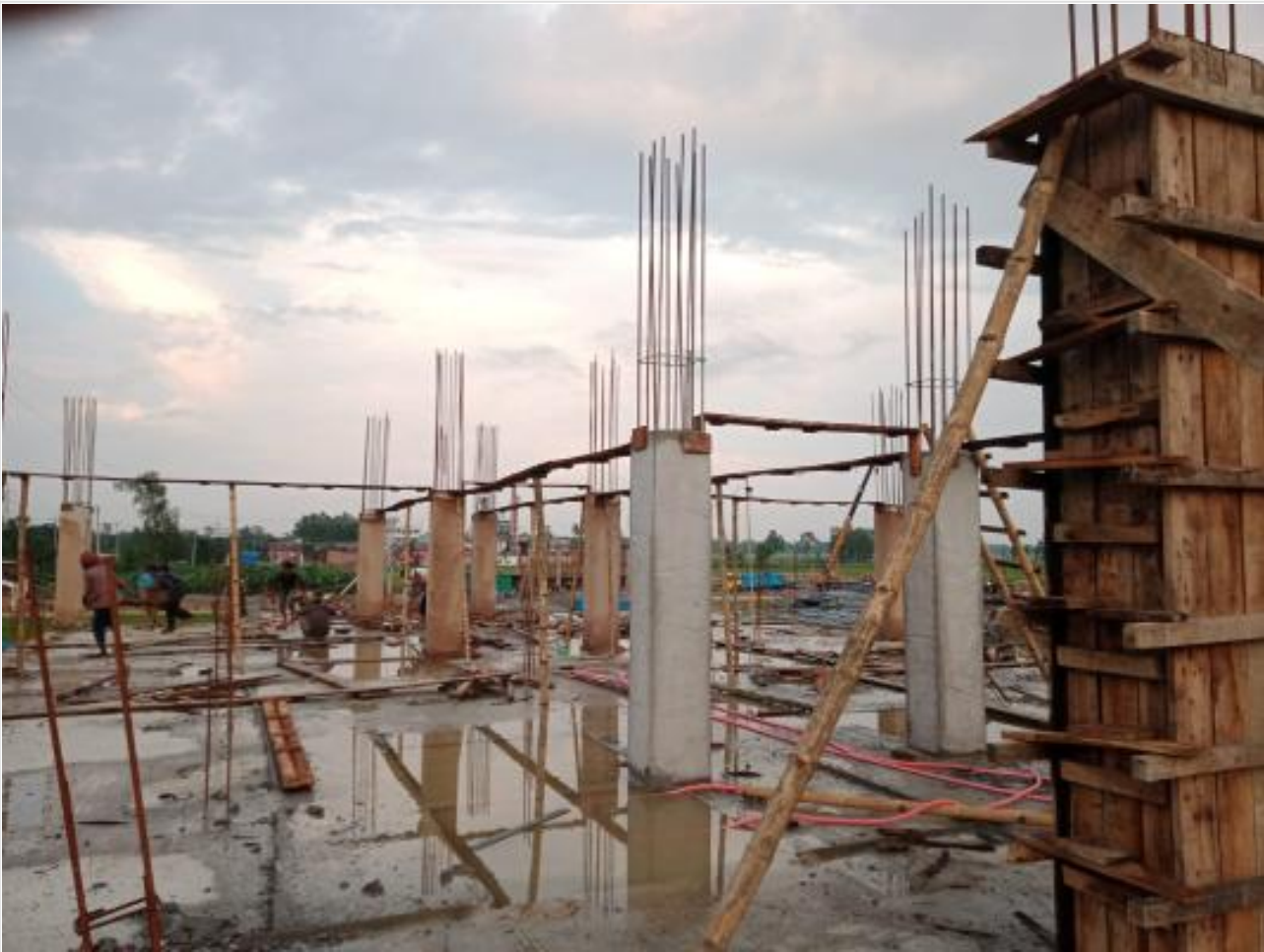
Comp. Bldg 1st floor roof slab work on 14-07-23
