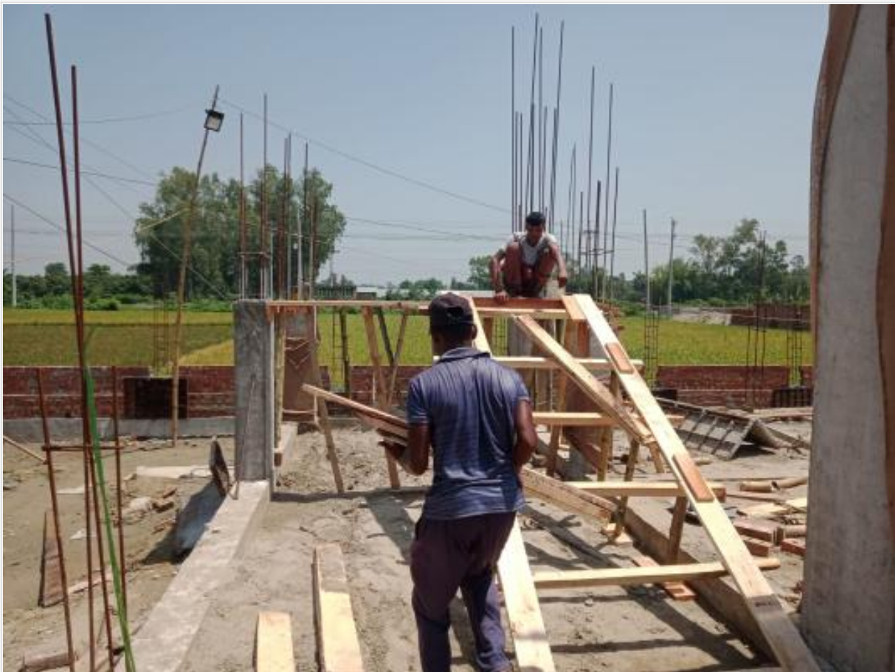
Comp. Bldg. Stair shuttering on 02-06-23
