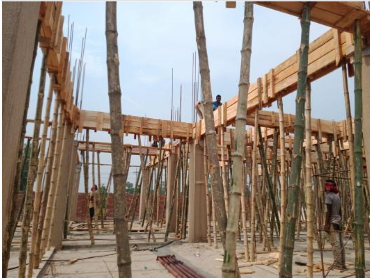
Comp. Bldg. Slab beam shuttering on 07-06-23
