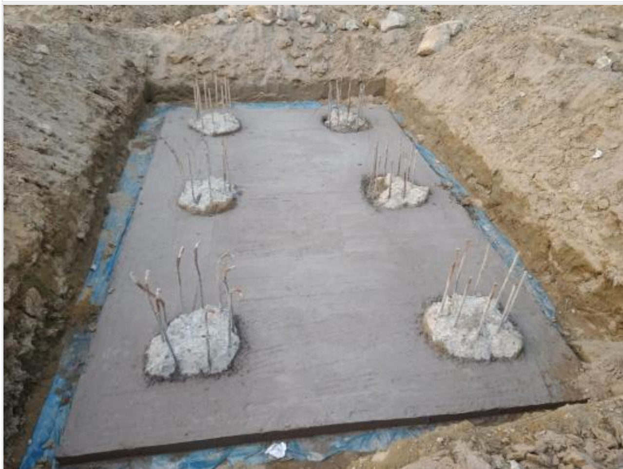
Pile head finishing for test on 03-04-23
