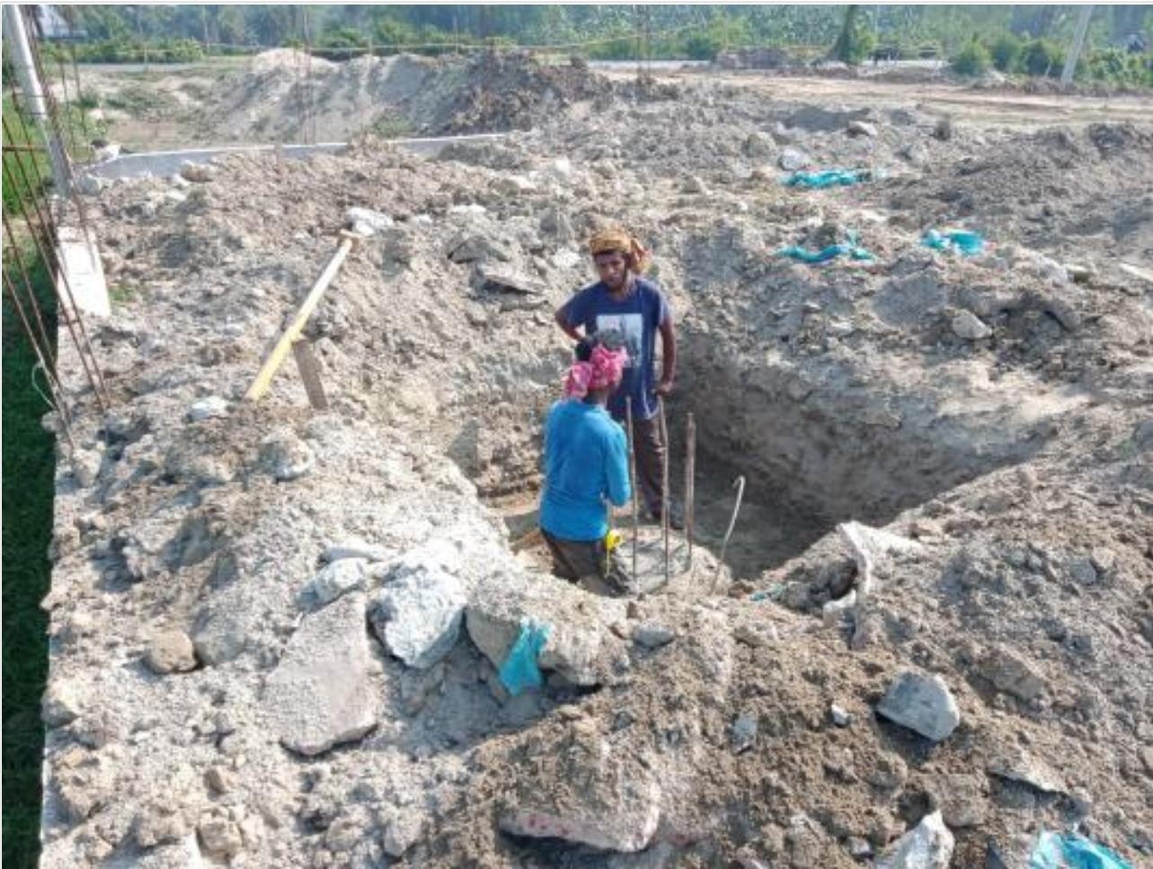
Dorm. Bldg. Earth cutting for PH Breakin on 02-05-23
