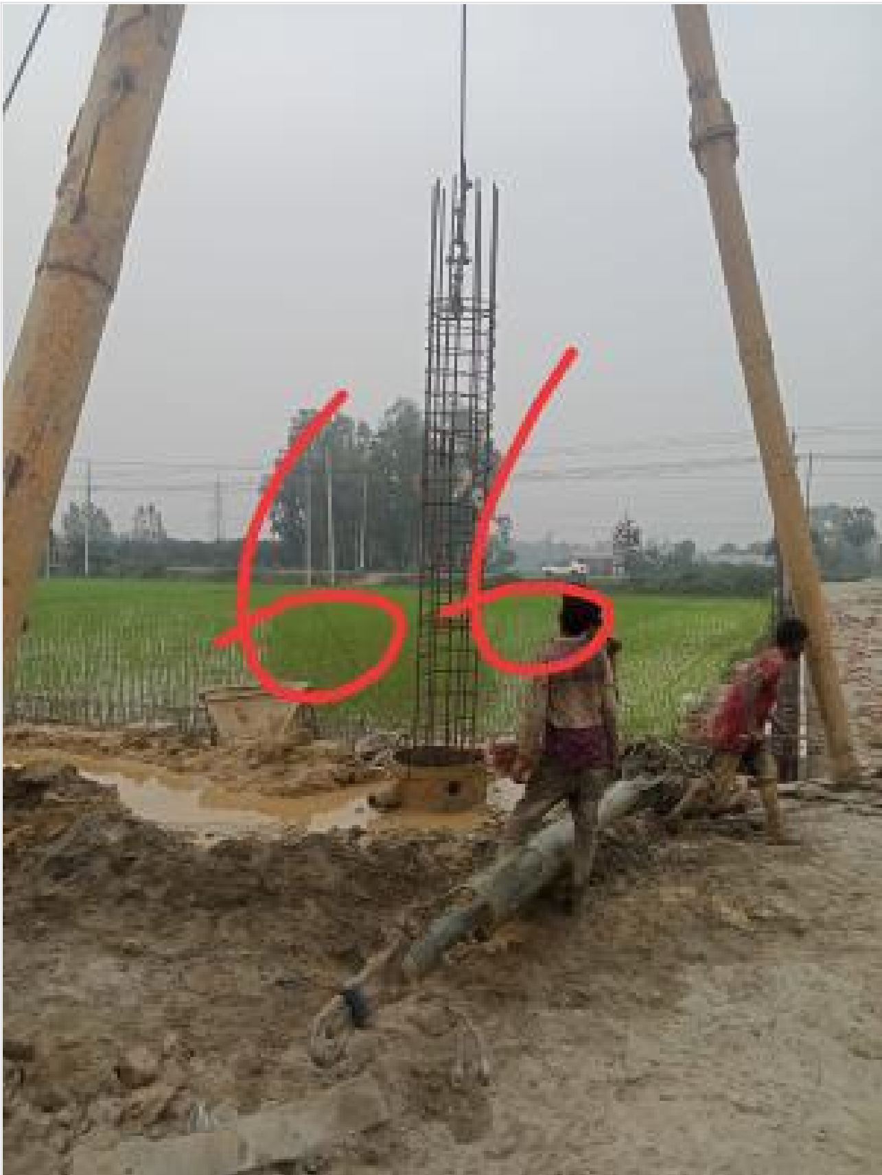
Com. Bldg. 66 Pile Boring on 16-03-23
