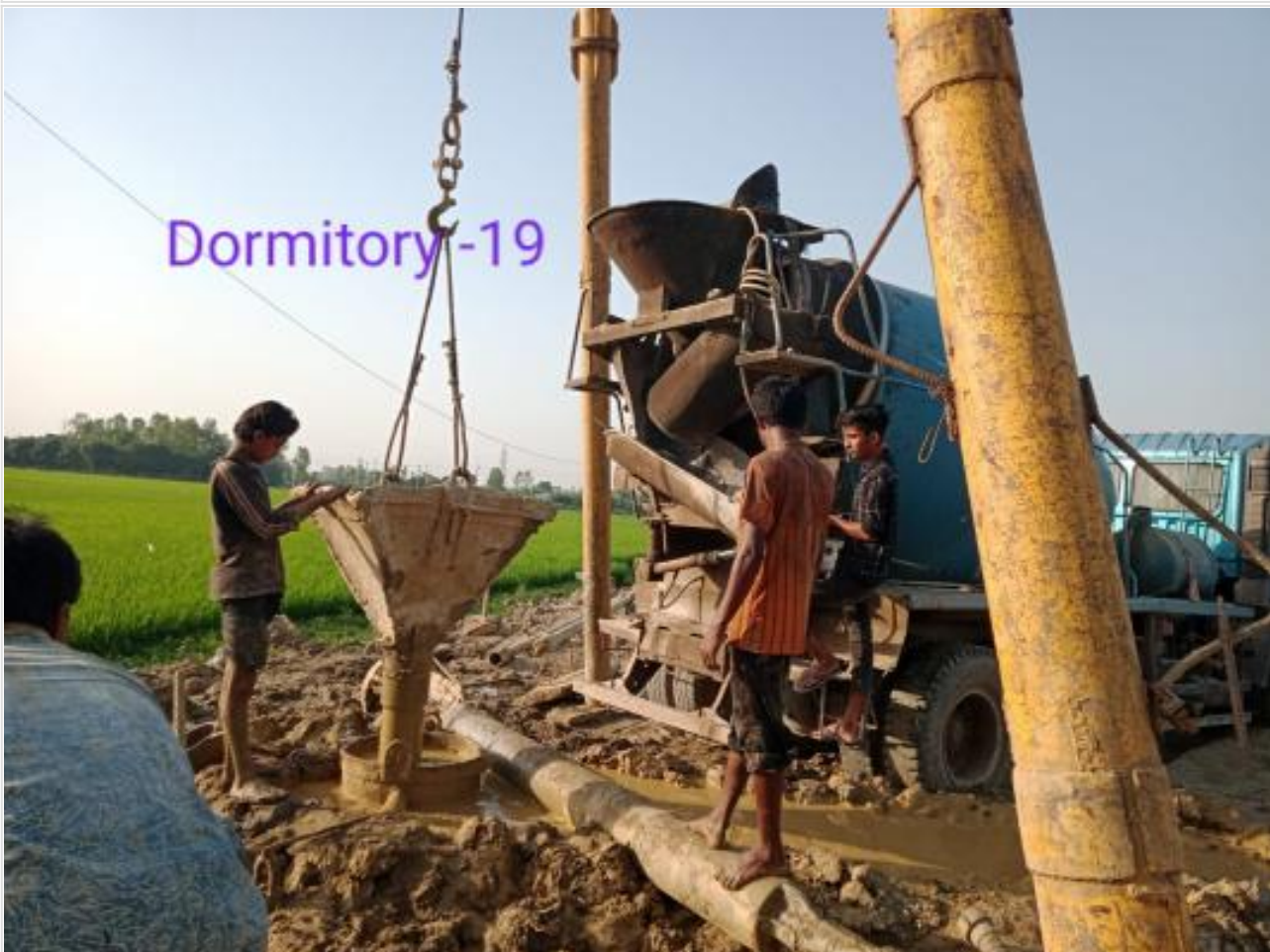
Pile cap bottom cc casting. on 04-04-23
