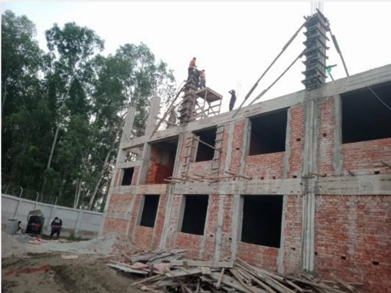
Dorm. Bldg. 2nd floor column work on 03-11-23
