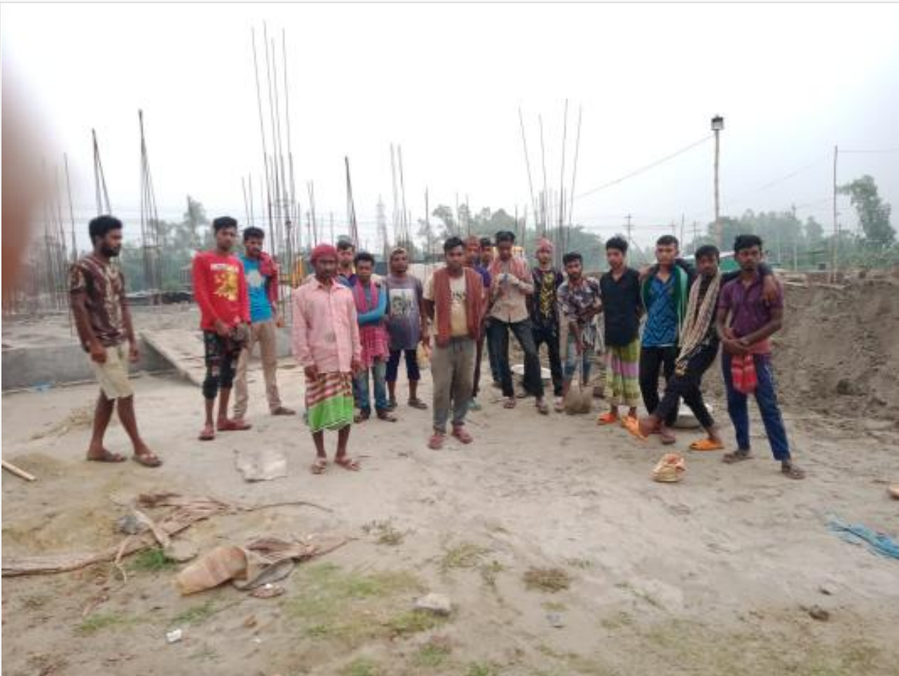
Civil worker on 21-05-23
