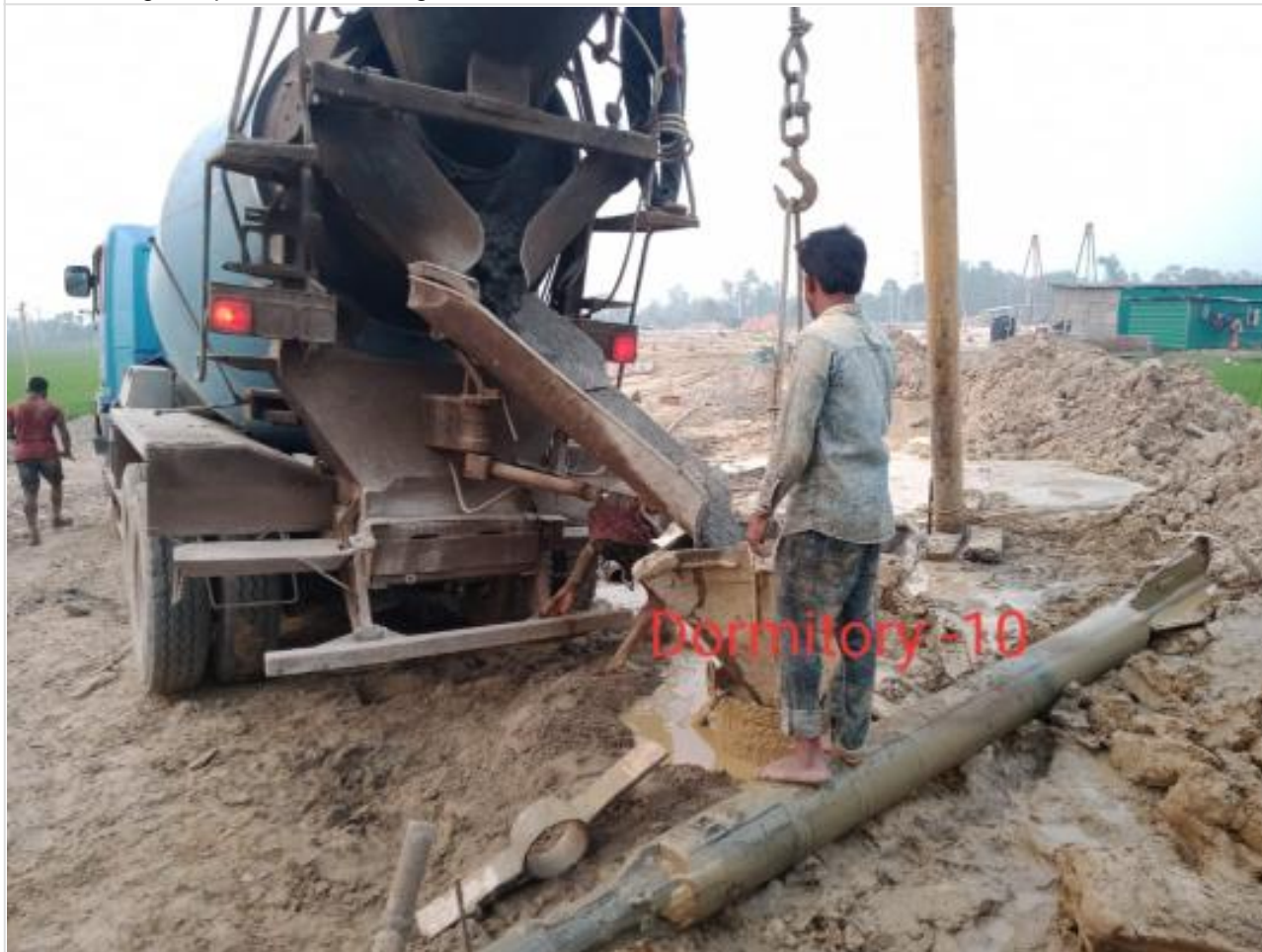
Dorm. Bldg. 10th pile concreting on 30-03-23
