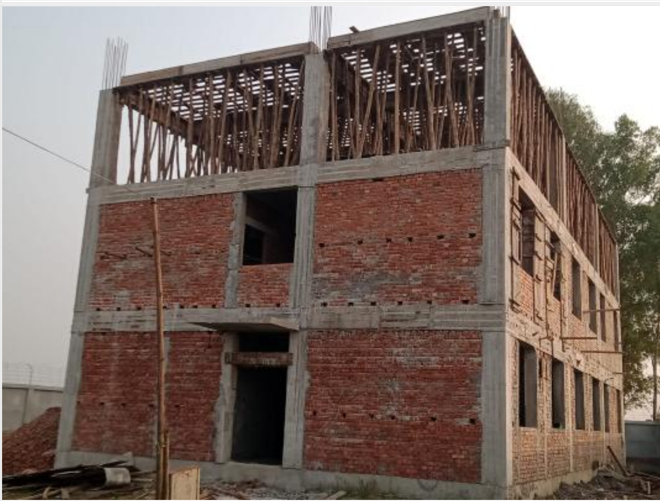
Dorm. Bldg. 3rd floor shuttering work on 09-11-23
