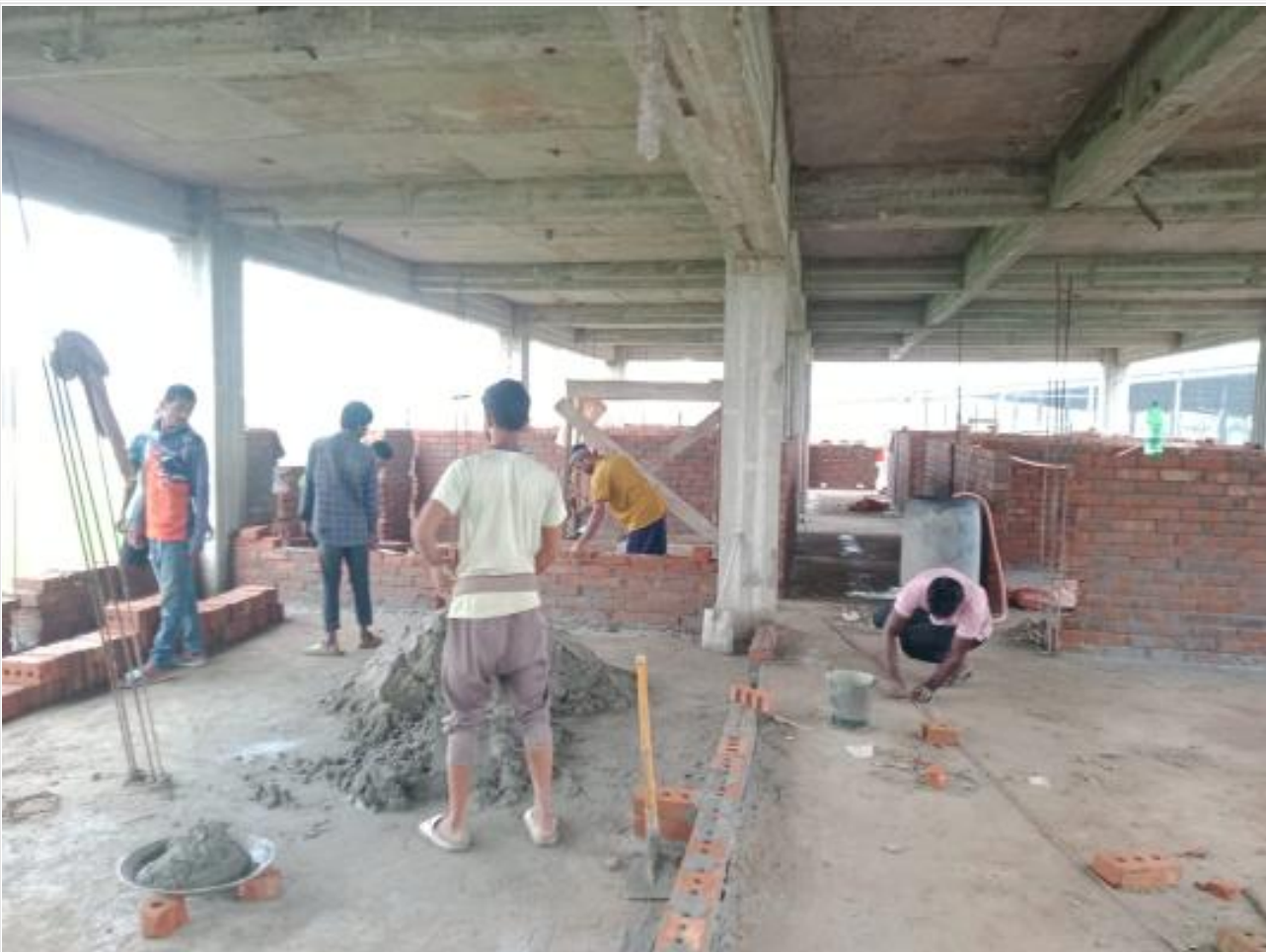
Dorm. 1st floor brick work on 07-10-23
