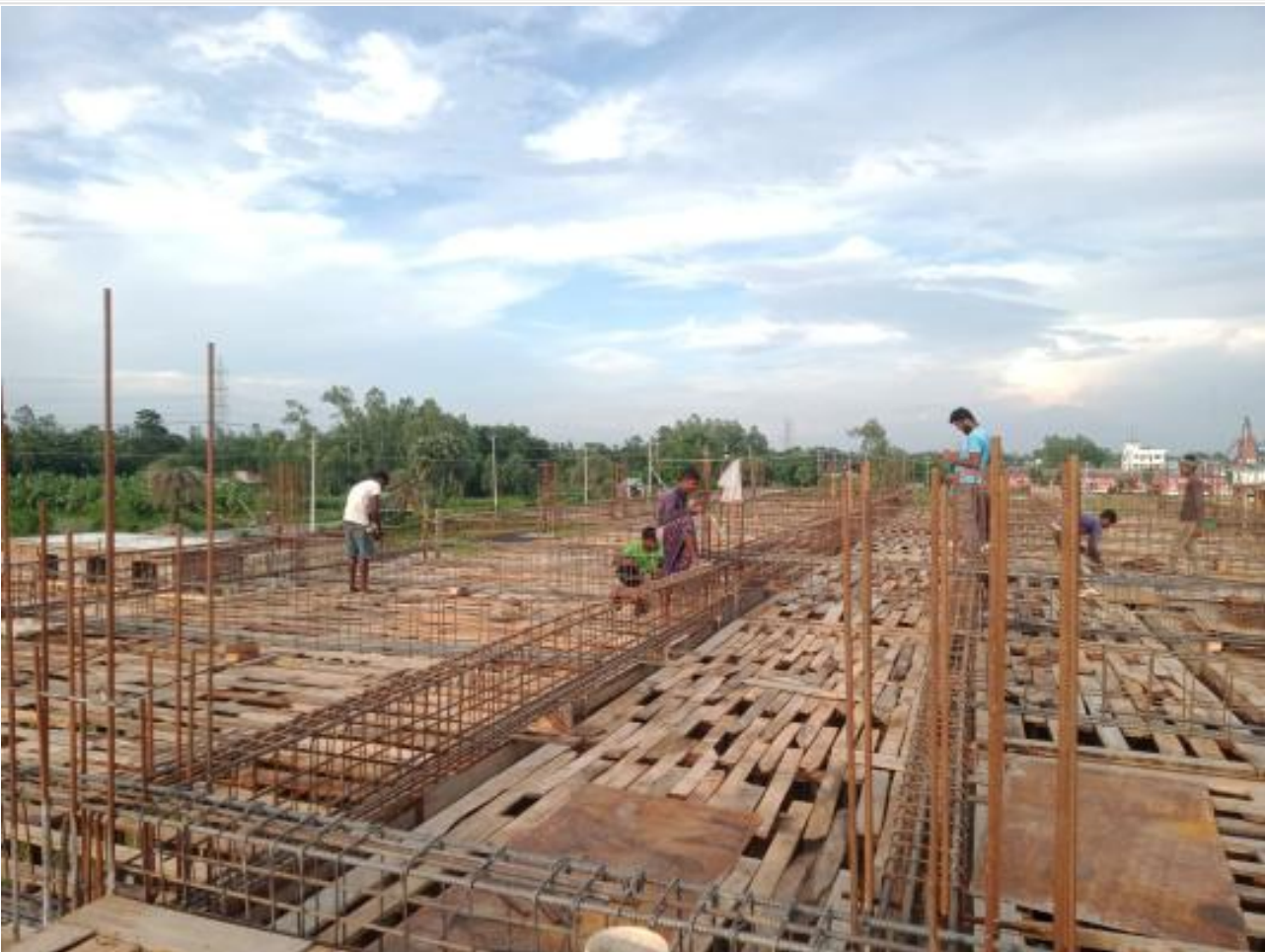
Comp. Bldg. 2nd Floor rebar work on 28-07-23
