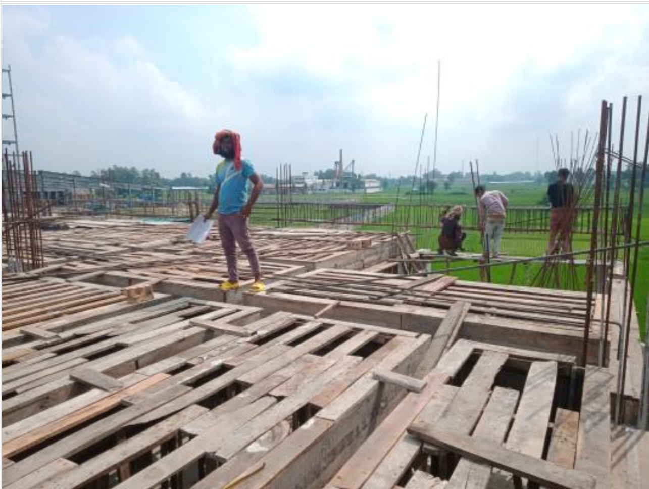
Dorm. Bldg. 2nd floor shuttering work on 06-09-23
