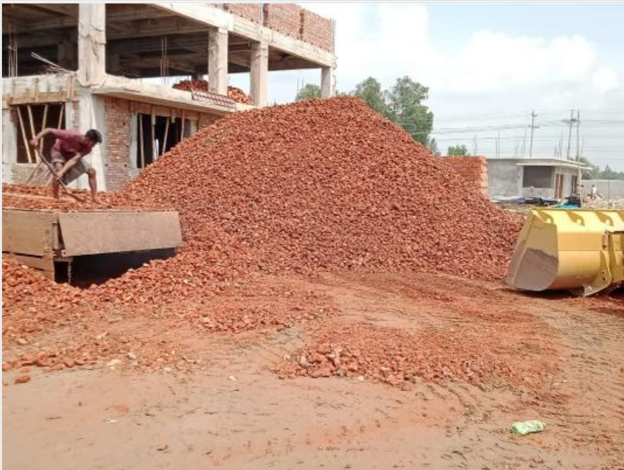
Material stock for Road Sub-base on 21-08-23
