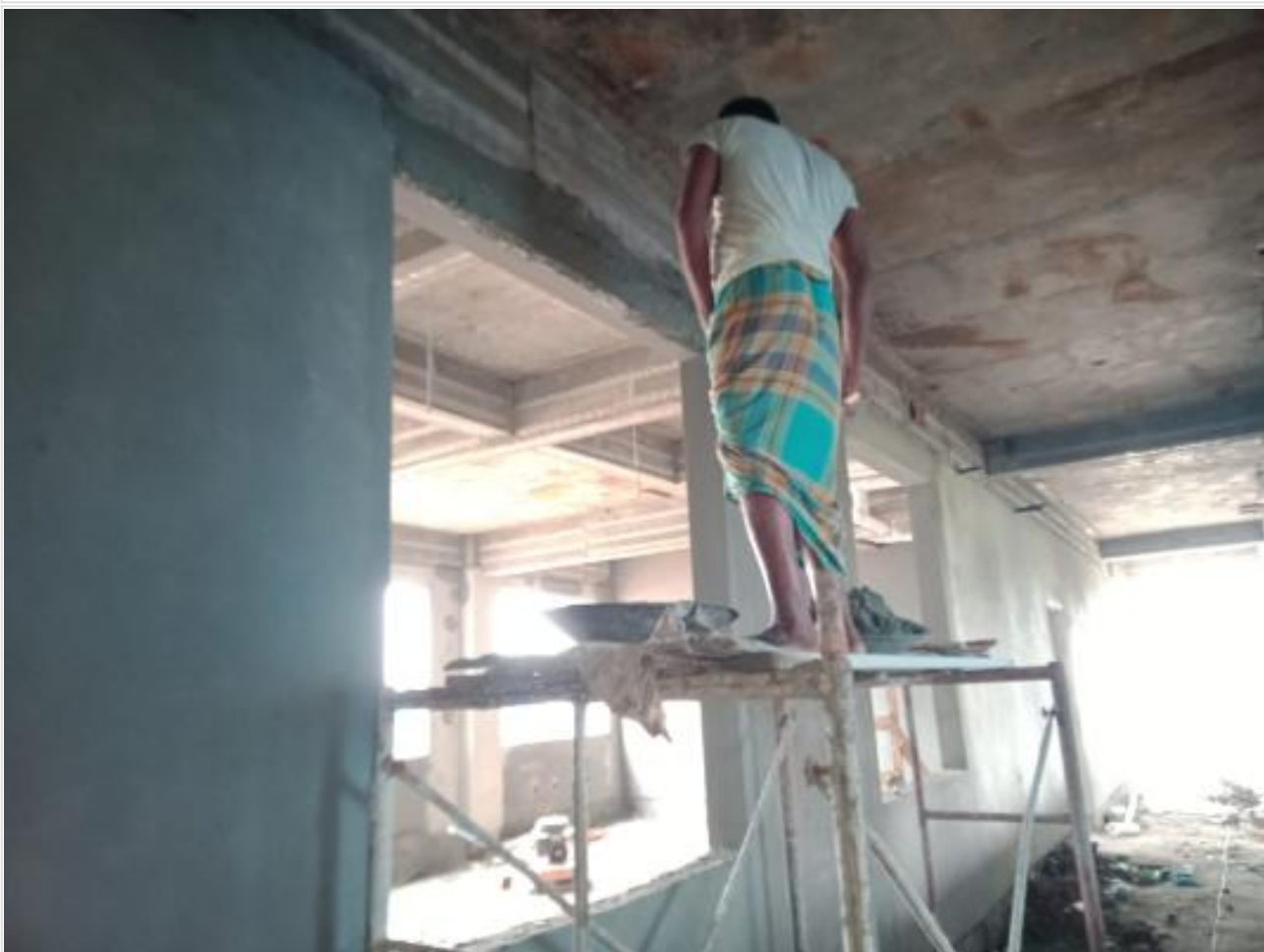
Comp. Bldg FF plastr wok on 19-09-23
