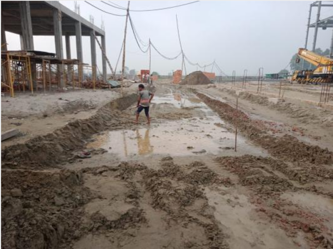
Road-Excavation-box cutting on 16-08-23
