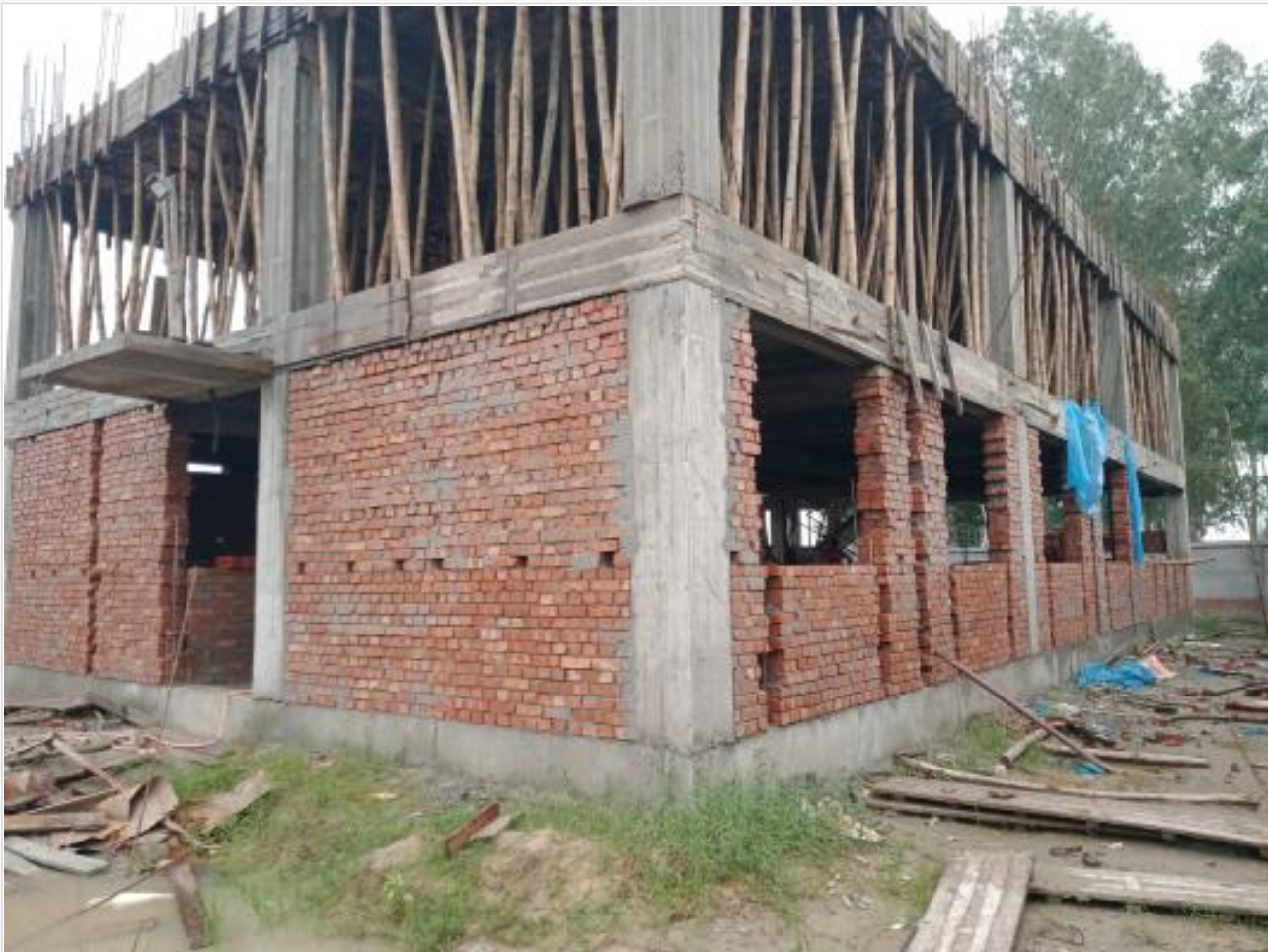
Dorm.Bldg. GF brick work on 25-09-23
