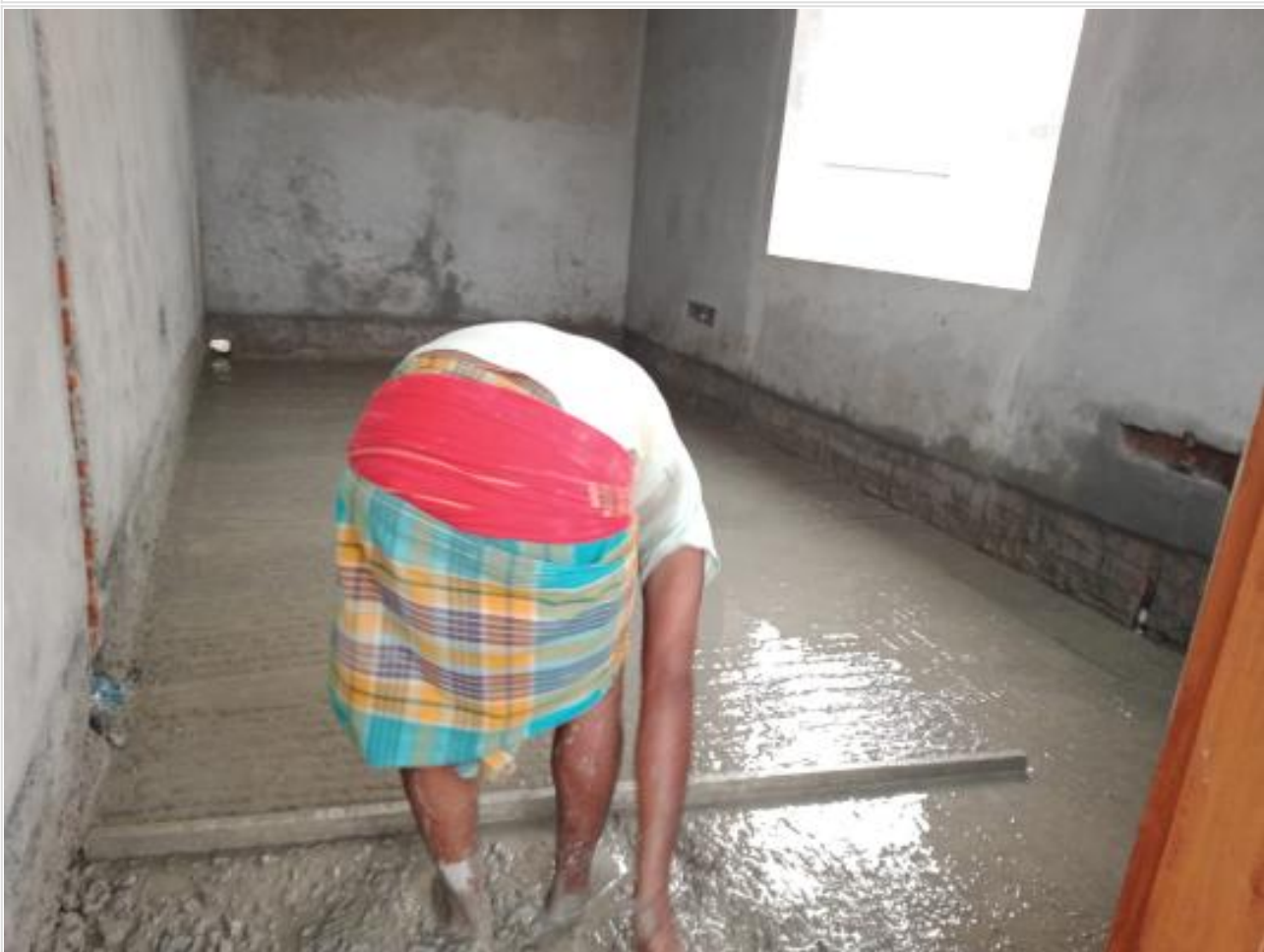
Gate House floor casting on 01-09-23
