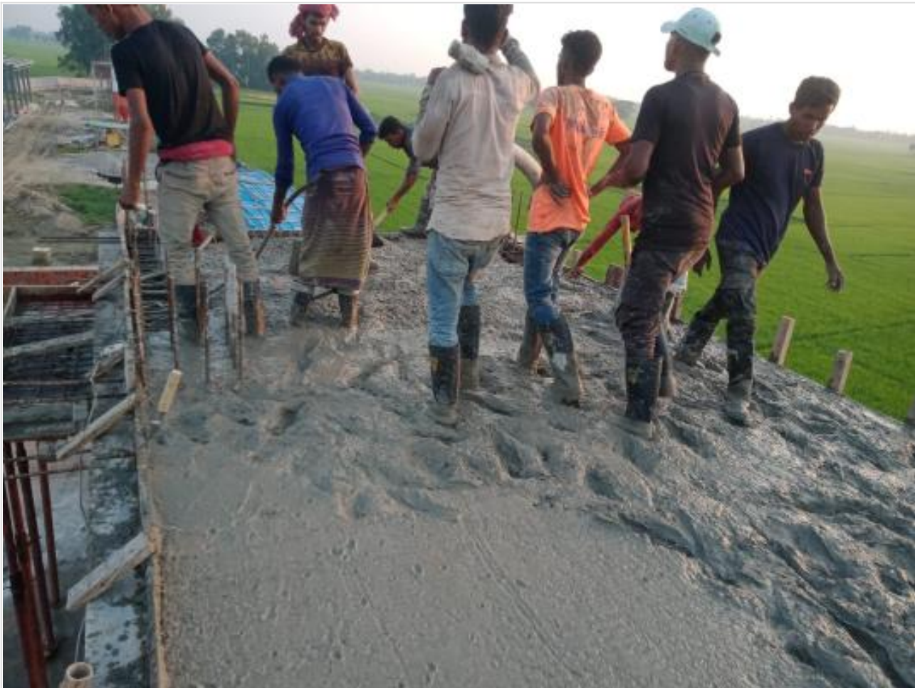
Comp. Bldg. Roof top concreting work on 16-09-23
