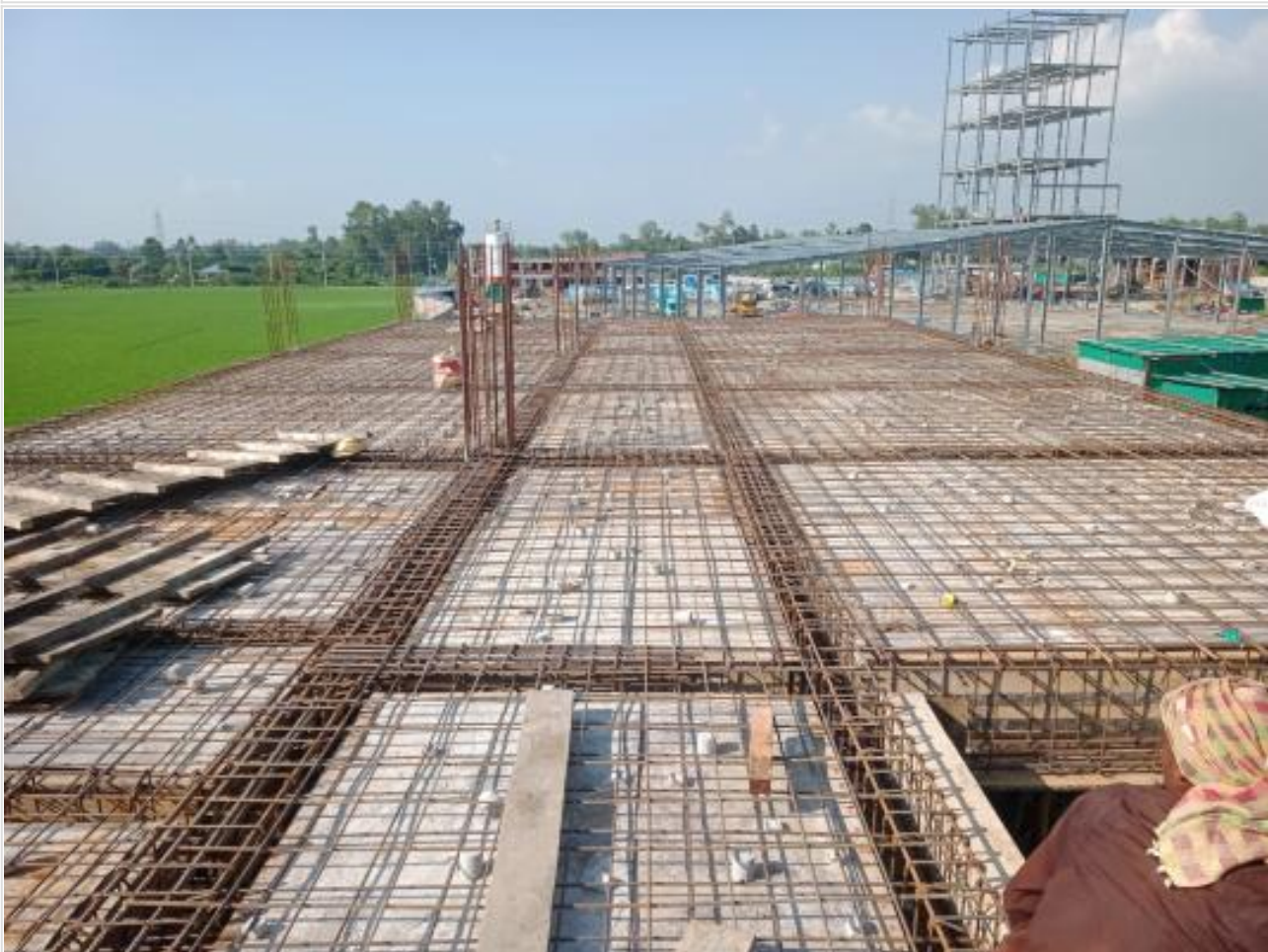
Dorm. Bldg. 2nd floor rebar work on 09-09-23
