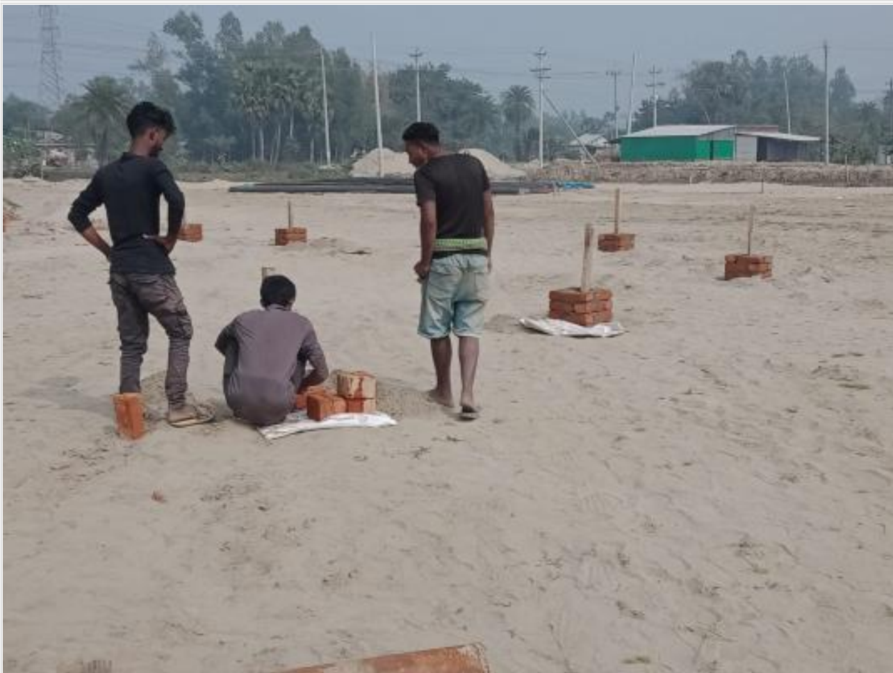
Brick-work around Pile point on 05-02-23
