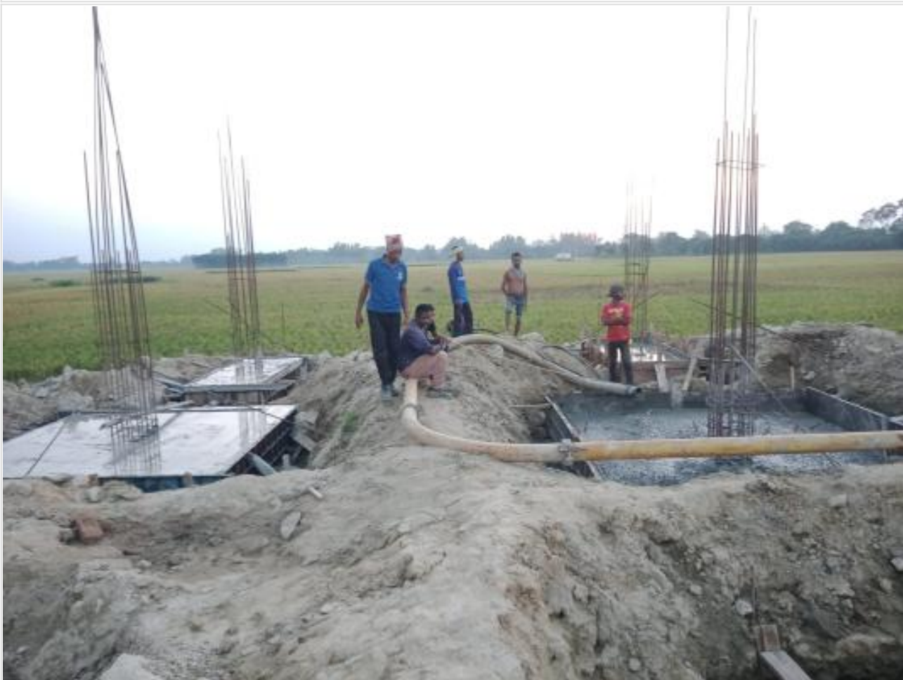
Dorm.Bldg. pile cap casting on 29-05-23
