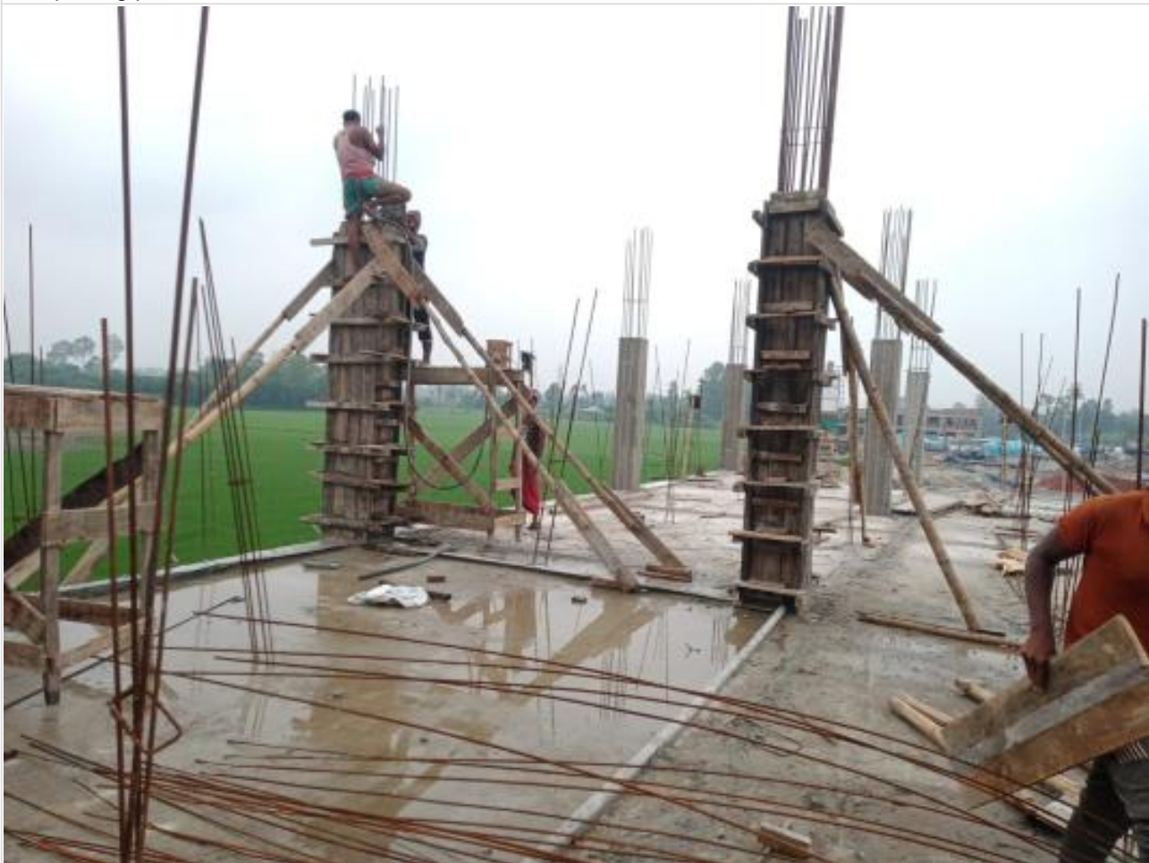
Dormitory bldg. Column casting on 26-08-23
