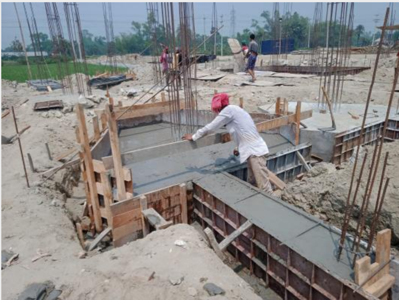
Pile cap concreting on 18-04-23
