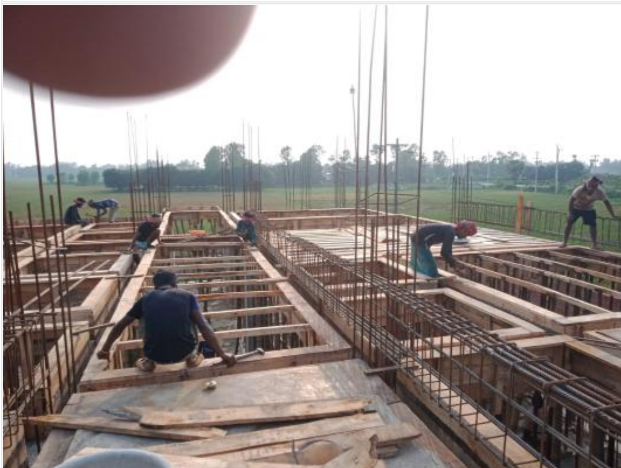
Comp. Bldg. Rebar work on 11-06-23
