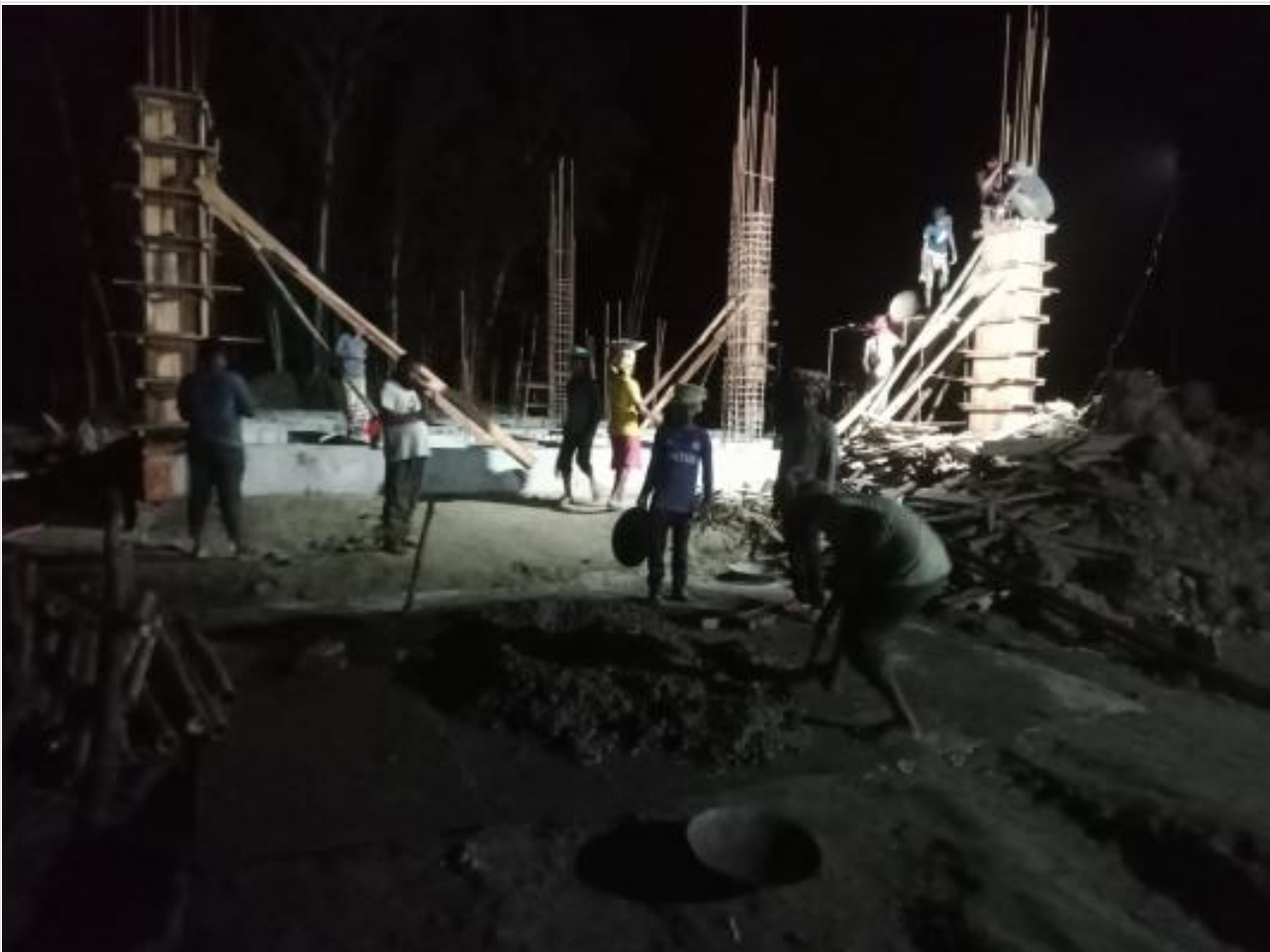
Dorm. Bldg. Column casting on 18-06-23
