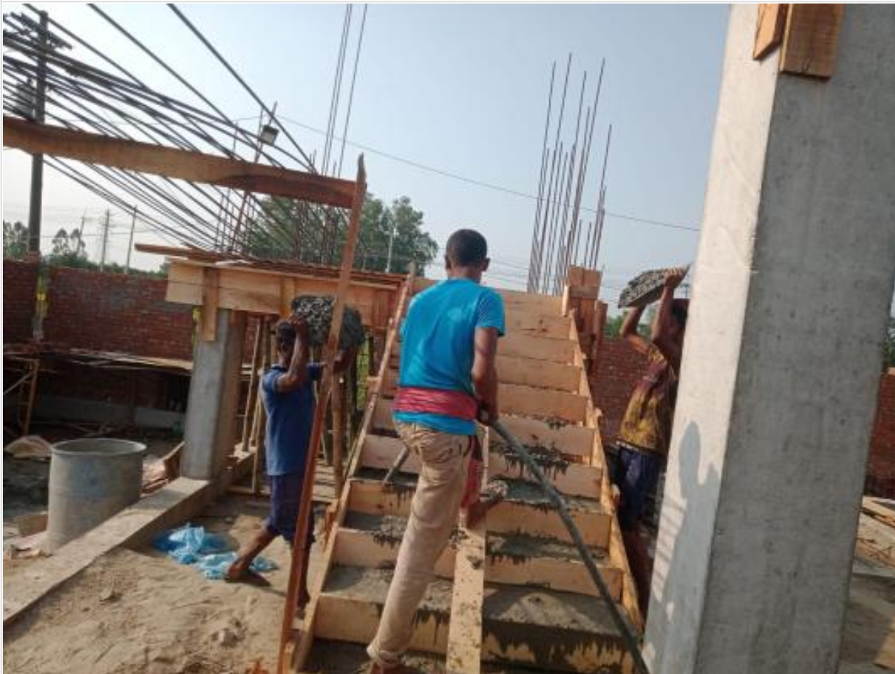
1st flight stair casting on 05-06-23
