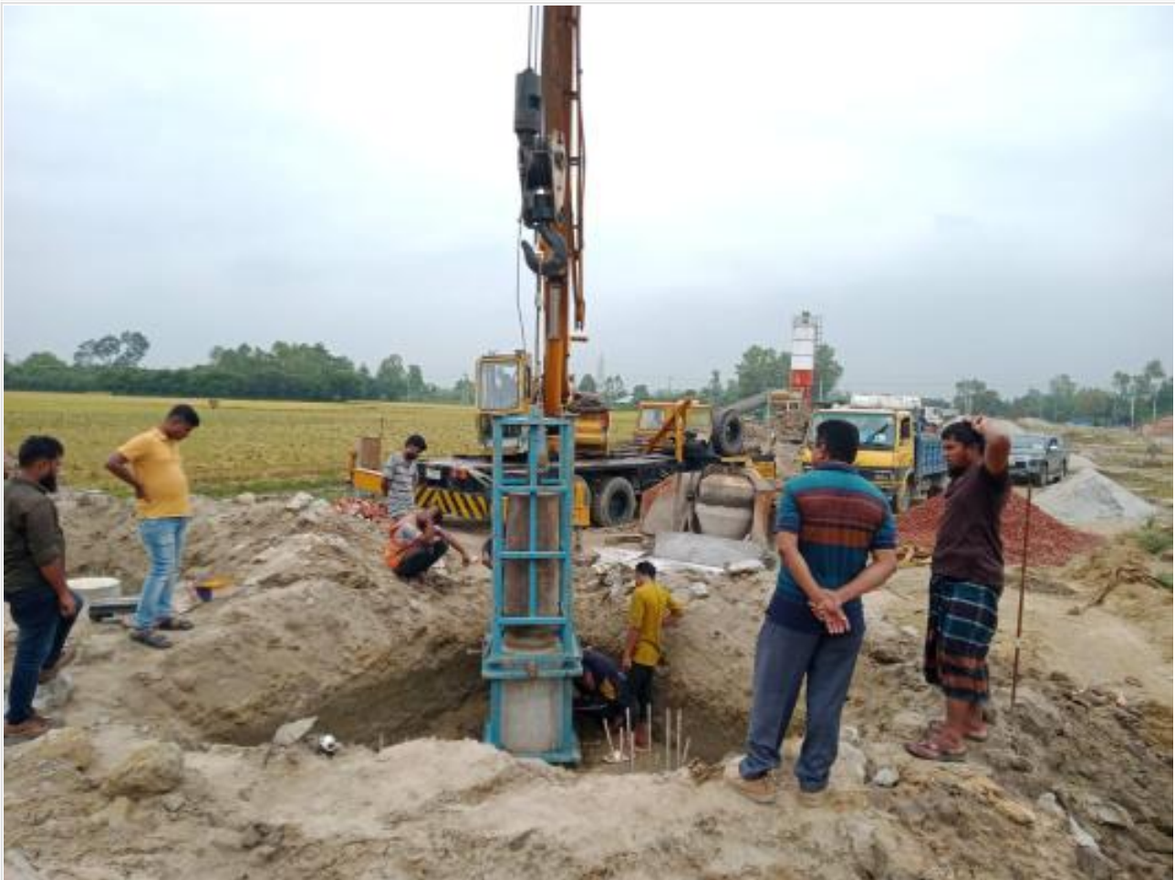
Pile load test on 19-05-23
