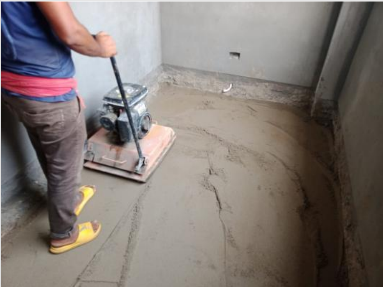
Dorm. Bldg. GF sand khoa cushion on 09-11-23
