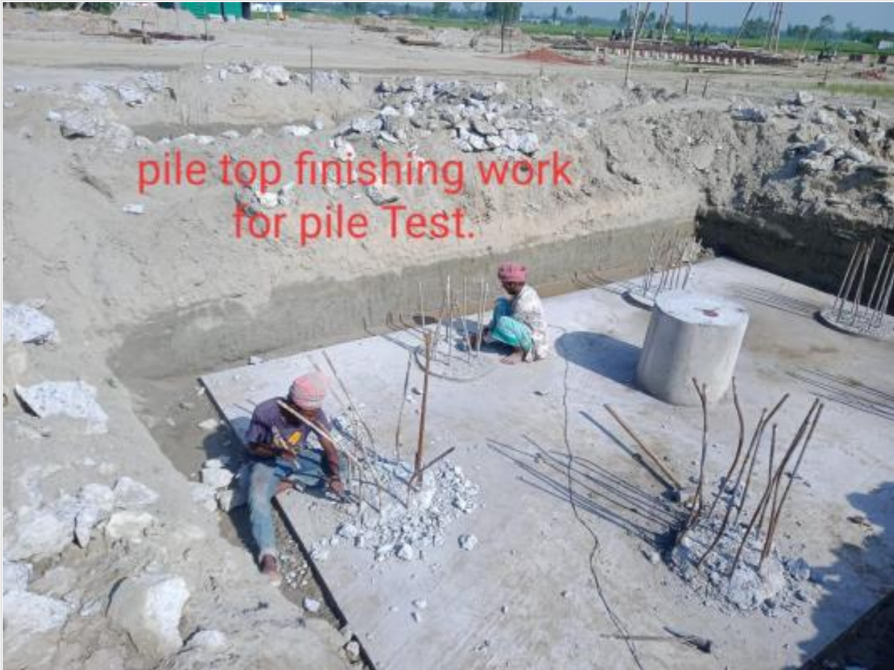
Pile head finishing for test on 07-04-23
