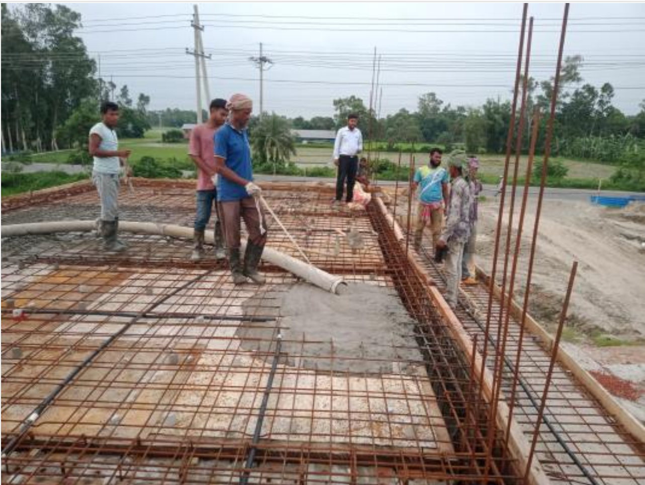
Gate House Slab casting on 11-07-23
