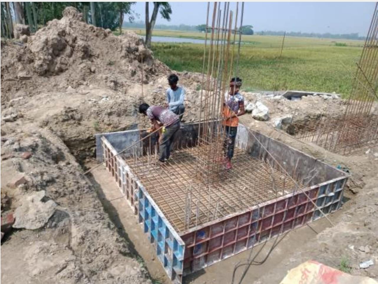
Dorm. Bldg pile cap work on 25-05-23
