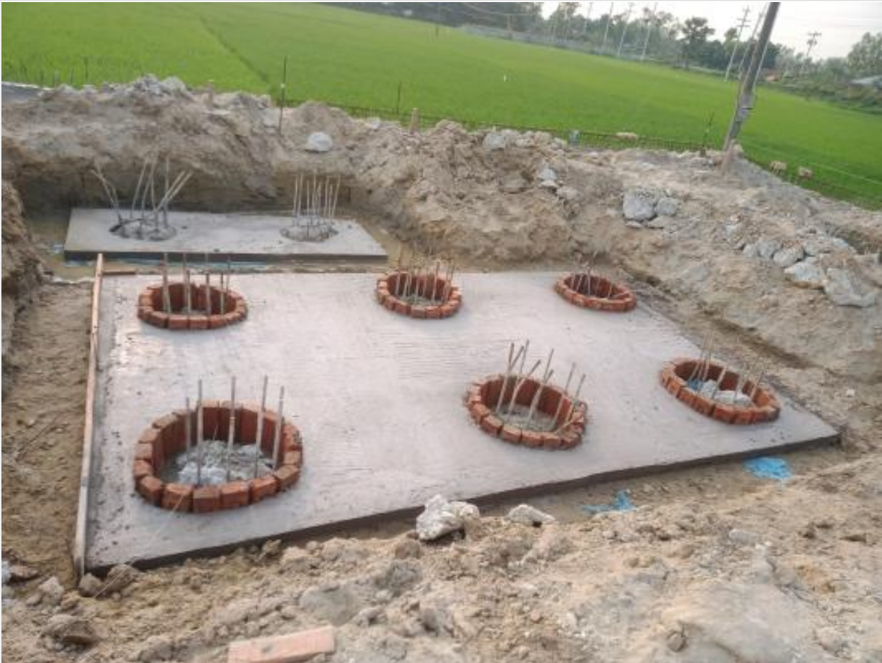
Pile cap bottom cc casting. on 04-04-23
