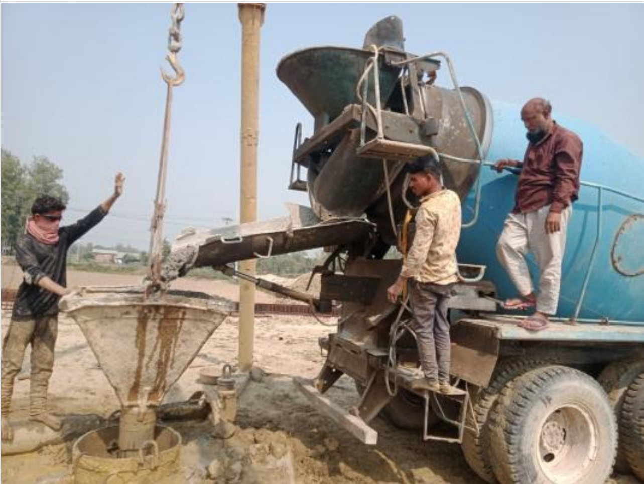
Ready mix concreting of pile on 15-02-23
