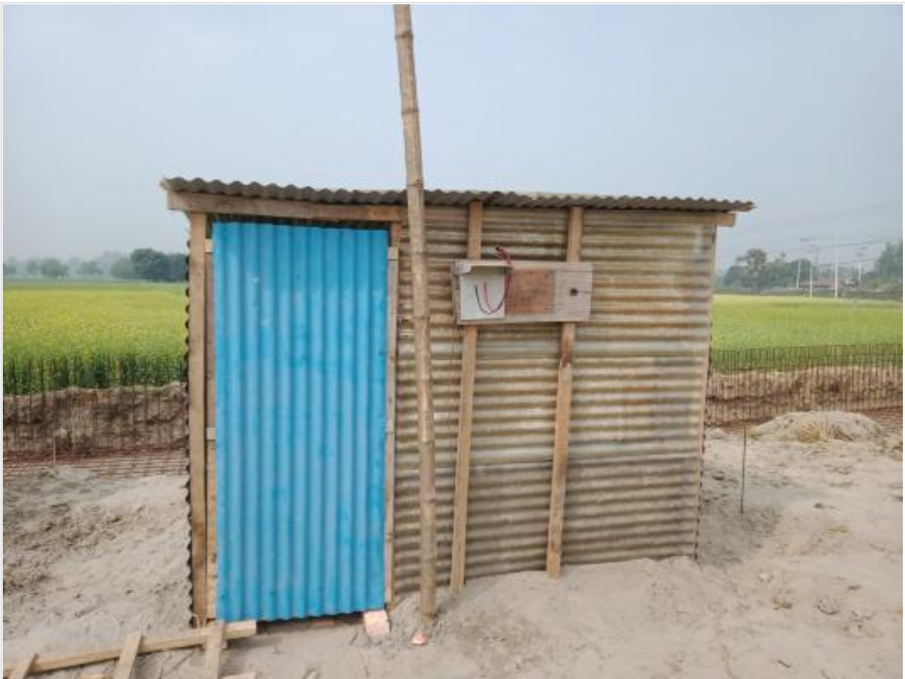
Electrical DB Setting on 31-01-23
