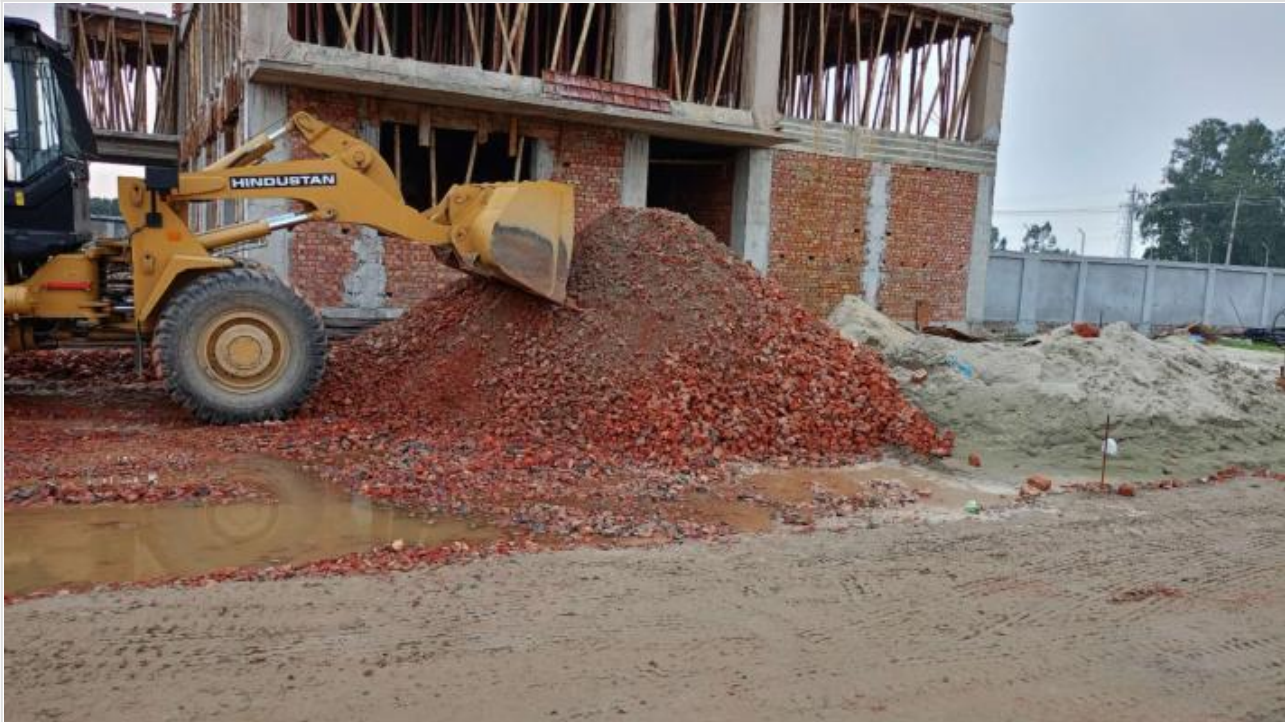
Sub-base-Khoa unloading on 14-08-23
