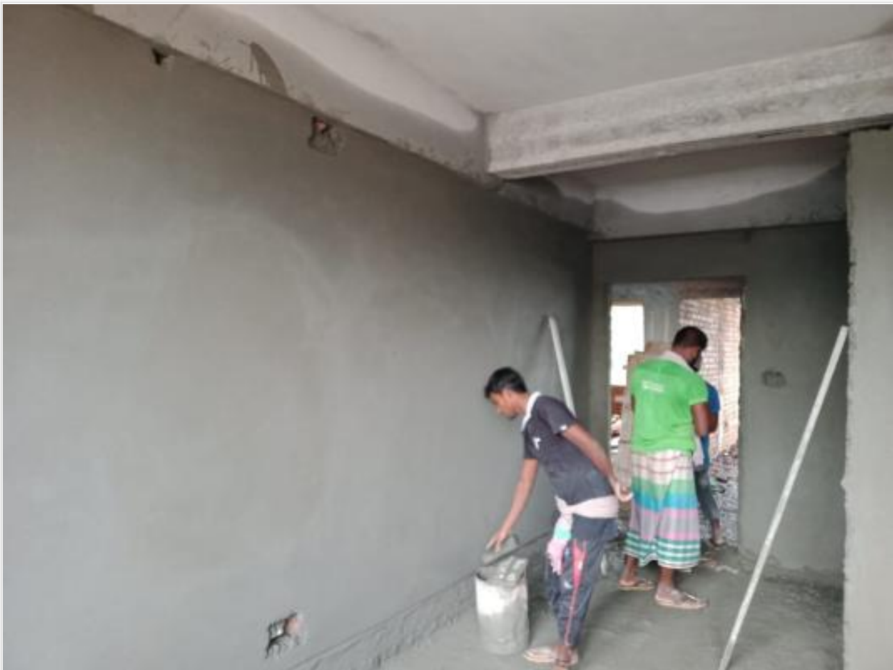
Comp. Bldg. Plaster work on 20-09-23
