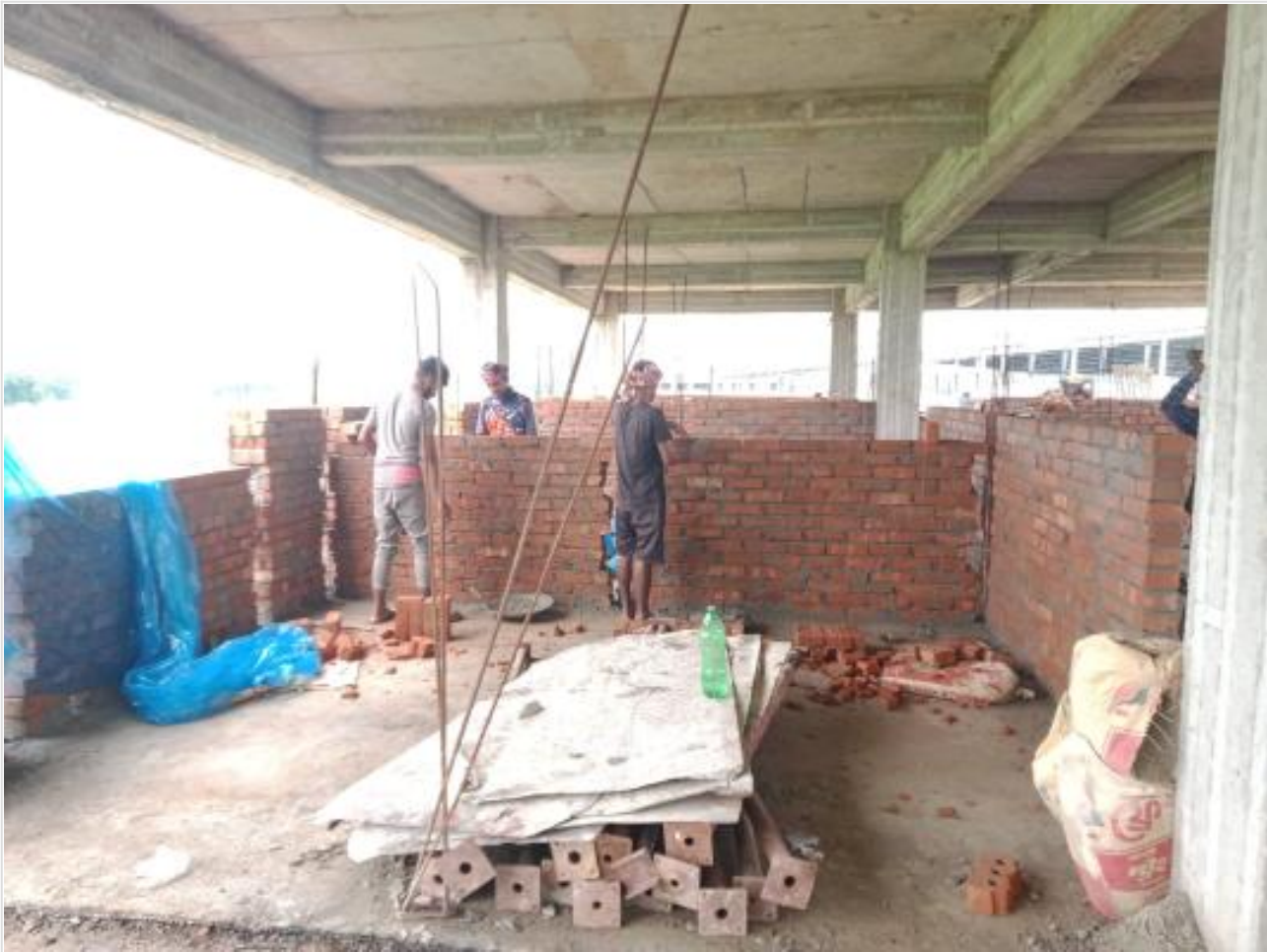
Dorm. Bldg Brick work on 07-10-23
