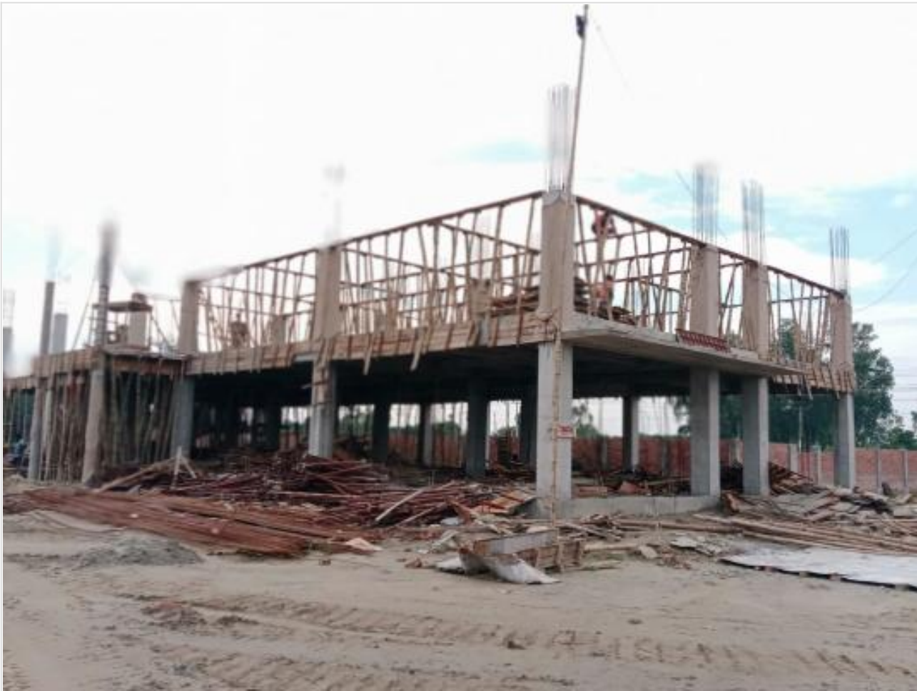
Comp. Bldg 2nd floor shuttering on 16-07-23
