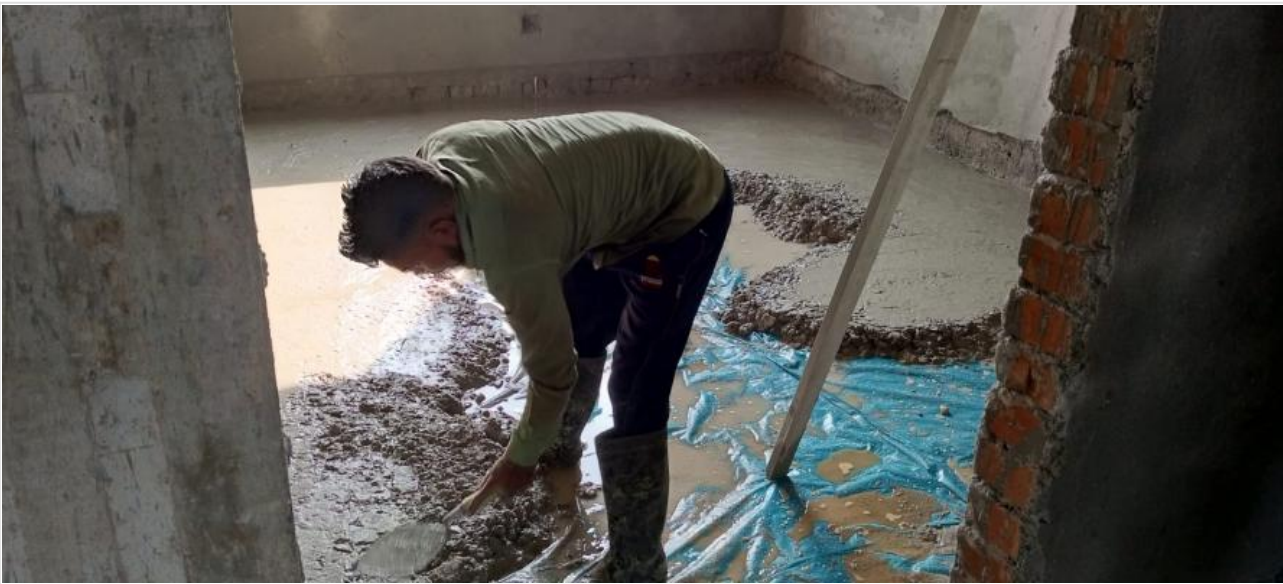
Dorm. Bldg. GF Concreting on 10-11-23
