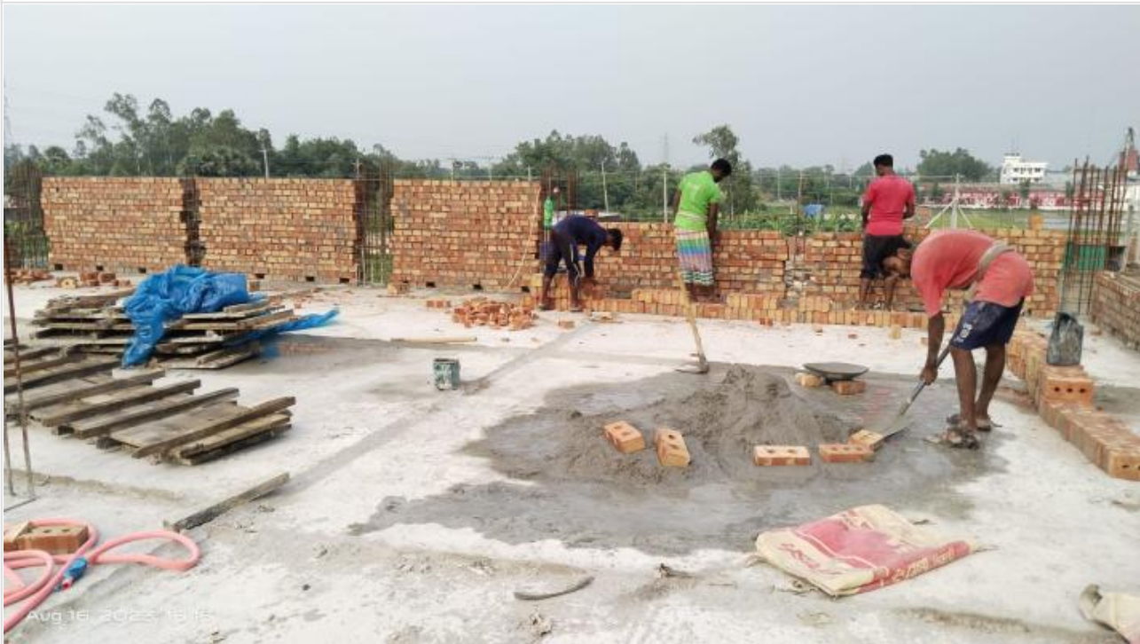
Comp-Parapet Brick-work on 17-08-23
