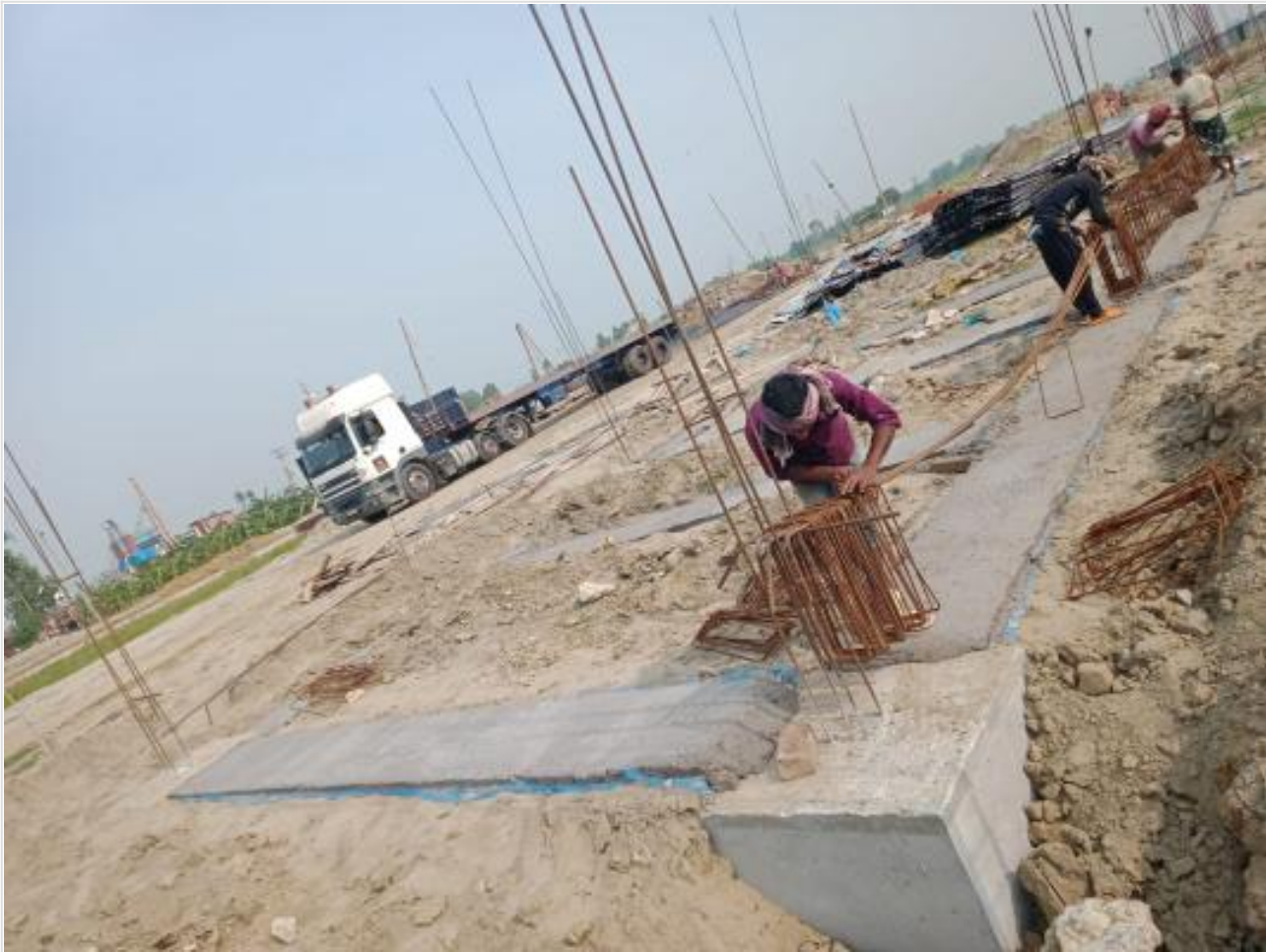
Re-bar work on 13-05-23
