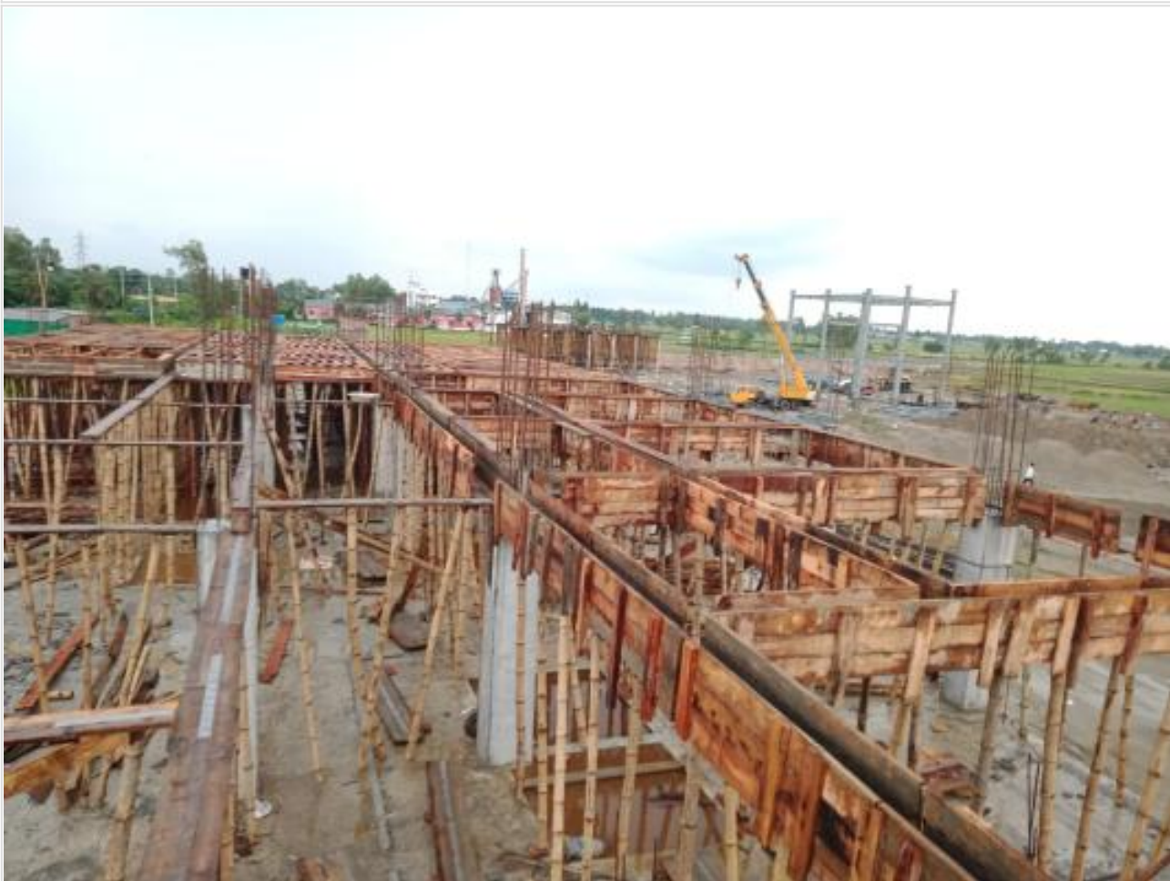
Comp. Bldg. 2nd Floor Slab beam shutteri on 21-07-23
