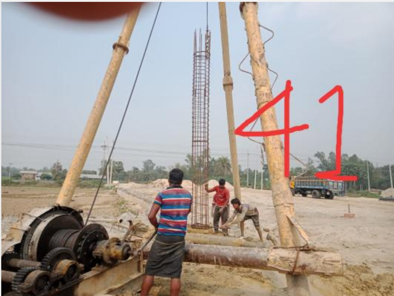
Com. Bldg. 41 Pile Boring on 03-03-23
