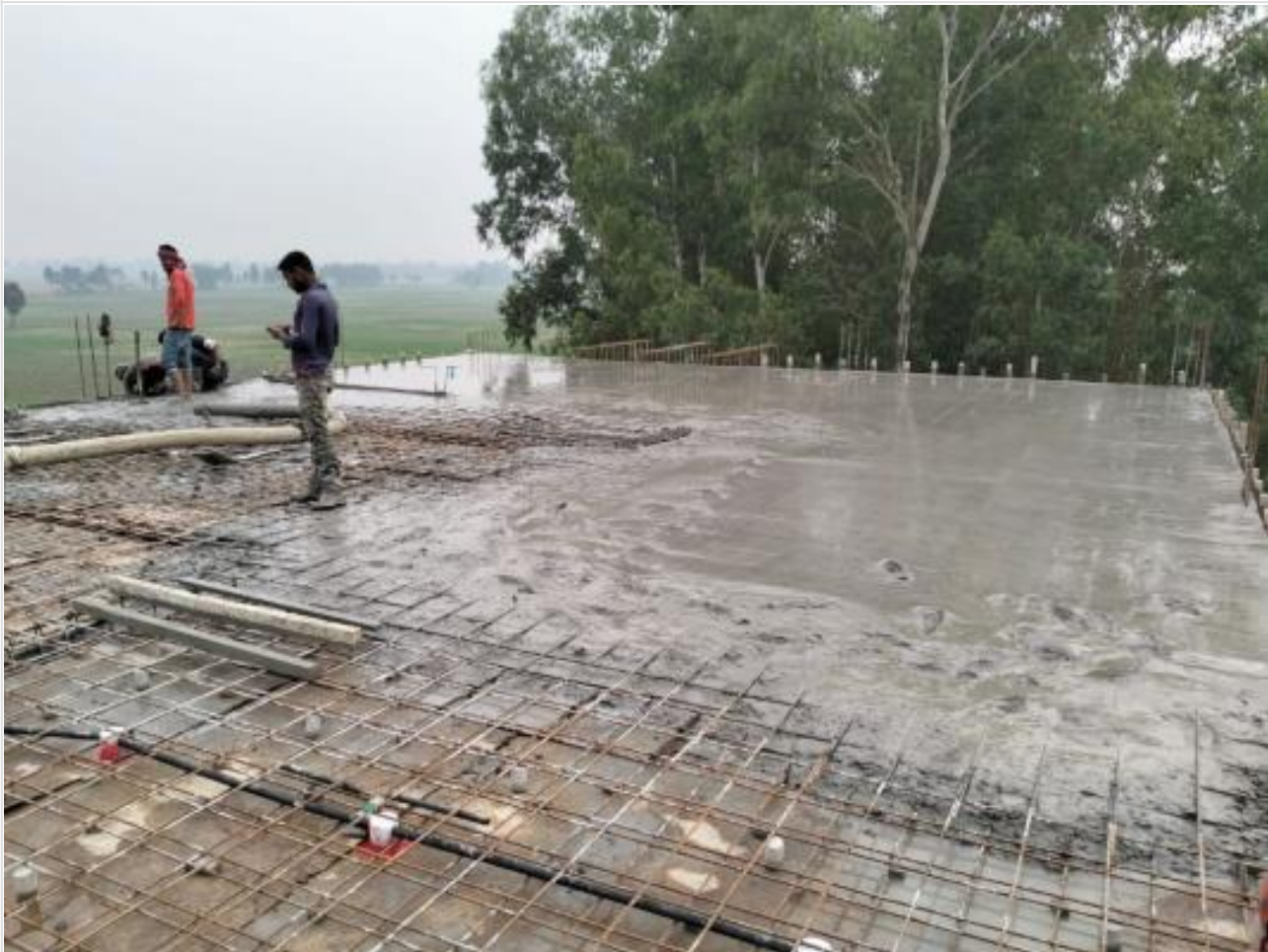
Dormitory-3rd Floor Slab Concreting on 23-12-23
