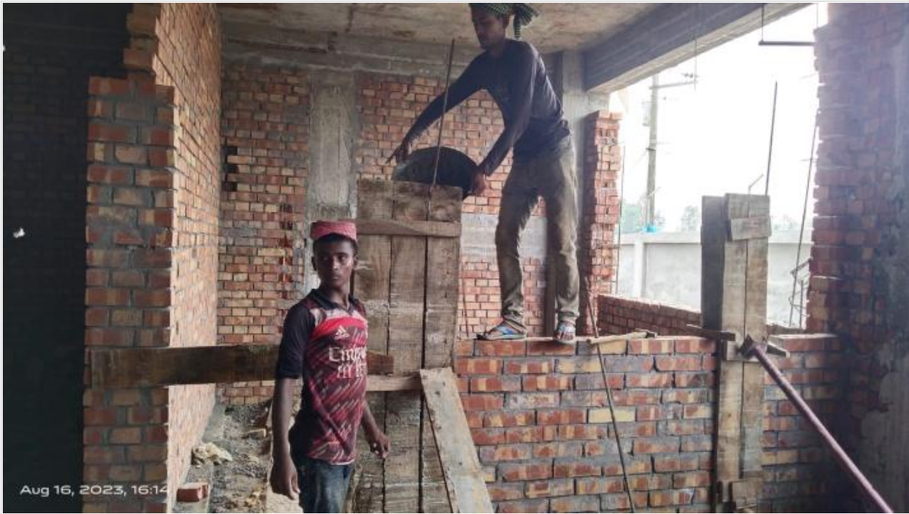
Comp-GF Column Concreting on 16-08-23
