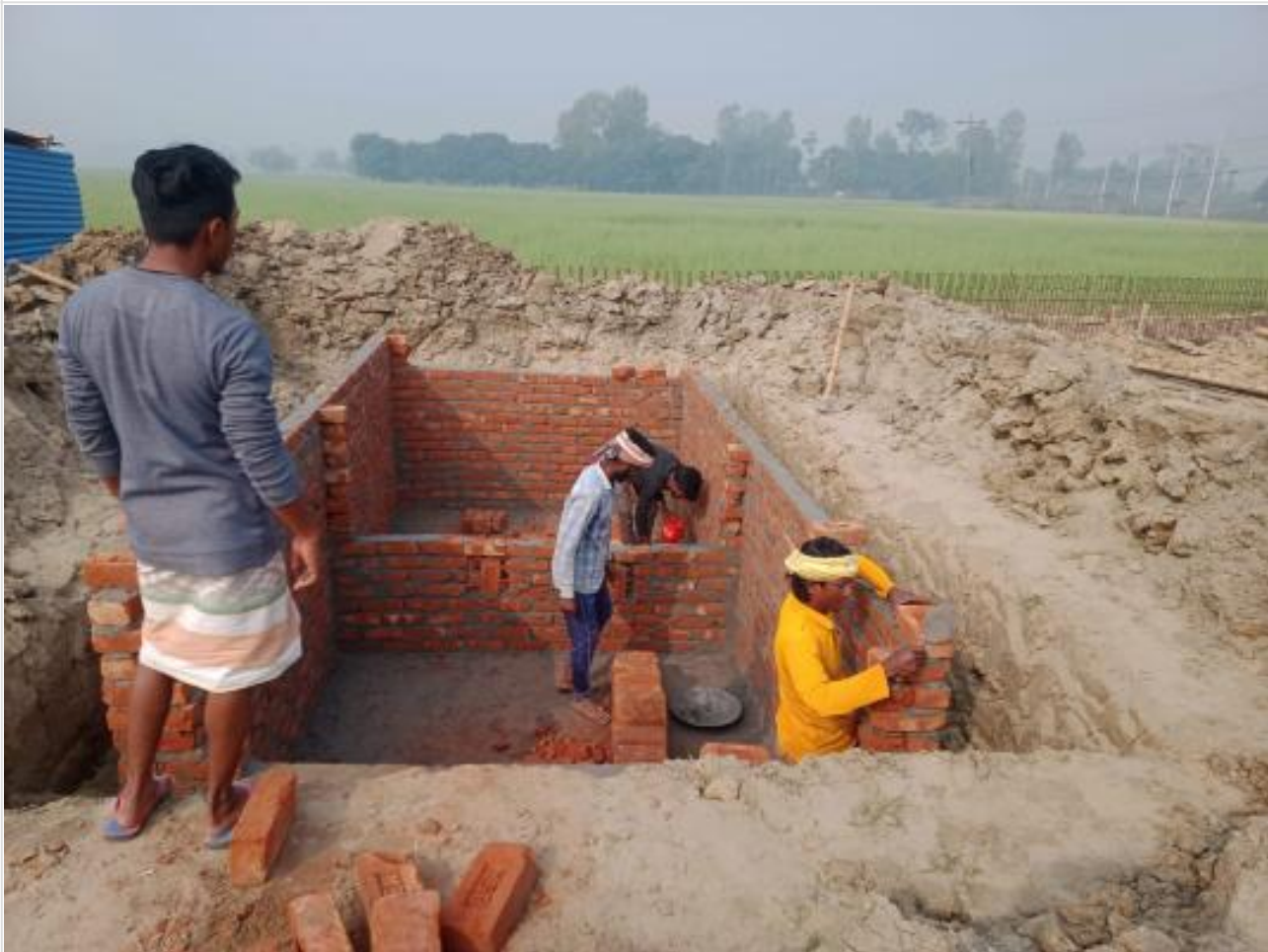
Mud Tank making on 06-02-23
