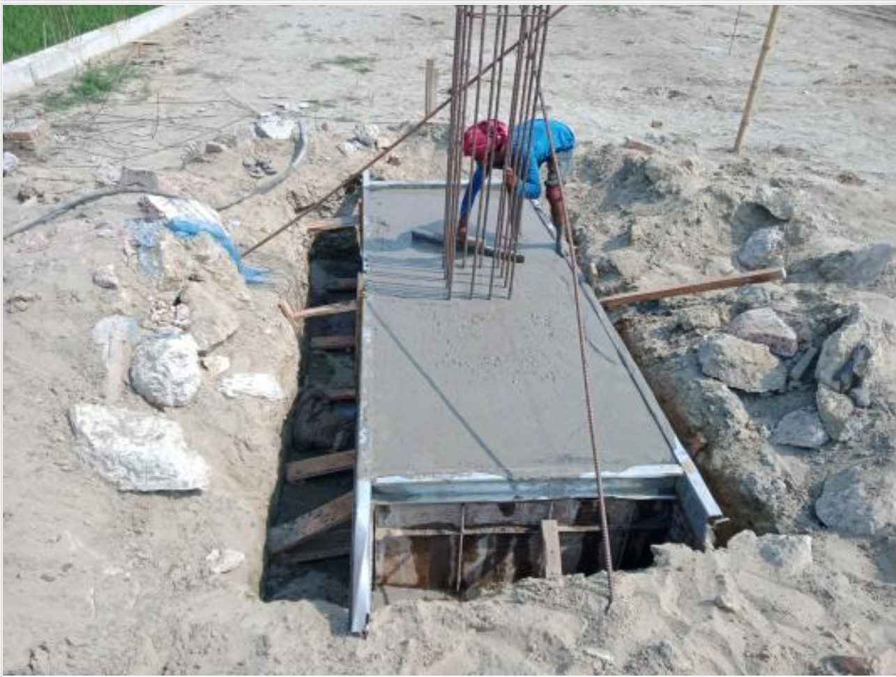
Pile cap casting on 17-04-23
