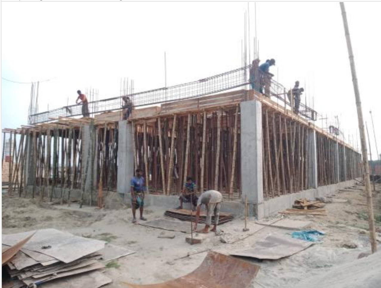
Comp. Bldg. Rebar work on 11-06-23
