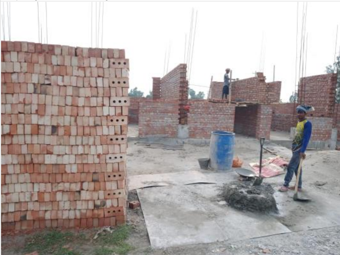
Gate house work on 15-06-23
