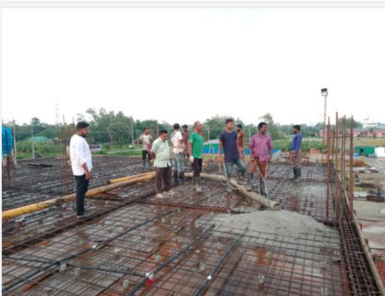
Tie column work at brick wall on 02-08-23
