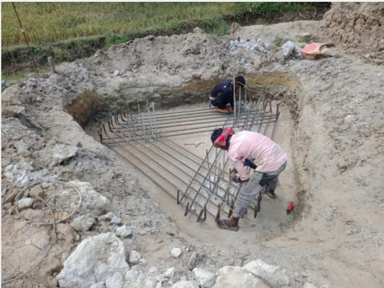
Dorm Bldg pile cap rebar binding on 23-05-23
