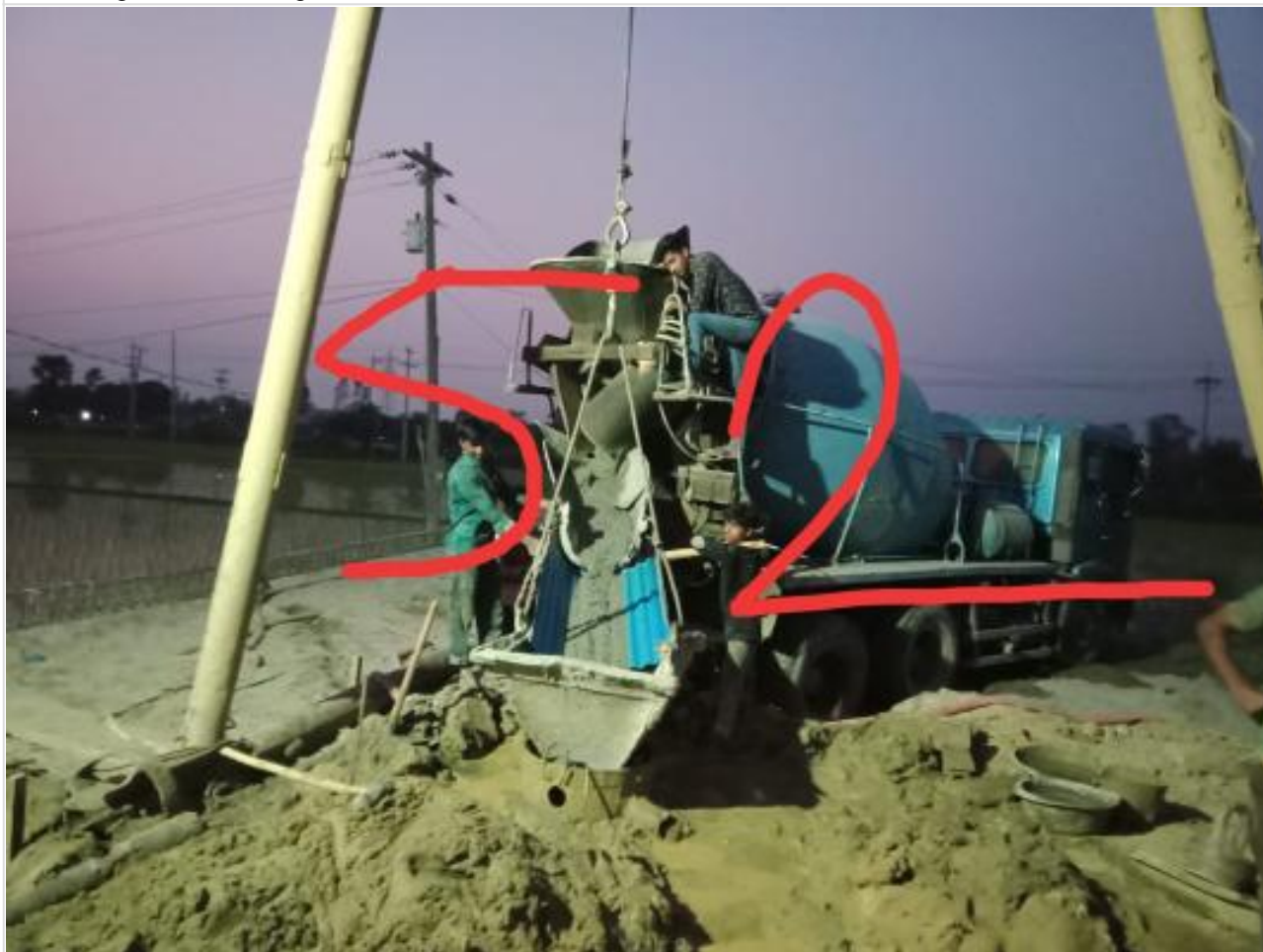
Ready mix concreting of pile on 10-03-23
