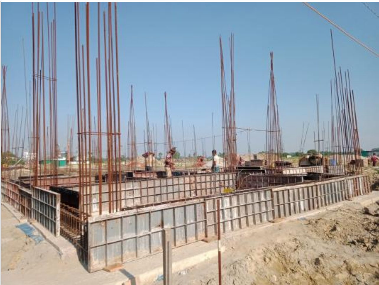
Comp. GB Shuttering on 06-05-23
