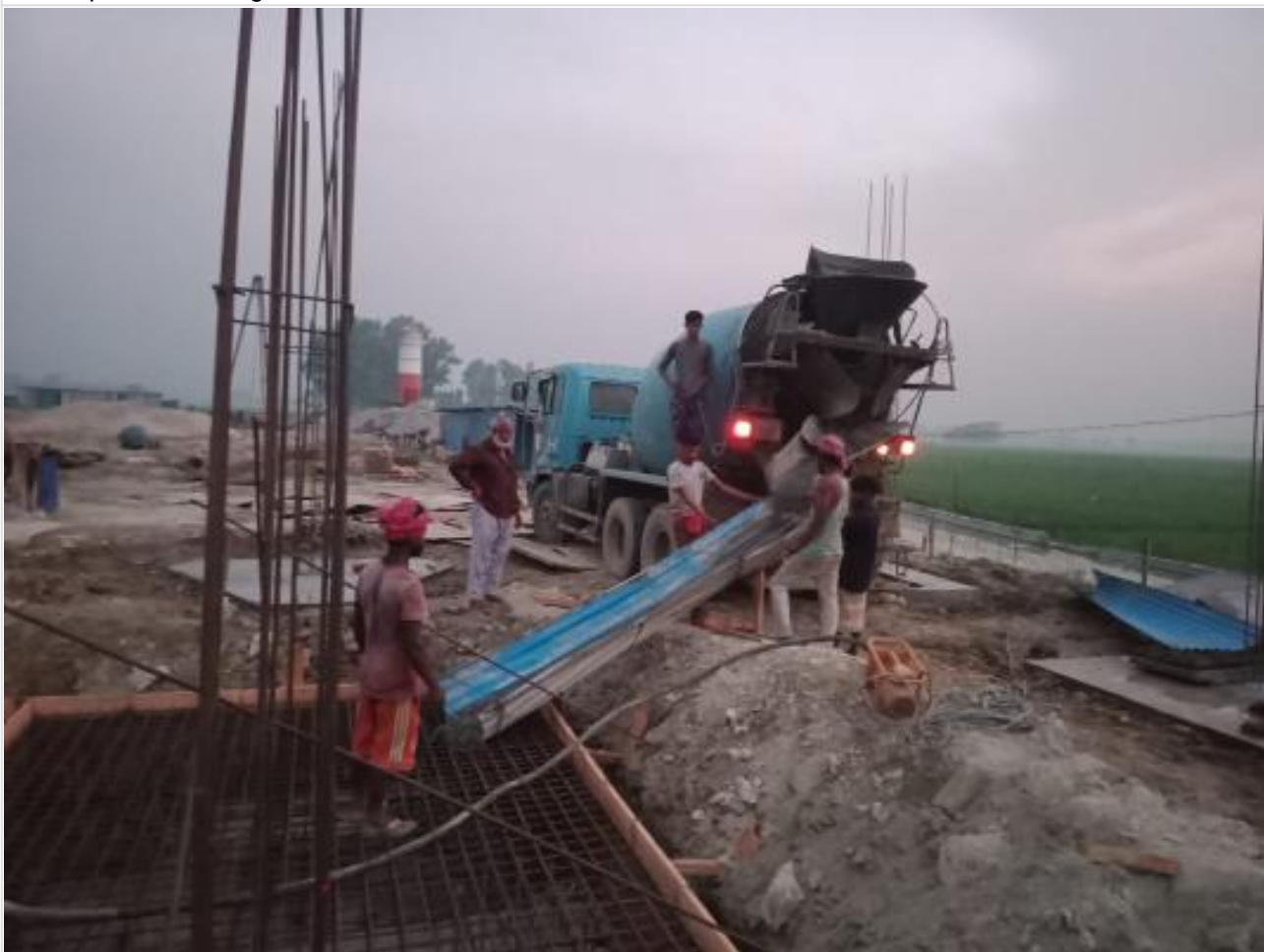
Pile Cap concreting. on 15-04-23
