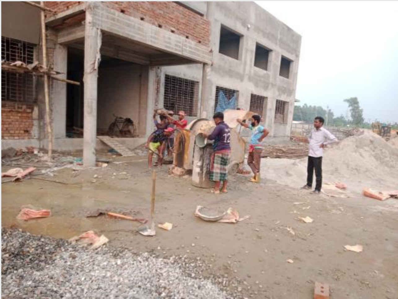
Comp. Bldg. GF casting on 16-10-23
