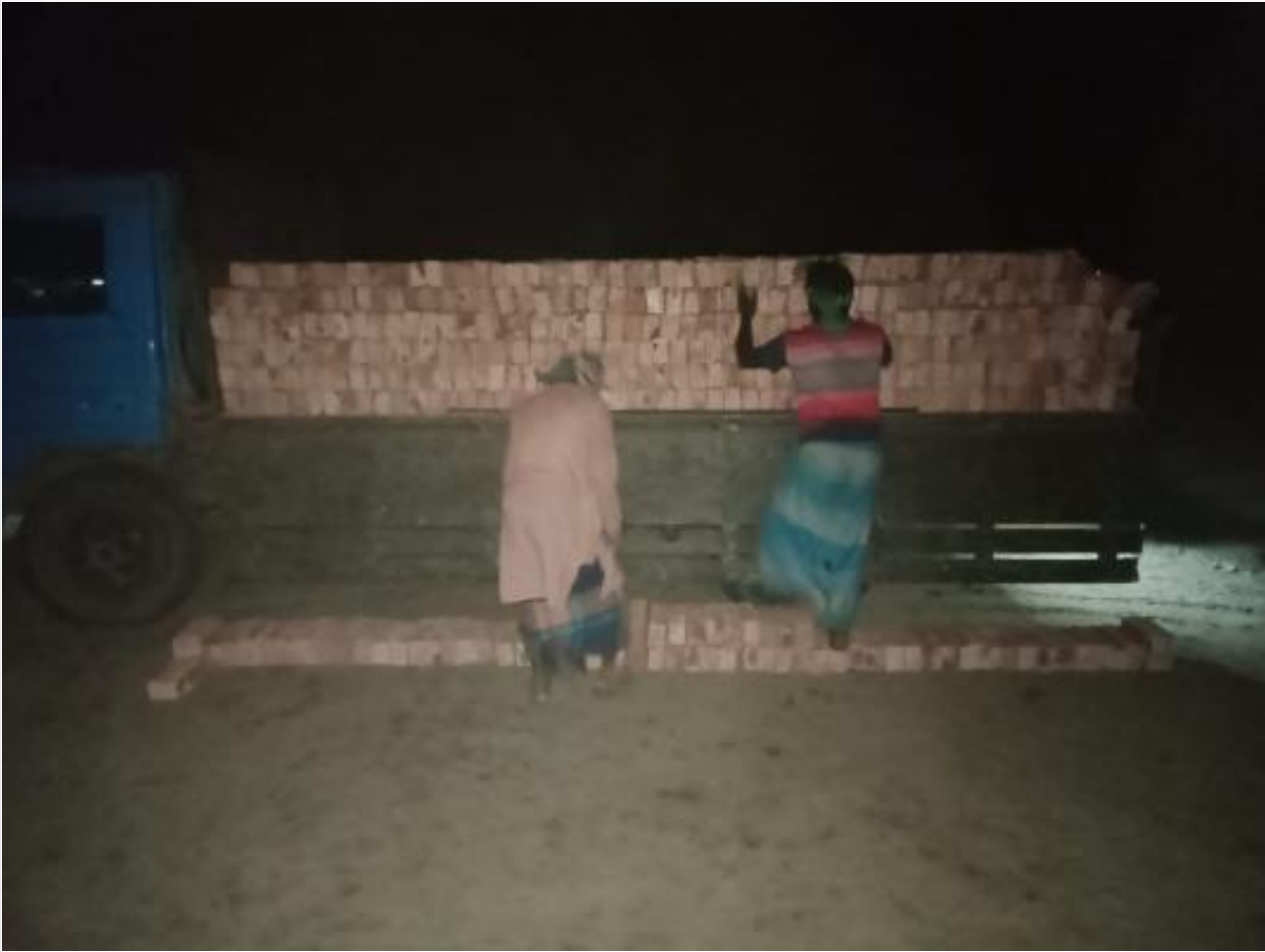
Brick un-loading on 09-01-23
