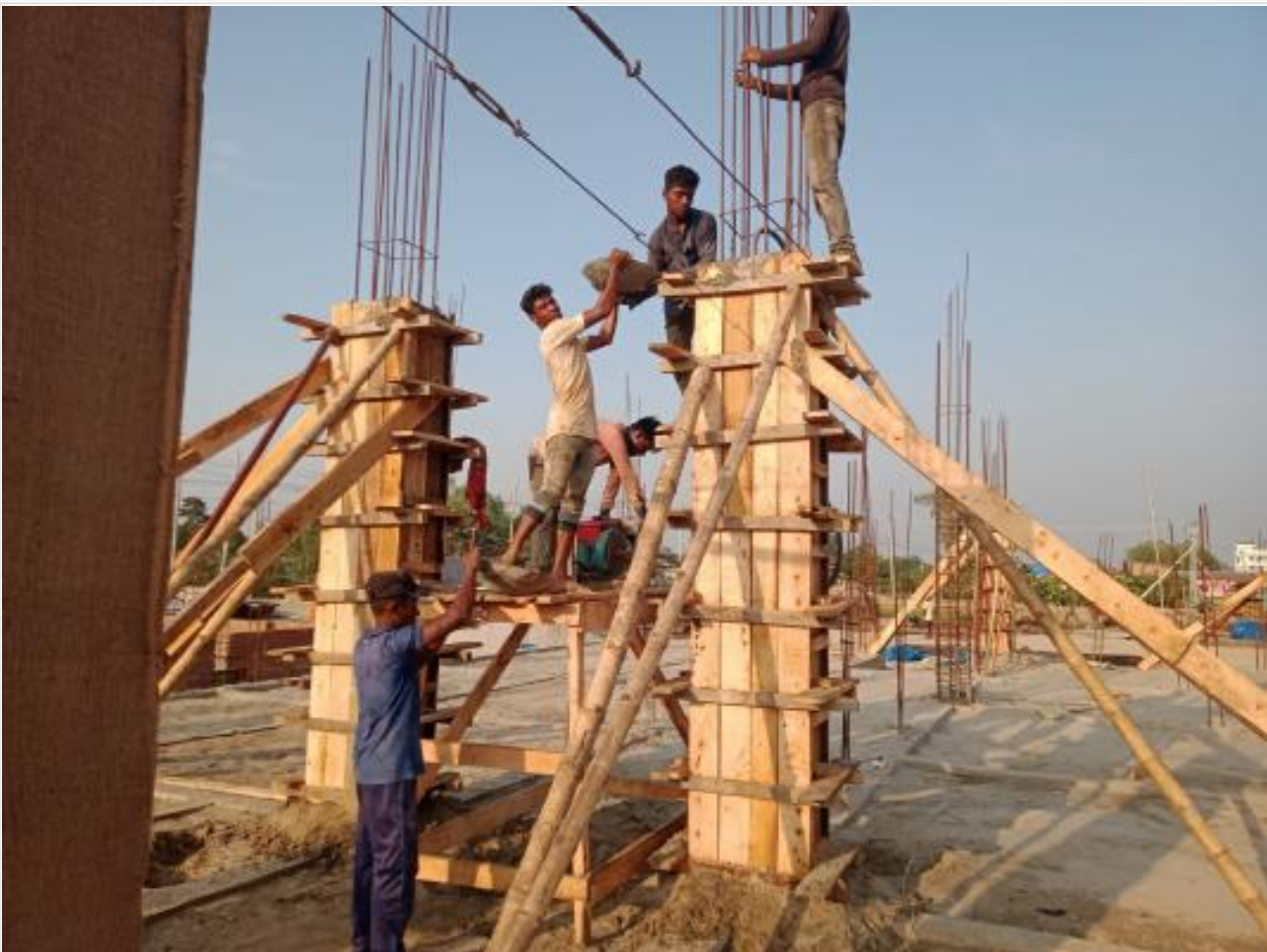
Comp. Bldg. Column casting on 30-05-23
