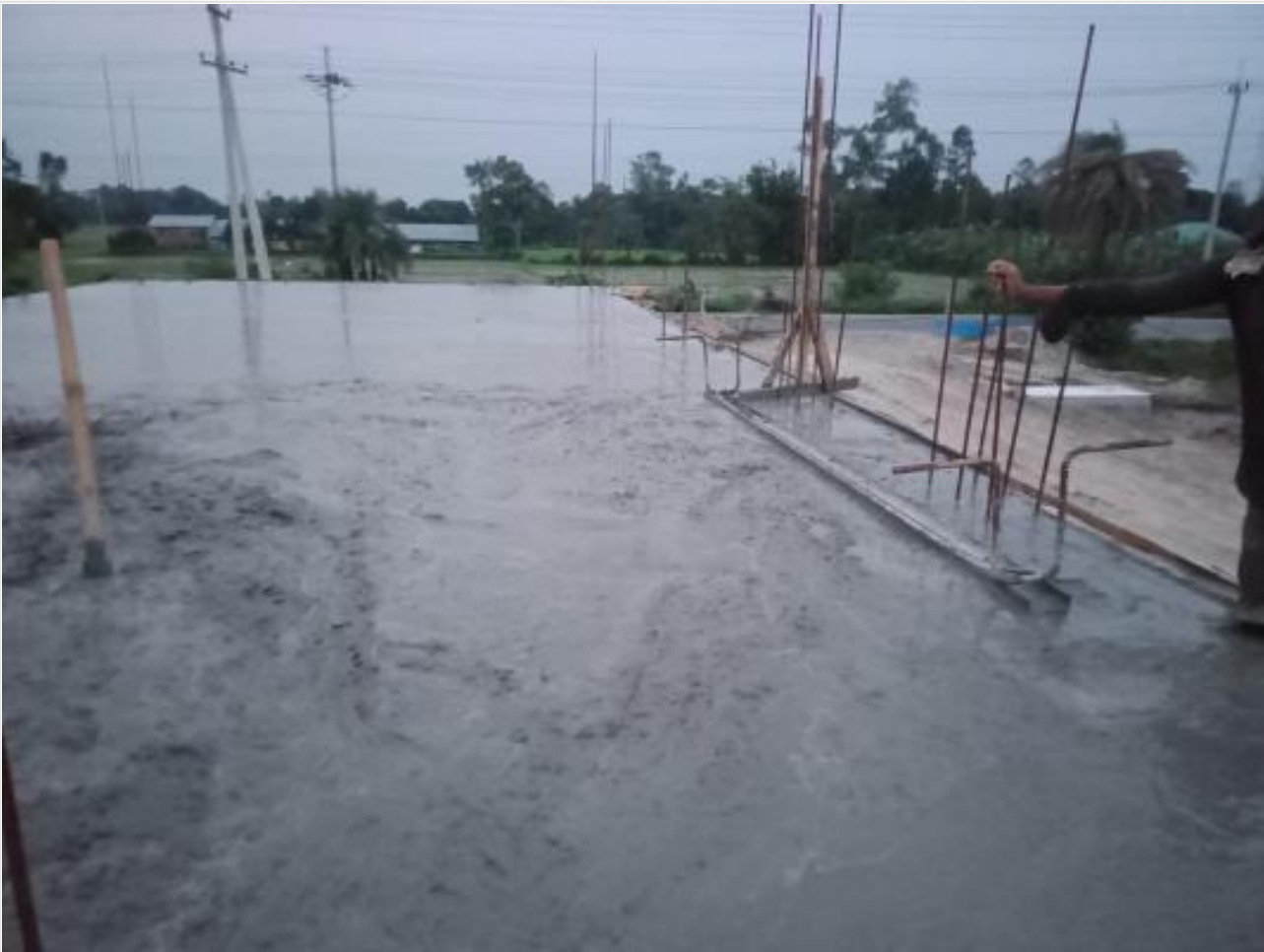
Gate House Slab Casting complete on 11-07-23
