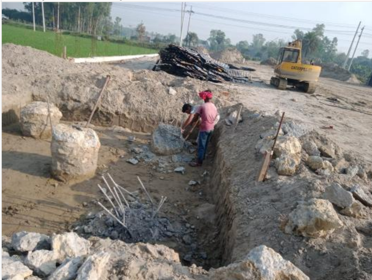
Pile head breaking on 28-03-23
