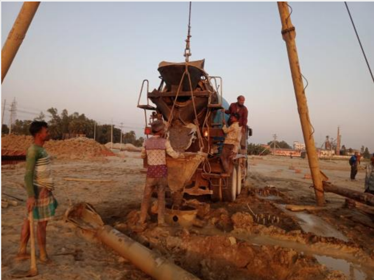
Ready mix concreting of pile on 13-02-23
