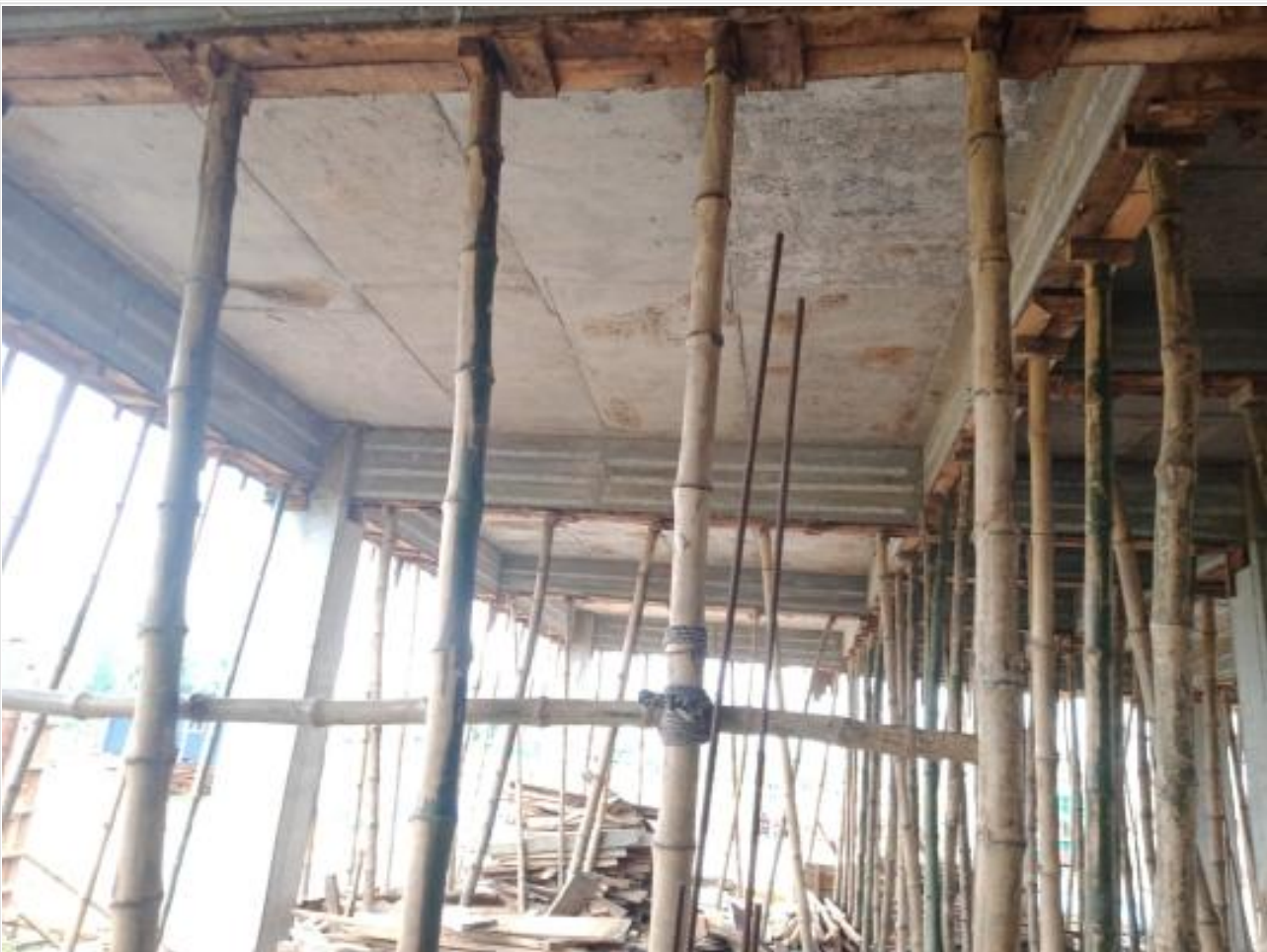
Comp. Bldg. Slab shutter opening on 12-07-23
