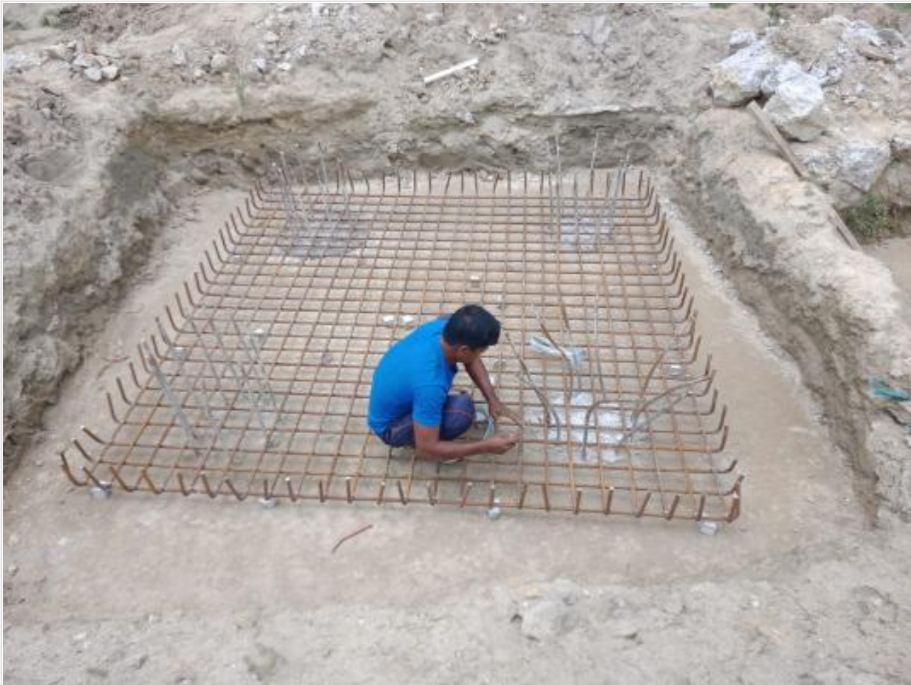
Dorm. Bldg. Pile cap rebar binding on 22-05-23
