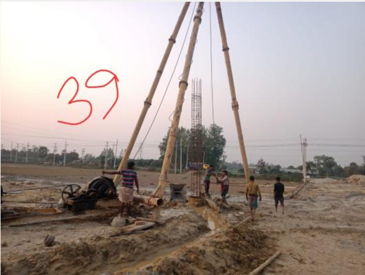
Com. Bldg. 39 pile boring on 02-03-23
