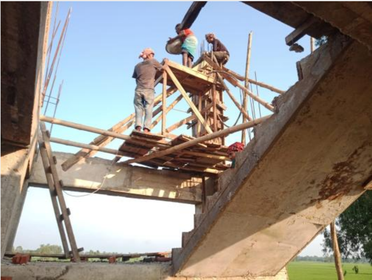
Dorm. Bldg. Roof top column casting on 08-10-23
