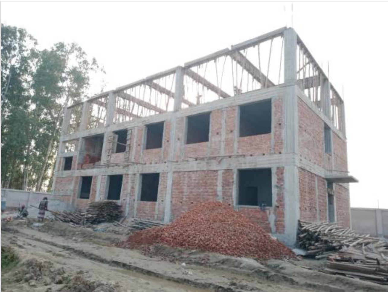
Dorm. Bldg. 2nd floor shuttering work on 06-11-23
