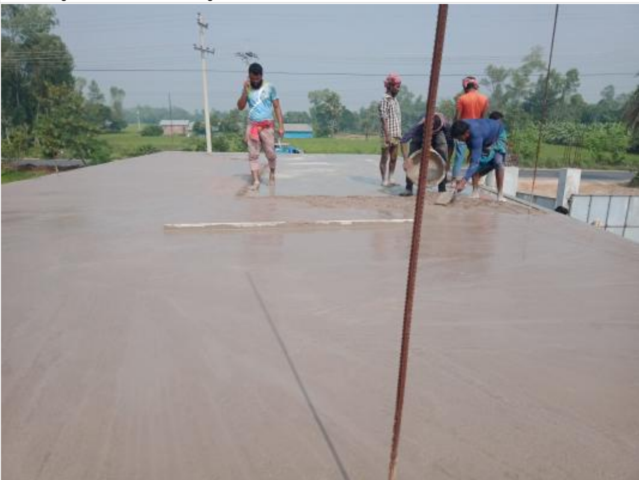
Gate roof top water proofing casting on 08-11-23
