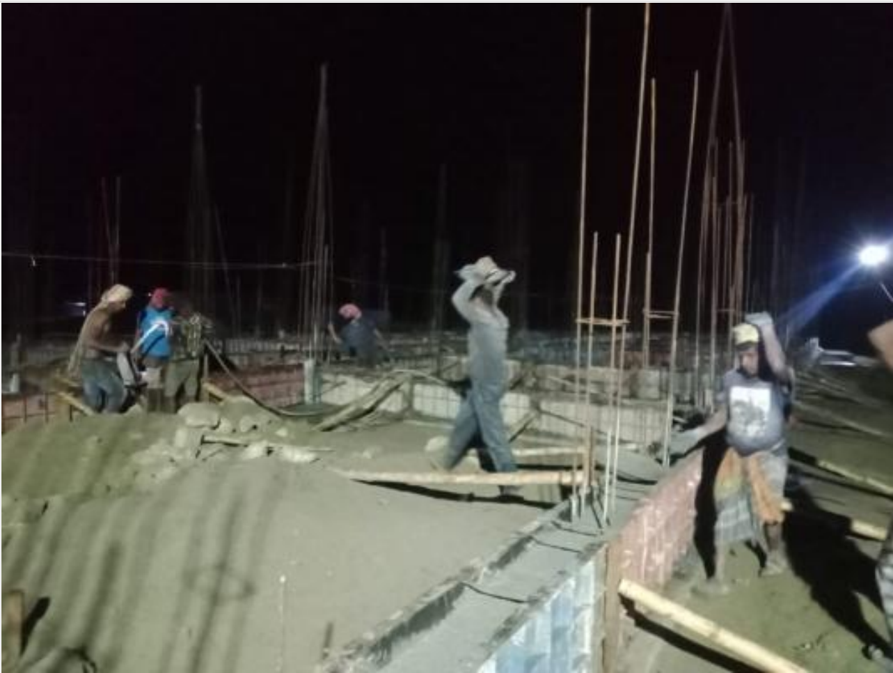
GB Concreting on 16-05-23
