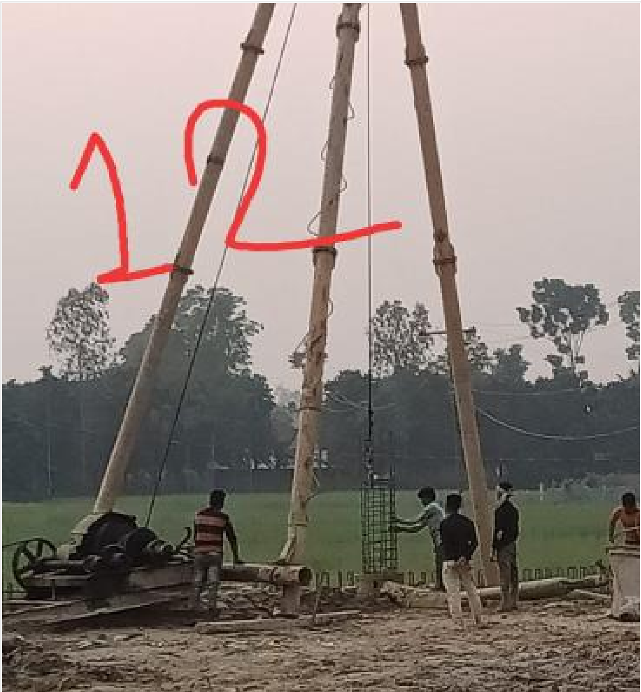
Com. Bldg. 12th pile boring on 17-02-23
