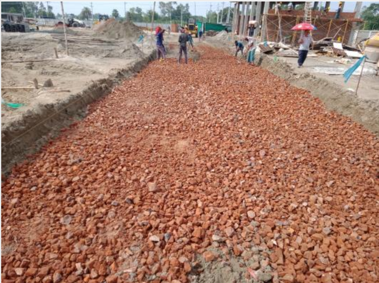
Road-Sub-base work on 21-08-23
