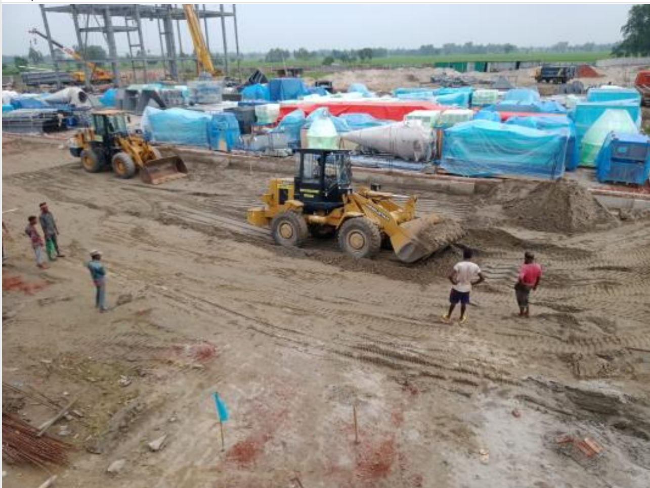
Road-Box cutting on 22-08-23
