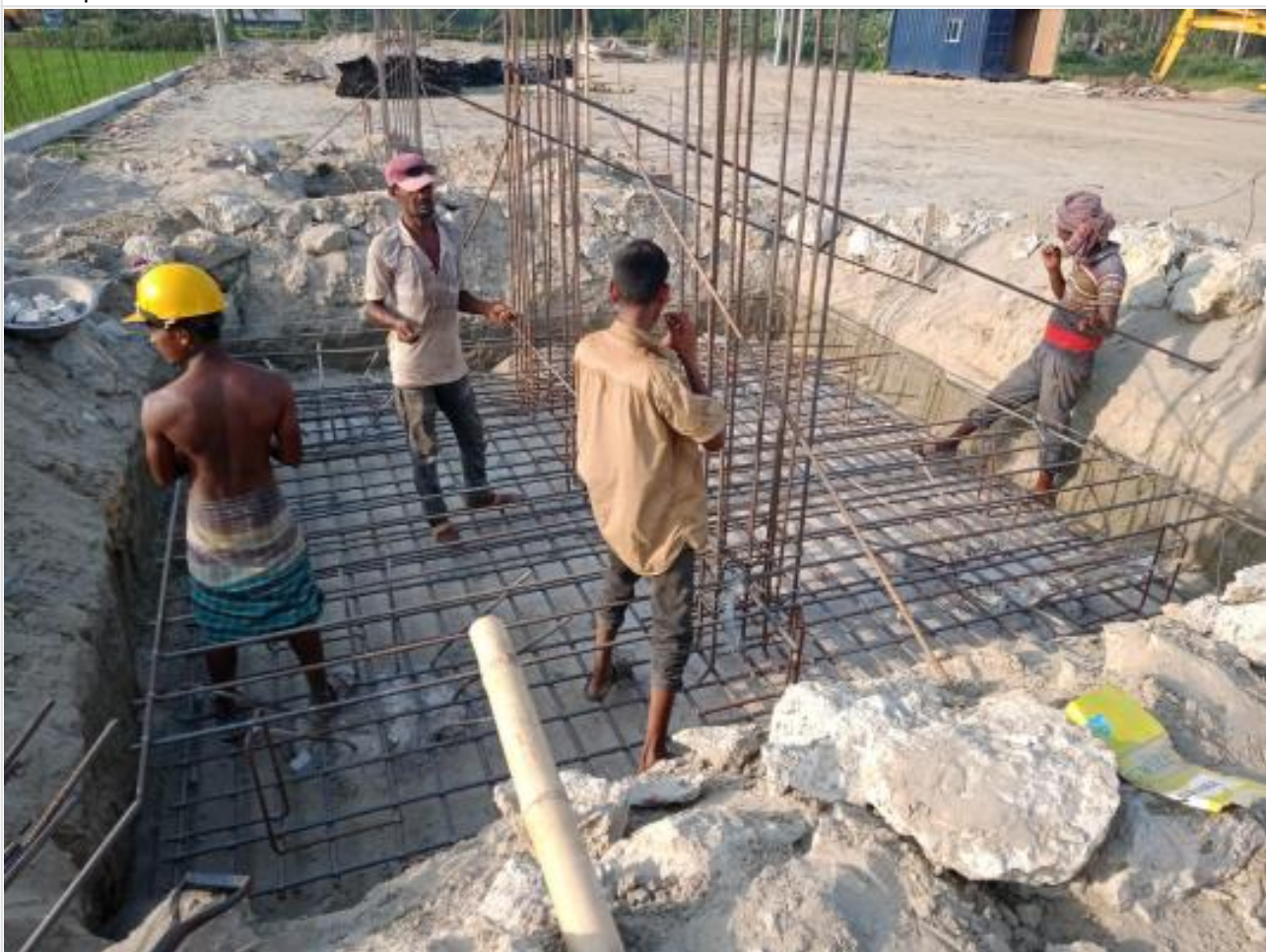
Pile cap rebar work on 14-04-23
