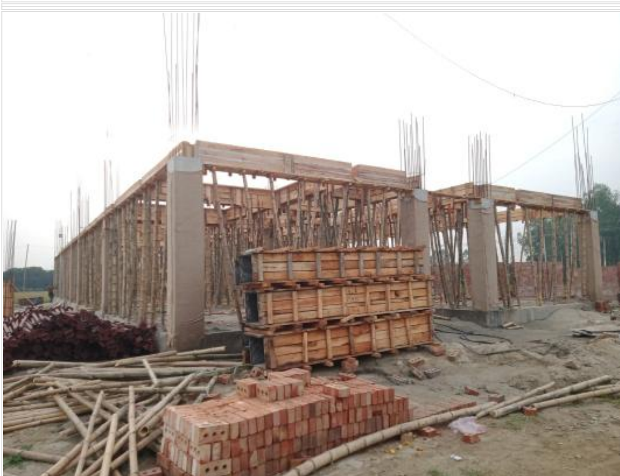
Comp. Bldg. Slab beam shuttering on 07-06-23
