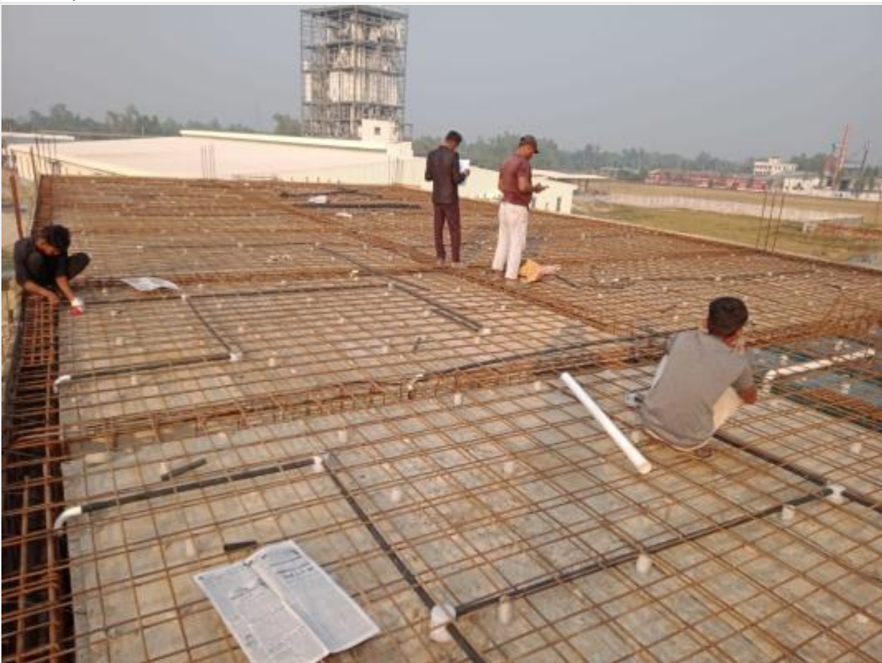
Dormitory-3rd Floor Slab Electrical Pipe on 18-12-23
