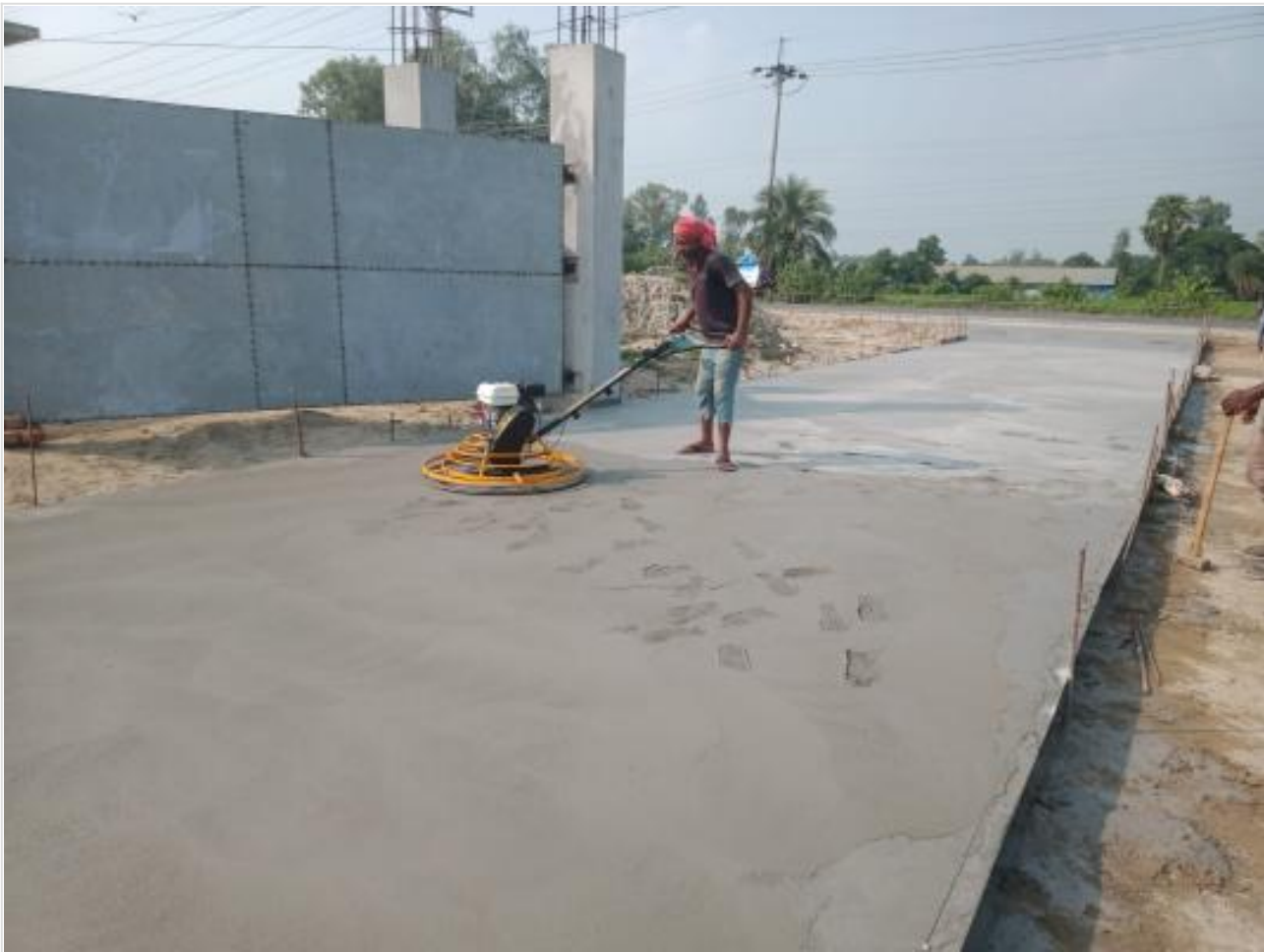
Road casting work on 18-10-23
