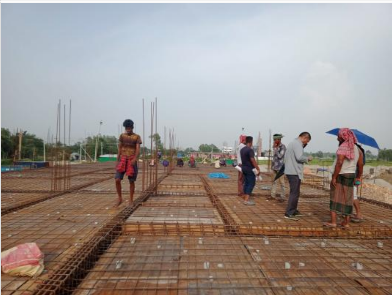
Comp. Bldg. Slab beam shuttering and Reb on 16-06-23
