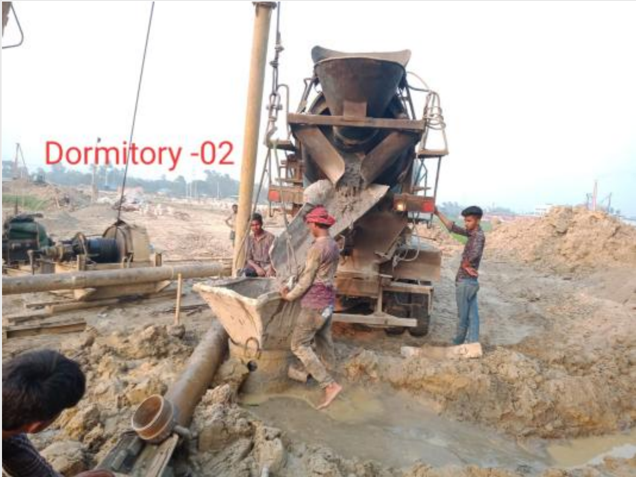
Ready mix concreting of pile on 25-03-23
