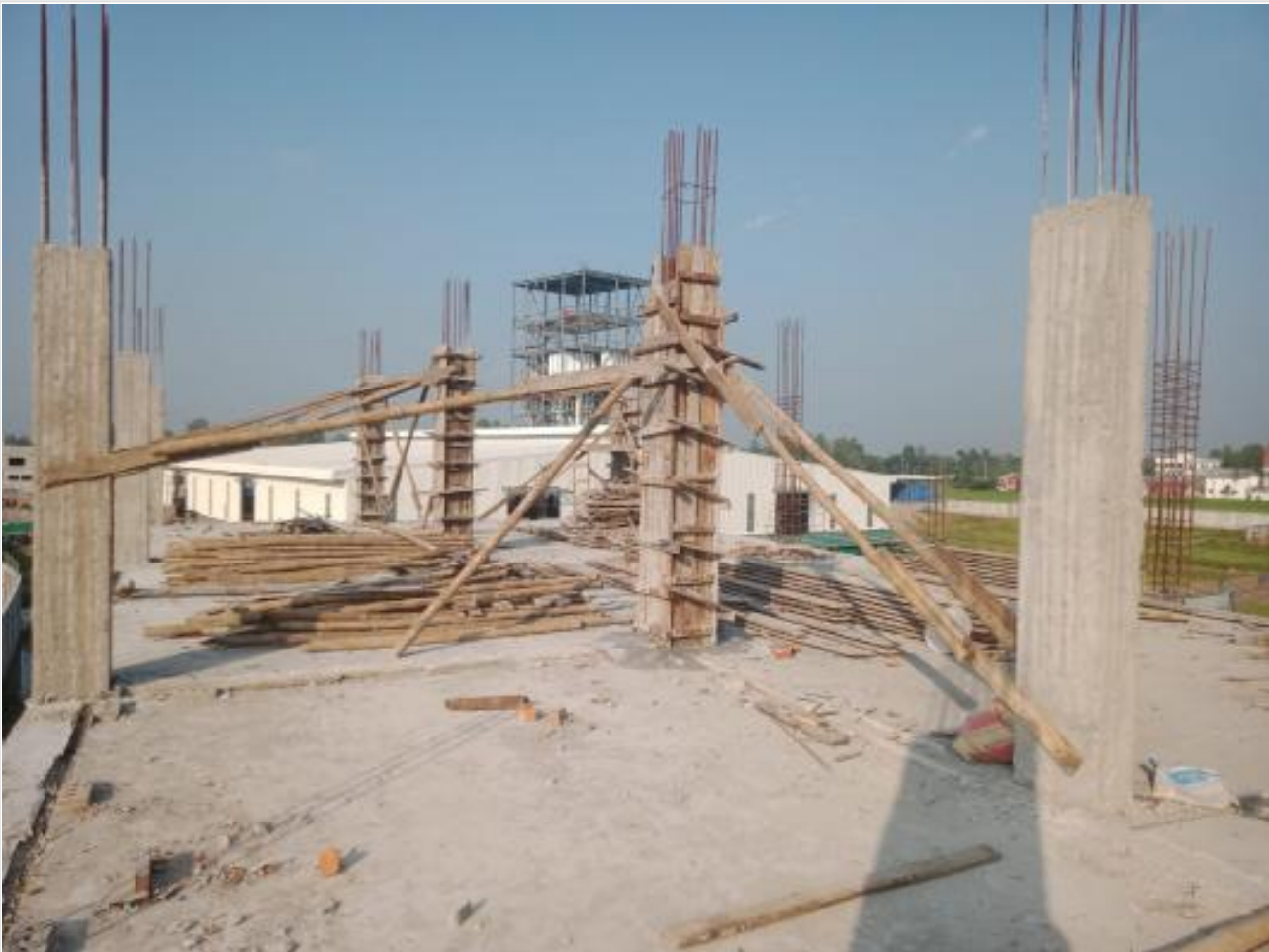
Dorm. Bldg. 2nd floor concreting work on 02-11-23
