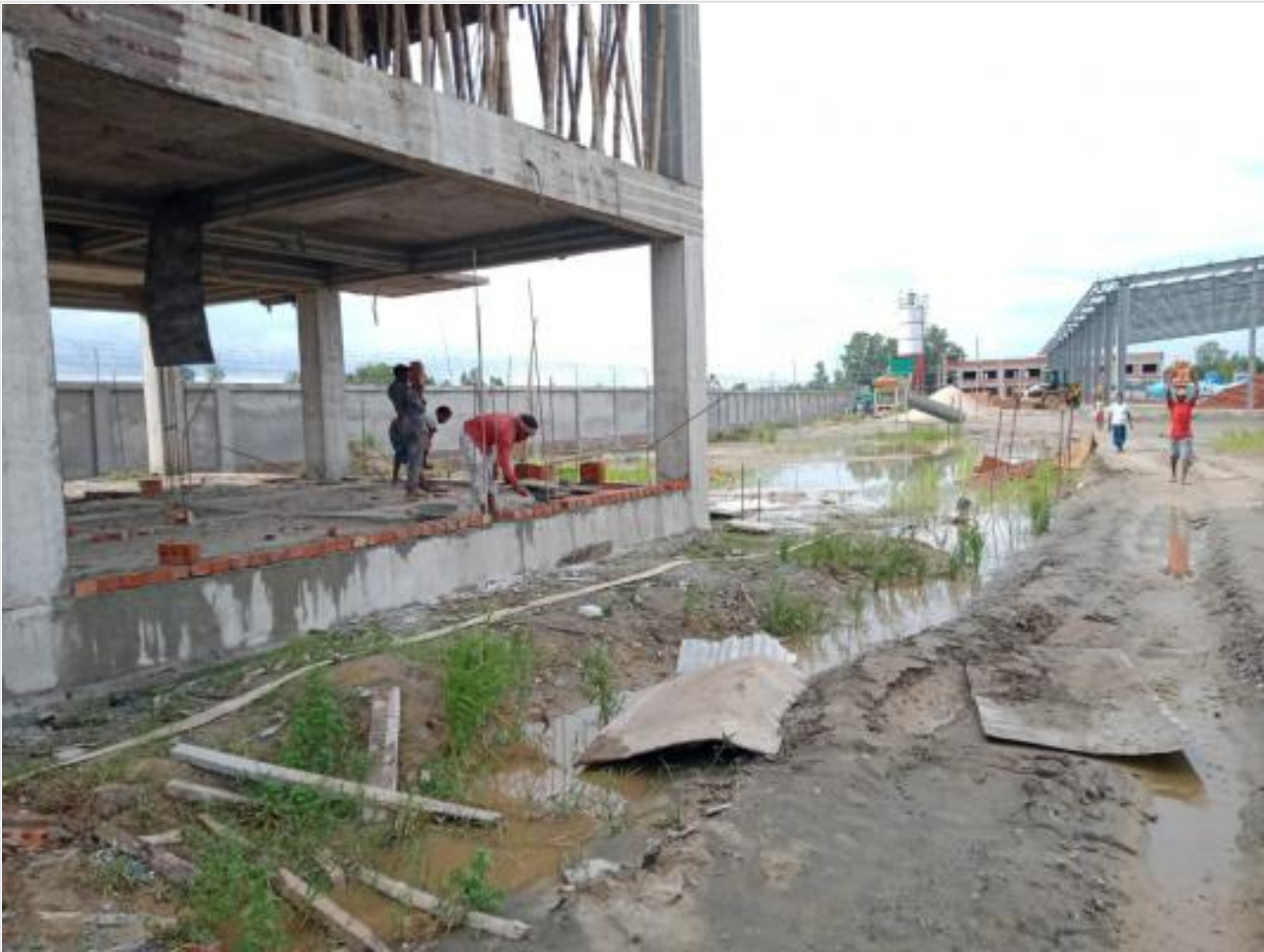
Dormitory GF-Brick Work on 20-09-23
