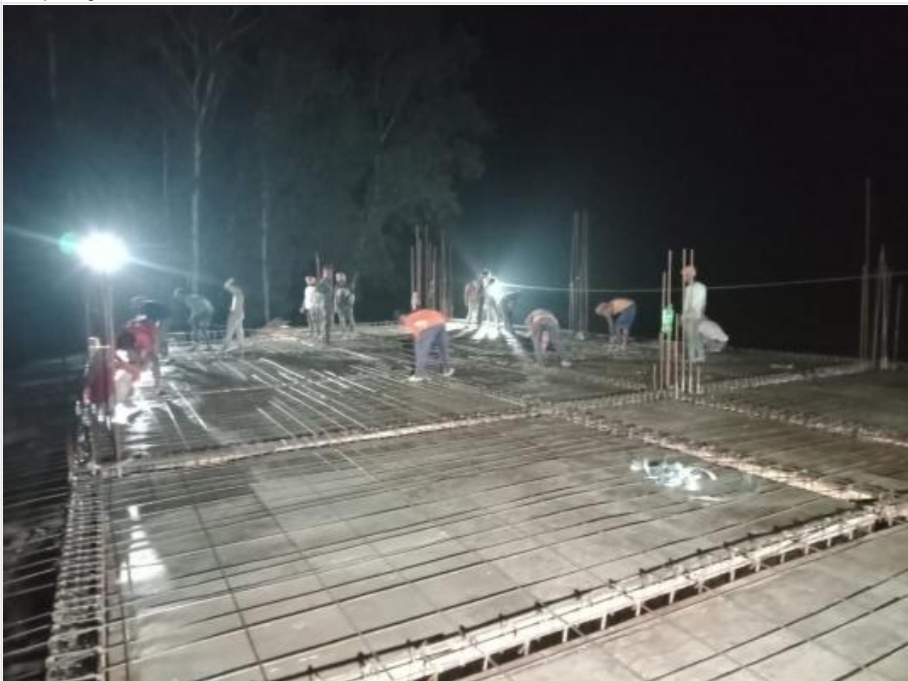
Dormitory 1st Floor Re-bar work on 06-08-23
