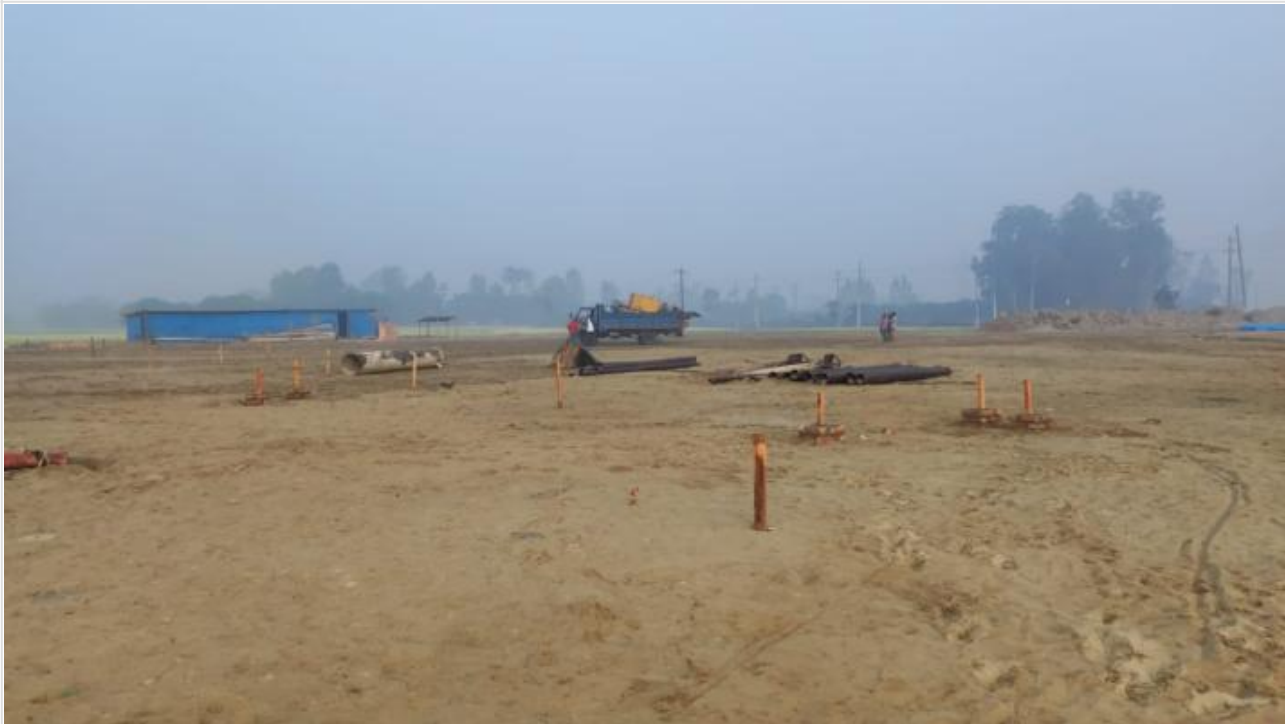
Piling Rig Mobilized on 29-01-23
