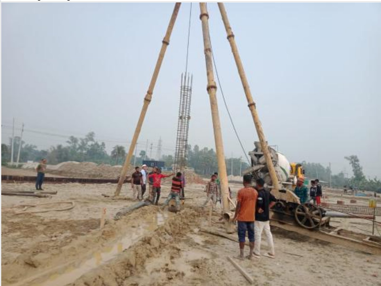
Pile Concreting on 09-02-23
