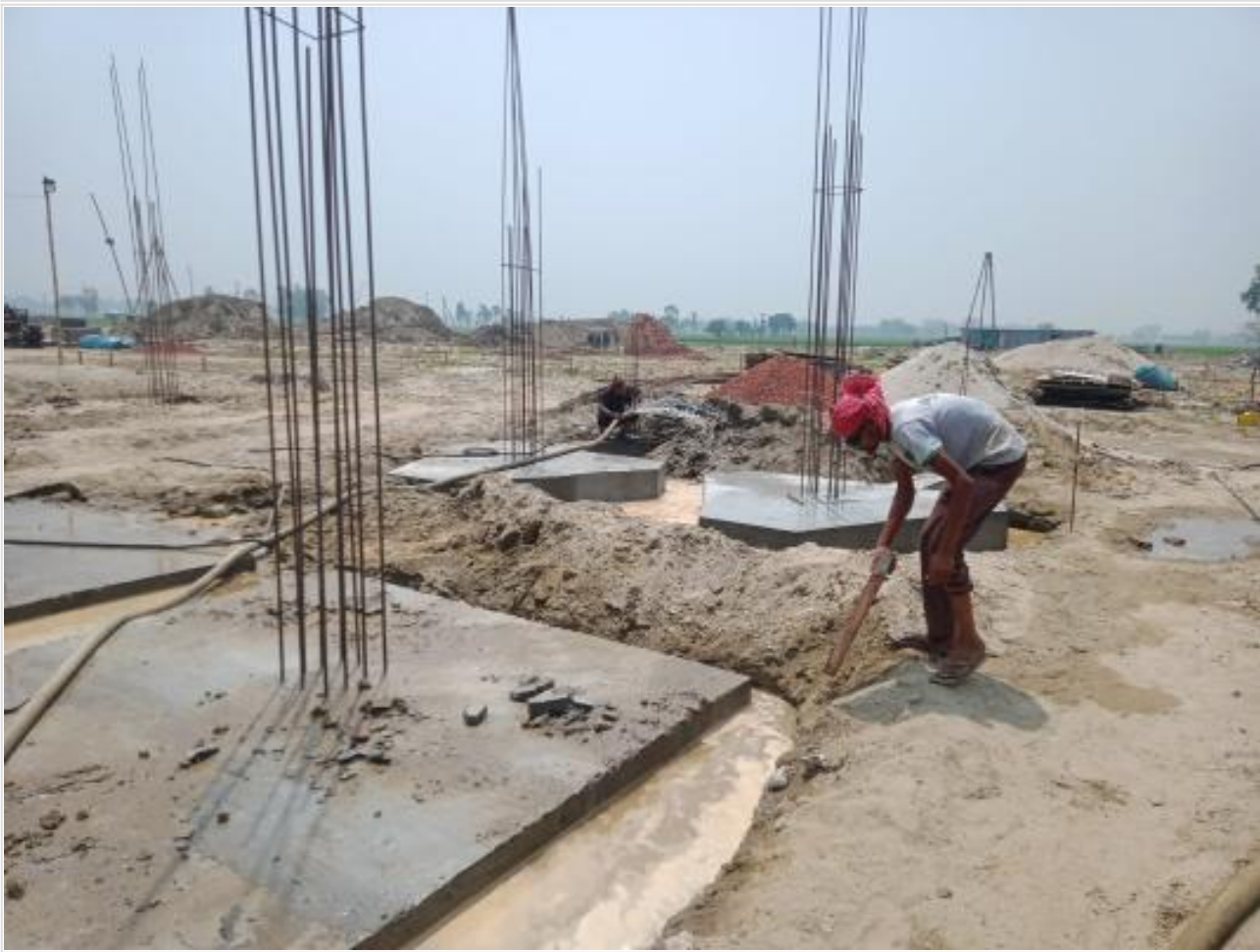
Comp. Bldg. Back filling on 19-04-23
