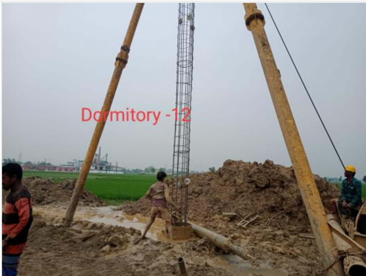
Dorm. Bldg. 10th pile concreting on 30-03-23
