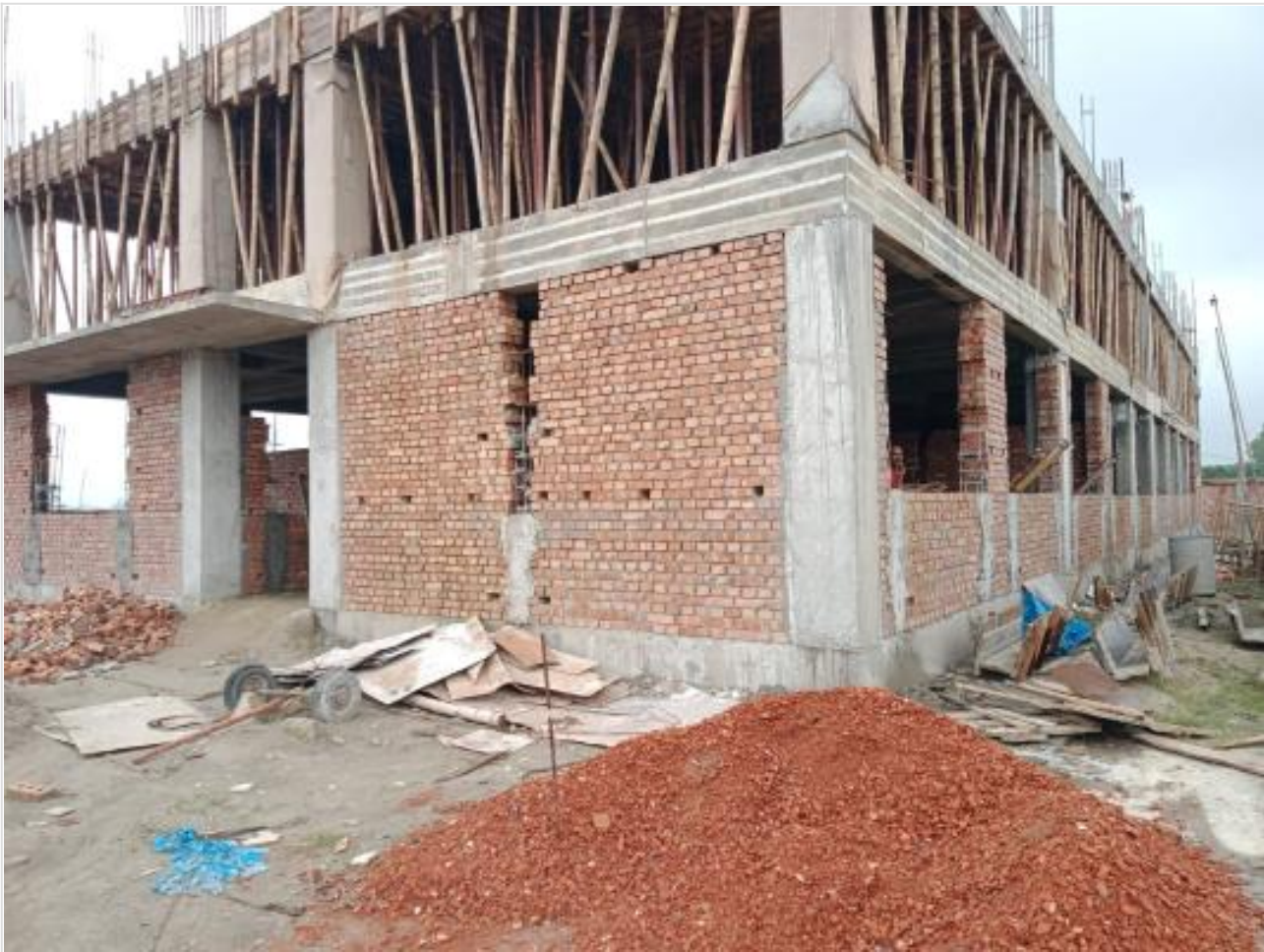
Comp.Bldg GF Brick work on 06-08-23
