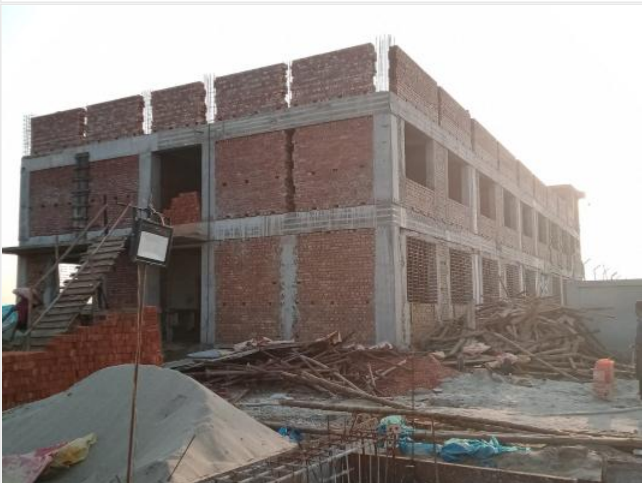
Comp. Bldg work on 15-09-23
