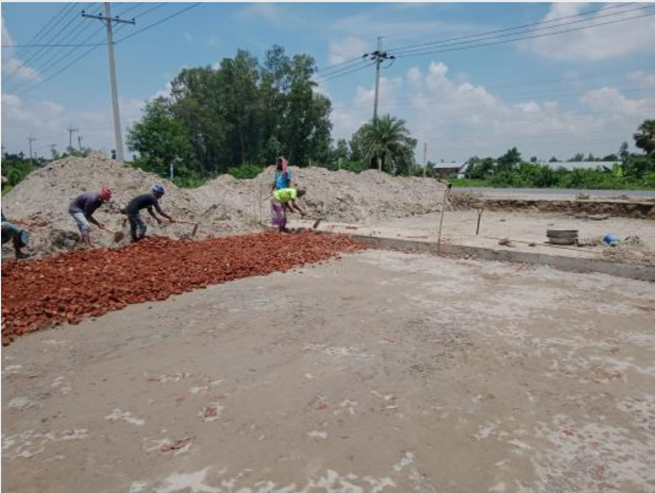
Road work on 31-07-23
