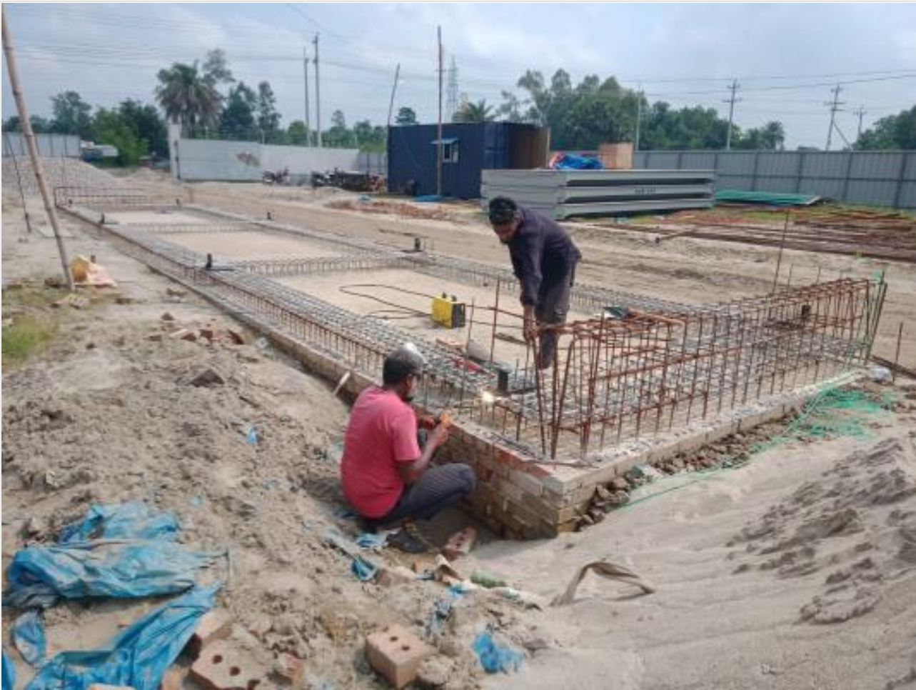
Anchor bolt fitting at scale on 06-09-23
