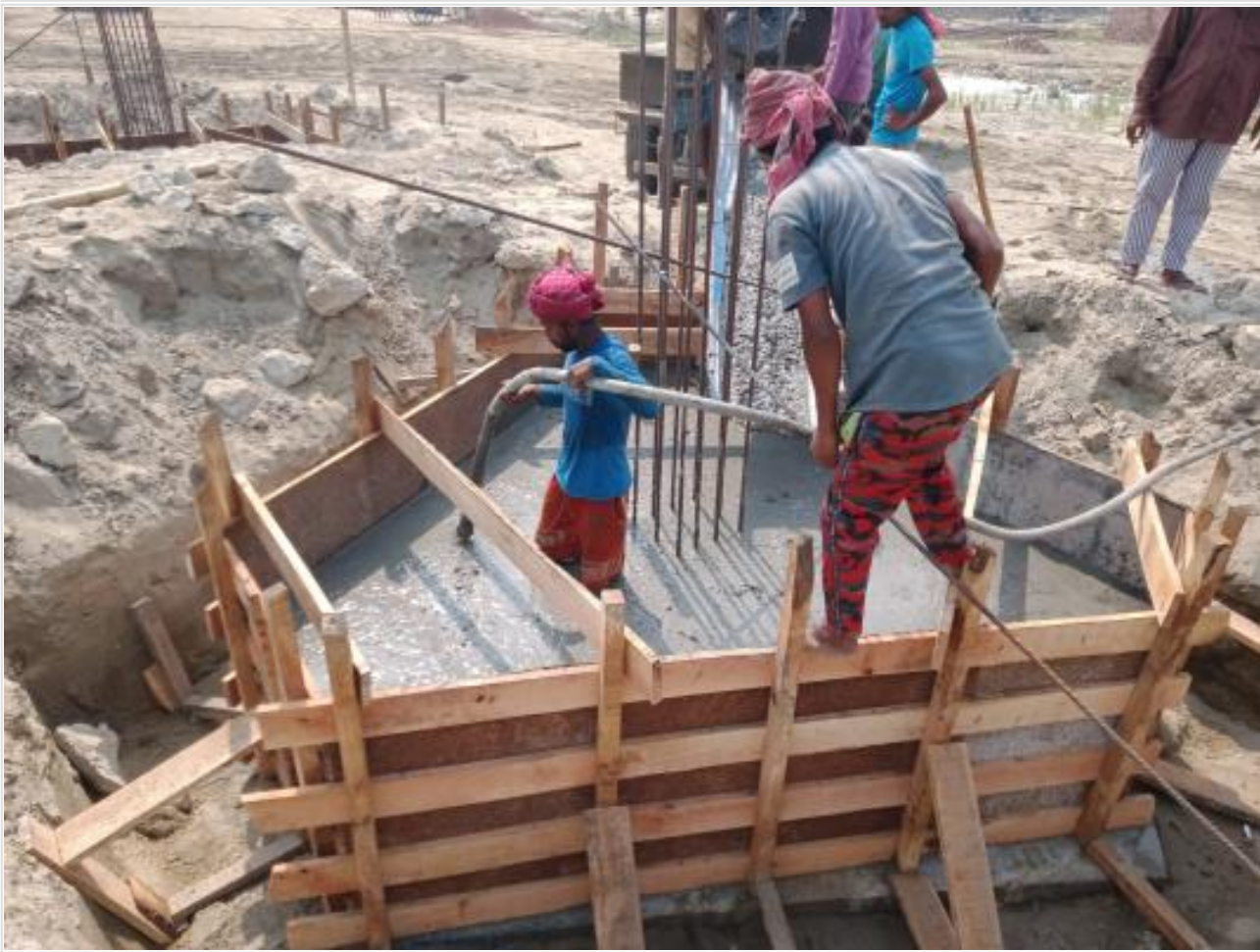
Comp. Bldg. Pile cap casting on 16-04-23
