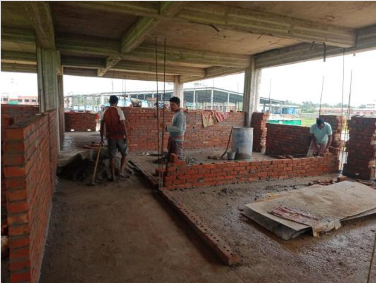
Dorm. Bldg. 1st floor brick work on 06-10-23
