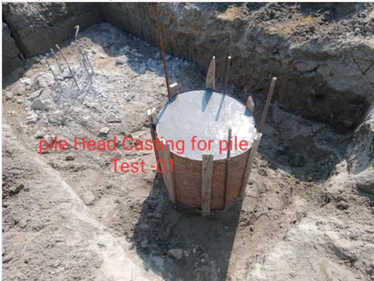
Pile head finishing for test on 03-04-23
