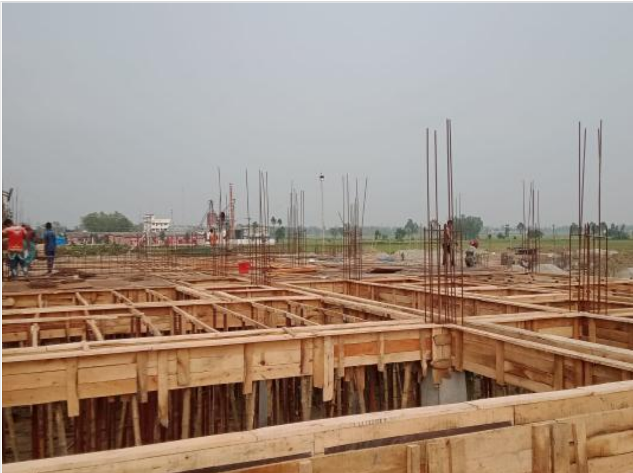
Comp. Bldg. Slab beam shuttering on 10-06-23
