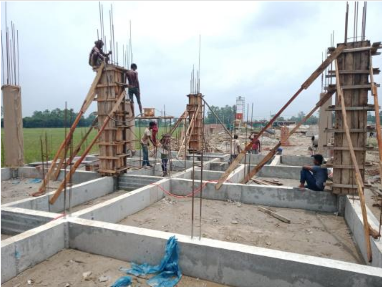
Dorm. Bldg. Column casting on 20-06-23
