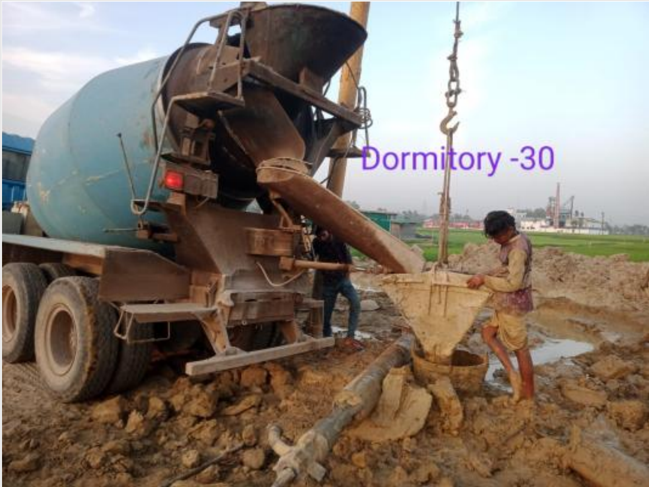
Ready mix concreting of pile on 08-04-23
