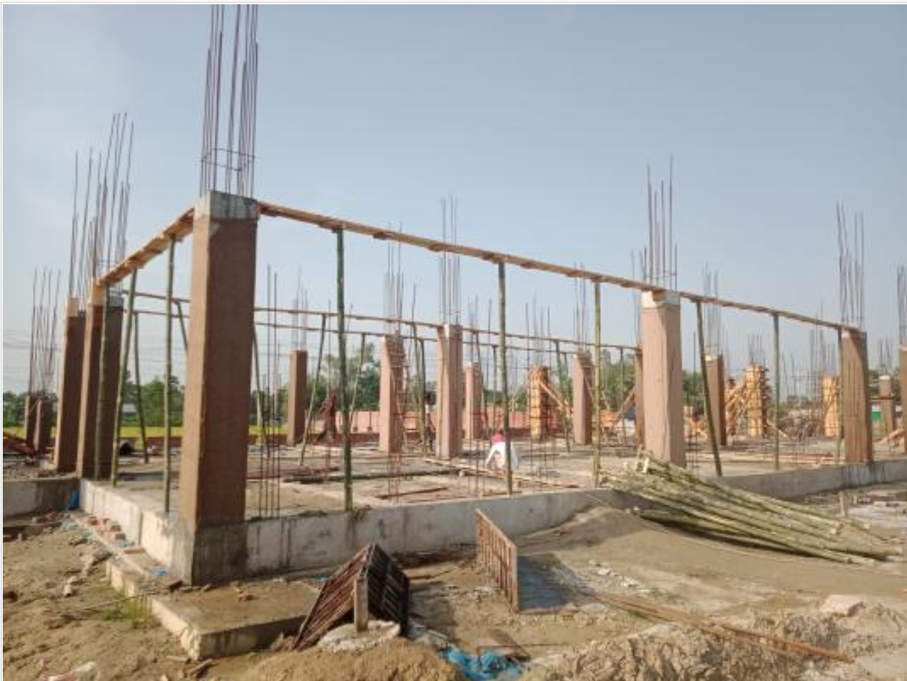
Comp. Bldg. Slab beam line shuttering on 01-06-23
