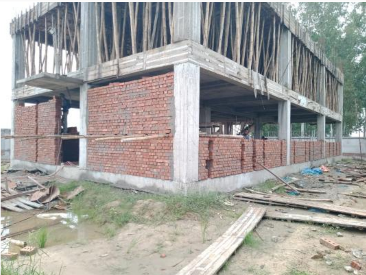
Dorm.Bldg. GF brick work on 23-09-23
