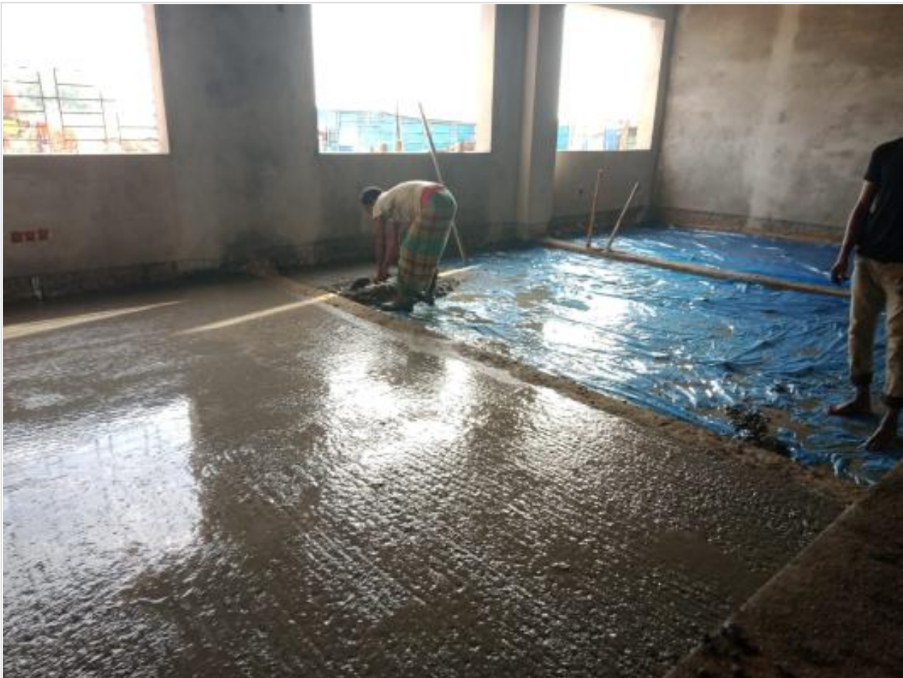
Comp. GF concreting on 29-09-23
