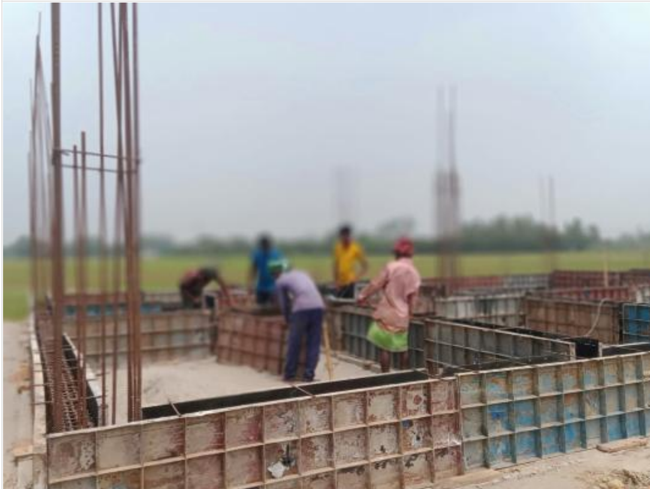
Dorm. Bldg. GB shuttering on 09-06-23
