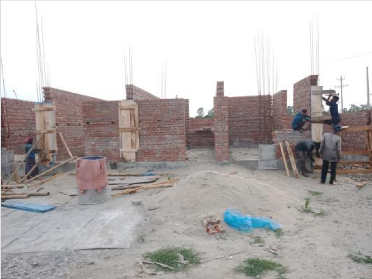
Gate house column shuttering work on 16-06-23
