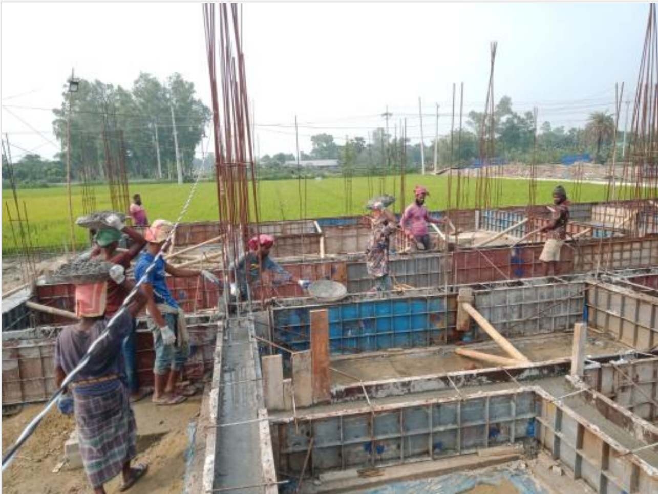
Comp. Bldg. GB casting work on 12-05-23
