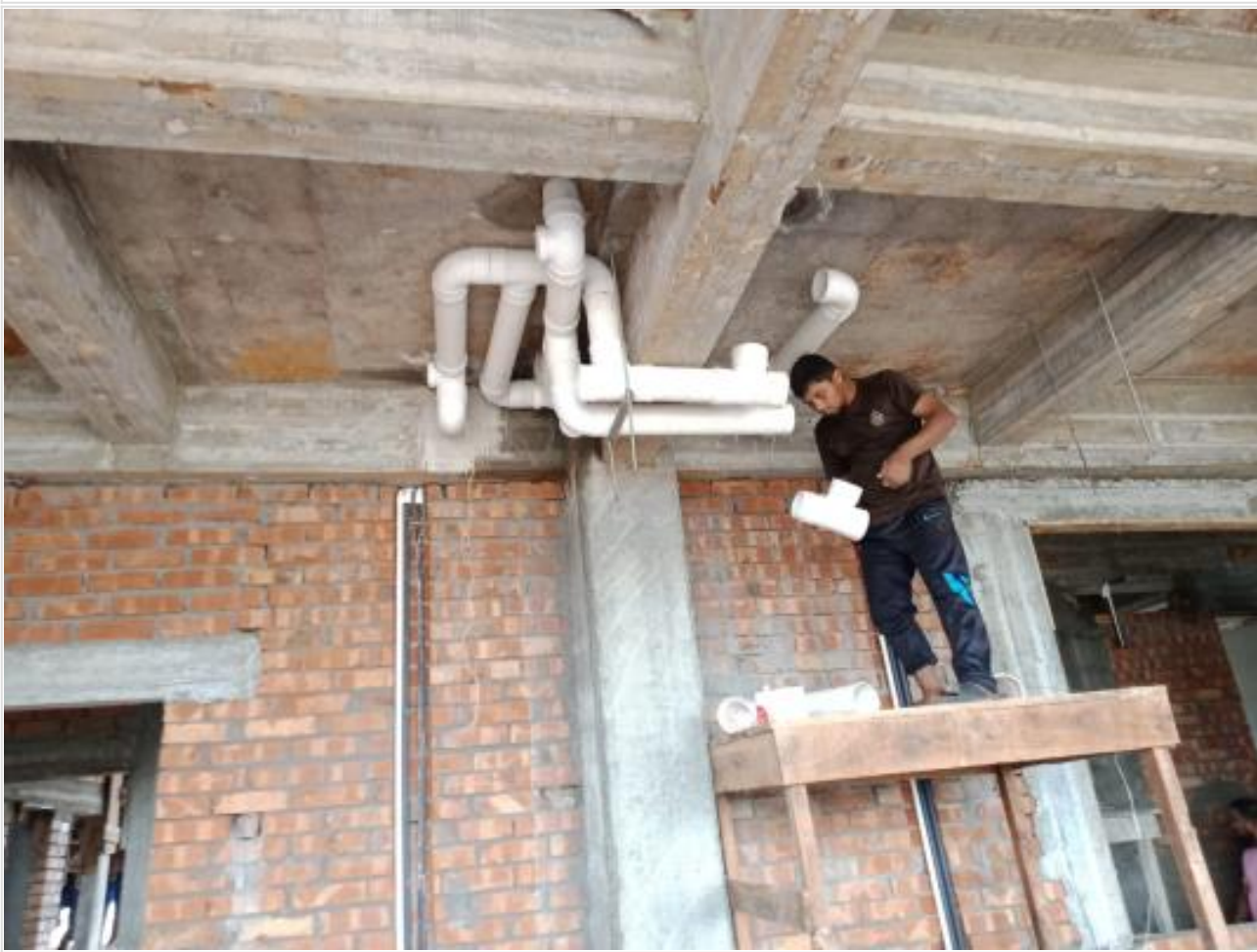
Comp. Bldg. Sanitary work on 29-08-23
