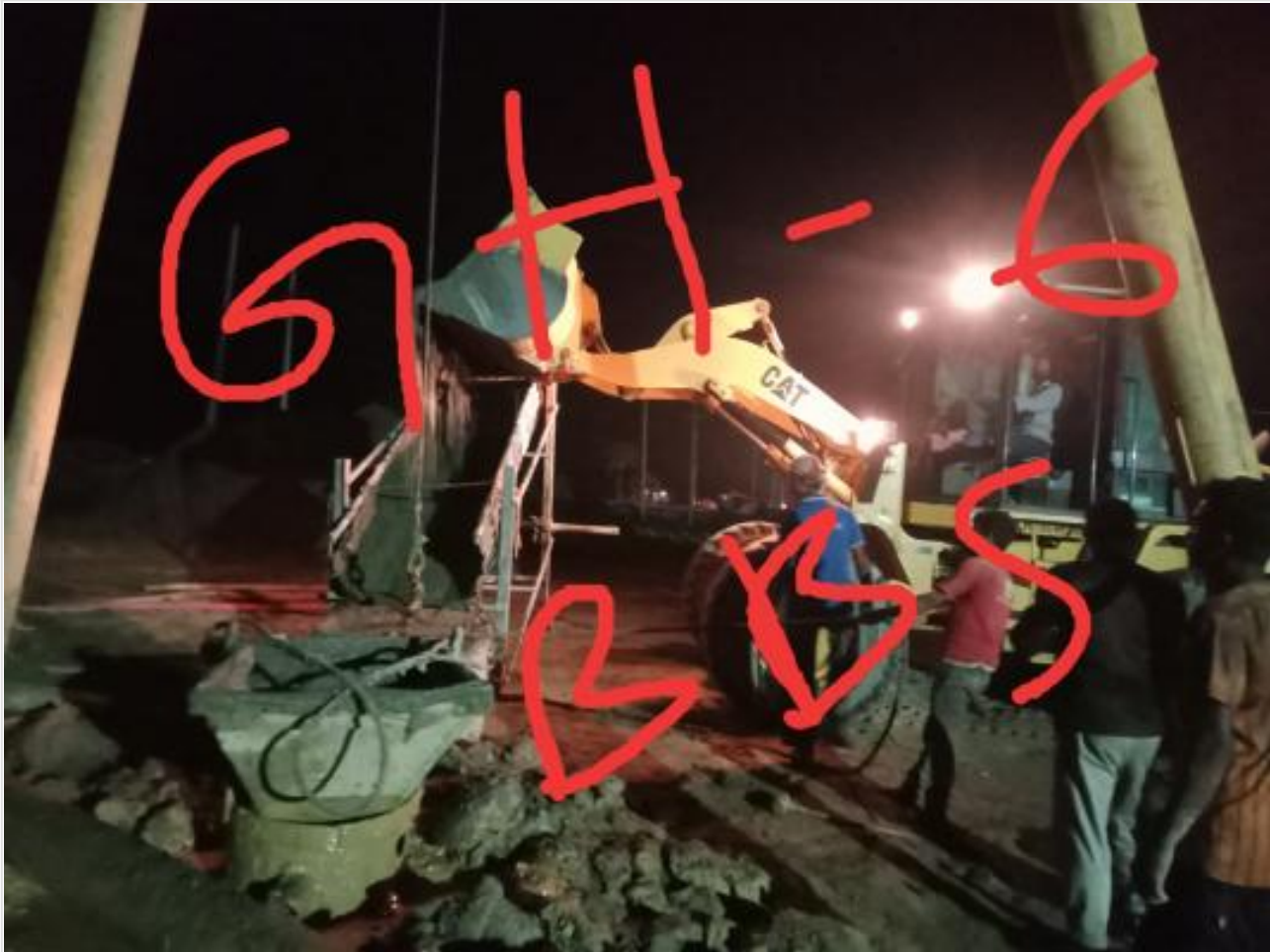
Ready mix concreting of pile on 21-03-23
