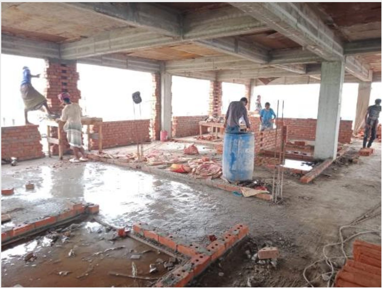
Comp. Bldg. 1st floor brick wall on 24-08-23
