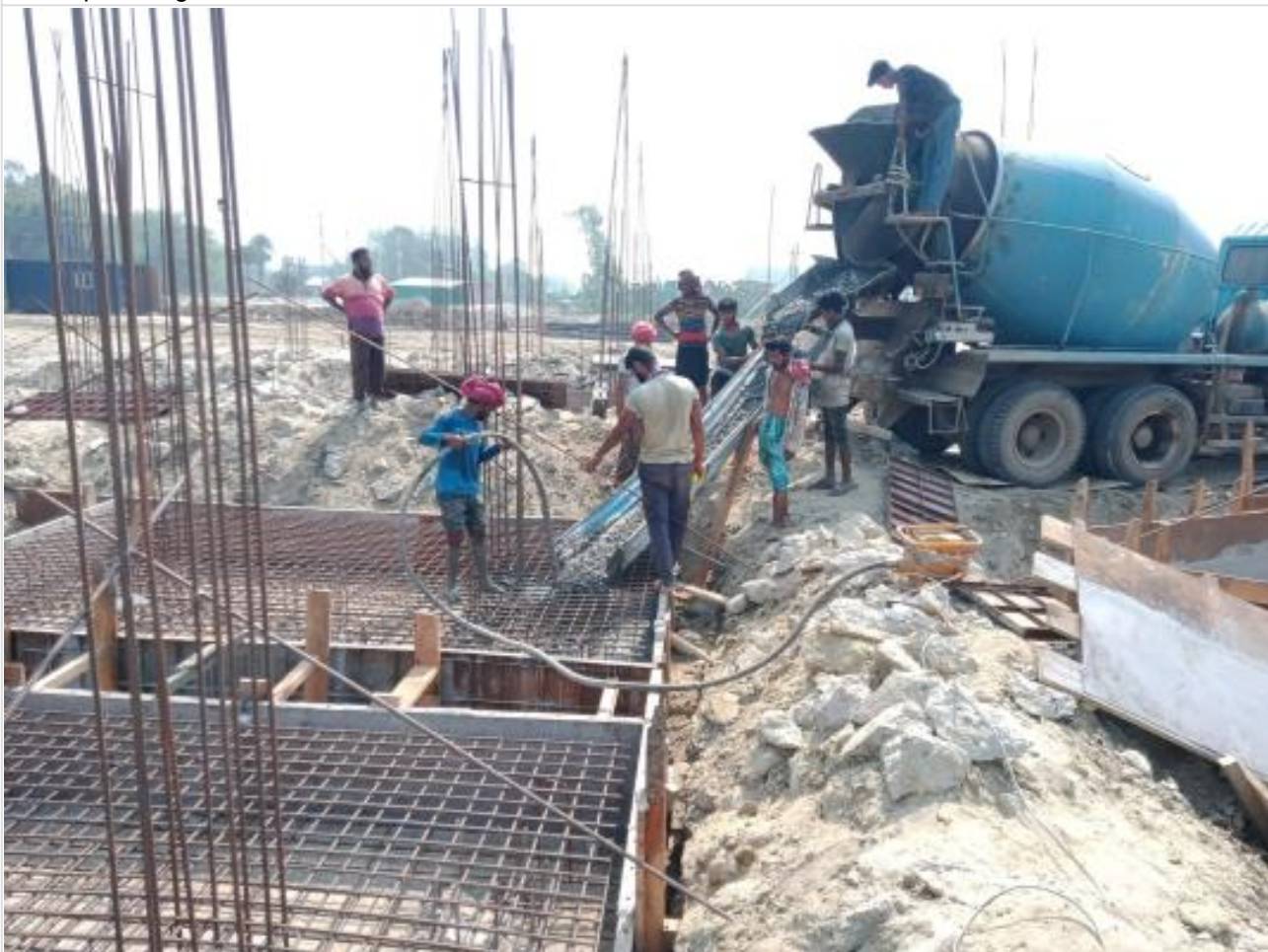
Com. Bldg. Pile cap casting on 17-04-23
