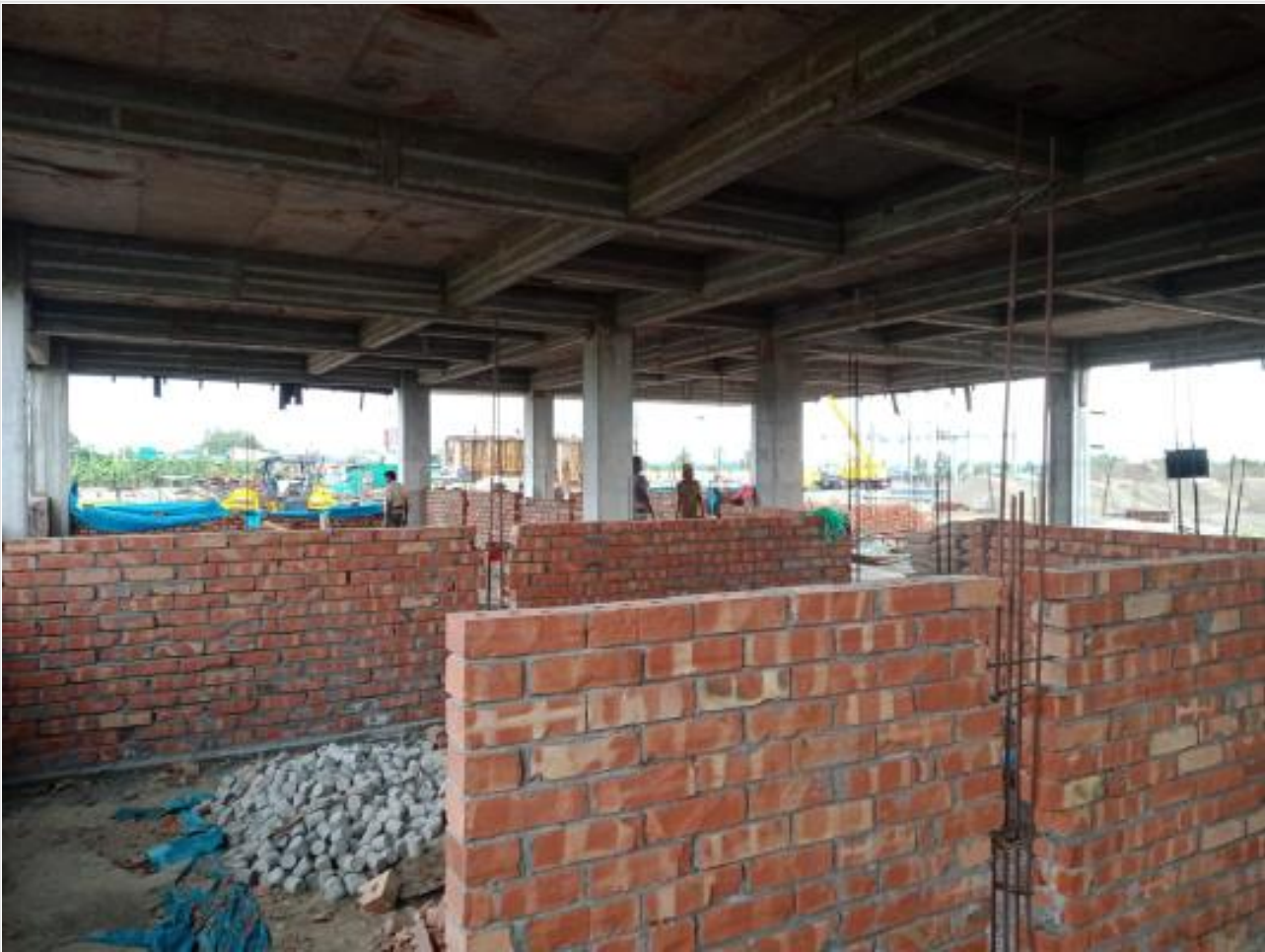
Comp. Bldg. GF Brick work on 21-07-23
