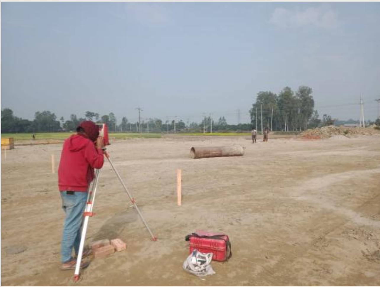
Pile Point Layout and Survey on 01-02-23
