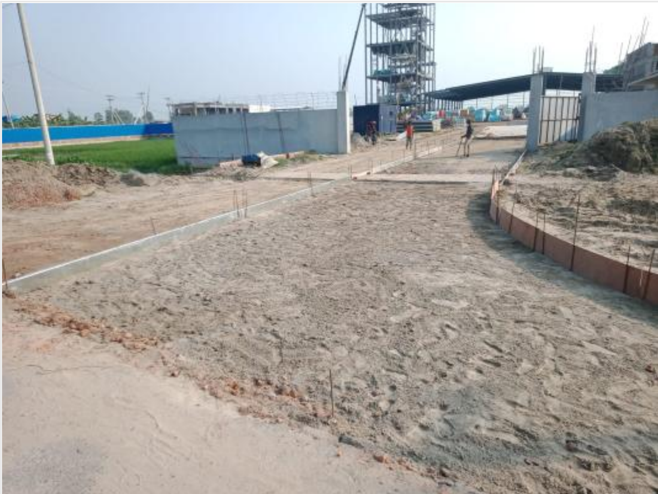
Road work on 14-10-23
