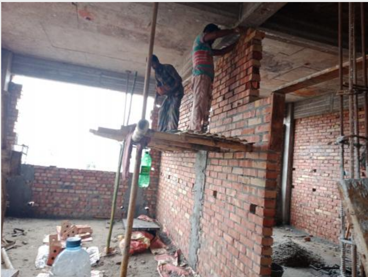
Comp-GF-Brick Work on 07-08-23
