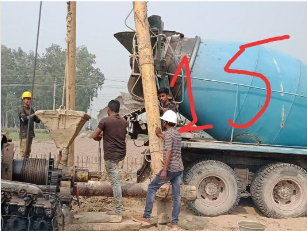
Ready mix concreting of pile on 19-02-23
