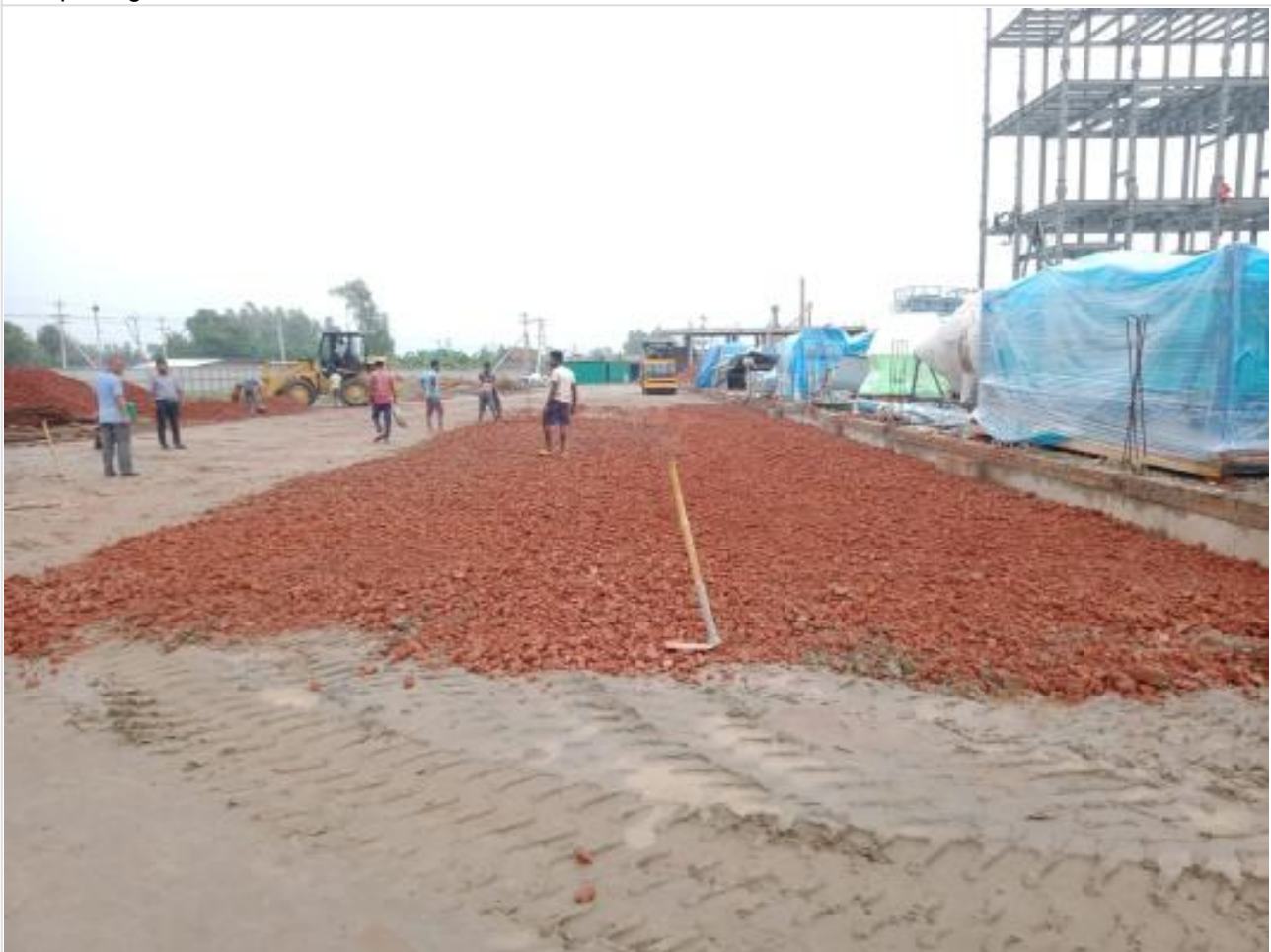
Road work on 24-08-23
