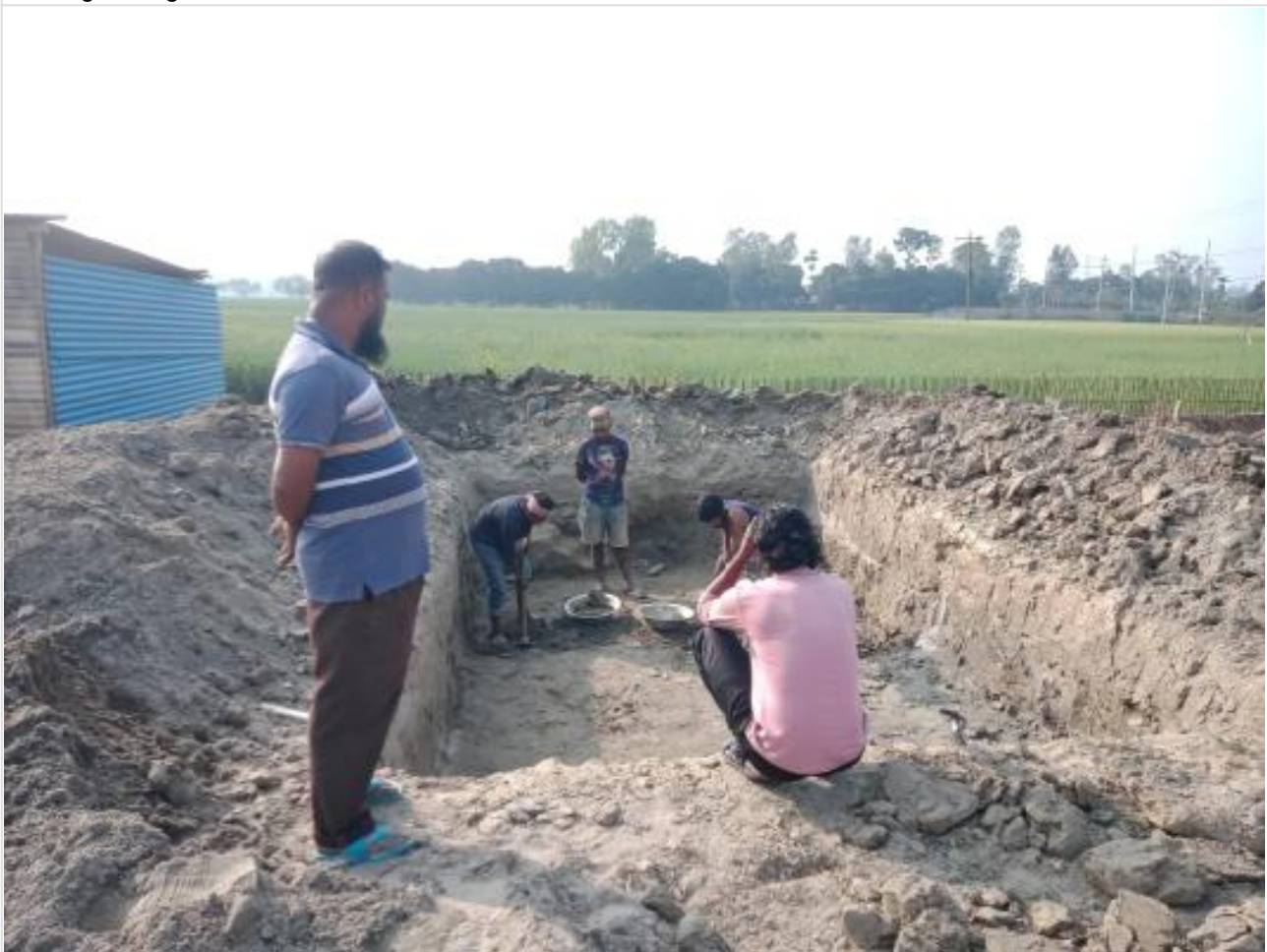
Excavation for Pile Mud Tank on 03-02-23
