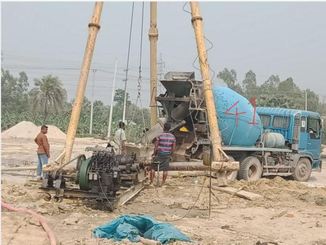
Ready mix concreting of pile on 03-03-23
