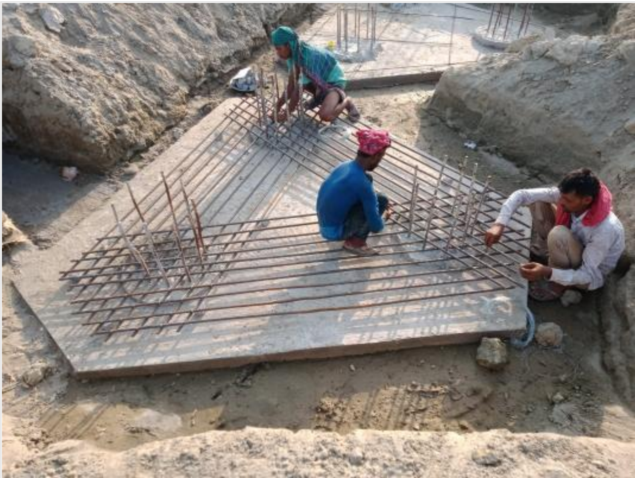
Pile cap work on 14-04-23
