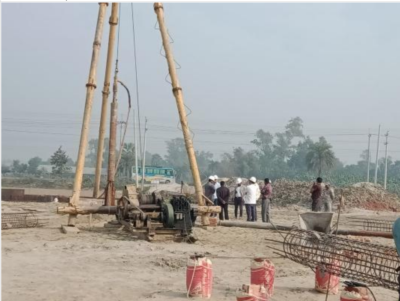
Inspection before Pile driving on 08-02-23
