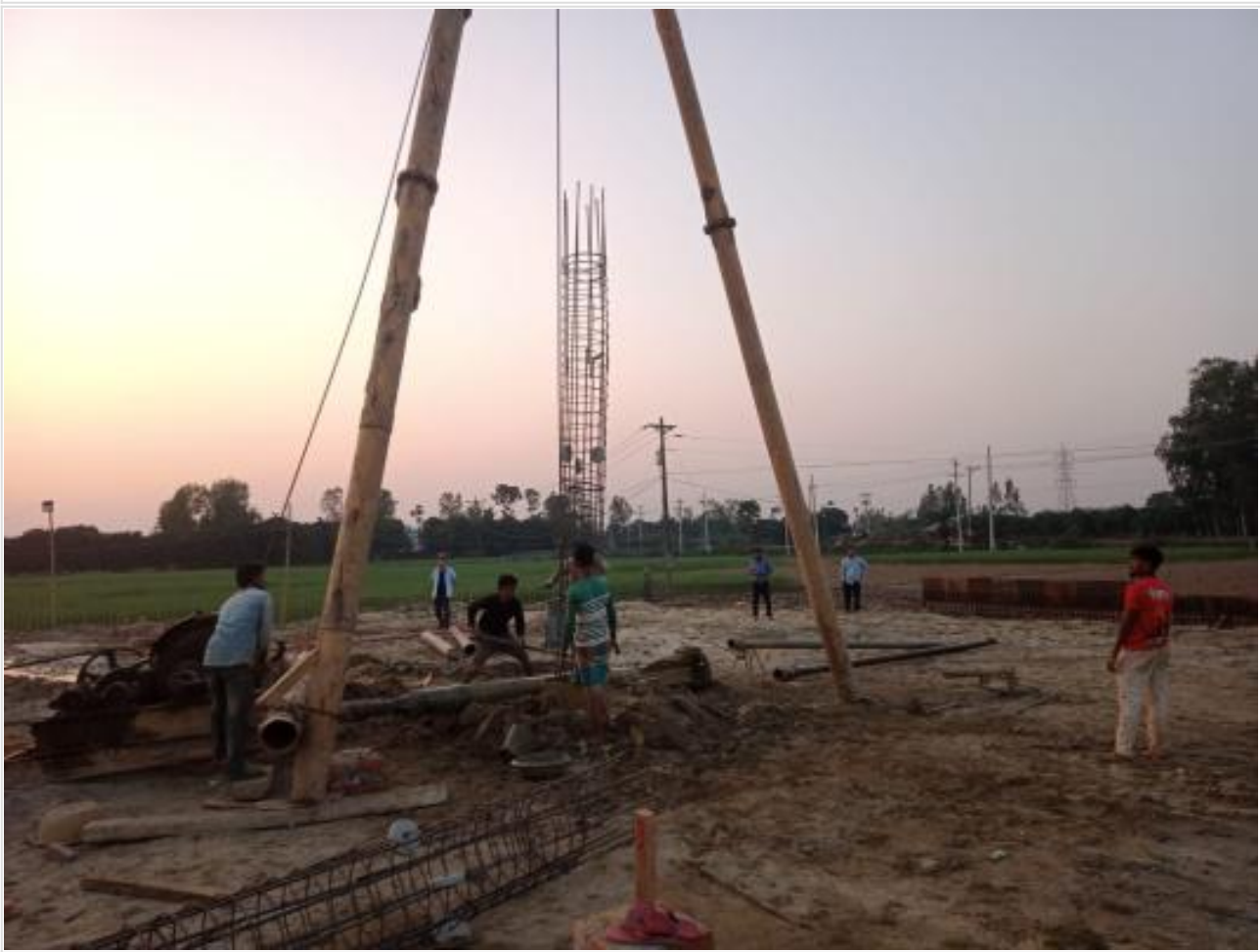
Pile boring work on 14-02-23
