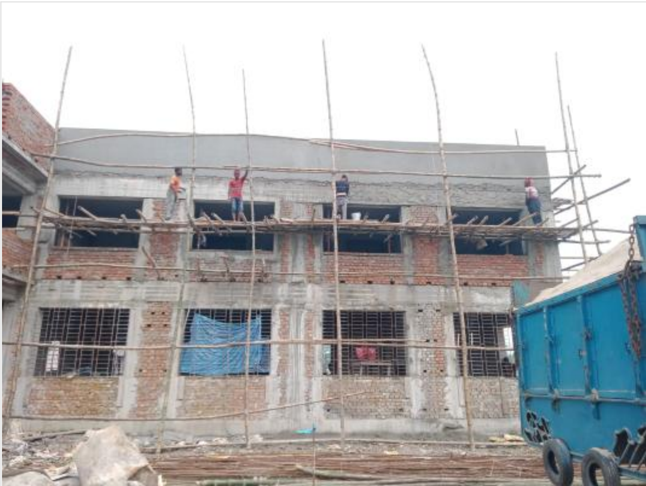
Comp. Bldg. Outside plaster work on 10-10-23
