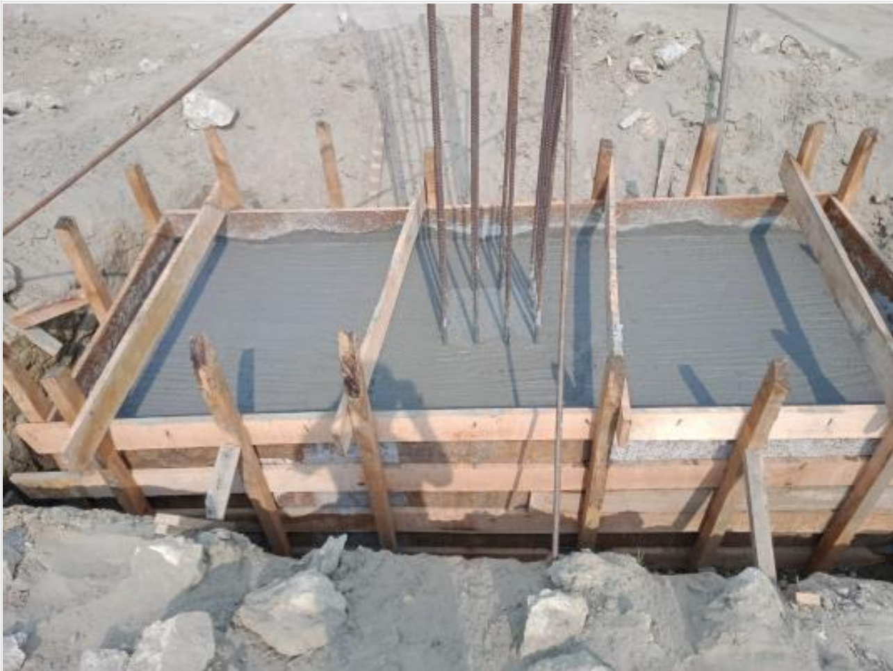
Pile Cap concreting. on 16-04-23
