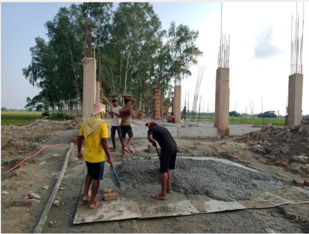
Dorm. Bldg. Column Casting on 23-06-23
