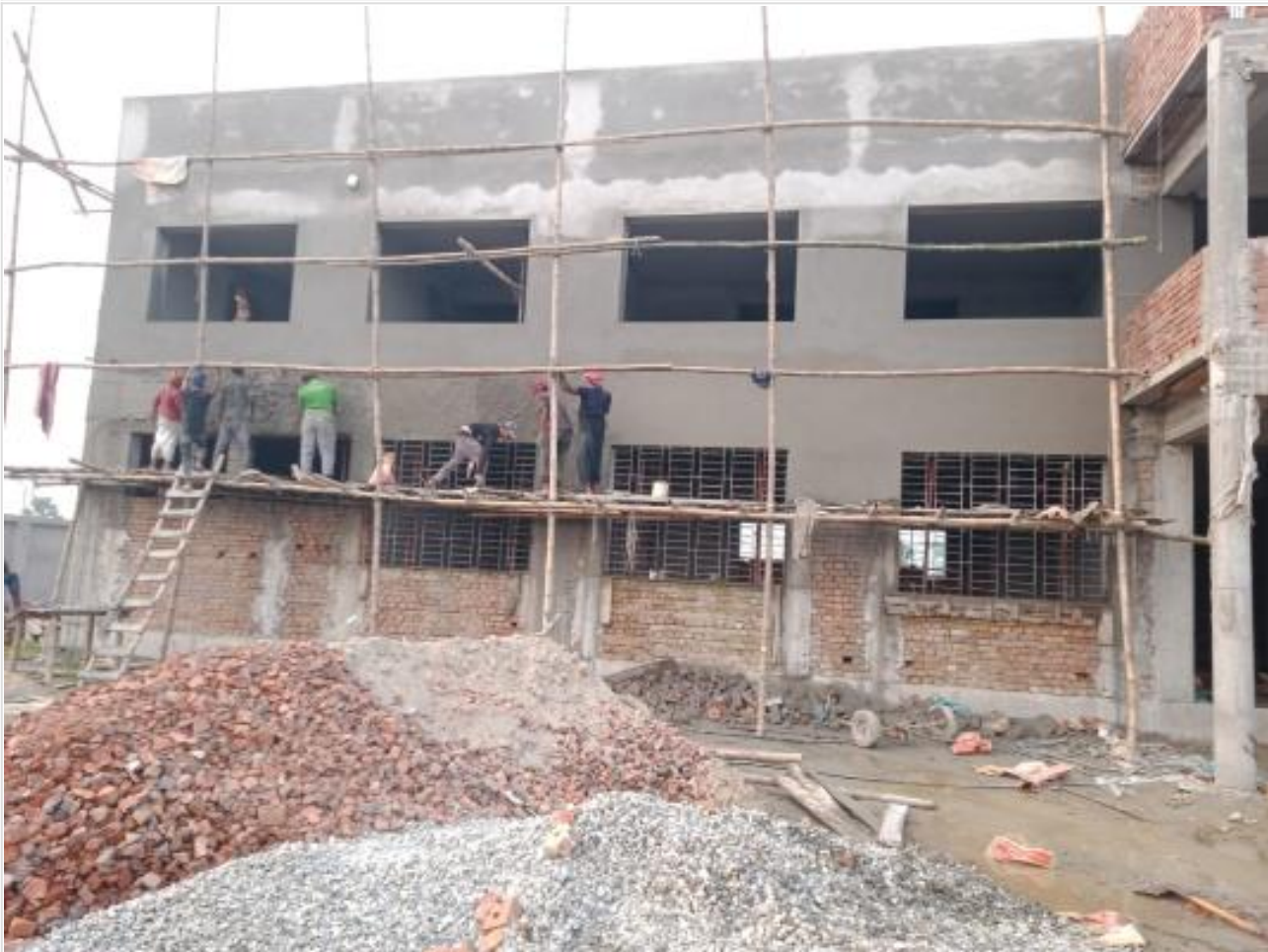
Comp. Bldg. Outside plaster work on 16-10-23
