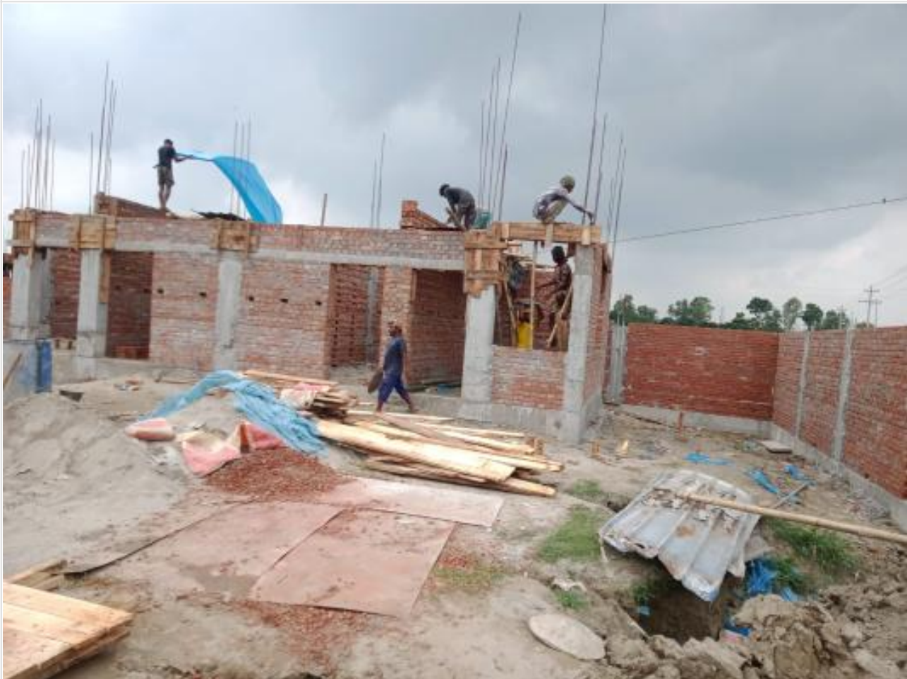
Gate House Lintel casting on 23-06-23
