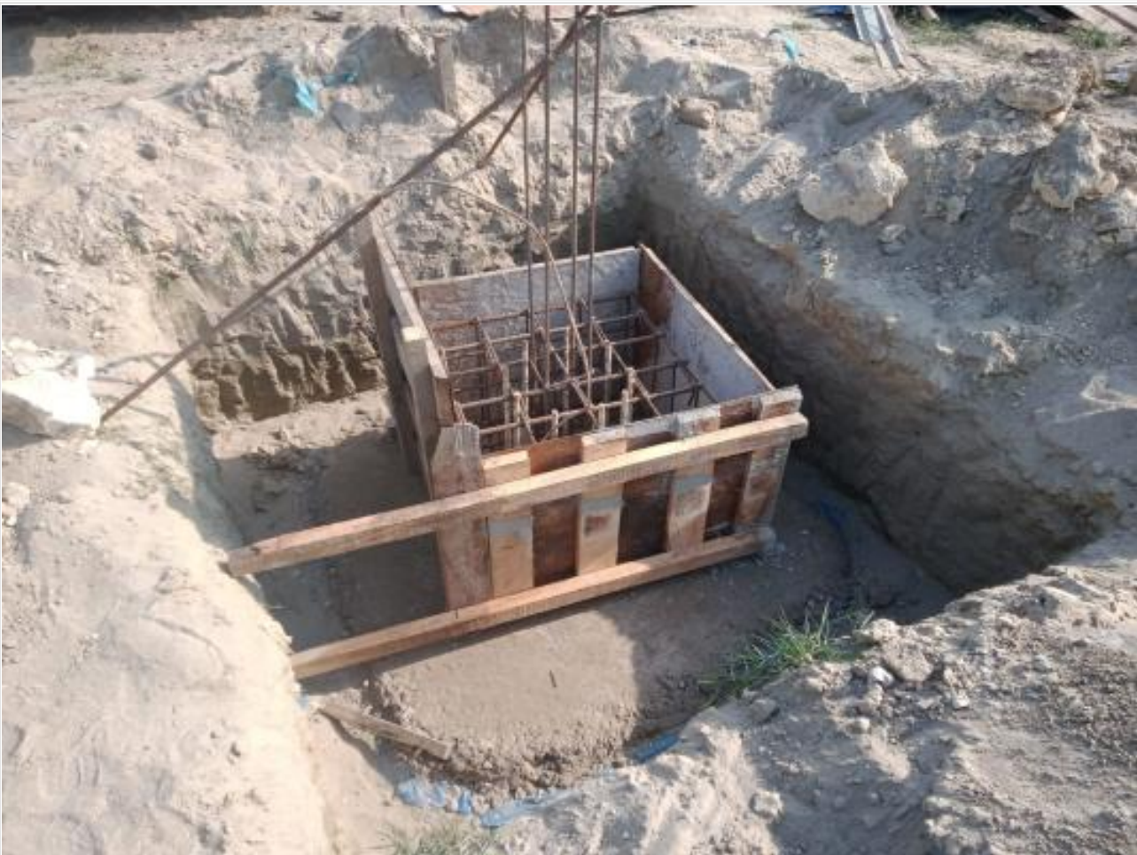
G.House Pile cap work on 09-05-23
