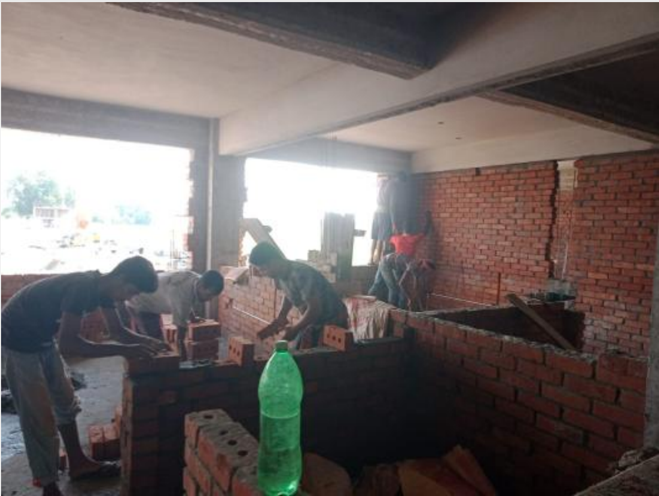
Comp. Bldg. FF Brick work on 09-09-23
