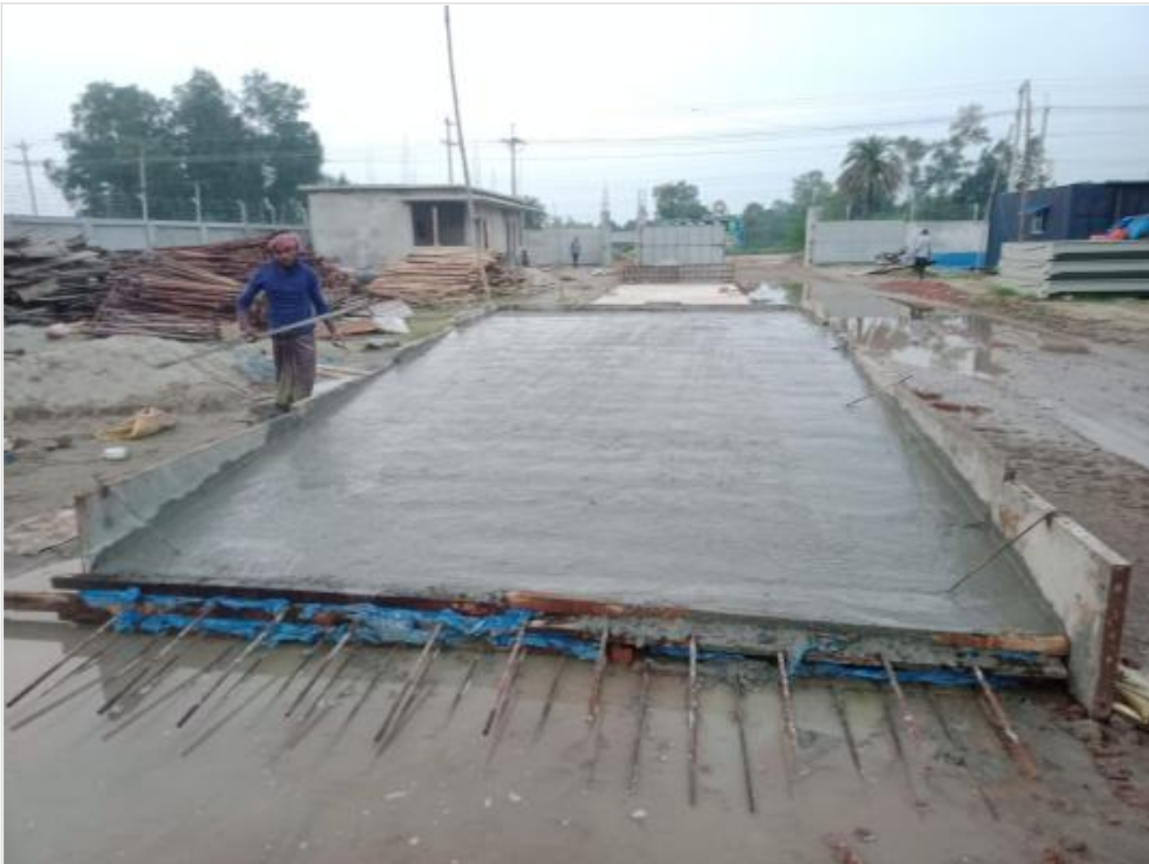
Weight scale concreting on 26-09-23
