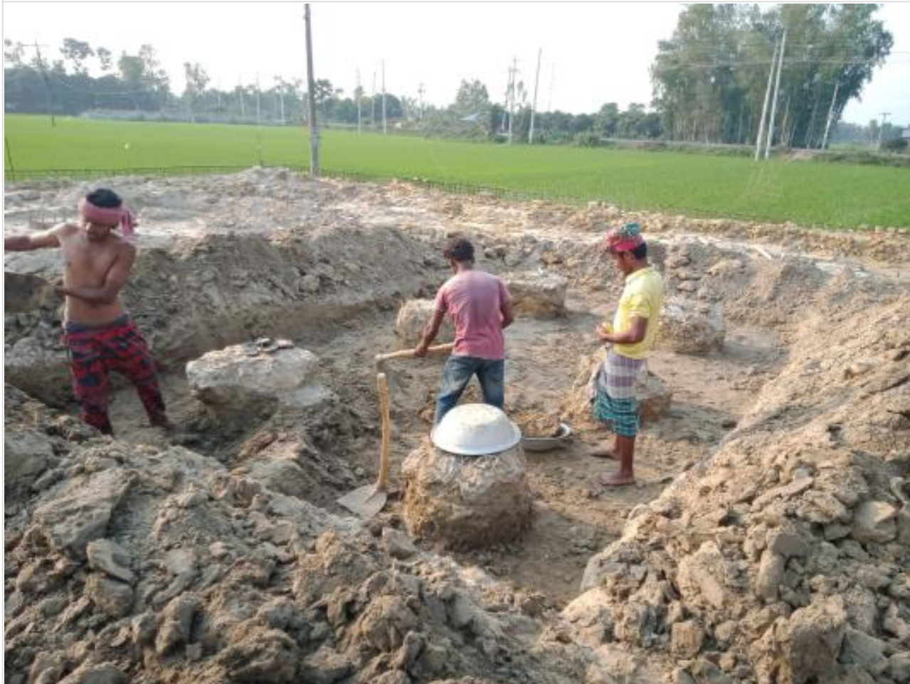
Pile head breaking on 24-03-23
