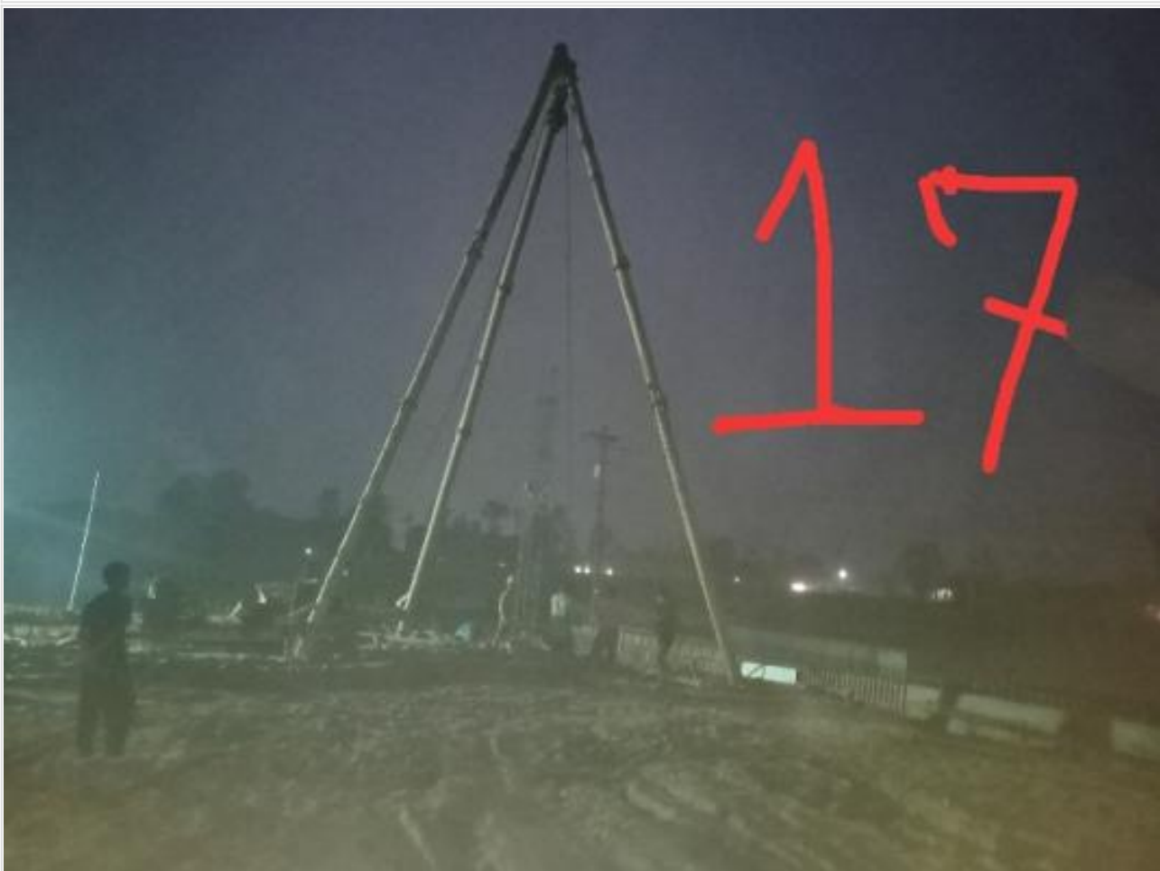
Com. Bldg. 17th Pile Boring on 21-02-23
