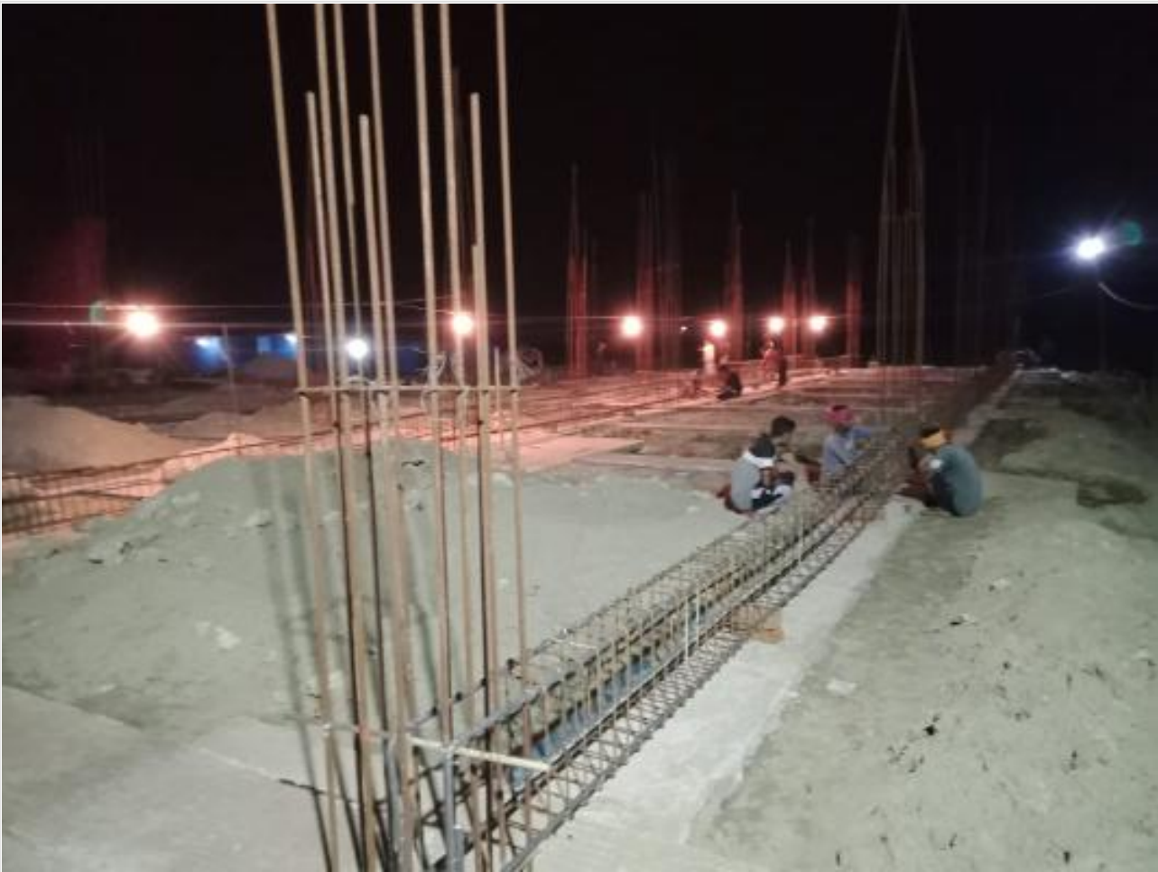
GB Re-bar work on 03-05-23
