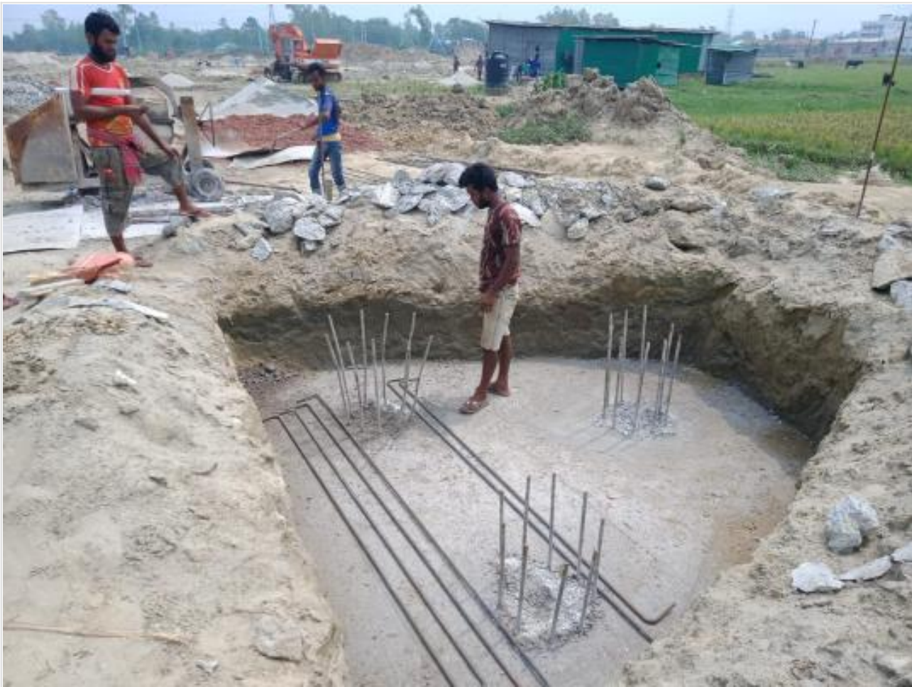
Pile cap rebar work on 23-05-23
