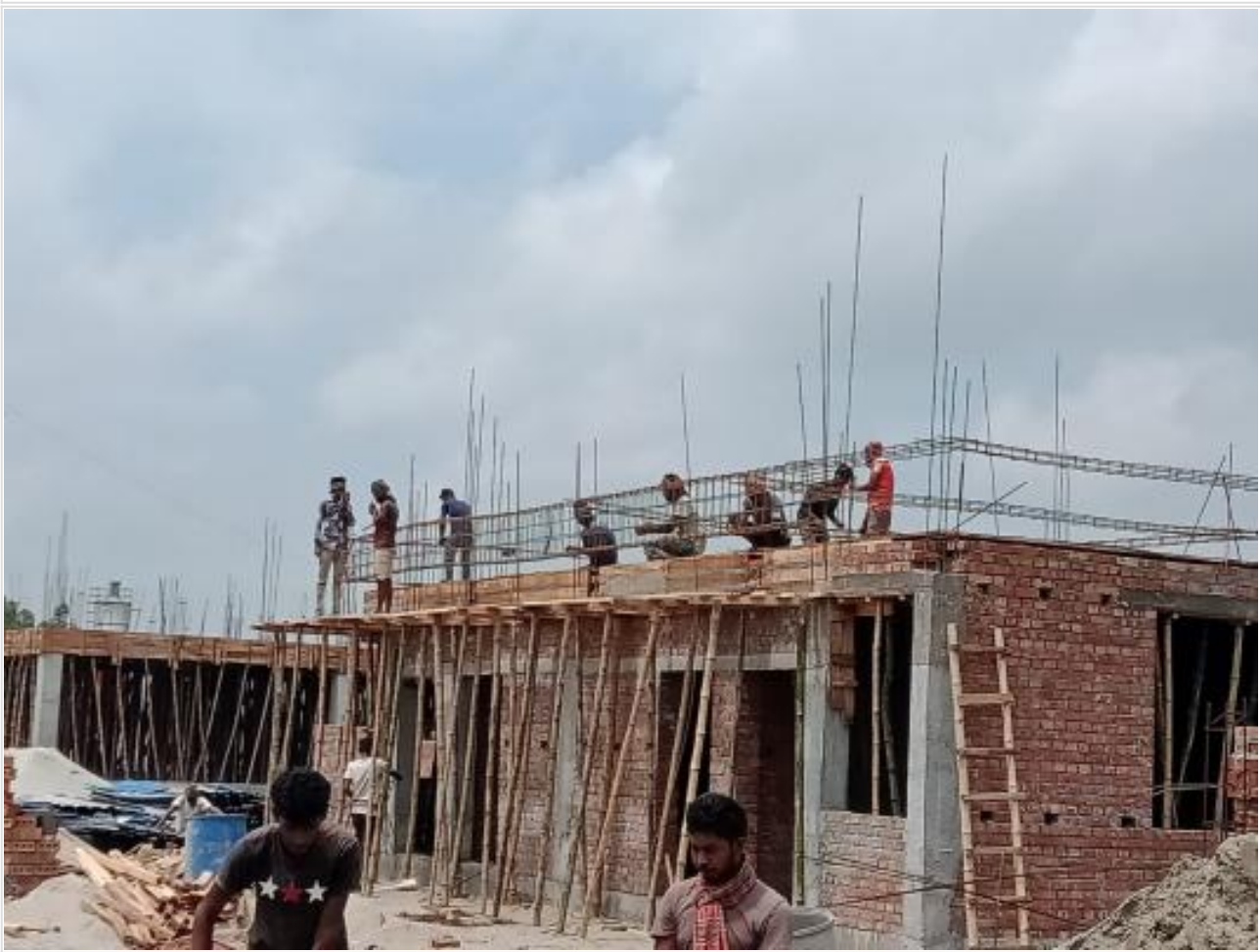
Gate House Slab shuttering and rod bindi on 25-06-23
