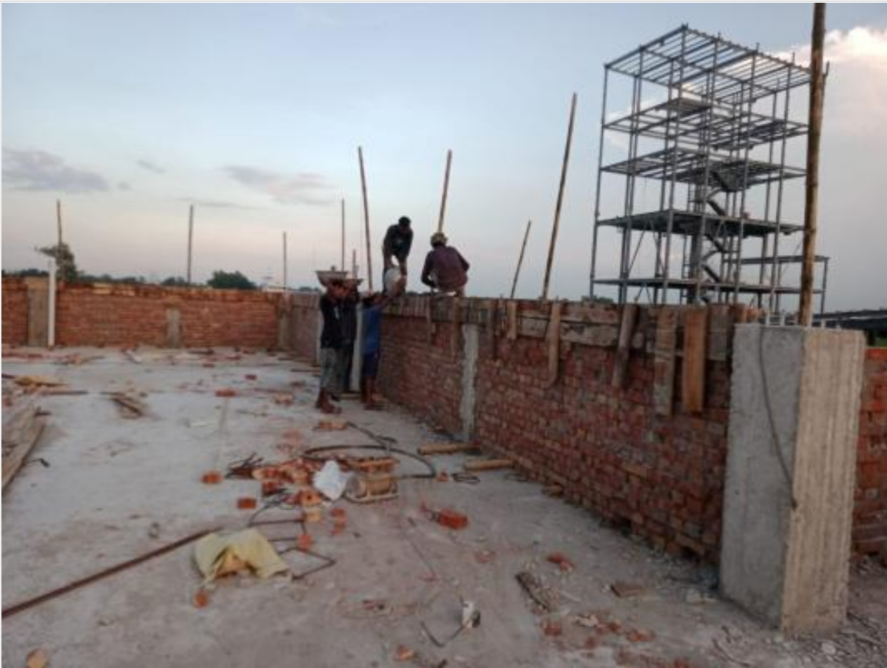
Comp. Roof top parapet work on 01-10-23
