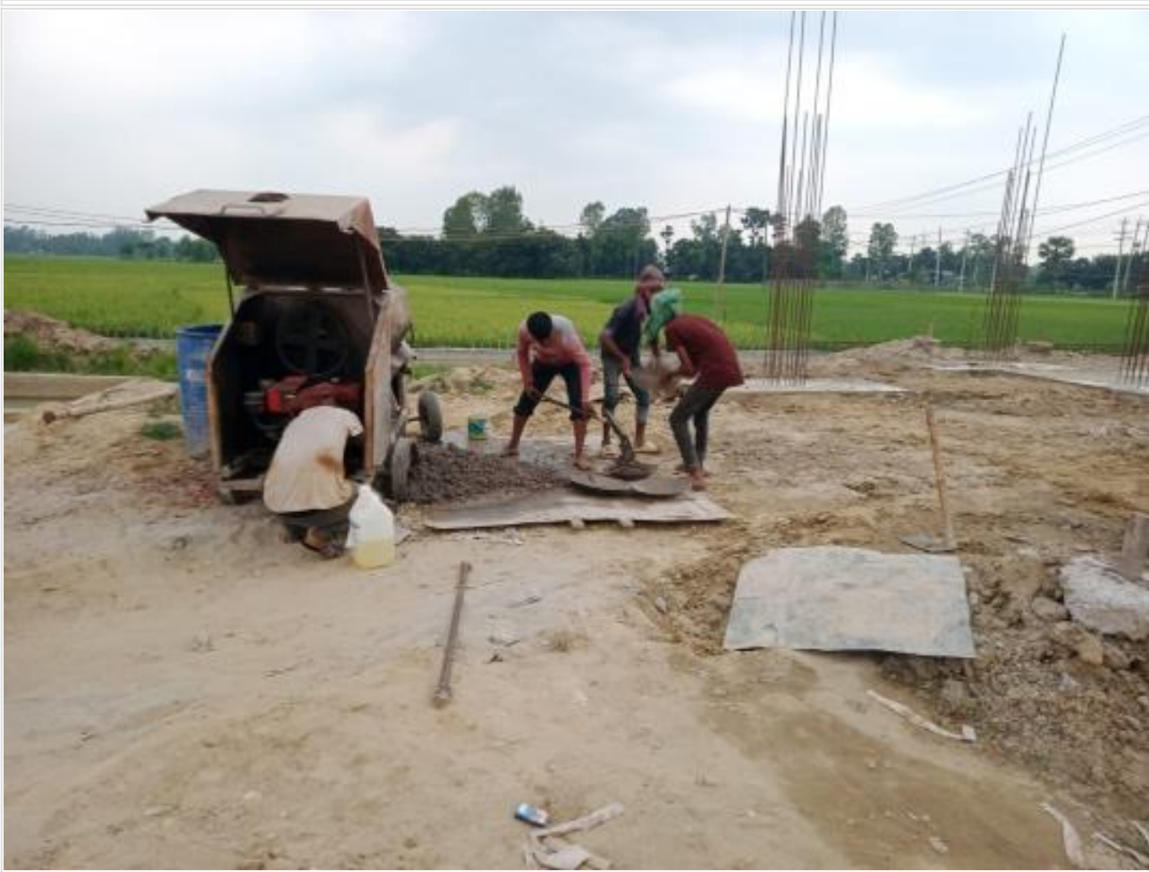
C.C work at GB Bottom of comp. Bldg. on 29-04-23
