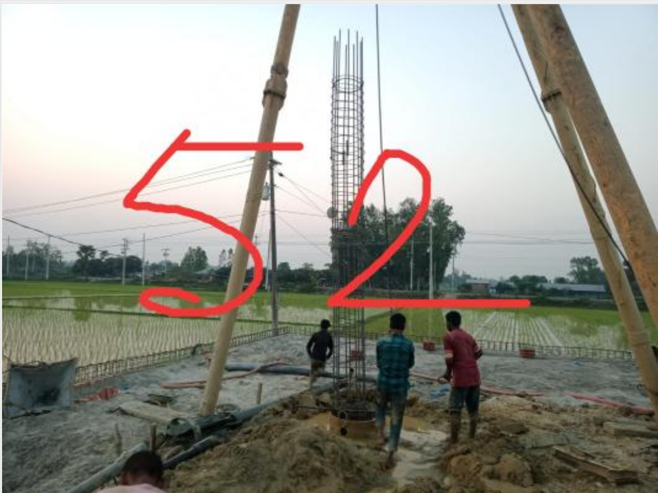
Ready mix concreting of pile on 09-03-23
