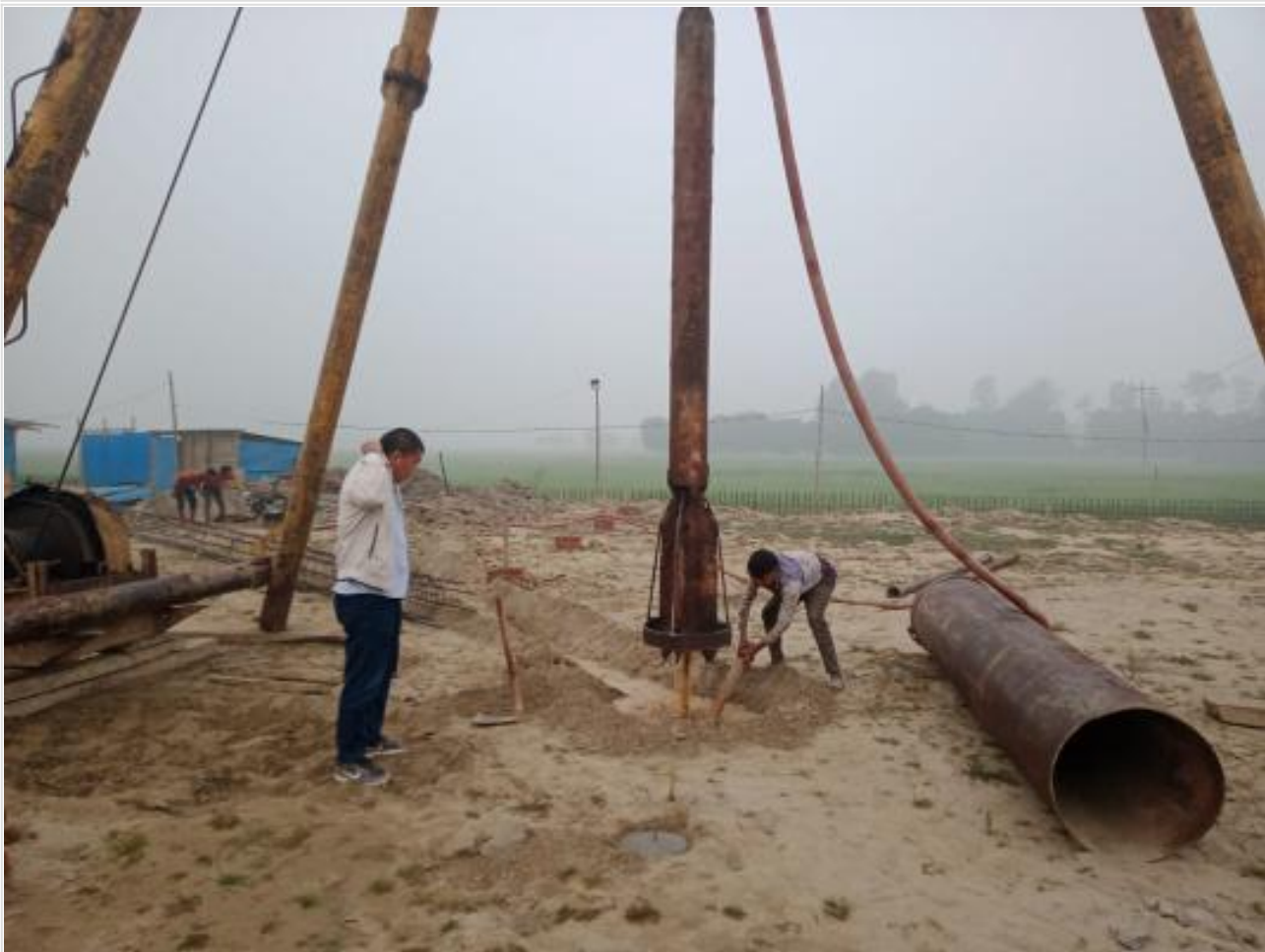
Pile Driving Starting on 09-02-23
