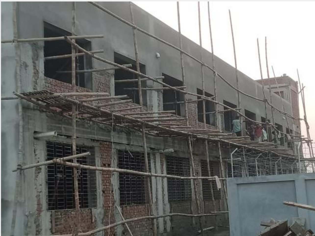
Comp. Bldg. Outside plaster work on 18-10-23
