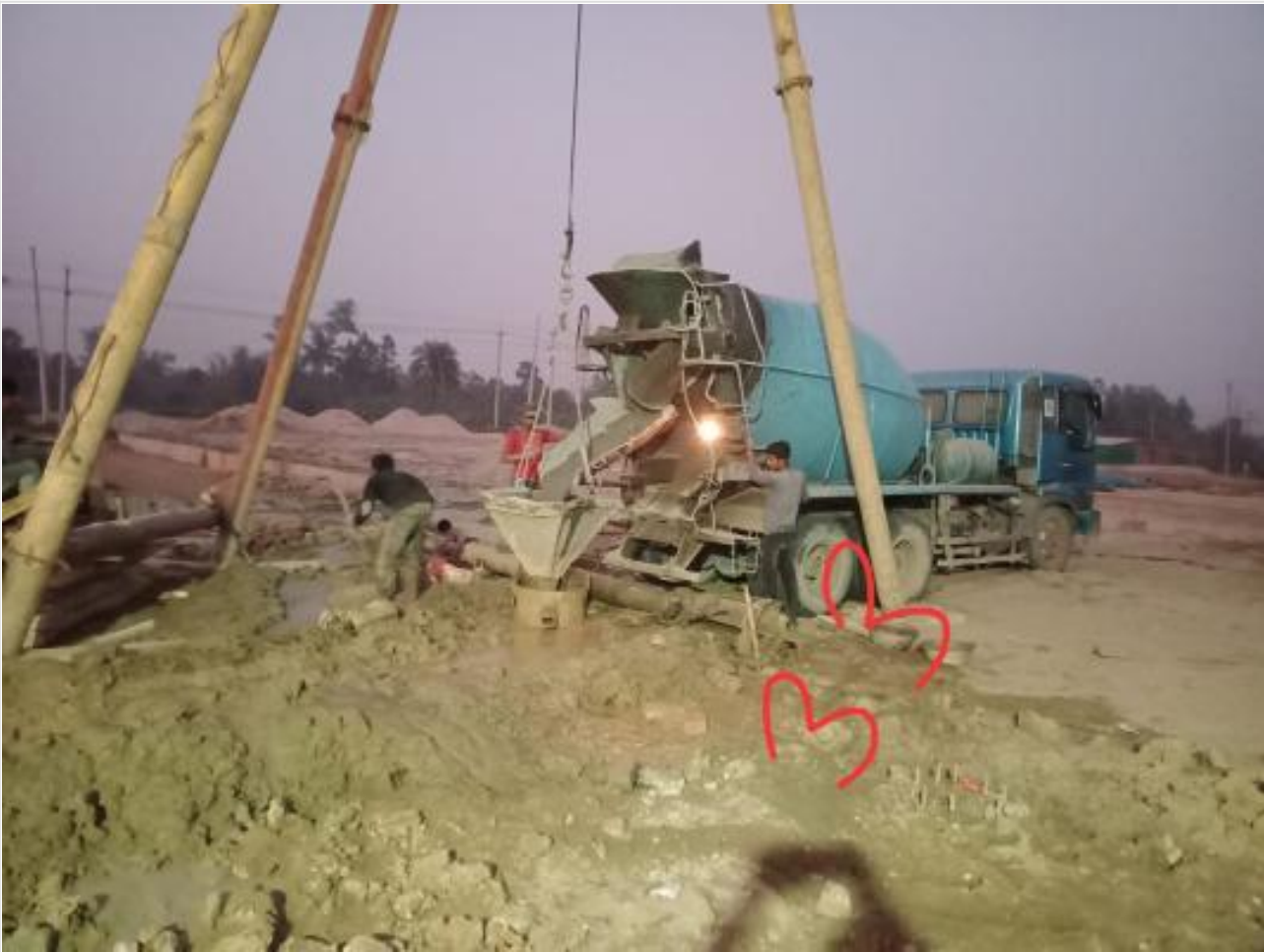
Ready mix concreting of pile on 27-02-23
