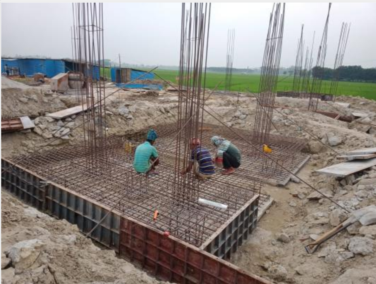
Pile Cap rebar binding on 15-04-23
