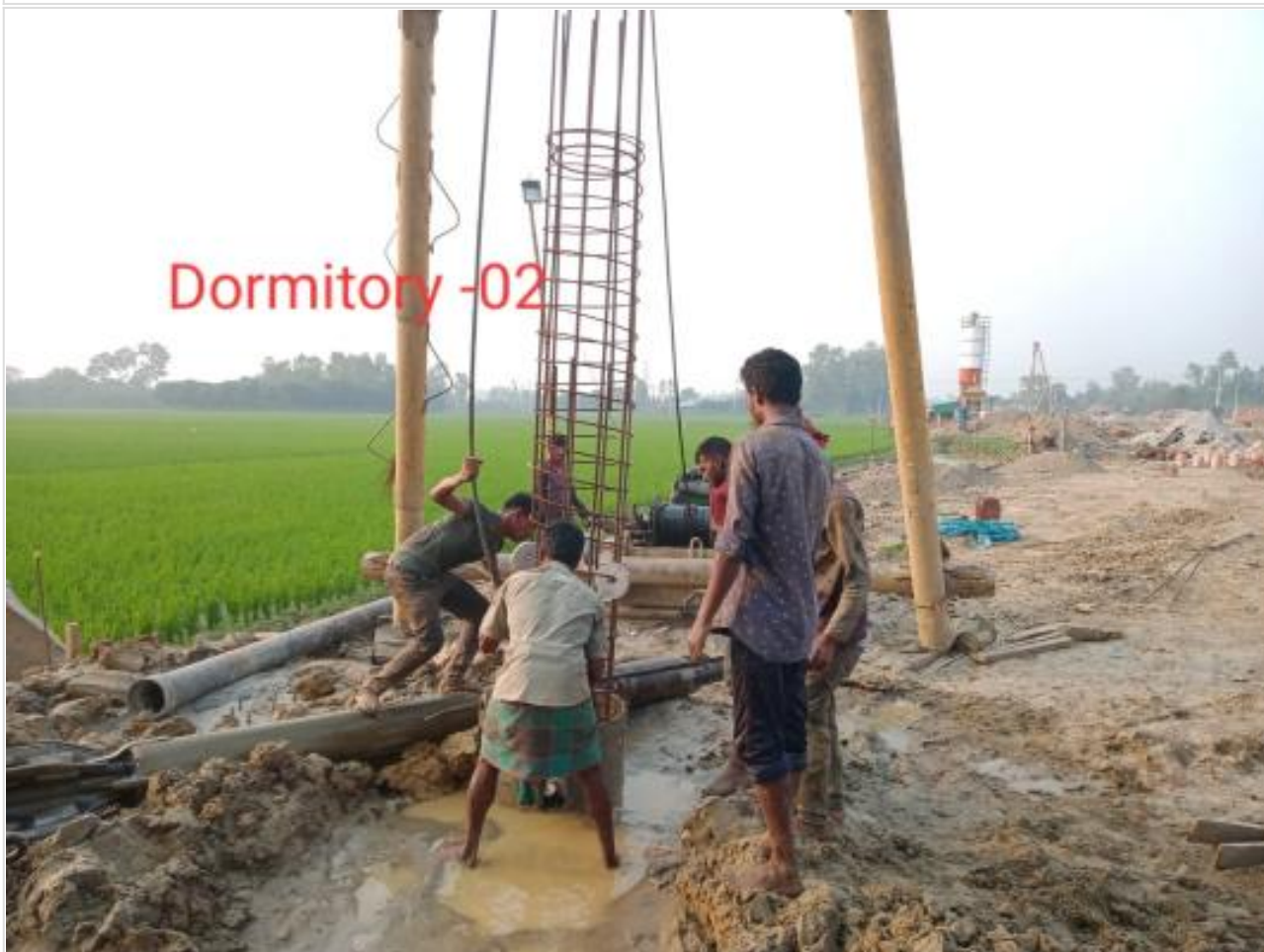
Pile head breaking on 24-03-23
