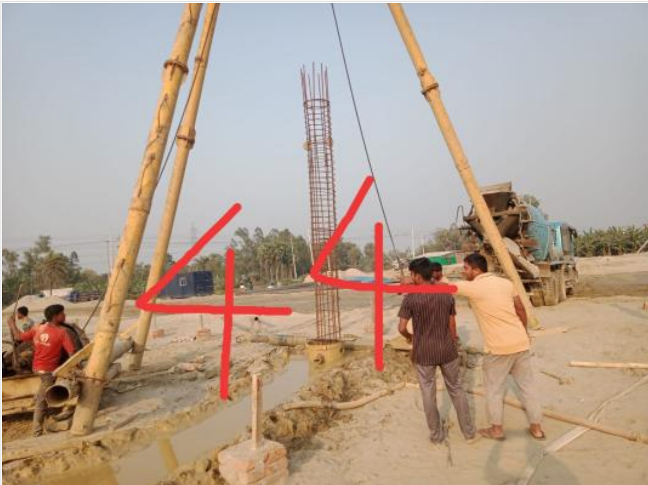
Com. Bldg. 44 pile boring on 05-03-23
