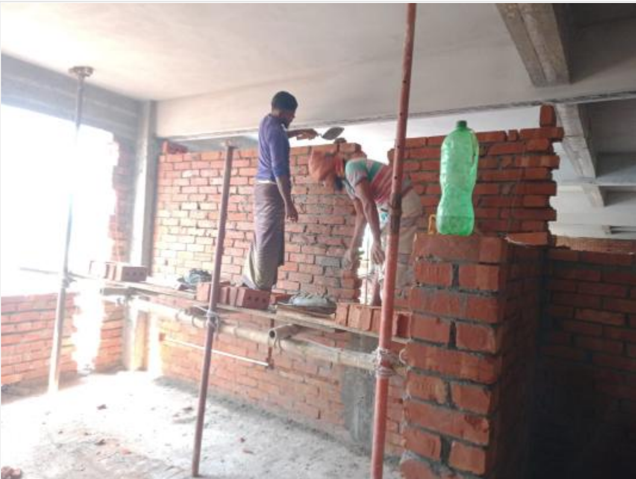
Comp. Bldg. 2nd Floor work on 10-09-23
