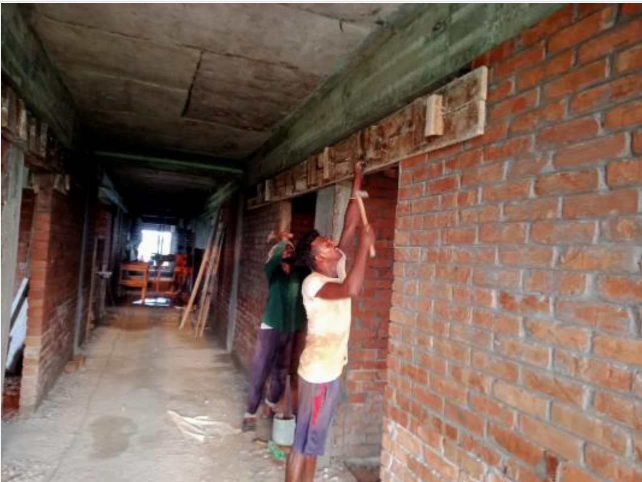
Comp. Bldg. Plaster work on 11-09-23
