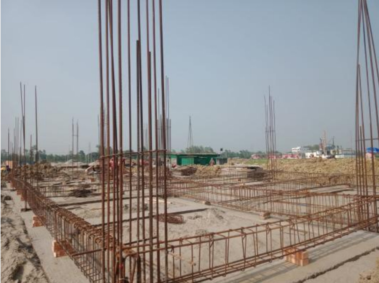
Dorm. Bldg. Rebar work for GB on 04-06-23
