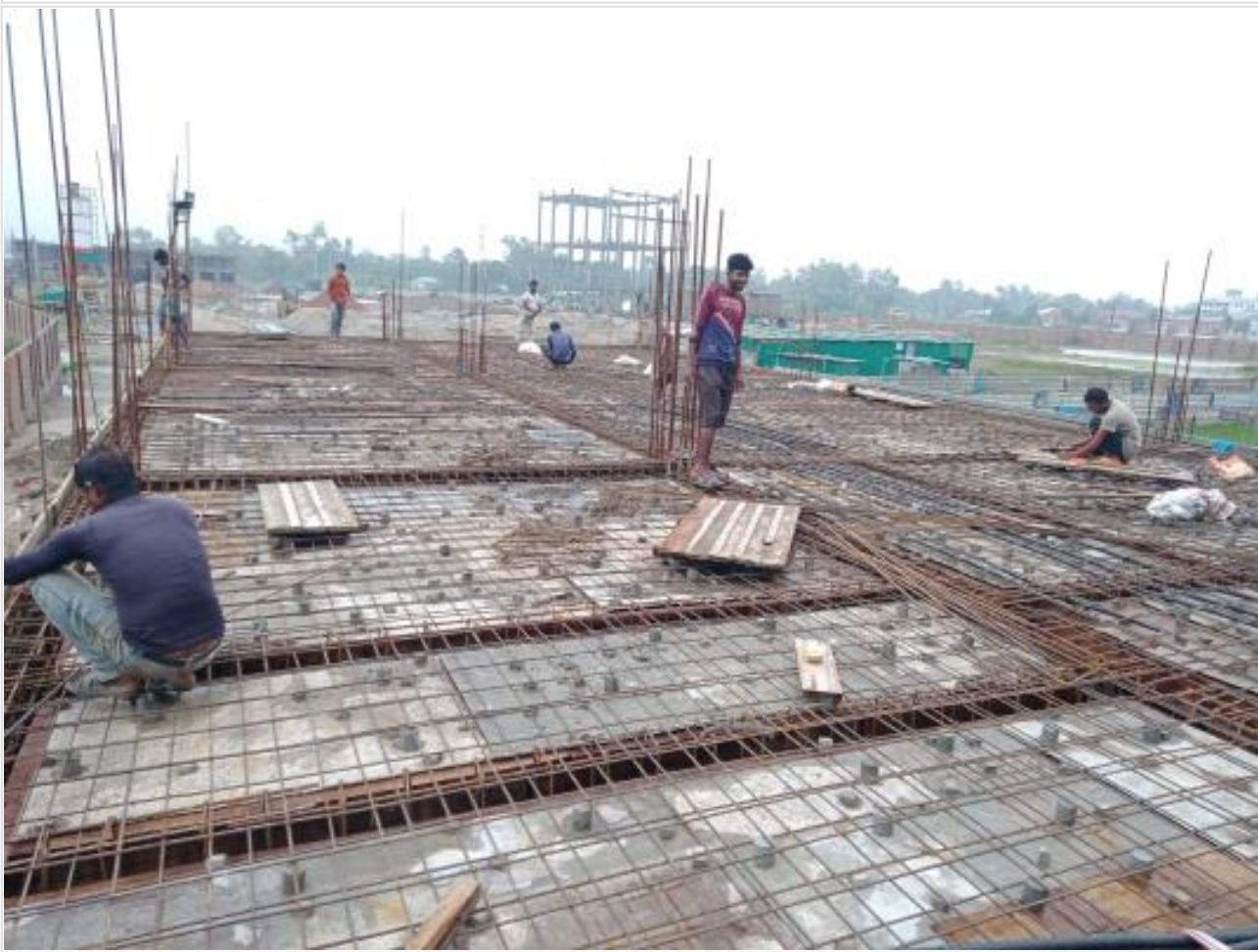
Dormitory Slab Electric Pipe Laying on 09-08-23
