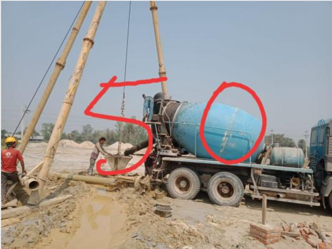
Ready mix concreting of pile on 09-03-23
