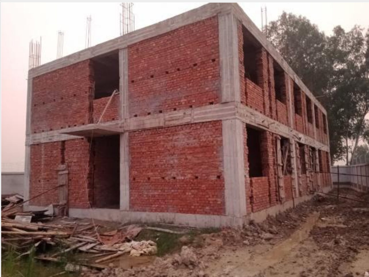
Dorm. Bldg. Brick work on 10-10-23
