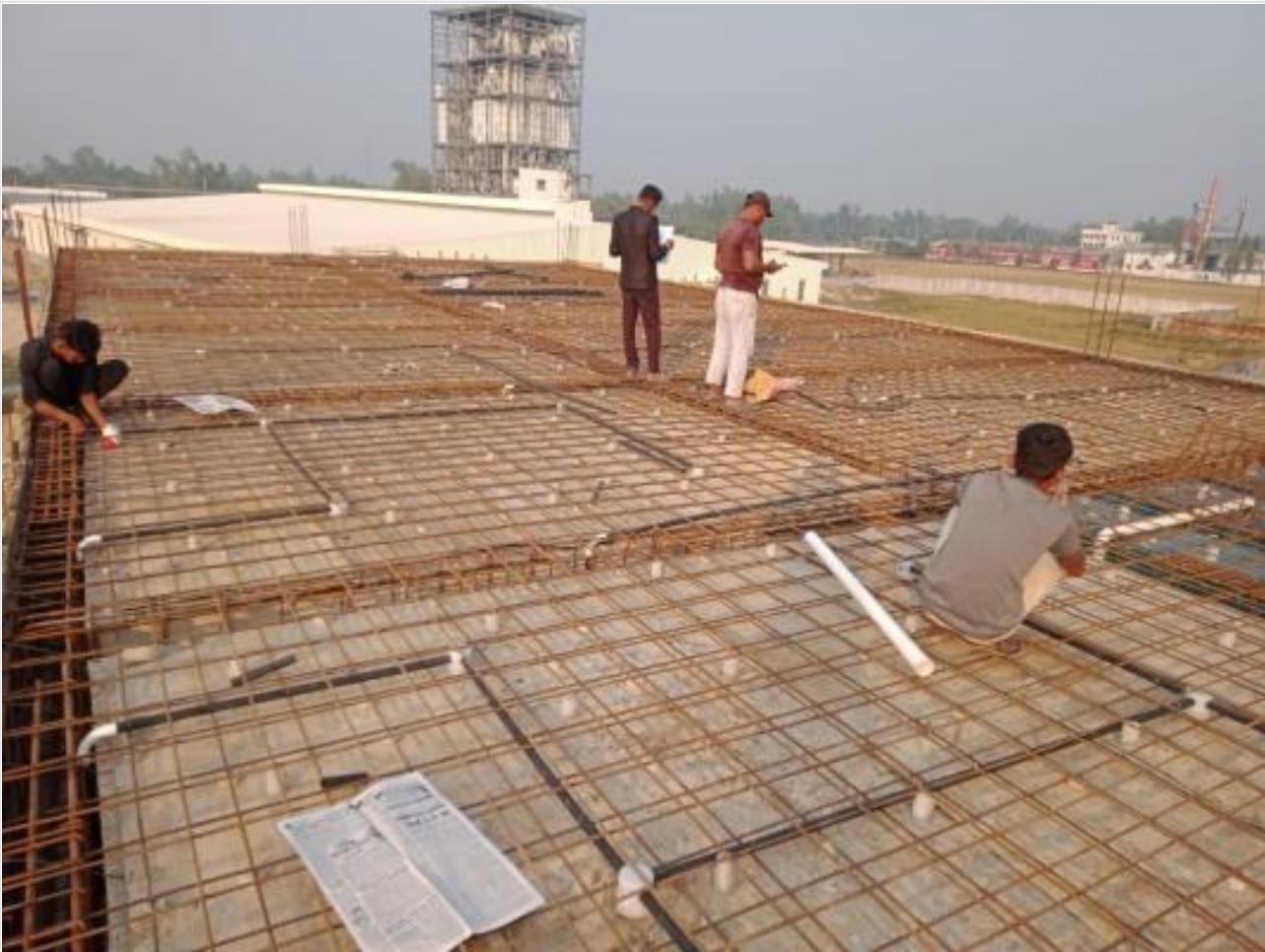
Dormitory-3rd Floor Slab Re-bar Work on 18-12-23
