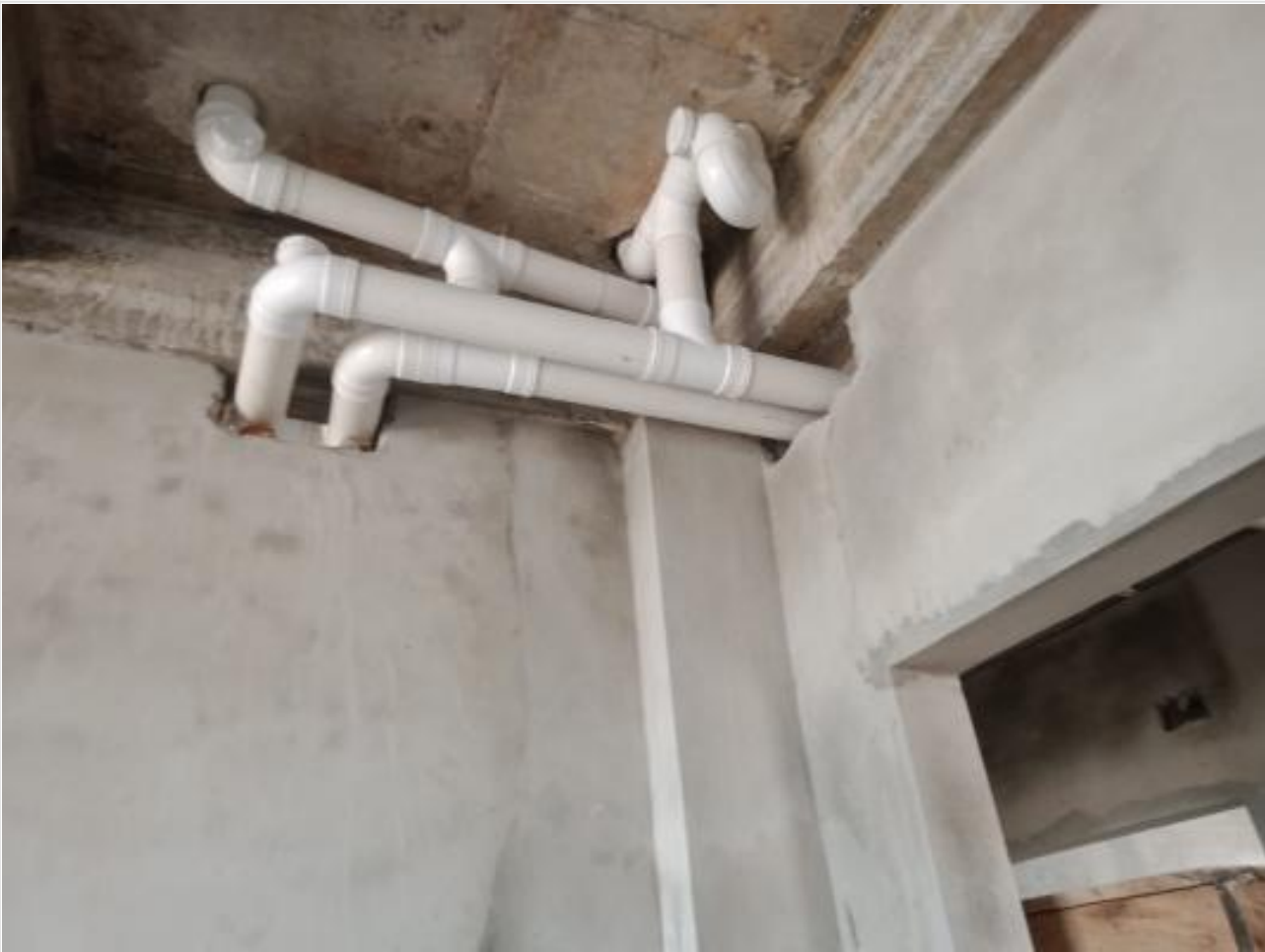
Comp. Bldg 1st floor sanitary work on 07-09-23
