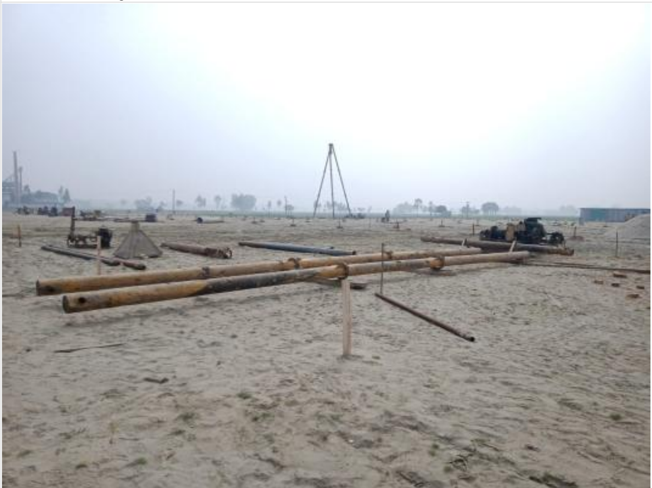
Pile Rig Installing on 31-01-23
