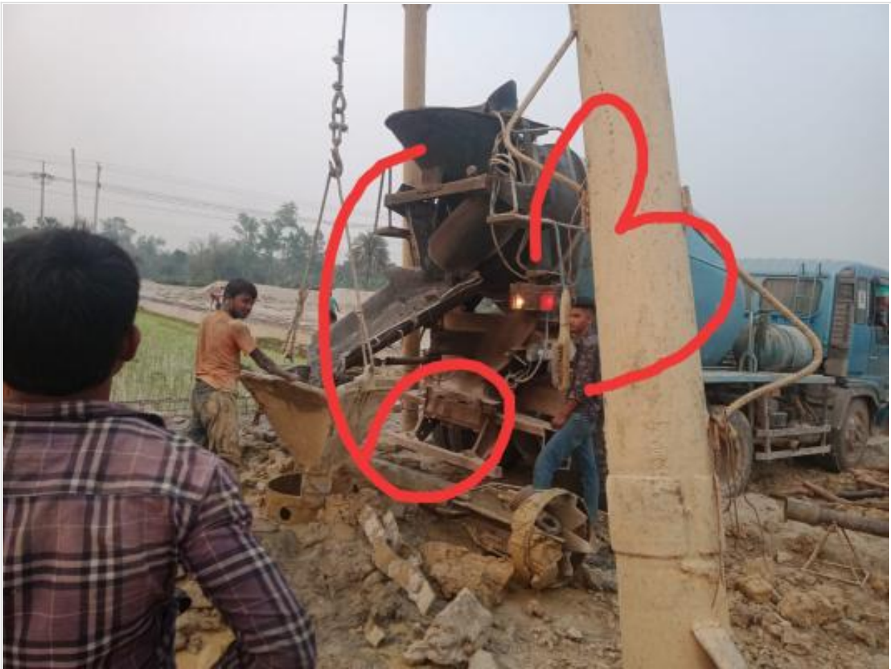
Ready mix concreting of pile on 14-03-23
