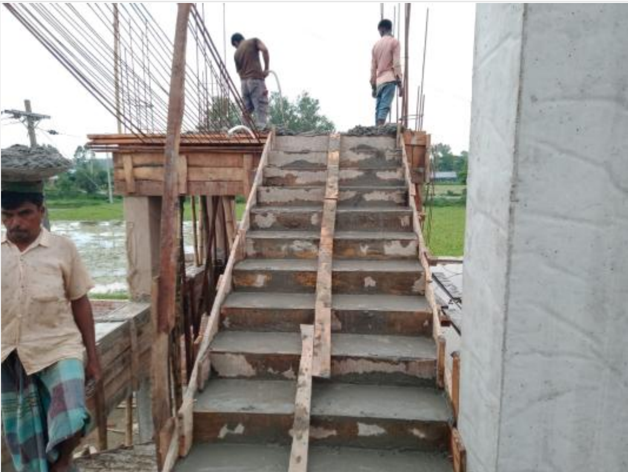
Comp. Bldg. 1st flight stair casting on 16-07-23
