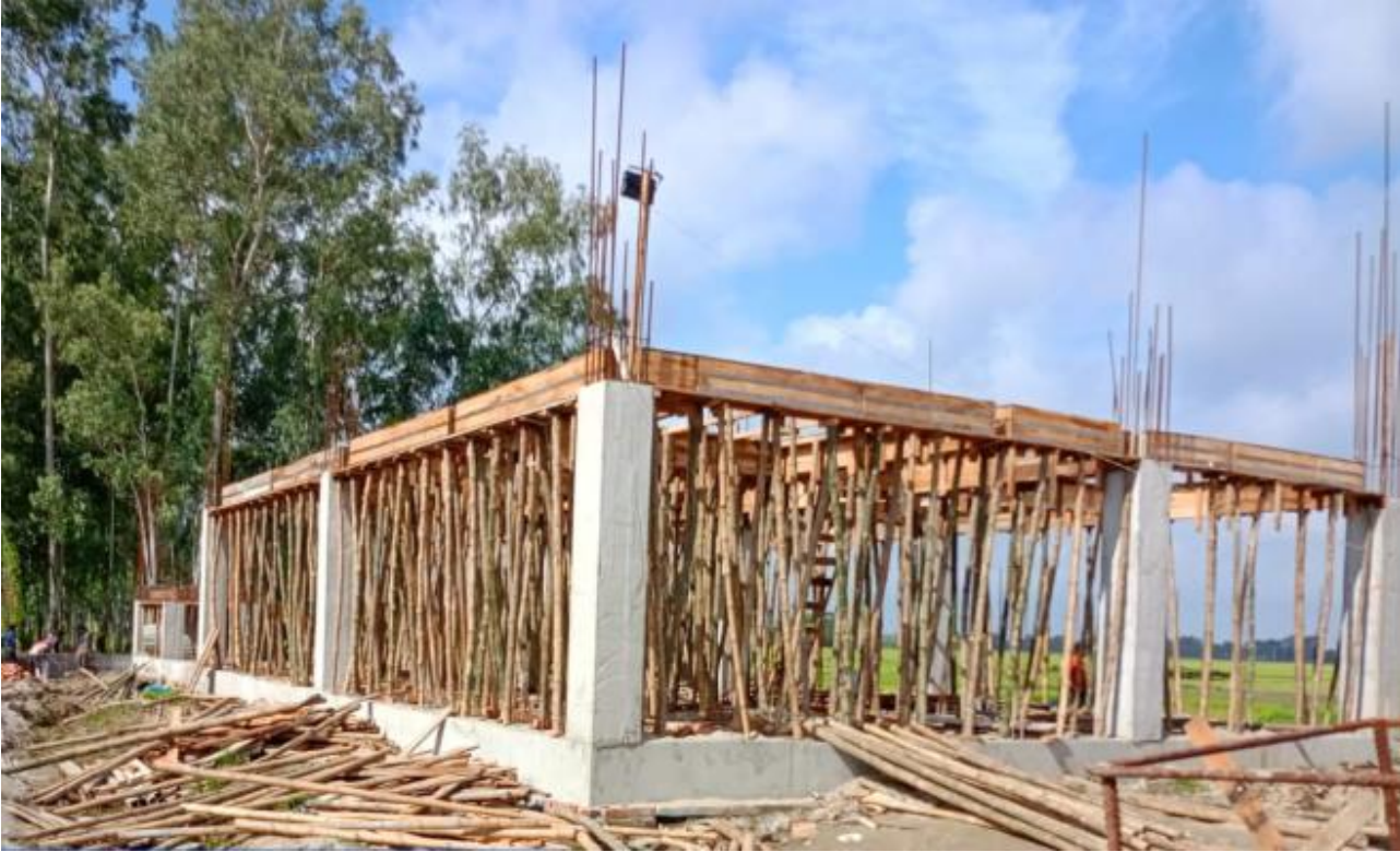
Dorm. Bldg shuttering work on 27-07-23
