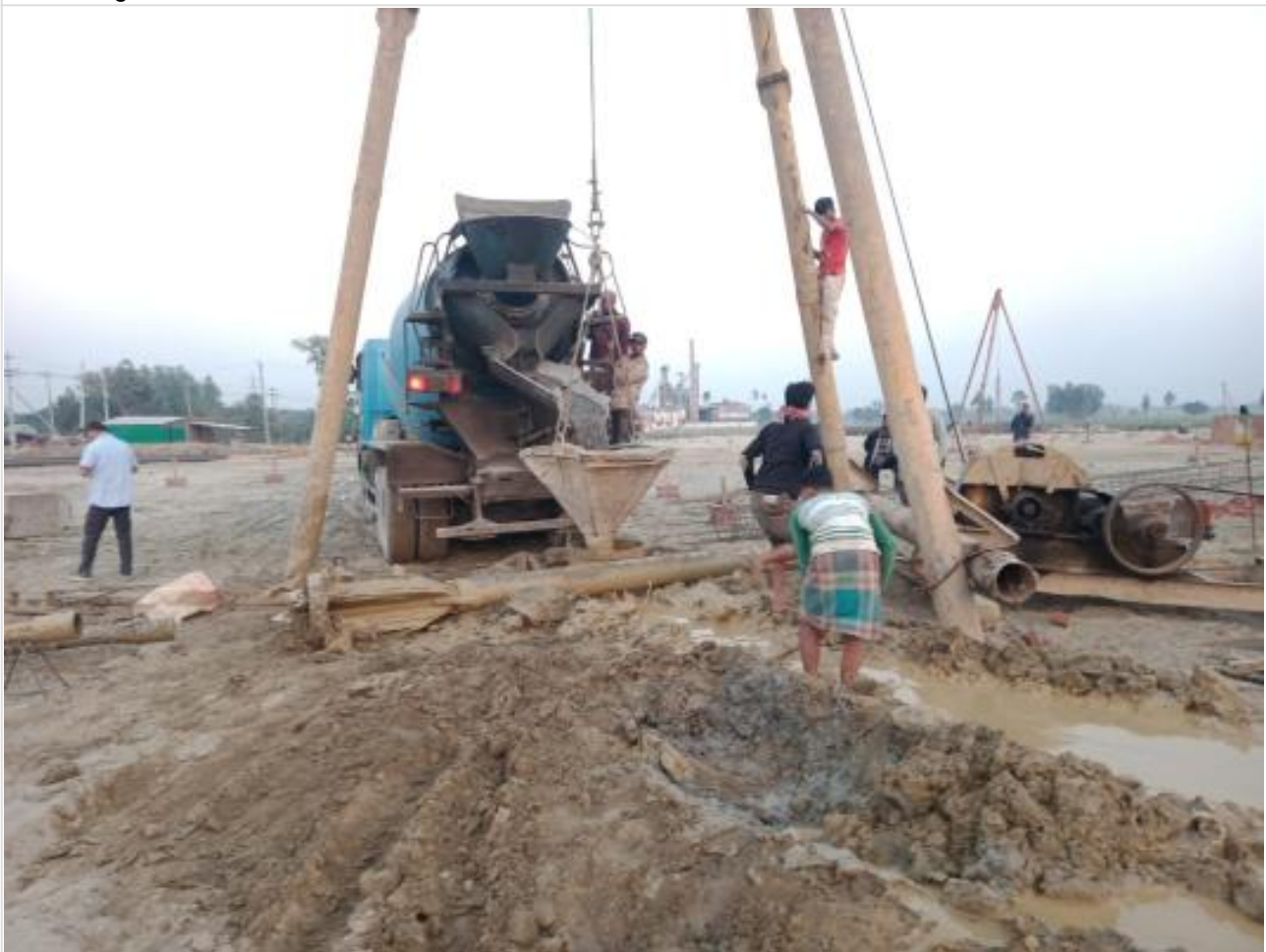
Ready mix concreting of pile on 14-02-23
