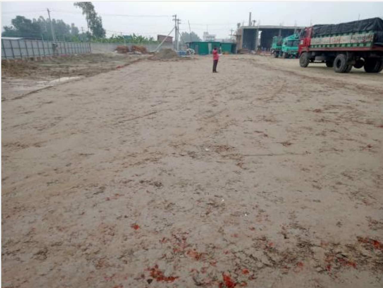
Road work on 13-09-23
