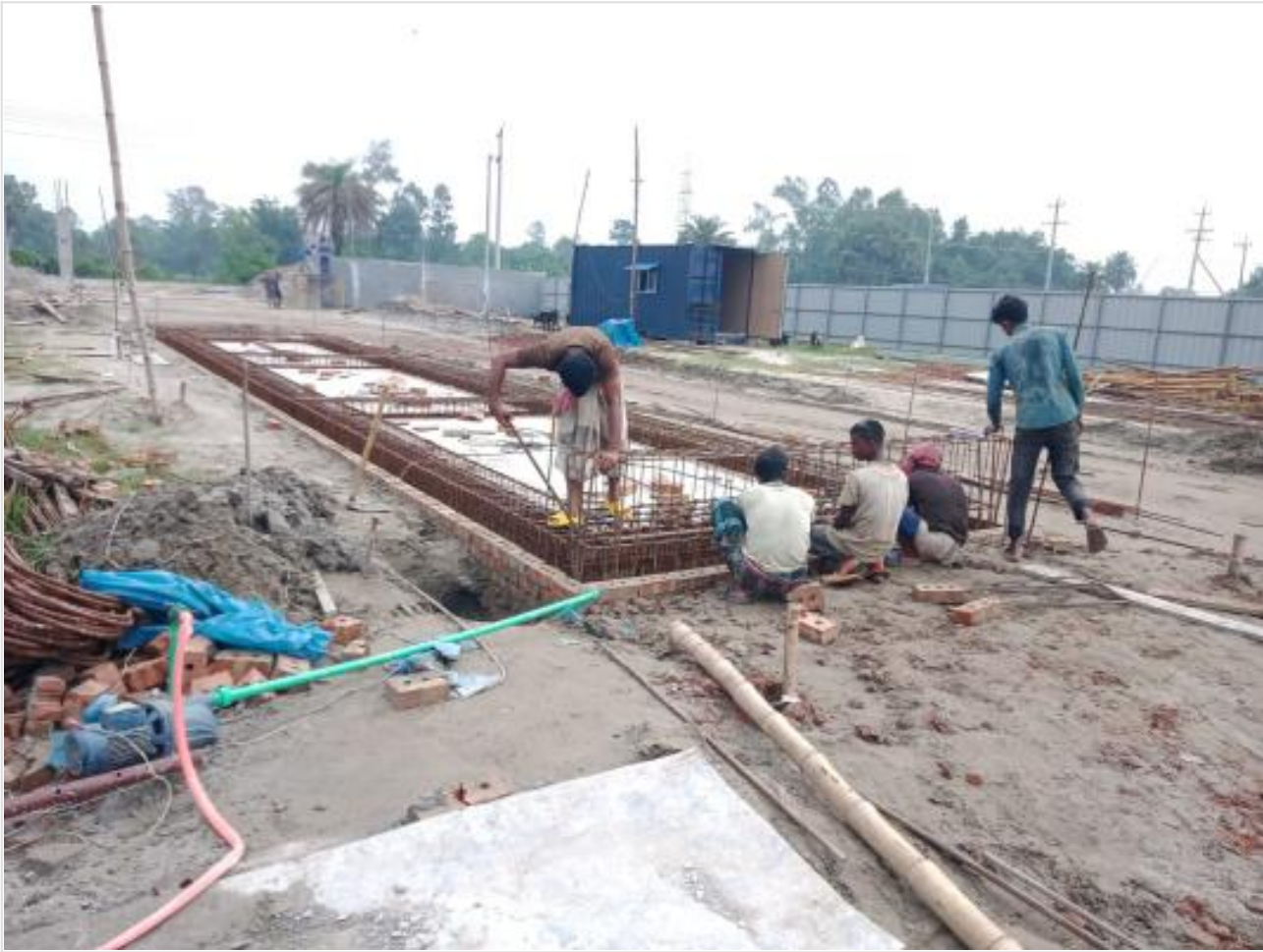
Weighing bridge re-bar work on 11-08-23
