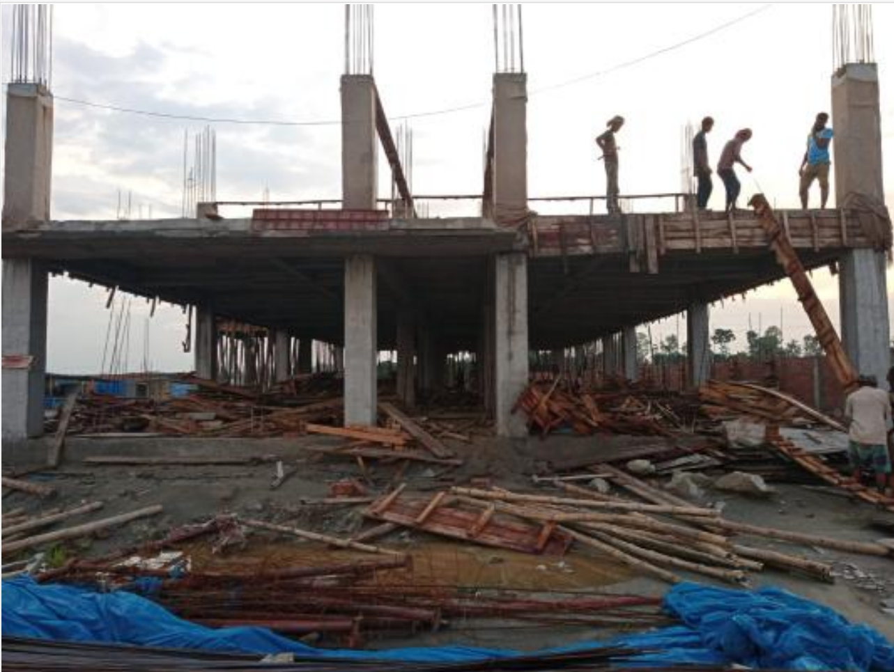
Comp. Bldg. 1st floor column work on 14-07-23
