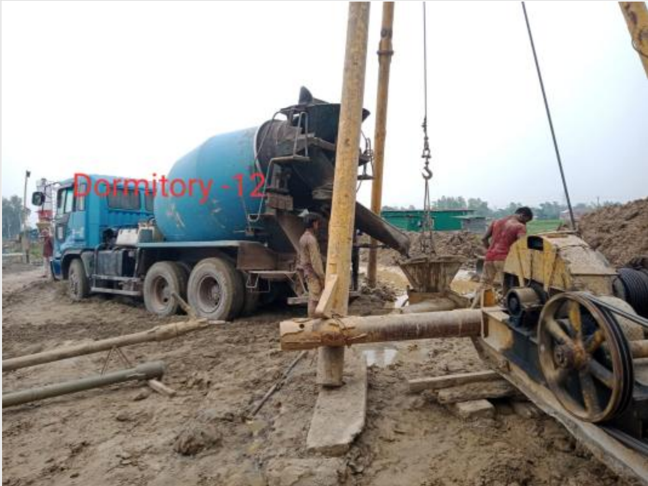
Ready mix concreting of pile on 31-03-23
