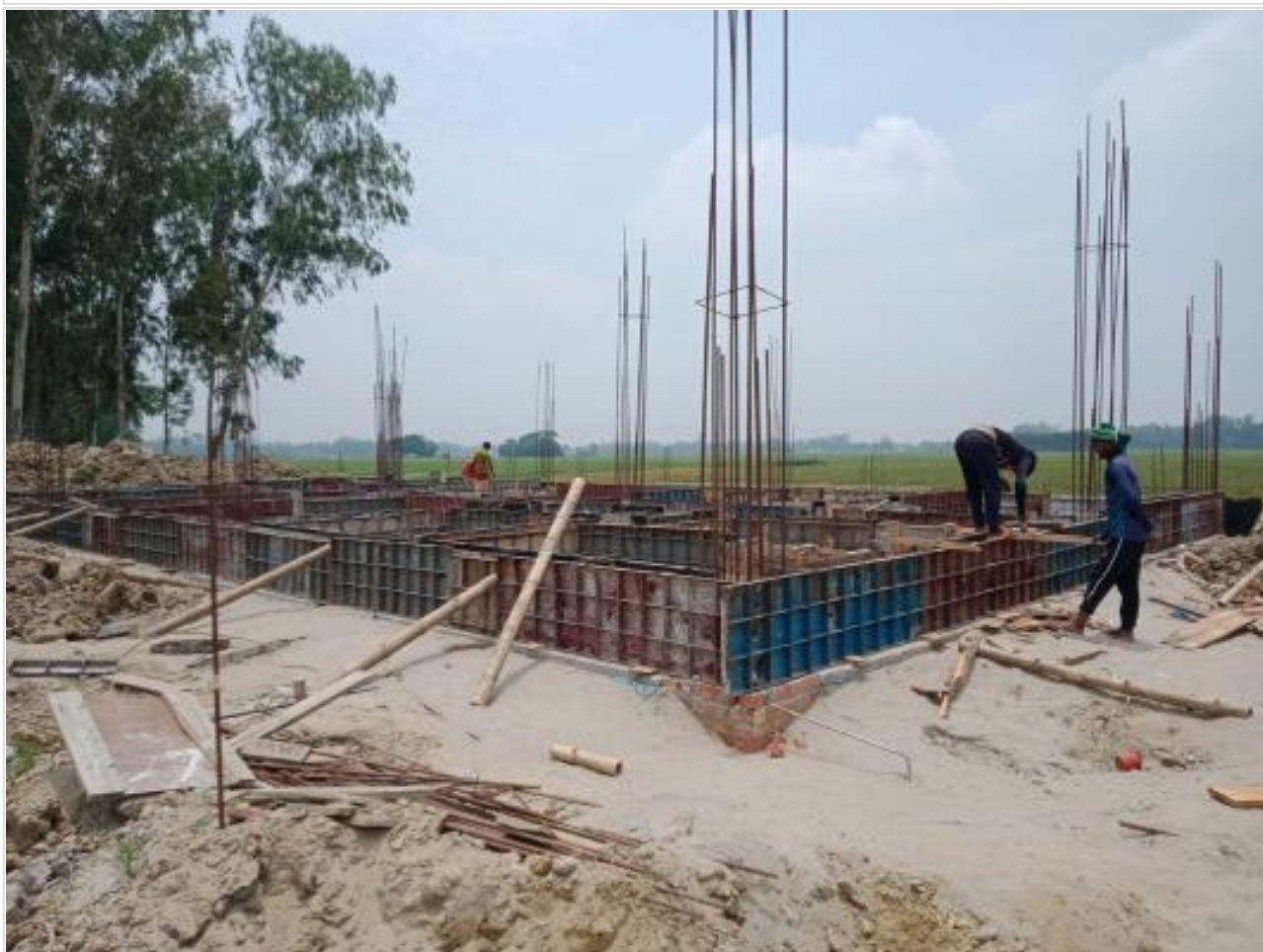
Dorm. Bldg. GB shuttering on 09-06-23
