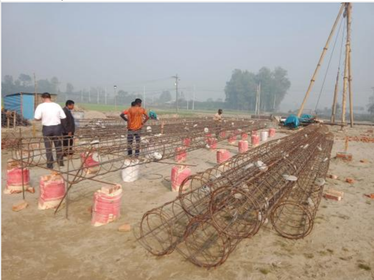
Pile Re-bar Work on 12-02-23
