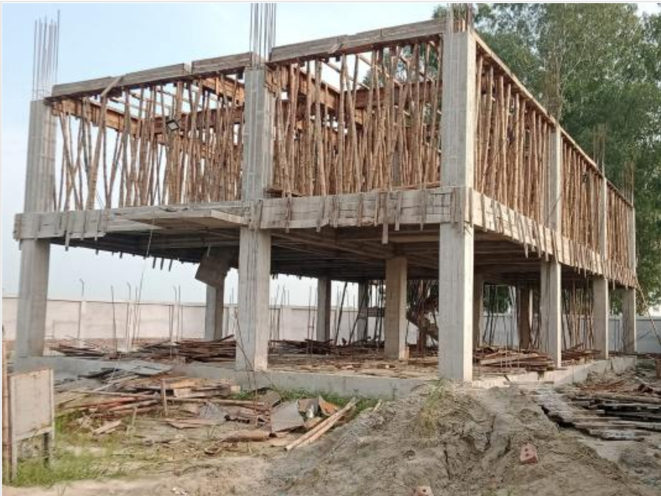
Dorm. Bldg. 2nd floor shuttering work on 03-09-23
