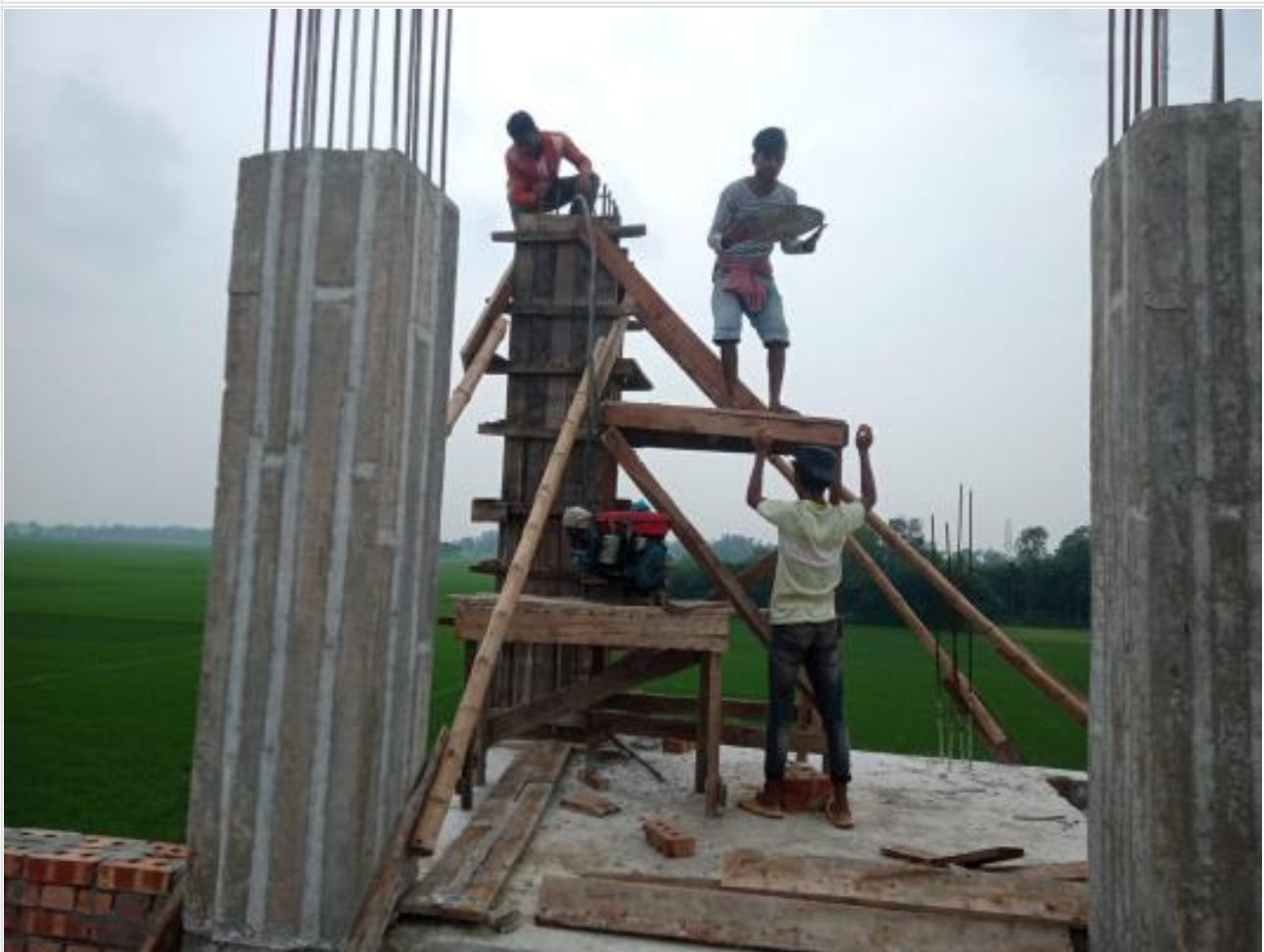
Comp. Bldg Column casting on 27-08-23
