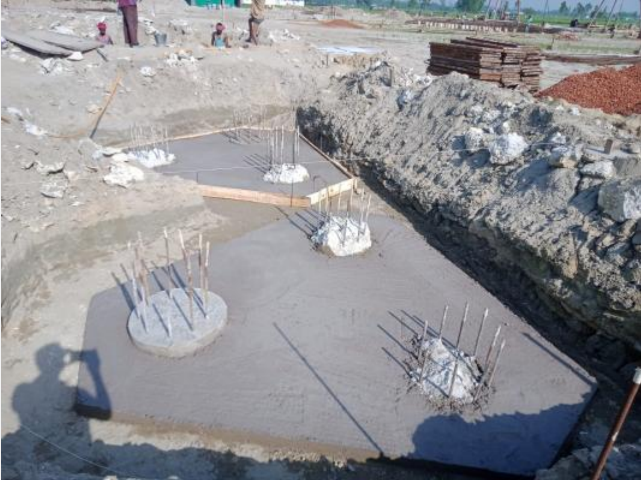
Pile cap CC work on 05-04-23
