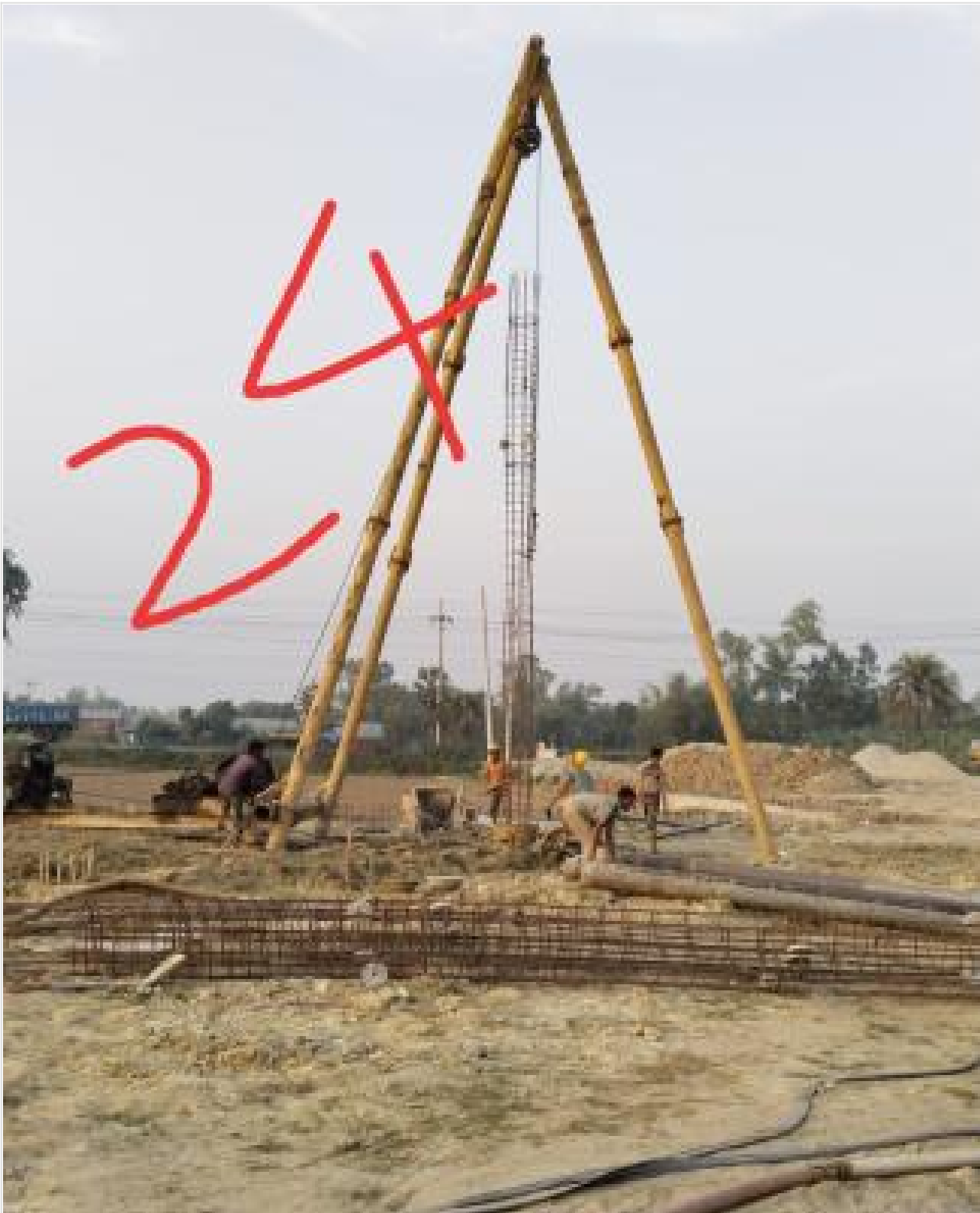
Com. Bldg. 24th pile boring on 24-02-23
