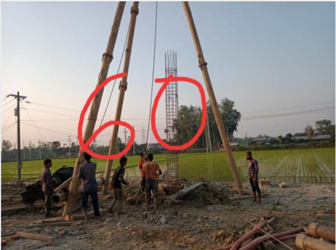
Ready mix concreting of pile on 12-03-23
