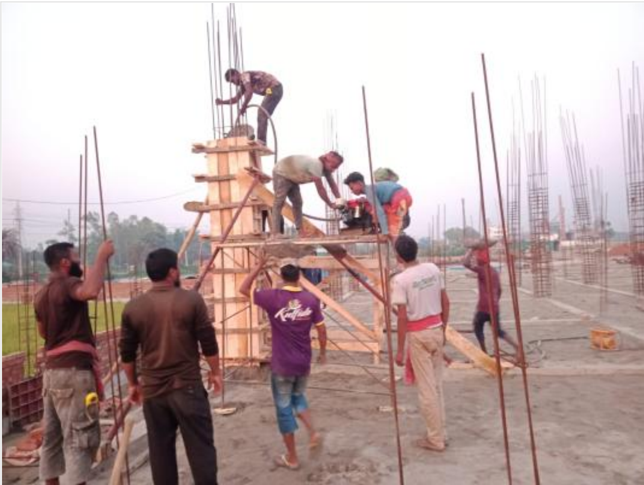
Comp. Bldg column casting on 28-05-23
