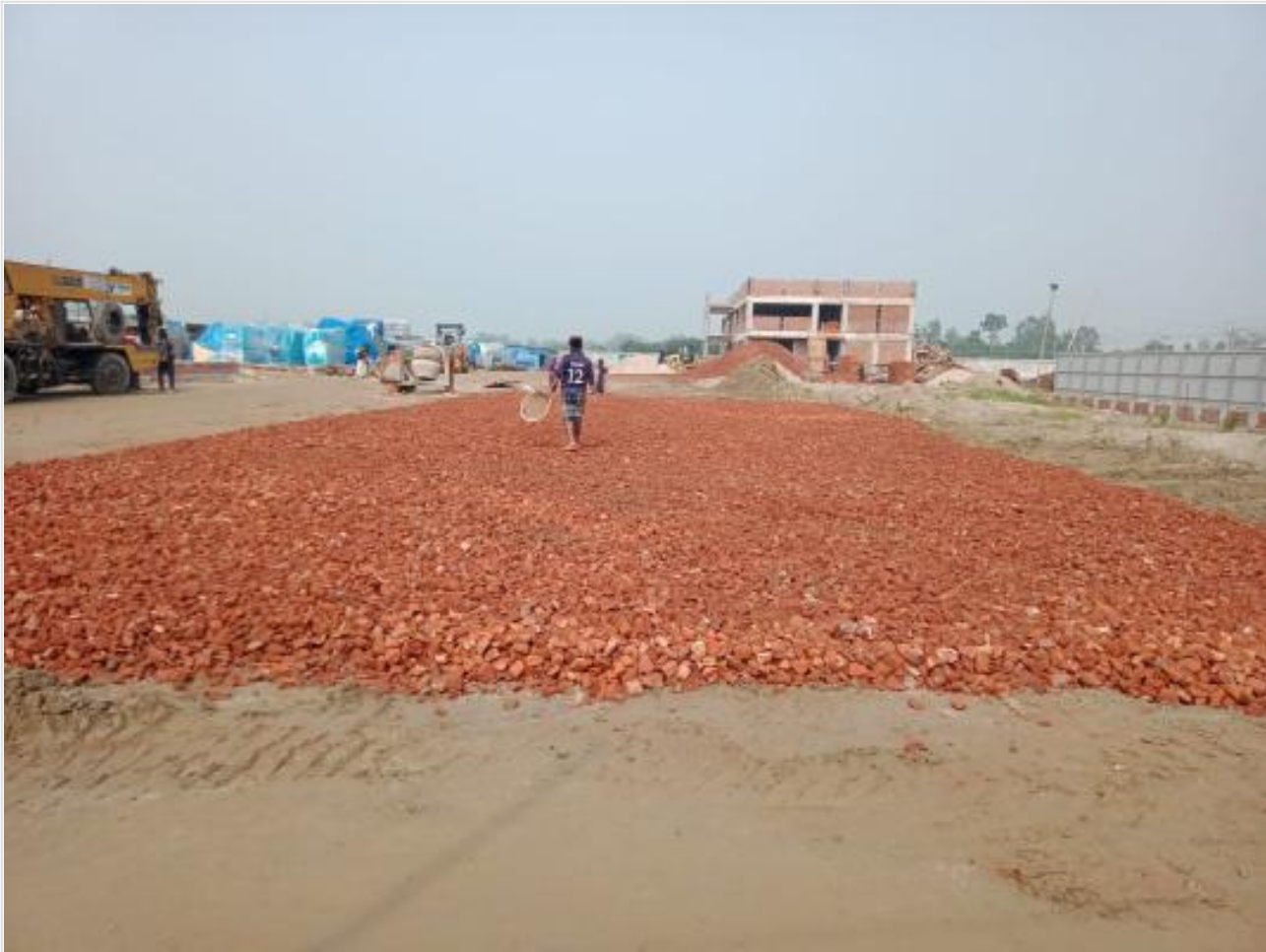
Road Sub-base work on 01-09-23
