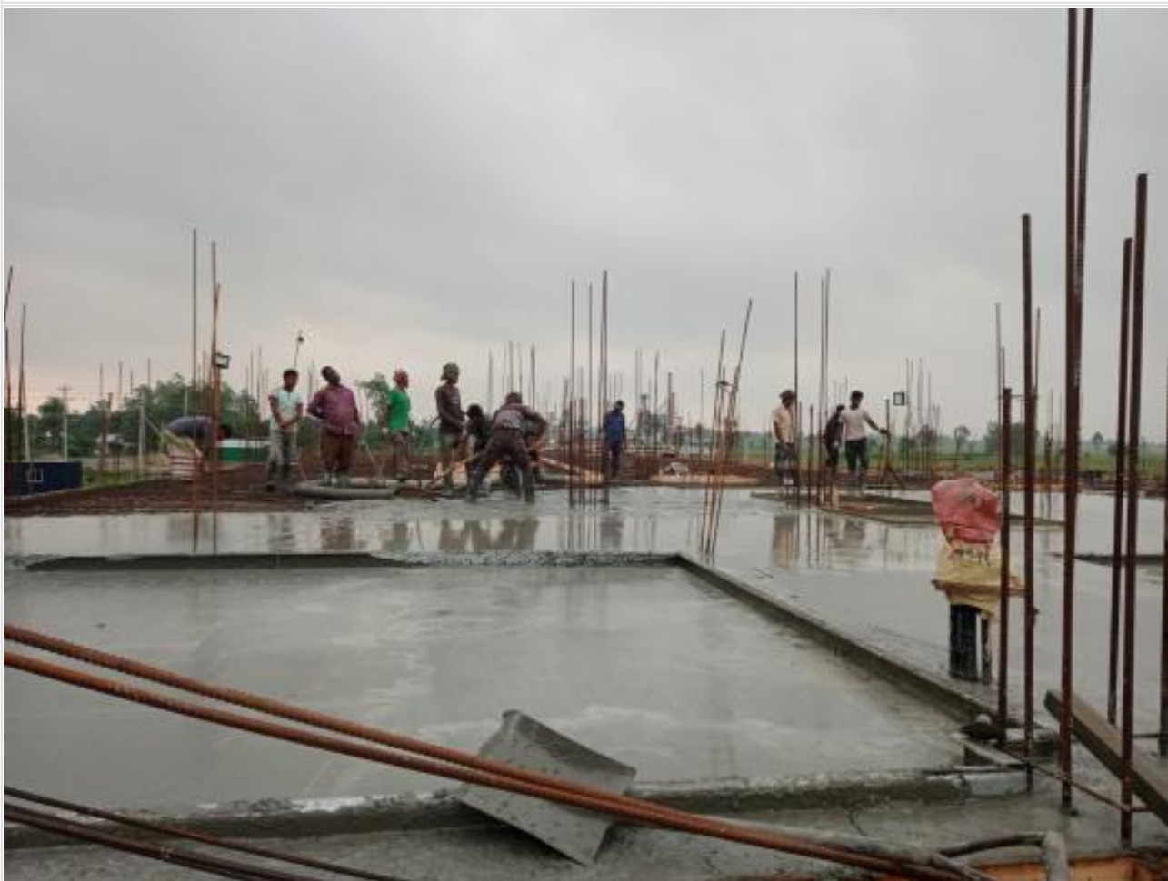
Com. Bldg. 1st floor slab casting on 27-06-23
