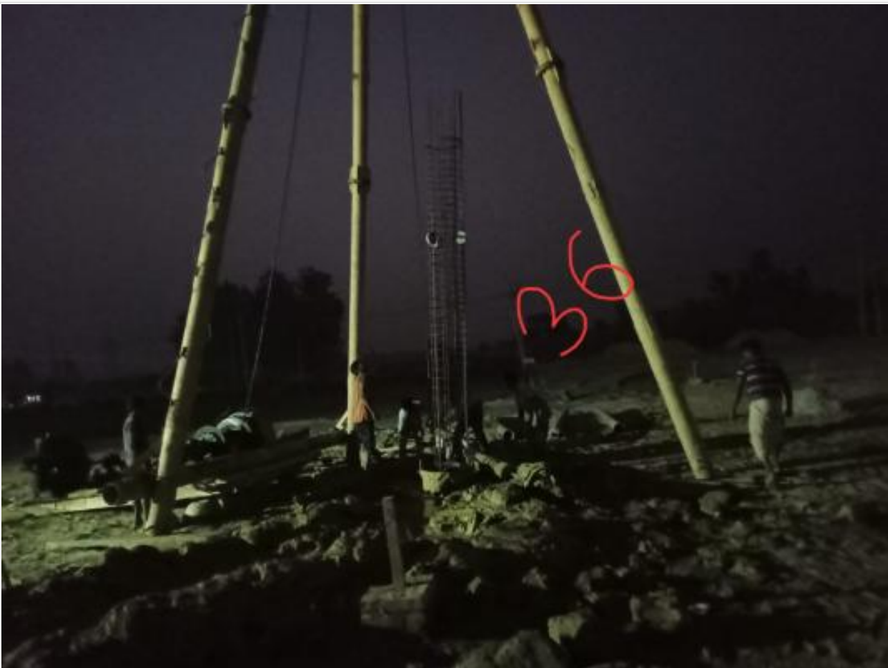
Com. Bldg. 36 Pile Boring on 28-02-23
