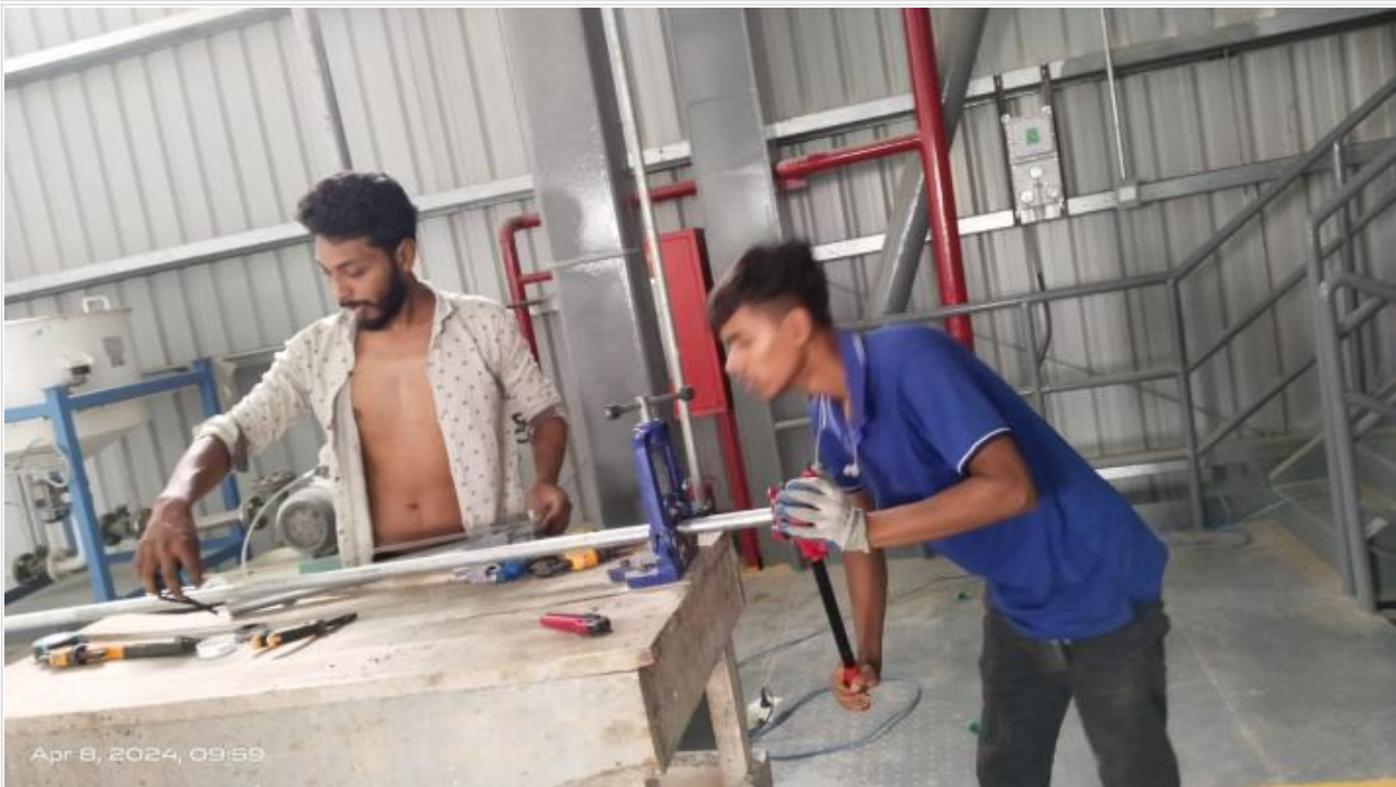
Electrical Work on 08-04-24
