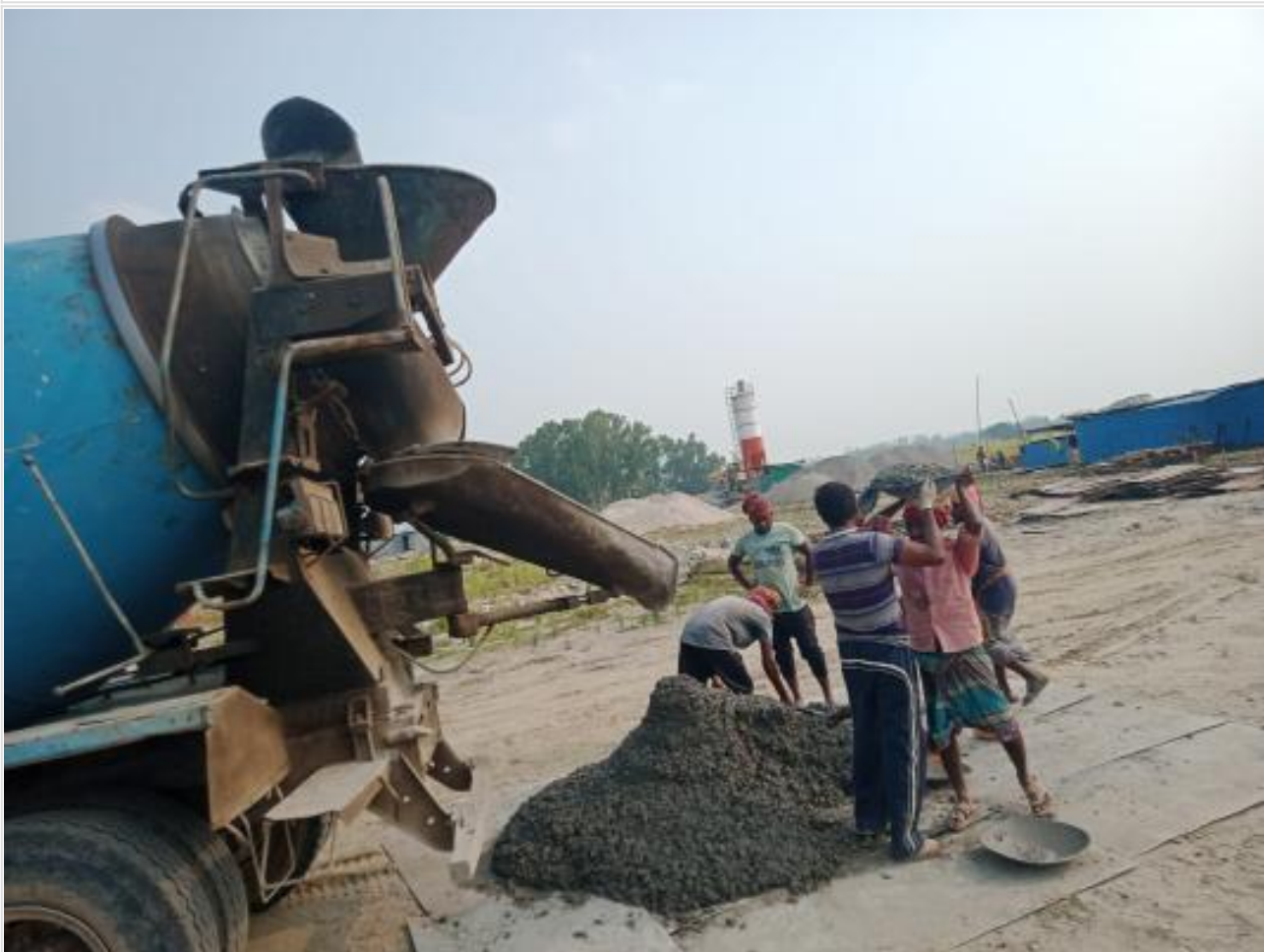
Comp. Bldg. GB casting work on 16-05-23
