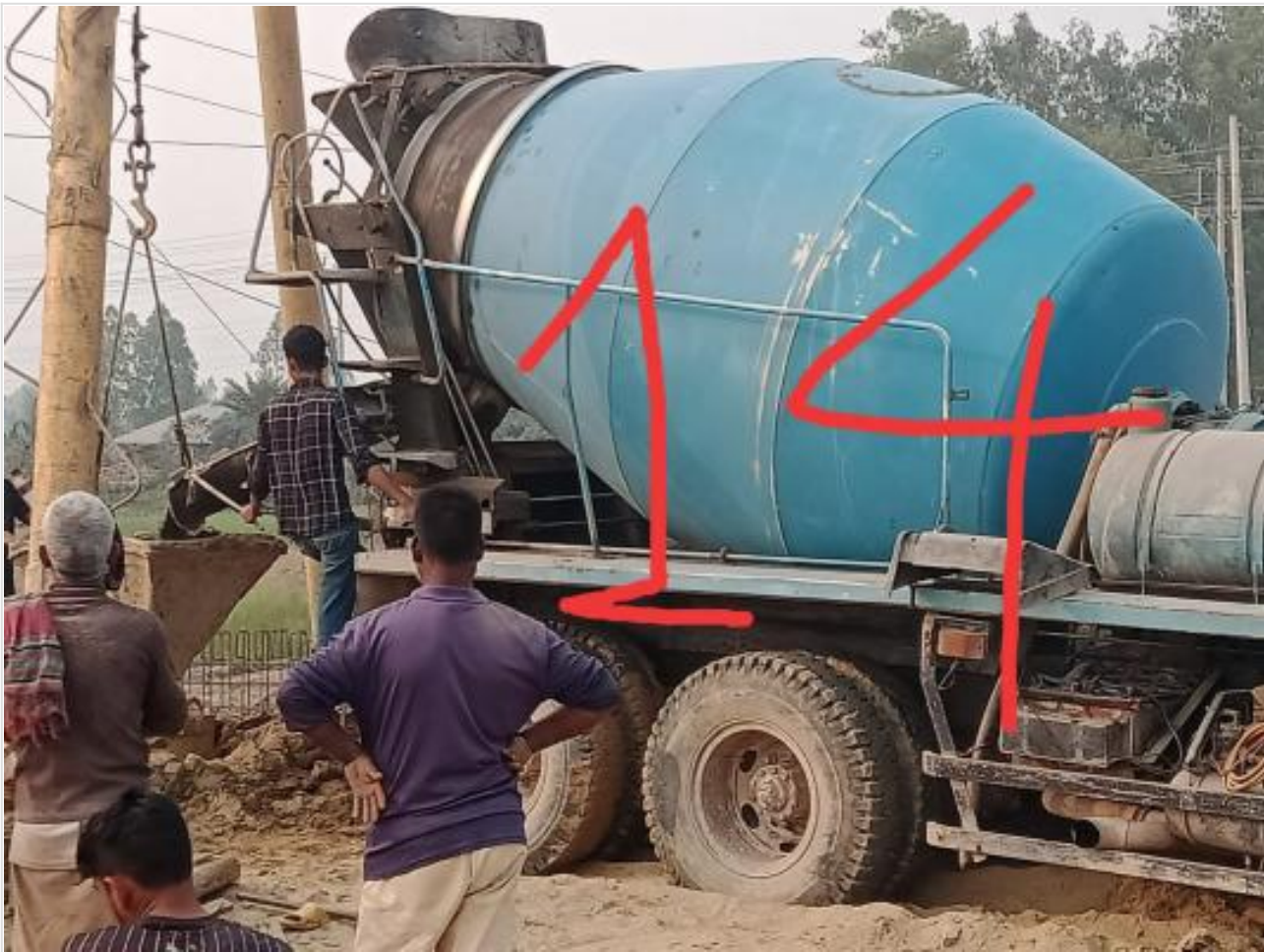
Ready mix concreting of pile on 18-02-23
