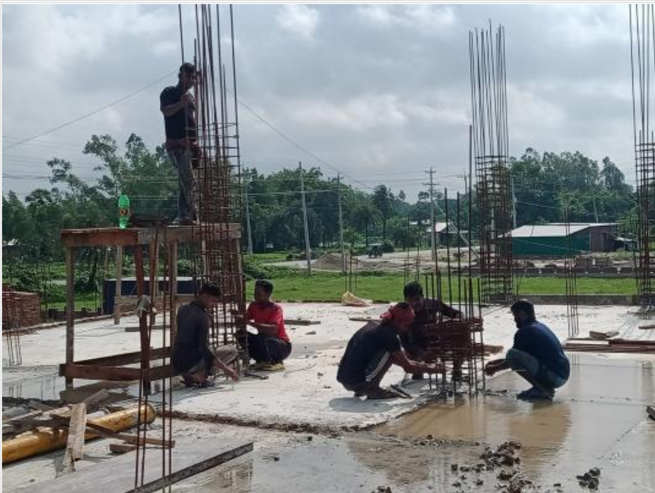
Comp. Bldg. 1st floor column work on 07-07-23
