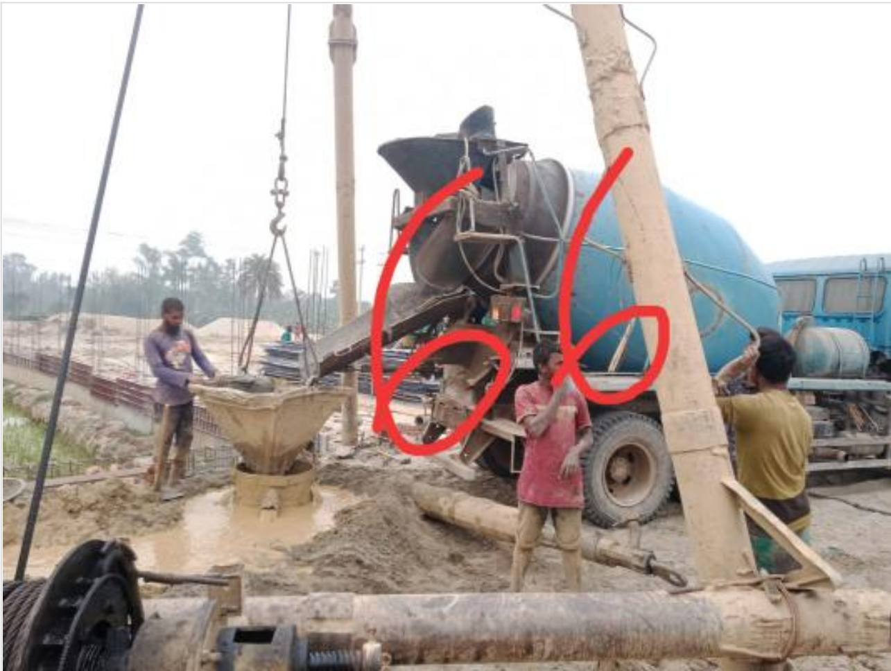
Ready mix concreting of pile on 16-03-23
