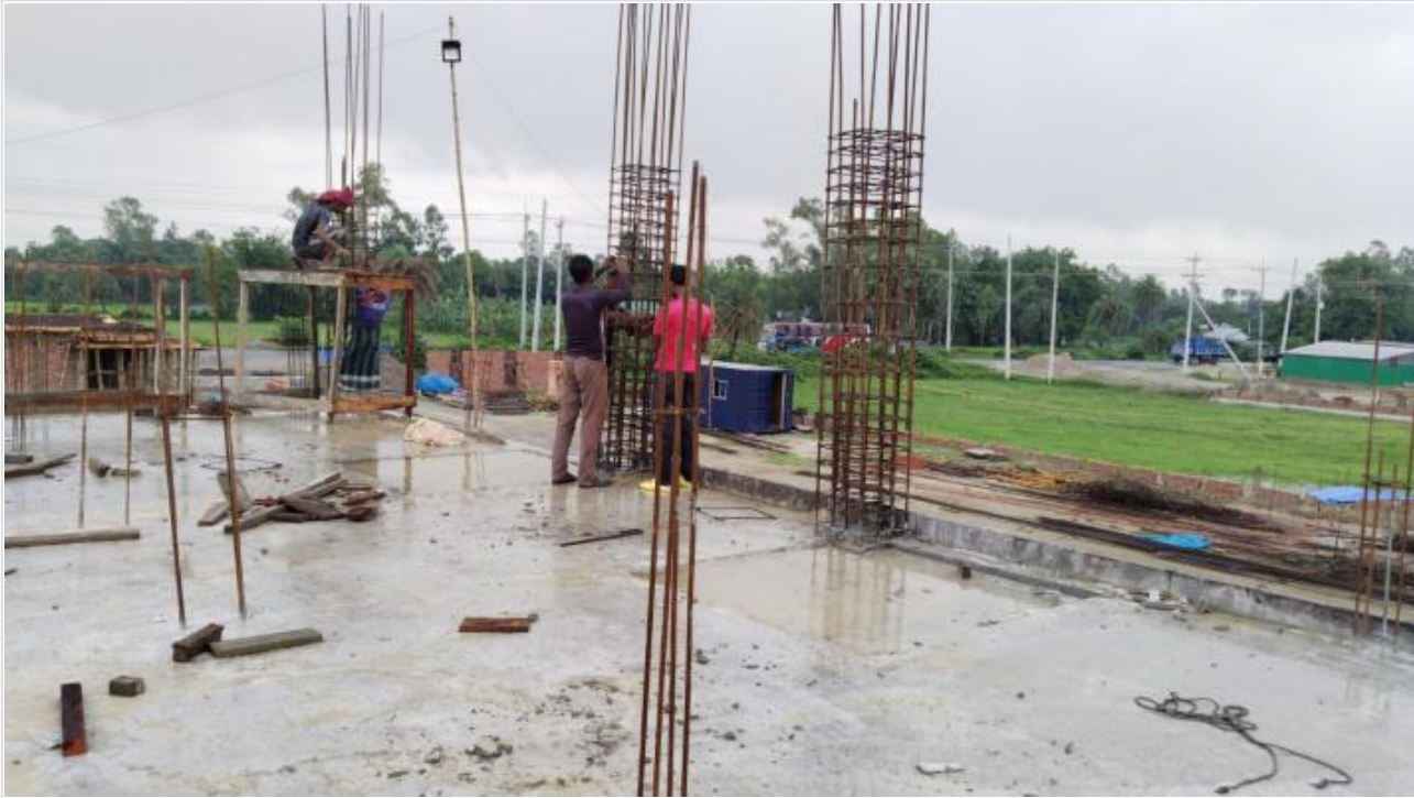
Comp Bldg-1st floor Column Re-bar work on 06-07-23
