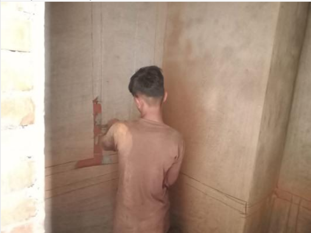
Sanitary group cutting on 06-11-23
