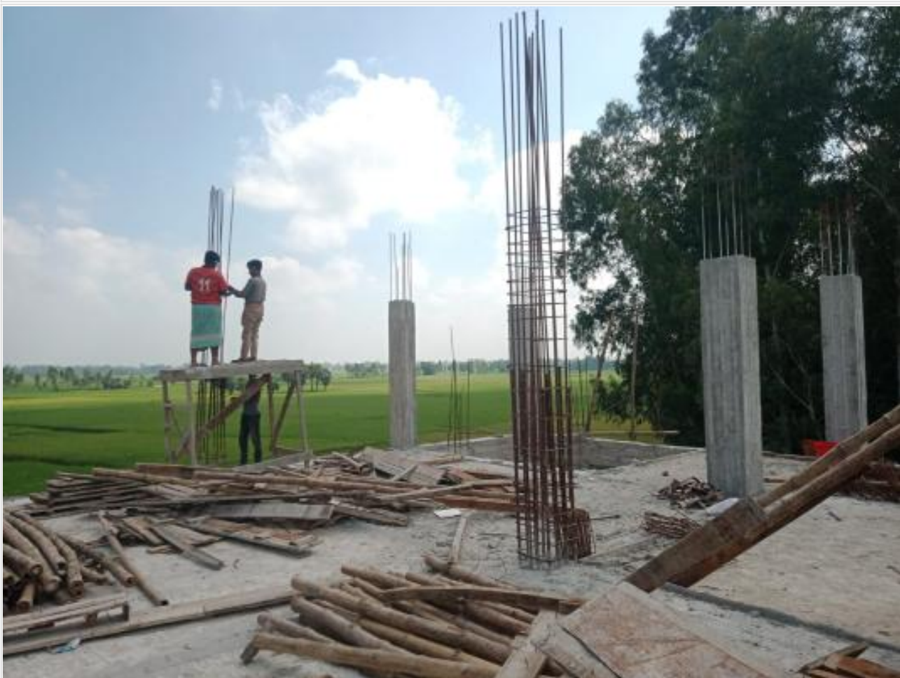
Dorm. Bldg. 2nd floor column work on 25-10-23
