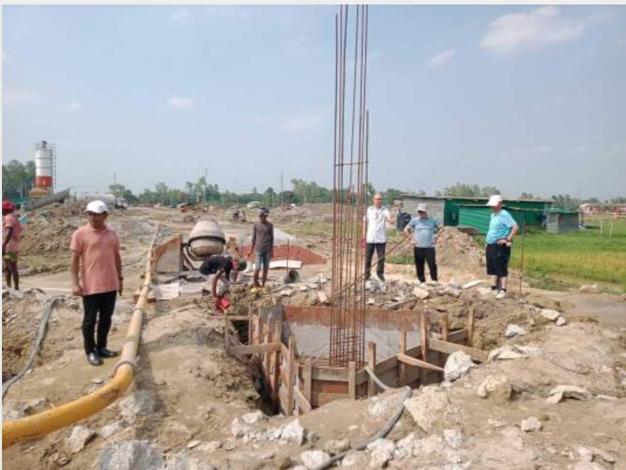
Dorm. Bldg pile cap work on 26-05-23
