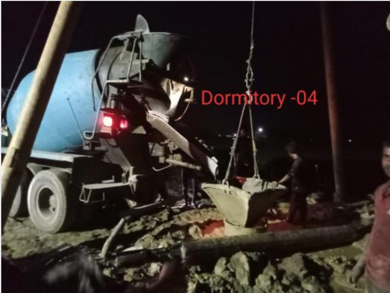
Ready mix concreting of pile on 26-03-23
