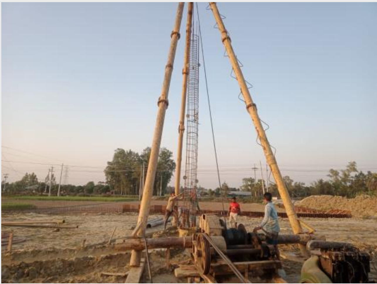
Pile boring work on 13-02-23
