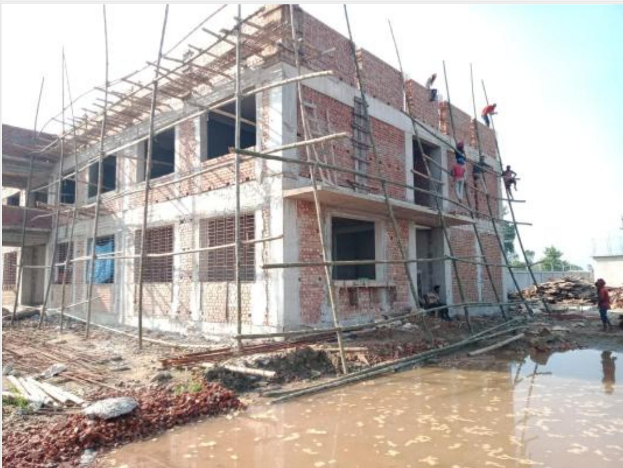
Comp. Bldg outside scaffolding on 28-09-23
