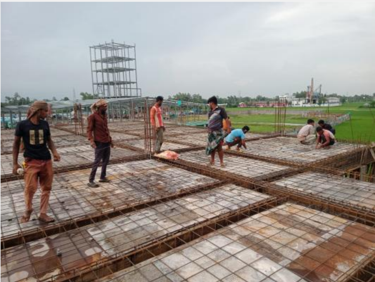
Dorm. Bldg. 2nd floor rebar work on 08-09-23
