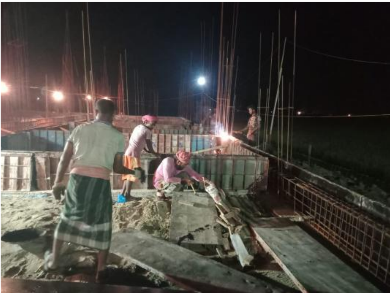
Com. GB Shuttering on 13-05-23
