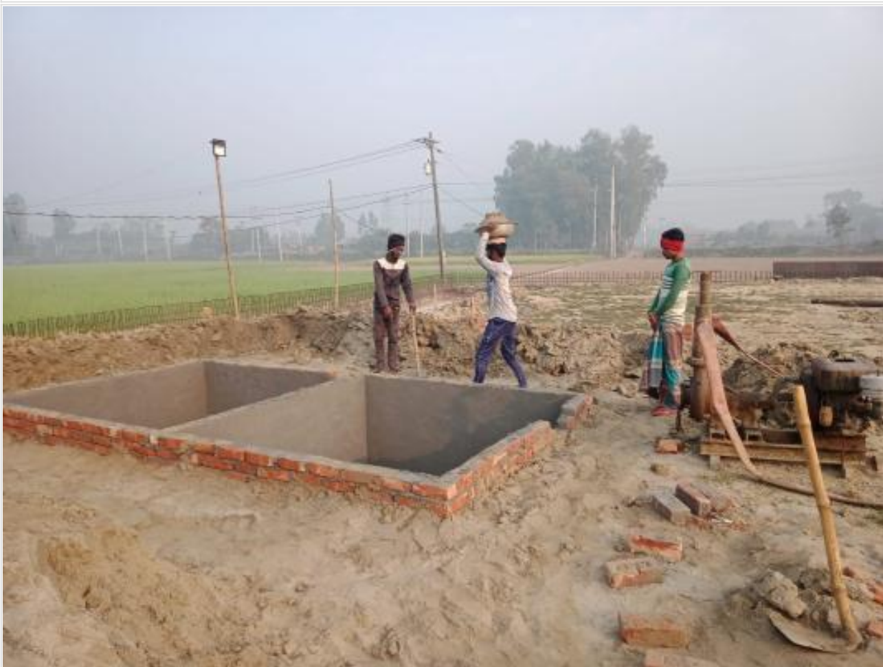
Mud Tank-1 Completed on 08-02-23
