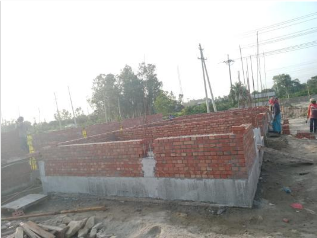
Gate house Brick work on 01-06-23
