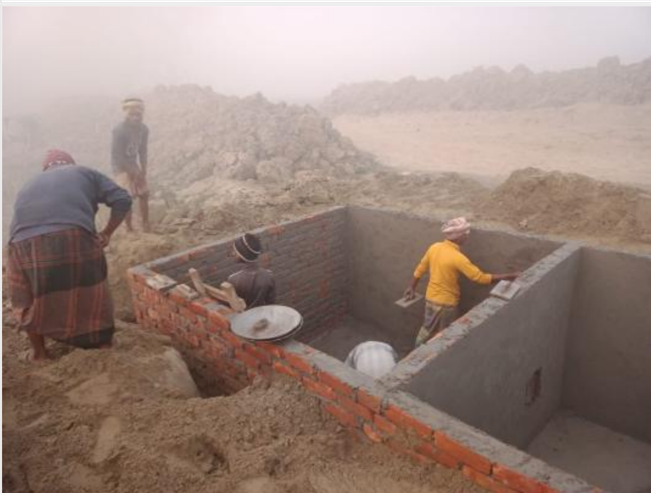
Mud Tank-2 Completed on 12-02-23
