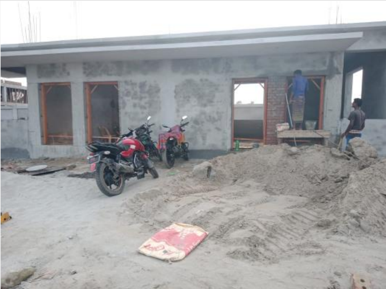
Gate House-Door Frame Fixing on 20-08-23
