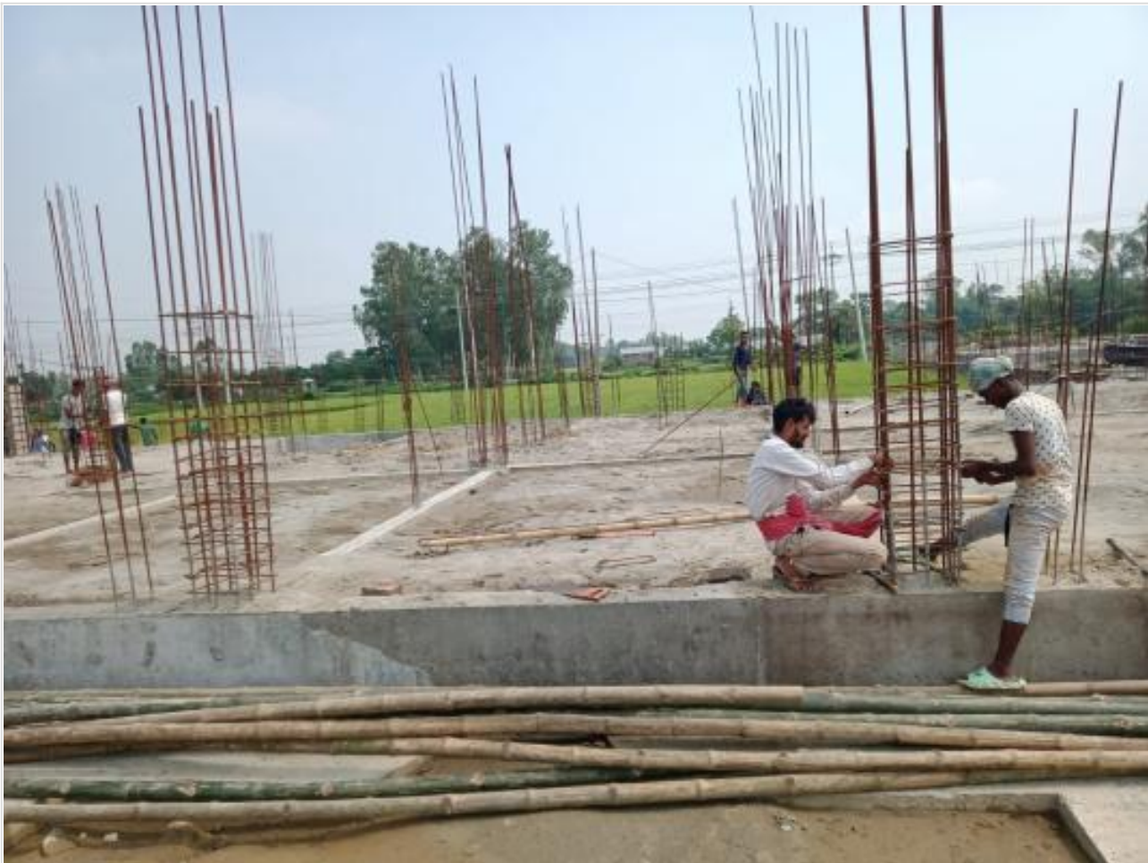
Comp. Bldg column work on 25-05-23
