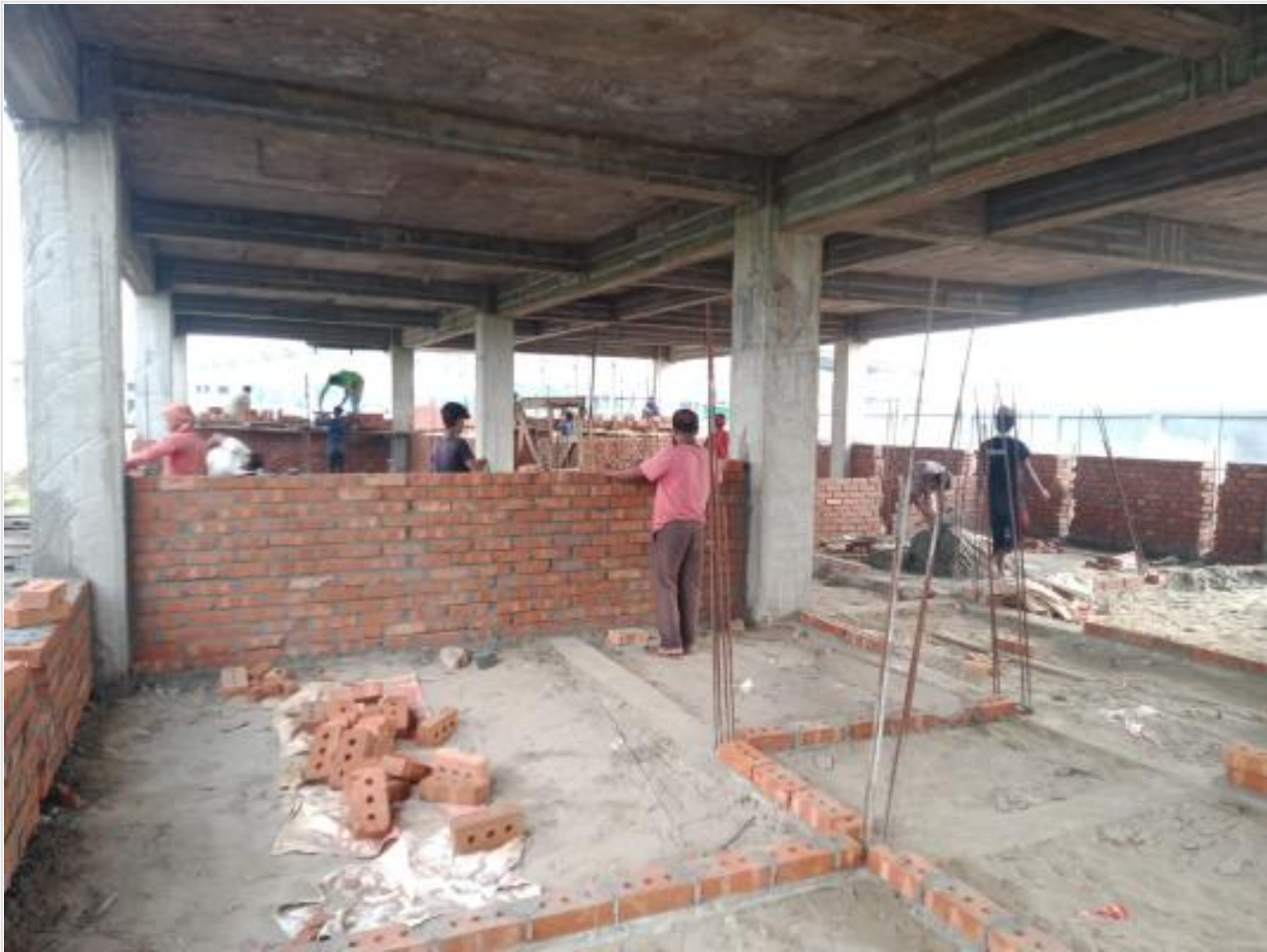
Dorm.Bldg brick work on 23-09-23
