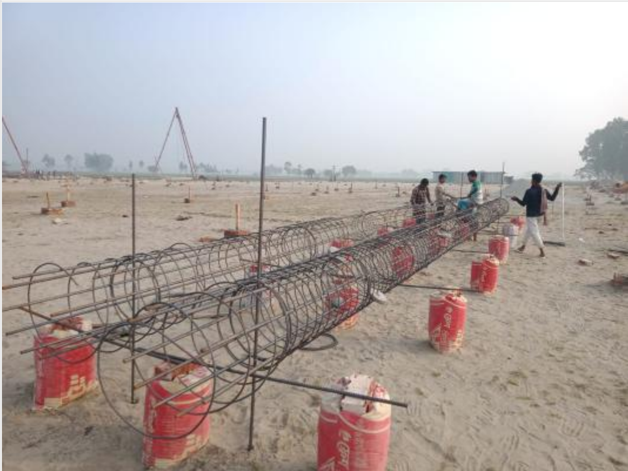
Pile Re-bar Work on 05-02-23
