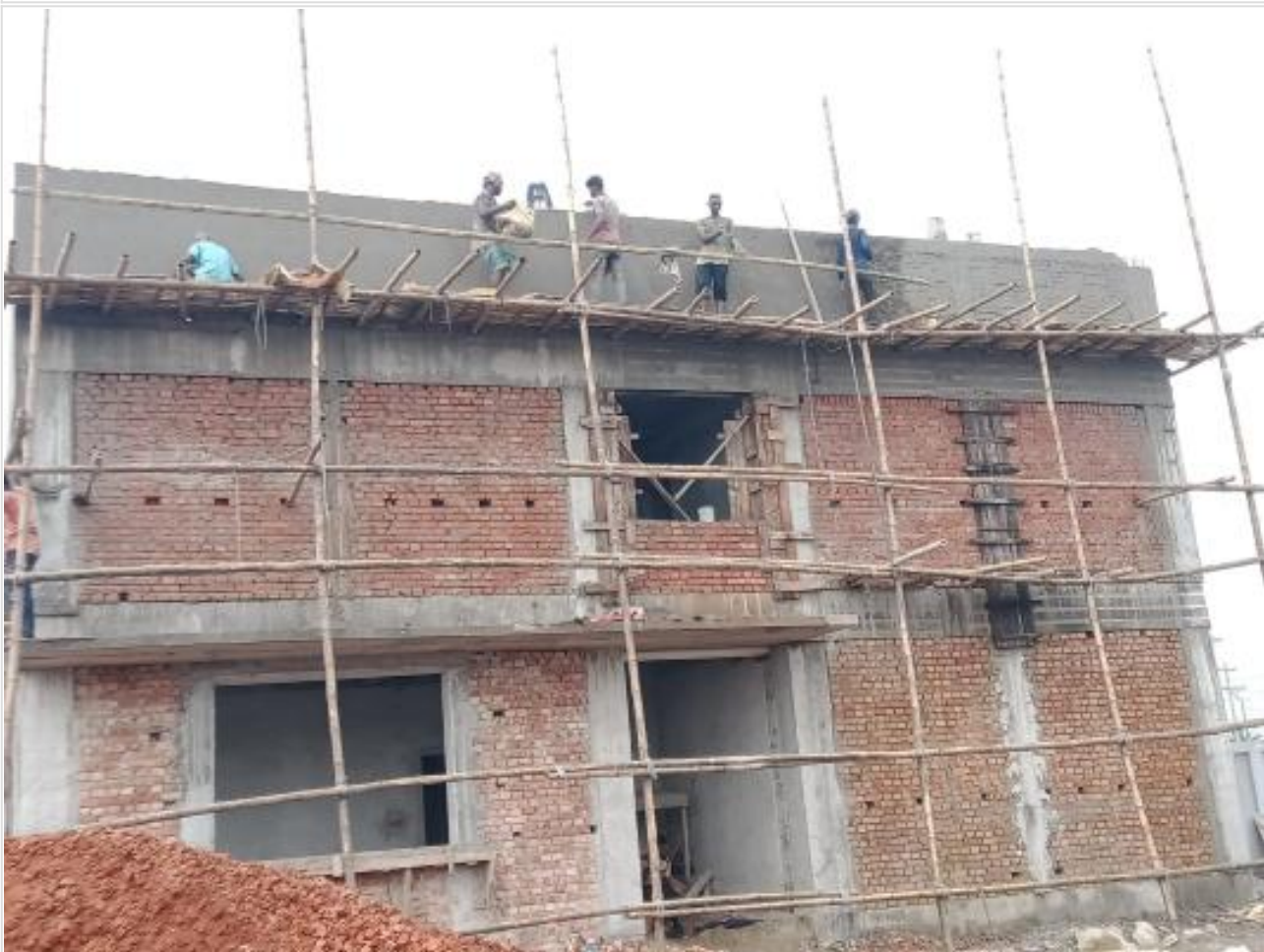
Comp. Bldg. Outside plaster work on 11-10-23
