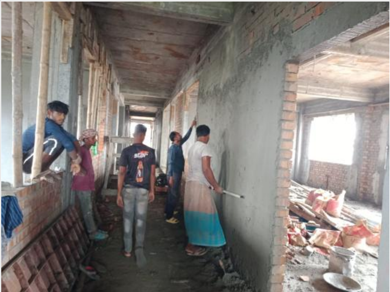
Comp. Bldg. GF plaster work on 27-08-23
