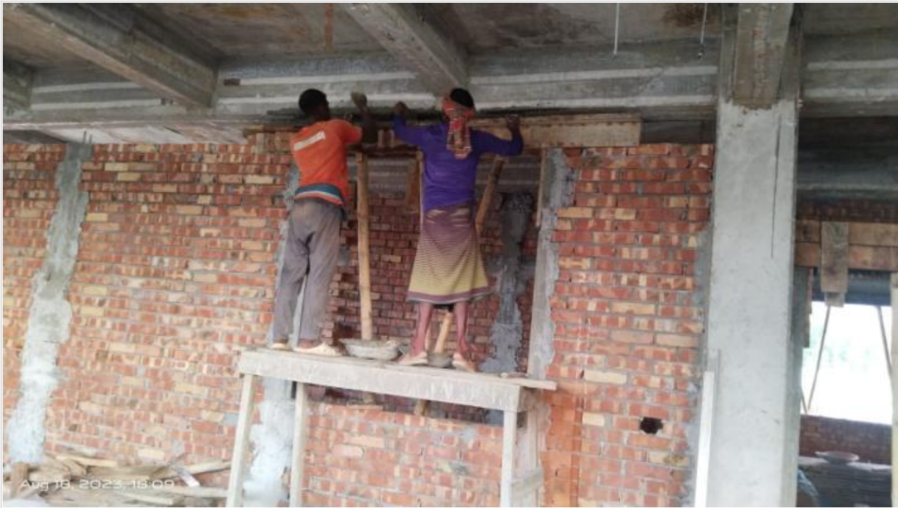
Comp-GF Brickwork on 18-08-23
