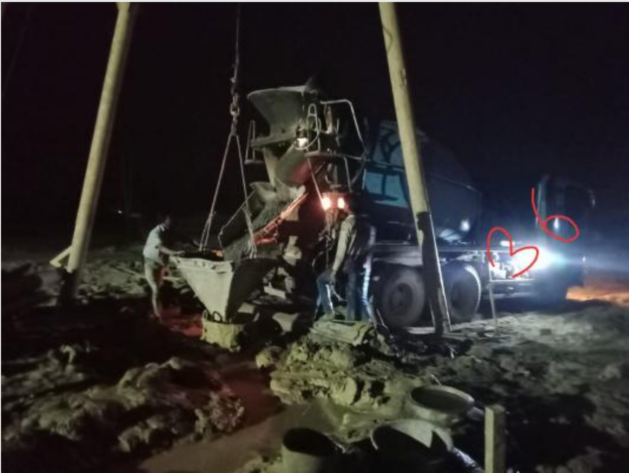
Ready mix concreting of pile on 28-02-23
