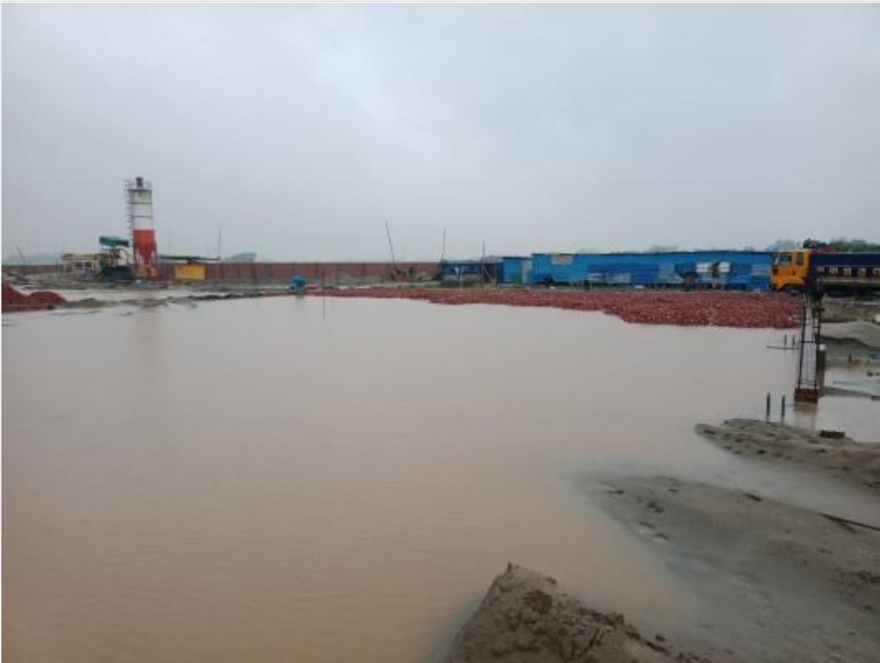
No work due to rain on 08-08-23
