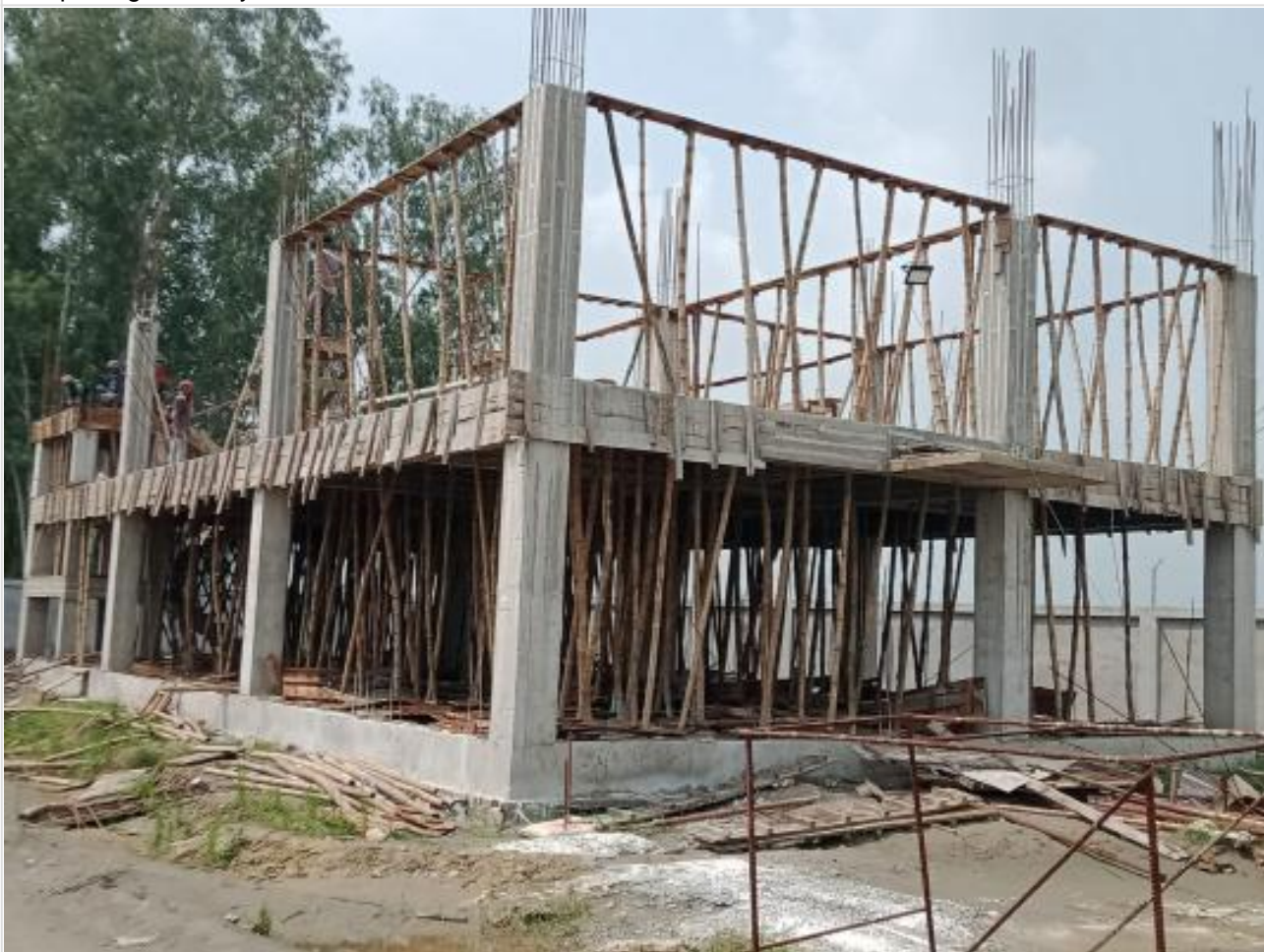
Dorm. Bldg. 2nd floor shuttering on 29-08-23
