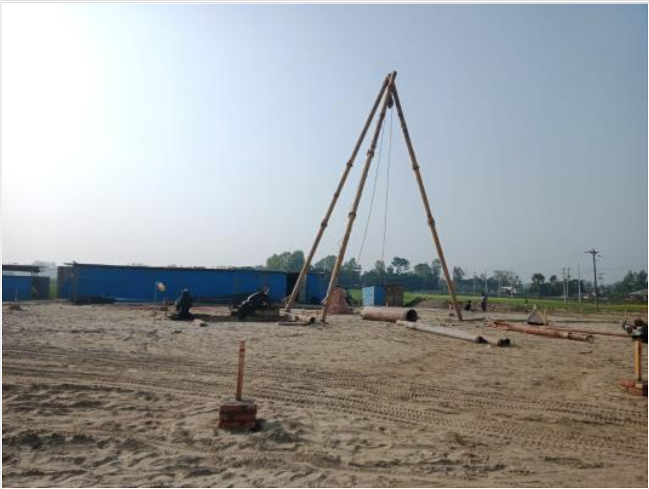
Pile Rig setting on 03-02-23
