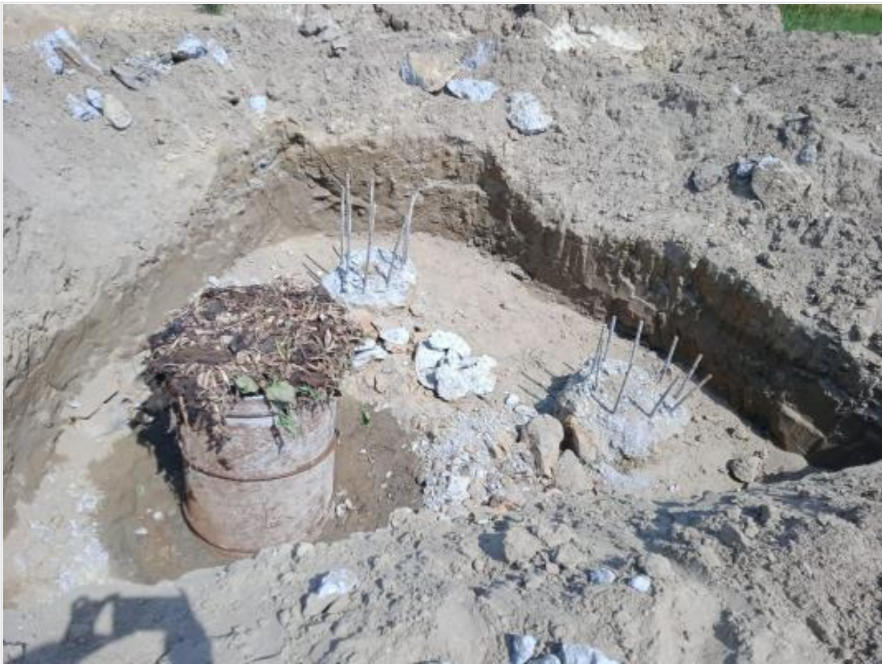
Pile head breaking on 10-05-23
