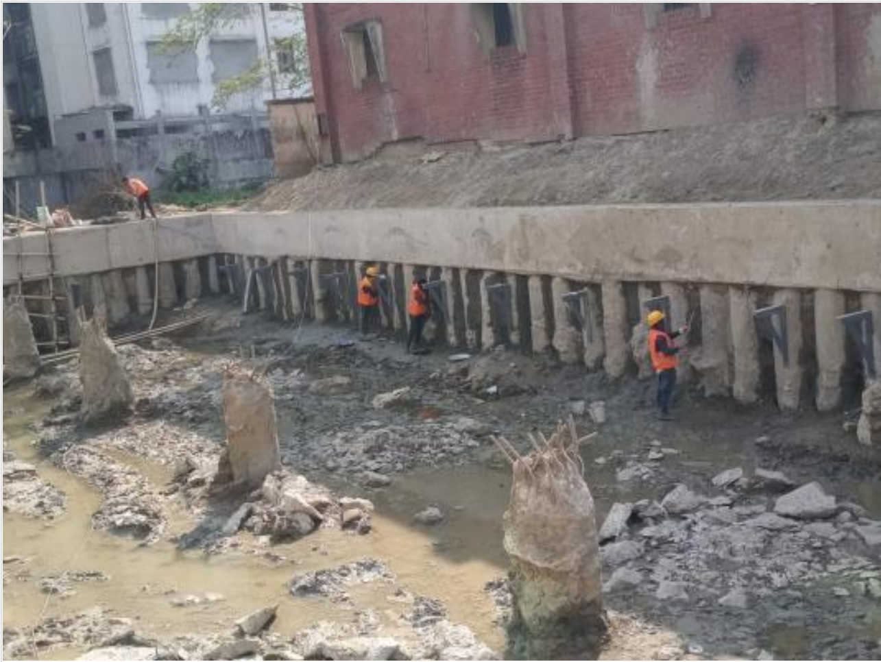
Shore pile Mortering on 16-03-22
