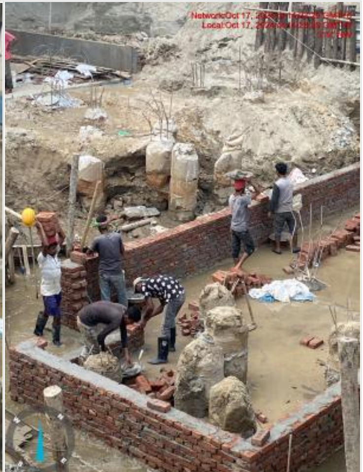
Water tank base brick wall shuttering
