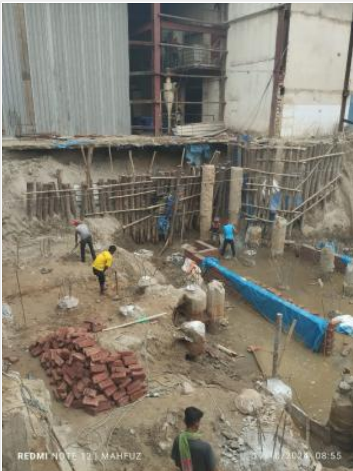
Pile head breaking
