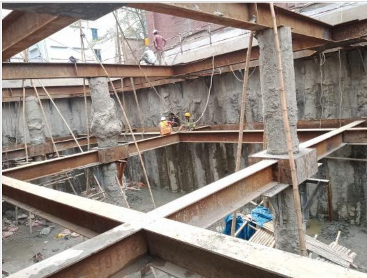
Water proofing work
