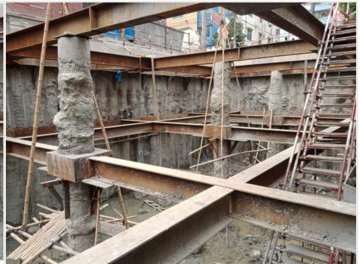
Pile gap water proofing
