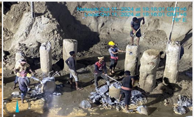
Pile head breaking on 11-10-24
