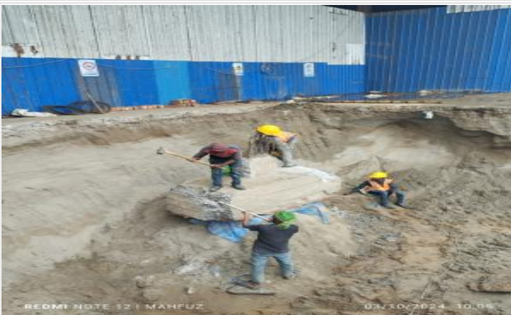
Obstacle RCC dismantling on 03-10-24
