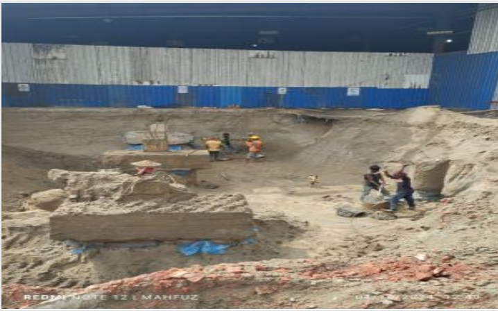
Pile Head breaking on 04-10-24
