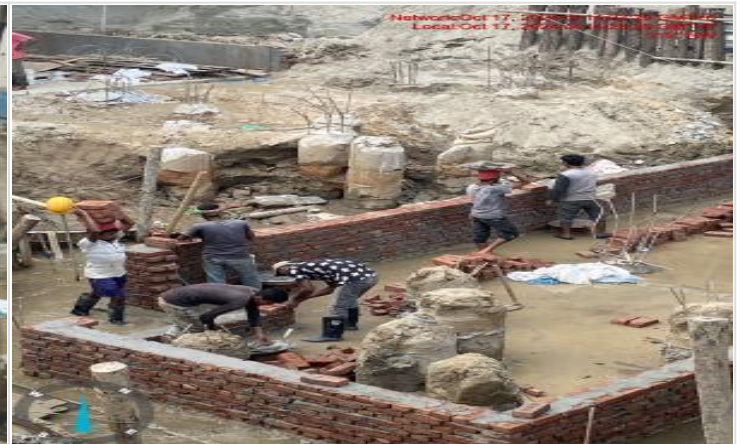
Water tank base brick wall shuttering on 17-10-24
