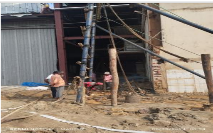
Wooden shore pile driving on 06-10-24
