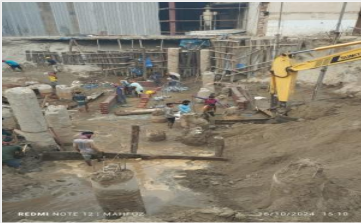
Excavation, brick-shuttering, steel shut on 16-10-24
