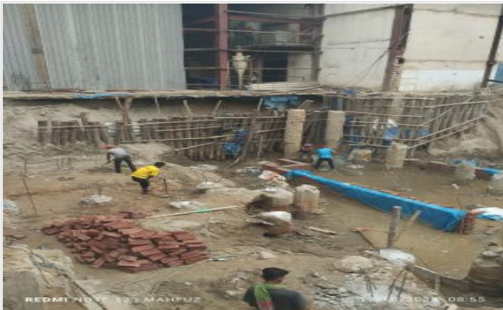
Pile head breaking on 17-10-24
