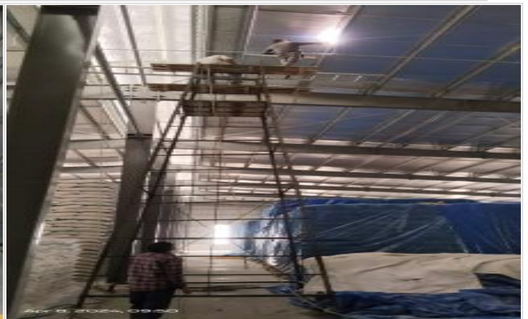
Electrical Work on 08-04-24
