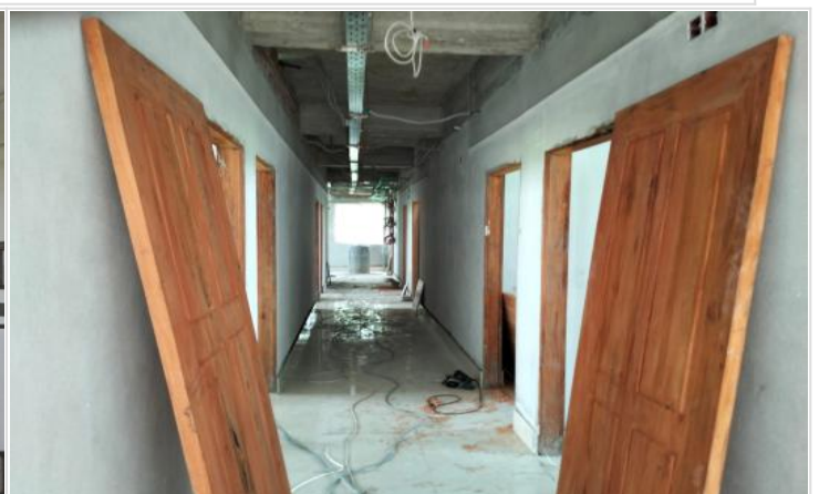
Dormitor-2nd Floor-Corridor on 23-04-24
