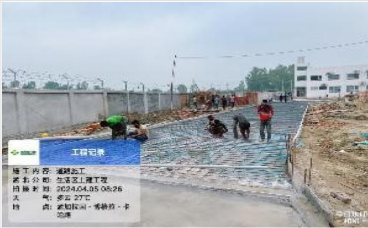
Road-Re-bar work on 05-04-24
