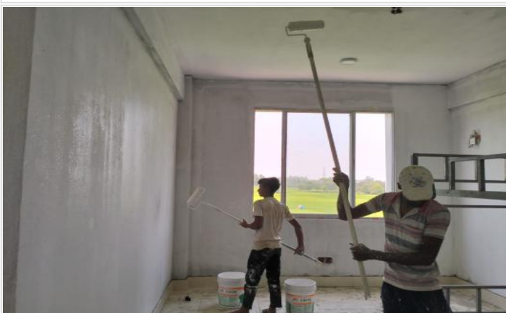
Dormitory-2nd Floor Painting on 23-04-24
