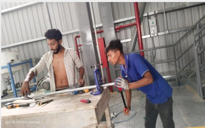
Electrical Work on 08-04-24
