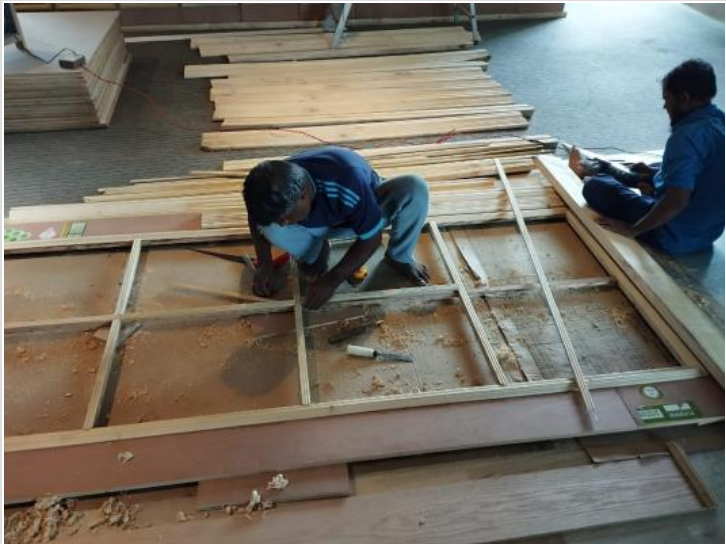
11th Floor Interior Work
