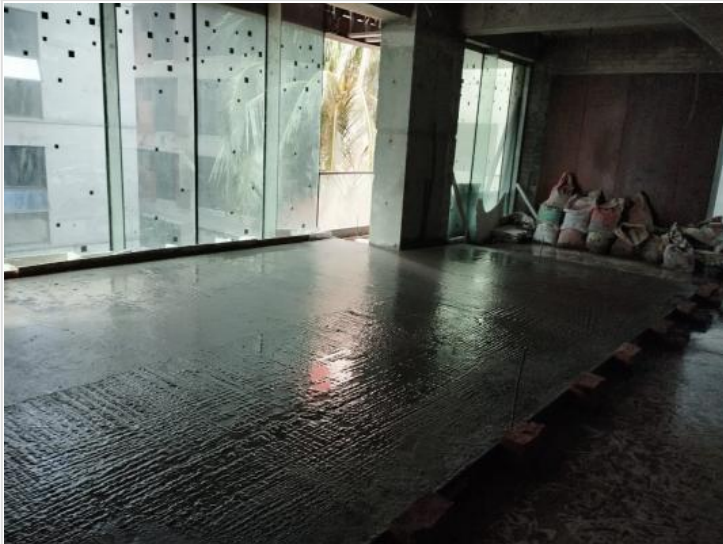
4th Flr-Floor Raining Concreting Complet
