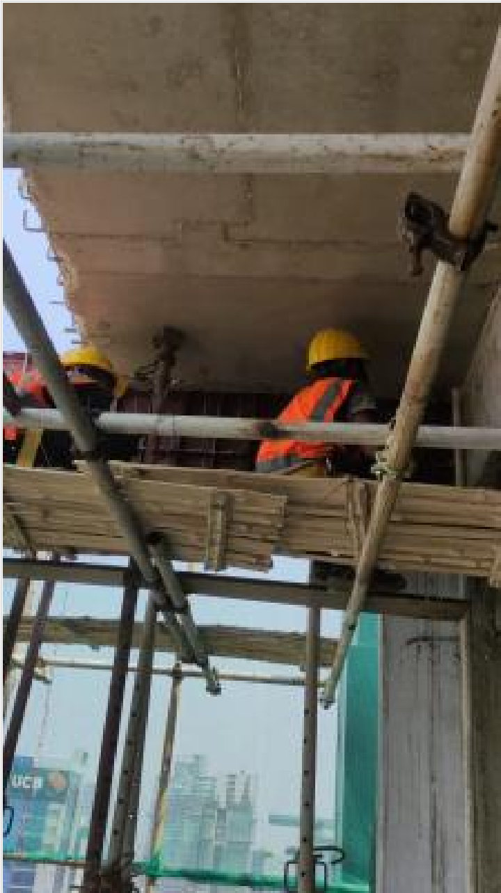
L-16-Beam Shutter removing
