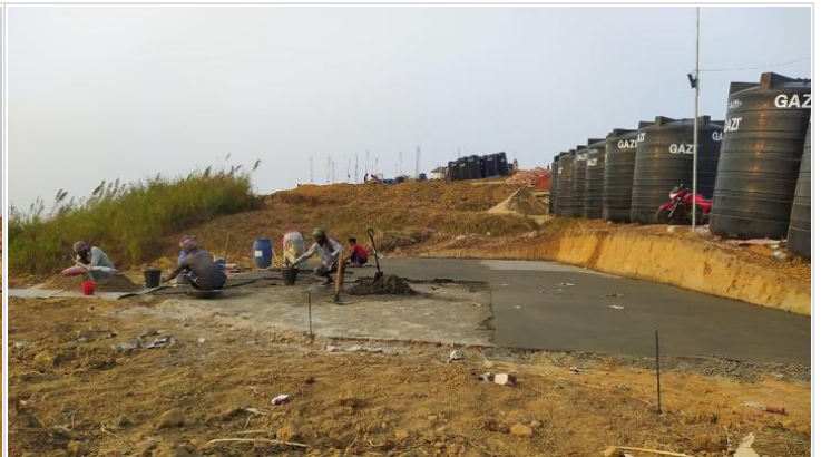
Solling joint fillup & plaster work at w
