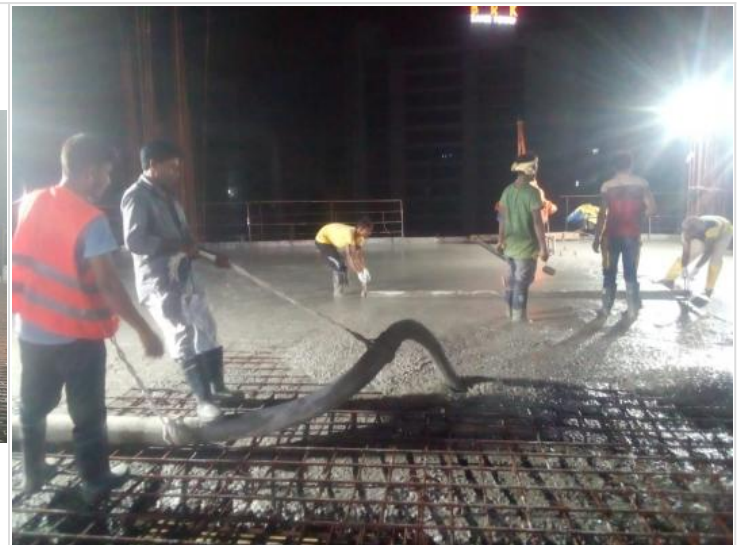
South Tower 11th Floor Slab Concreting
