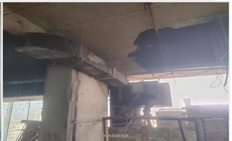
L-14-AC Duct installation on 06-01-24
