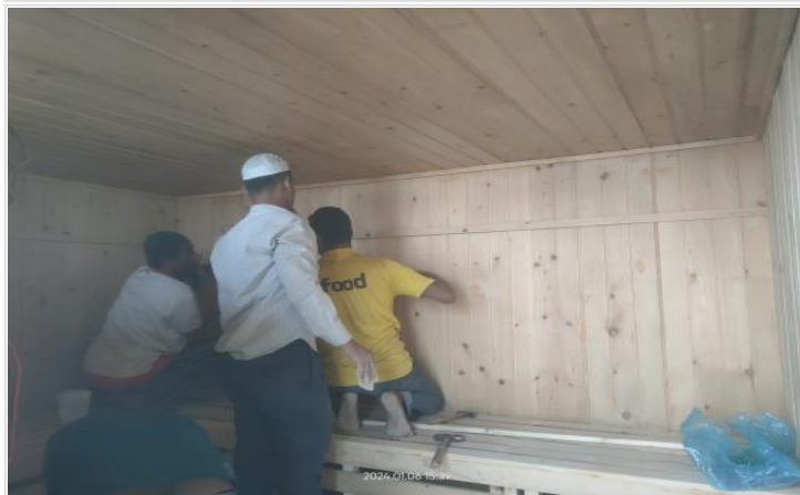
L-11-Suana-Wooden Wall Work on 06-01-24
