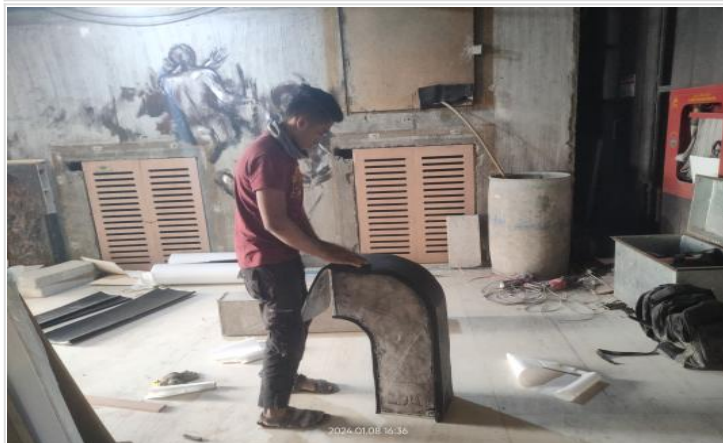
L-14-AC Duct fabrication on 08-01-24
