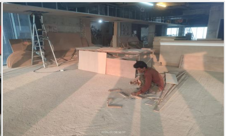
L-14-False Ceiling Work on 08-01-24
