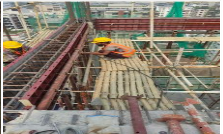
L-16-Beam shuttering on 18-04-23
