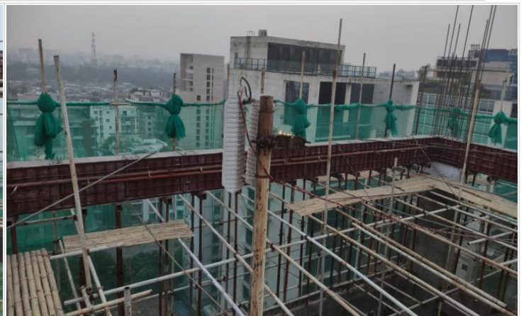
L-16-Beam concreting complete on 19-04-23
