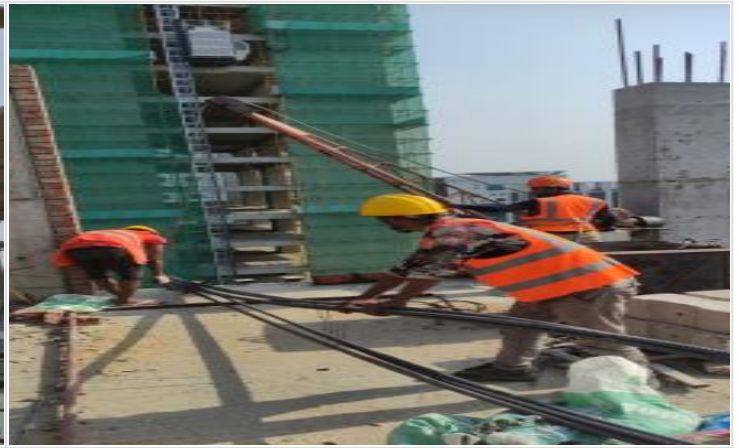
L-16-Beam Re-bar fabrication on 15-04-23
