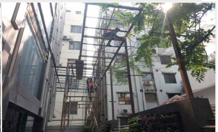
Coffee shop outside shed sheeting on 09-03-23
