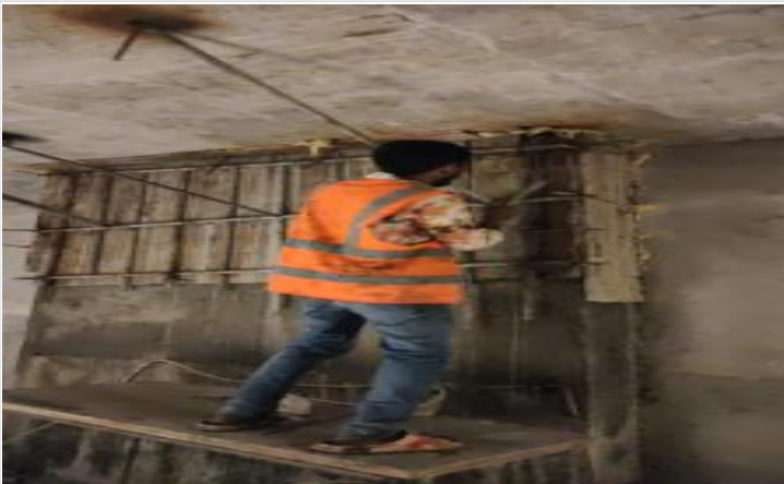
B2-Column retrofit shutter removing on 05-04-23
