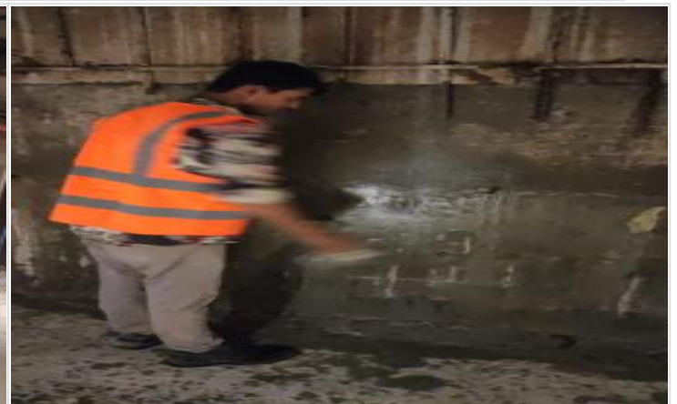
B2-Column Retrofit-Curing on 09-04-23
