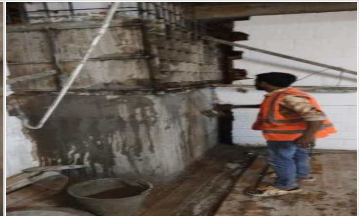
B-2-Column retrofit curing on 05-04-23
