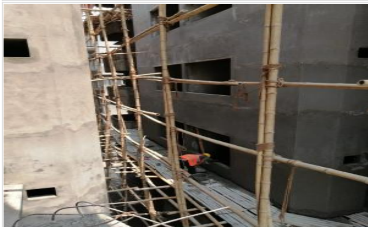
Out-side Plastering on 02-05-21
