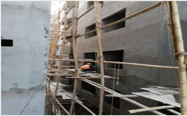
Bulding-Q-Out-side Plastering on 09-05-21
