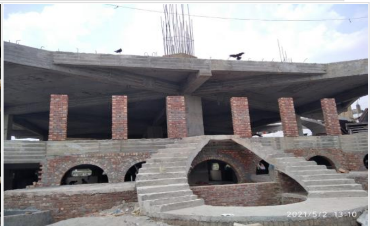
Mosque-Gr./1st Floor-Ancillary Works on 02-05-21
