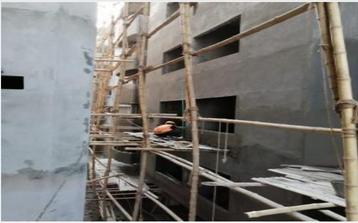
Bulding-Q-Out-side Plastering on 09-05-21
