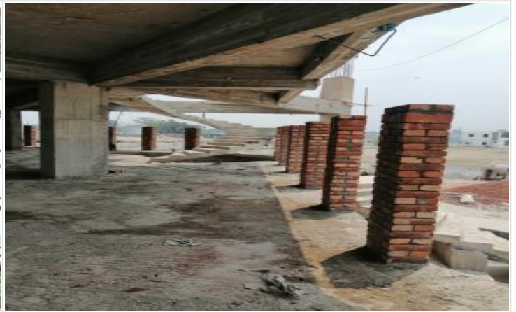
Out-side Plaster Work on 01-05-21
