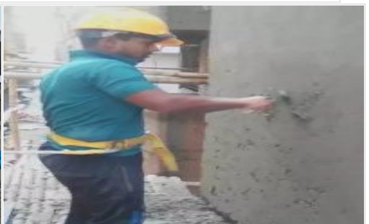
Out-side Plaster Work on 04-05-21
