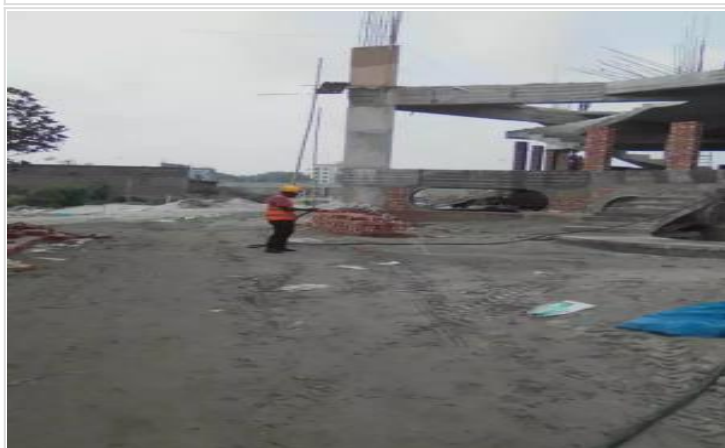
Mosque-Gr/1st Floor-Anciliary works on 04-05-21
