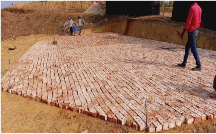
Soling for PVC Water Tank on 20-01-21
