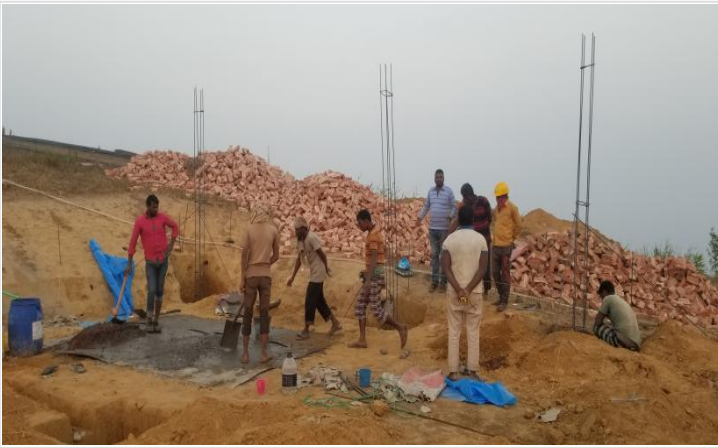
Footing & column casting work on going on 13-01-21
