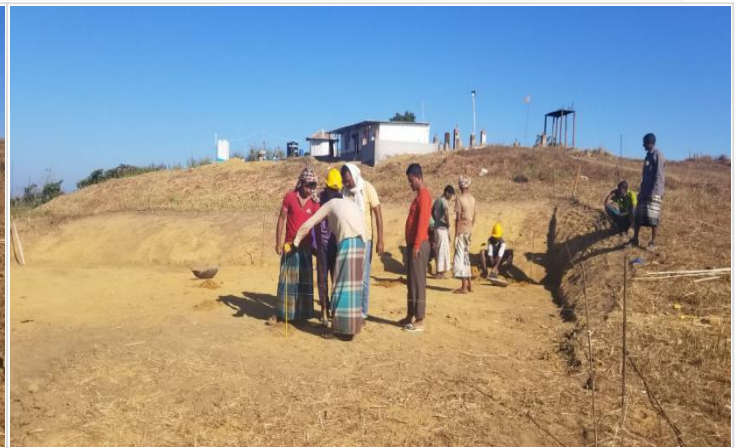
Guest House-Preparation for Layout on 06-01-21
