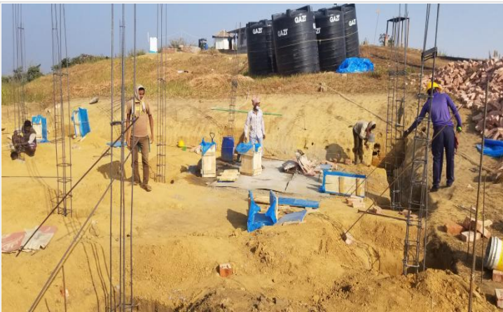
Shuttering fitting work for short column on 17-01-21
