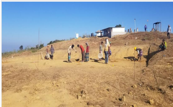
Guest House-Preparation for Layout on 07-01-21
