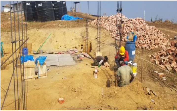
Shuttering fitting work for short column on 16-01-21
