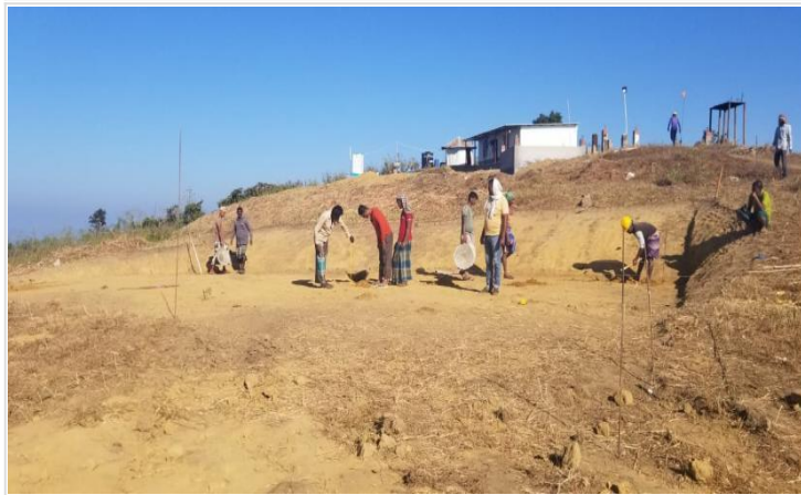
Guest House-Preparation for Layout on 06-01-21
