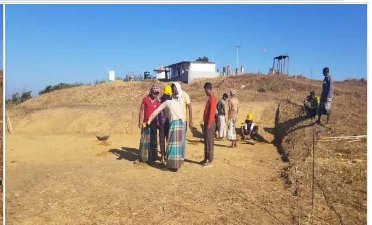
Guest House-Preparation for Layout on 07-01-21
