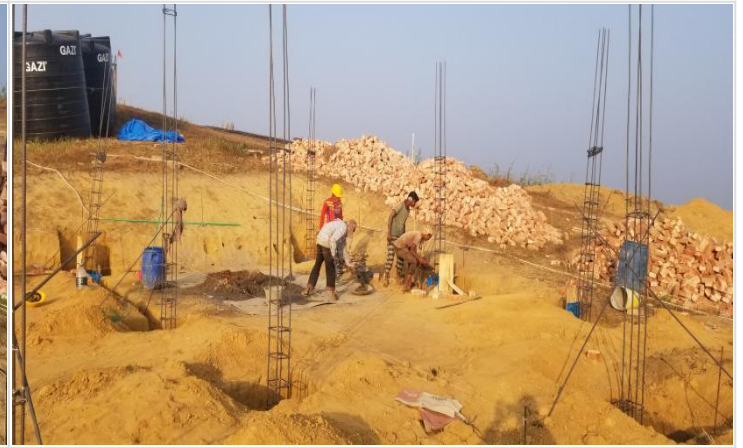
Short column casting work for guest hous on 16-01-21
