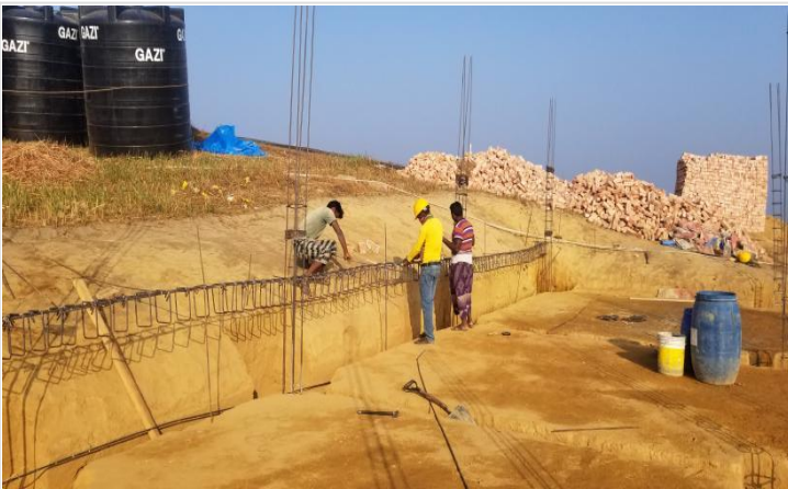
MS rod cutting & binding work for grade on 19-01-21
