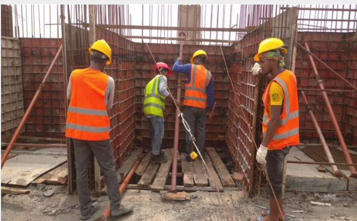
Ground floor Lift Core Shuttering on 07-06-21
