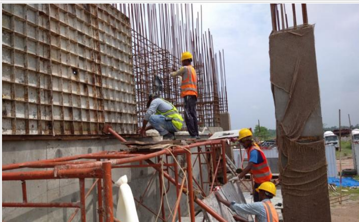
Ground Floor Lift Core Shuttering on 15-06-21
