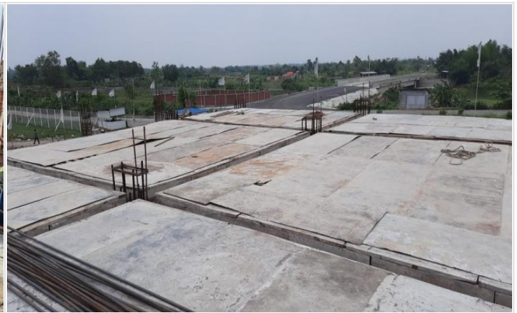
1st floor Slab Shuttering on 09-06-21
