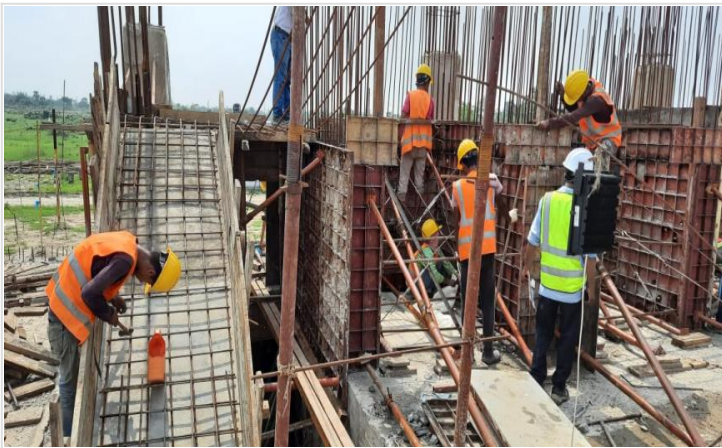
Ground Floor Stair Re-bar work on 09-06-21
