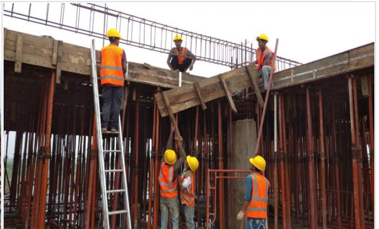
1st Floor Beam Shuttering on 06-06-21
