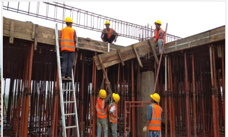
1st Floor Beam Shuttering on 06-06-21
