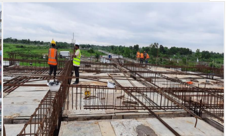
1st floor Slab Shuttering on 12-06-21
