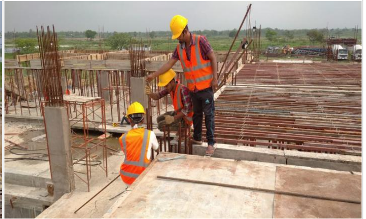
1st Floor Slab Shutter Levelling on 03-06-21
