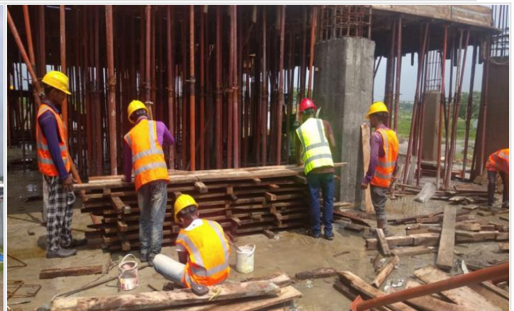
1st floor Slab Shuttering on 15-06-21
