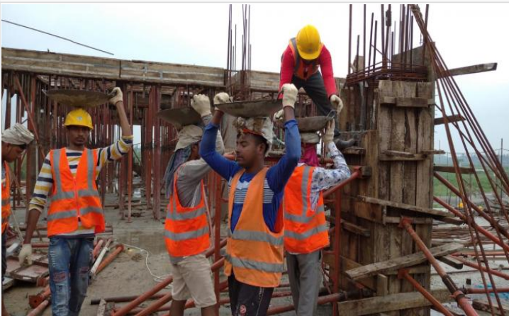
Ground Floor Column Concreting on 06-06-21
