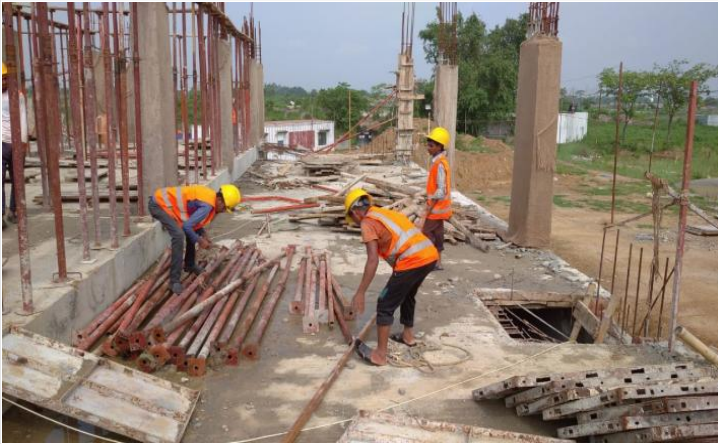
1st Floor Slab Shuttering on 03-06-21
