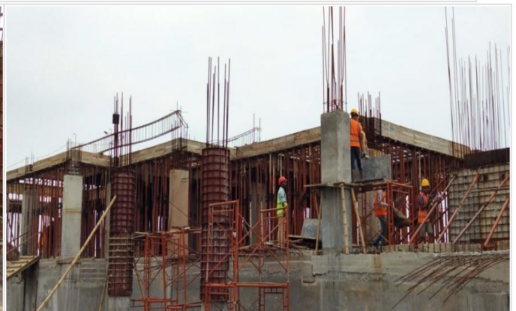
Ground Floor Construction on 07-06-21
