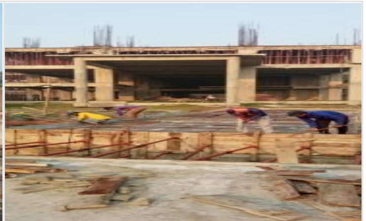
East Septic Tank Slab Shuttering
