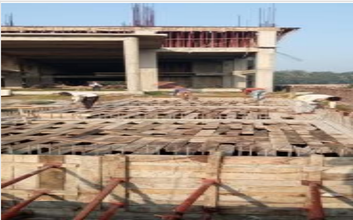
East Septic Tank Slab Shuttering
