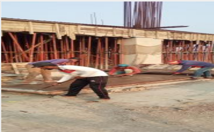
Column/Wall Steel Shutter Cleaning, Oili
