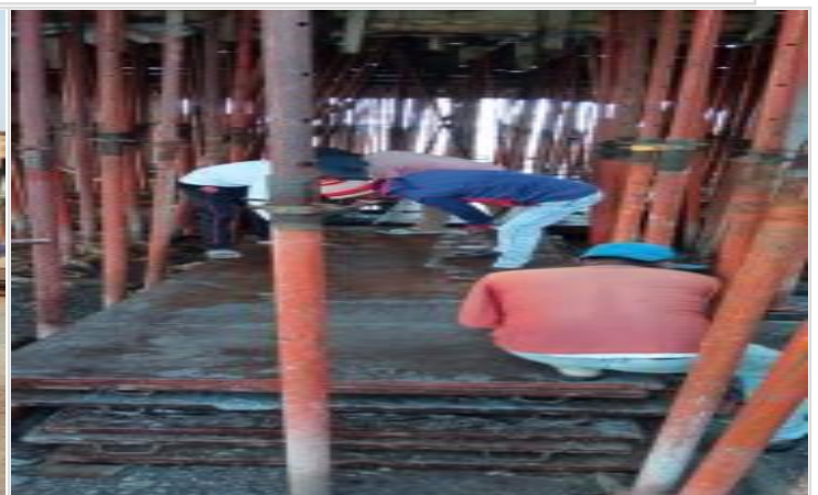
Column/Wall Steel Shutter Cleaning, Oili
