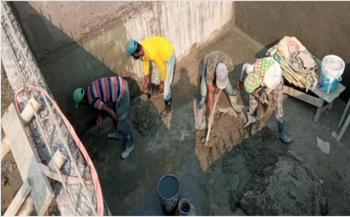
East Septic Tank Plastering
