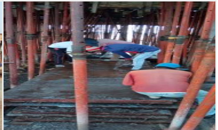
Column/Wall Steel Shutter Cleaning, Oili
