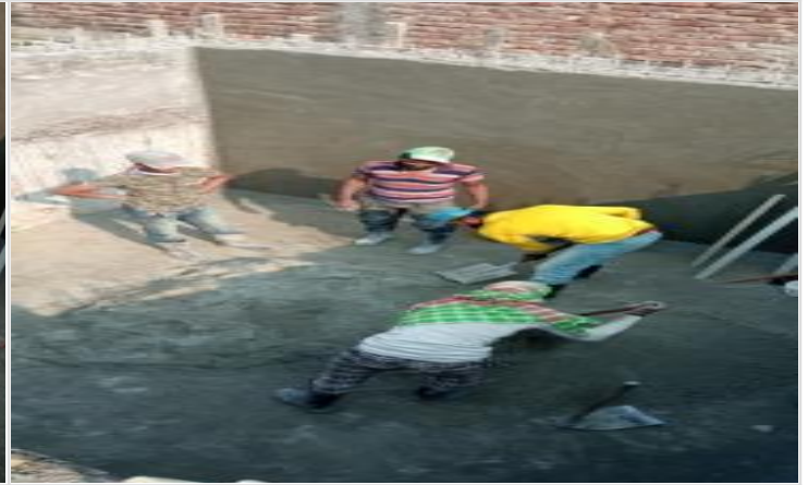
East Septic Tank Plastering
