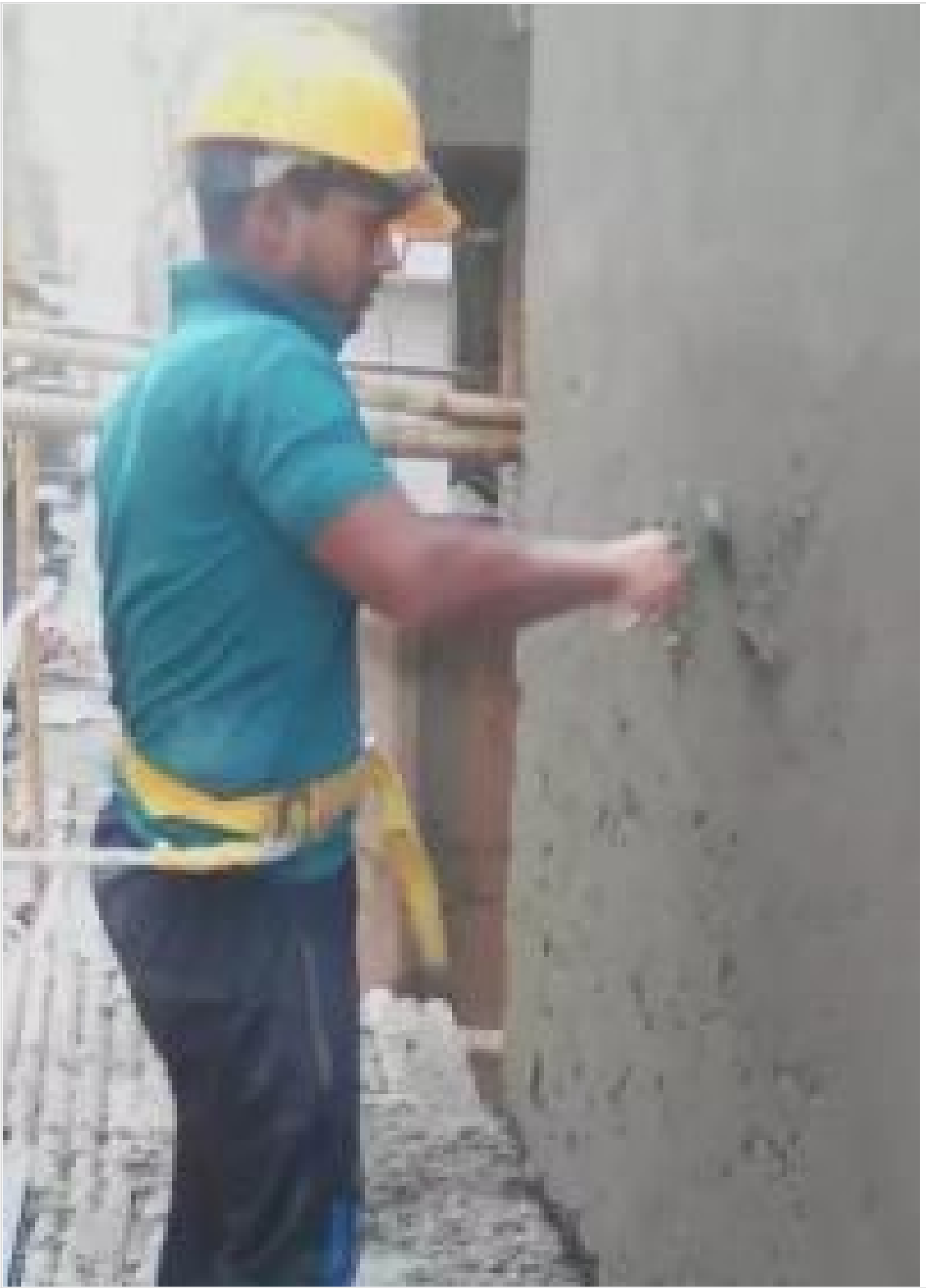
Out-side Plaster Work on 04-05-21
