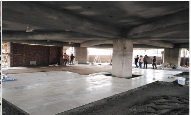
Mosque-Basement Tiles Work
