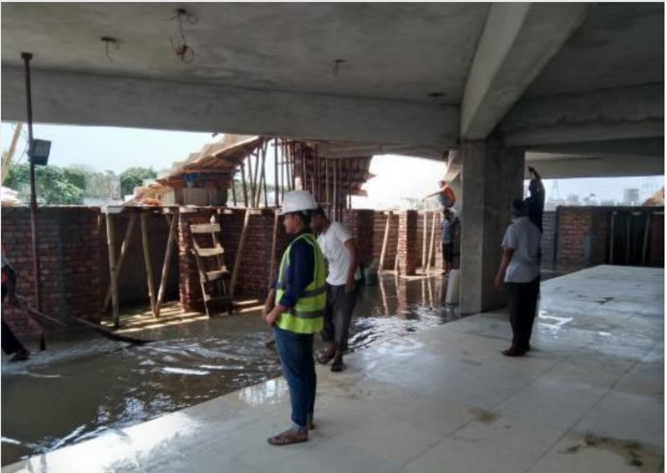
Mosque-Basement-Ancliary Work on 17-04-21
