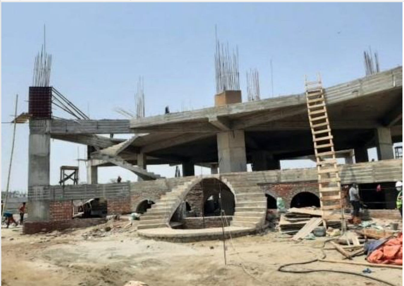
Mosque-Basement-Anclary Work on 26-04-21
