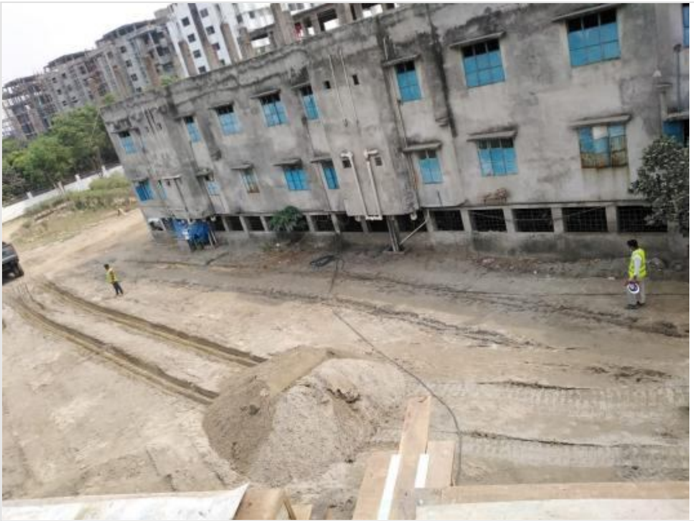
Mosque-20ft Connecting Road-Filling on 31-03-21
