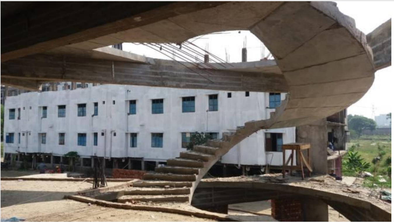
Mosque-Stair Case on 25-04-21
