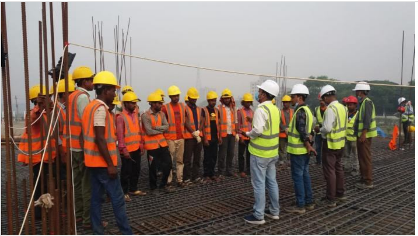
Breifing instruction before Concreting on 21-03-21
