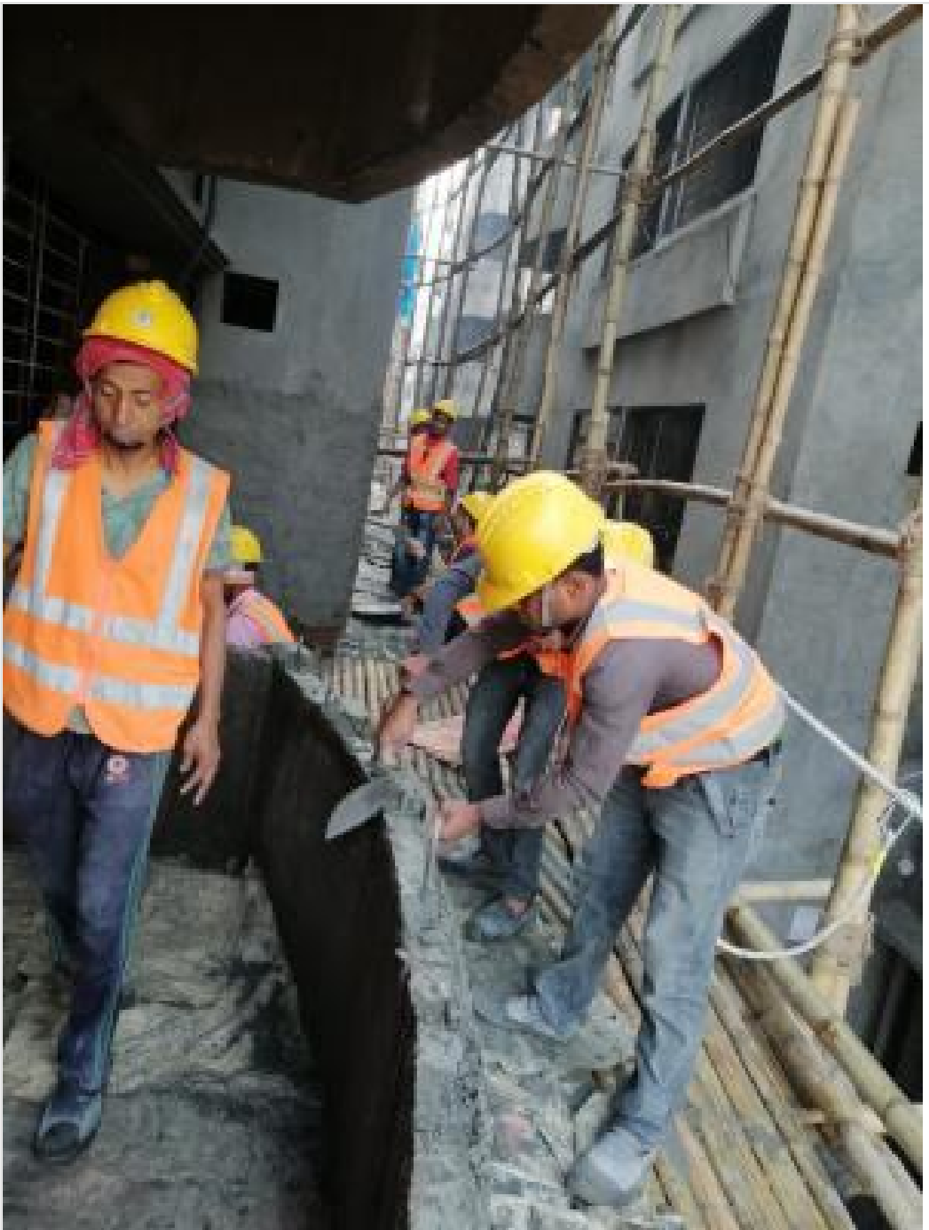
Out-side Plaster Work on 05-02-21
