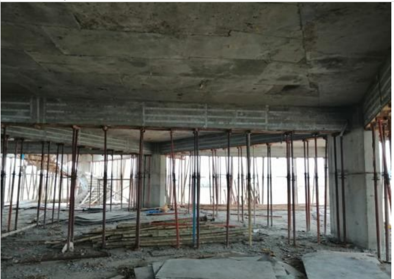
Mosque-Ground Floor-Roof Slab de-shutter on 22-04-21
