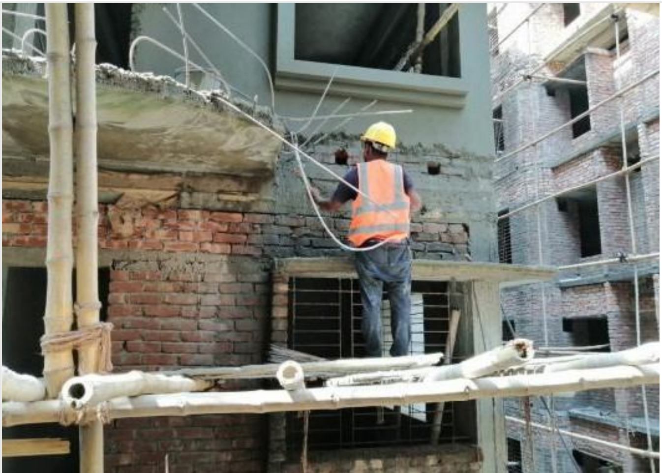
Out-side Plastering on 20-04-21
