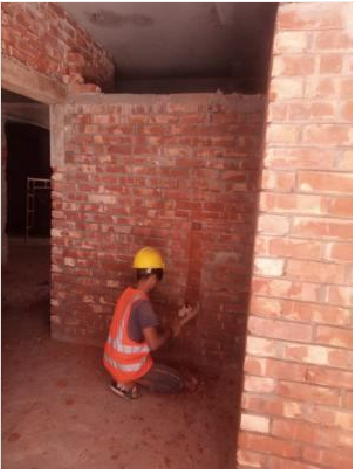
Electrical Conduit Conesealing on 25-02-21
