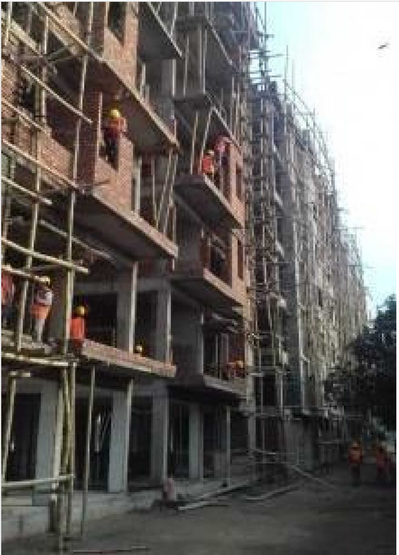
Scaffolding for outside plastering Build on 29-01-21
