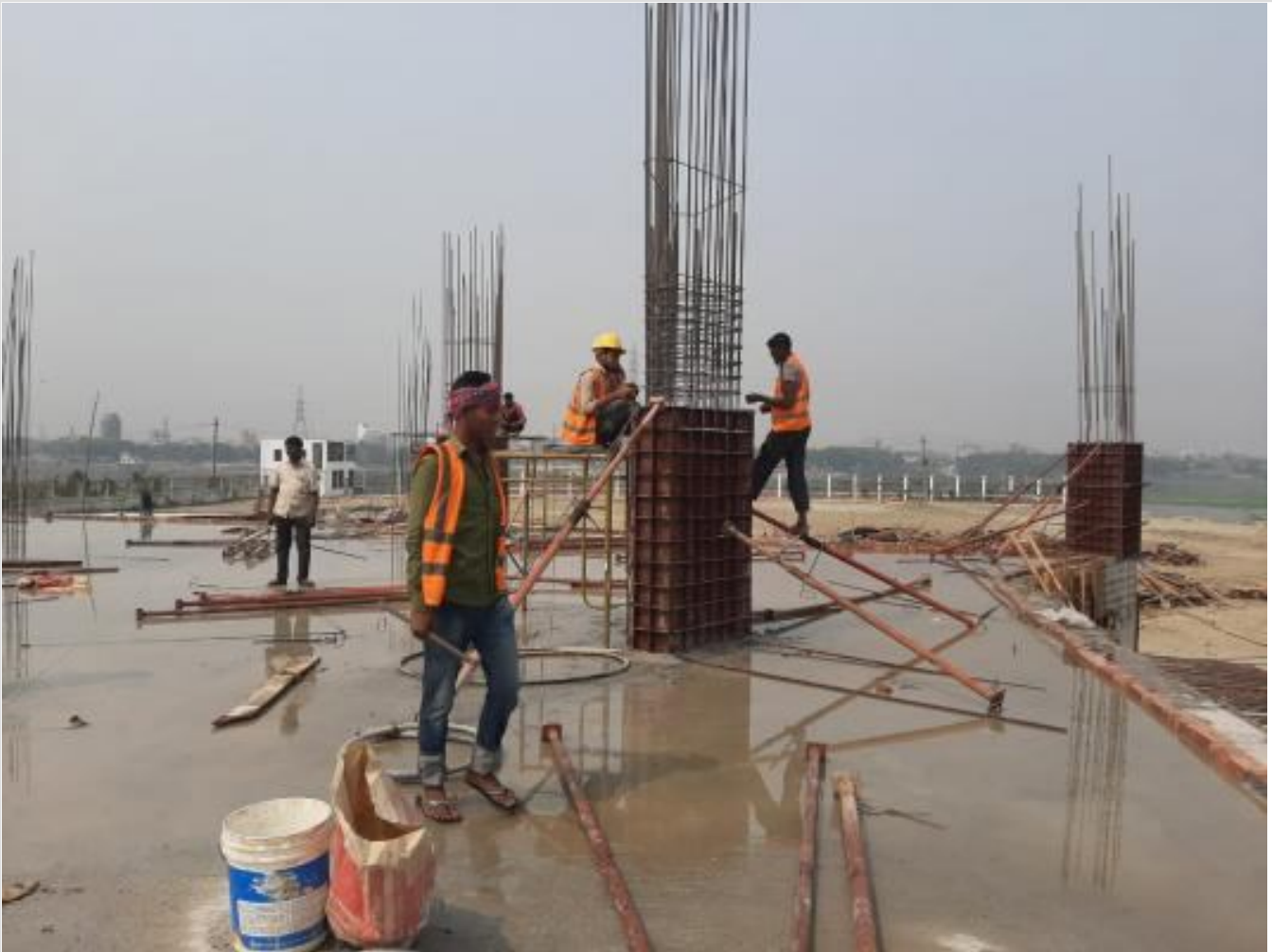
Mosque GF Column 2nd Lift Re-bar Work on 24-03-21
