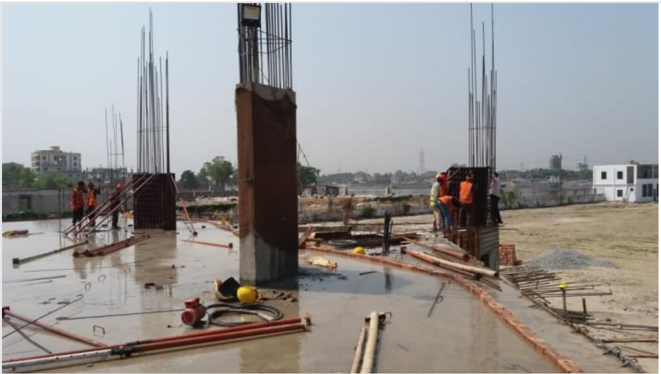
Mosque-GF Column Work on 25-03-21
