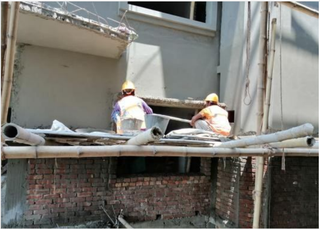
Out-side Plastering on 19-04-21
