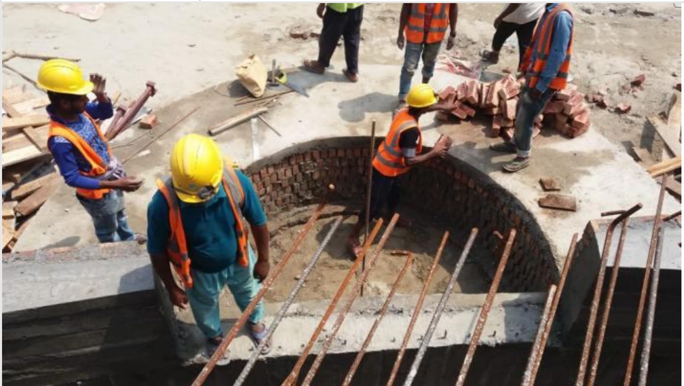
Mosque Ground Floor Stair Concreting on 28-03-21
