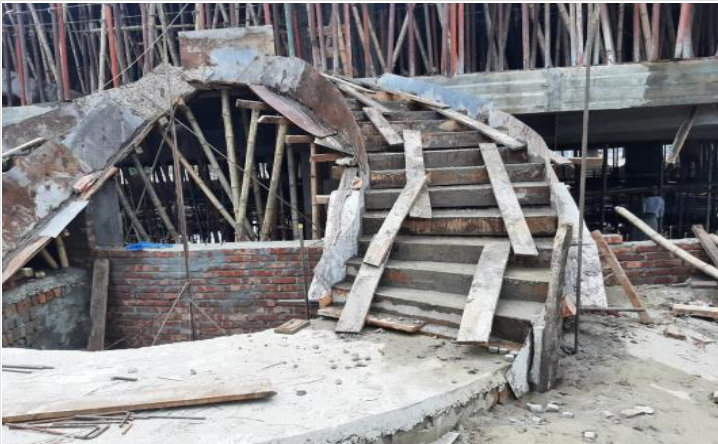
Mosque-Esatside Stair Case
