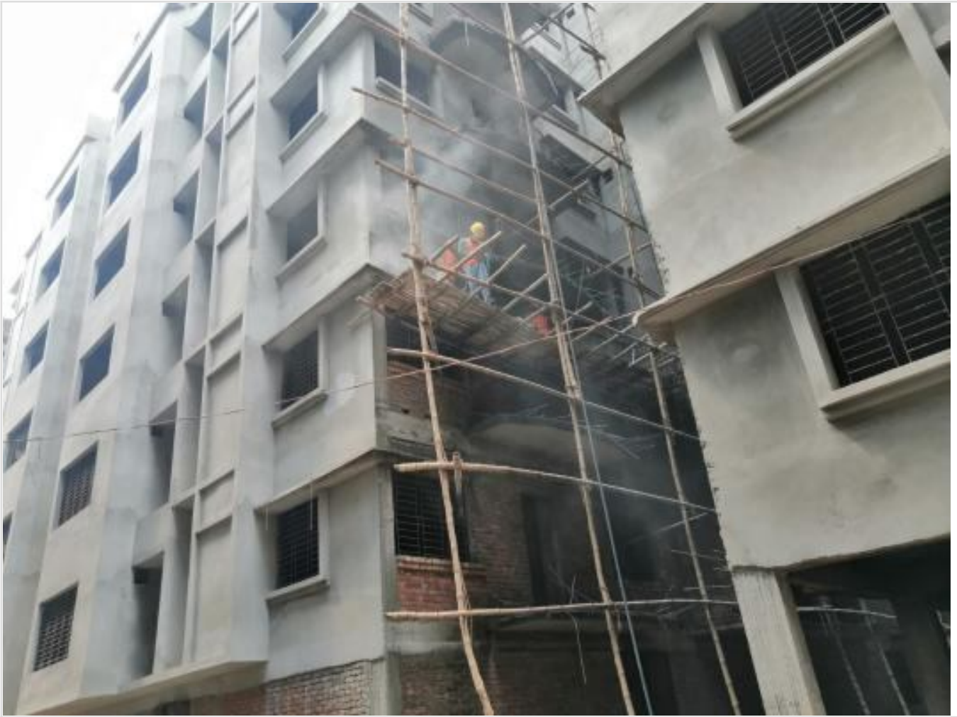
Building Outside Plastering on 08-03-21
