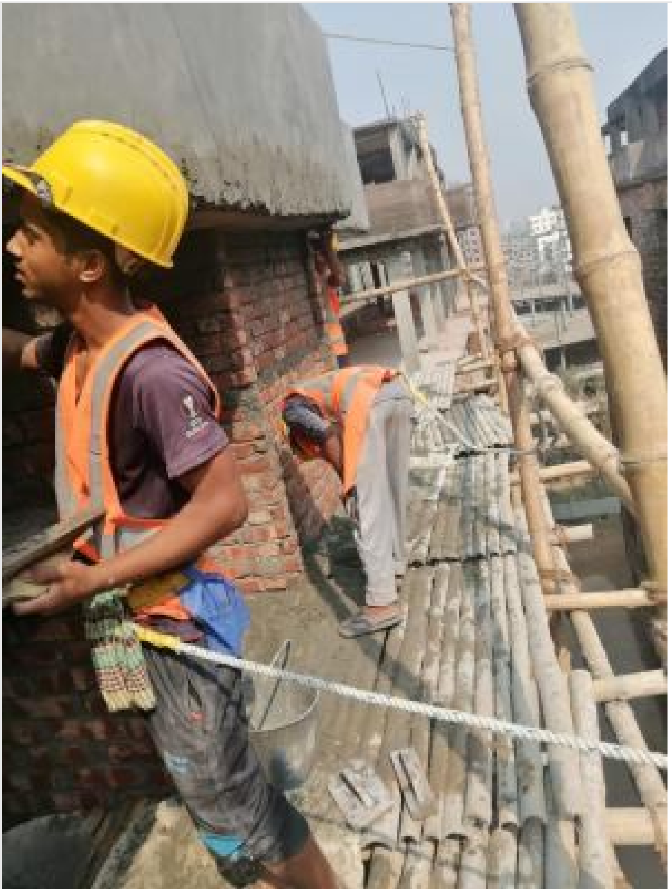
Building Outside Plastering on 01-03-21
