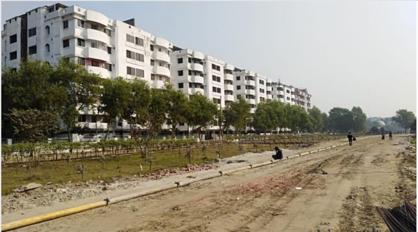
Building Outside Painting on 08-02-21
