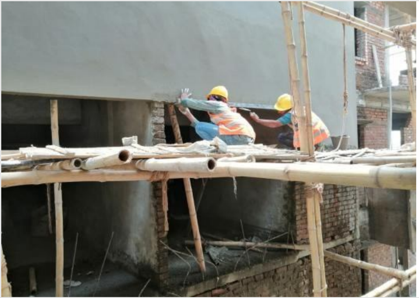
Out-side Plastering on 28-04-21
