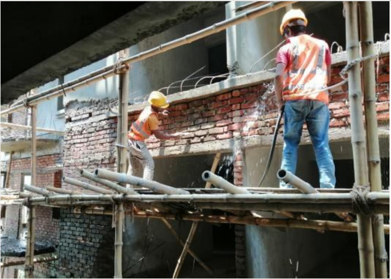
Out-side Plastering on 17-04-21
