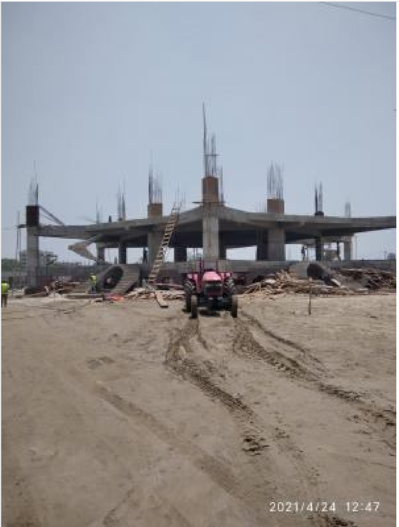
Mosque Building in Construction on 24-04-21
