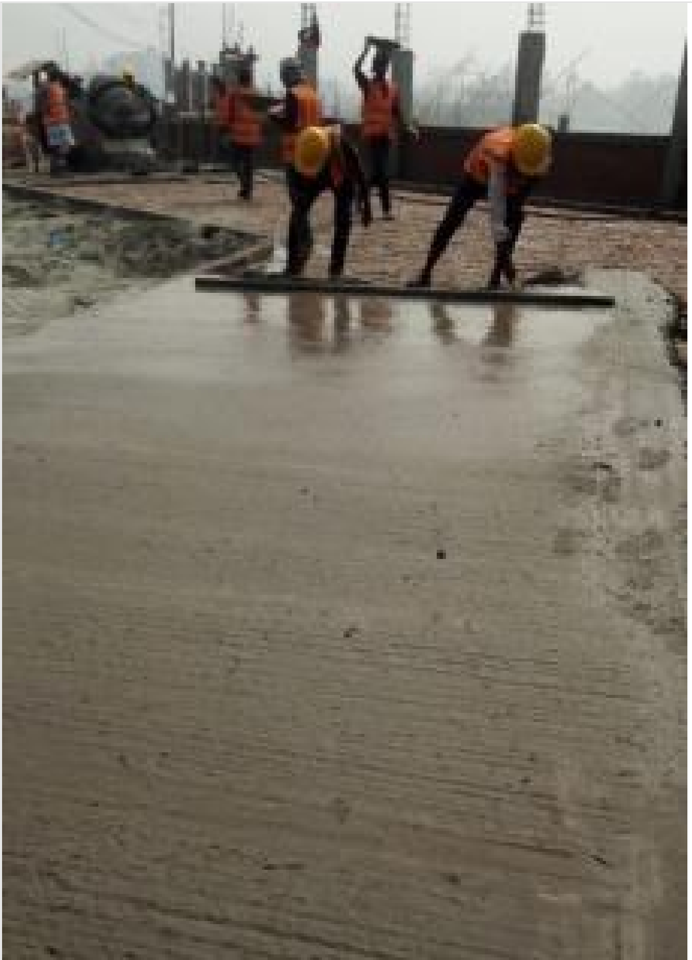
Riverside walkway CC work on 28-01-21
