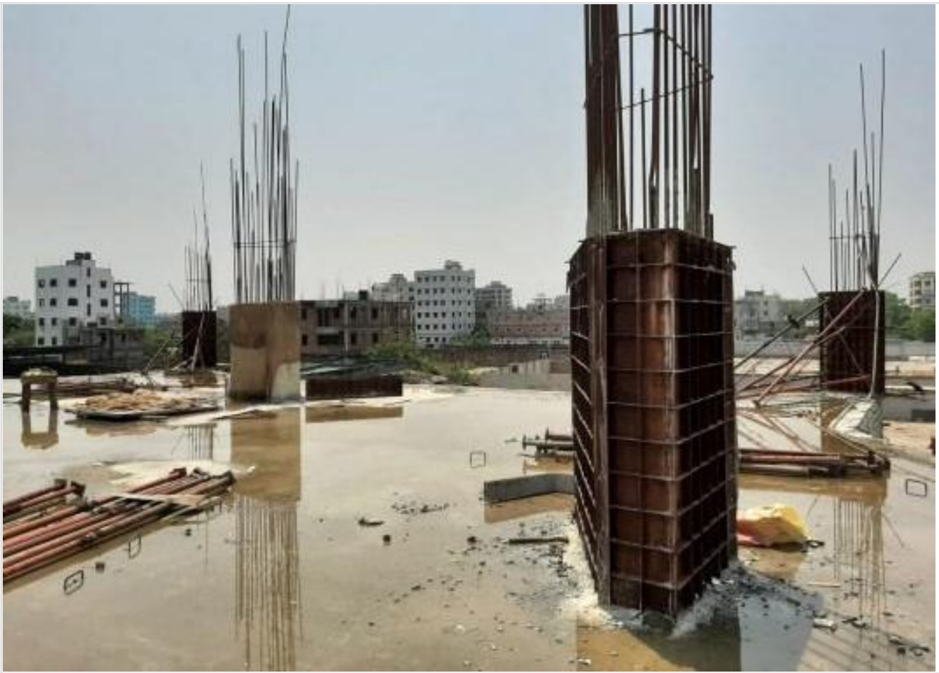
Mosque-1st Floor-Column Shuttering on 26-04-21
