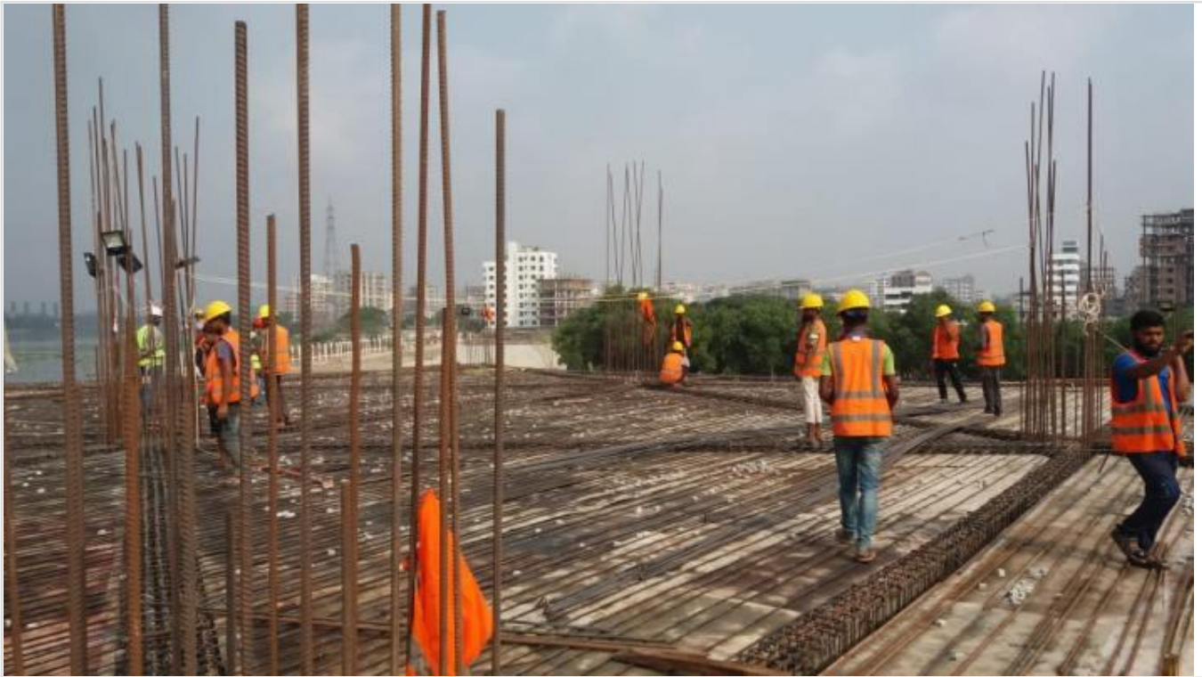
Mosque 1st Floor Slab Re-bar Work on 03-04-21
