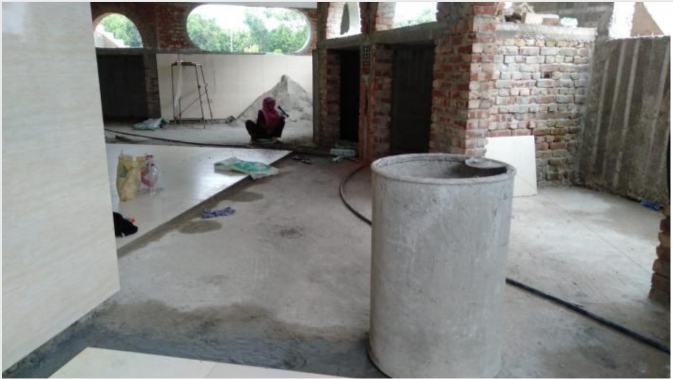
Mosque-Basement-Tile Work on 31-05-21
