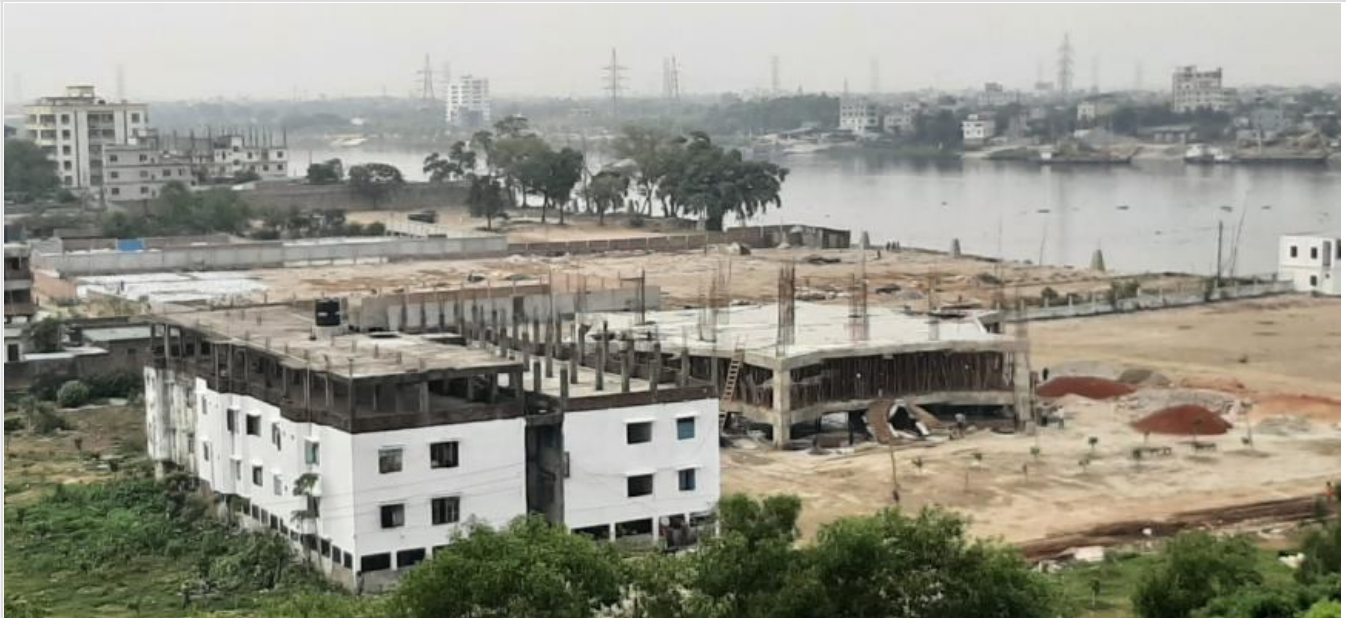
Mosque in Construction on 15-04-21
