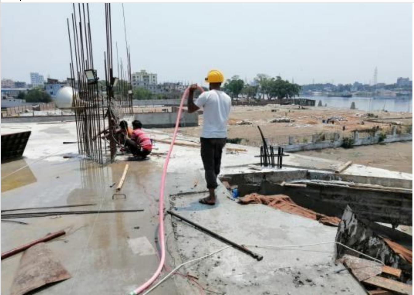
Mosque-Basement-Anclary Work on 16-04-21
