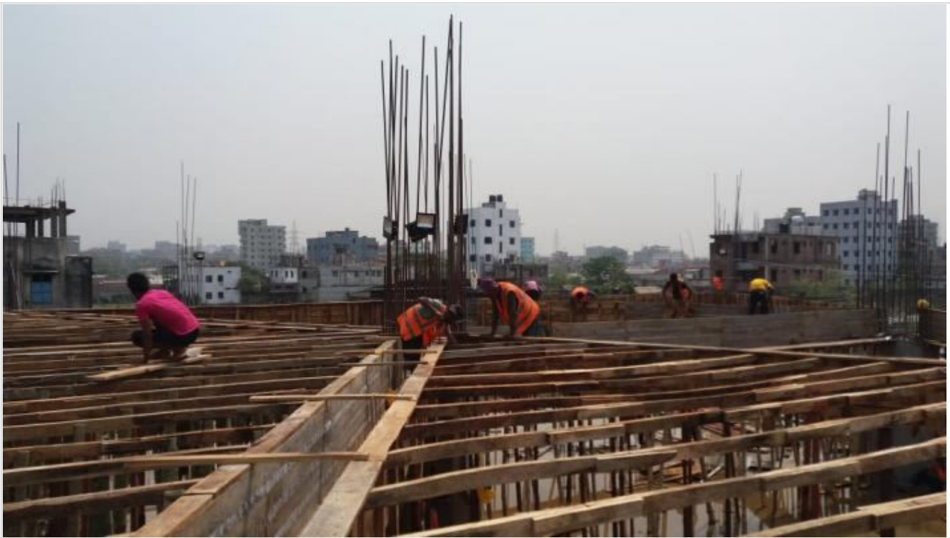
Mosque 1st Floor Slab Shuttering on 28-03-21
