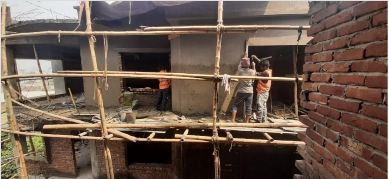
Out-side Plastering on 15-04-21
