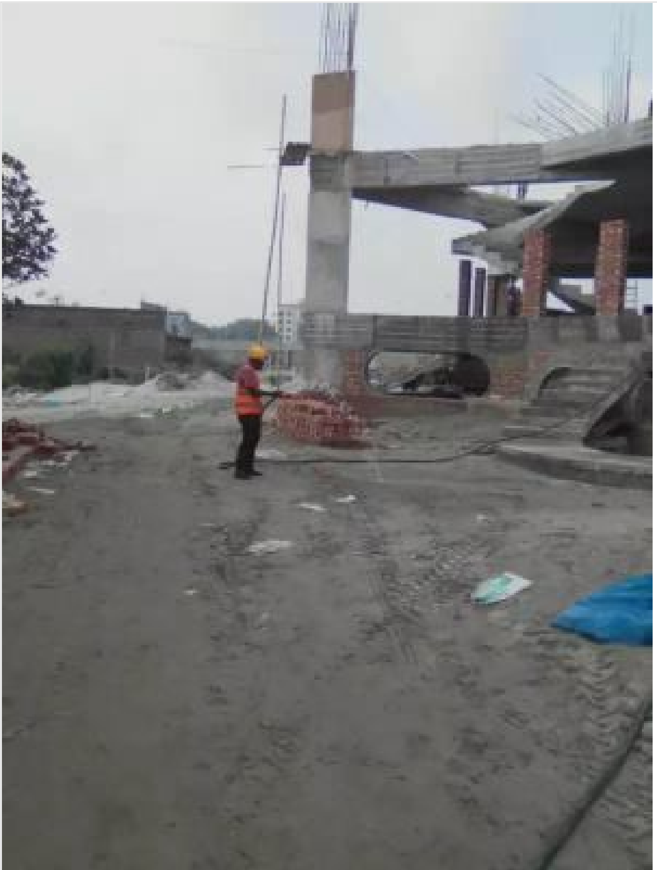
Mosque-Gr/1st Floor-Anciliary works on 04-05-21
