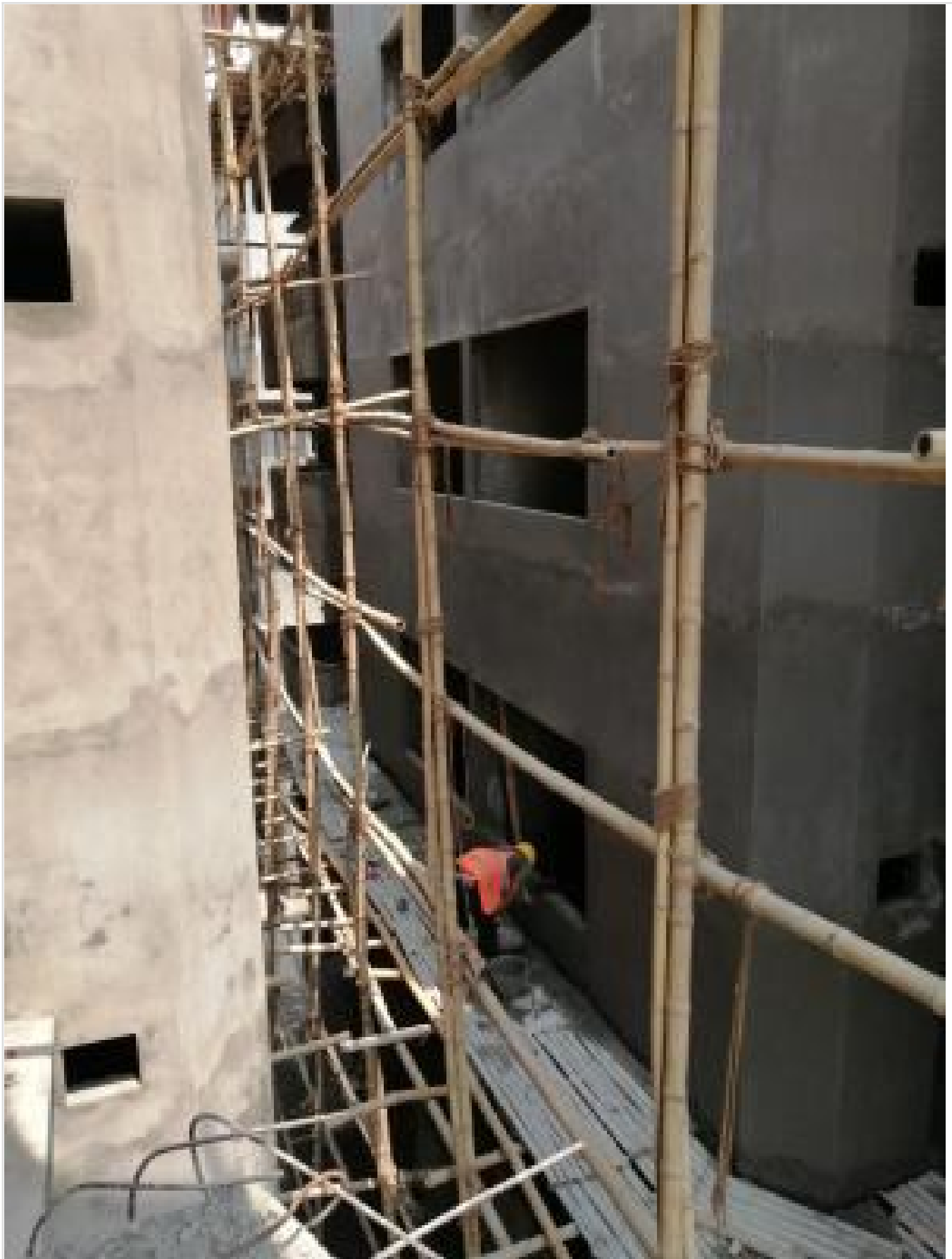
Out-side Plastering on 02-05-21
