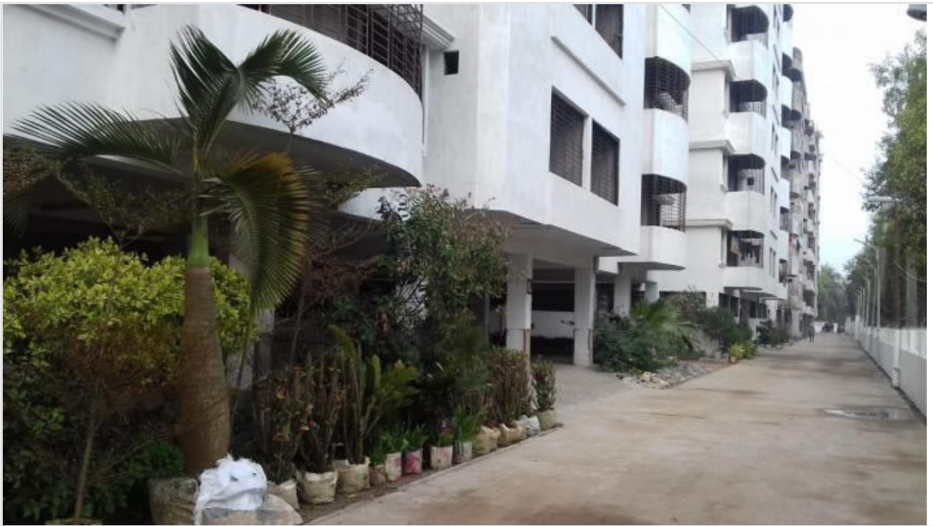
Building- outside plastering on 29-01-21
