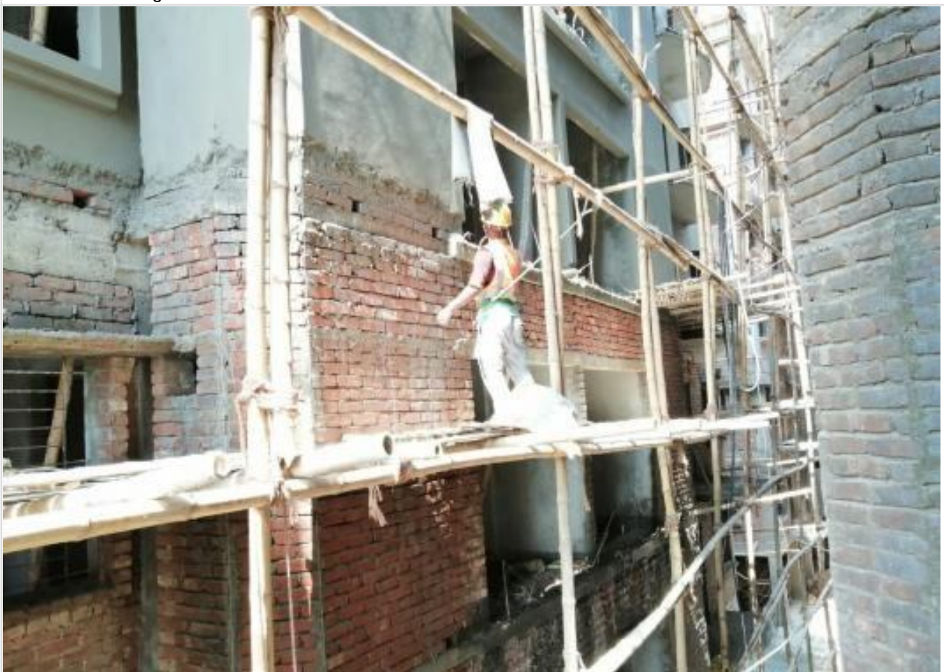
Out-side Plaster Work on 20-04-21
