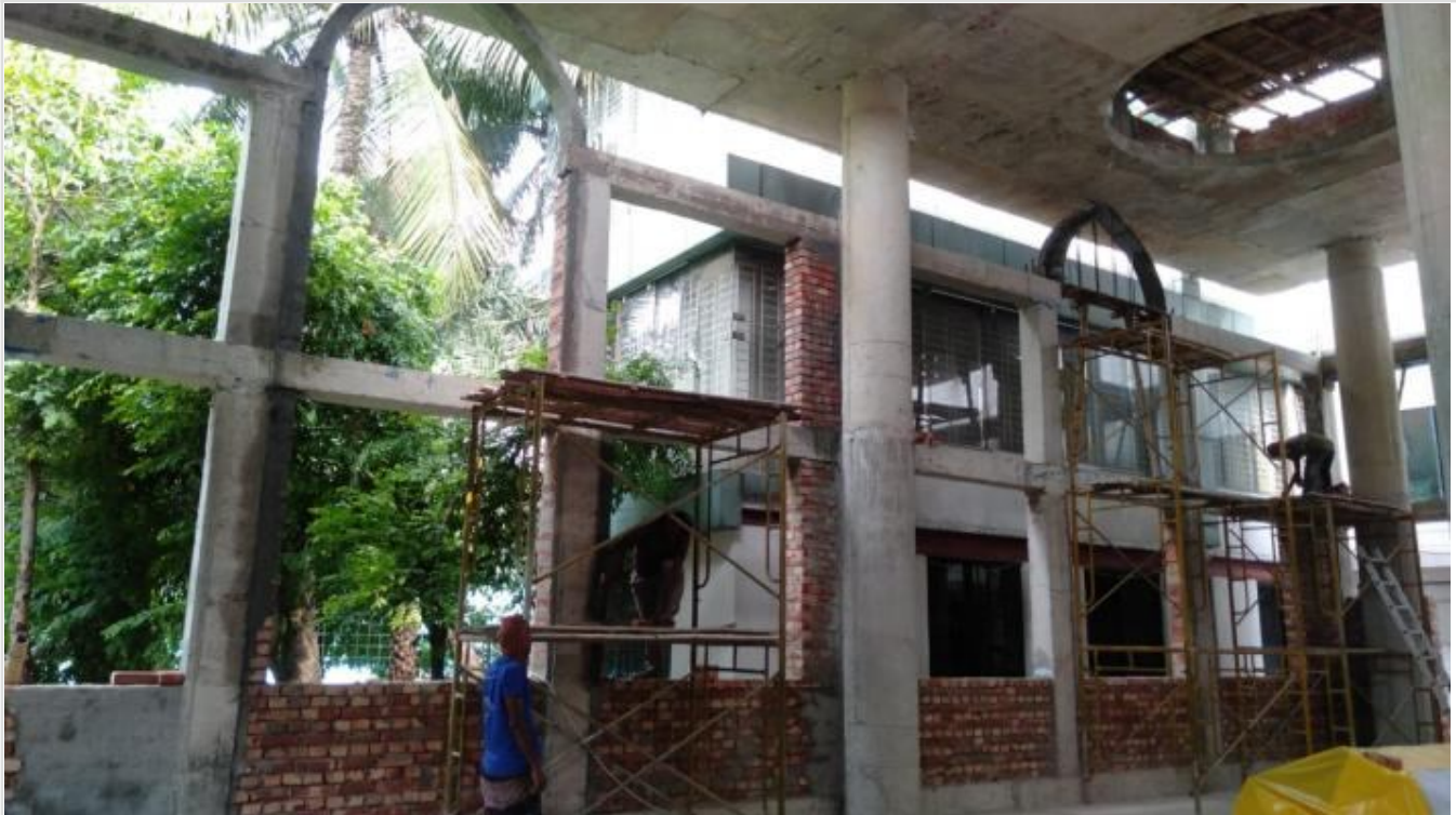
Mosque-Ground Floor-Ancillary Works on 31-05-21
