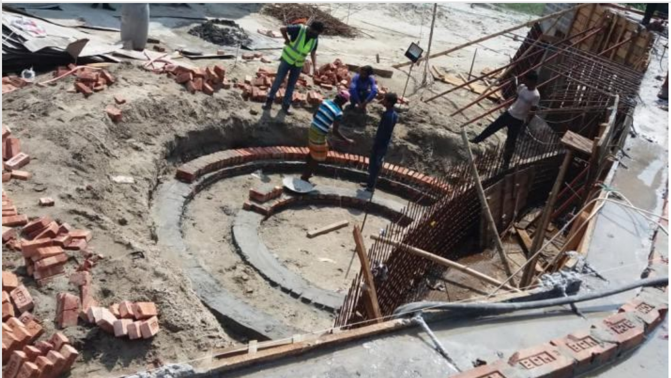
Mosque-GF-Stair Case Foundation Work on 25-03-21
