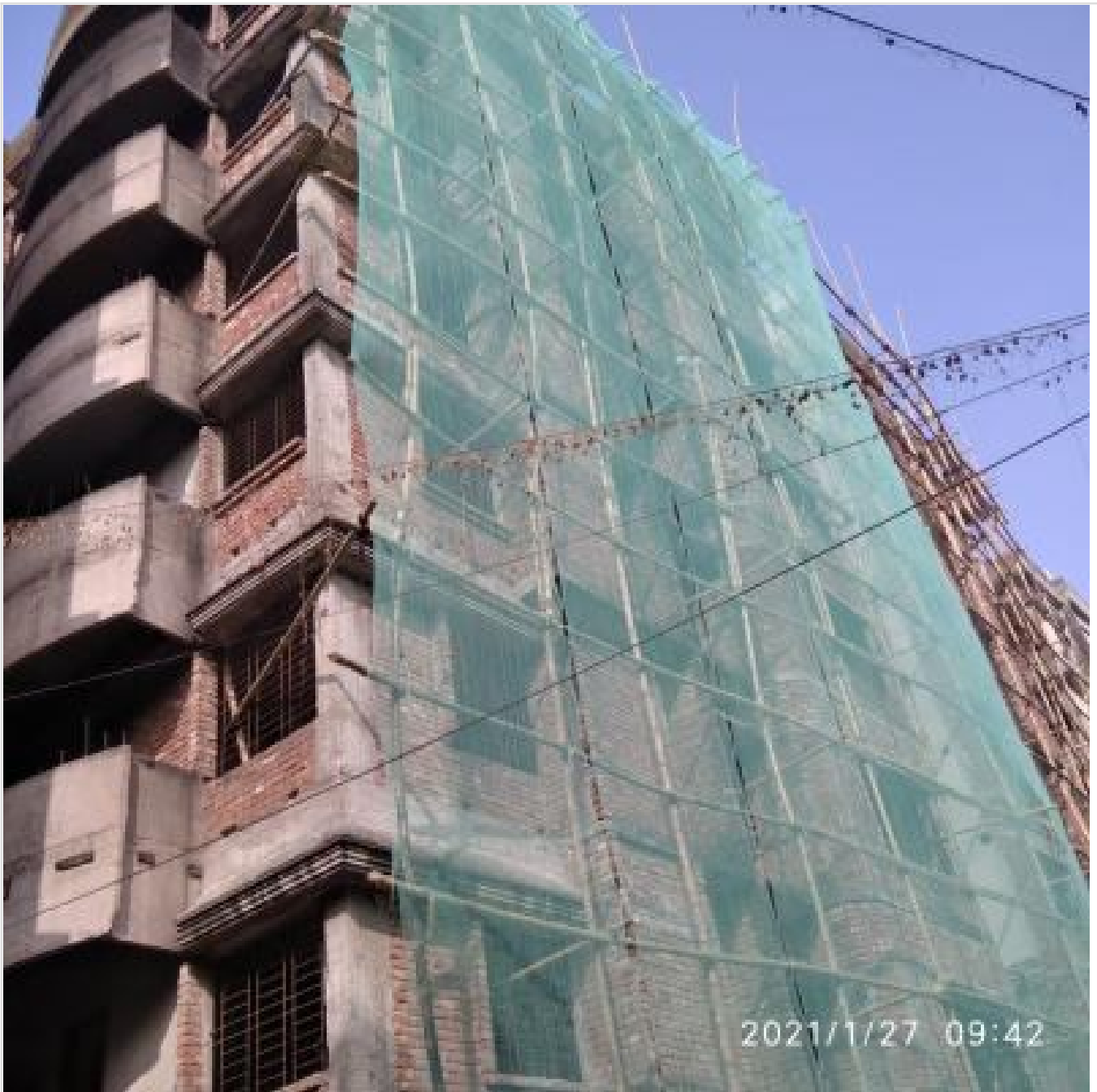
Scaffolding for Outside Plaster-Buildin on 27-01-21
