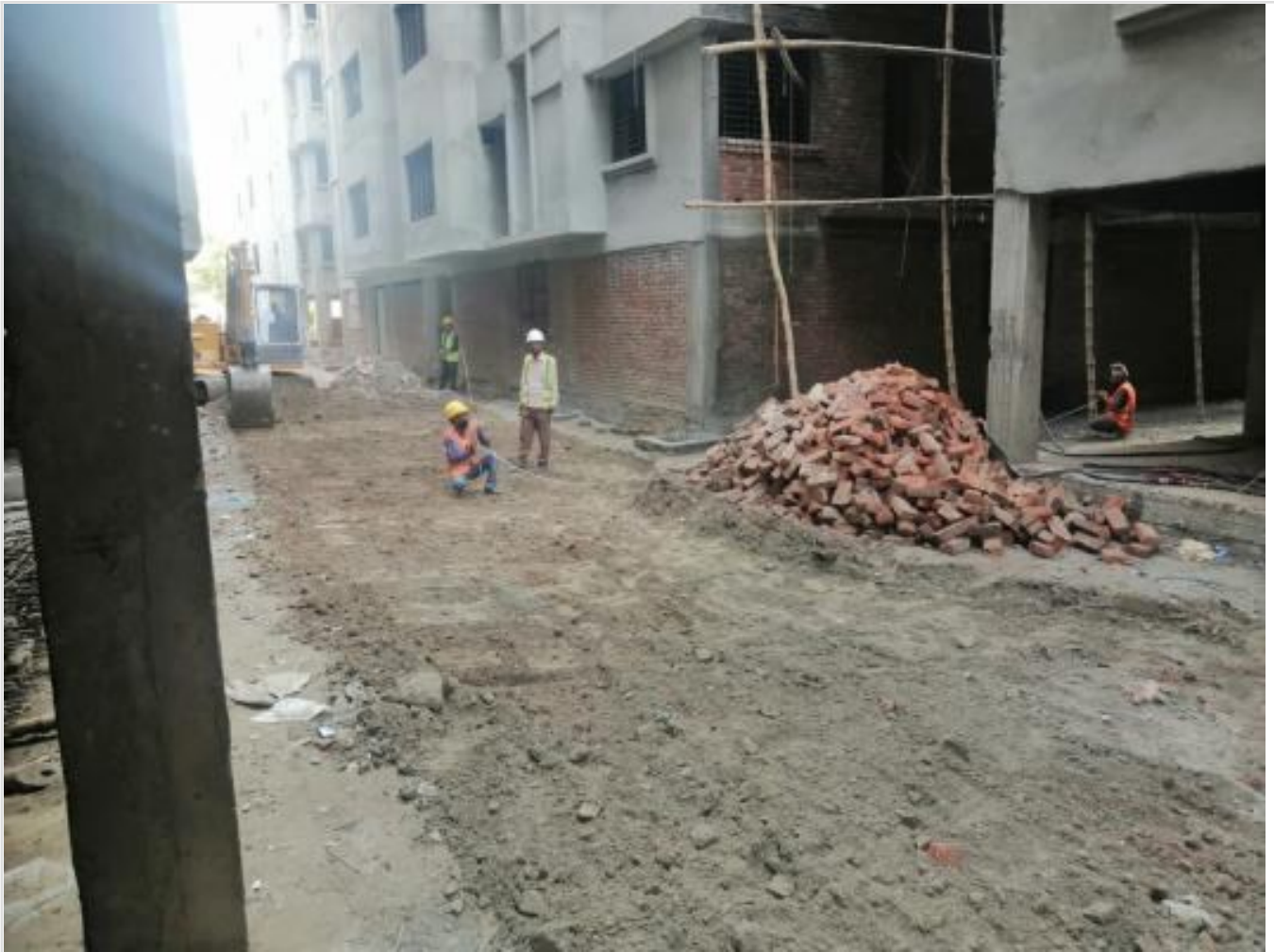
12 ft Road Filling on 28-02-21
