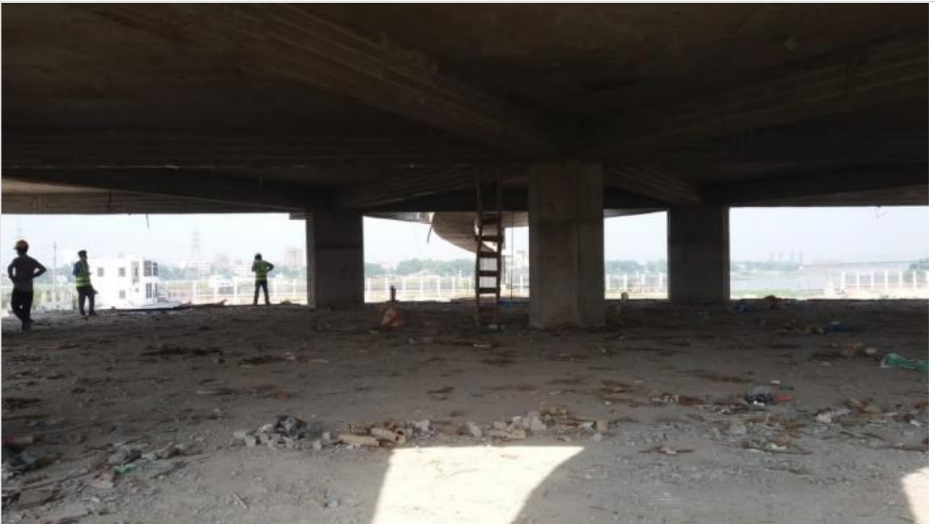
1st Floor Roof-De-shuttering on 25-04-21
