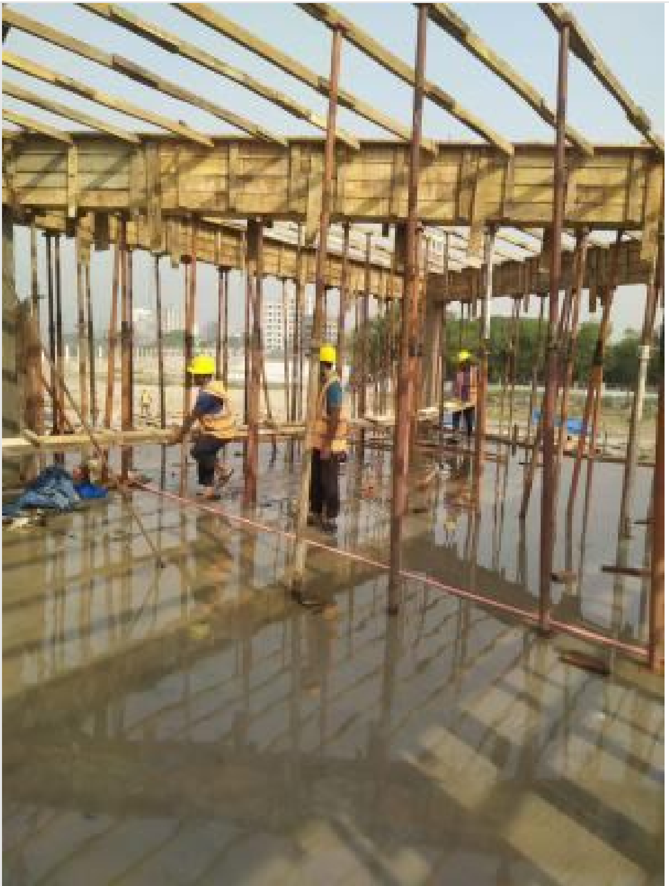
Mosque 1st Floor Slab Shuttering on 27-03-21
