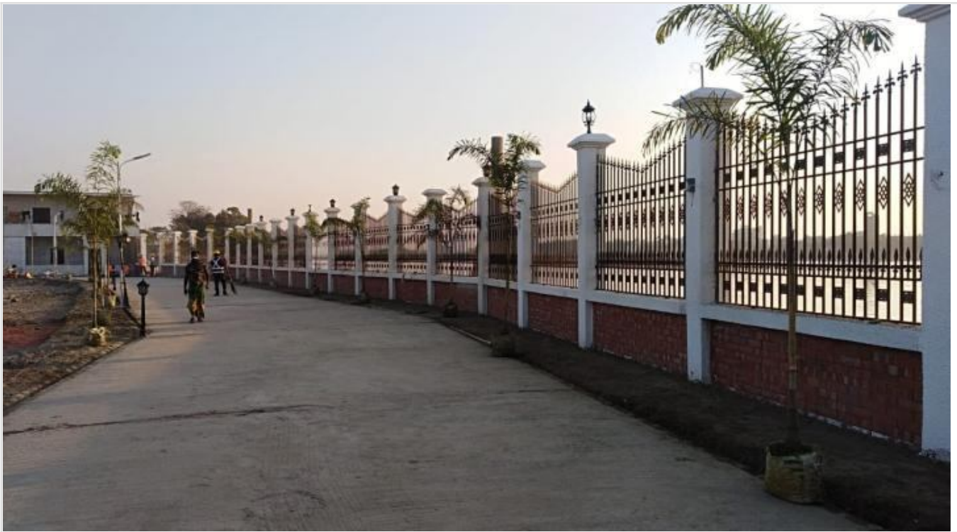
River Side Boundary Fencing on 10-02-21
