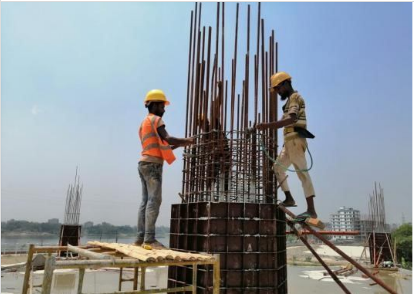
Mosque-1st Floor Column Re-bar Work on 19-04-21
