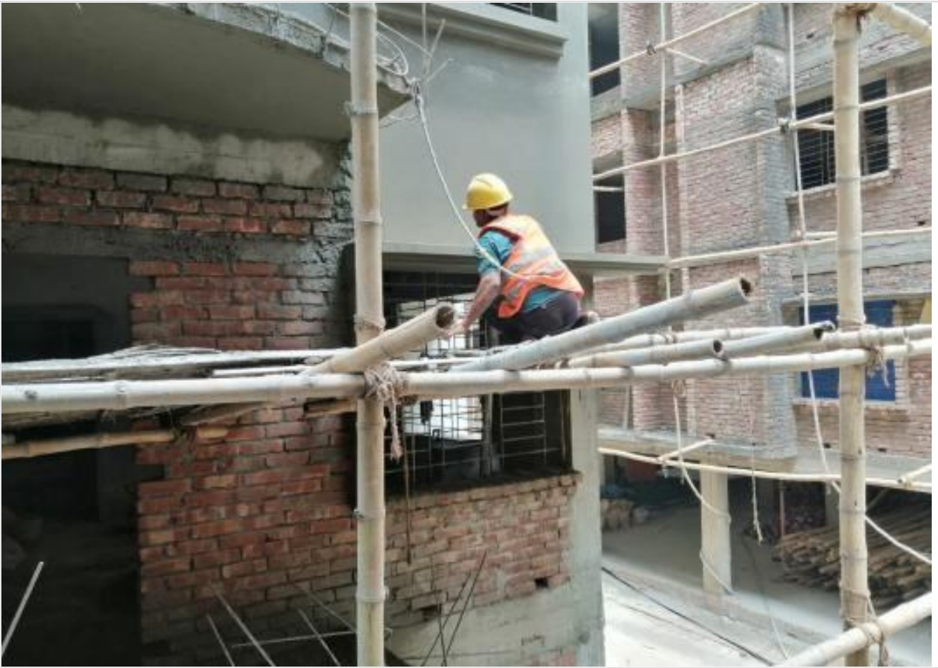
Out-side Plastering on 22-04-21
