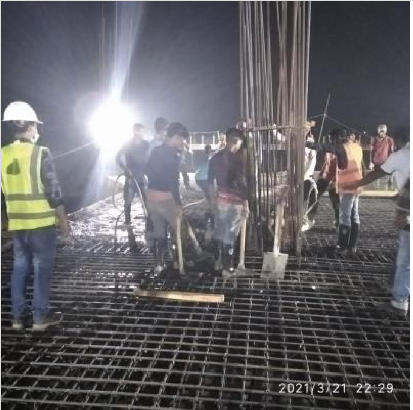
Mosque Ground Floor Slab Concreting on 21-03-21
