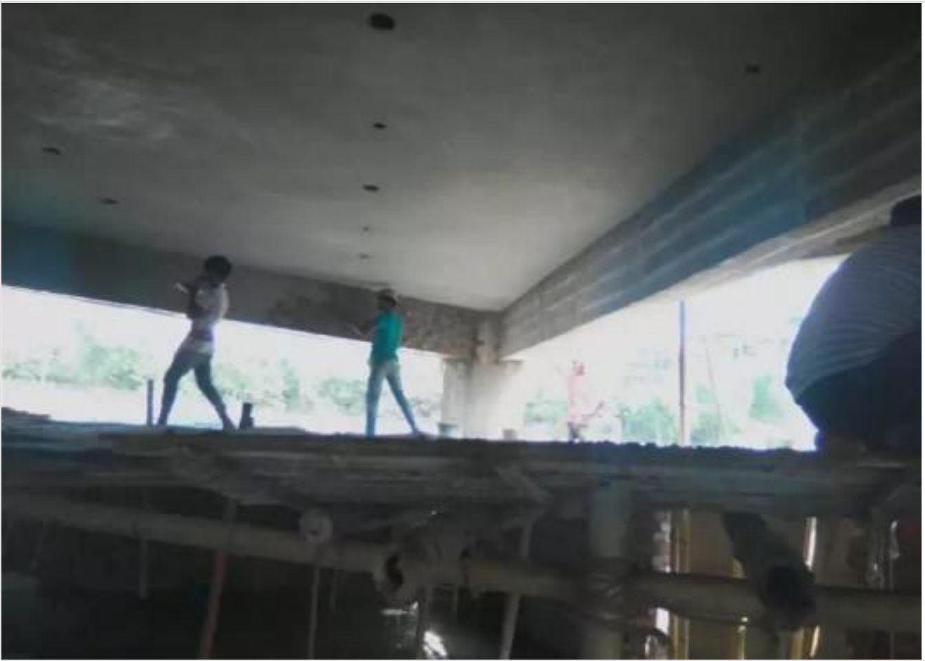
Mosque-Basment Plaster Work on 14-04-21
