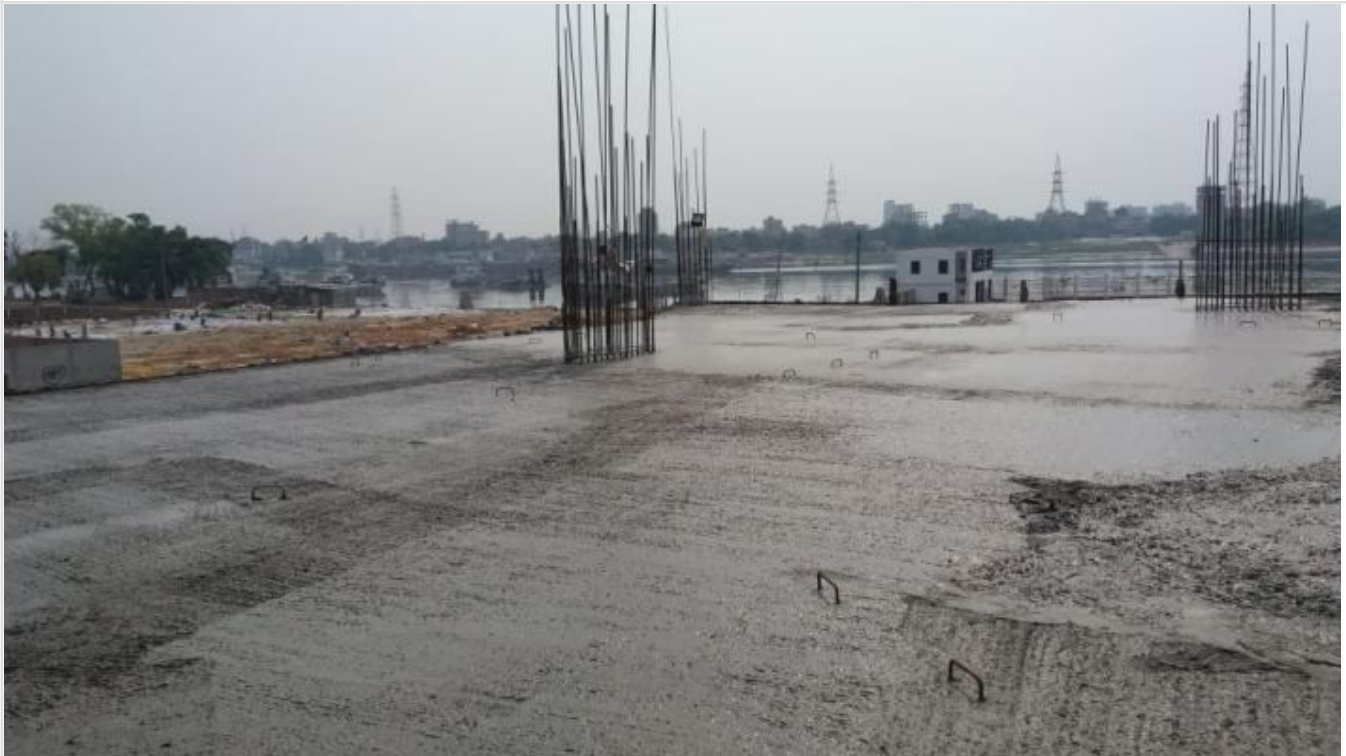
Mosque 1st Floor Slab Concreting on 06-04-21
