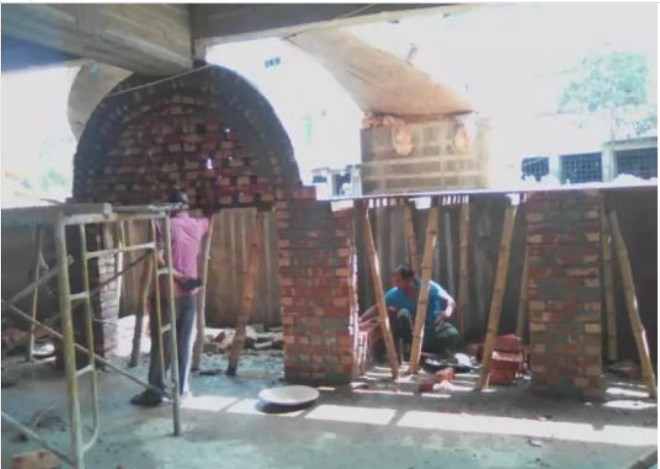
Mosque-Ground Floor Ancillary Works on 14-04-21
