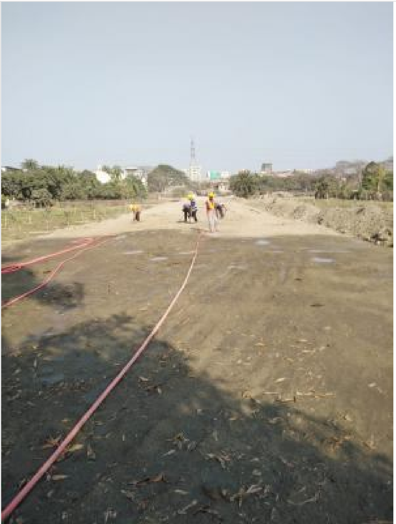
40 ft Road Dressing and Levelling on 28-02-21
