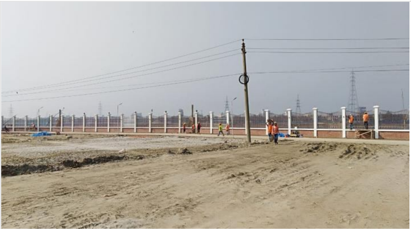
Riverside Boundary Fencing on 08-02-21
