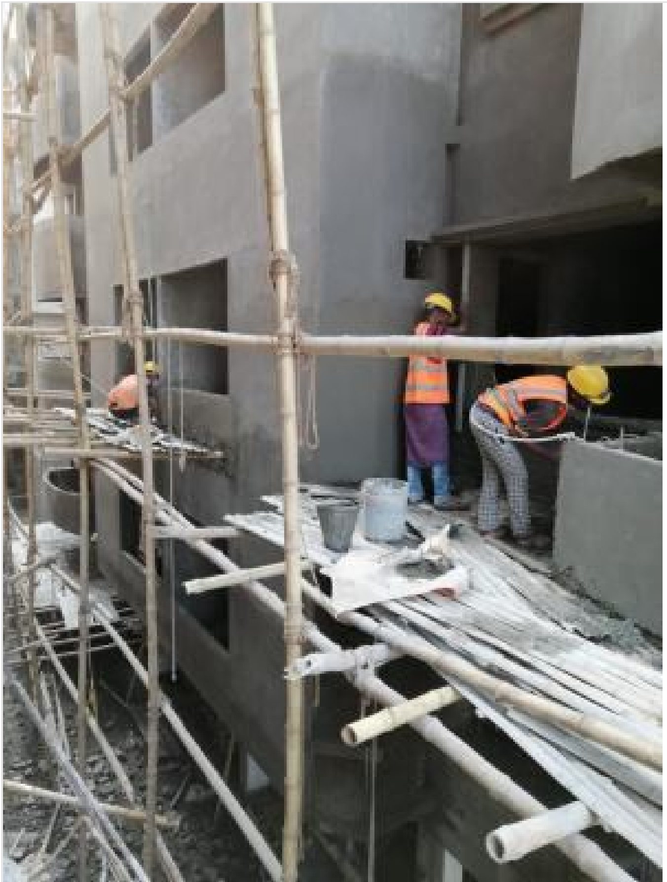
Bulding-Q-Out-side Plastering on 09-05-21
