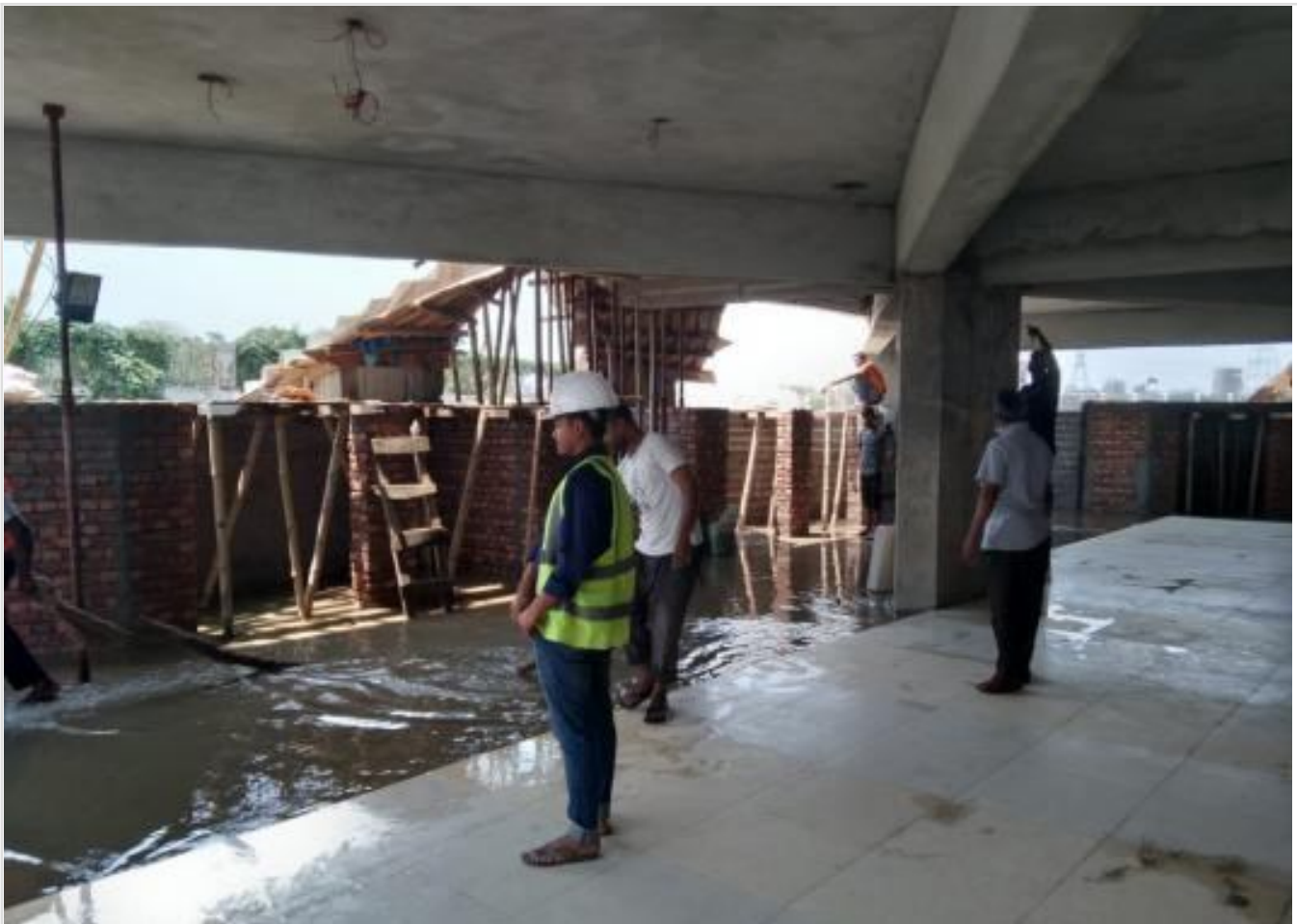
Mosque-Basement-Tile Work on 16-04-21
