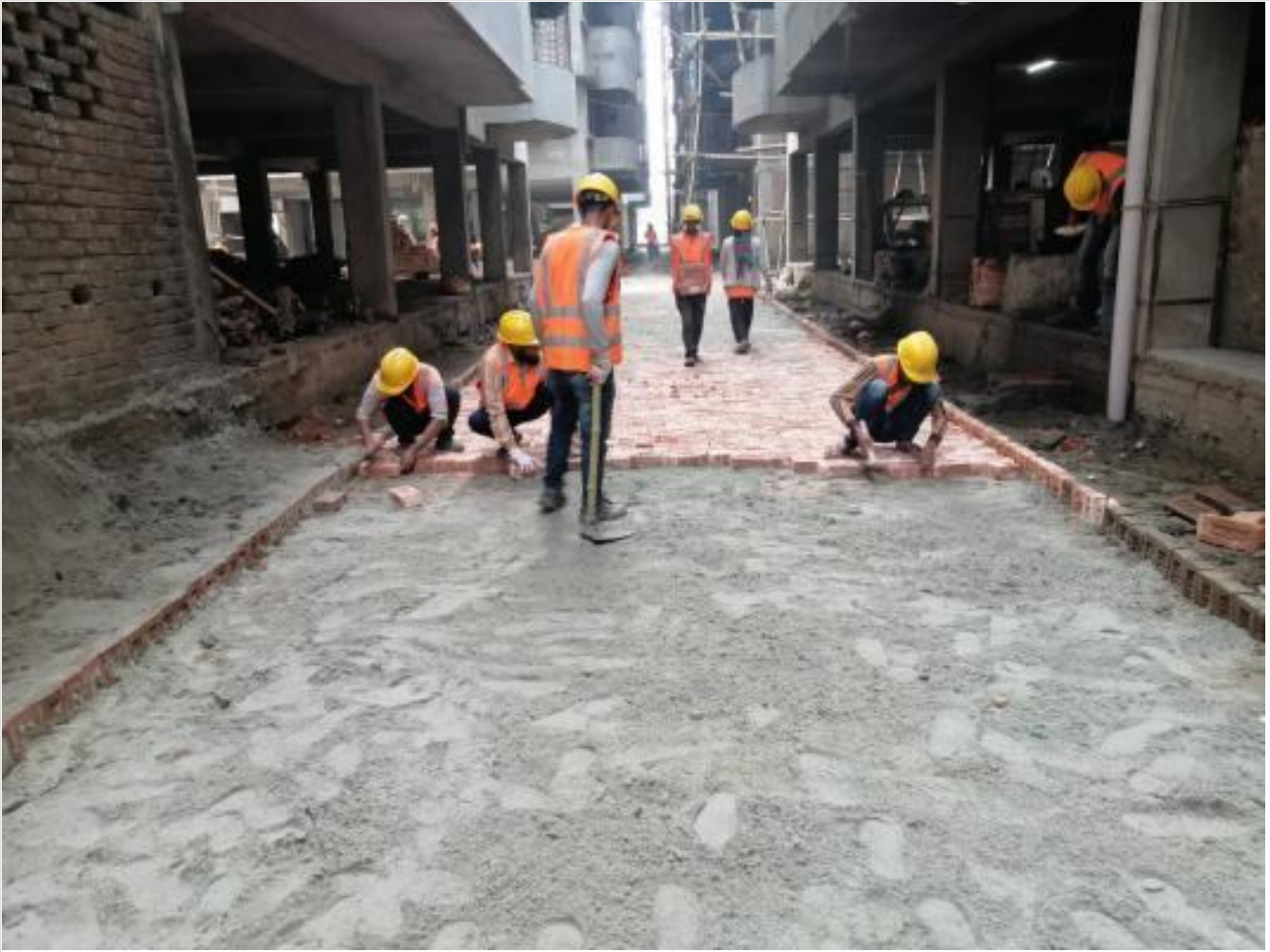
Inner Road CC Work on 27-01-21
