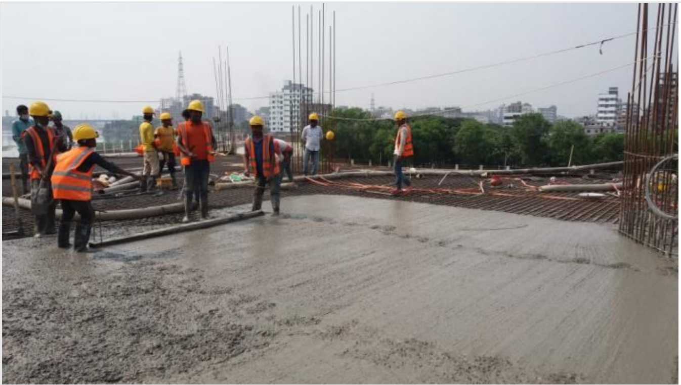
Mosque 1st Floor Slab Concreting on 06-04-21
