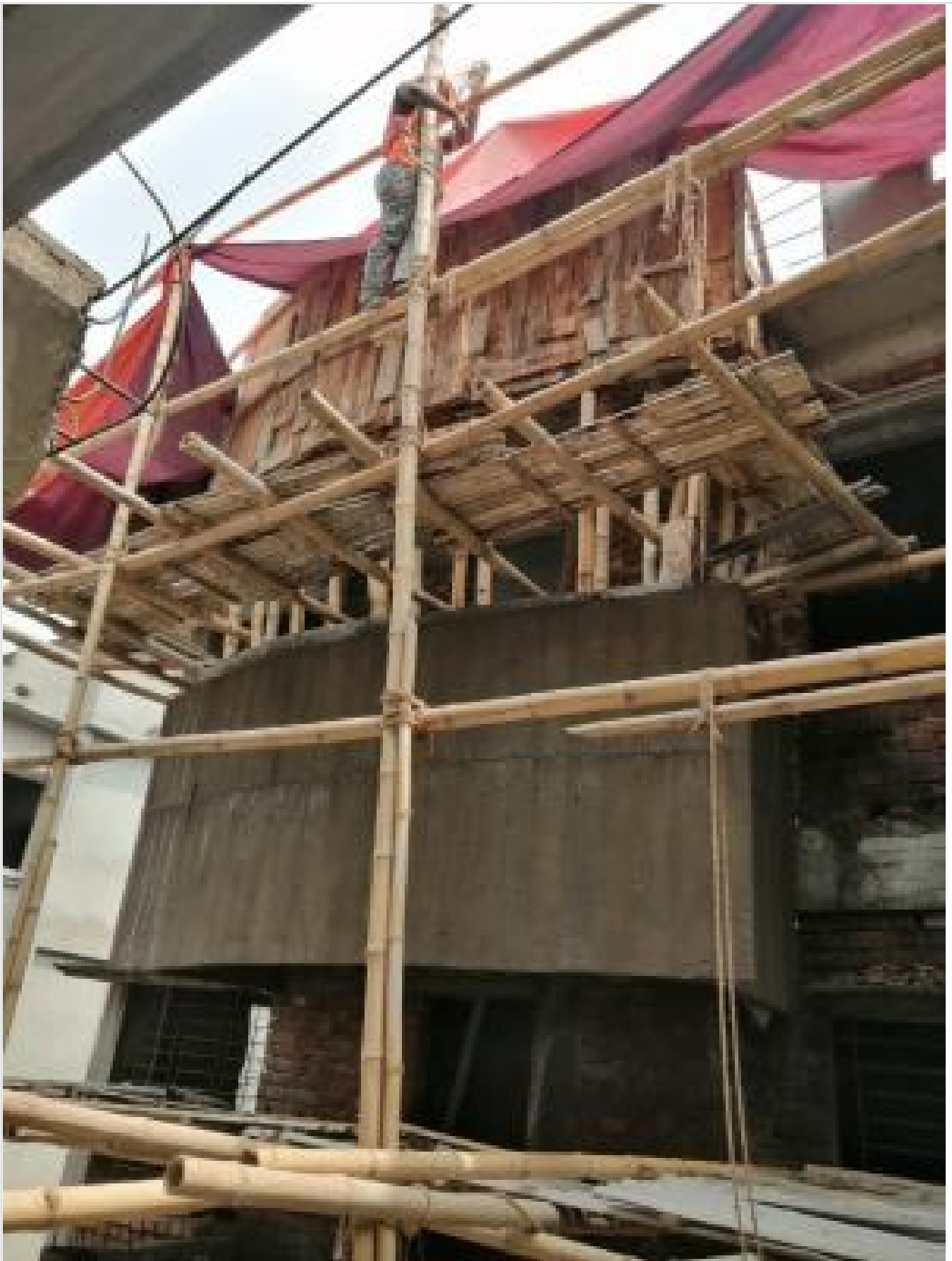
Drop Wall Shuttering on 28-04-21
