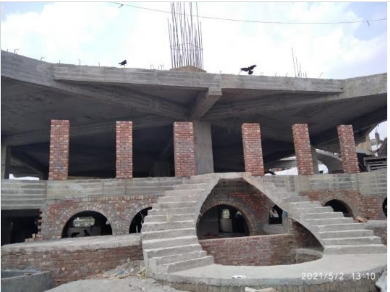
Mosque-Gr./1st Floor-Ancillary Works on 02-05-21
