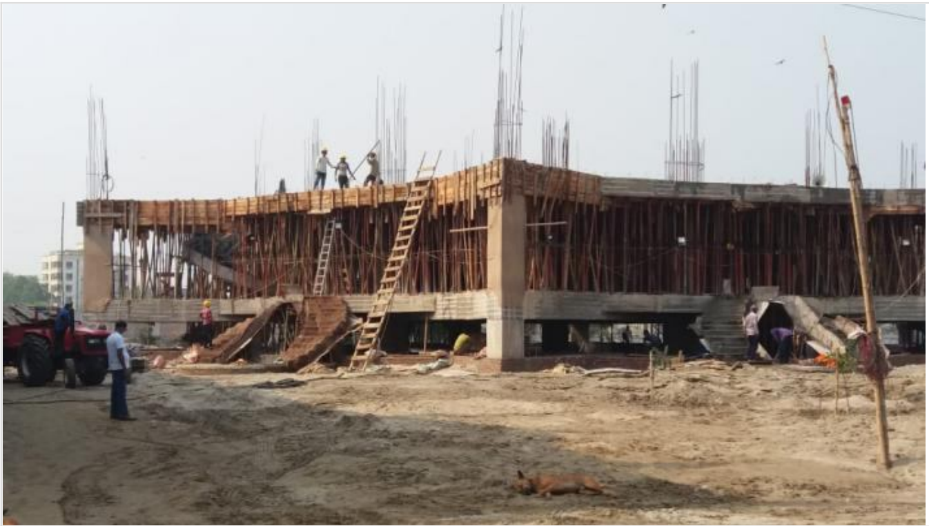
Mosque under Construction on 13-04-21
