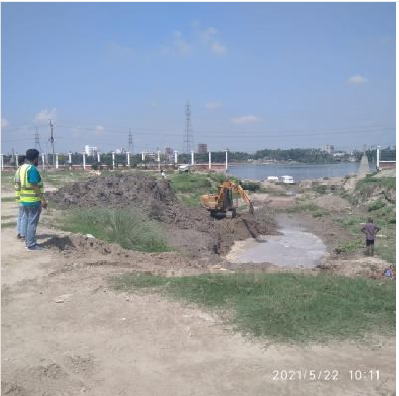
Landing Station-Excavation on 22-05-21
