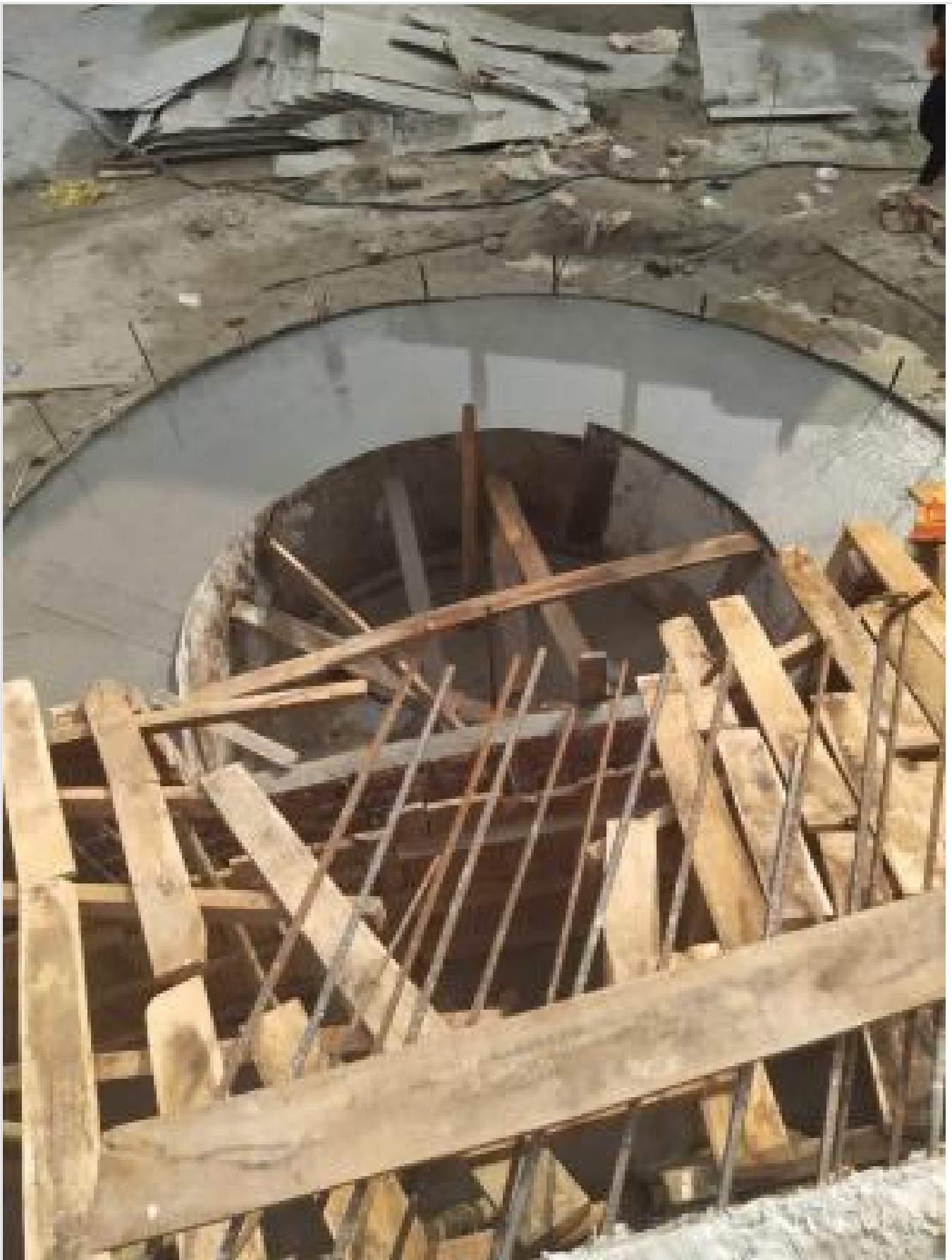
Mosque Ground Floor Stair Concreting on 27-03-21
