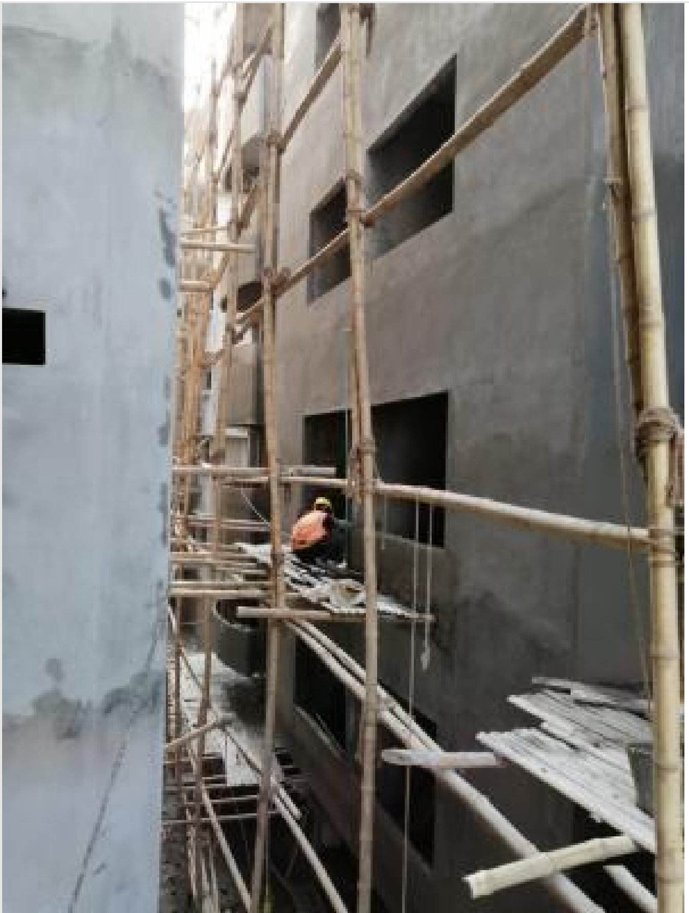
Bulding-Q-Out-side Plastering on 09-05-21
