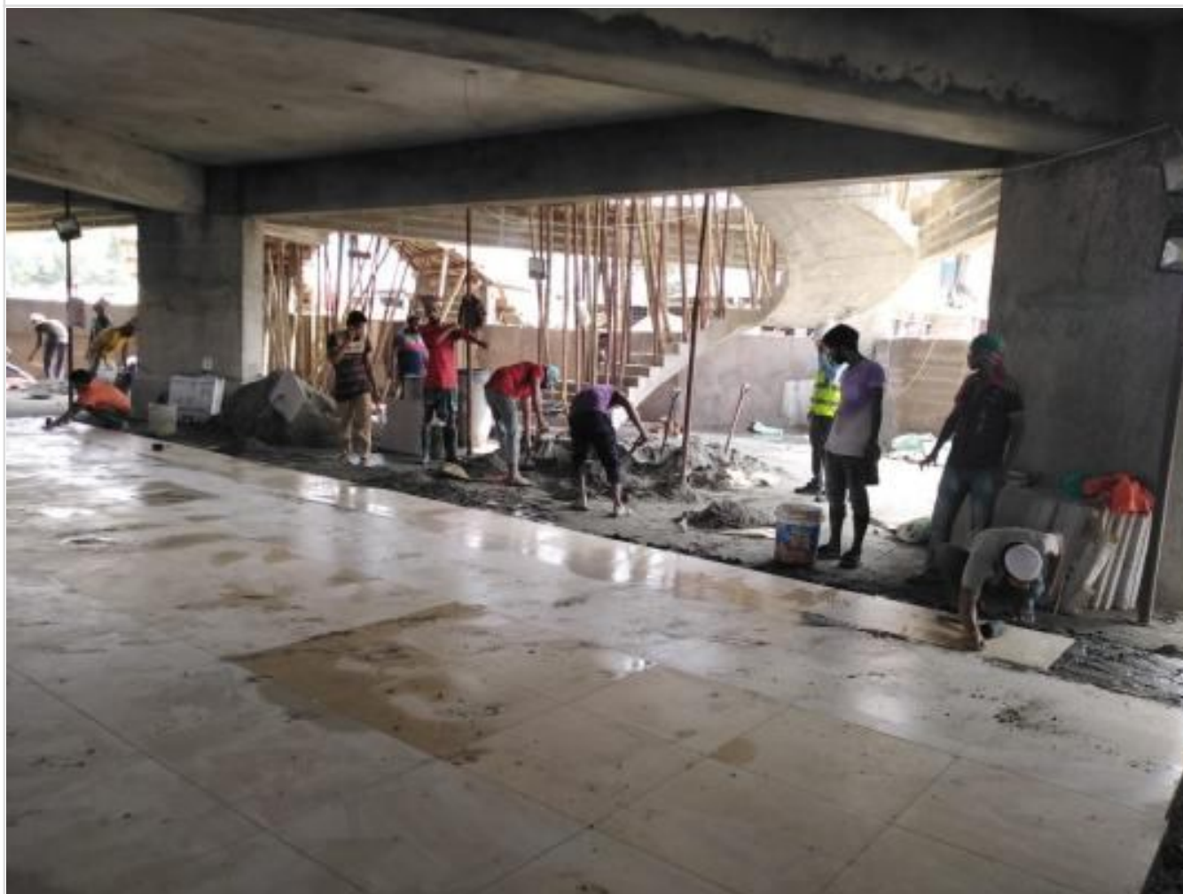
Mosque-Basement-Tile Work on 12-04-21
