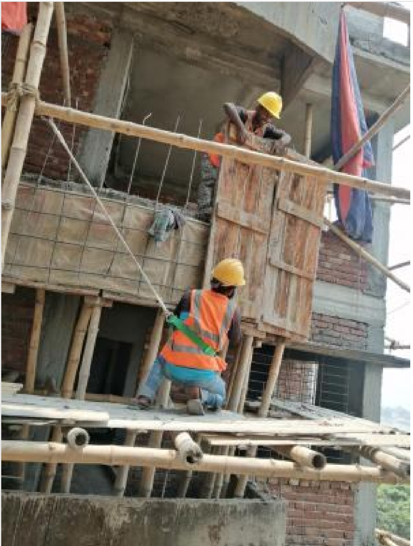
Drop Wall Shuttering on 01-05-21
