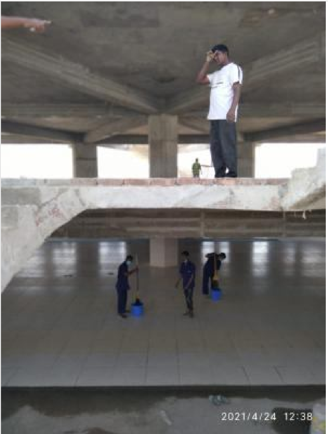
Mosque-Gr.Floor Roof De-shuttering on 24-04-21
