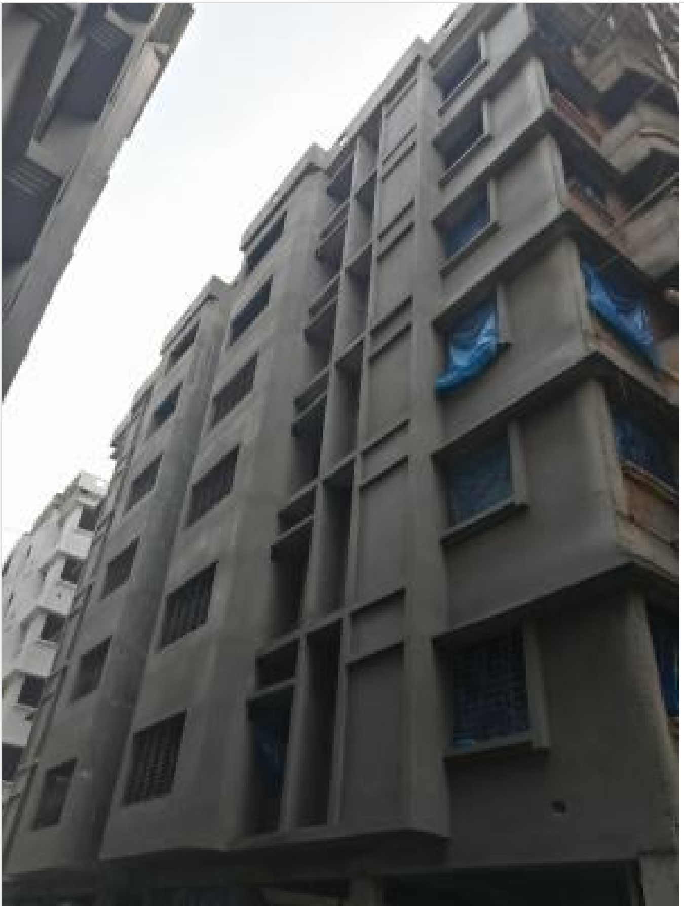
Building-J outside plastering on 28-01-21
