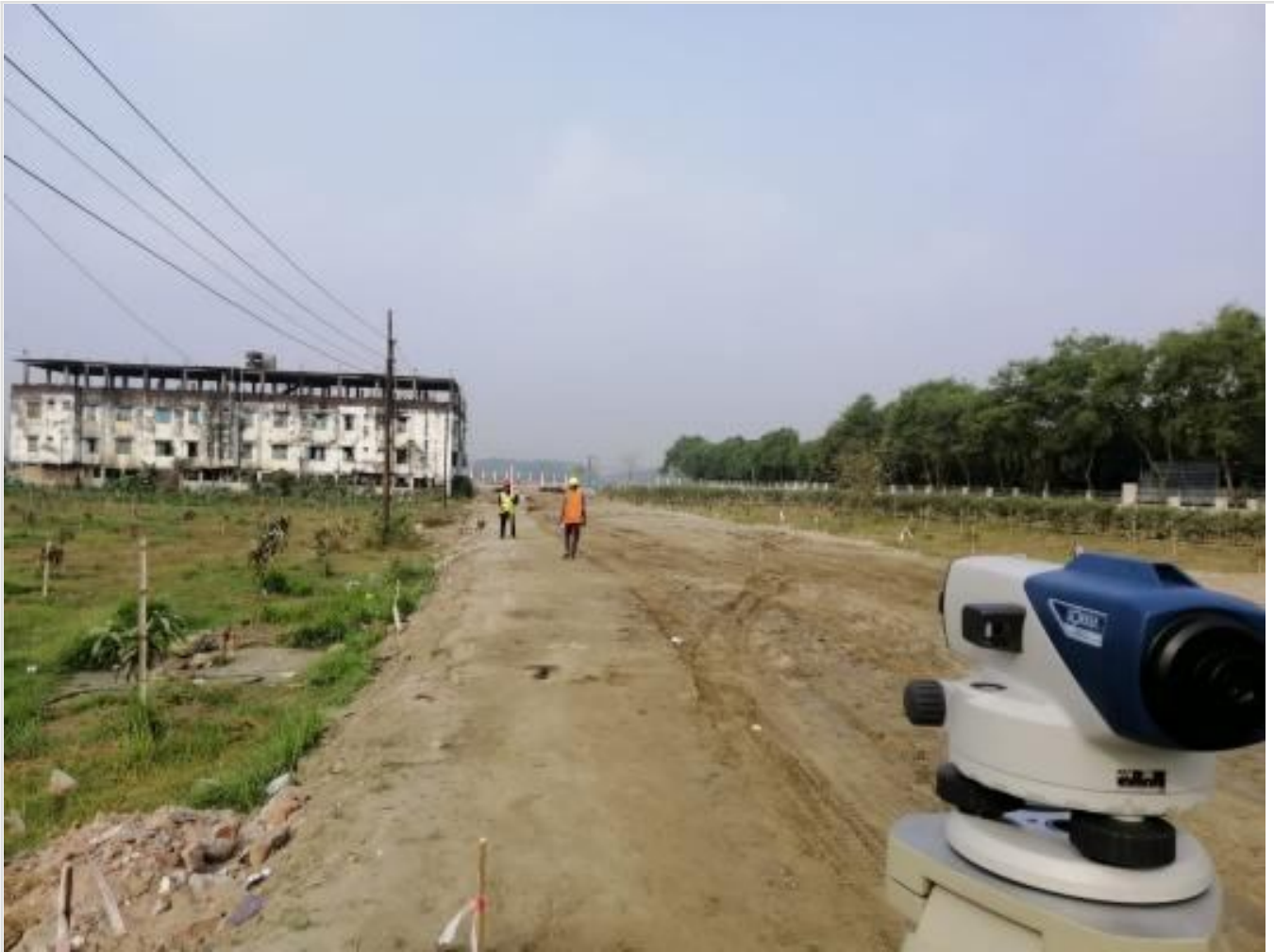
40 ft Road Dressing and Levelling on 01-03-21
