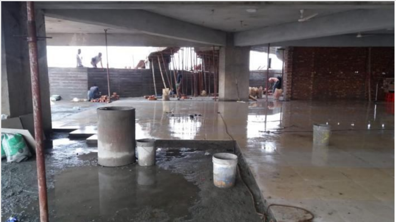
Mosque-Basement-Tile Work on 13-04-21
