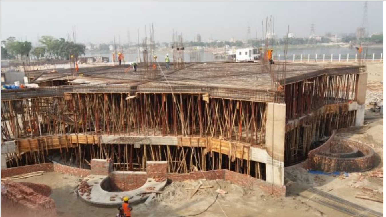
Mosque Building in Construction on 03-04-21
