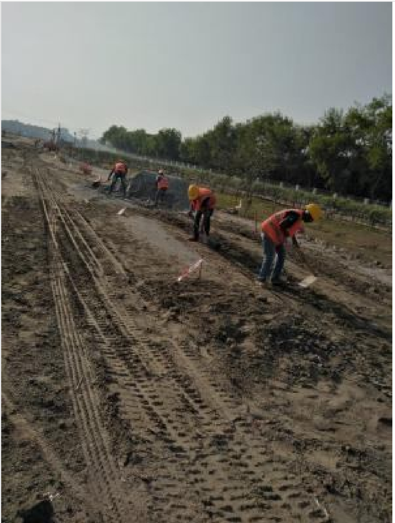
40 ft Road Levelling and dressing on 10-02-21
