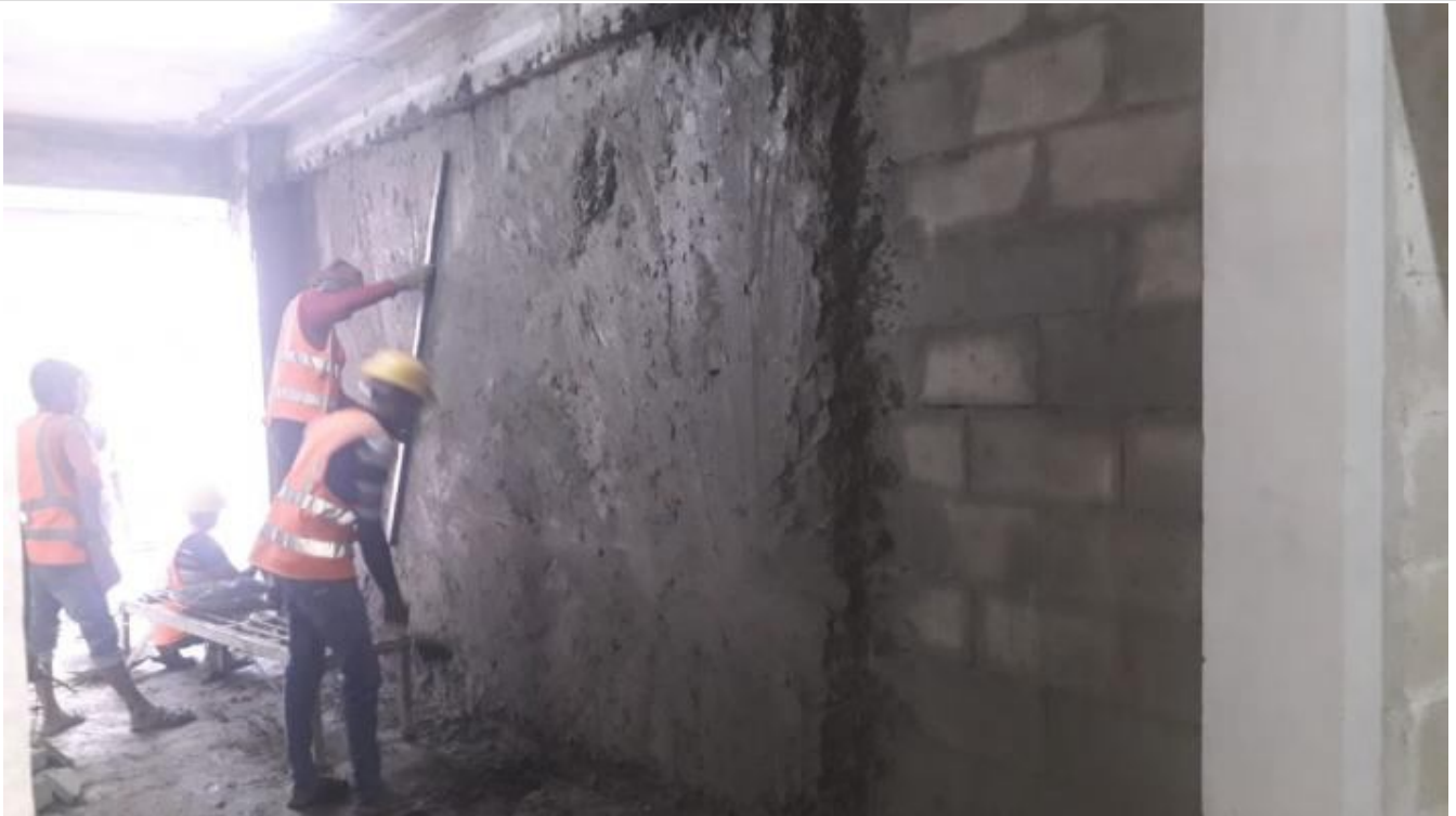
5F Car Lift West Wall Plastering
