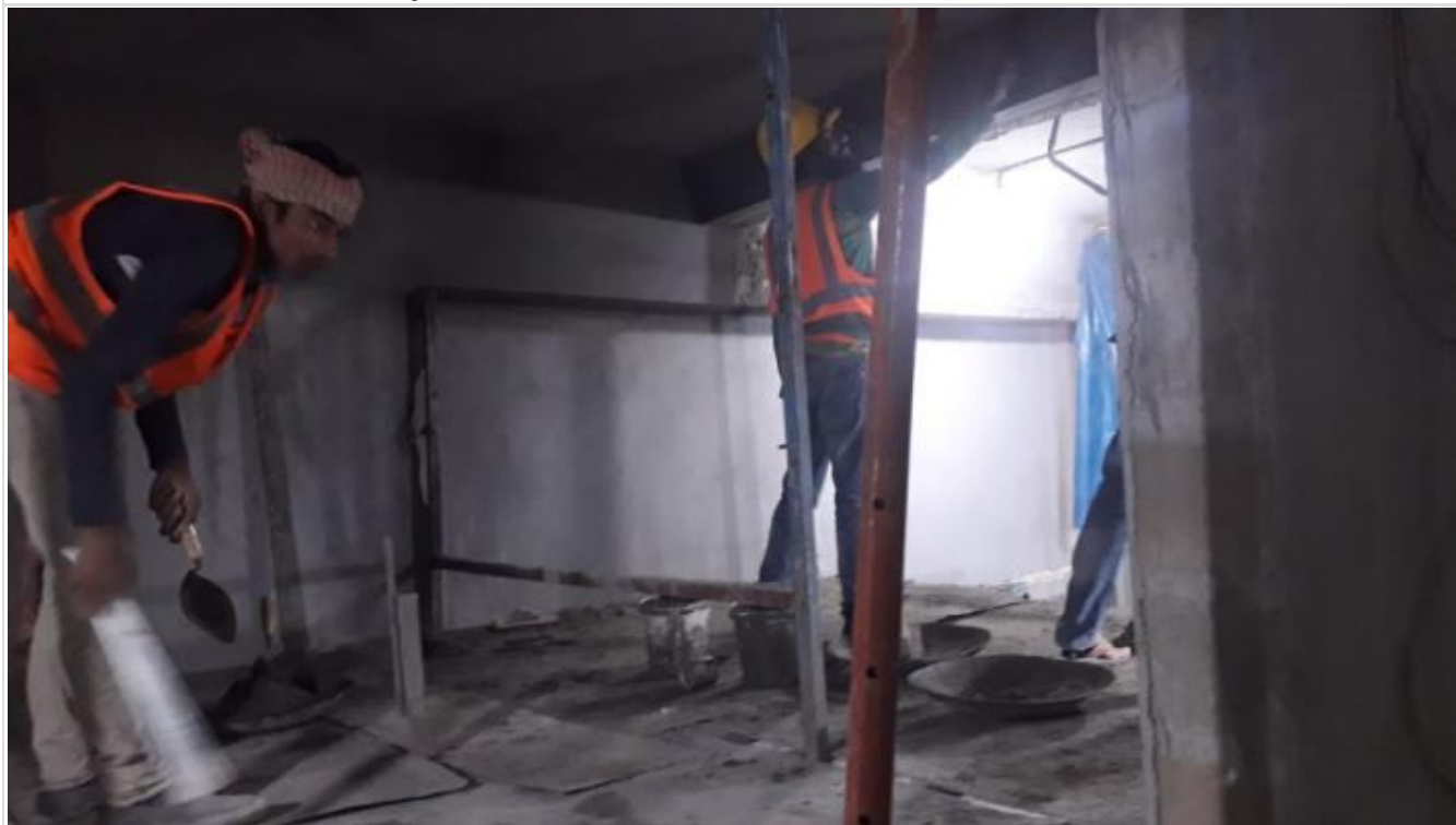
6F-Drive-way Beam Plaster
