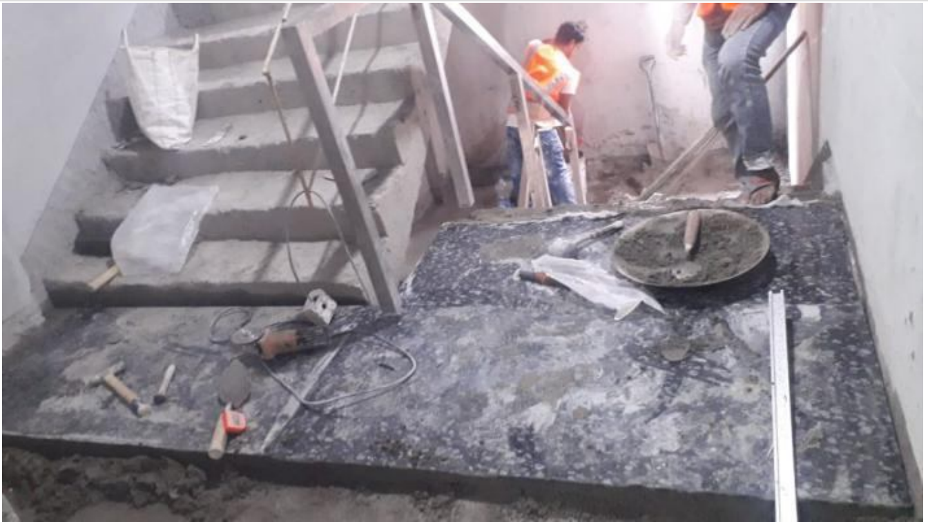
4F-Stair Marble Fixing
