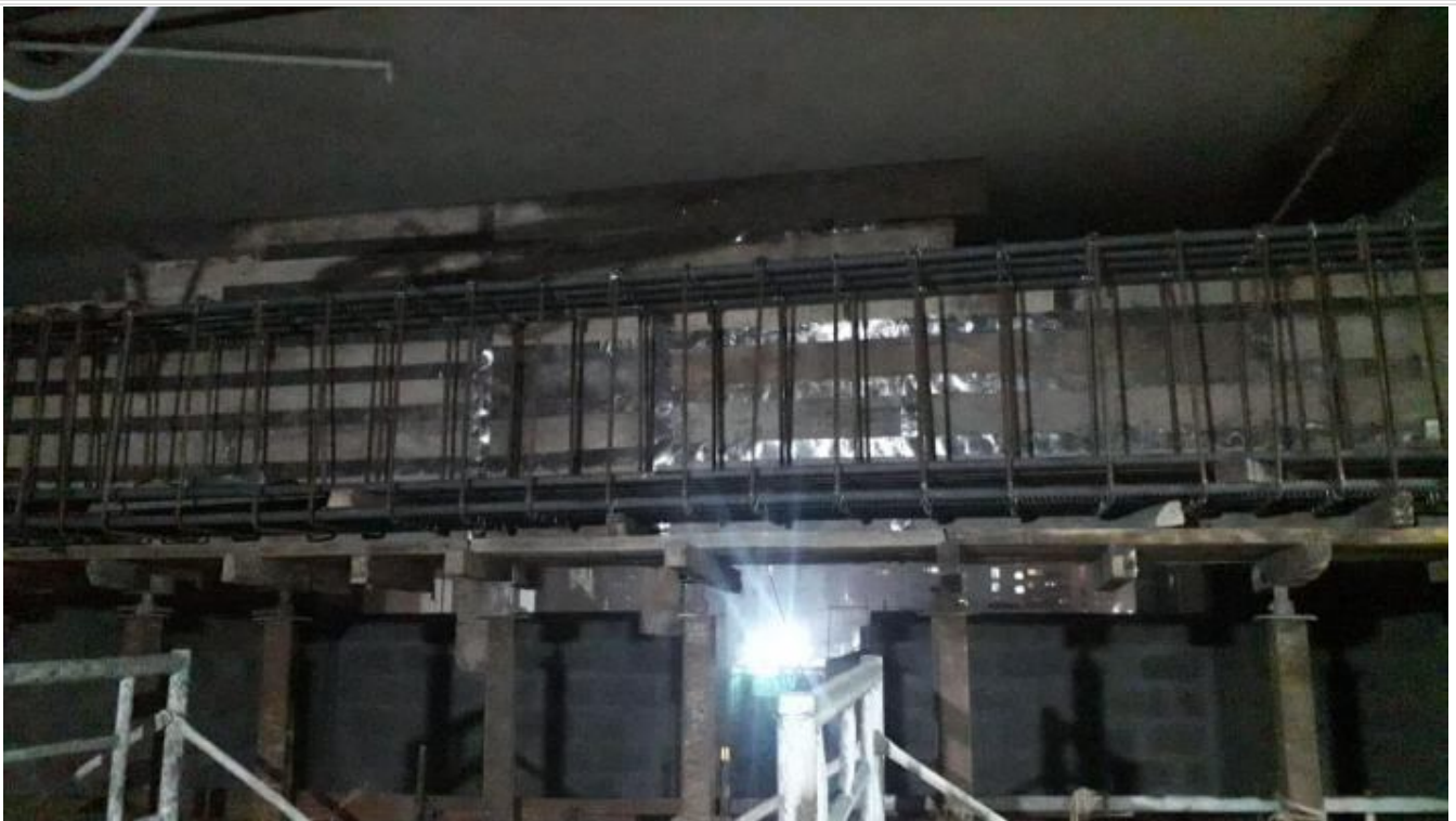
8F-Car Lift Beam Re-bar Work
