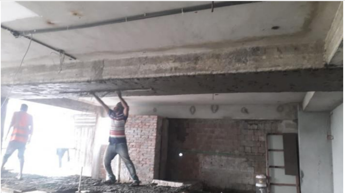
6F Parking Zone Beam Plaster
