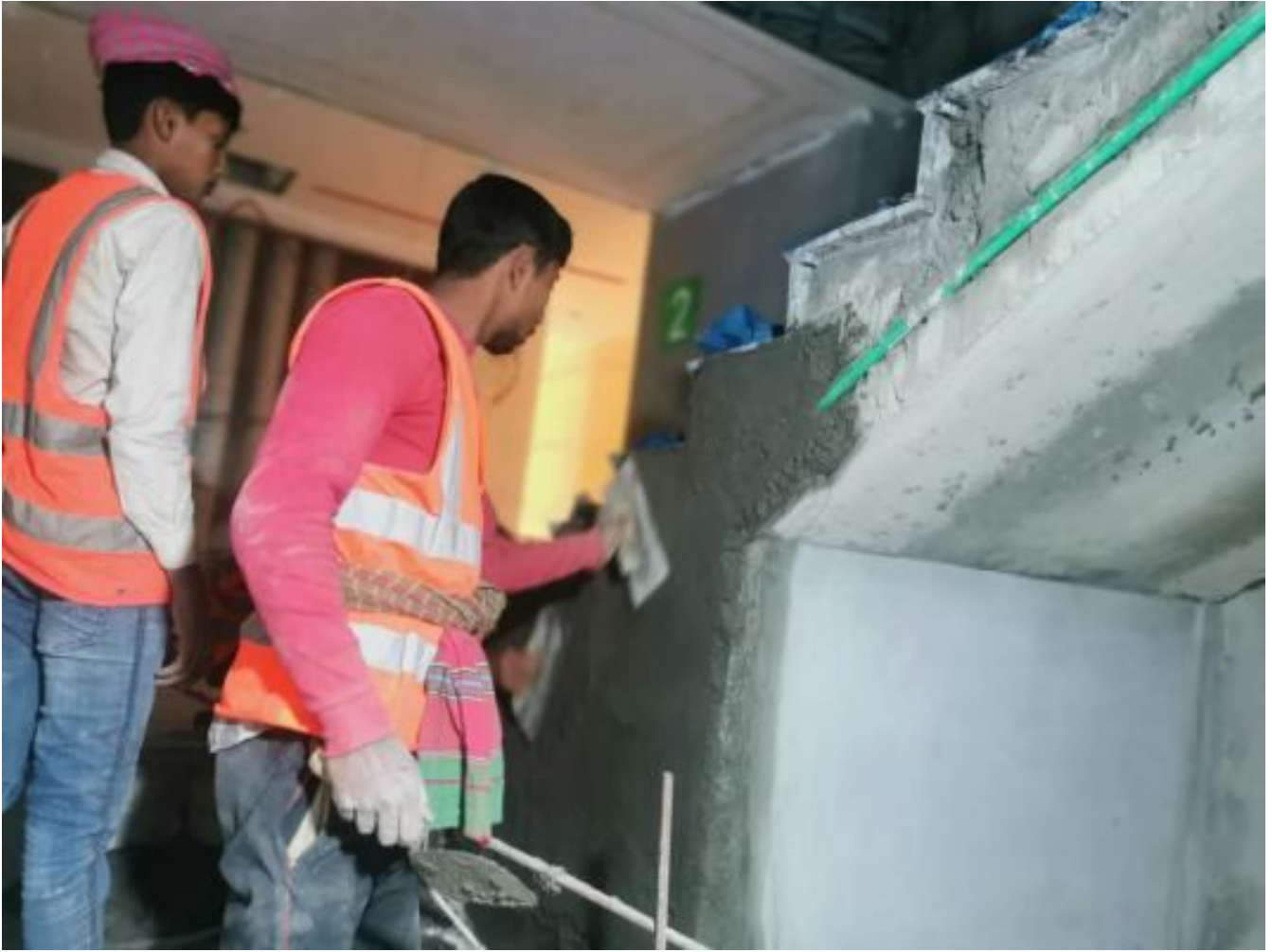
South Stair Side Plaster
