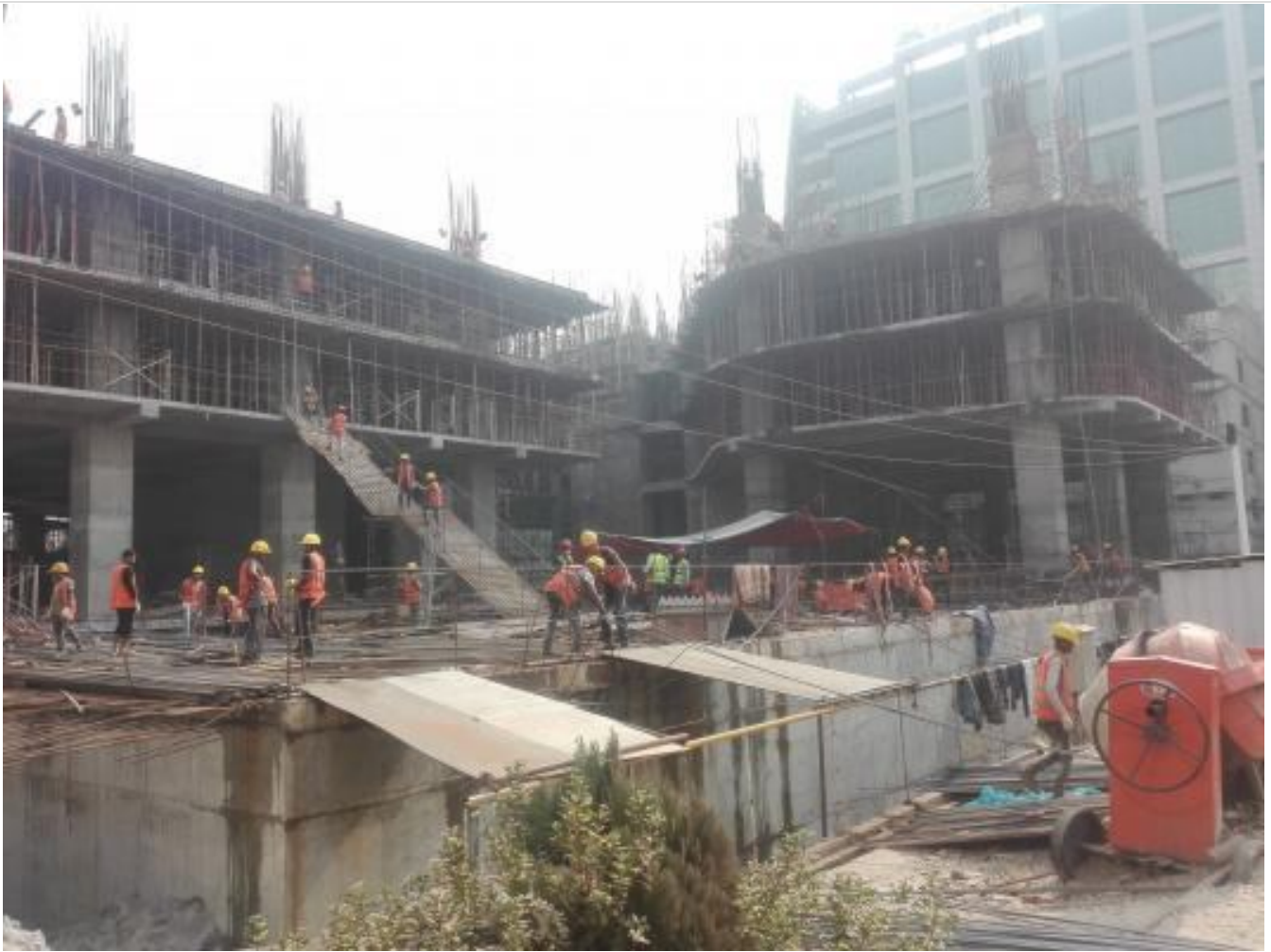
7F-Parking Zone Beam Plaster
