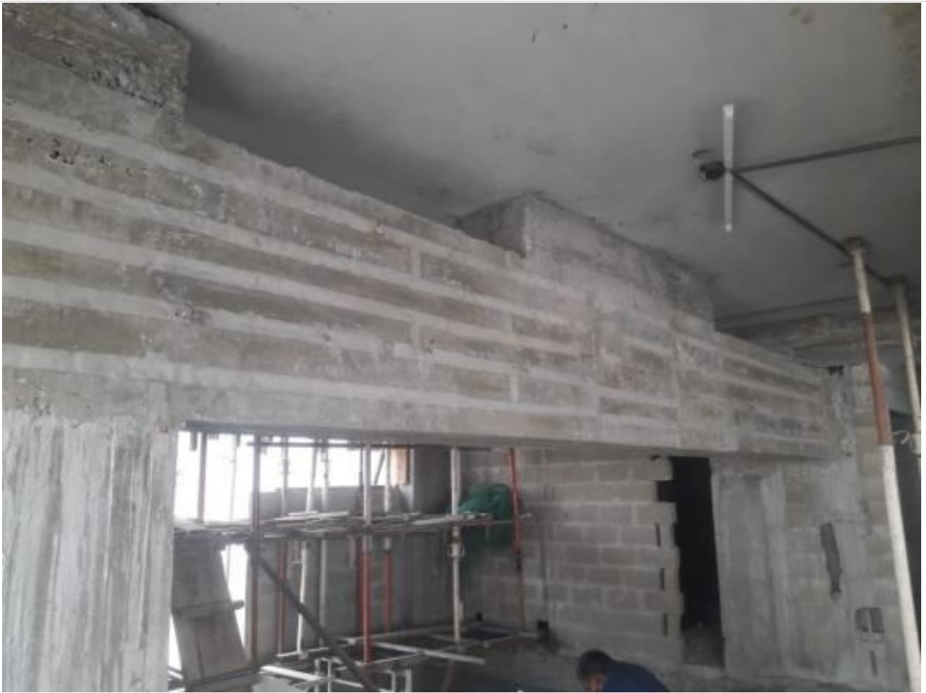
8F Car Lift M/c Room Extra Load Bearing
