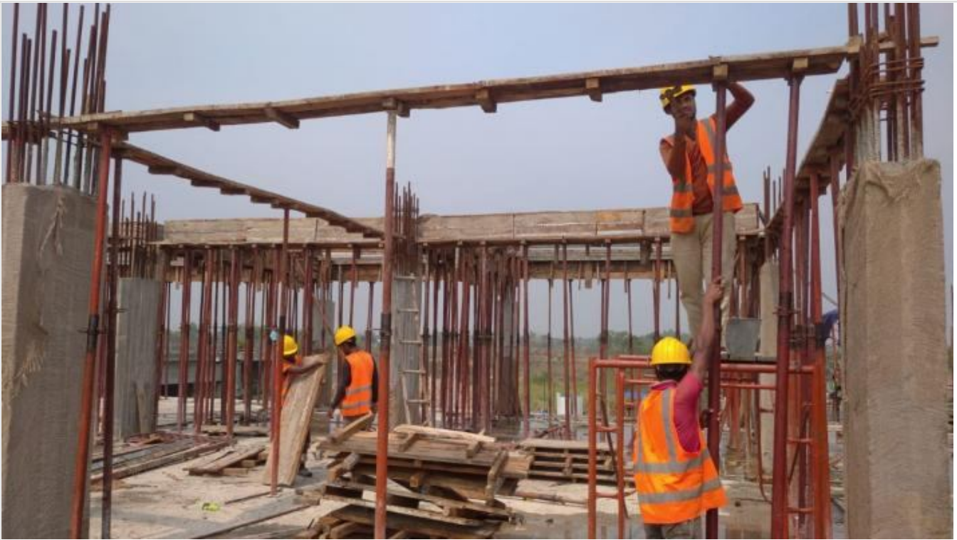
Beam Shuttering on 03-05-21
