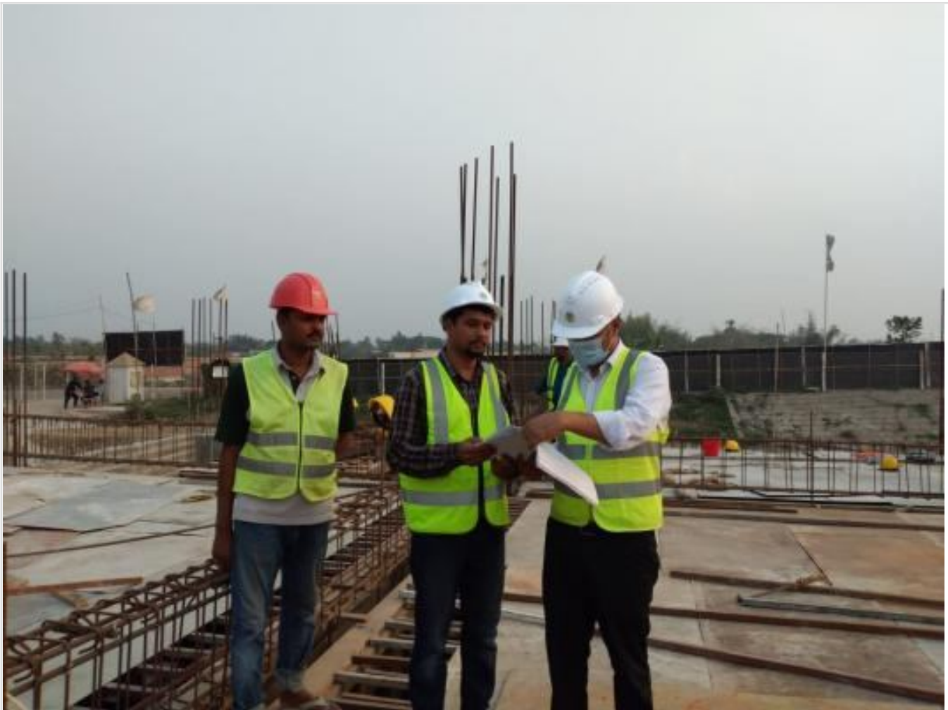
GF Slab Re-bar Inspection on 07-03-21
