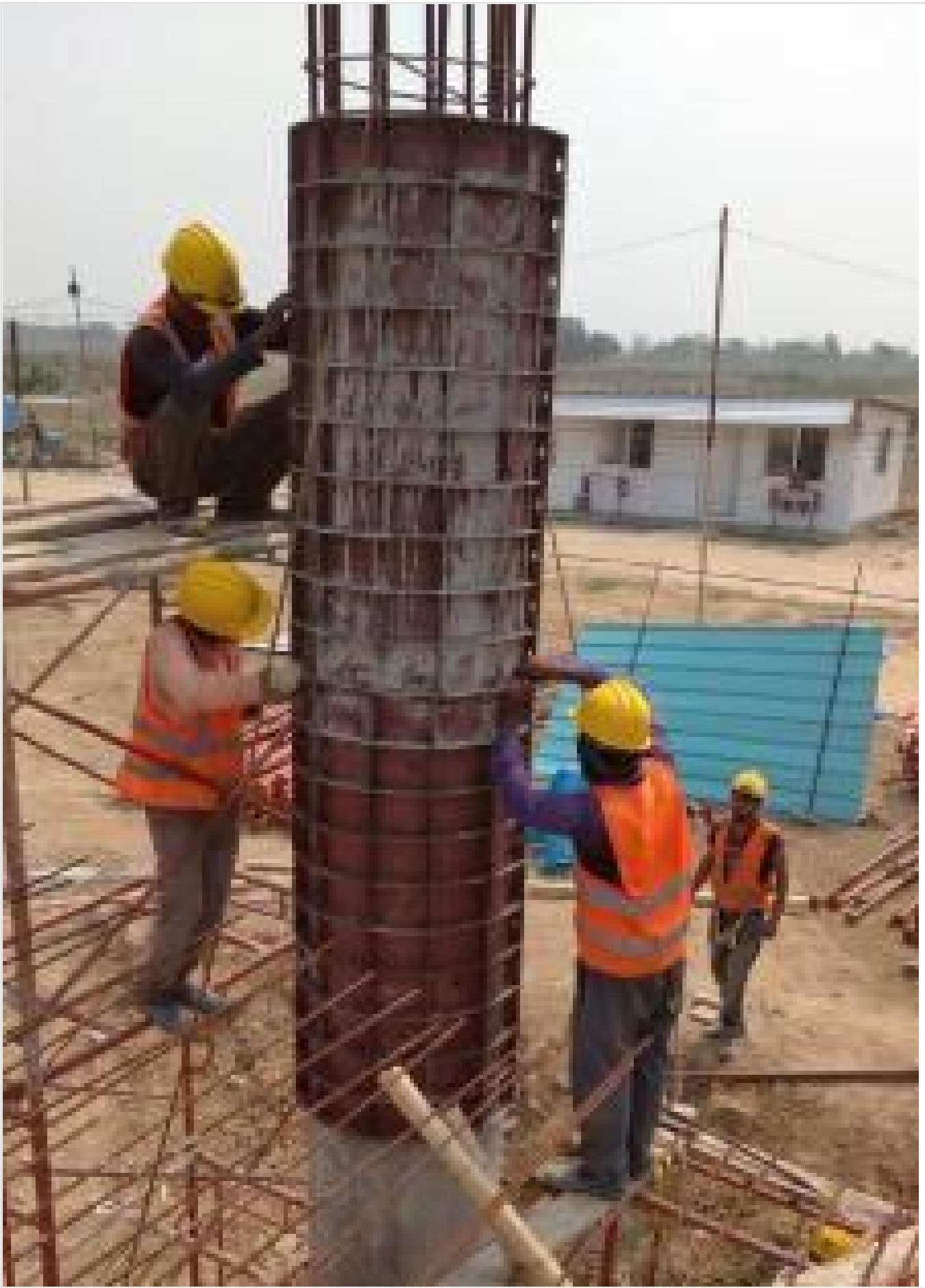
Column Shutteeing on 30-04-21
