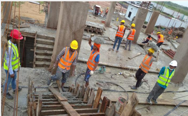
Ground Floor Stair Concreting
