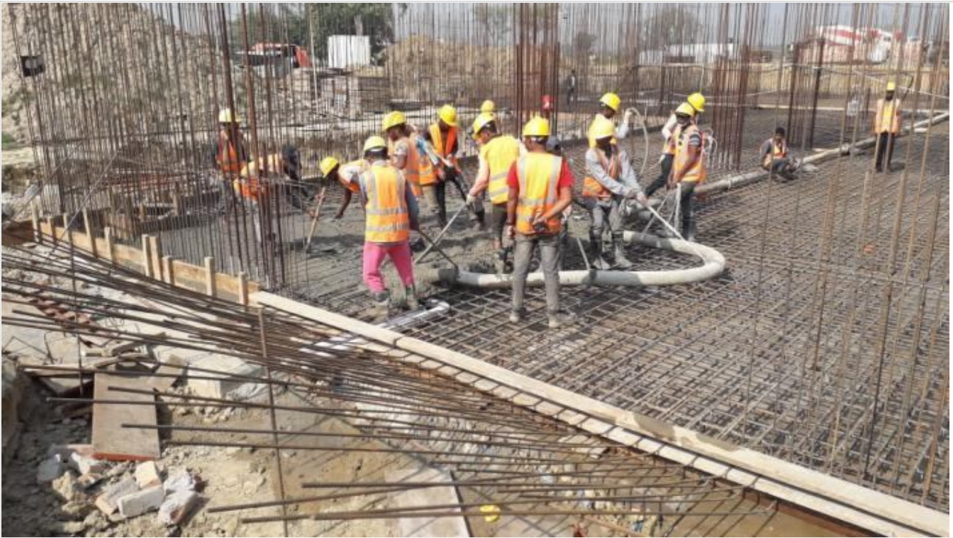
Mat Concreting on 05-01-21
