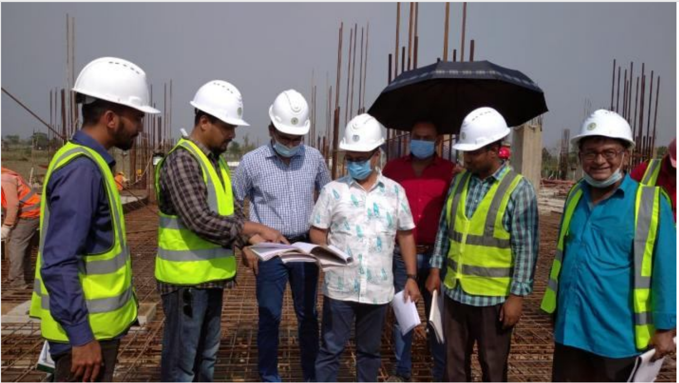
Inspection before GF Slab Concreting on 25-04-21
