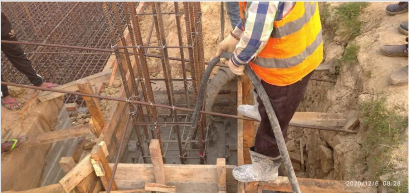
Pile Cap Concreting on 06-12-20
