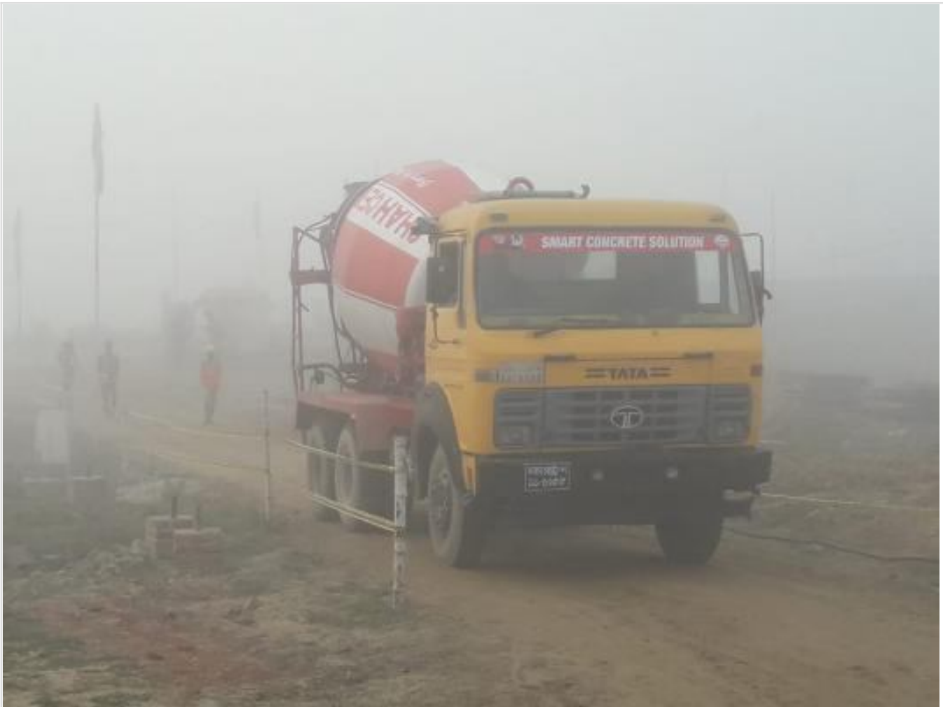
Pile Cap Concreting on 06-12-20
