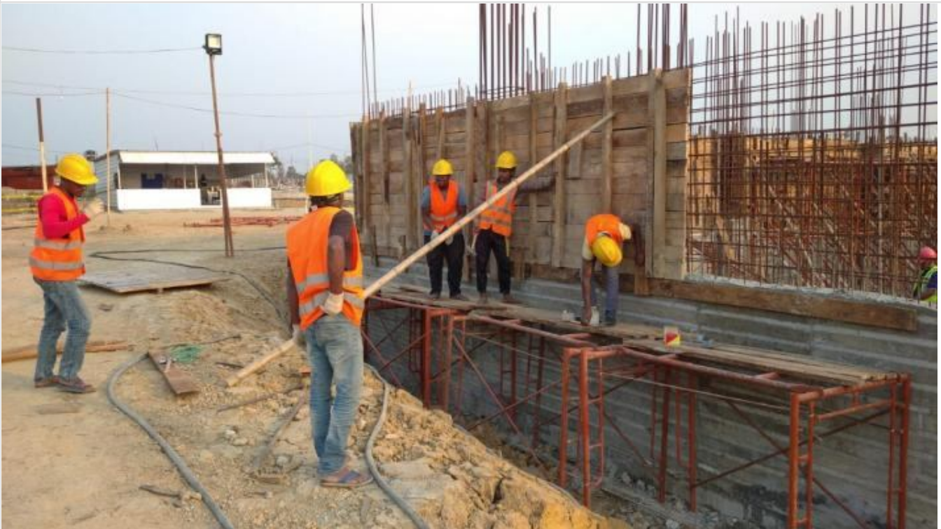
Retaining Wall Shuttering on 18-02-21
