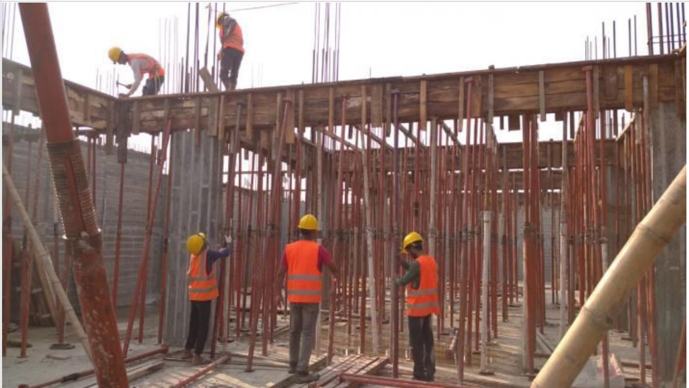
Ground Floor Slab Shuttering on 25-02-21
