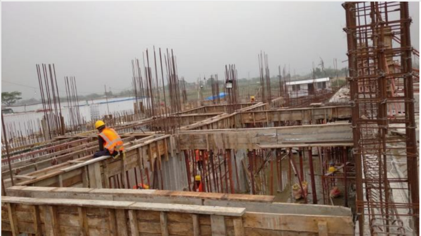
Ground Floor Slab Shuttering on 10-04-21
