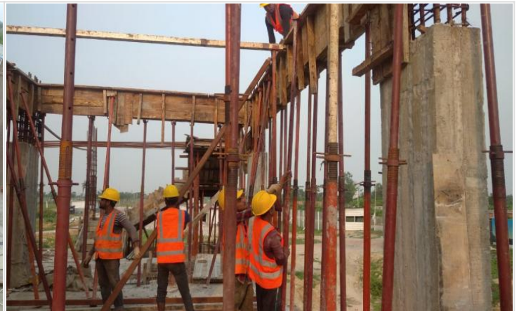
Ground Floor Roof Slab Shuttering
