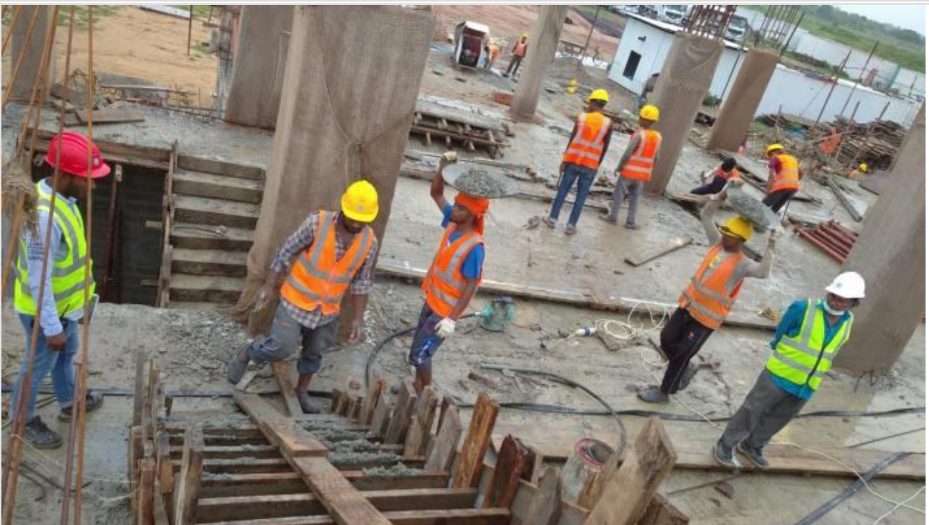
Ground Floor Stair Concreting on 31-05-21
