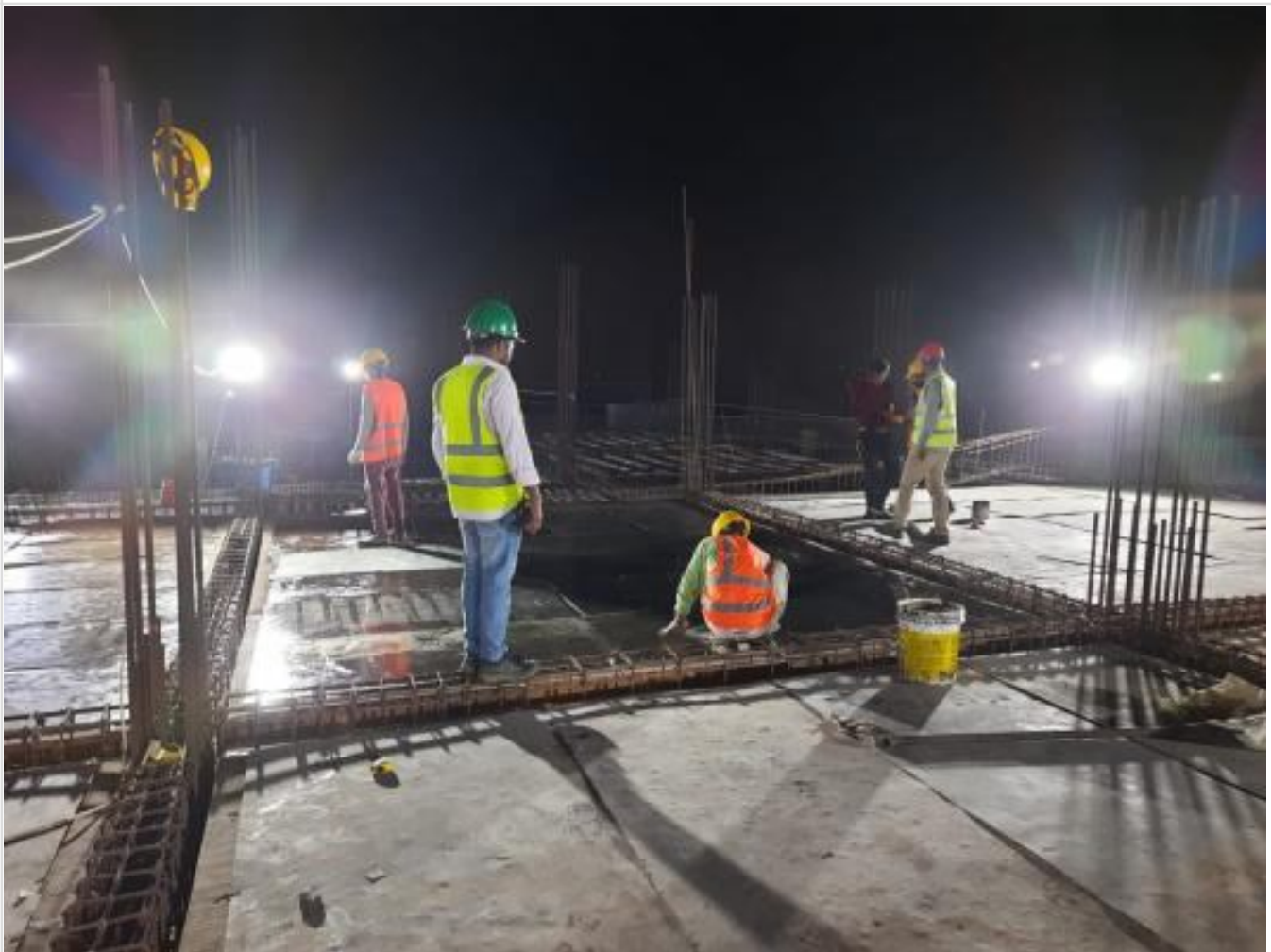
GF Slab Shuttering at Night Shift on 10-03-21
