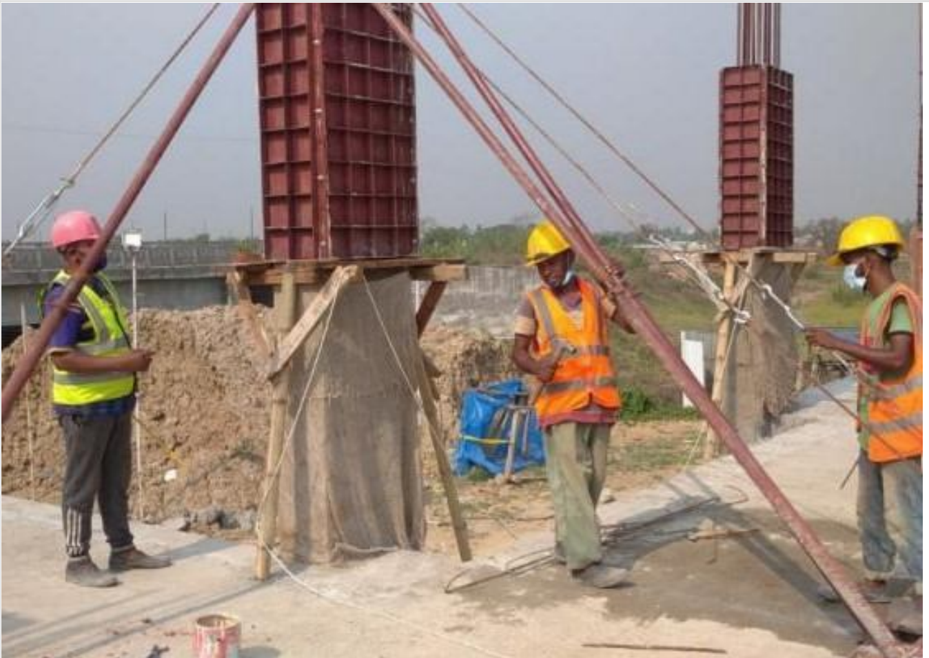
Column Shuttering on 09-05-21
