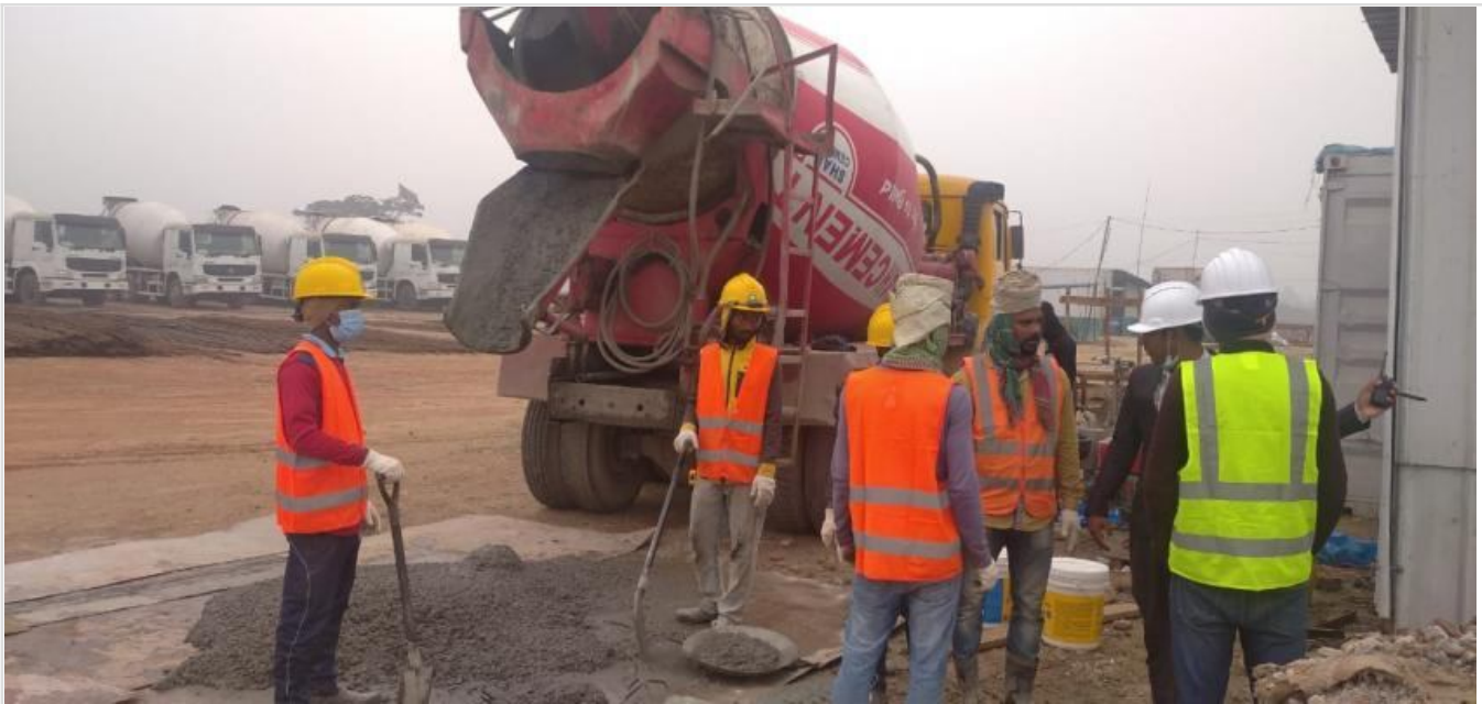
Retaining wall and Column Concreting on 28-01-21
