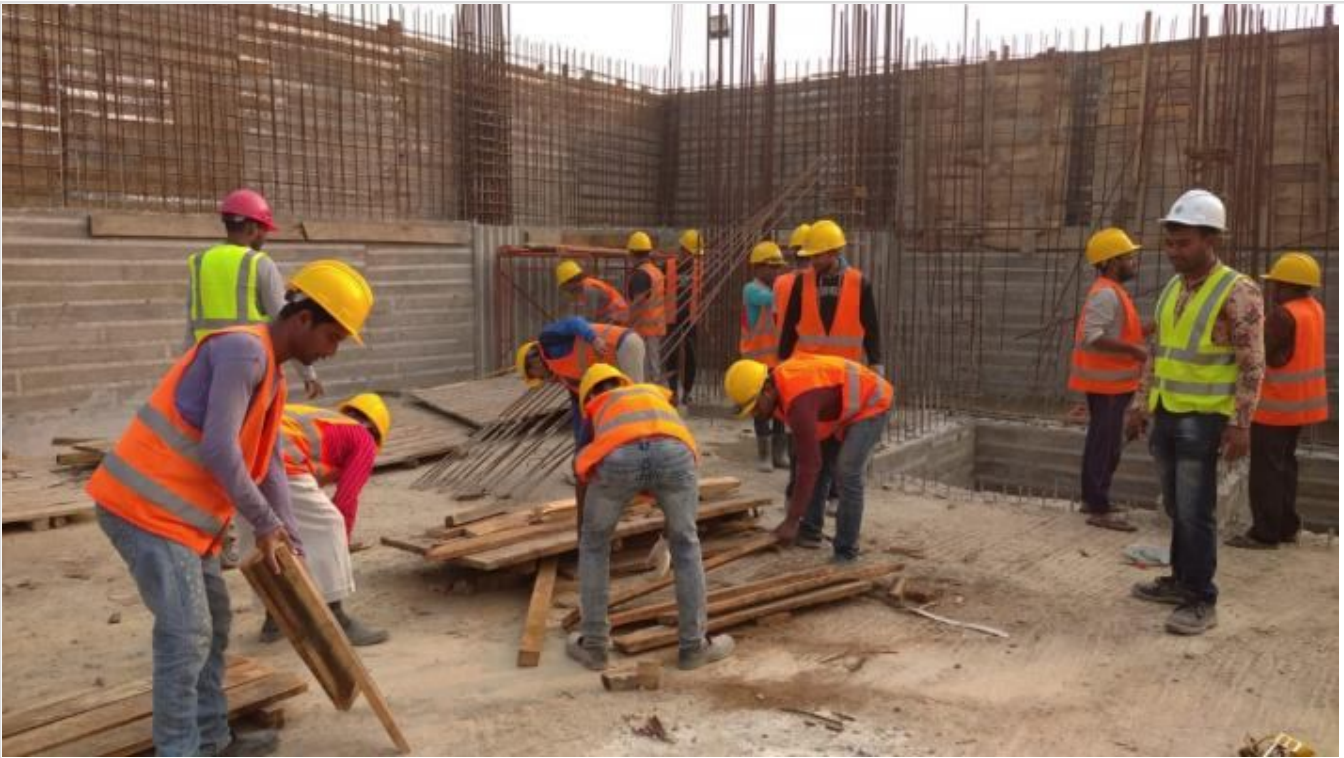
Retaining Wall Shuttering on 18-02-21
