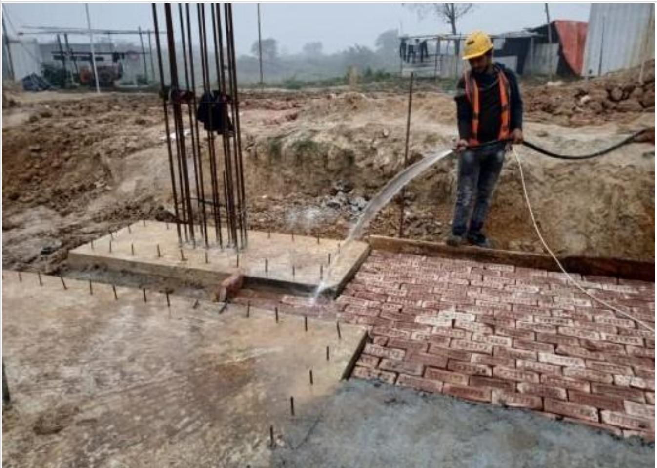
Footing Curing on 15-12-20
