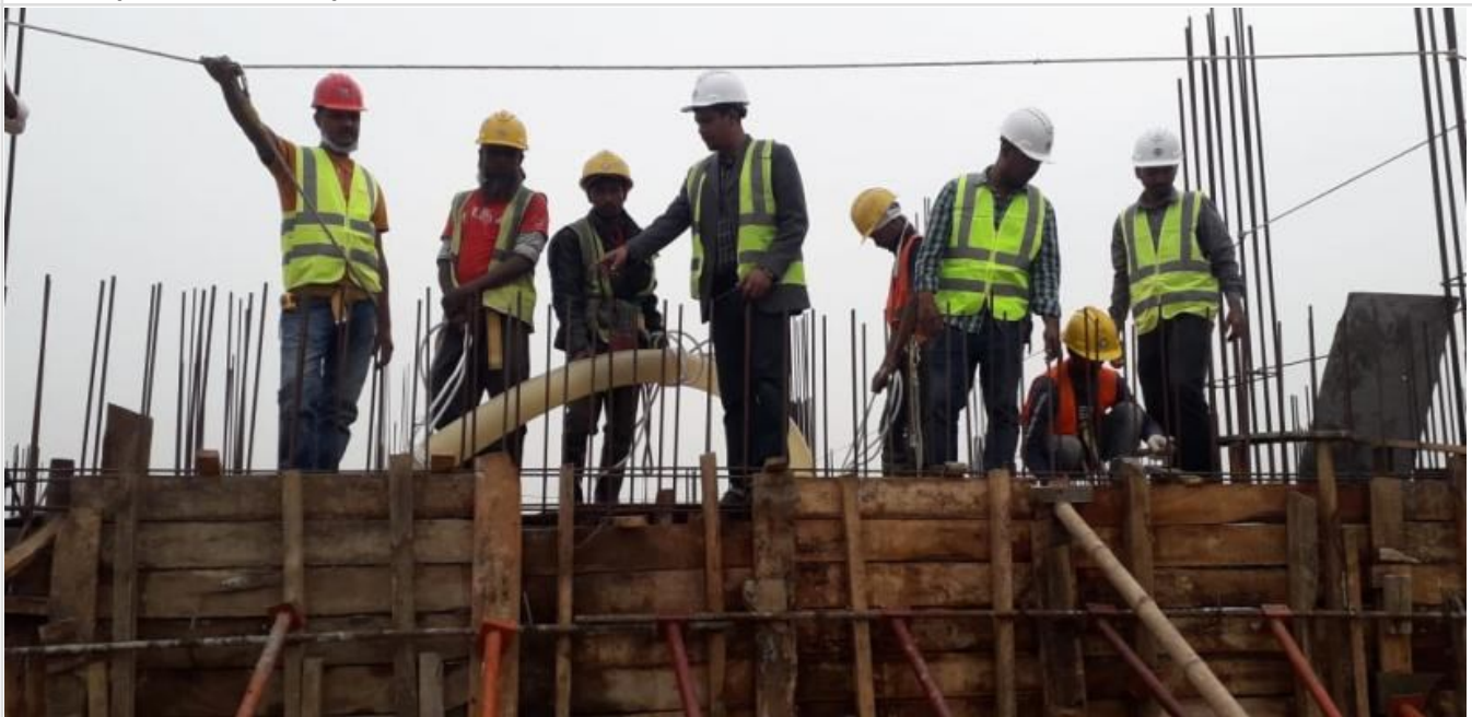
Retaining wall Concreting on 20-02-21
