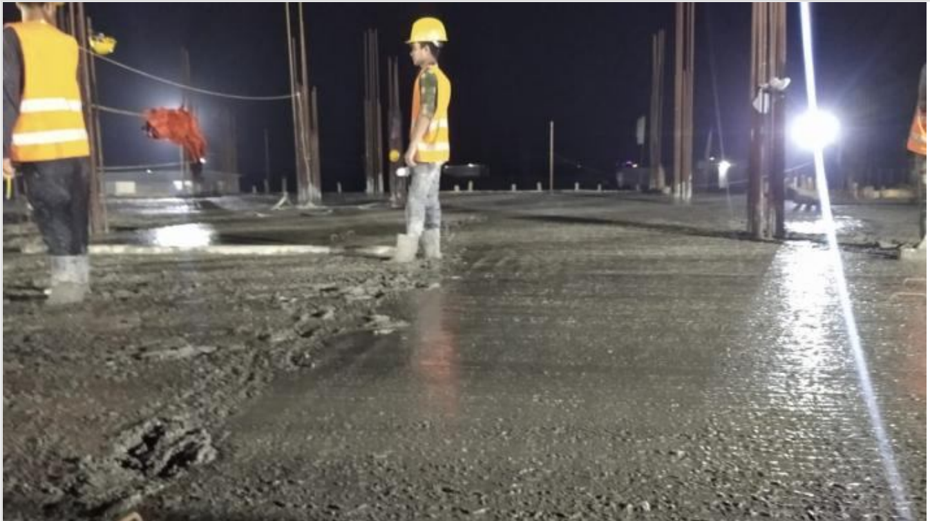
GF Slab Concreting complete at night on 15-03-21
