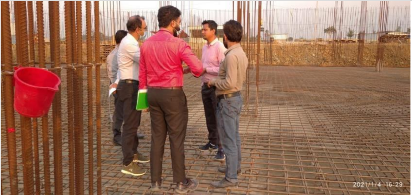
Inspection before Mat Concreting on 05-01-21
