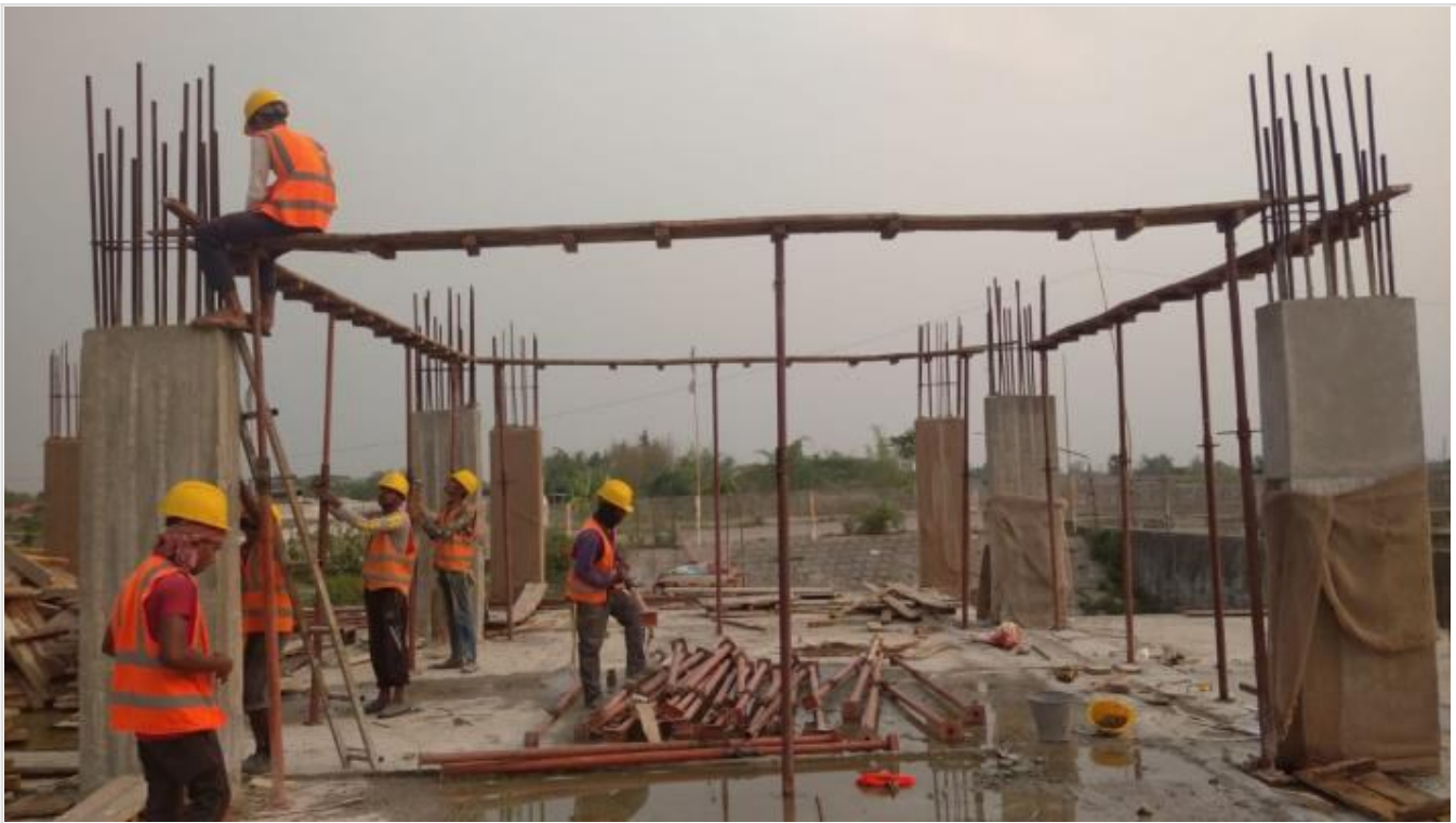
Beam Shuttering on 30-04-21
