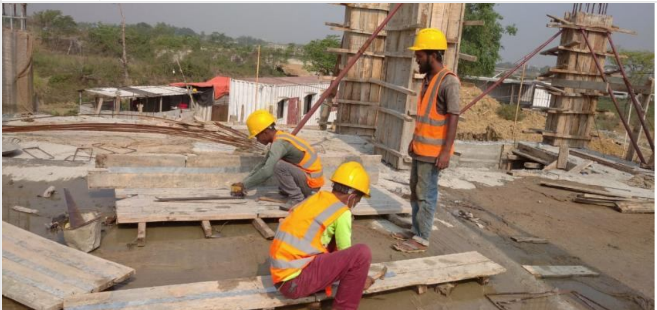
Ground Floor-Column Shuttering Work on 12-05-21
