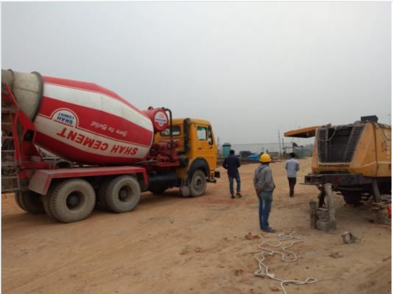
Retaining Wall Concreting on 20-02-21
