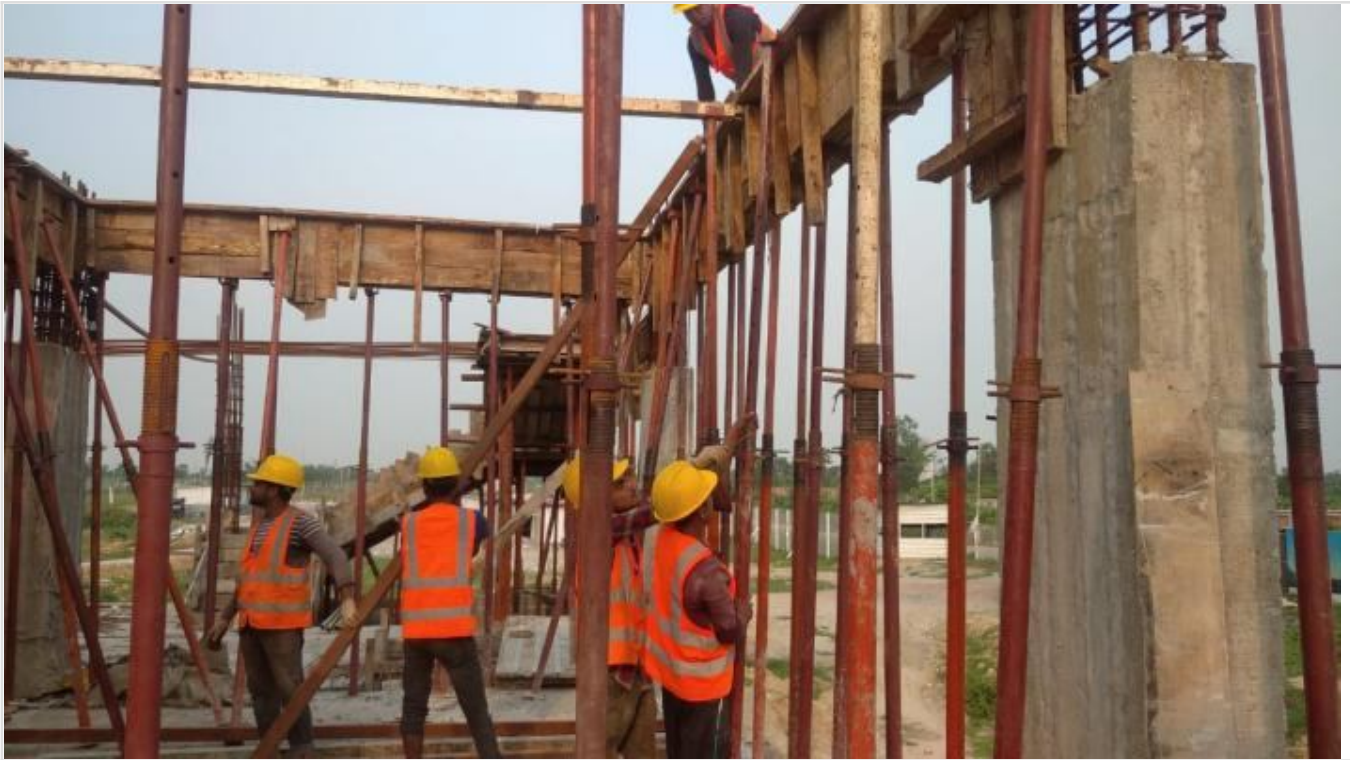
Ground Floor Roof Slab Shuttering on 31-05-21
