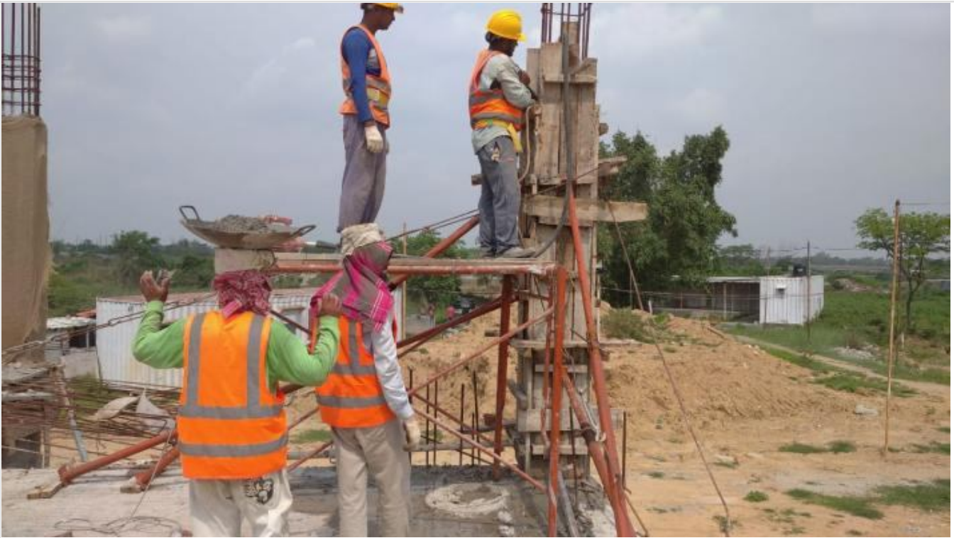
Ground Floor-Column Concreting on 30-05-21
