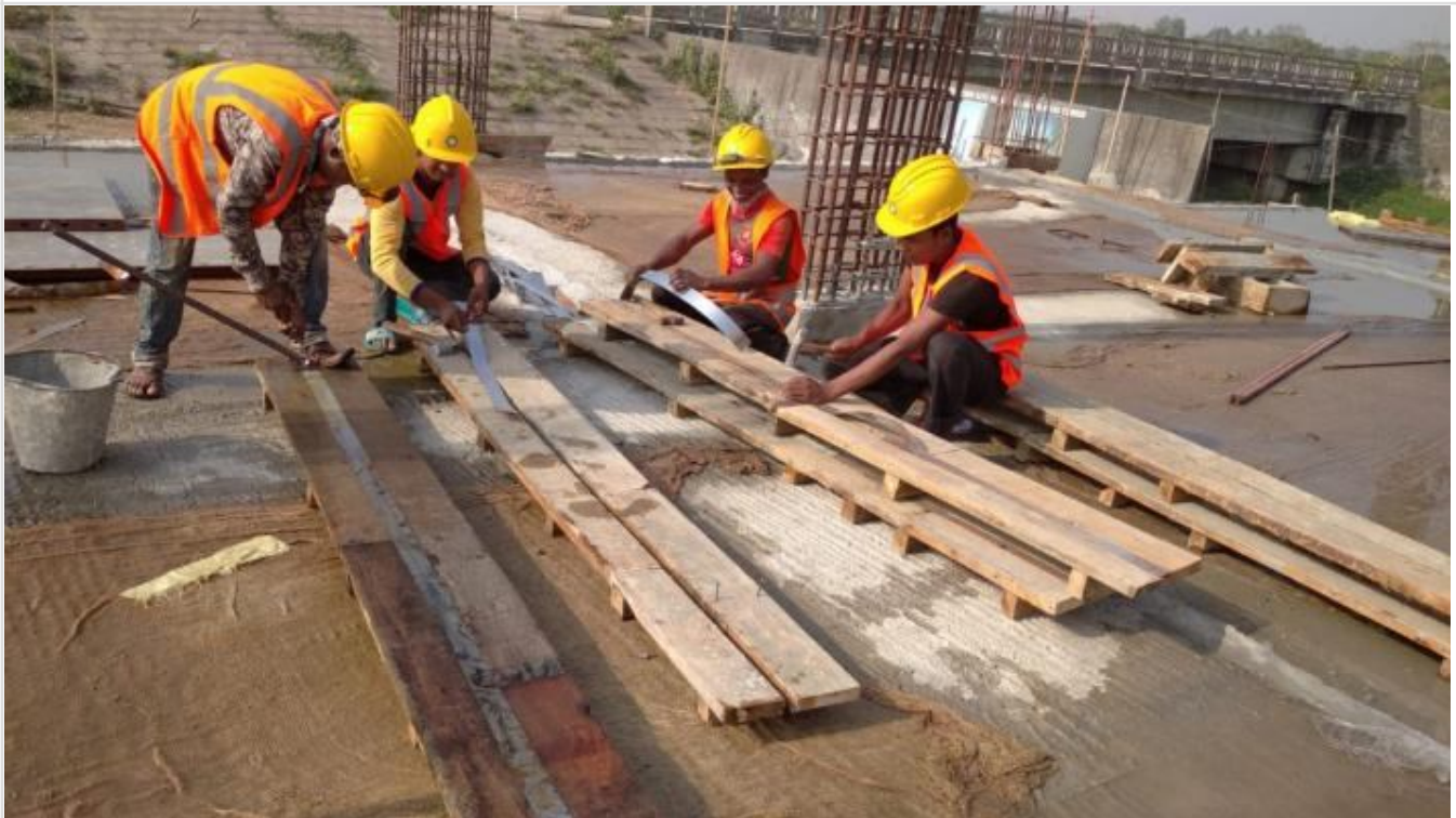
Beam Shutter Making on 01-04-21
