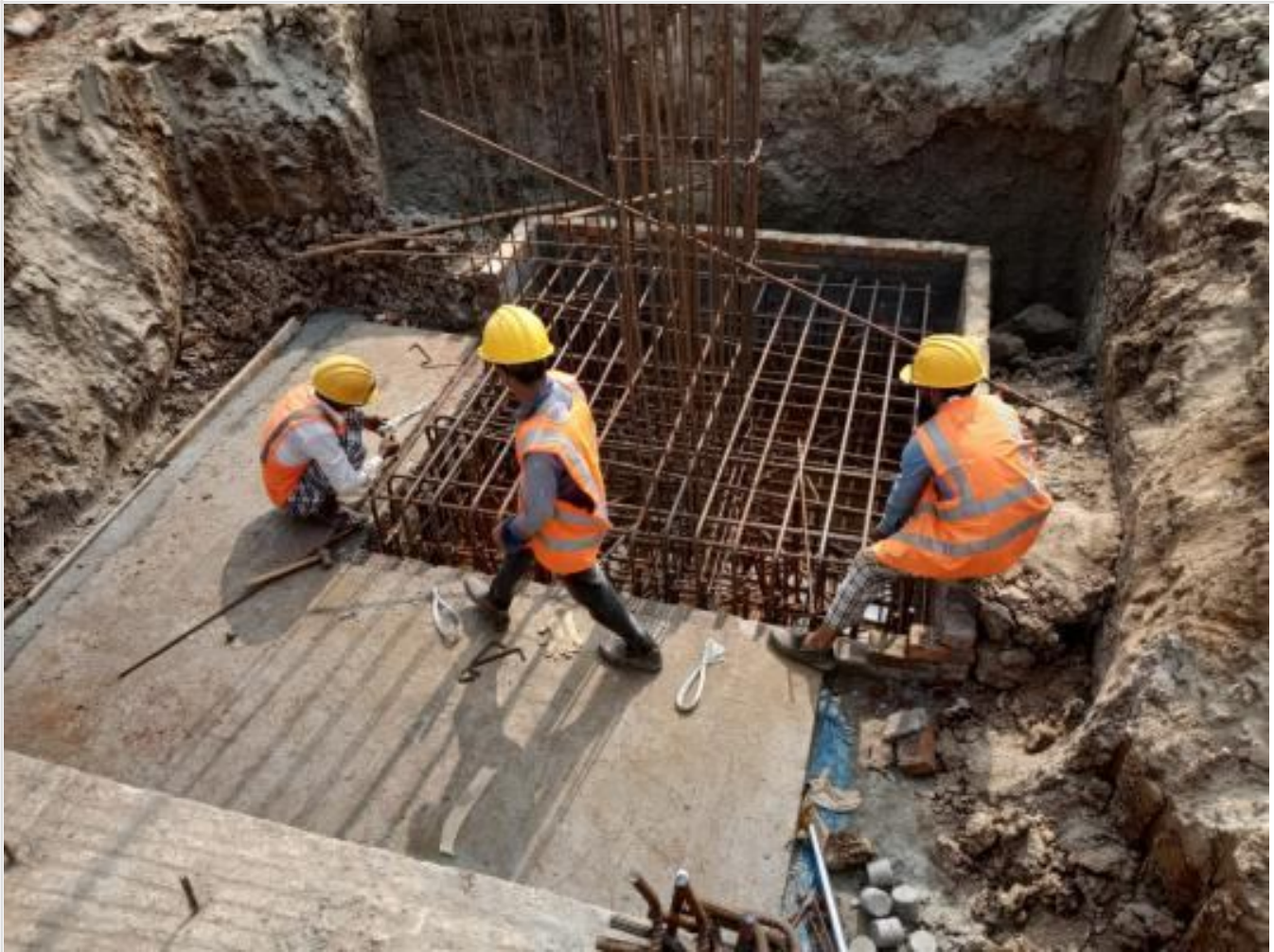
Footing Re-bar Placing on 19-12-20
