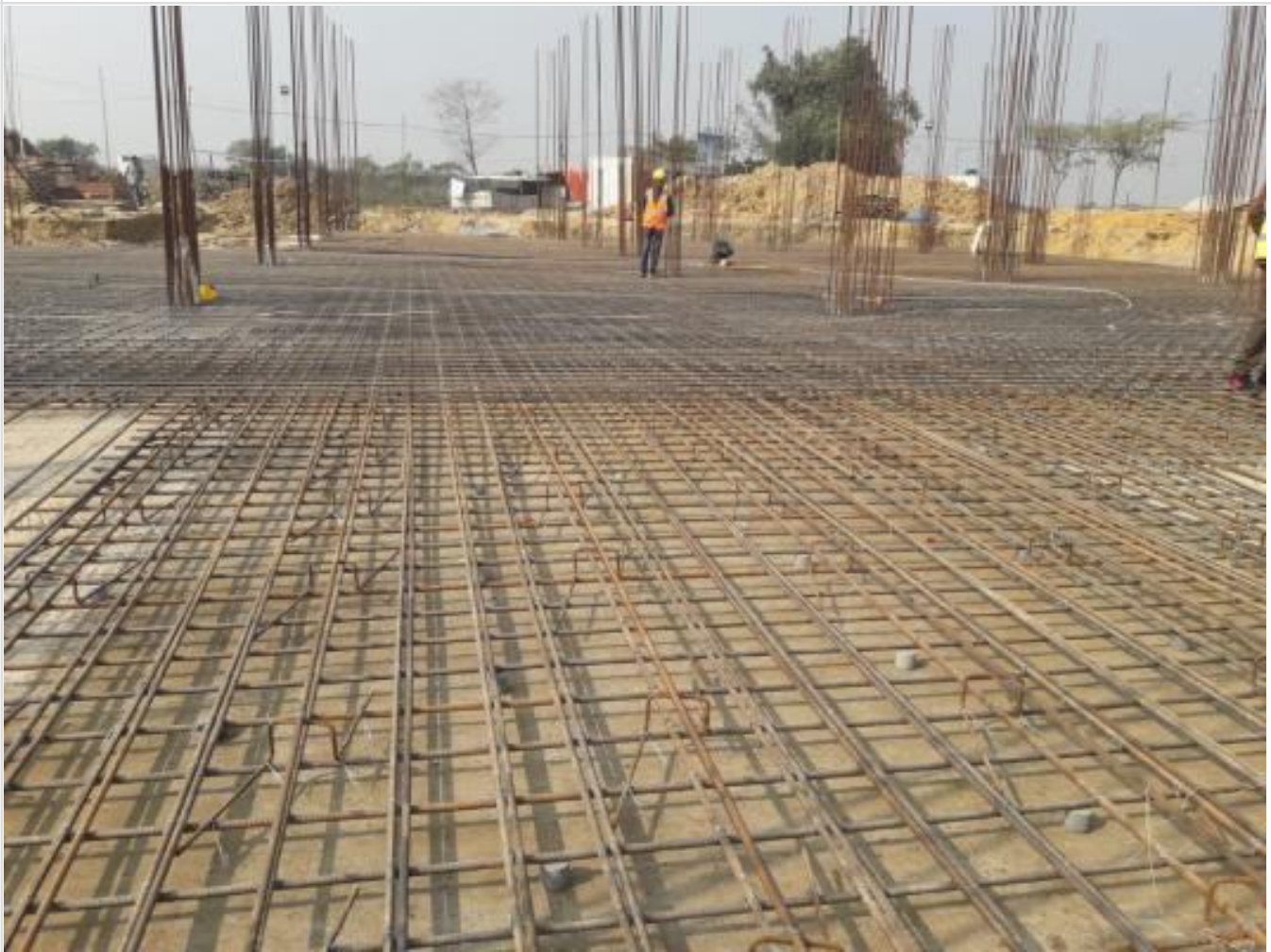
Mat Re-bar Work on 29-12-20
