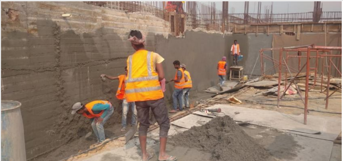
Basement West Wall Plastering on 07-03-21
