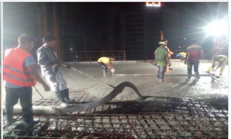
South Tower 11th Floor Slab Concreting
