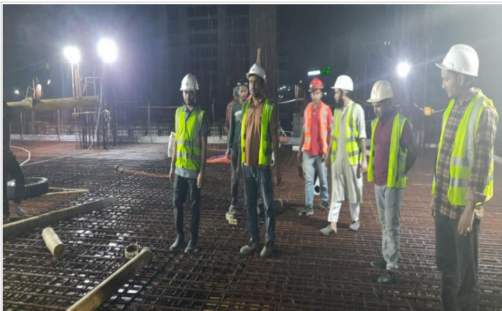
South Tower 11th Floor Slab Concreting
