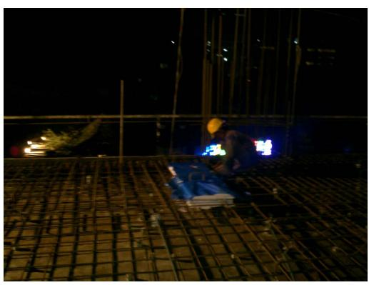
Taking Preparation (stylo -foam fixing for duct opening) for Slab Casting on 09 Dec 2011
