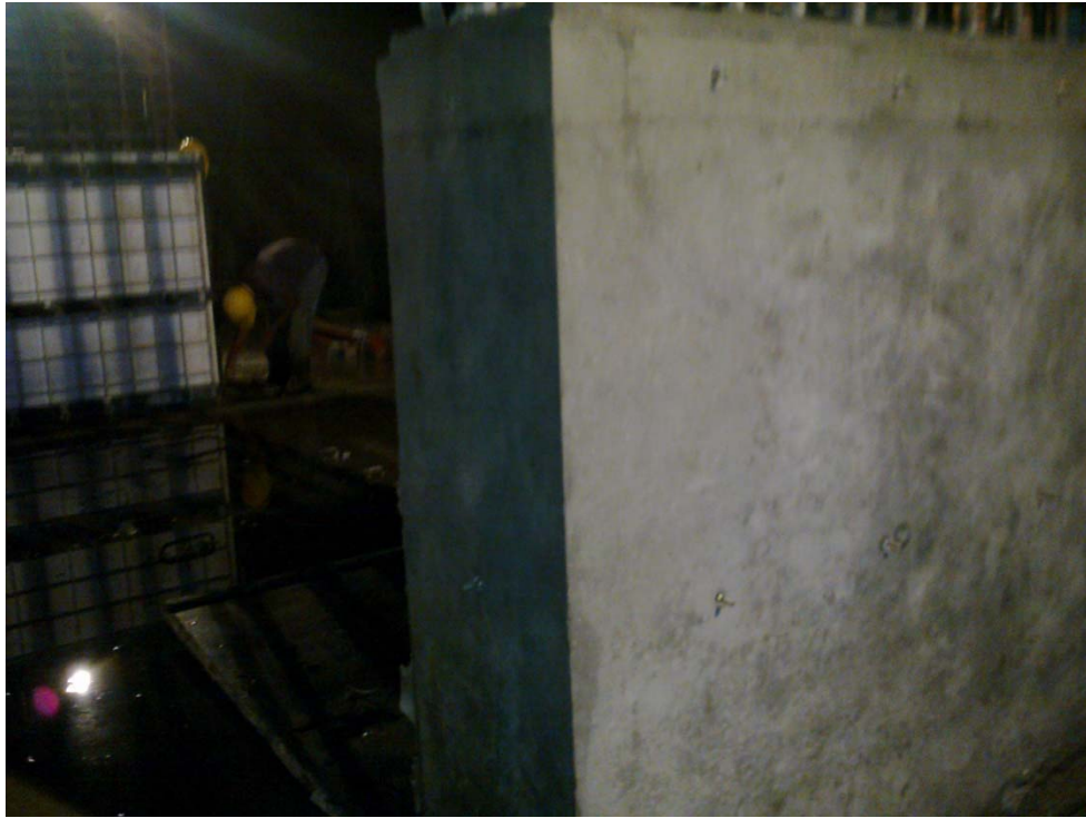
CONCRETE SURFACE AFTER SHUTTER REMOVING
