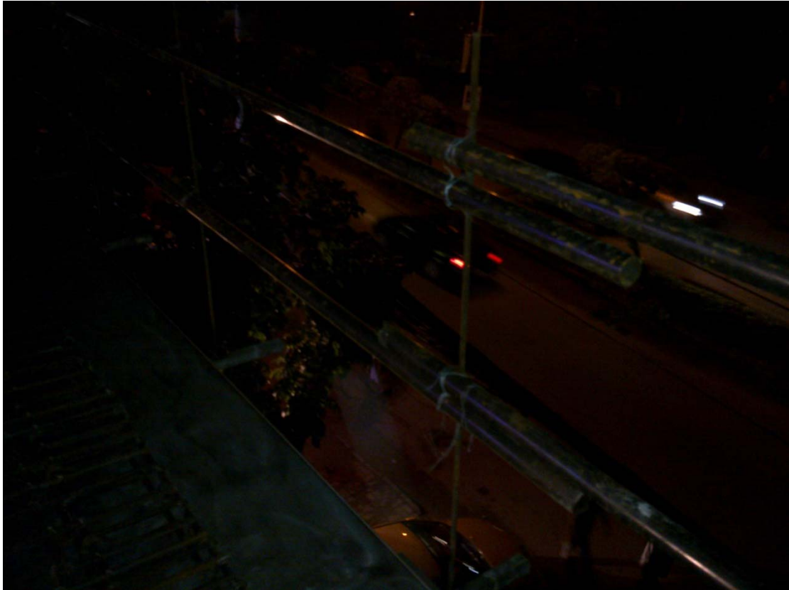
POOR ROOF EDGE PROTECTION (16mm dia vertical rod cannot bear 1.5" dia Horizontal GI Pipe )
