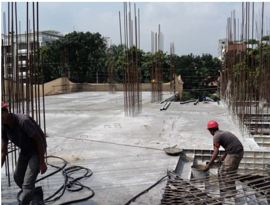
1ST FLOOR ROOF SLAB CONCRETING-FINISHING WORK
