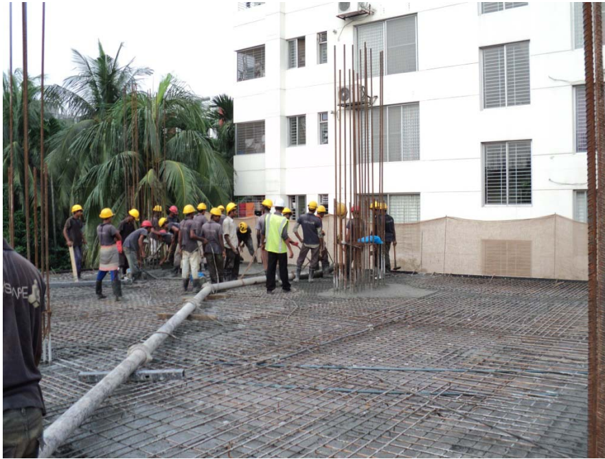
1ST FLOOR ROOF SLAB CONCRETING
